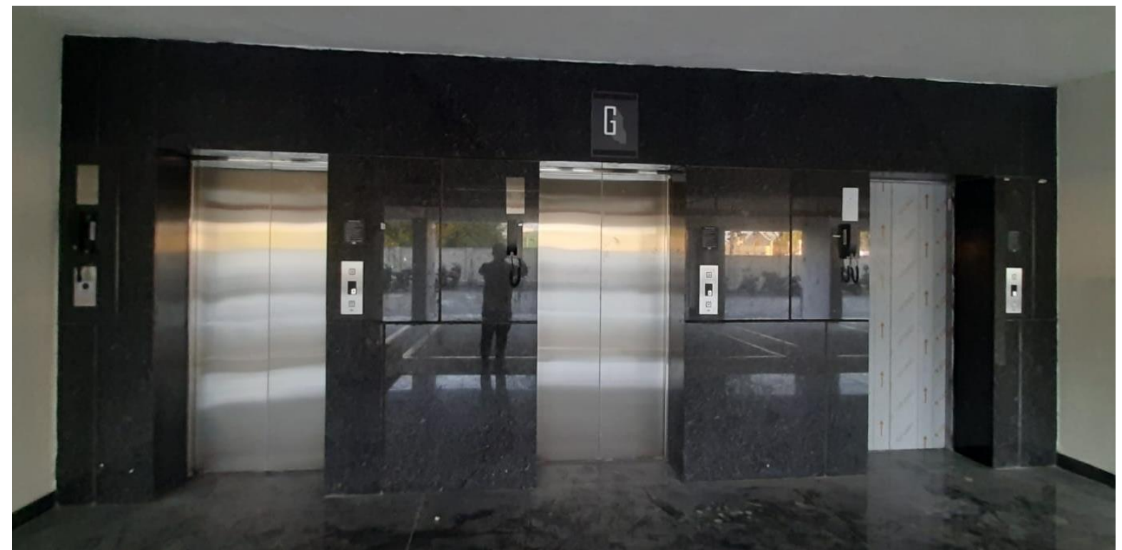
Lift Work Completed
