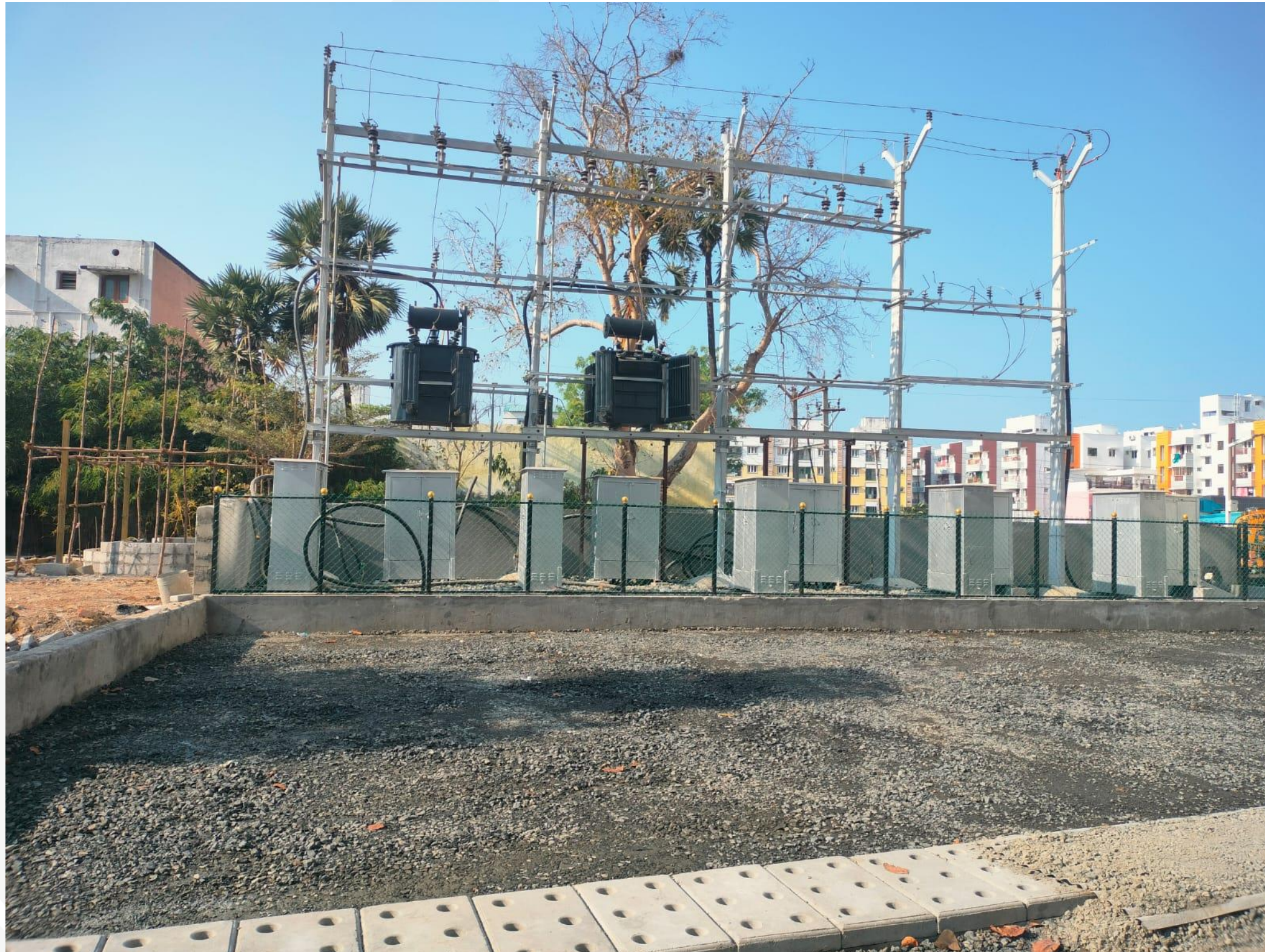
Transformer Yard Work Completed
