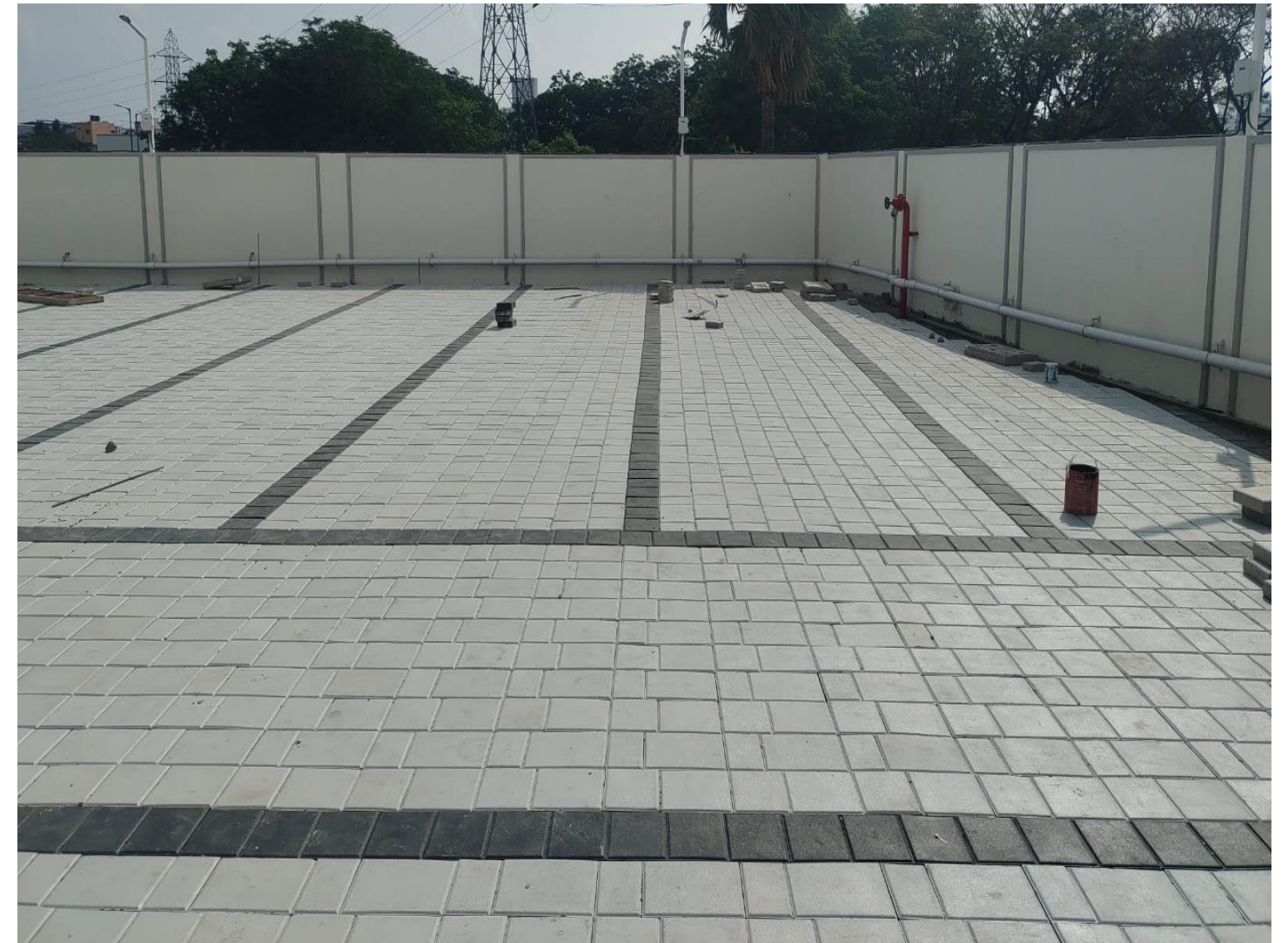
External Paver Block Laying Work In Progress
