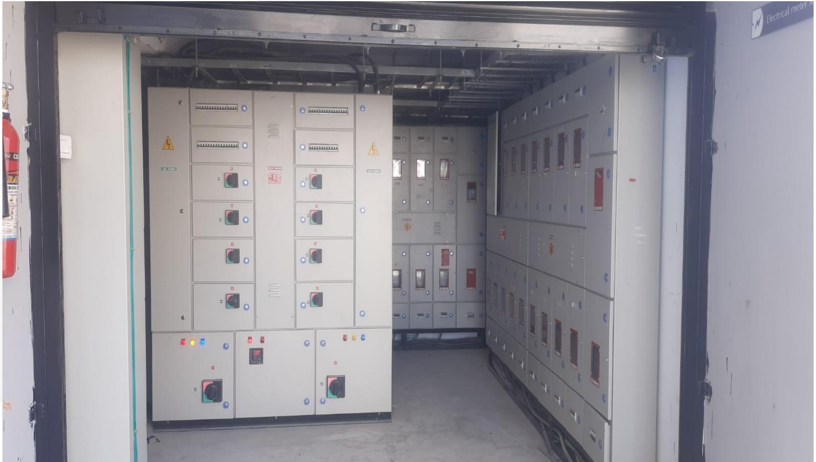
Electrical Meter Room Work Completed
