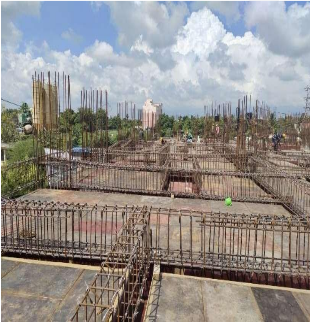
First Floor Roof Pour-2 Shuttering & Reinforcement Work In Progress
