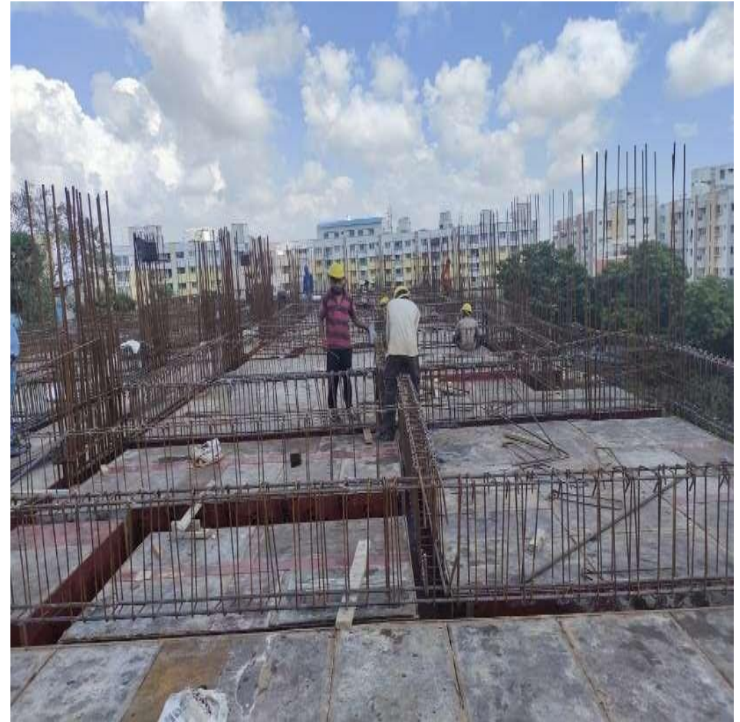
First Floor Roof Pour-2 Shuttering & Reinforcement Work In Progress
