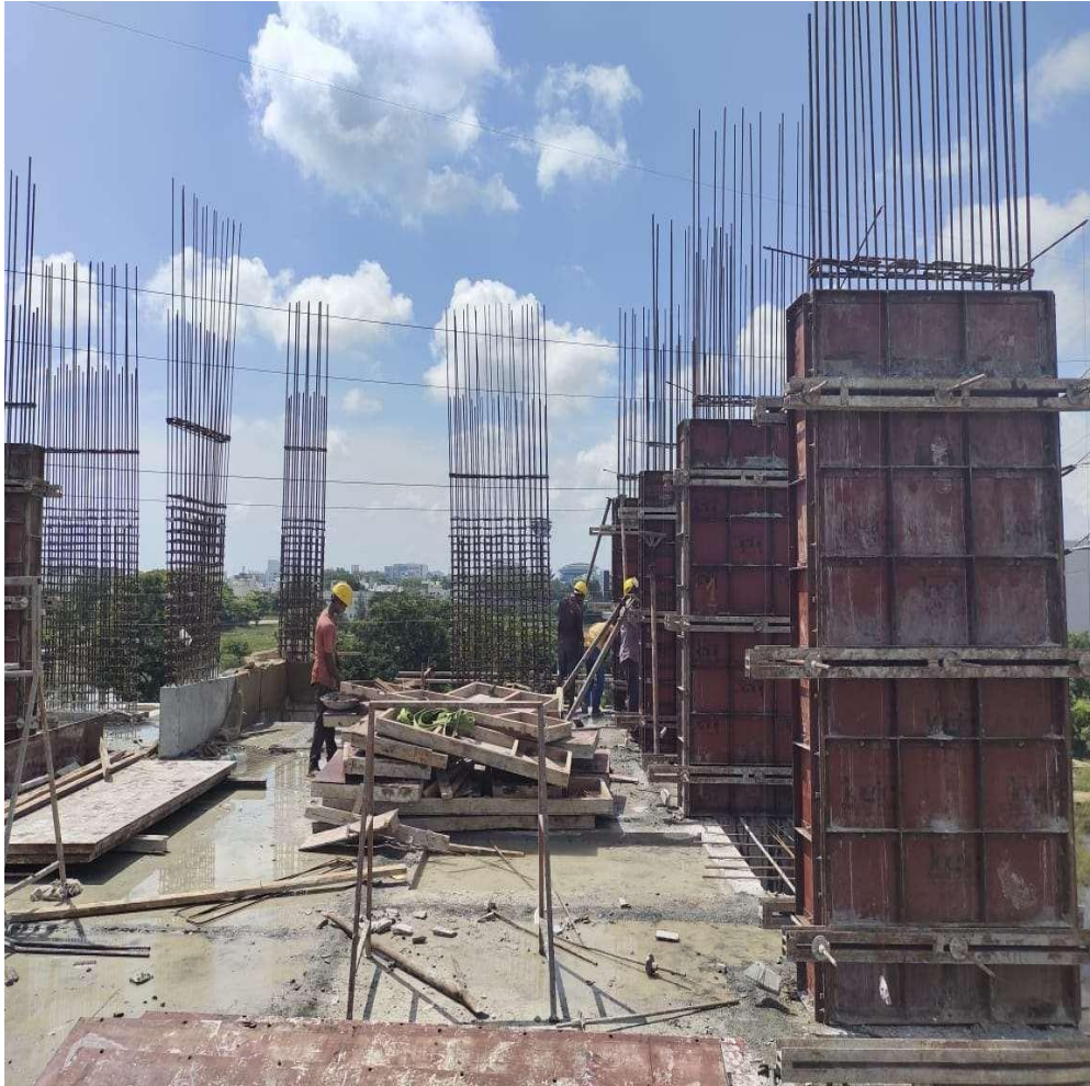
Second Floor Column Reinforcement & Shuttering work in progress
