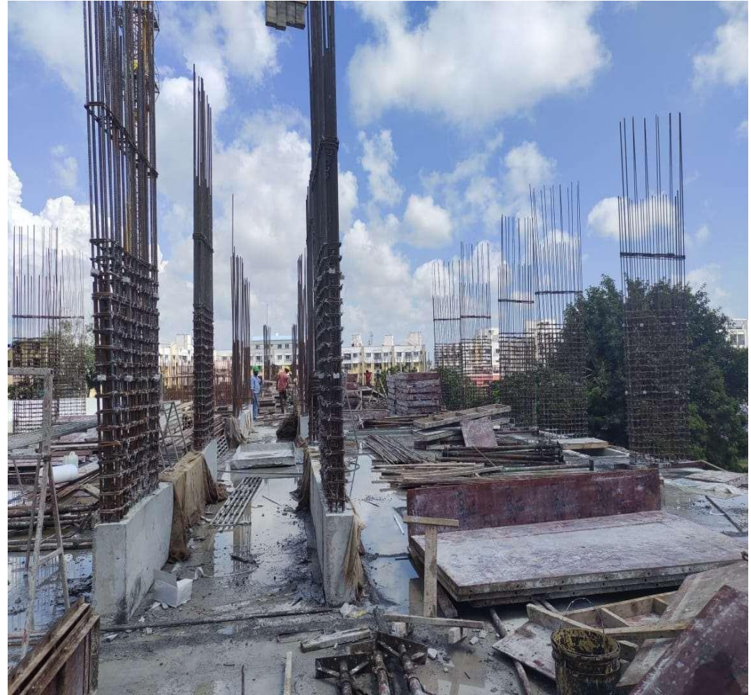
Second Floor Column Reinforcement & Shuttering work in progress
