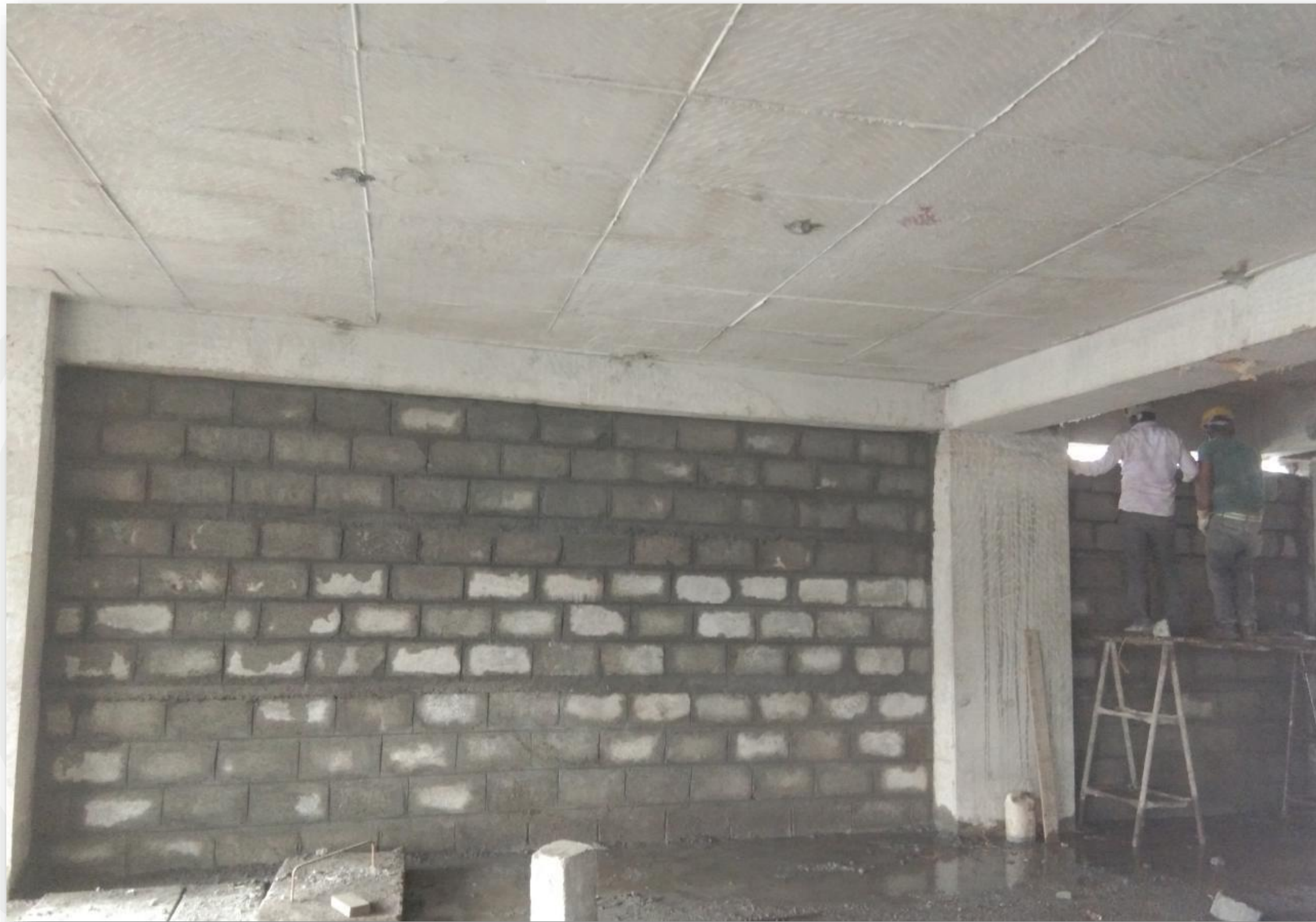
Stilt Floor Blockwork Work In Progress
