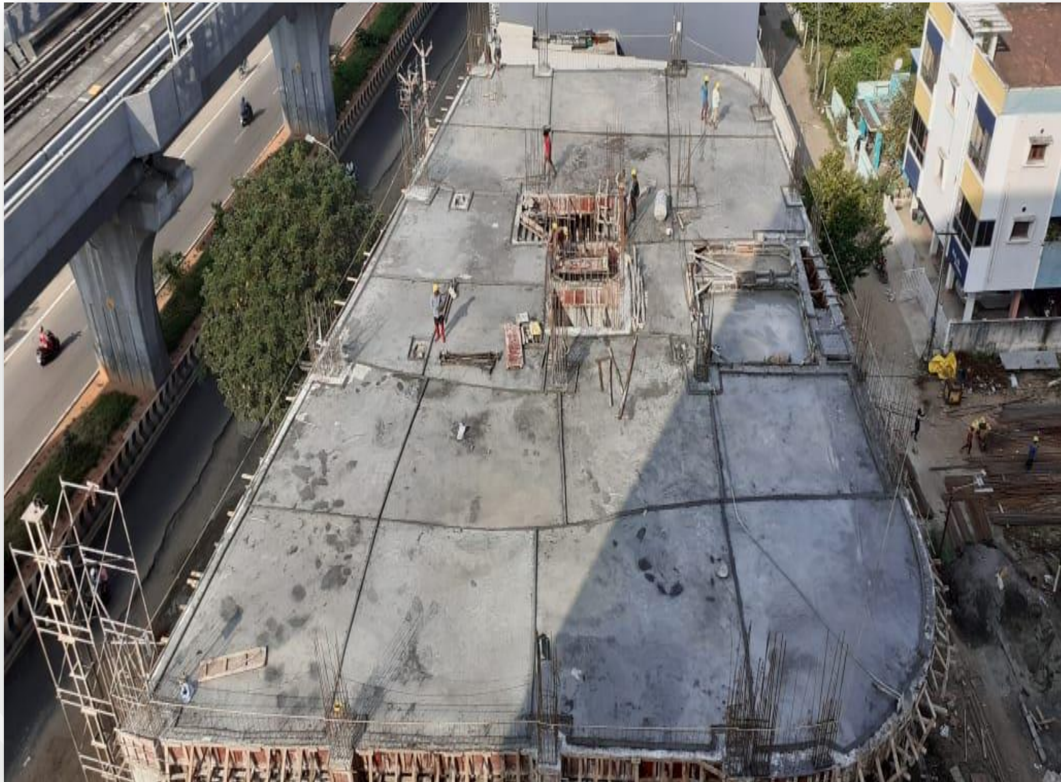
Third Floor Slab Concreting Work Completed
