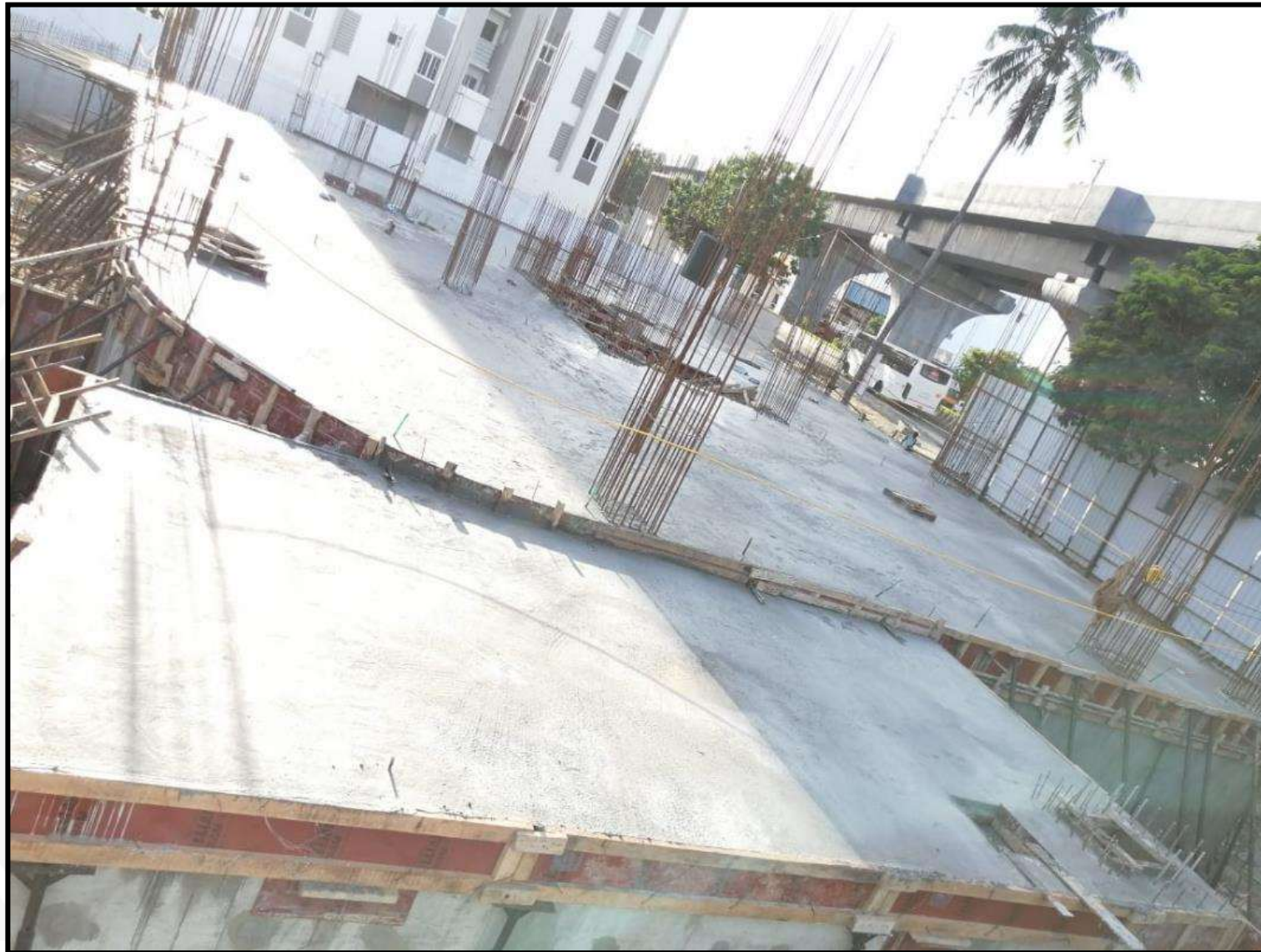
Basement Roof Slab Concreting Work Completed
