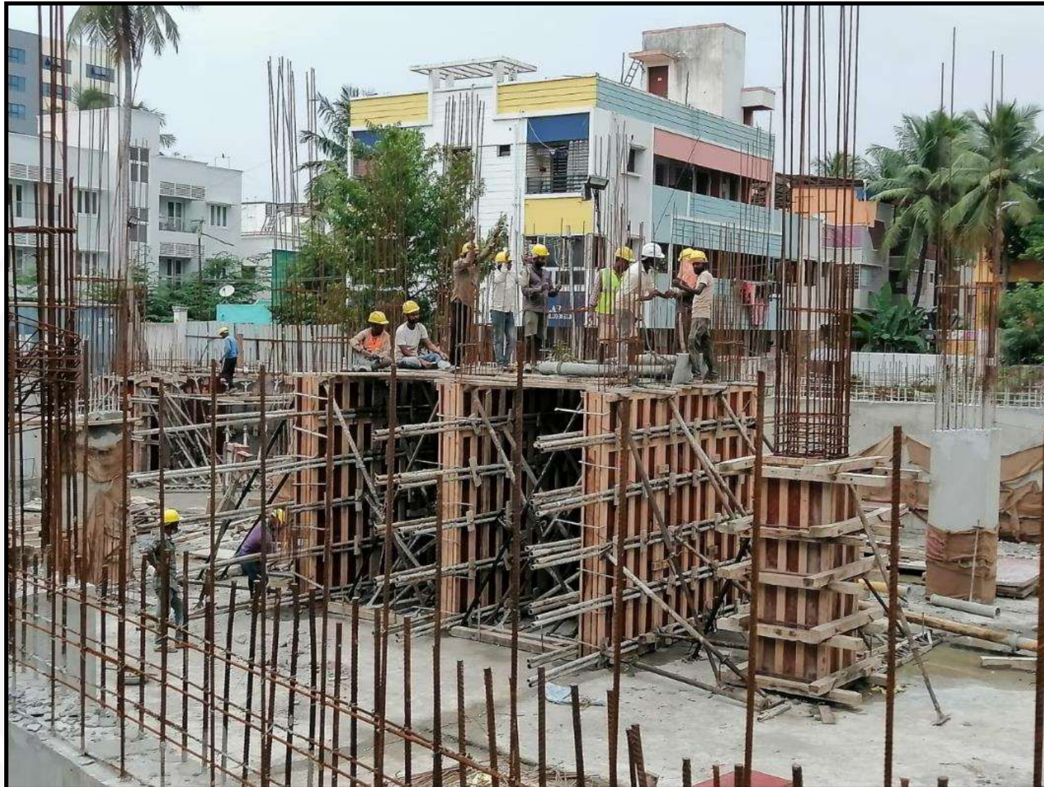
Basement Lift Wall Concreting Work Completed
