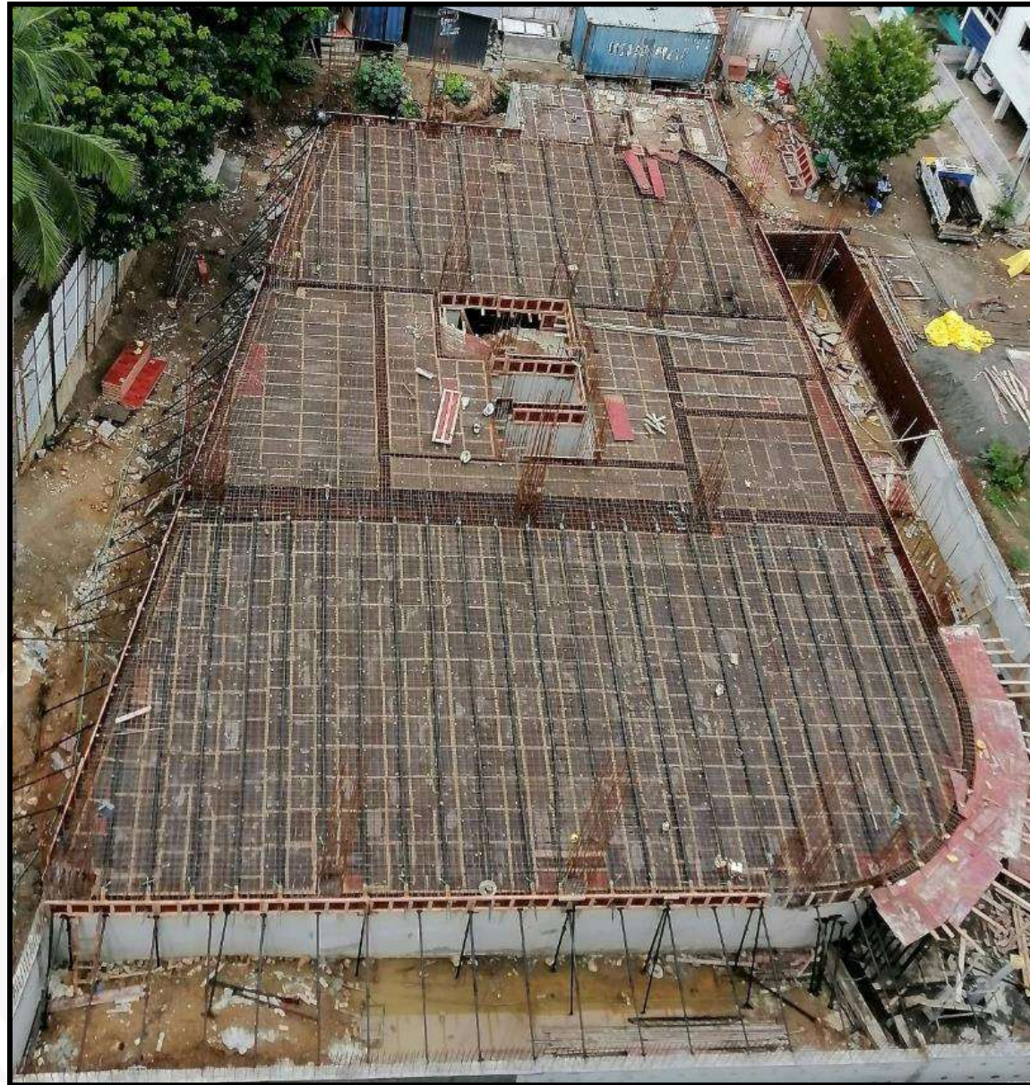
Basement Roof Slab Reinforcement Work In Progress
