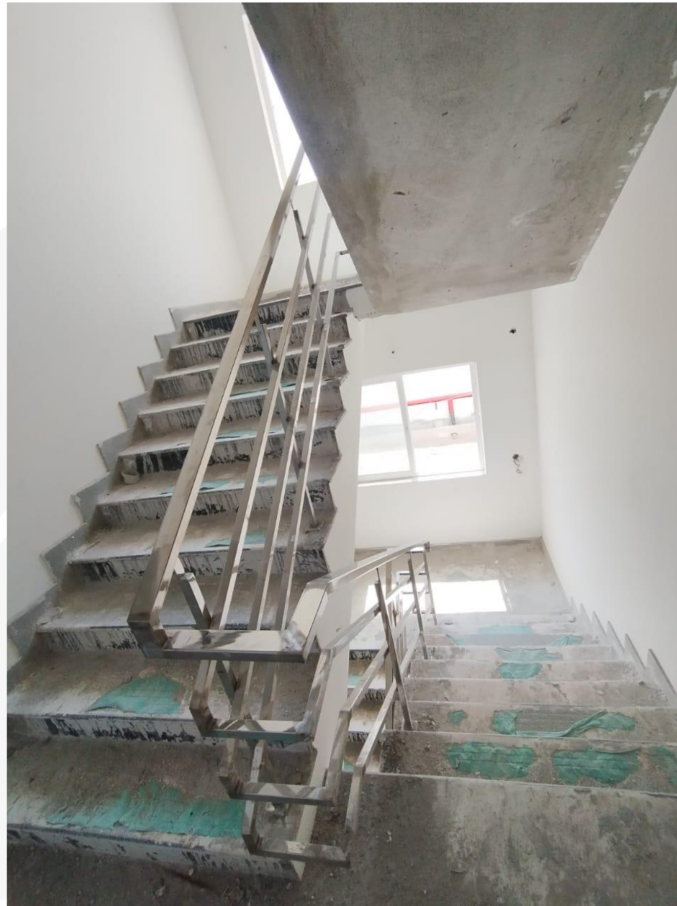
Staircase Handrail Work In Progress
