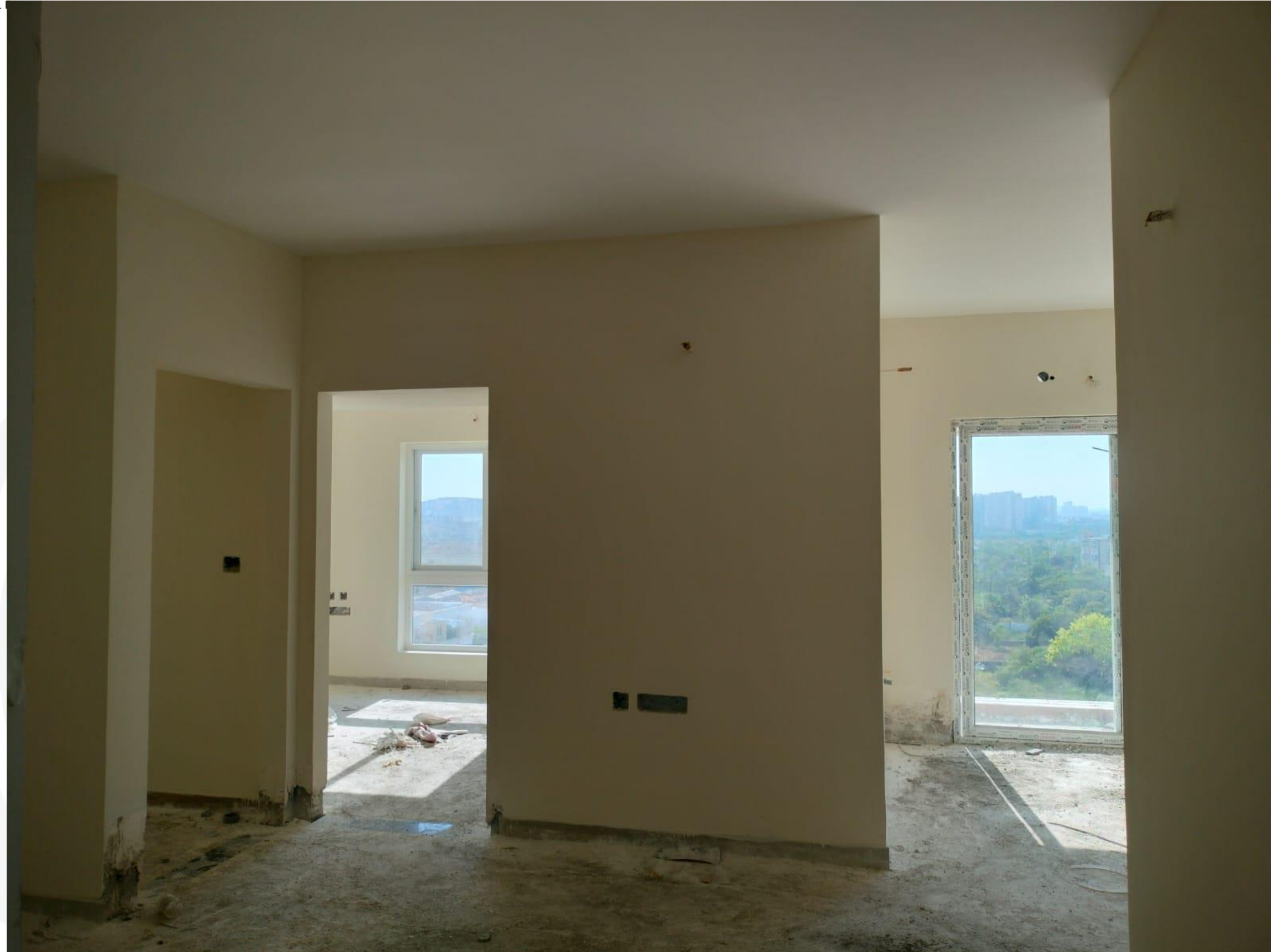
Internal Flats Painting Work In Progress
