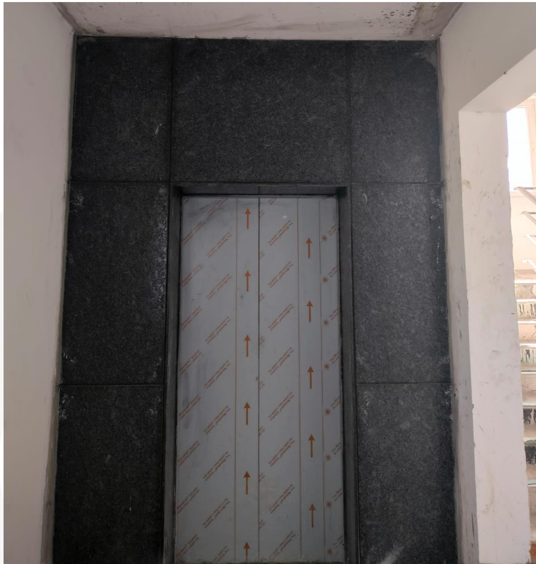
Lift Granite Gladding Work In Progress
