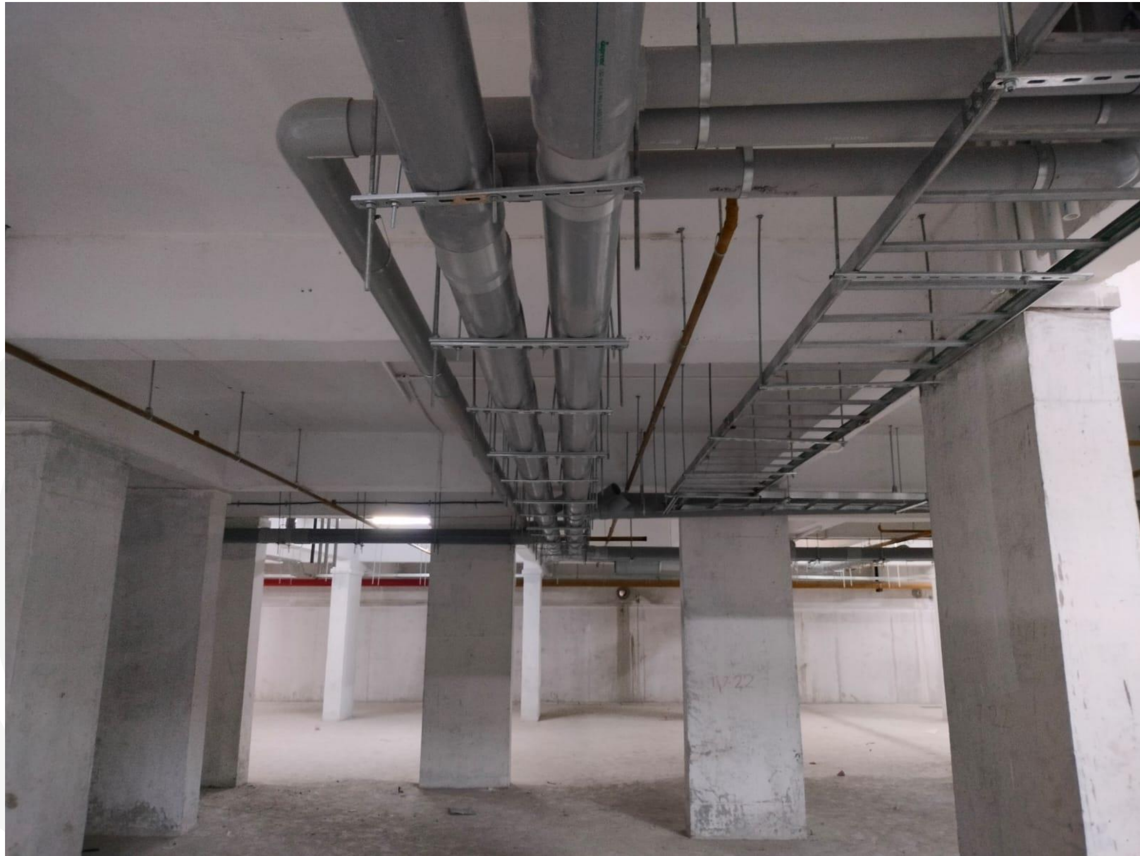
Basement Plumbing Work In Progress
