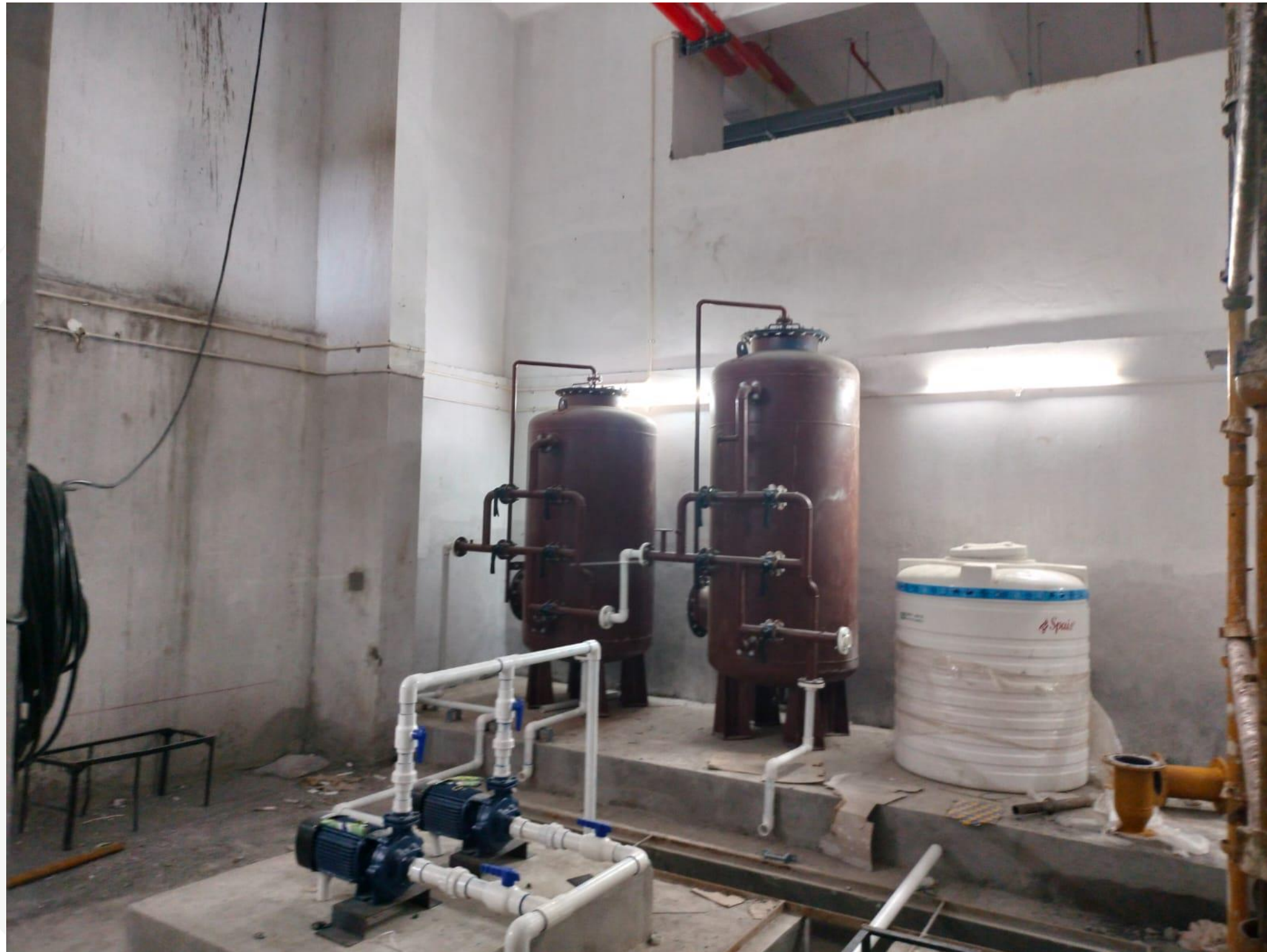
WTP Pump Room Erection Work In Progress
