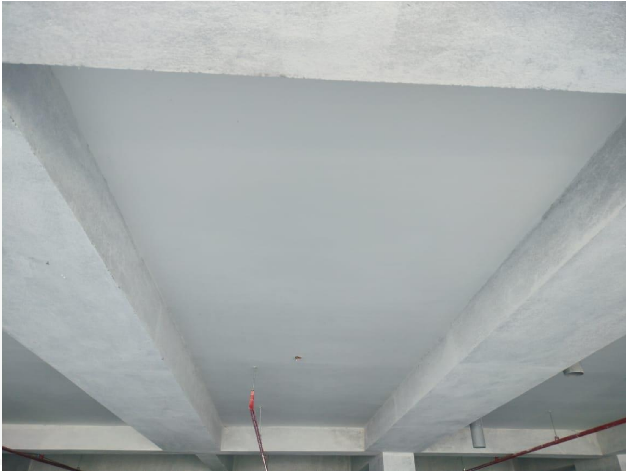
Stilt Floor Ceiling Painting Work In Progress
