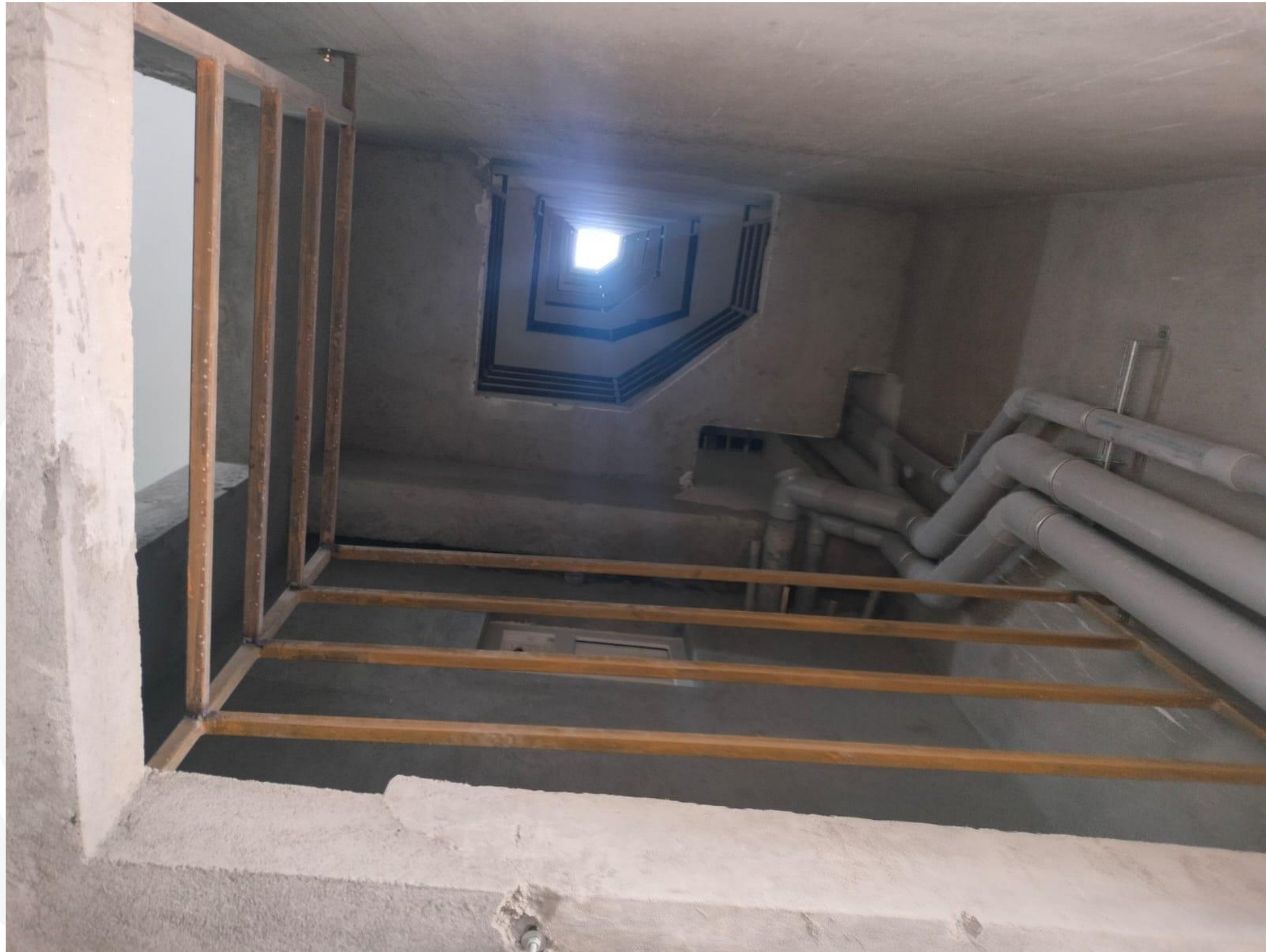
AC Service Slab Handrail Work Completed
