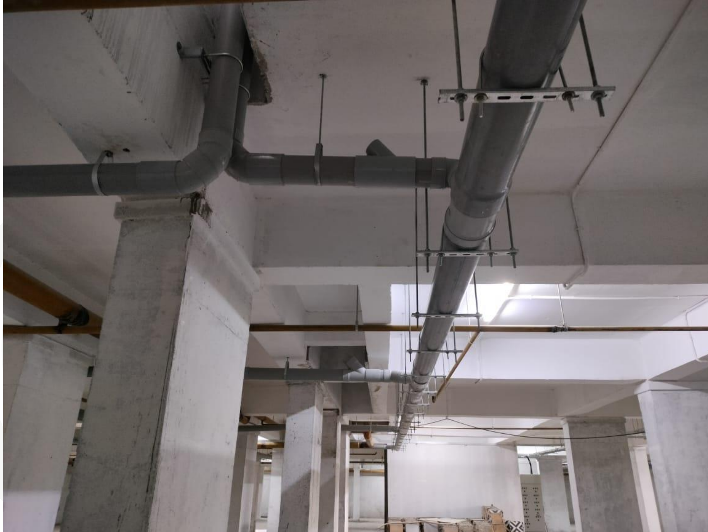
Basement Plumbing Suspended Line Work In Progress
