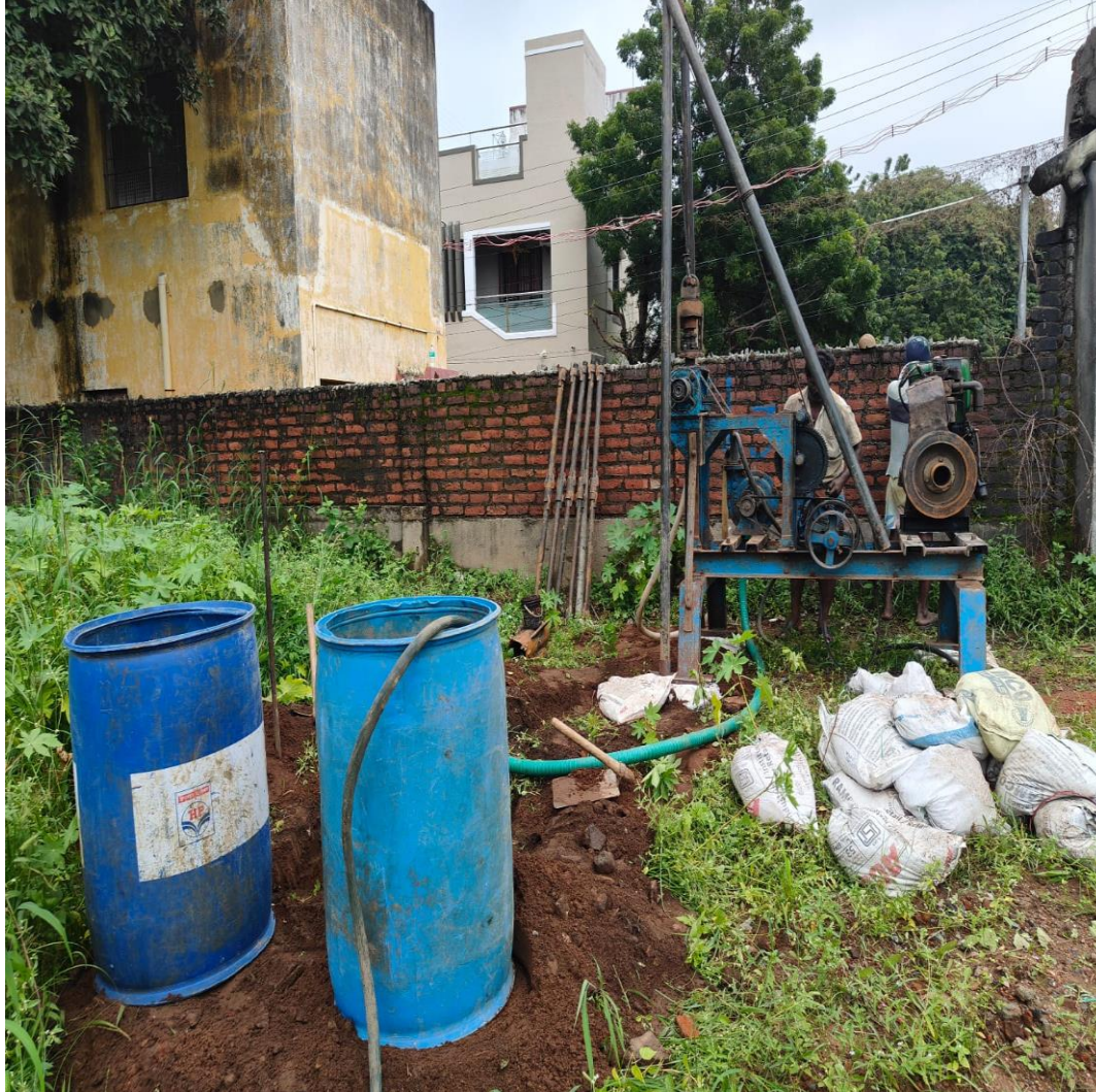
Bore well work completed(260 Ft)
