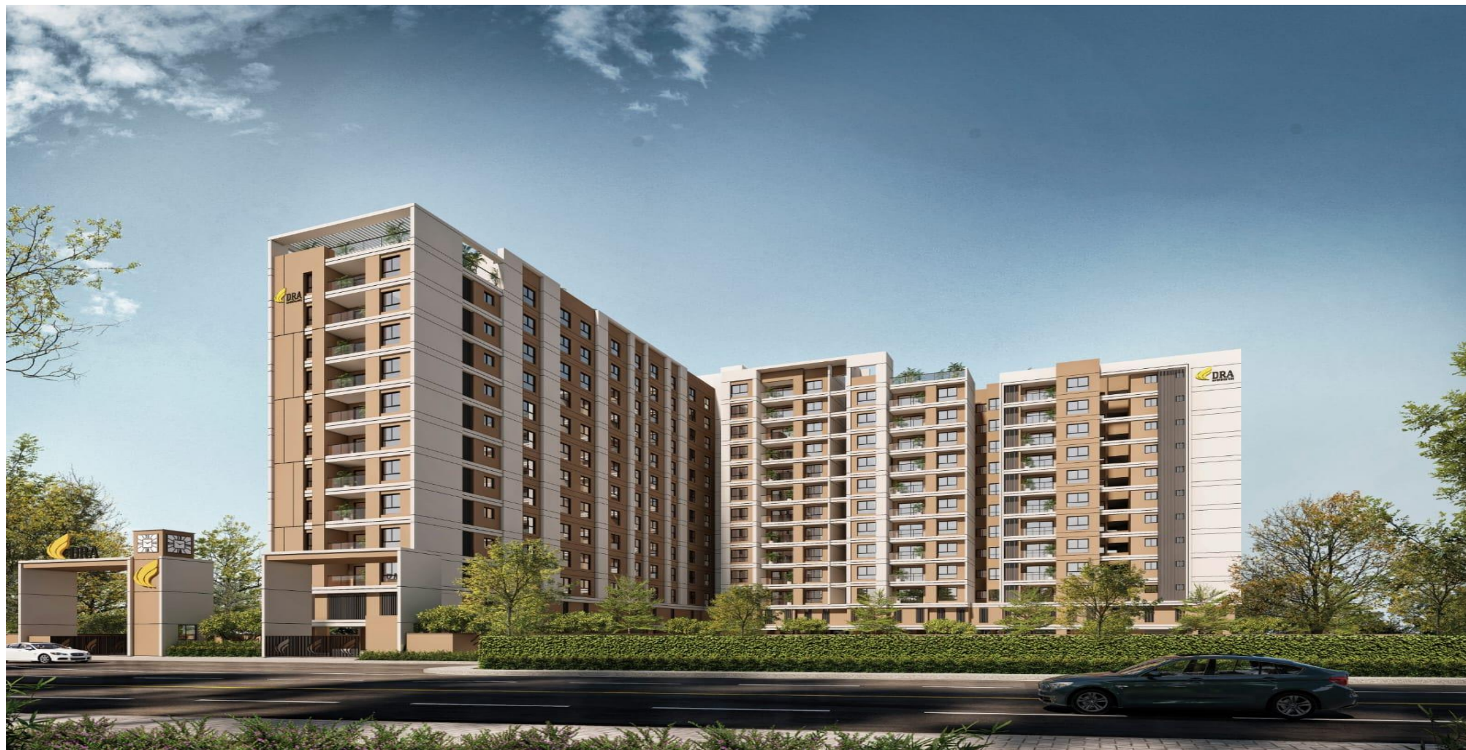
DRA ASTRA Construction update photos – December 2024
