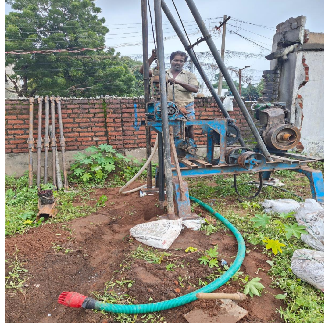
Bore well work completed(260 Ft)
