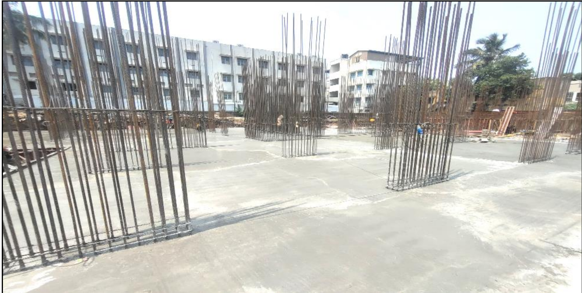
Main building – Pour 4 Raft concrete work completed (573cum).
