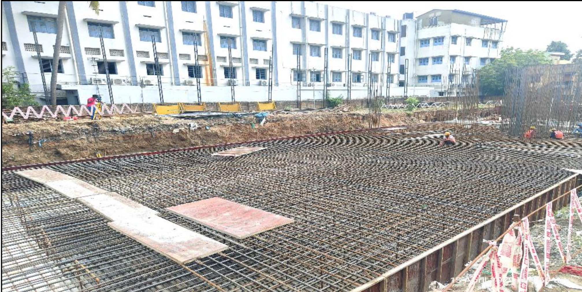
Main building – Pour 4 Raft shuttering work completed.
