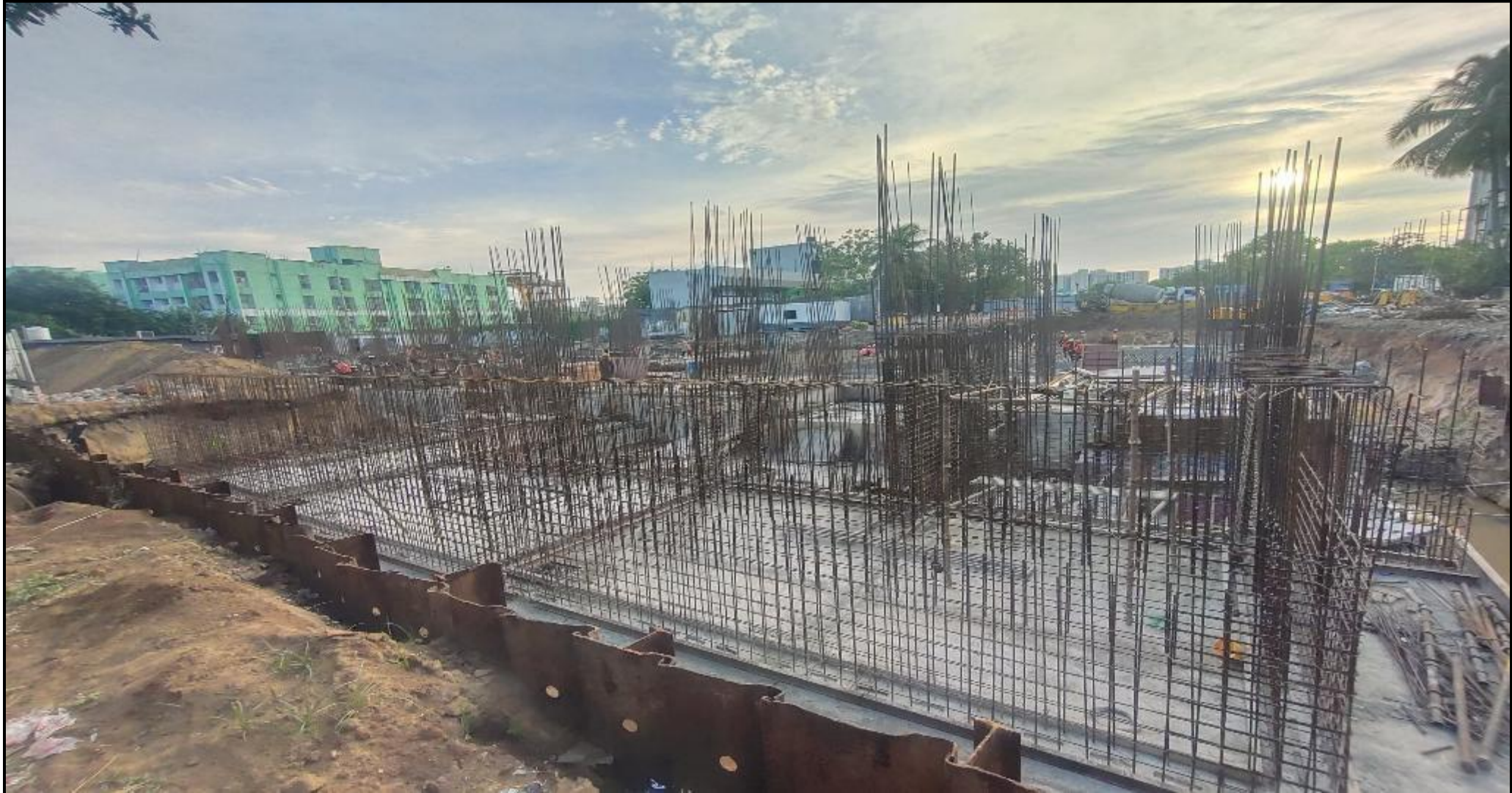
UG Sump wall reinforcement work completed.
