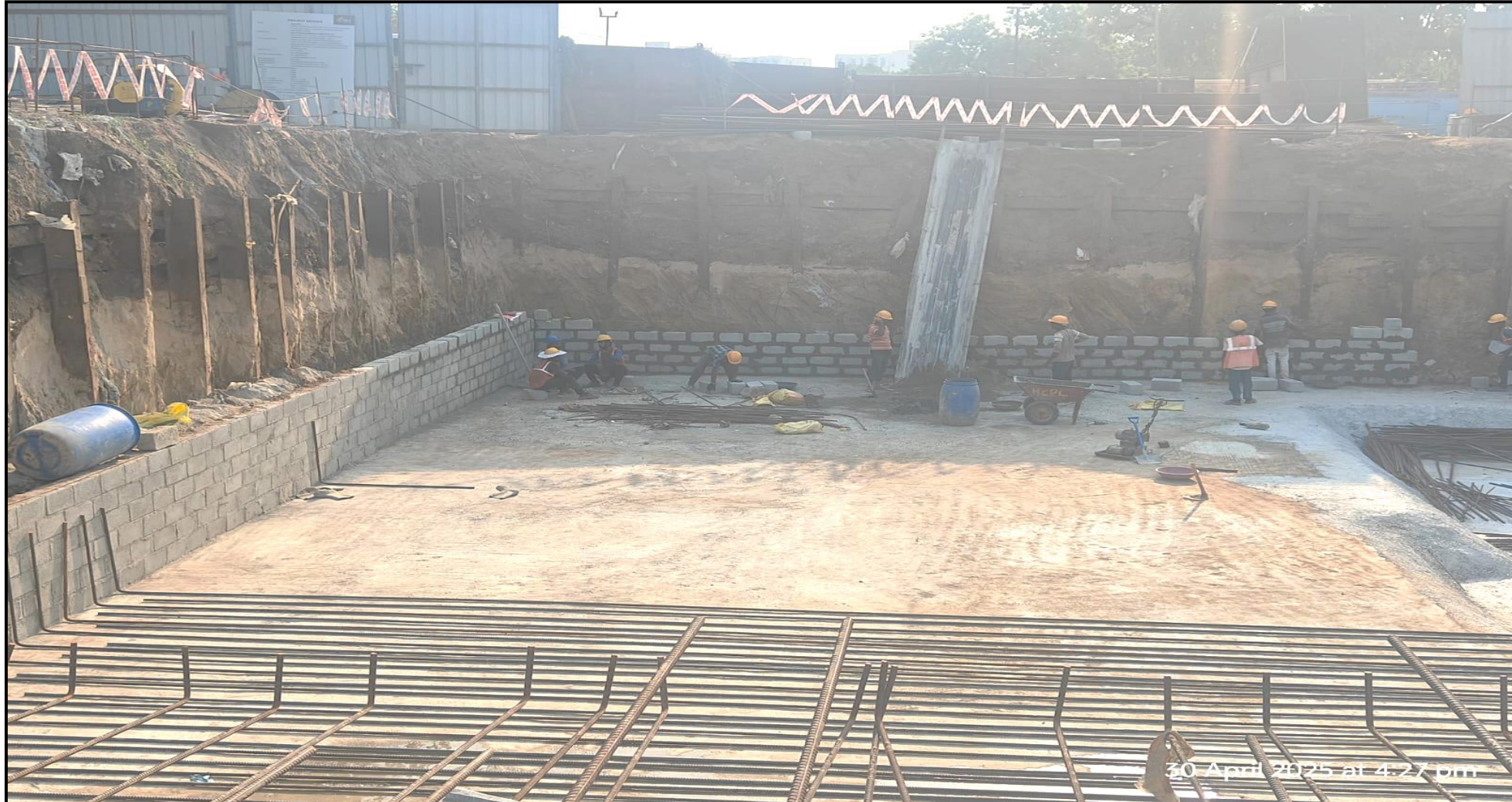
STP – Raft shuttering block work in progress
