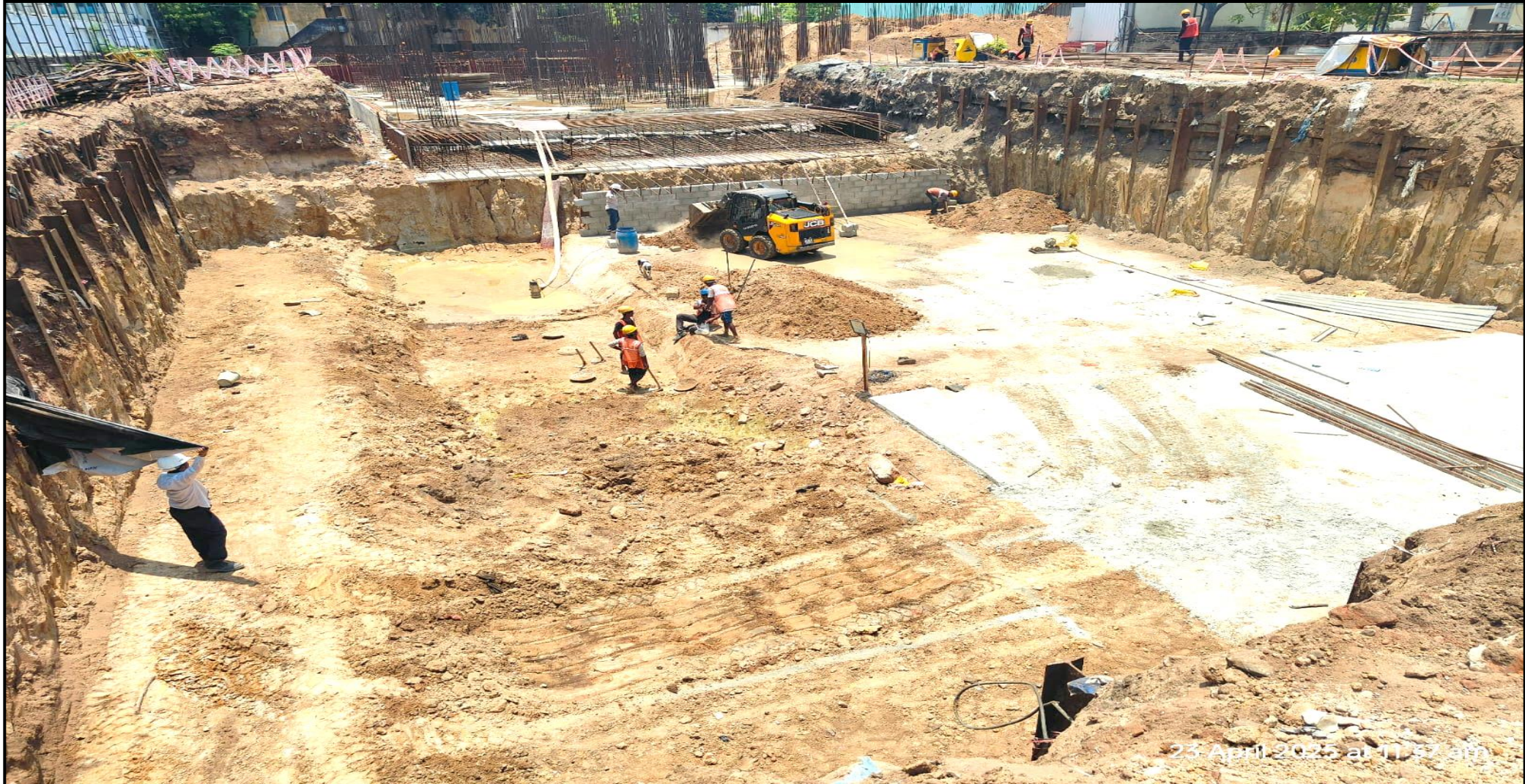
STP – Surface dressing for PCC completed
