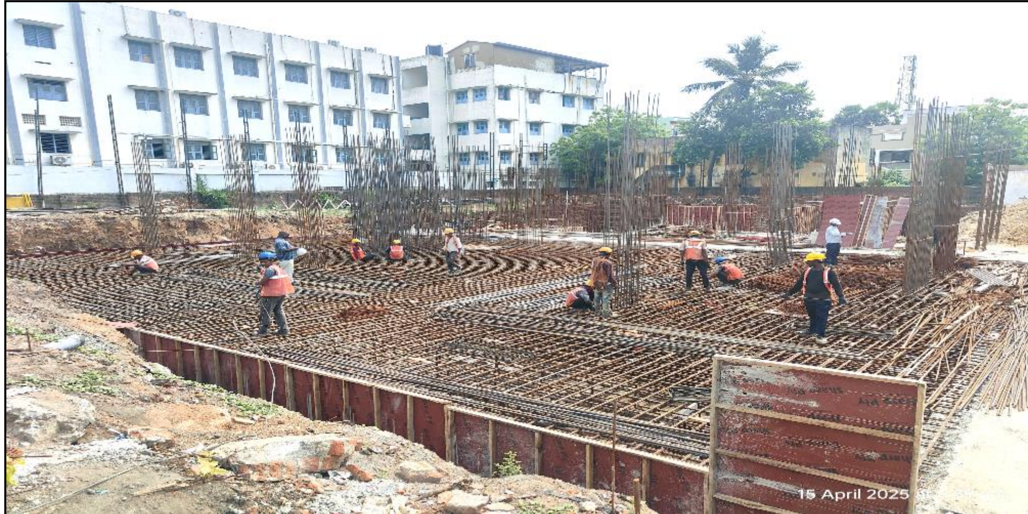
Main building – Pour 4 Raft reinforcement work completed
