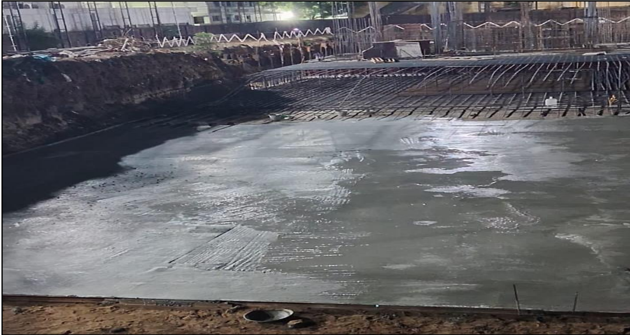
Main building – Pour 4 Raft PCC completed.
