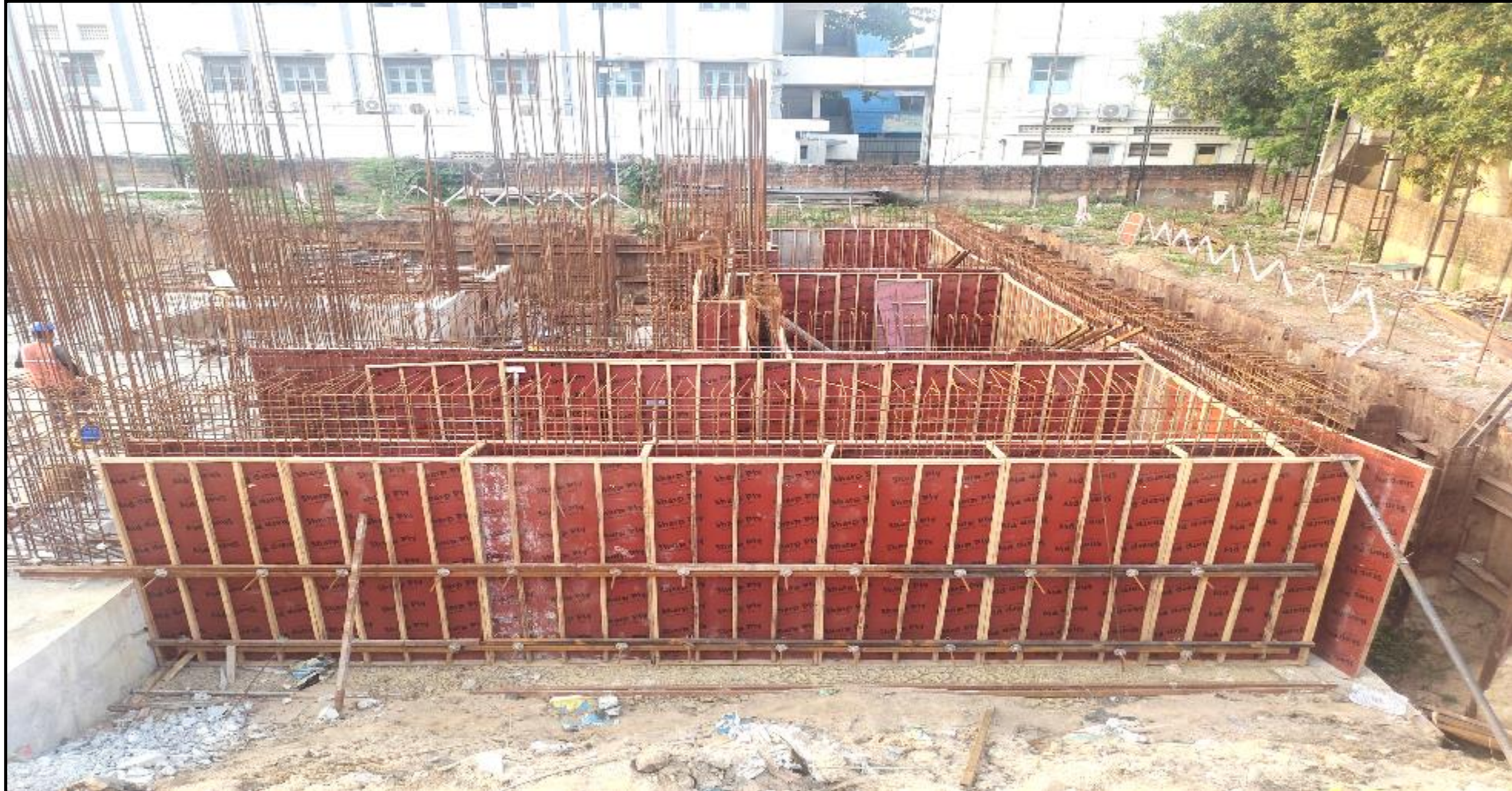
UG Sump – 1 st Lift wall shuttering work completed
