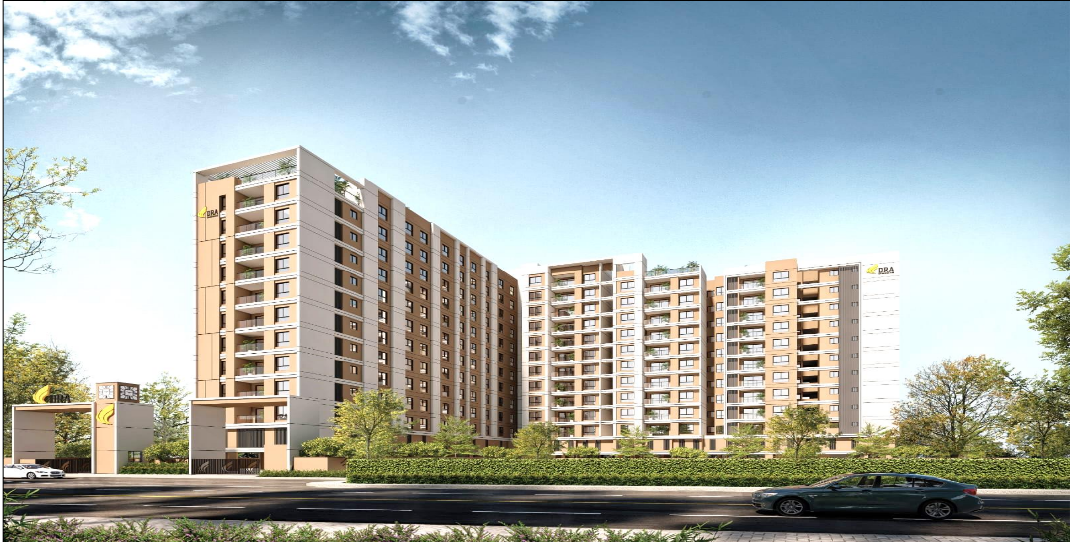
DRA ASTRA Construction update photos – February 2025
