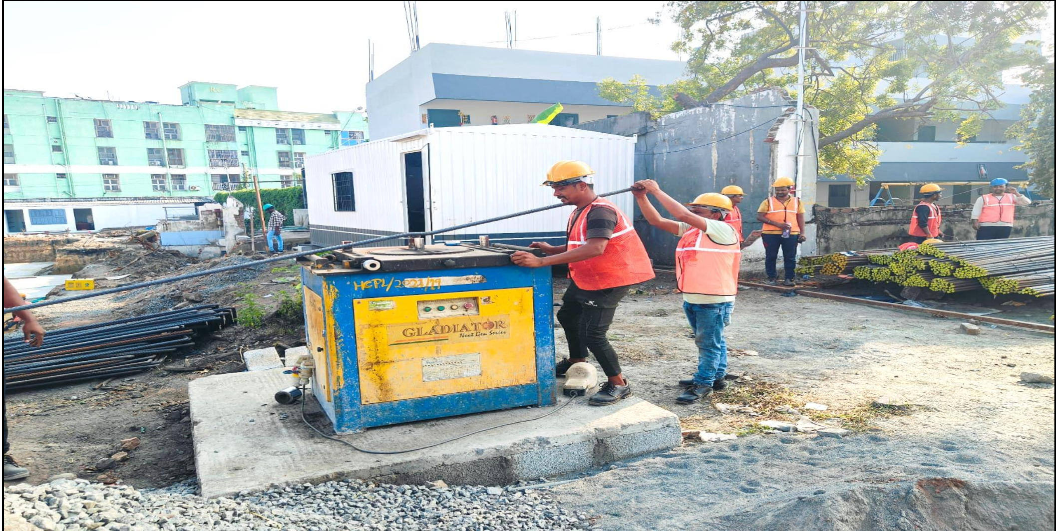
Steel cutting & bending work in progress for raft foundation work
