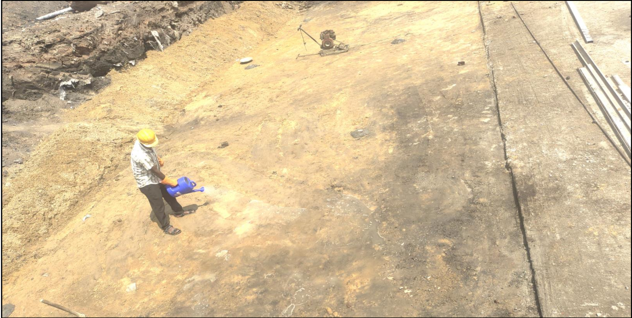
Main building – ATT work in progress (1689/2659 sqm)
