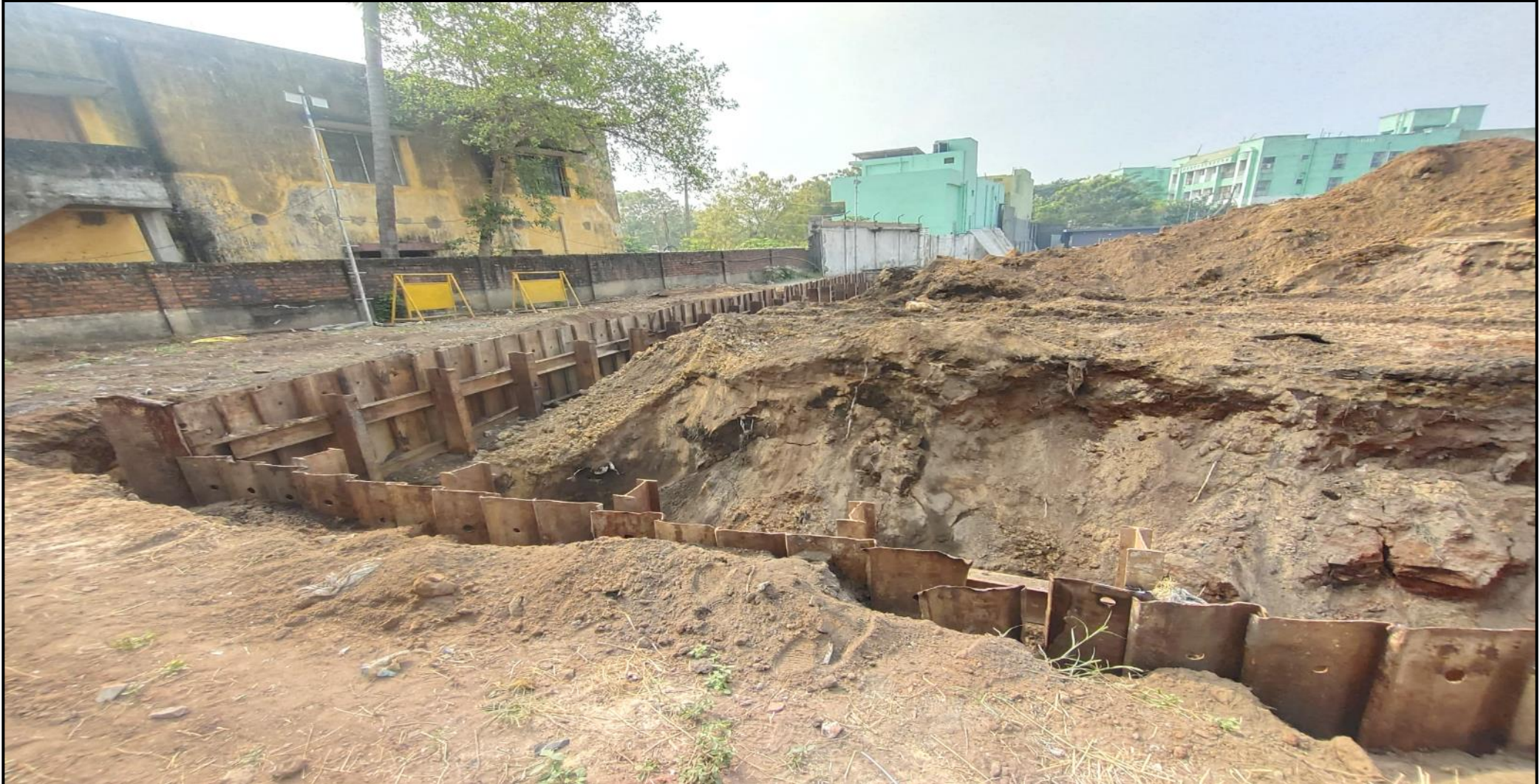
UG Sump shoring work completed (41.6/41.6m completed)
