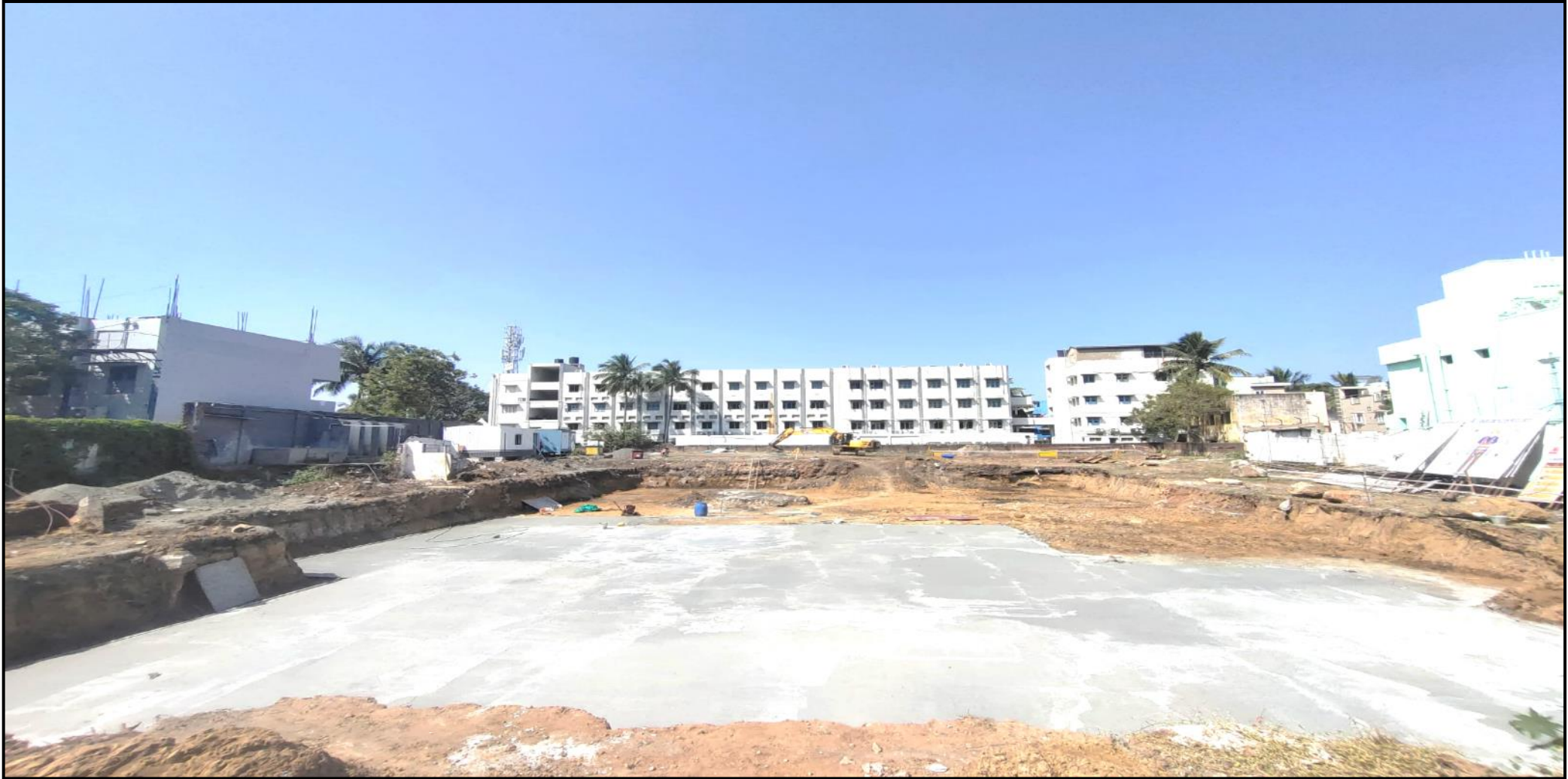
Main building – Raft PCC work in progress (81/123 cum completed)
