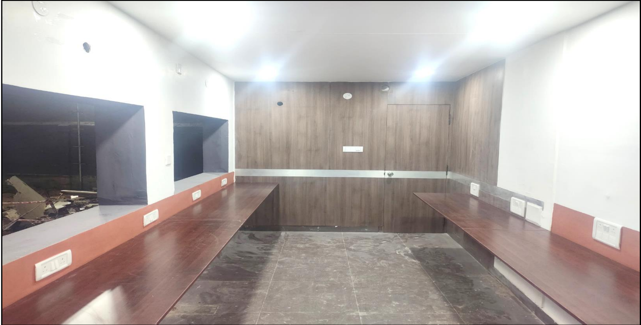
Site office renovation work completed
