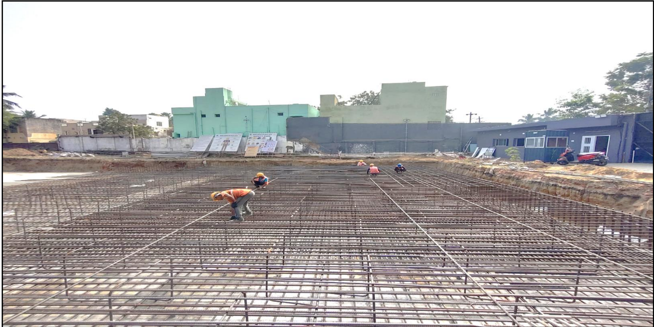
Main building – Raft reinforcement work in progress
