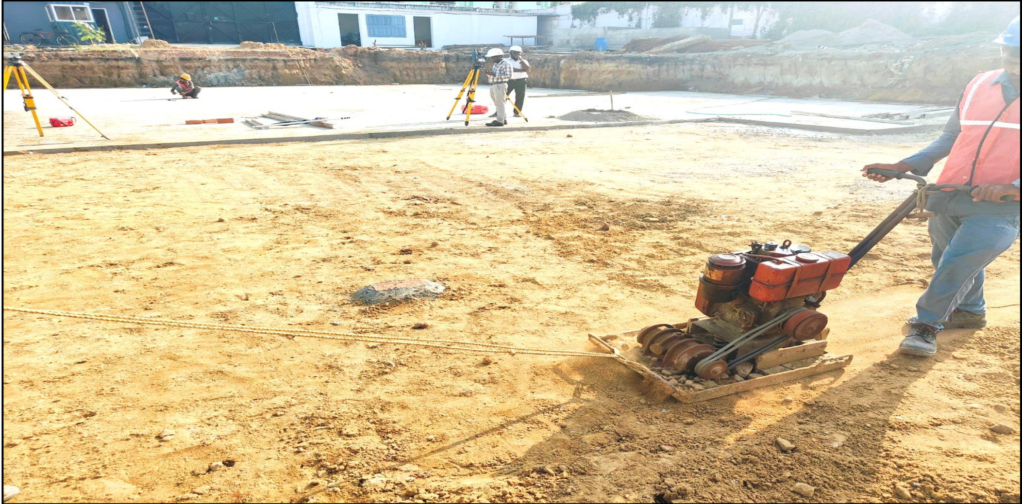
Main building – Base preparation work for raft PCC
