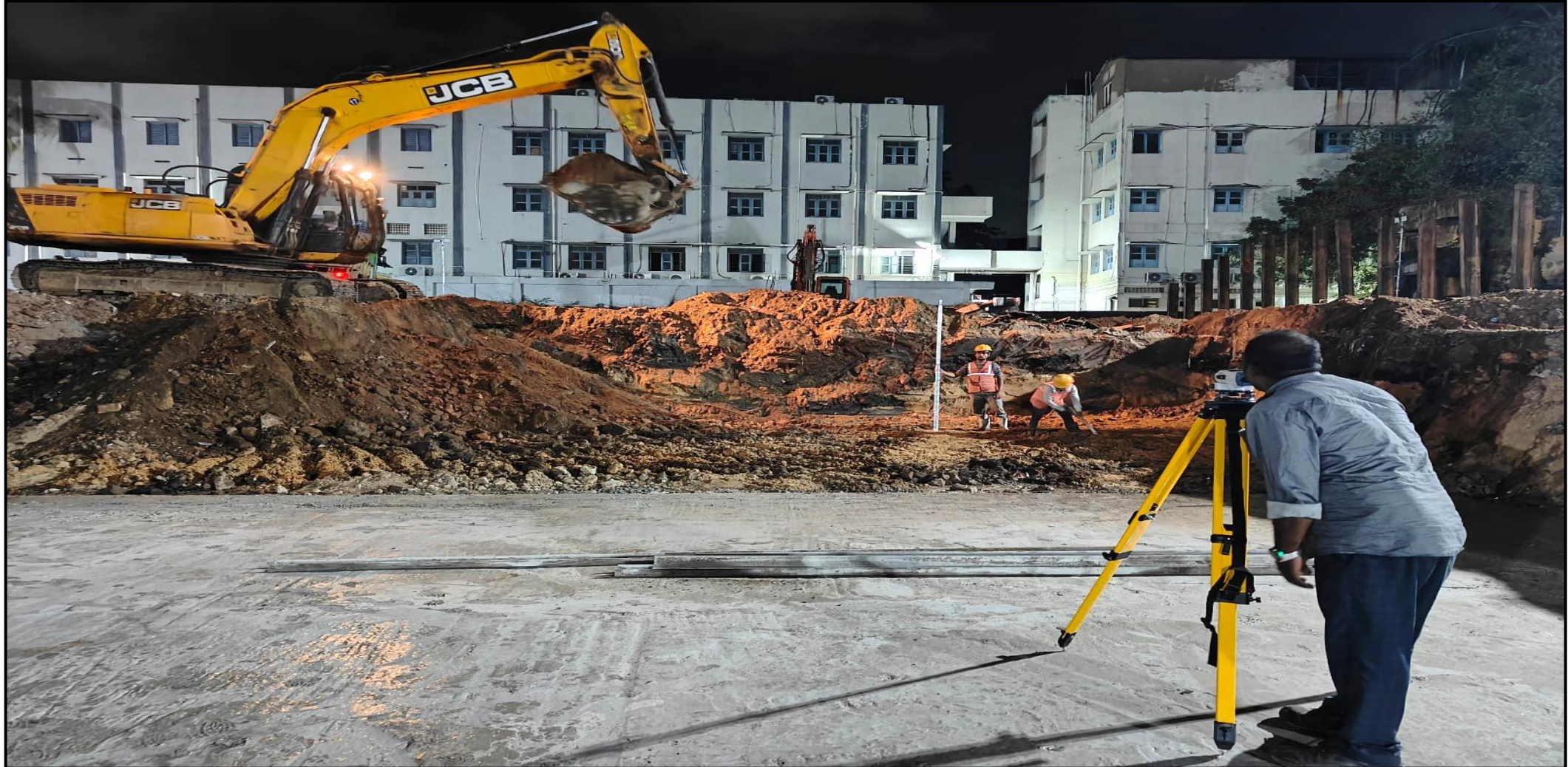
Main building – Raft excavation work in progress (3834/7838 cum)
