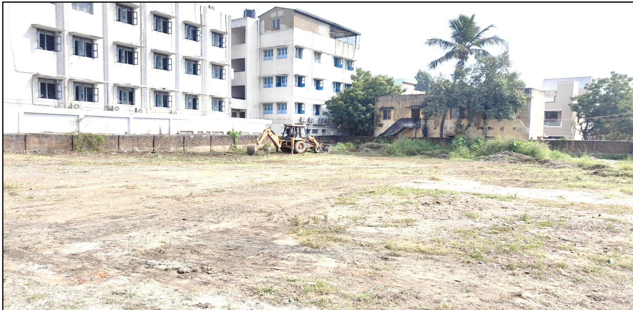
Site cleaning work completed
