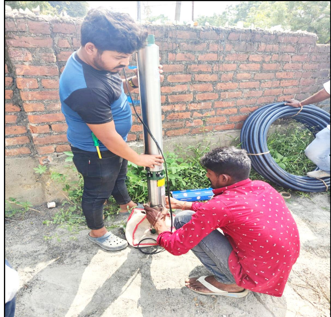
Bore well pump installation work completed
