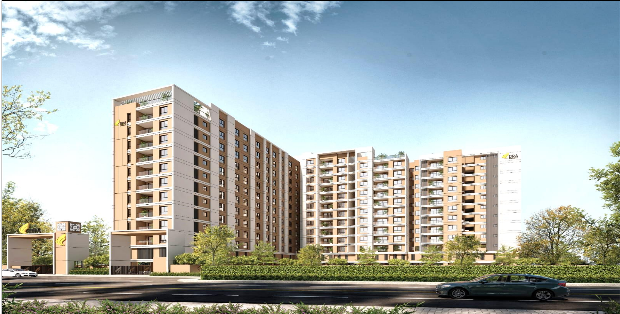
DRA ASTRA Construction update photos – January 2025
