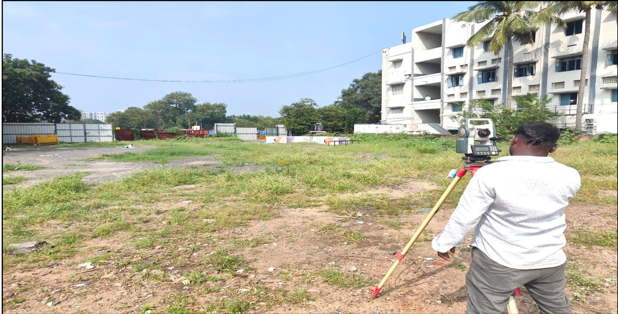
Boundary line survey marking work in progress
