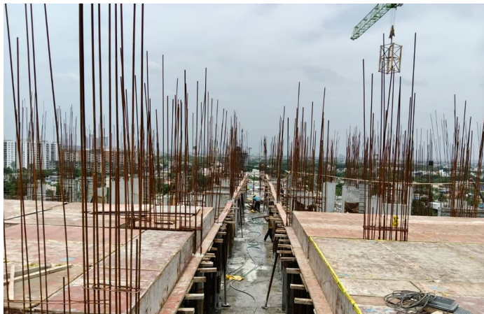
Tenth Floor P2 - Roof Slab Shuttering
