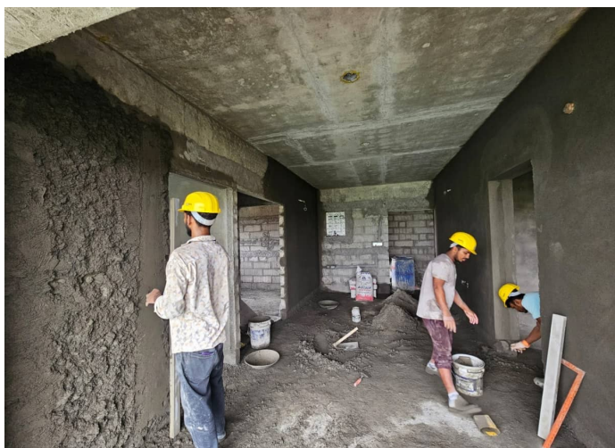
Ninth Floor P2 - Roof Slab Concreting
