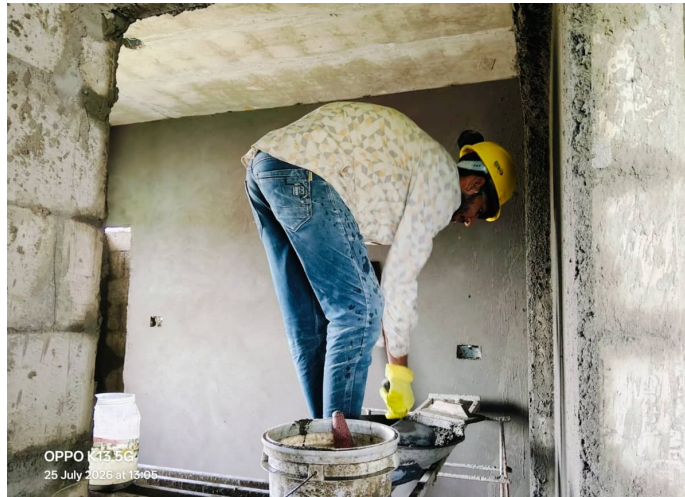
Ninth Floor P2 - Roof Slab Concreting
