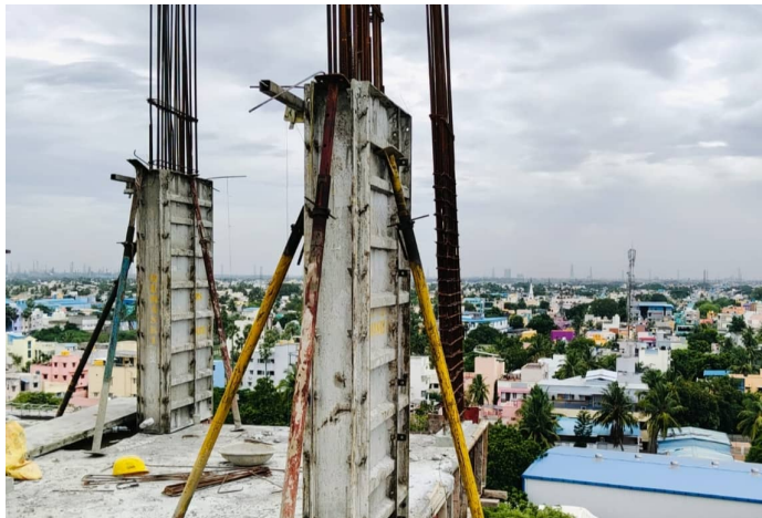
Tenth Floor P2 - Column Shuttering
