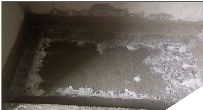
4F - Toilet Waterproofing
