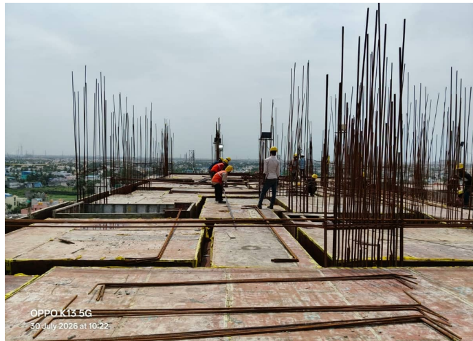
Tenth Floor P1 - Roof Slab Shuttering
