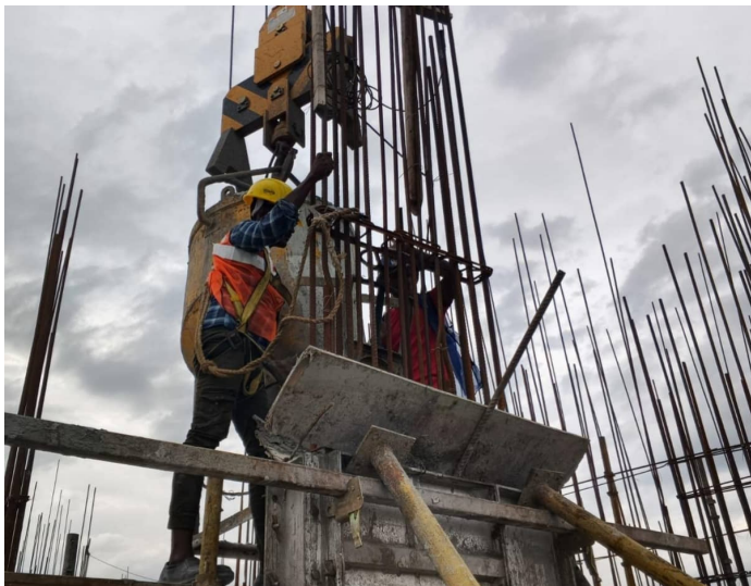
Tenth Floor P2 - Column Concrete
