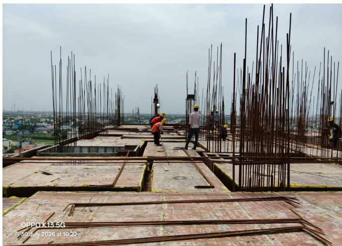
Tenth Floor P1 - Slab & Beam Reinforcement
