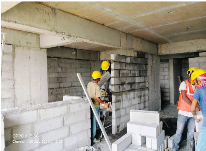
Second Floor P1 - Roof Slab Shuttering
