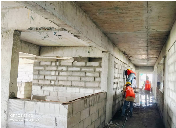
Second Floor P1 - Roof Slab Shuttering
