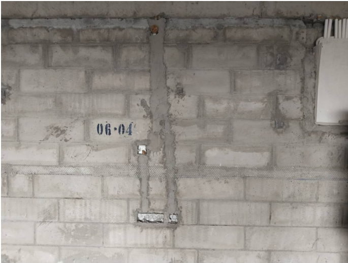
Eighth Floor P1 - Col Marking & Reinforcement
