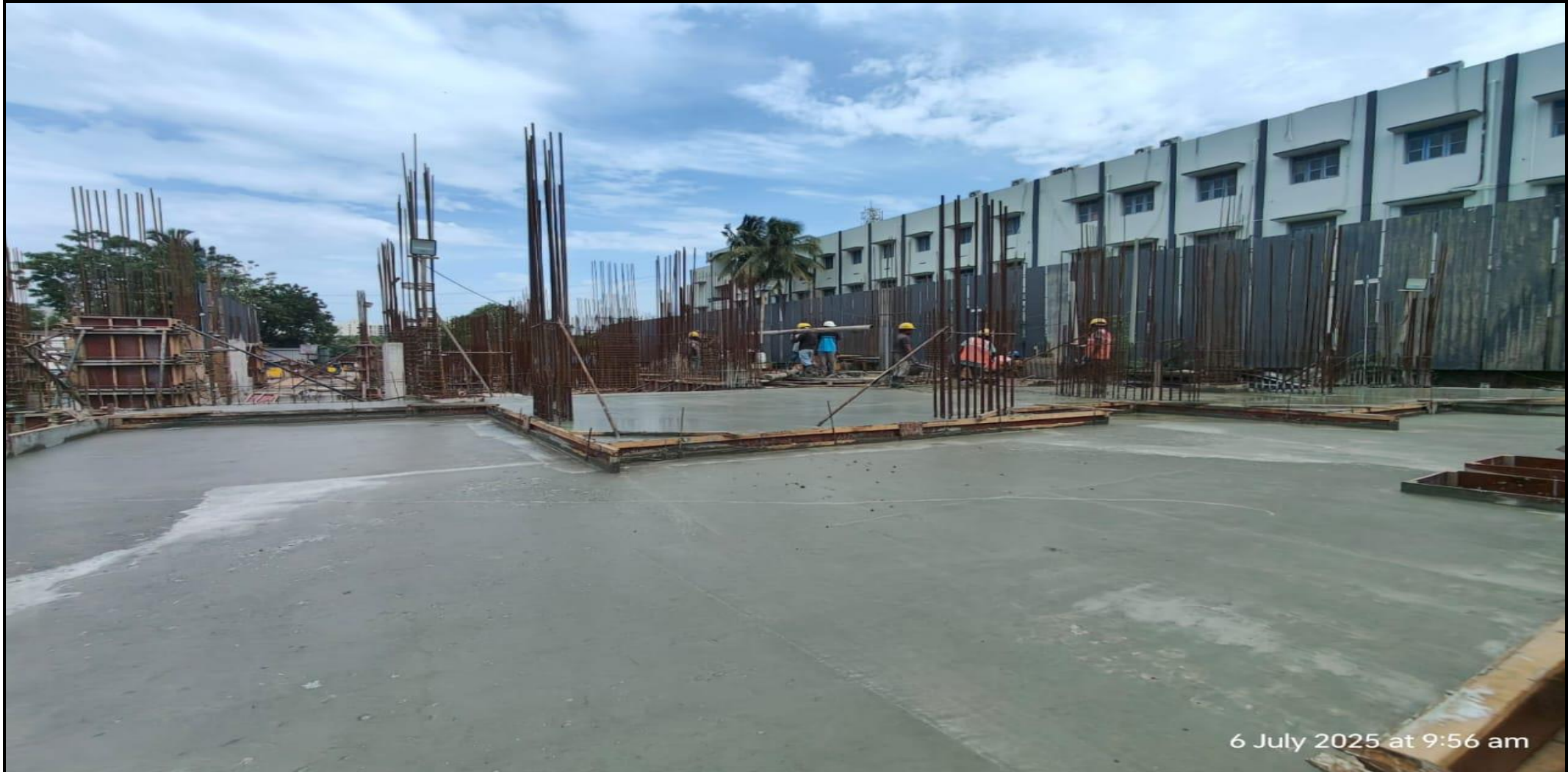
UG sump cover slab concrete work completed.
