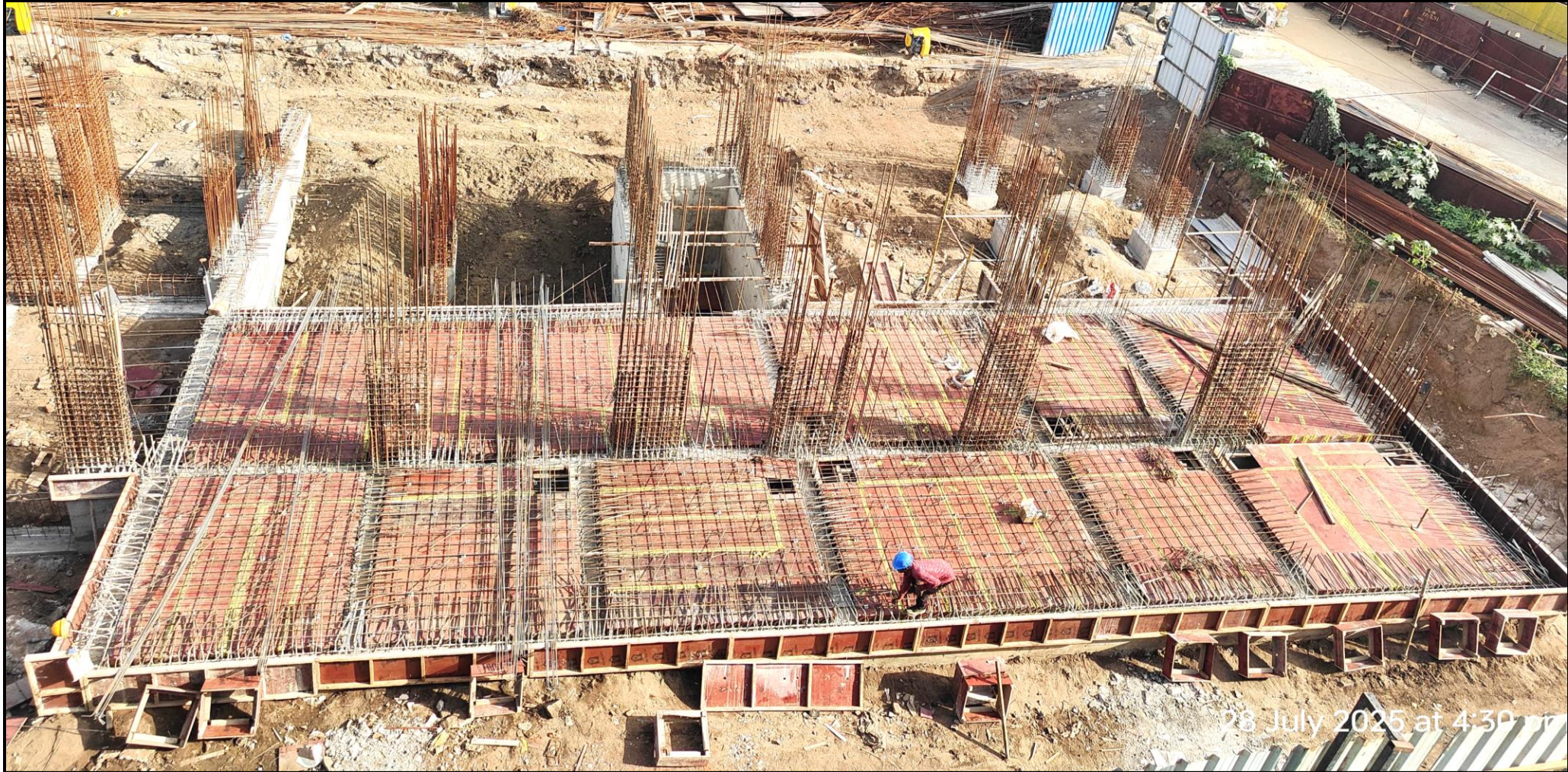
STP Cover slab shuttering and Reinforcement work completed
