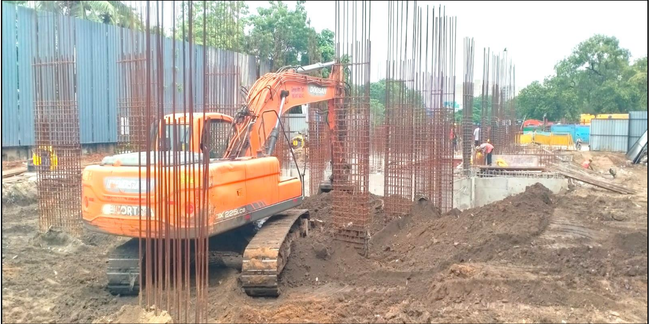
Main building – Pour 04 Plinth beam PCC bottom soil levelling work completed.
