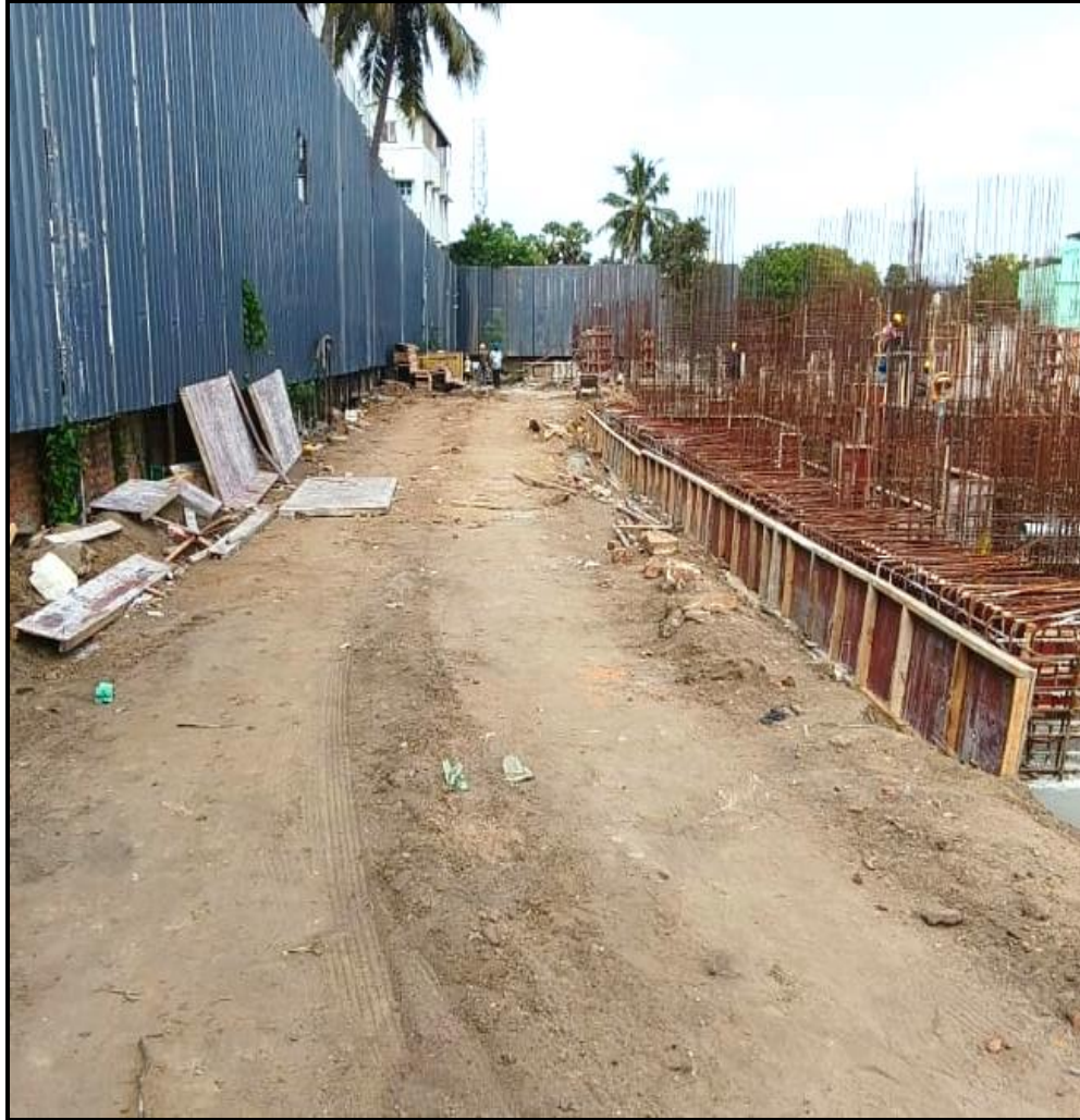
STP North and south side back filling work completed.
