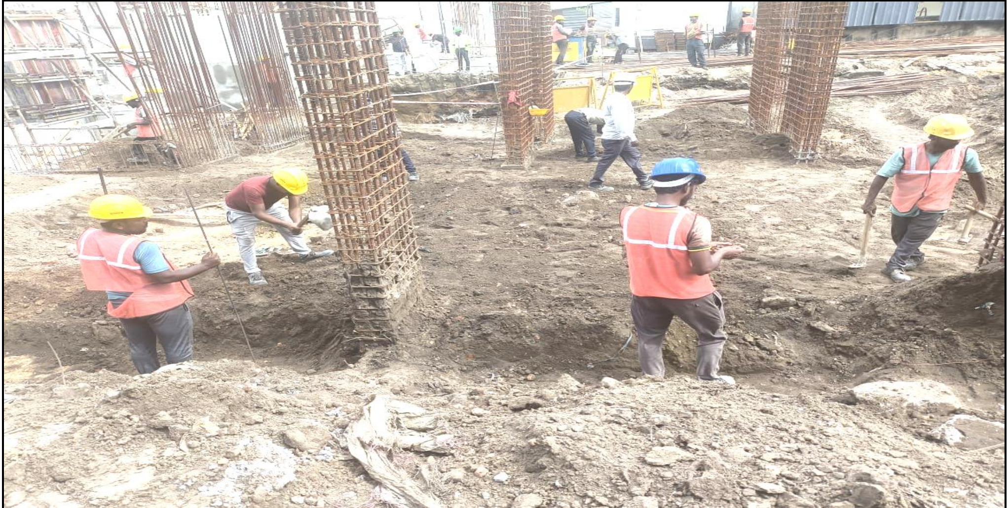
Main building – Pour 04 Plinth beam PCC preparation work completed
