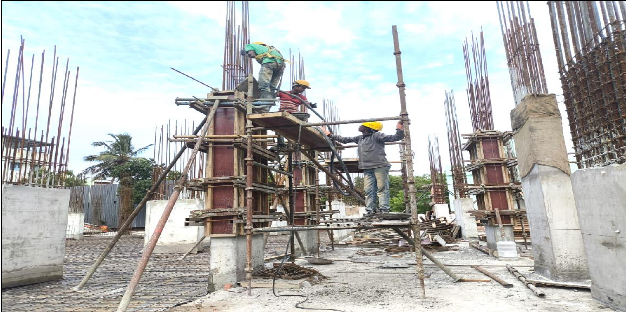
Main building – Pour 1 stilt floor 2 nd lift column concrete completed
