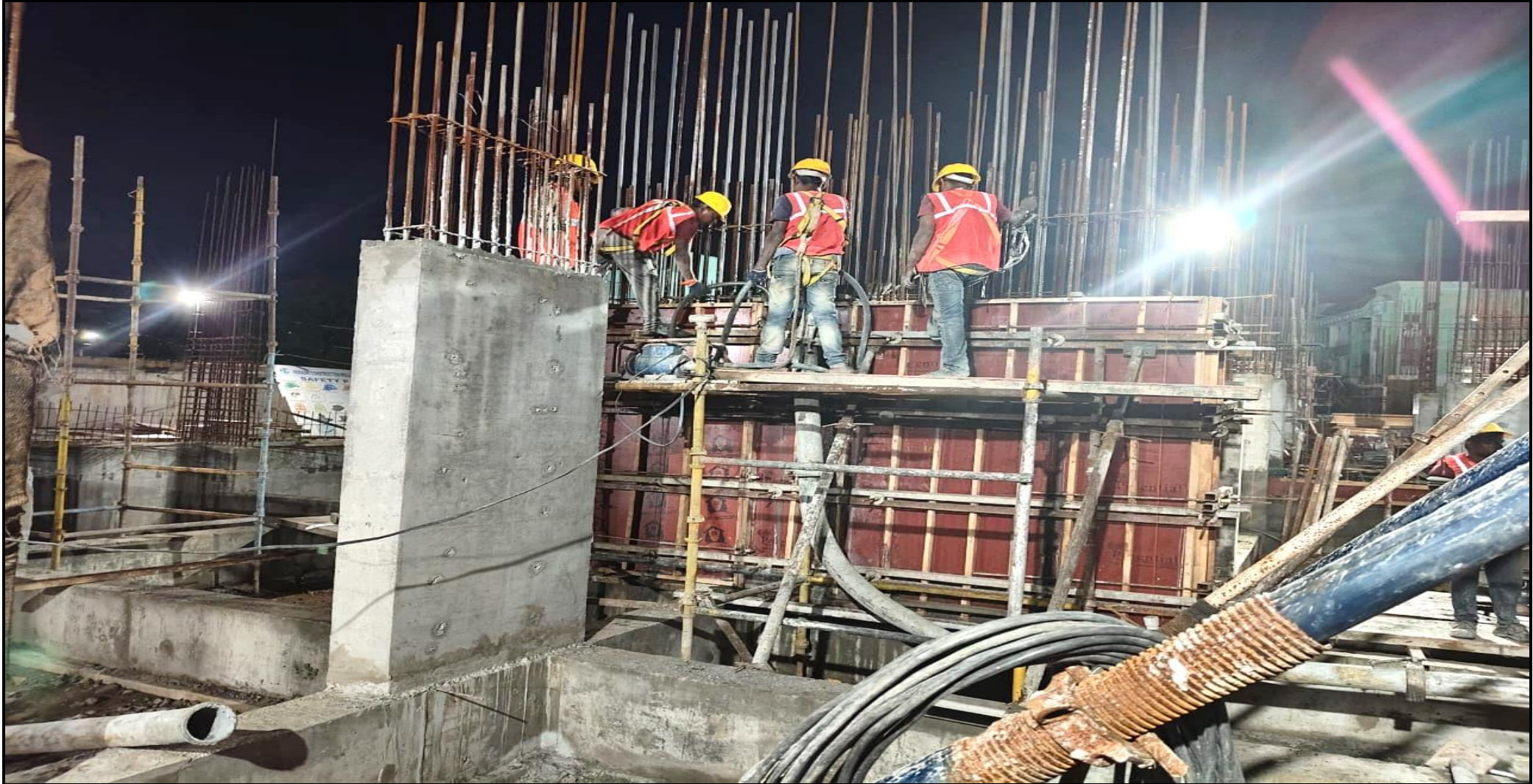
Main building – Core wall 1 st lift concrete 2 no's completed (3/3 no's)
