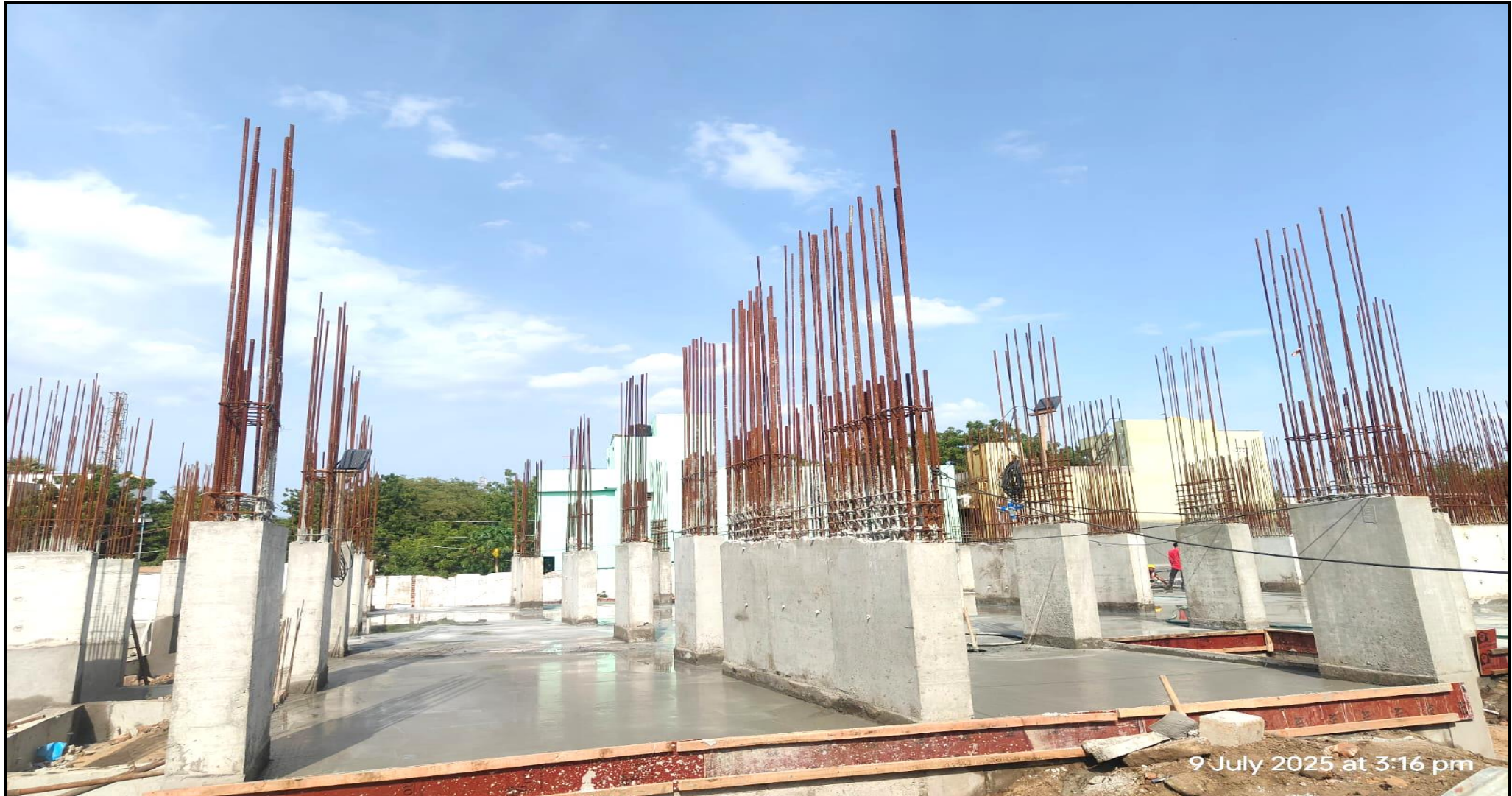
Main building – Pour 1 grade slab concrete completed
