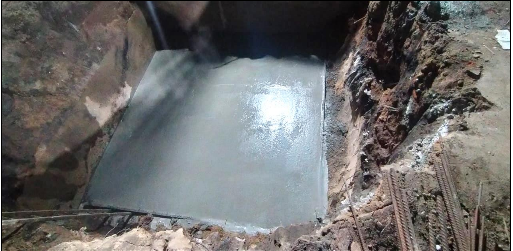
Tower crane Excavation and PCC work completed.
