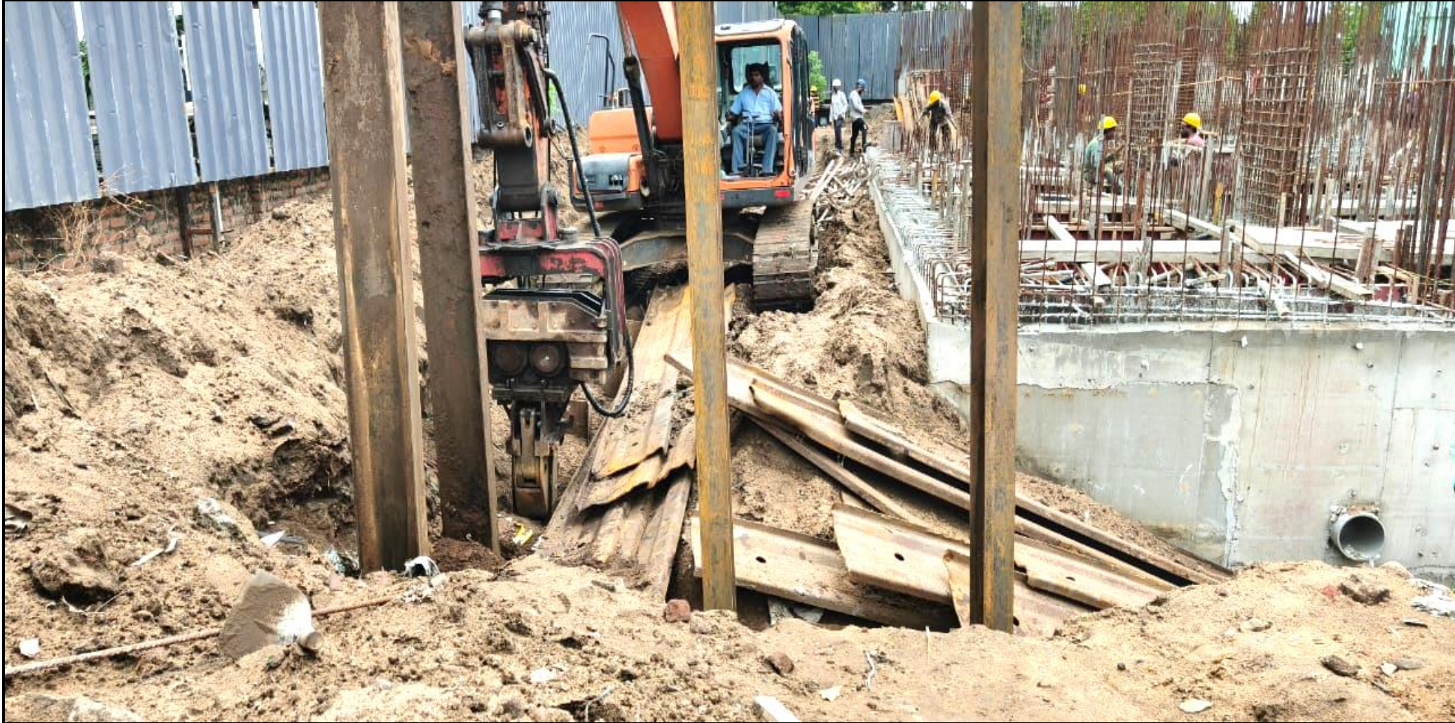
STP – shoring removal work completed
