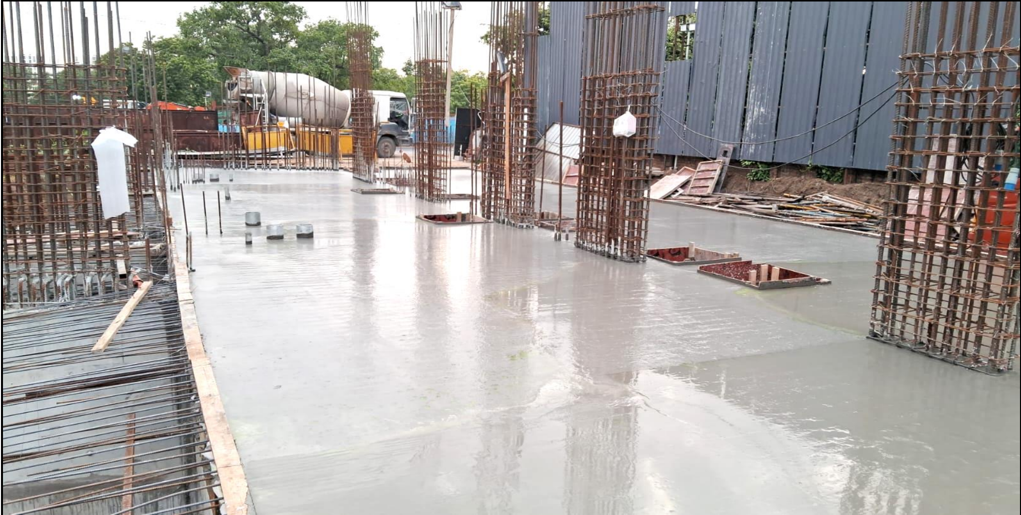
STP Cover slab concrete work completed
