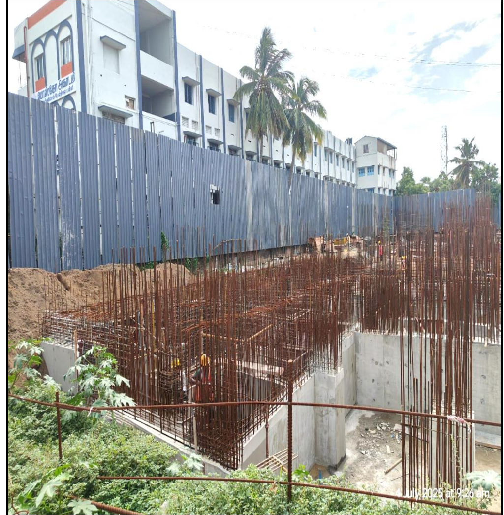
STP – 2 nd lift Reinforcement work completed.
