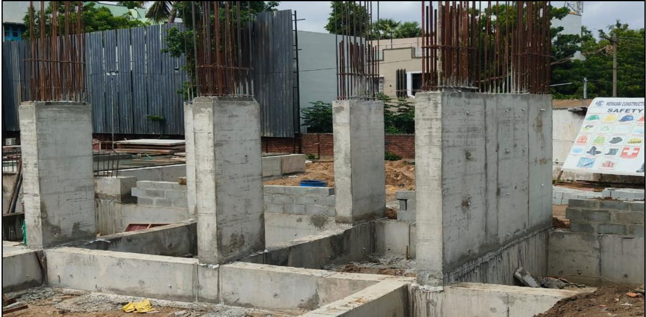
Main building – Pour 1 1 st lift column concrete completed (94/127 no's)
