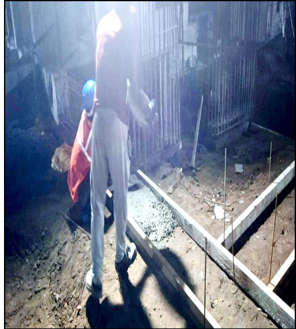
Main building – Pour 04 Plinth beam Below ATT & PCC work completed .
