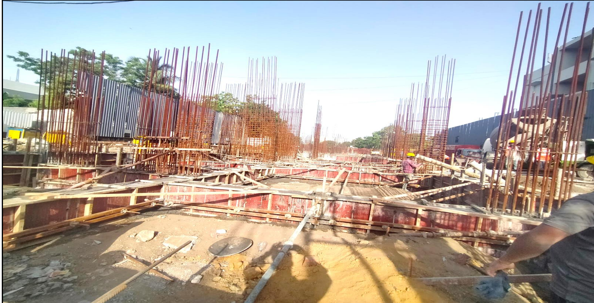
Main building – Pour 04 Plinth beam concrete completed
