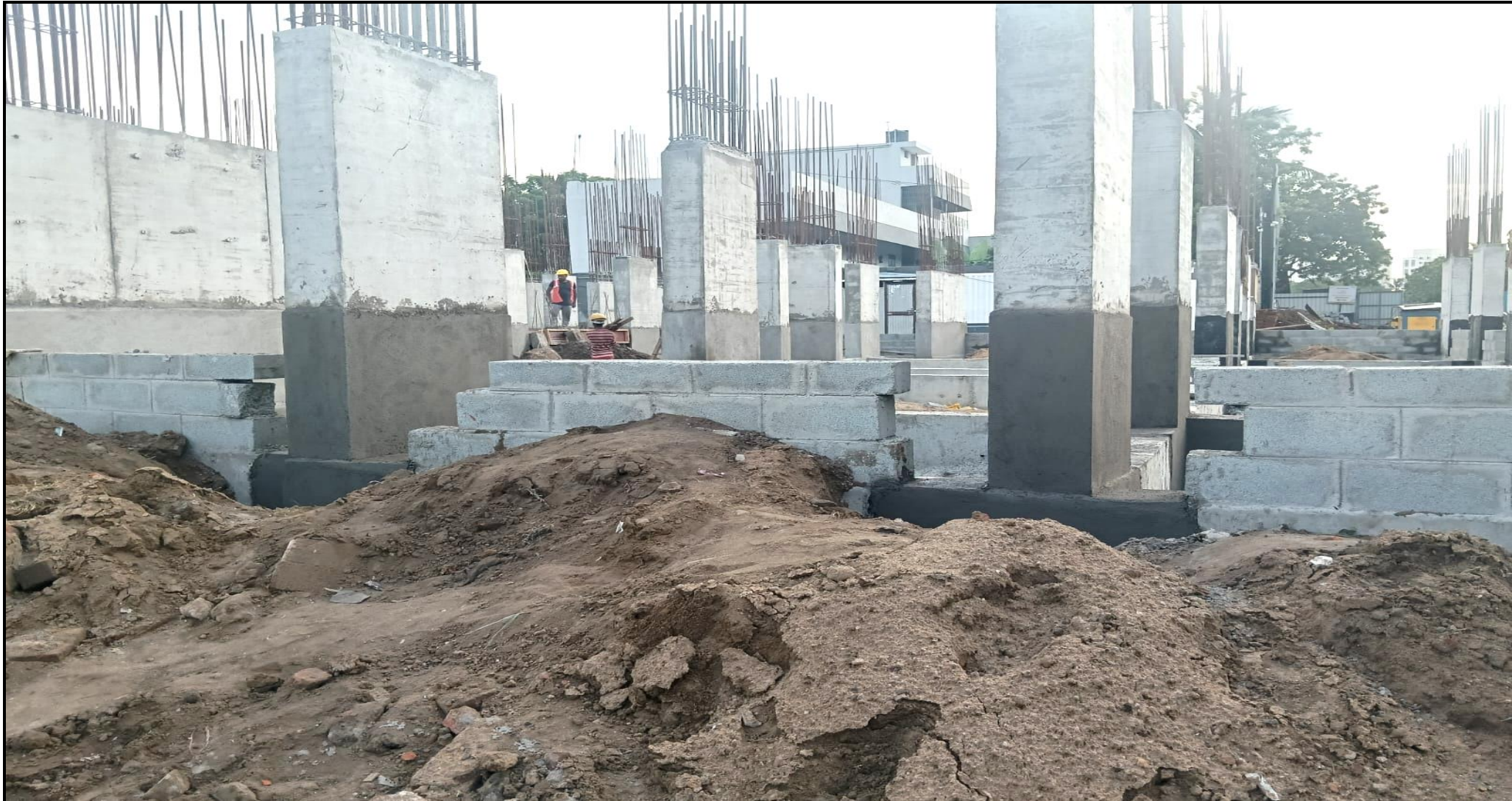
Main building – Pour 01 DPC protective plastering work completed
