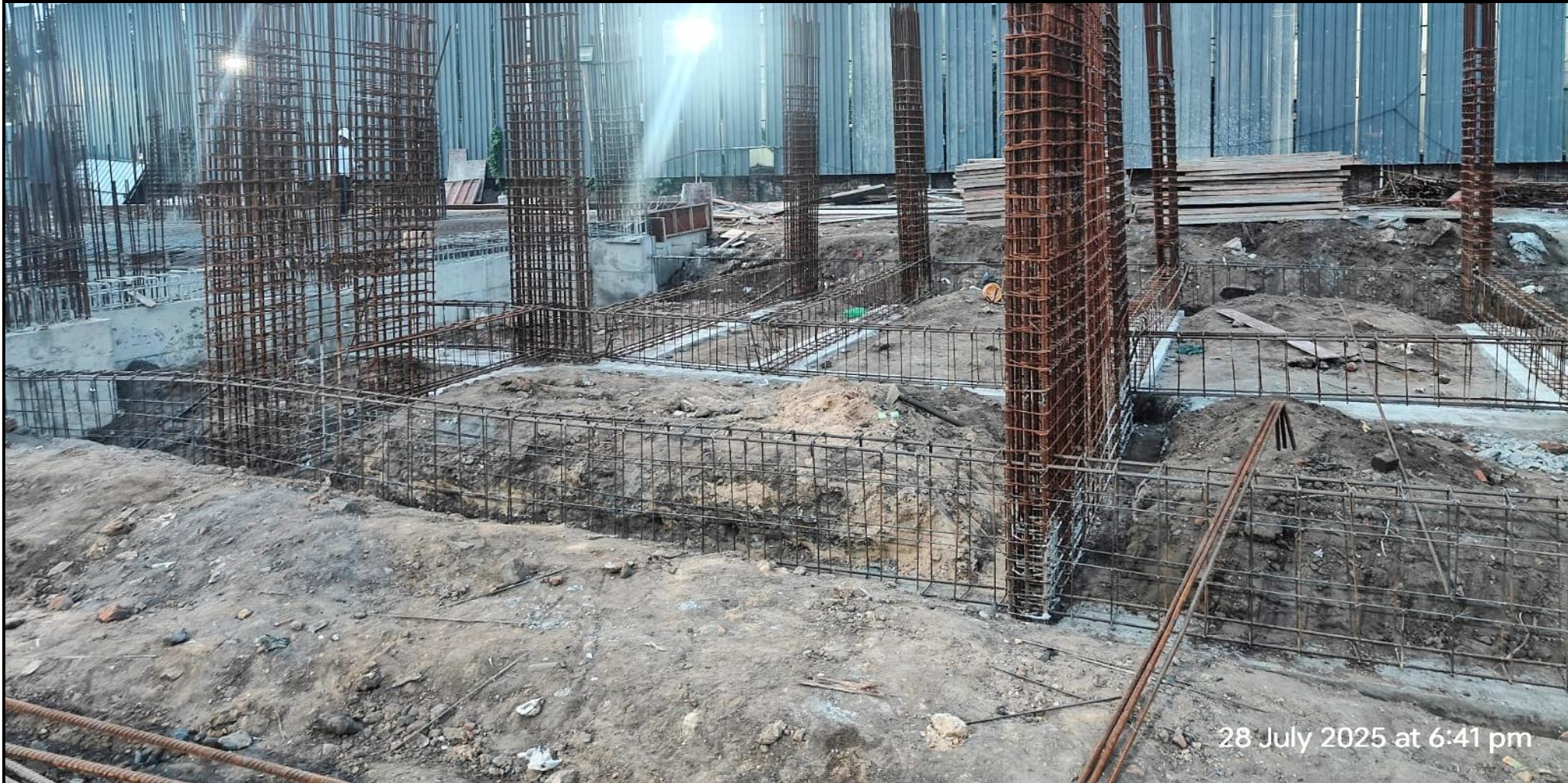
Main building – Pour 04 Plinth beam PCC and Reinforcement work completed.
