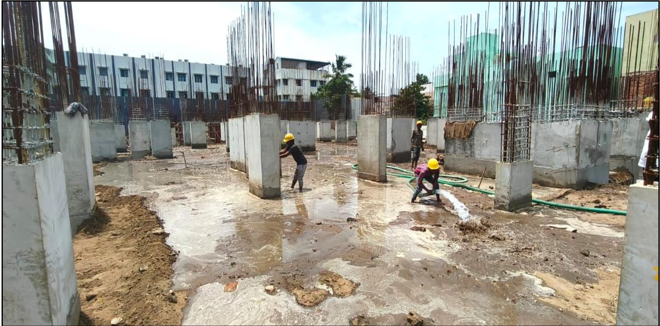
Main building – Pour 01 back filling consolidation work completed.
