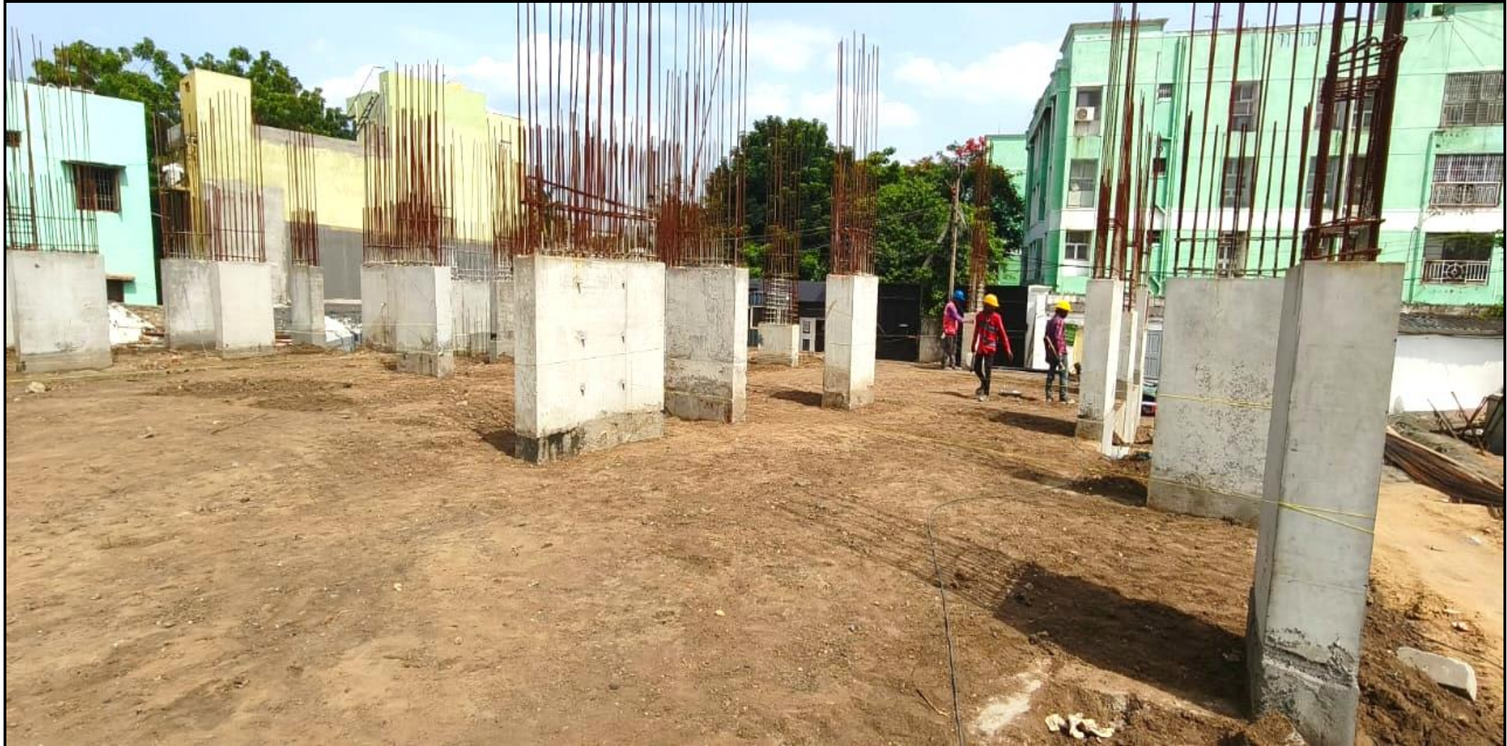
Main building – Pour 01 back filling dressing work completed.
