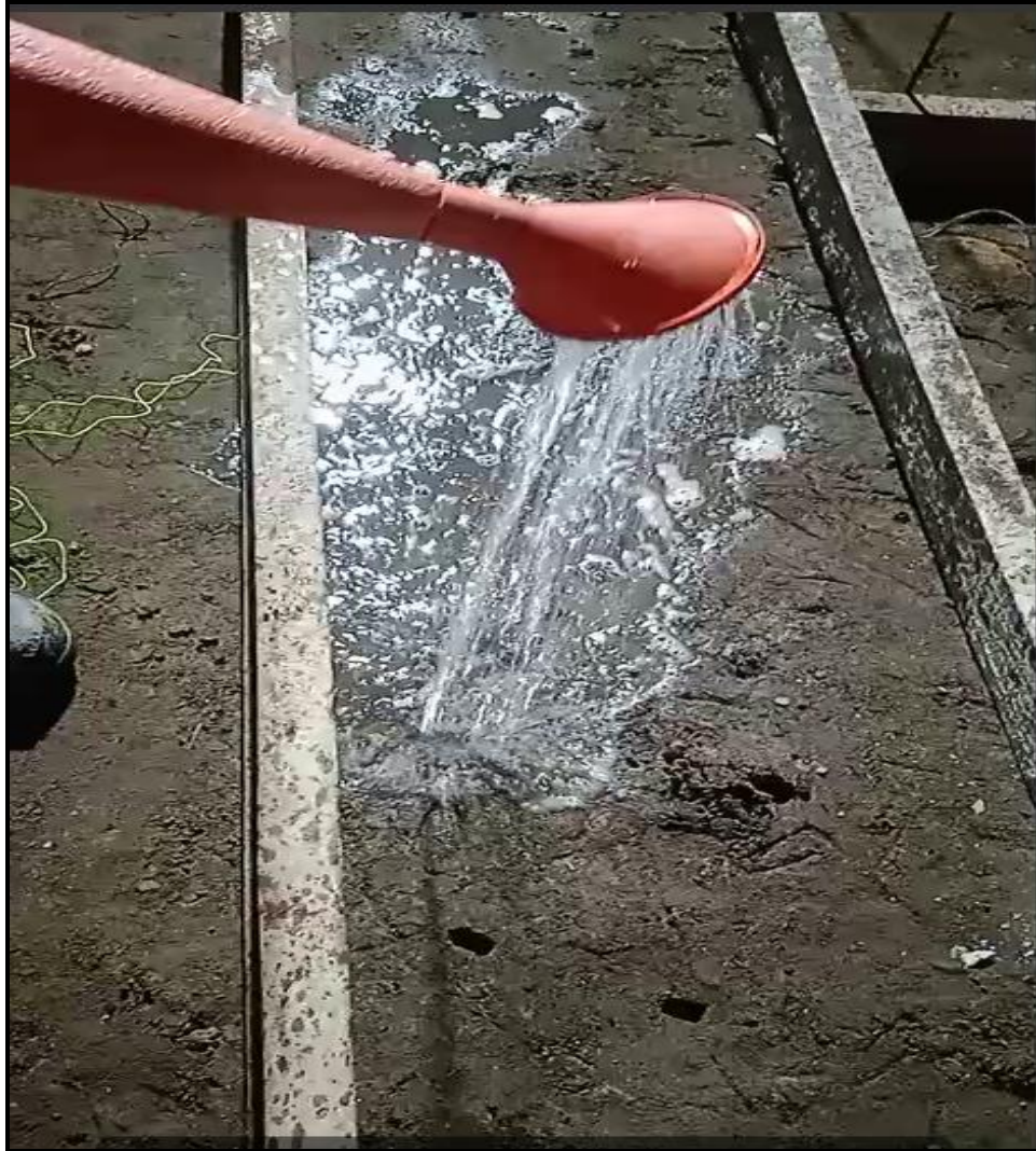
Main building – Pour 04 Plinth beam Below ATT & PCC work completed .
