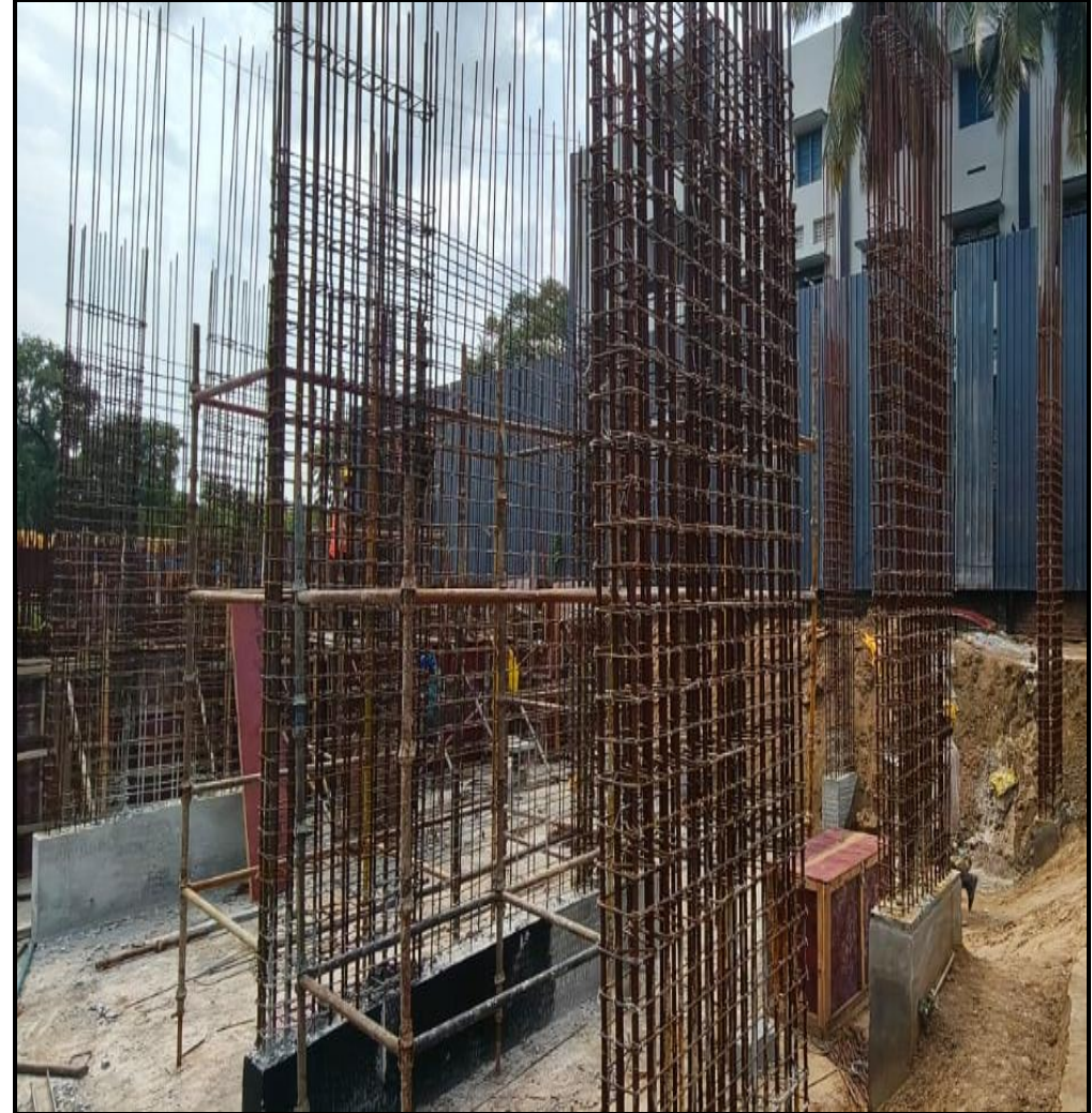
Main building – Pour 1 1 st lift Column Reinforcement work (99/127 no's)
