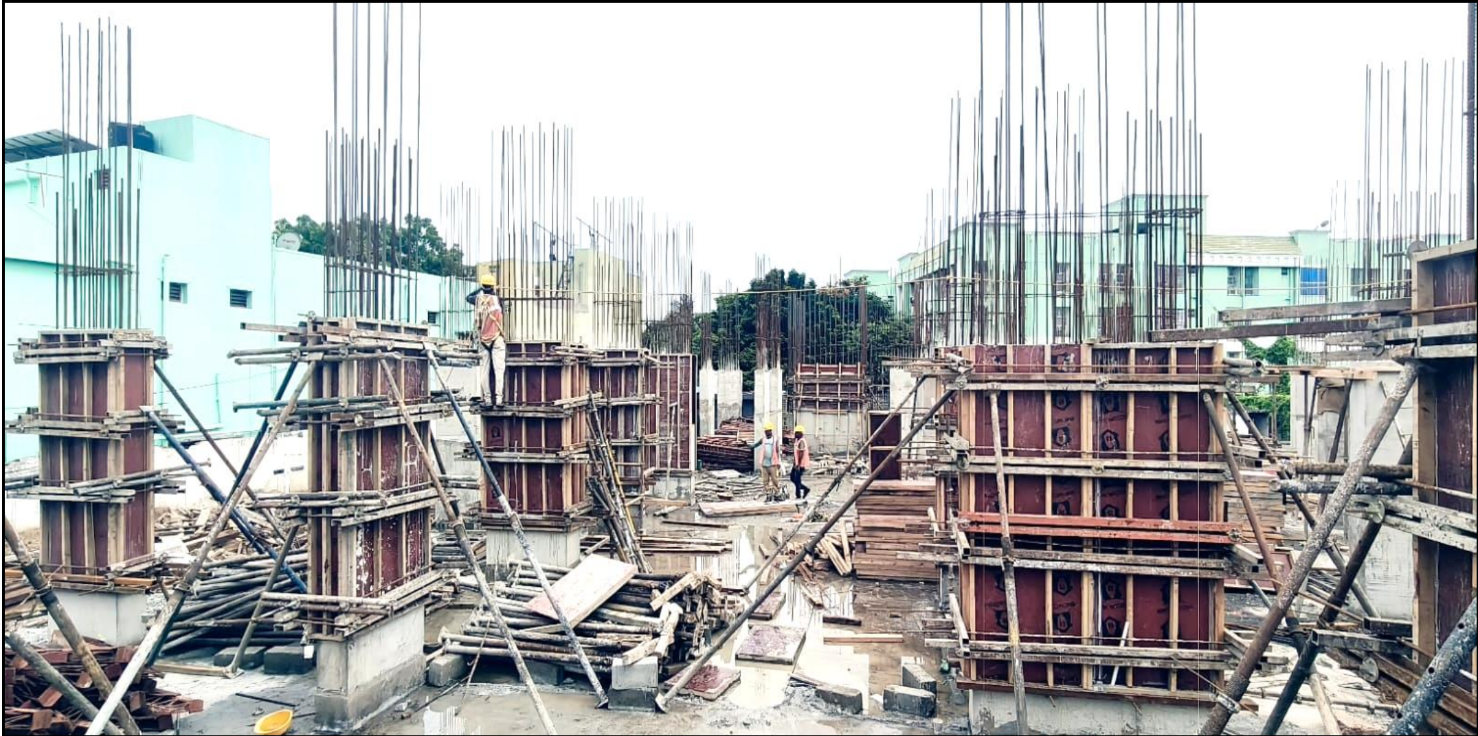
Main building – Pour 1 stilt floor 2 nd lift column shuttering completed
