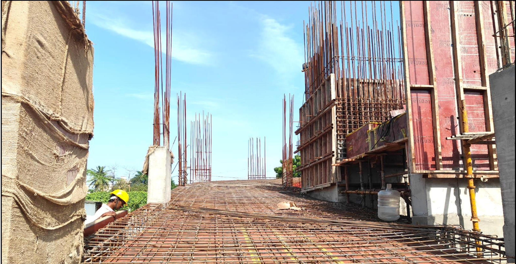
Main building – Pour 01 Ramp shuttering and Reinforcement work in progress
