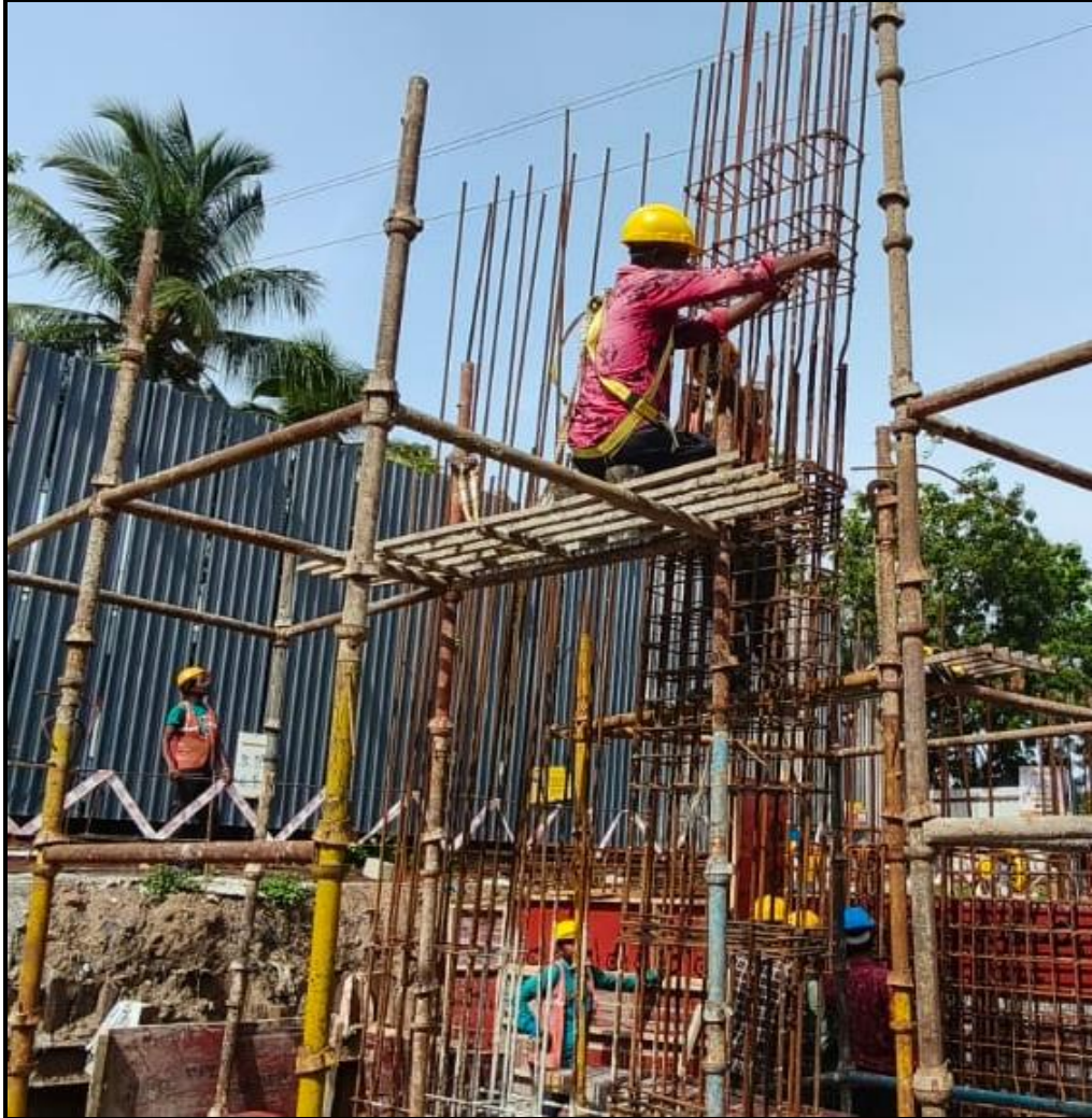
Main building – Pour 1 1 st lift Column Reinforcement work (99/127 no's)
