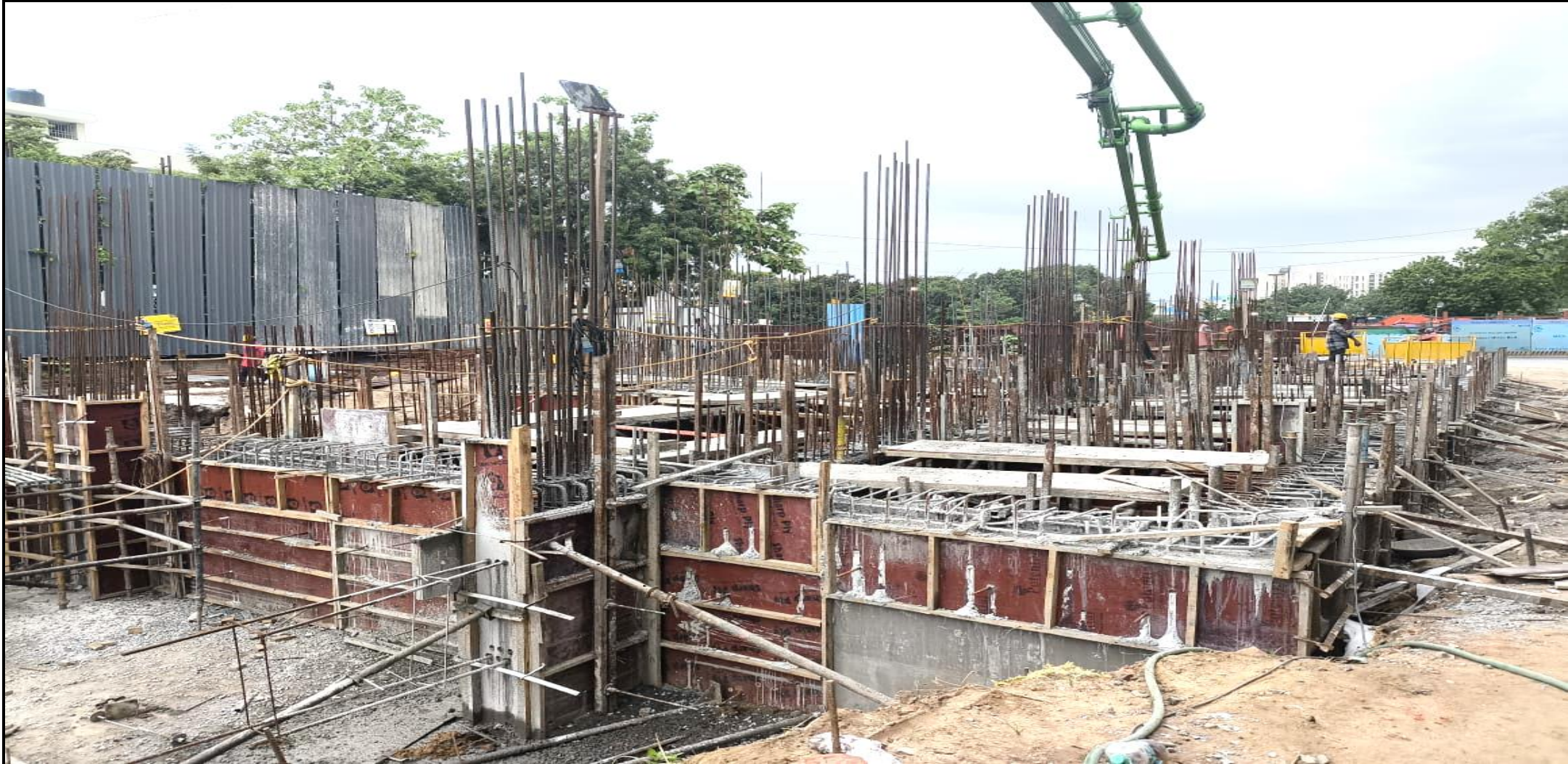
STP – 2 nd lift wall concrete completed
