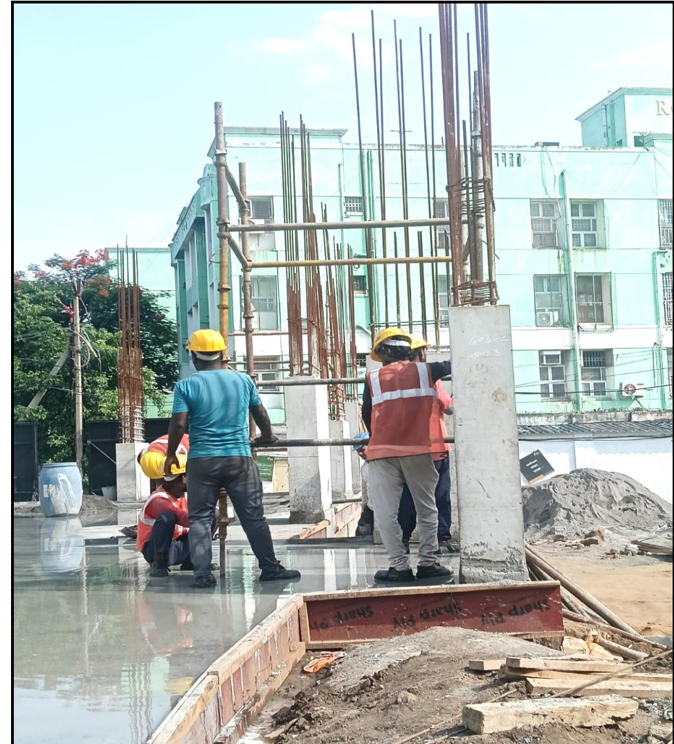
Main building – Pour 1 stilt floor 2 nd lift column reinforcement completed
