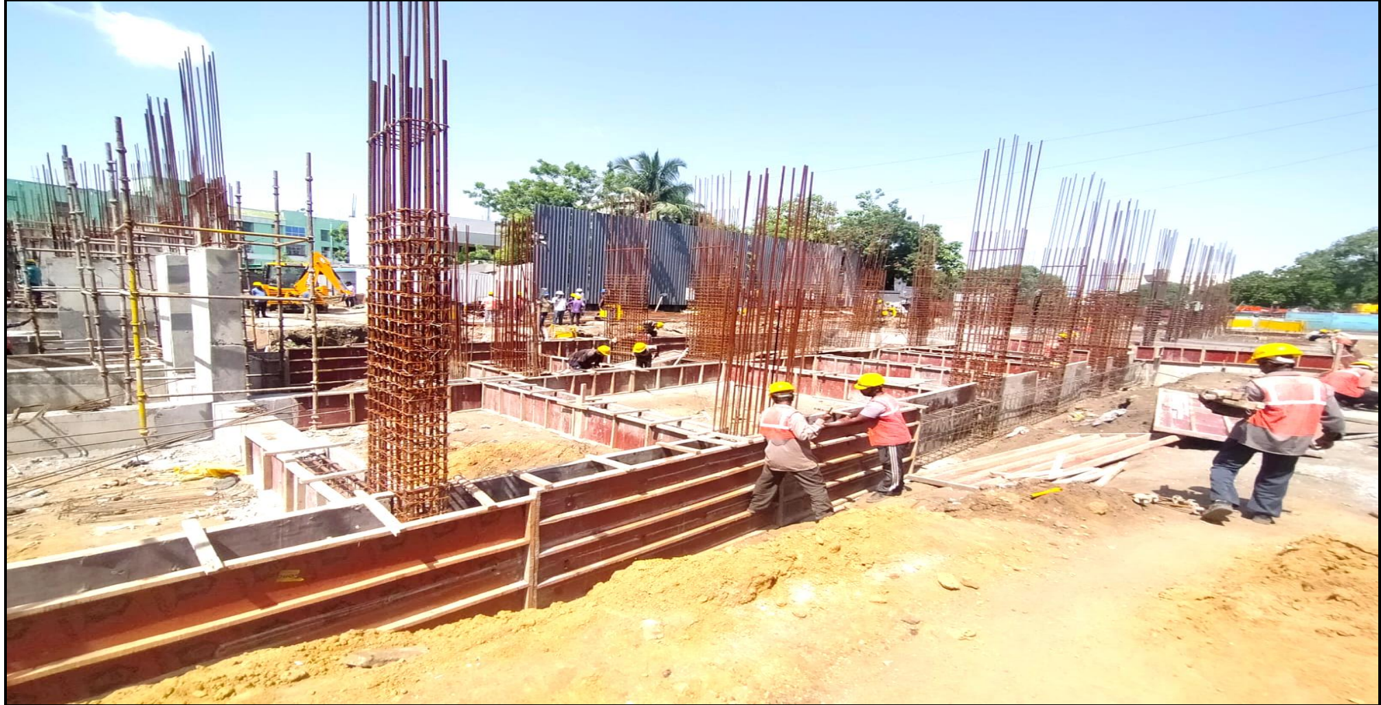
Main building – Pour 04 Plinth beam PCC and Reinforcement work completed.
