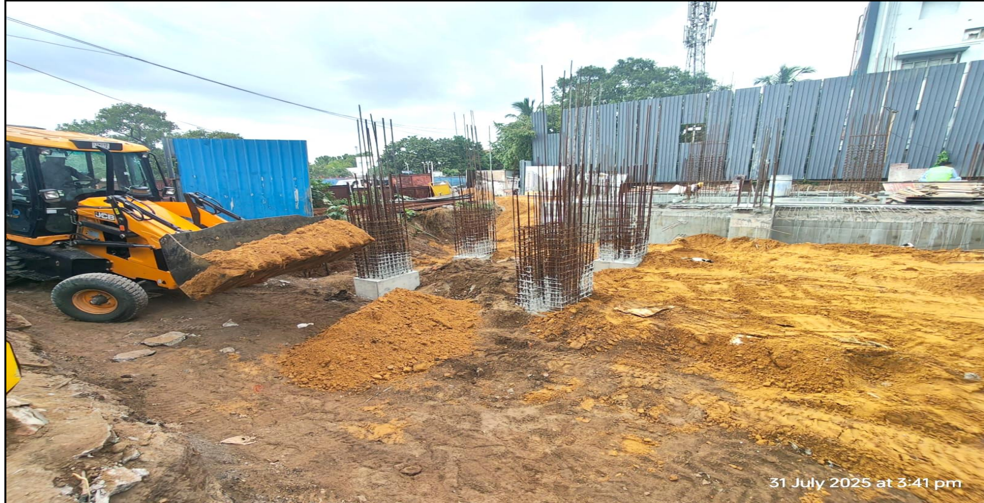
STP back filling work completed
