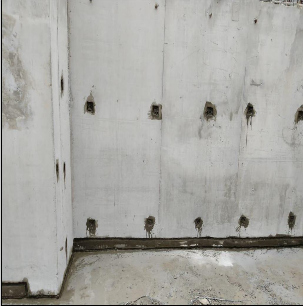
STP wall external water proofing work in progress.
