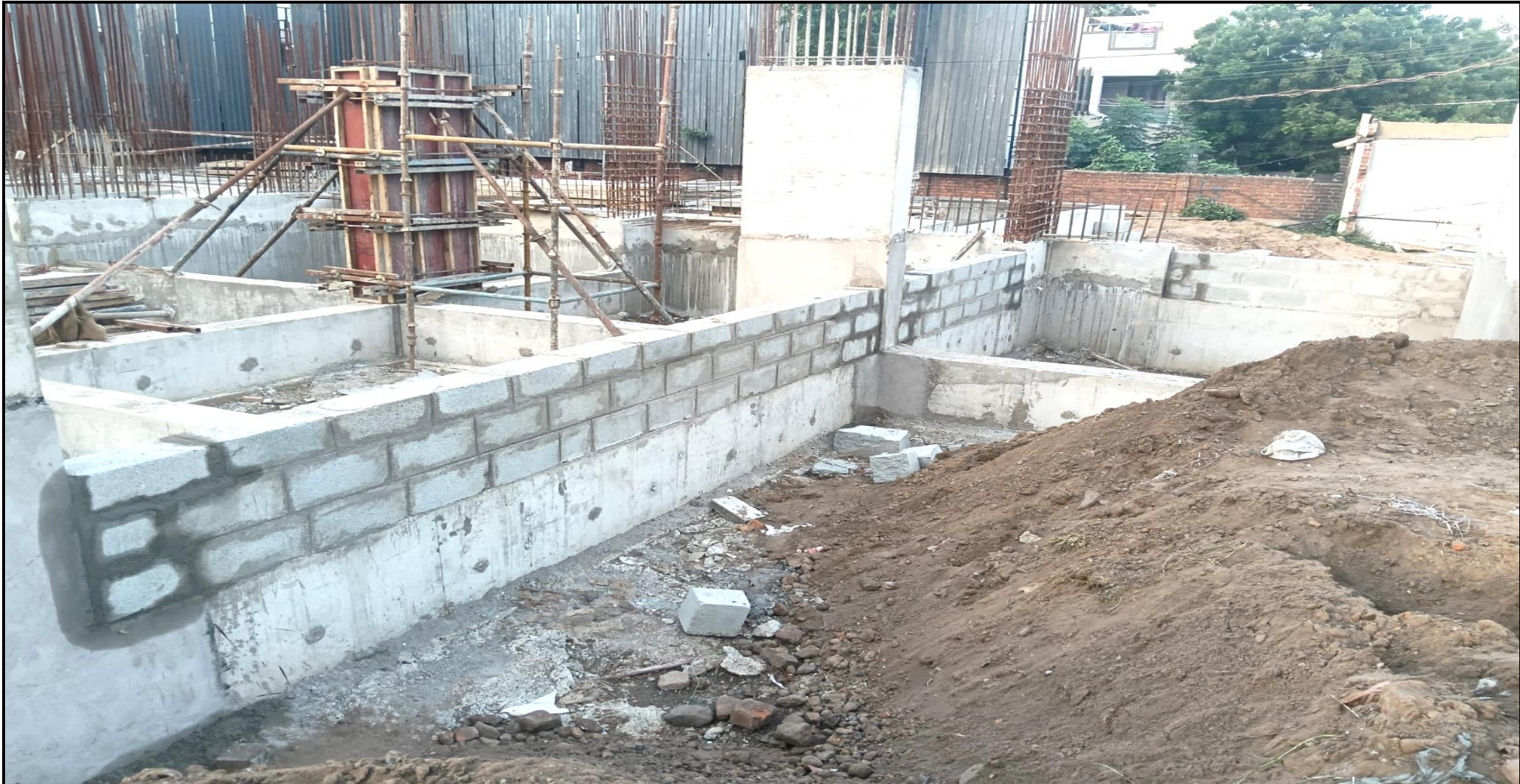
Main building – Pour 1 basement block work completed
