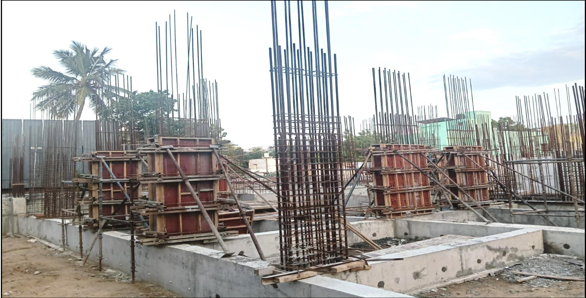
Main building – Pour 1 1 st lift column shuttering work (94/127 no's)
