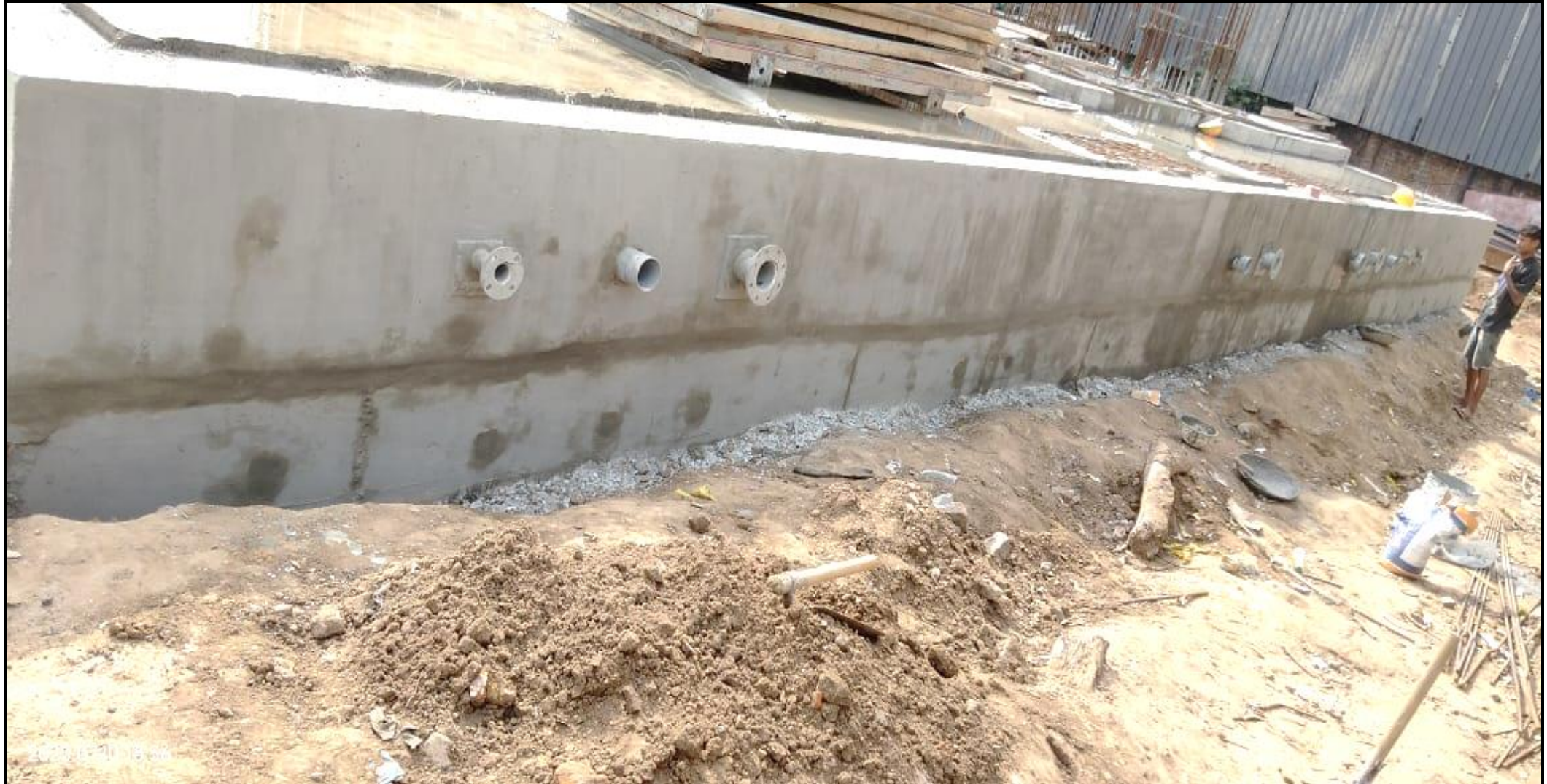
UG sump external wall water proofing work completed
