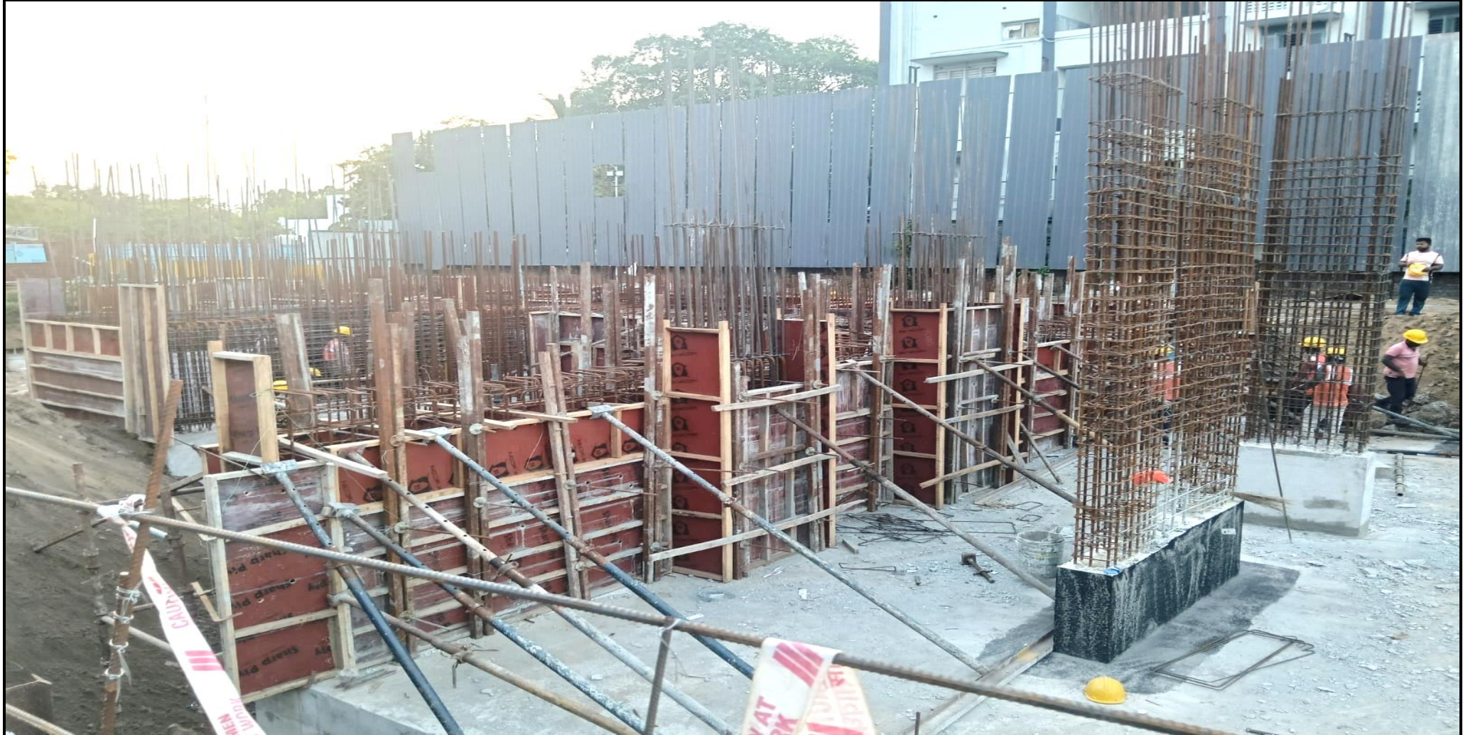
Main building – Pour 04 & 05 RC wall shuttering work completed
