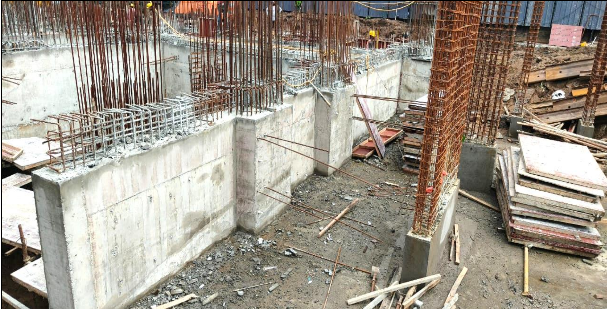
Main building – Pour 04 & 05 RC wall concrete work completed
