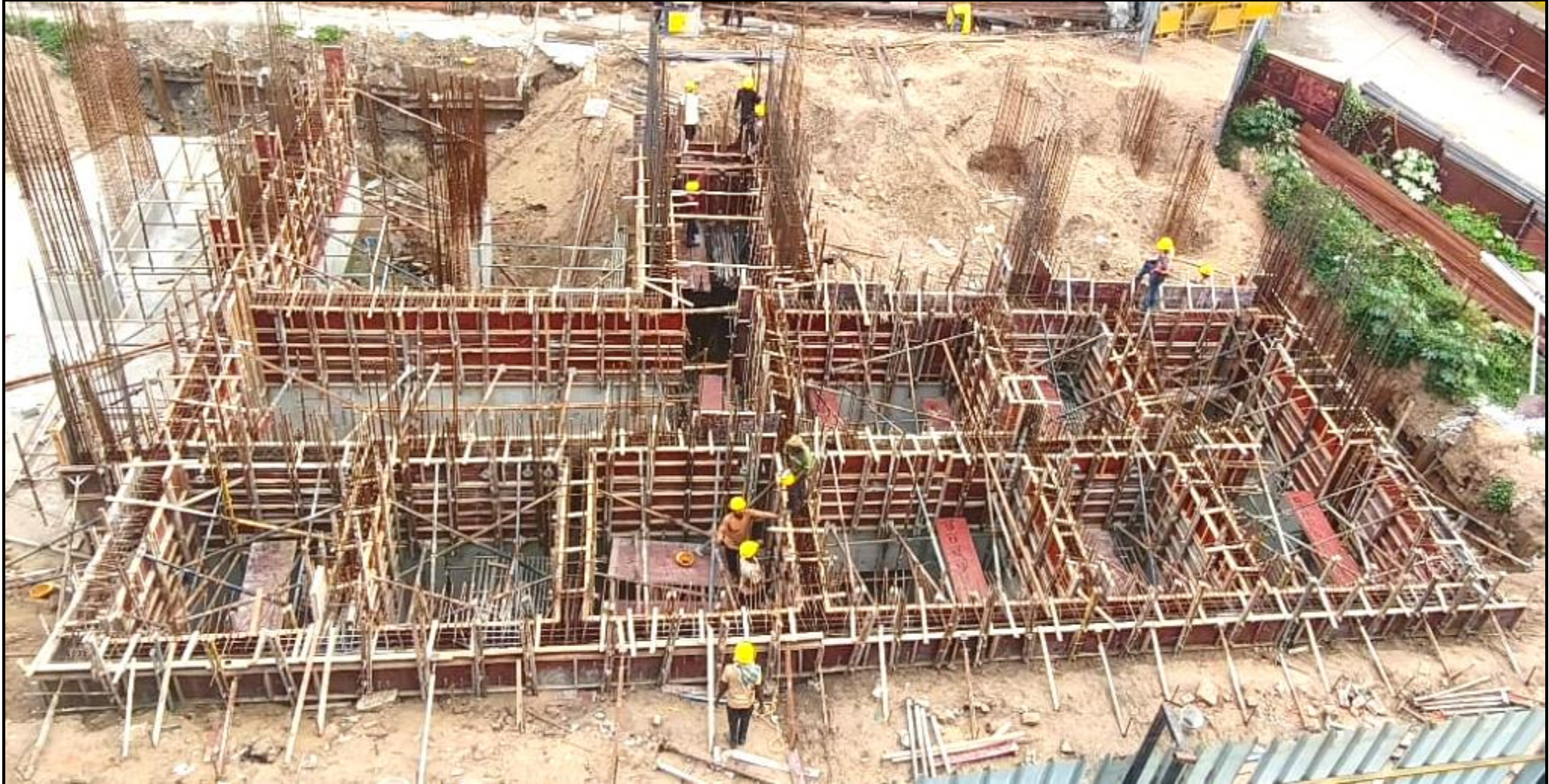
STP – 2 nd lift wall shuttering work completed
