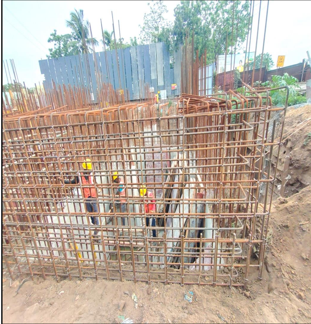
STP – 2 nd lift Reinforcement work completed.
