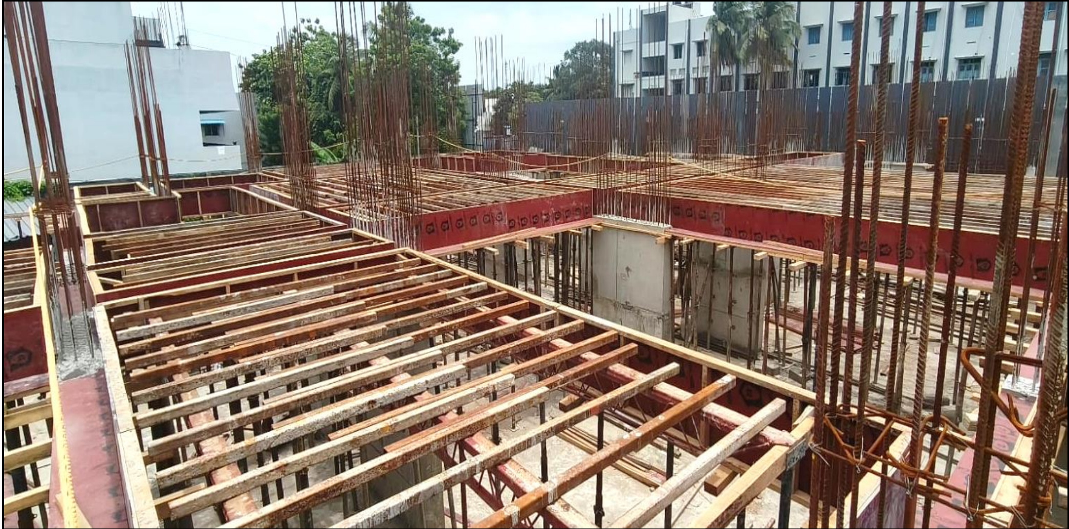
Main building – Pour 01 Stilt floor Roof slab beam bottom and Slab Shuttering work in progress
