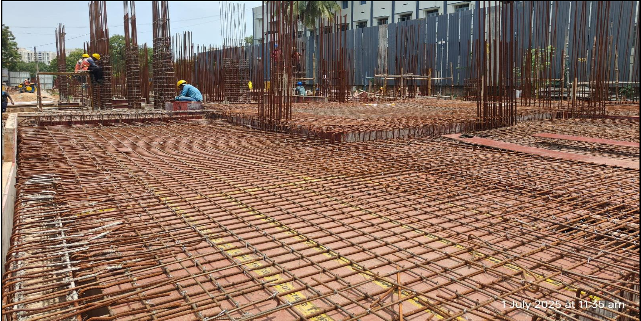
UG sump cover slab reinforcement work completed.
