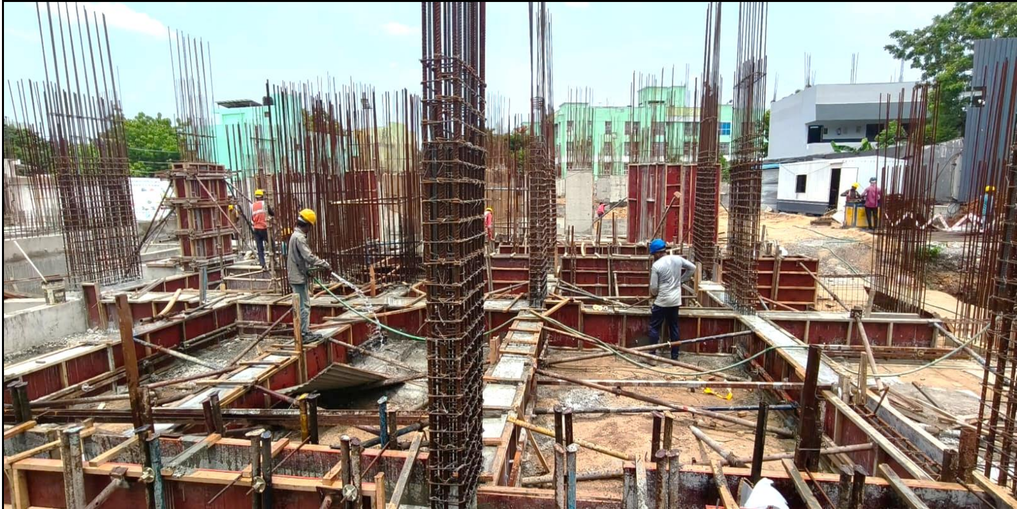
Main building – Pour 03 & 04 plinth beam shuttering & concrete work completed
