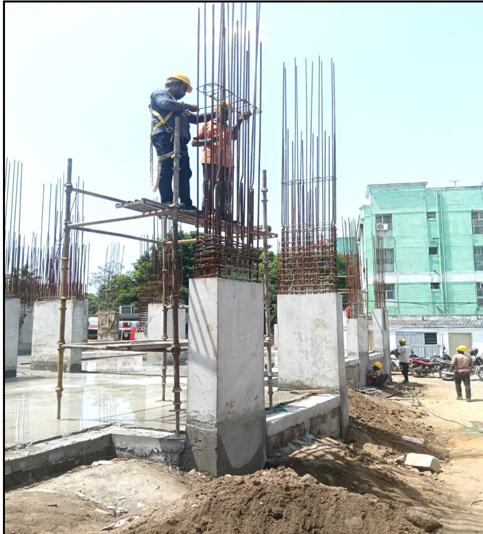
Main building – Pour 1 stilt floor 2 nd lift column reinforcement completed
