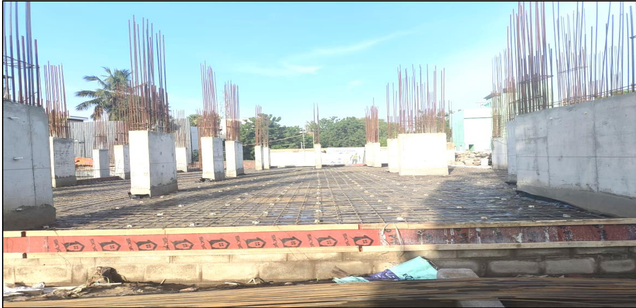
Main building – Pour 1 grade slab LDPE sheet laying & reinforcement work completed
