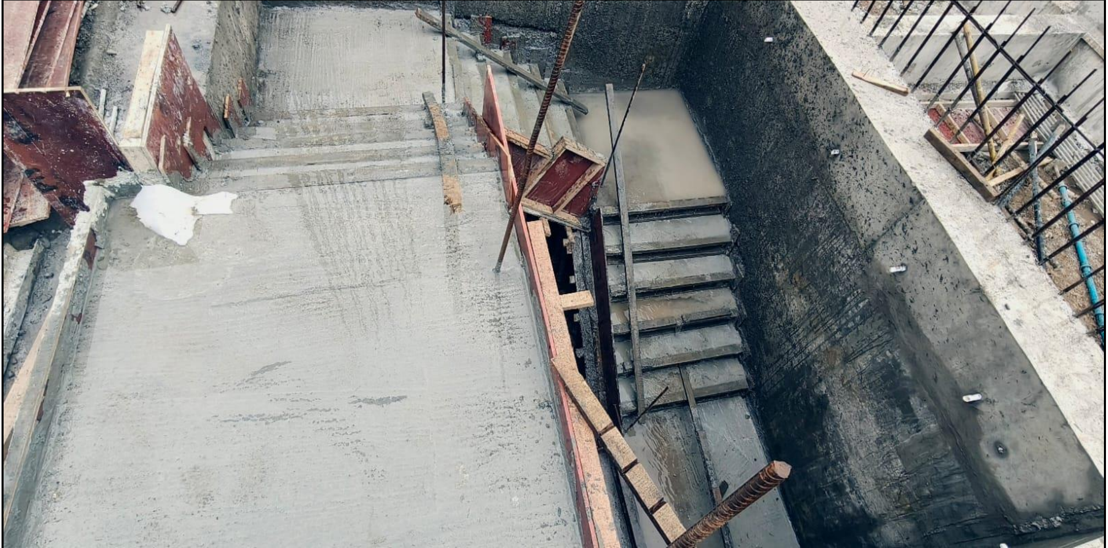
UG Sump – Staircase concrete work completed
