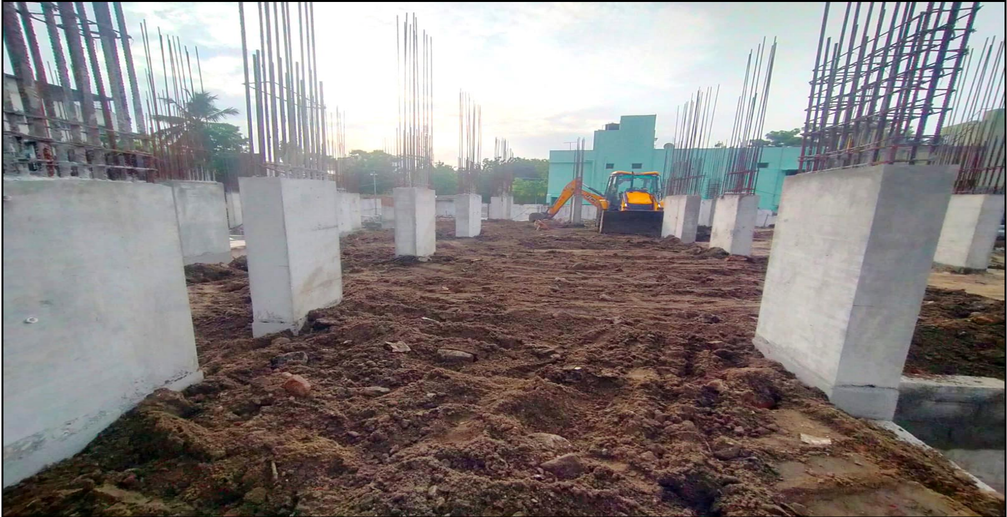
Main building – Pour 01 back filling work completed.
