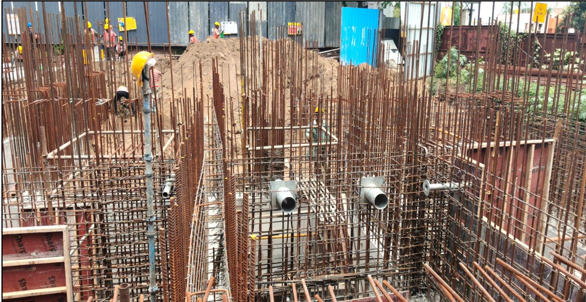
STP – 2 nd lift Puddle flange & Sleeve fixing work completed
