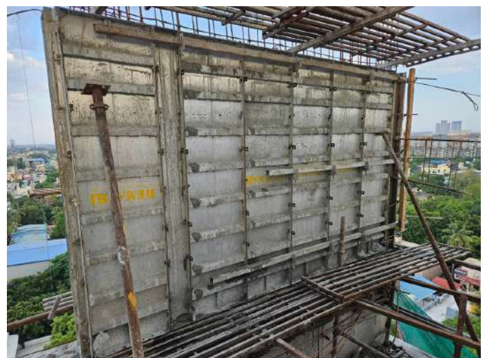
Eleventh Floor P2 - Column Shuttering
