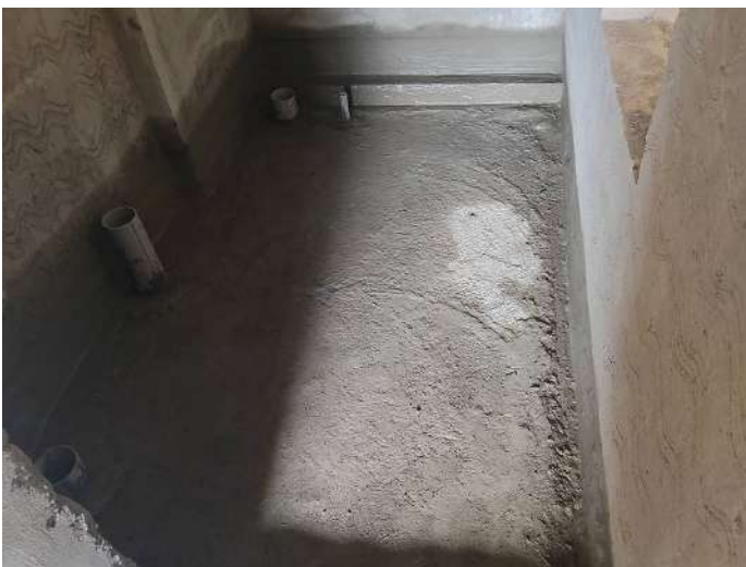
6F - Toilet Waterproofing
