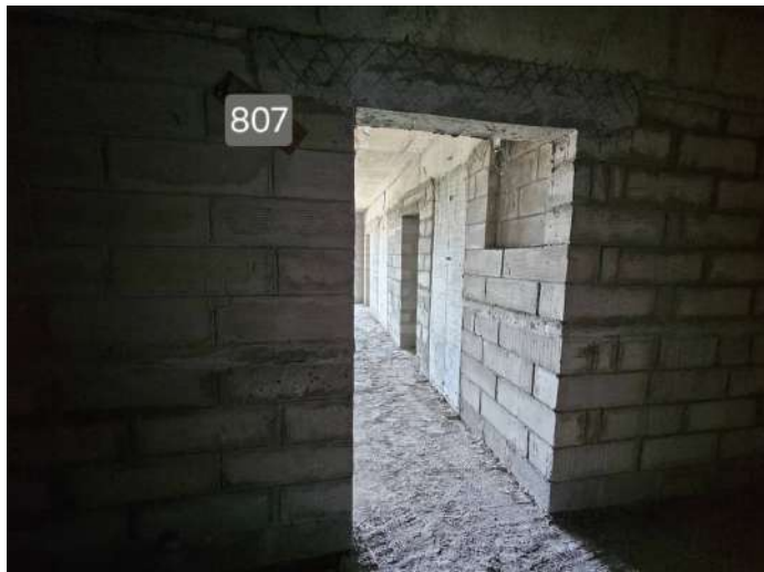
On Completion of Blockwork - 8th Floor - 807
