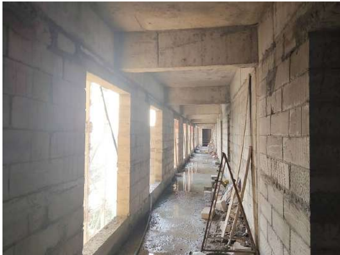
BW Corridor area - Sixth Floor
