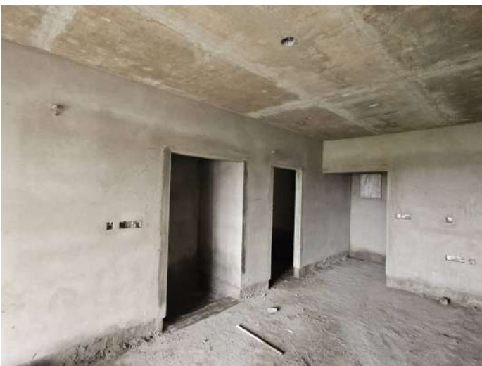
On Completion of Plastering - 6th Floor - 601
