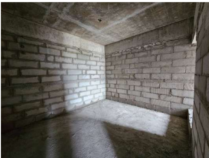
On Completion of Blockwork - 8th Floor - 810
