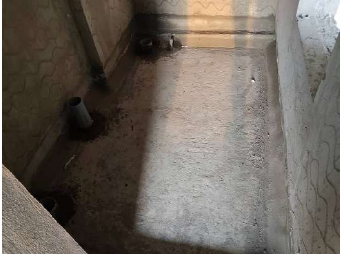
7F - Toilet Waterproofing
