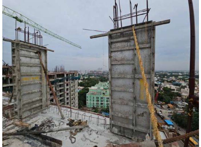
Twelfth Floor P1 - Column Concrete
