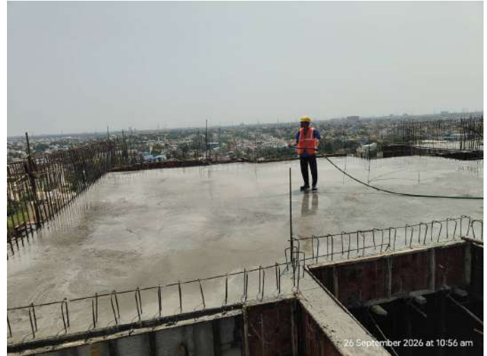
Twelfth Floor P2 - Roof Slab Concreting
