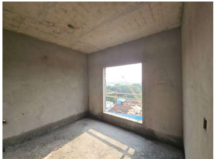
On Completion of Plastering - 6th Floor - 608
