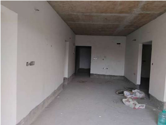
2F - Putty 1st Coat
