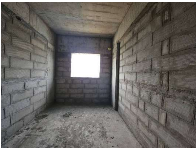
On Completion of Blockwork - 8th Floor - 813
