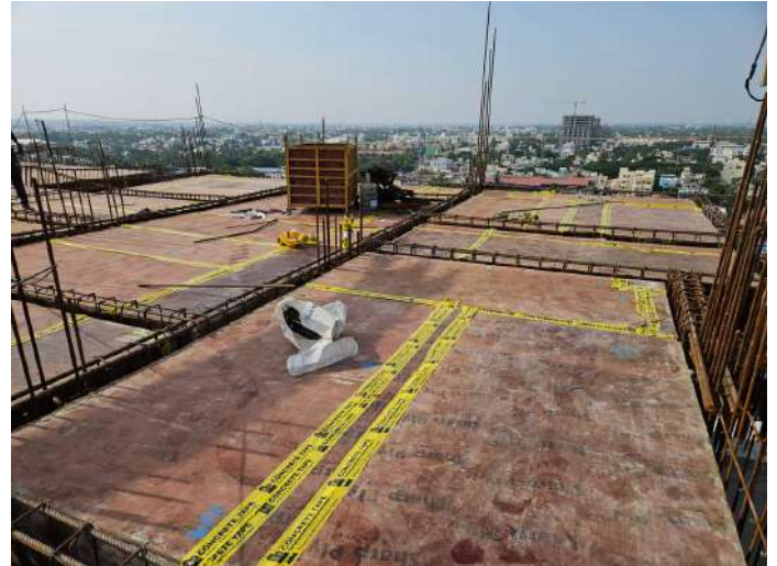
Twelfth Floor P1 - Roof Slab Shuttering
