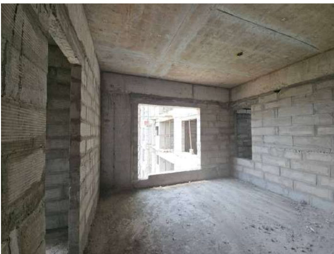
On Completion of Blockwork - 8th Floor - 813
