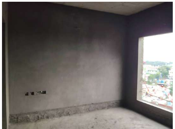
7F - Internal Plastering
