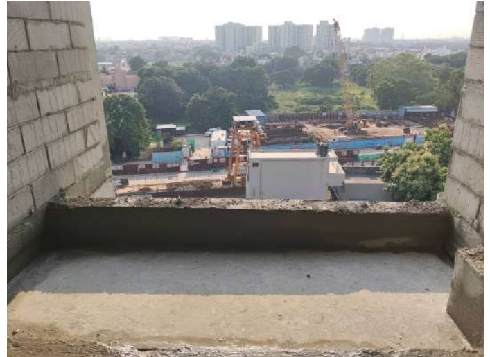
7F - Balcony Surface Cleaning
