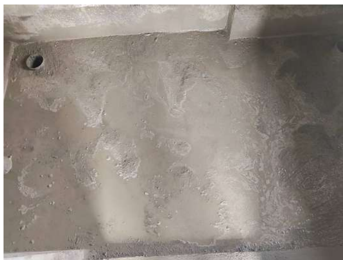
6F - Sunken Pipe Laying
