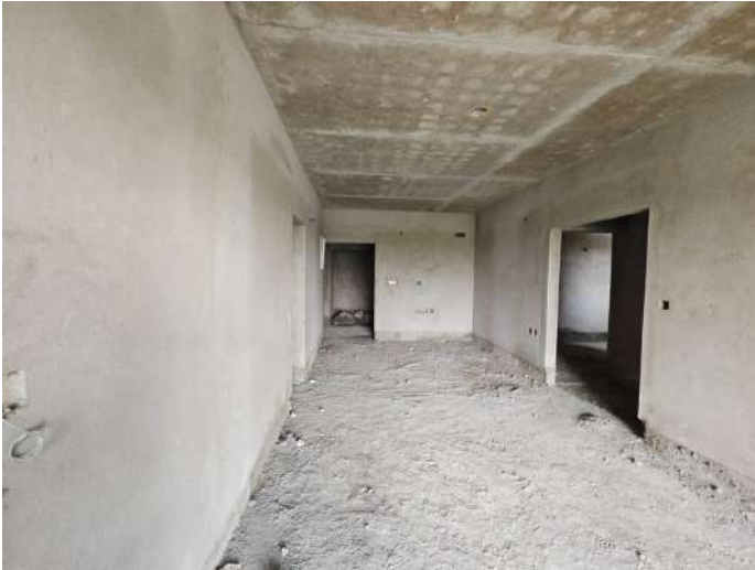
On Completion of Plastering - 6th Floor - 606
