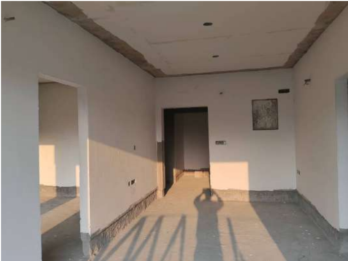
2F - Putty 1st Coat
