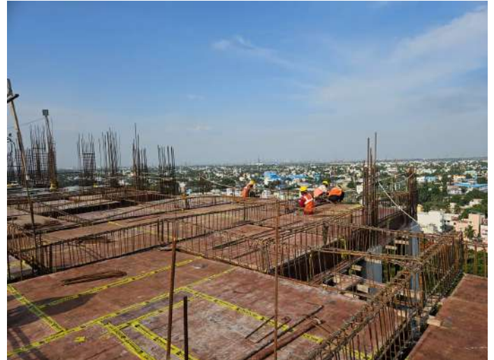
Eleventh Floor P2 - Slab & Beam Reinforcement
