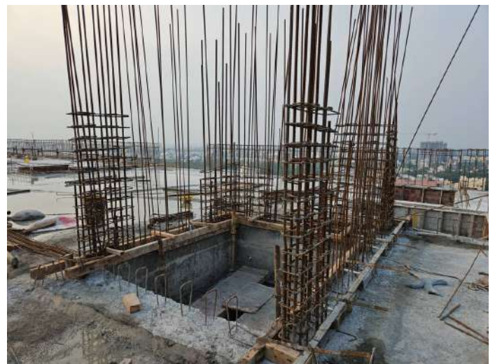
LMR - Reinforcement, Shuttering, Concreting
