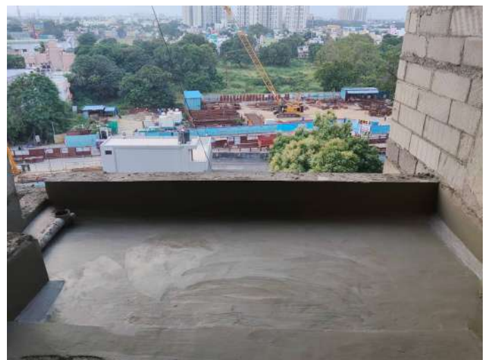
7F - Balcony Waterproofing
