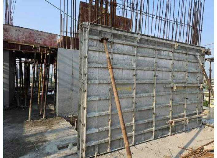
Twelfth Floor P1 - Column Shuttering
