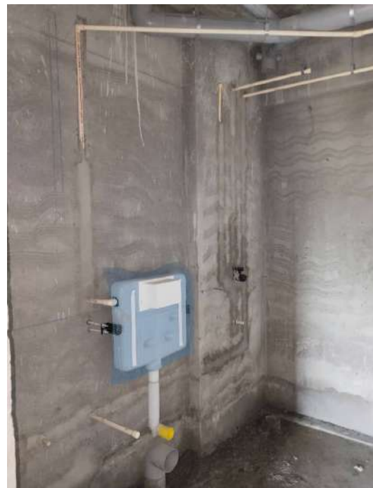
2F - Plumbing Packing & Protection
