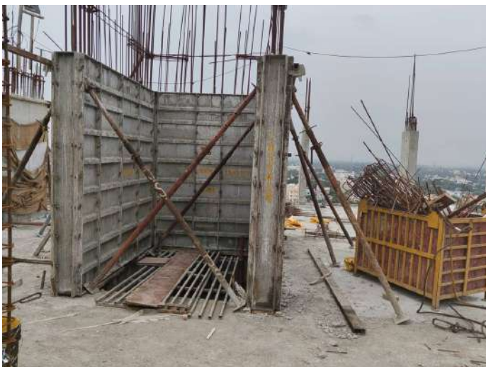
Twelfth Floor P1 - Column Shuttering
