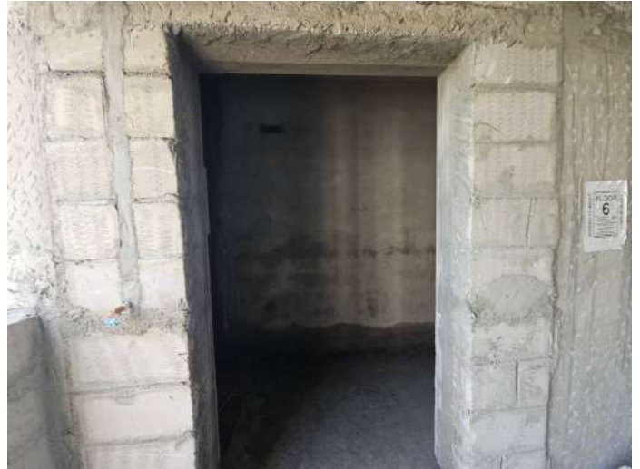
On Completion of Plastering - 6th Floor - 608
