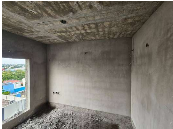
On Completion of Plastering - 6th Floor - 612
