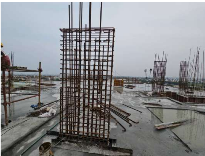
Twelfth Floor P2 - Col Marking & Reinforcement
