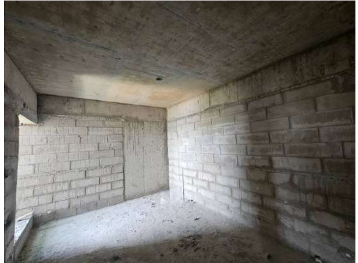
On Completion of Blockwork - 8th Floor - 802
