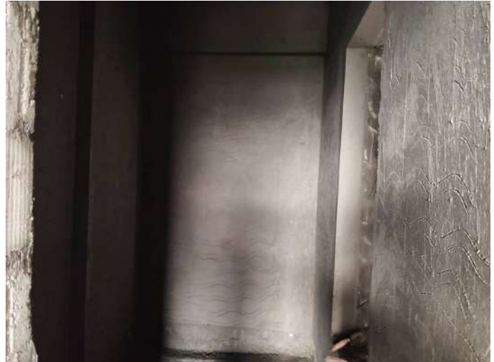
9F - Internal Plastering
