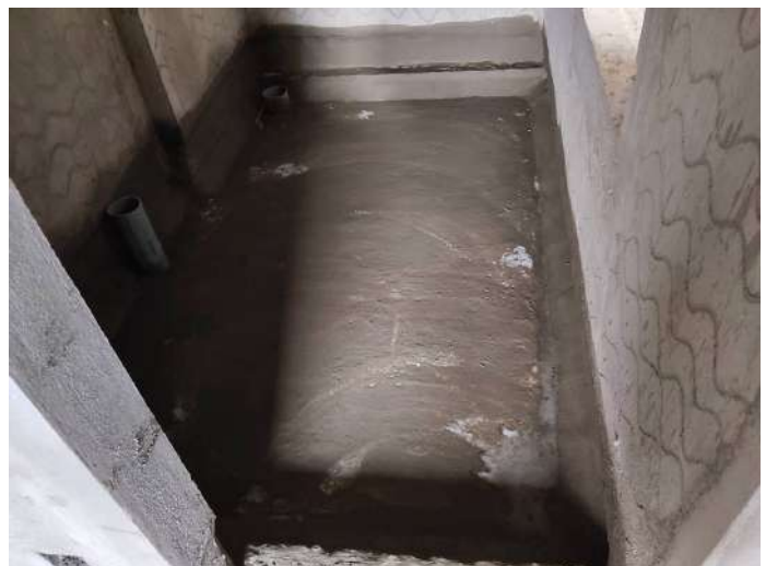
7F - Toilet Waterproofing
