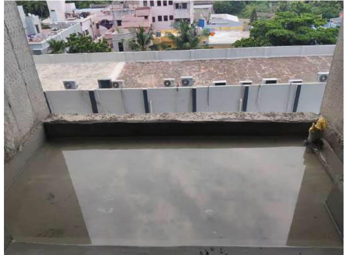
6F - Balcony Water Bond Test
