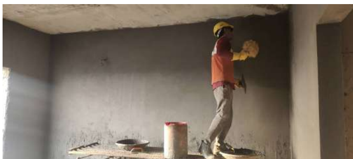
8F - Internal Plastering
