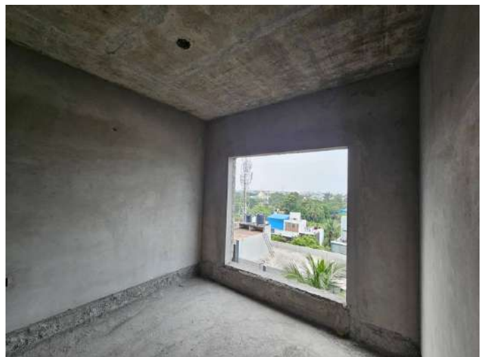
On Completion of Plastering - 6th Floor - 610
