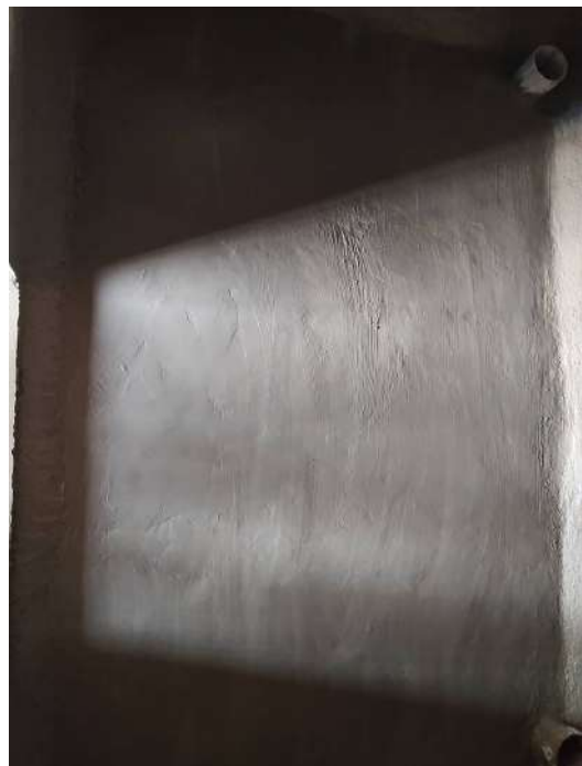
6F - Toilet Waterproofing
