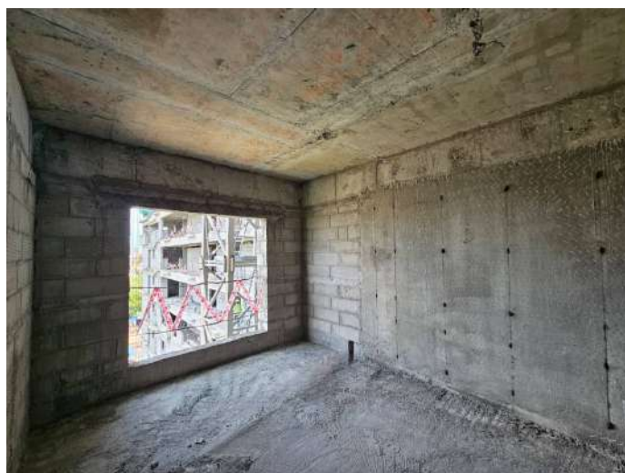
On Completion of Blockwork - 8th Floor - 807
