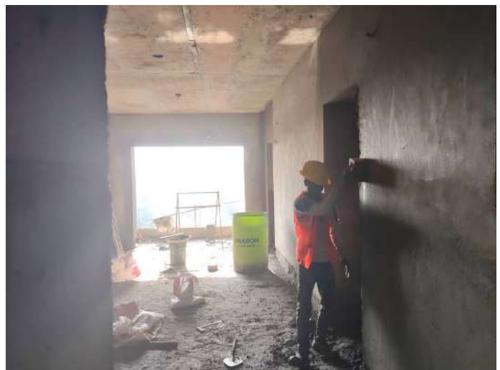
7F - Internal Plastering
