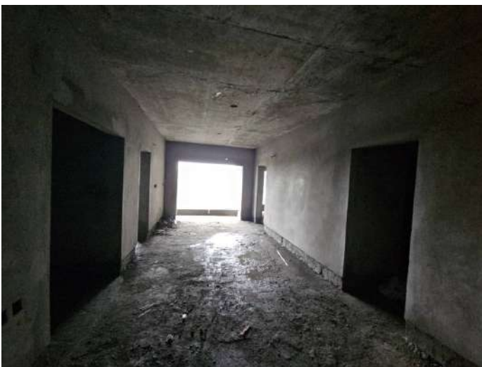
On Completion of Plastering - 6th Floor - 607
