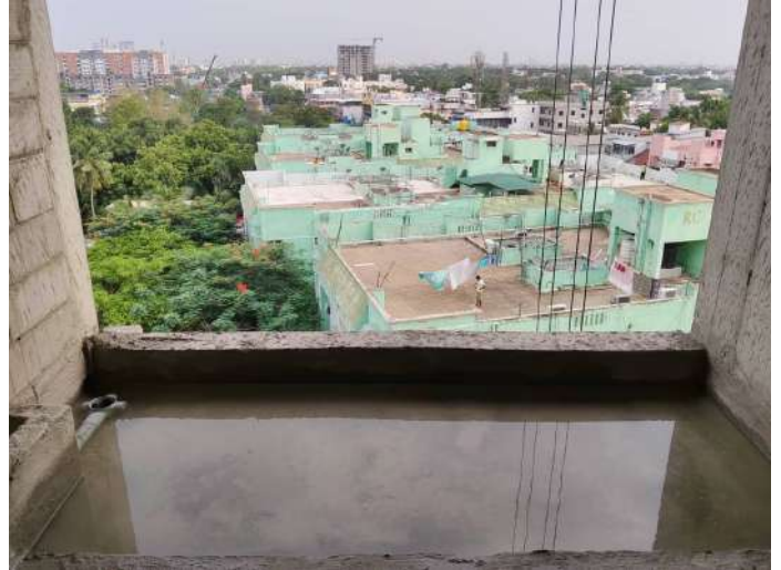
7F - Balcony Water Bond Test
