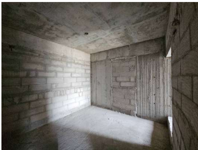
On Completion of Blockwork - 8th Floor - 811
