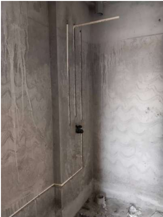
4F - Wall Concealed Pipe laying & Suspended Line
