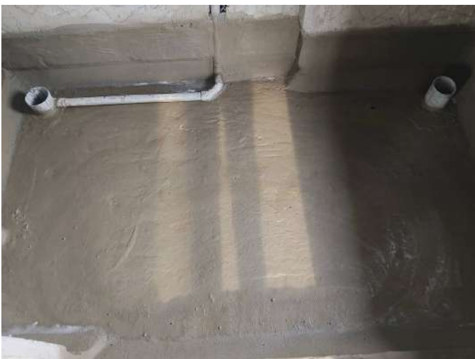
6F - Toilet Waterproofing
