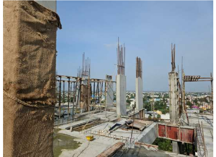
Twelfth Floor P2 - Column Concrete
