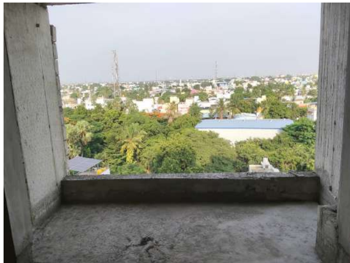
6F - Balcony Surface Cleaning
