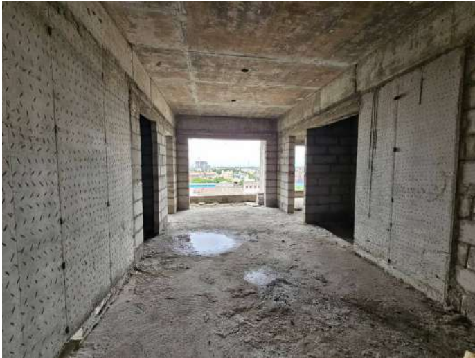
On Completion of Blockwork - 8th Floor - 810
