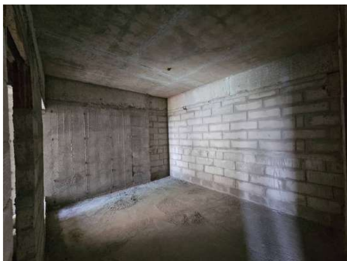
On Completion of Blockwork - 8th Floor - 807
