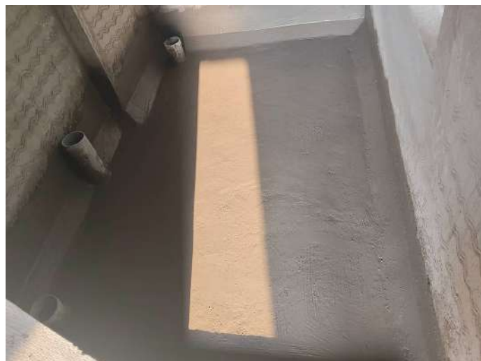
4F - Toilet Waterproofing
