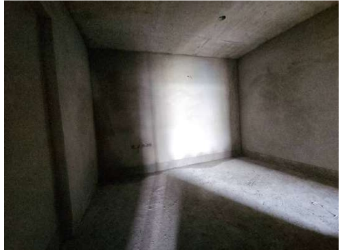
On Completion of Plastering - 6th Floor - 609
