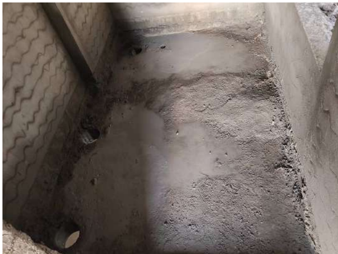
8F - Core& Wall Cutting
