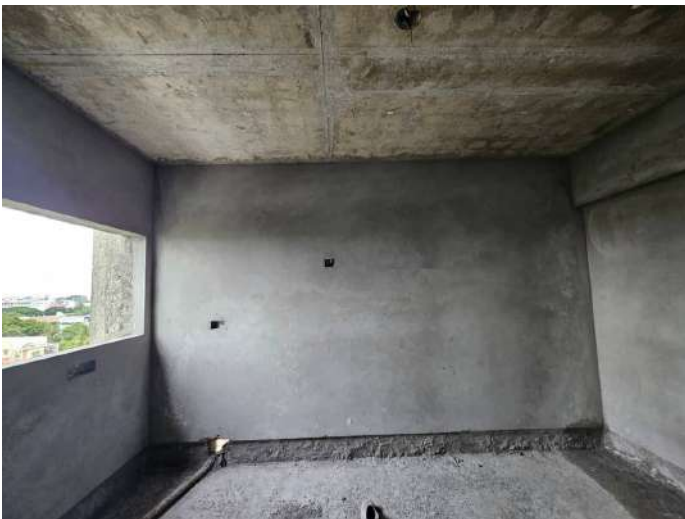
On Completion of Plastering - 6th Floor - 602
