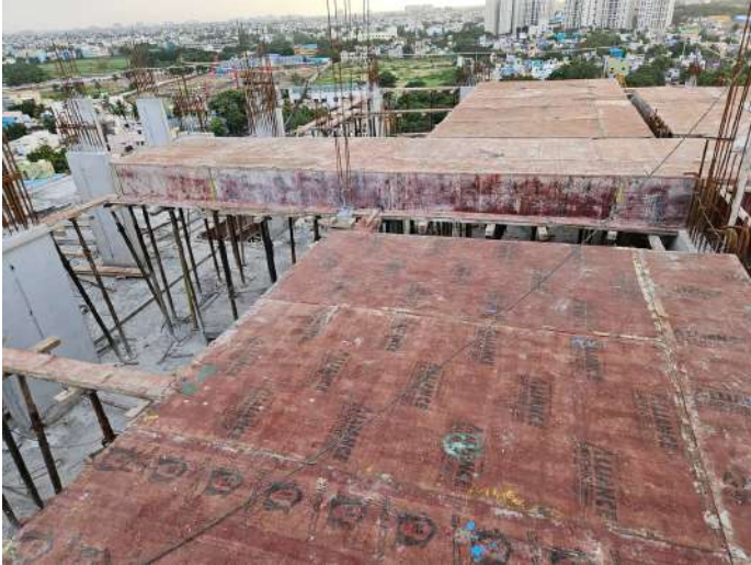
Eleventh Floor P2 - Roof Slab Shuttering
