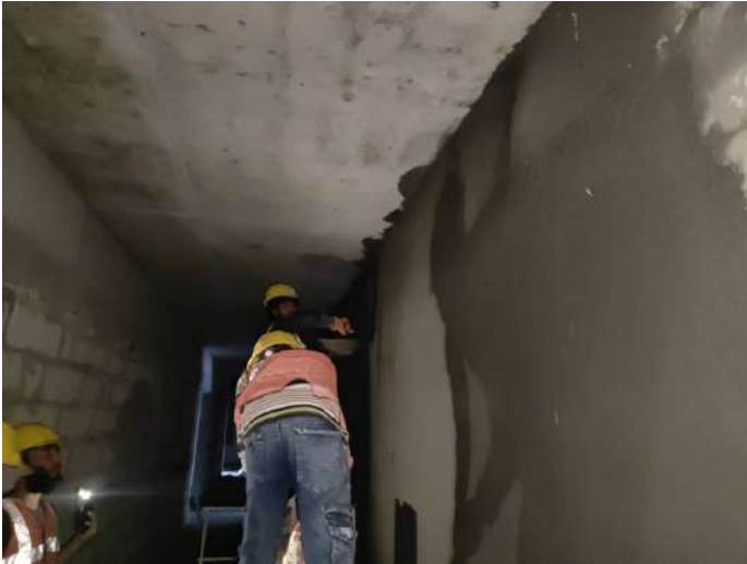
6F - Internal Plastering Corridor Area
