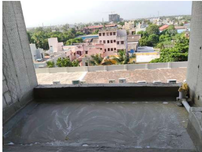
6F - Balcony Waterproofing
