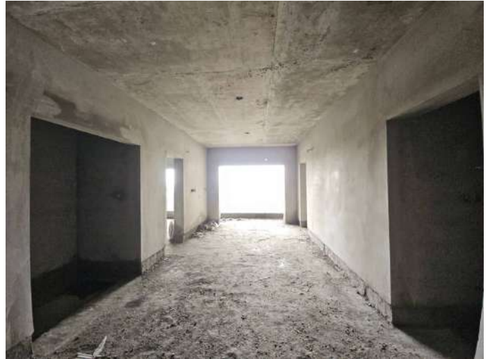
On Completion of Plastering - 6th Floor - 607
