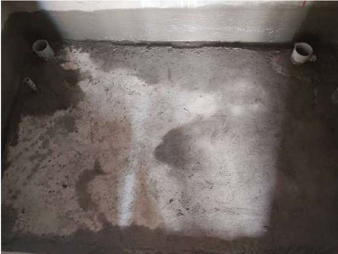
6F - Toilet Waterproofing
