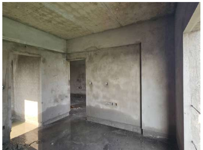
On Completion of Plastering - 6th Floor - 604
