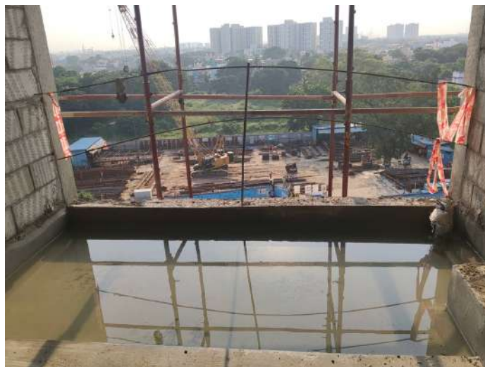
6F - Balcony Water Bond Test
