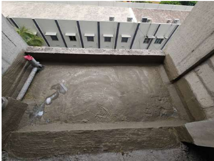
6F - Balcony Waterproofing
