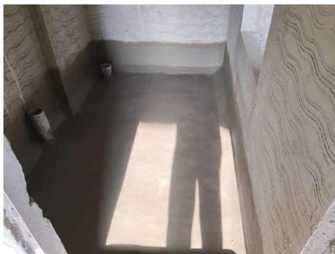
6F - Toilet Waterproofing
