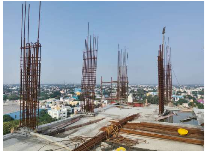
Twelfth Floor P1 - Col Marking & Reinforcement
