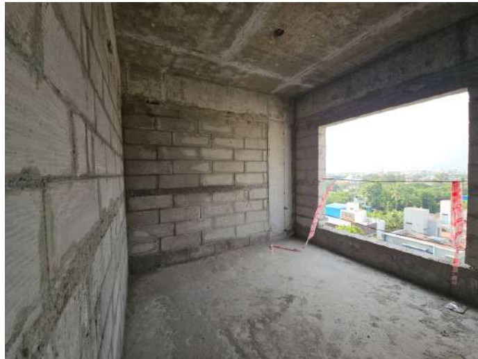
On Completion of Blockwork - 8th Floor - 811
