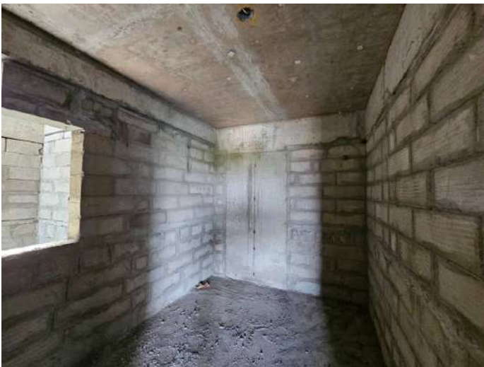
On Completion of Blockwork - 8th Floor - 812
