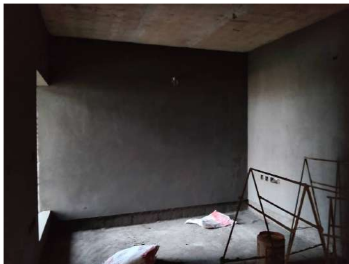
7F - Internal Plastering
