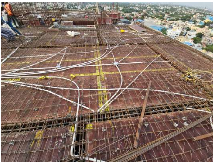
Twelfth Floor P2 - Slab & Beam Reinforcement
