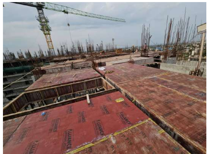
Eleventh Floor P2 - Roof Slab Shuttering
