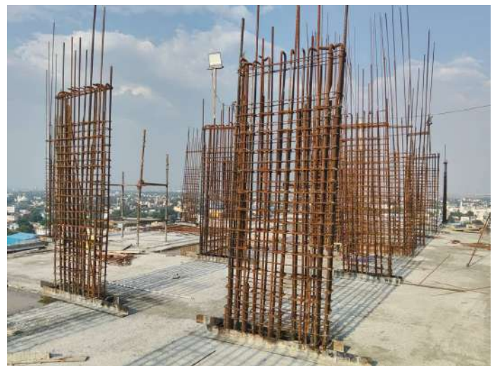
Twelfth Floor P1 - Col Marking & Reinforcement
