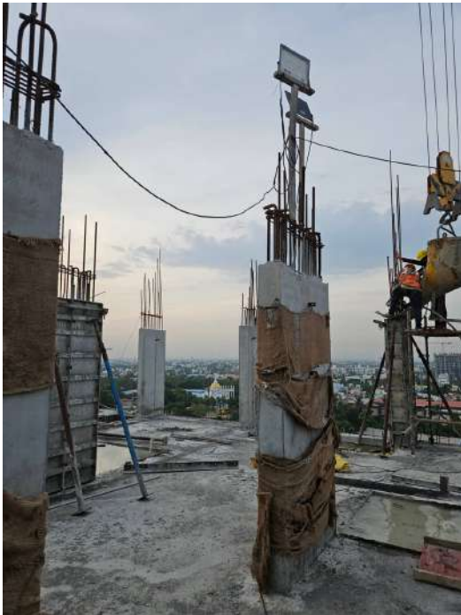
Twelfth Floor P1 - Column Concrete
