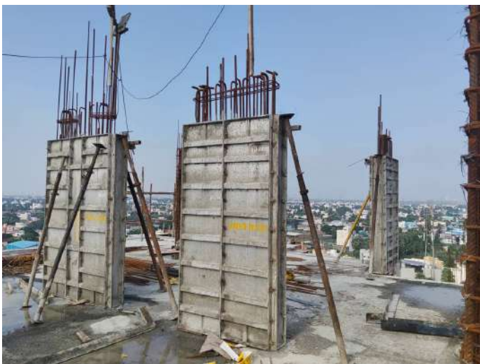
Twelfth Floor P1 - Column Shuttering
