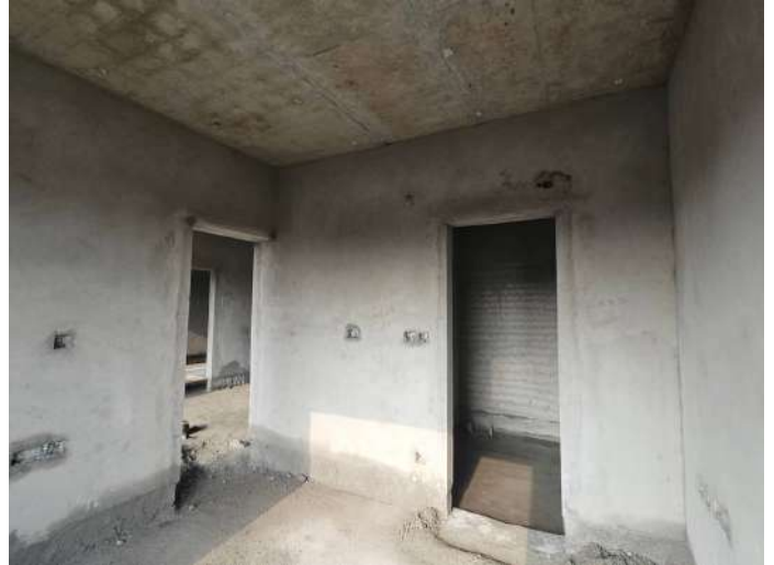
On Completion of Plastering - 7th Floor - 705
