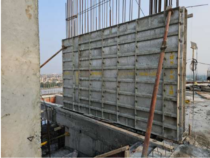
SHR - Column Shuttering
