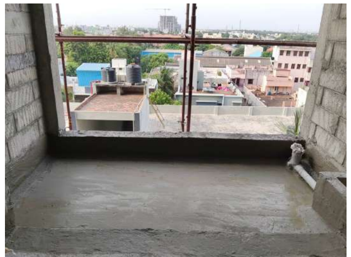
6F - Balcony Waterproofing
