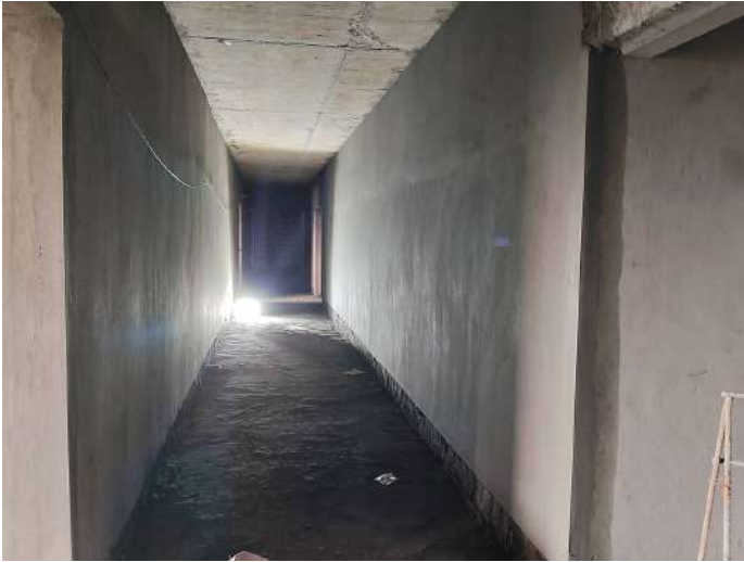
7F - Internal Plastering Corridor Area
