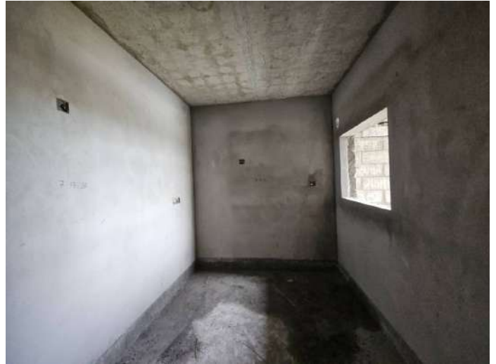
On Completion of Plastering - 6th Floor - 606
