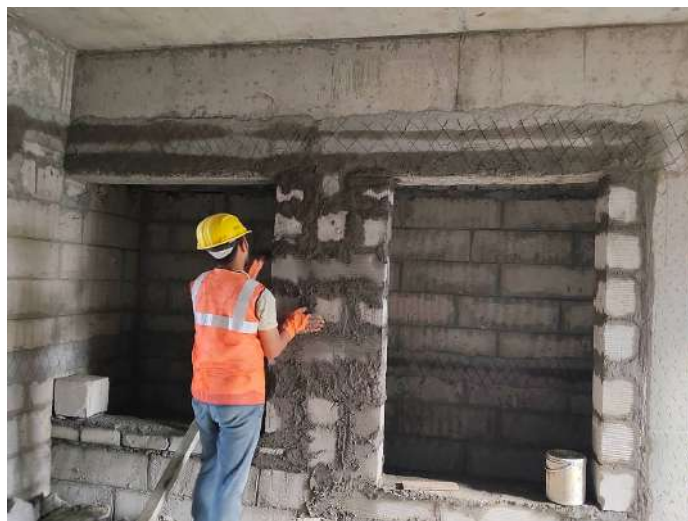
BW Corridor area - Sixth Floor
