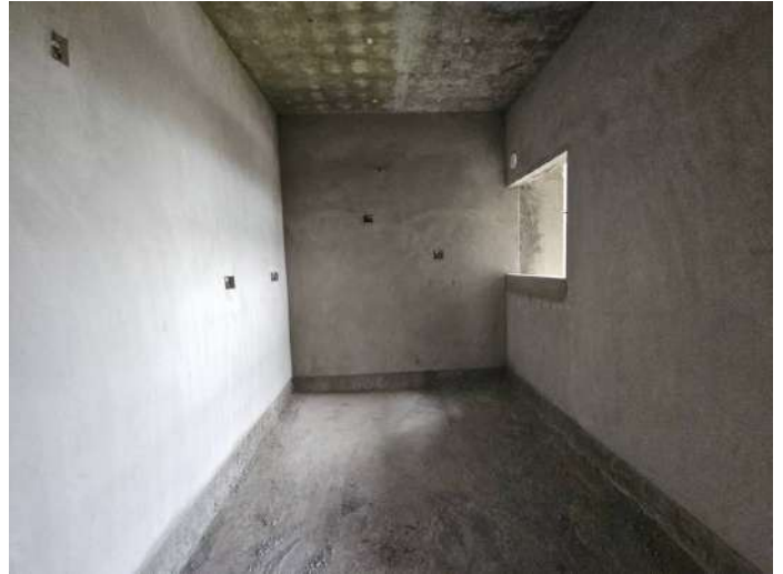
On Completion of Plastering - 6th Floor - 605
