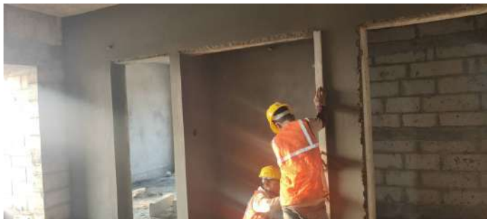
7F - Internal Plastering
