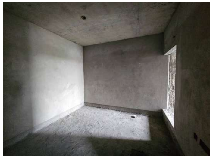
On Completion of Plastering - 6th Floor - 610
