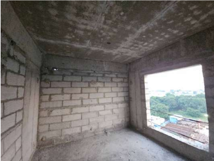
On Completion of Blockwork - 8th Floor - 808
