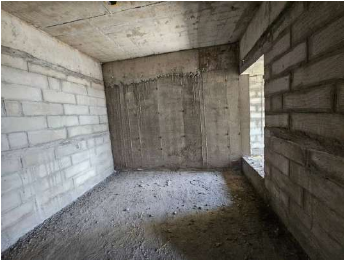
On Completion of Blockwork - 8th Floor - 812
