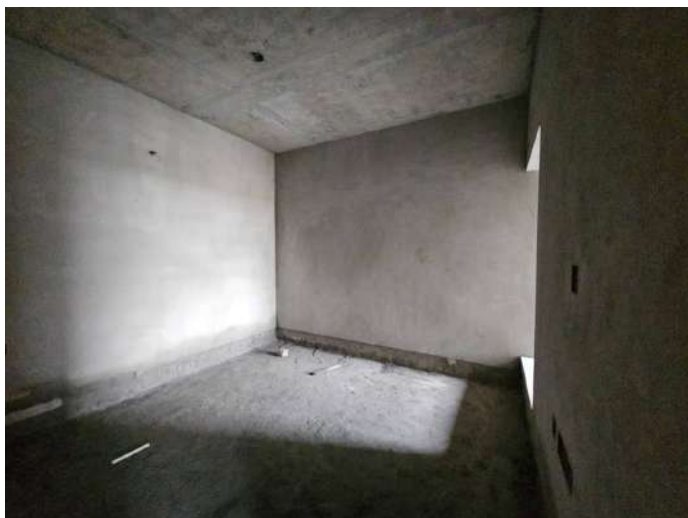
On Completion of Plastering - 6th Floor - 612
