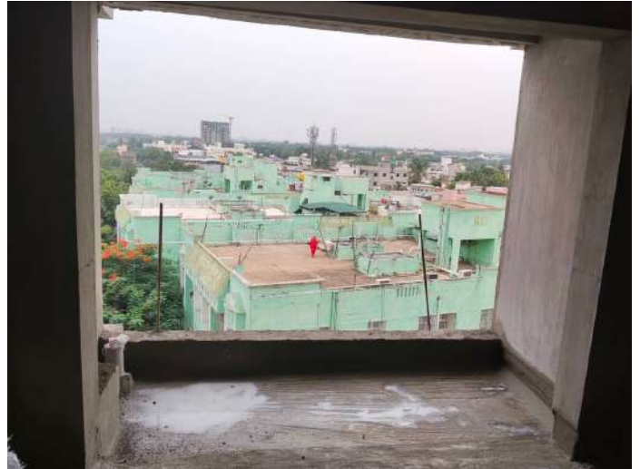
6F - Balcony Waterproofing
