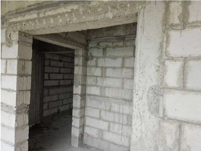
On Completion of Blockwork - 8th Floor - 809
