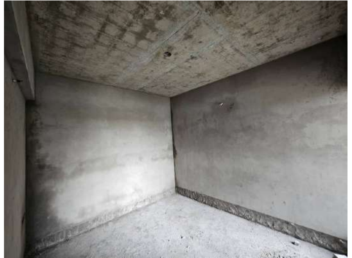
On Completion of Plastering - 6th Floor - 603
