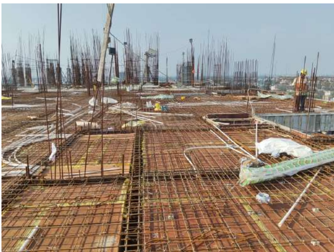
Eleventh Floor P2 - Slab & Beam Reinforcement
