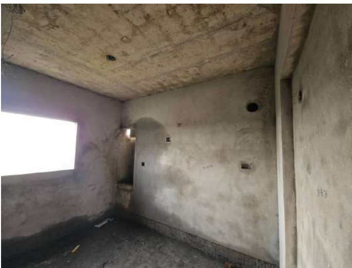
On Completion of Plastering - 6th Floor - 604
