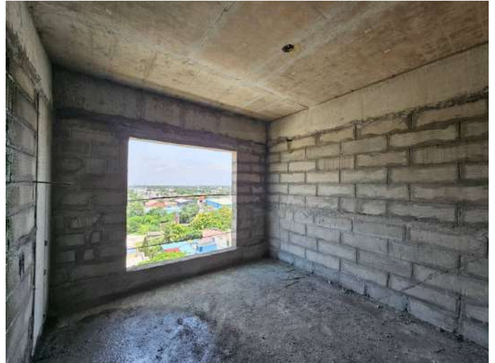
On Completion of Blockwork - 8th Floor - 812
