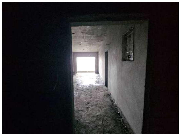
On Completion of Plastering - 6th Floor - 607
