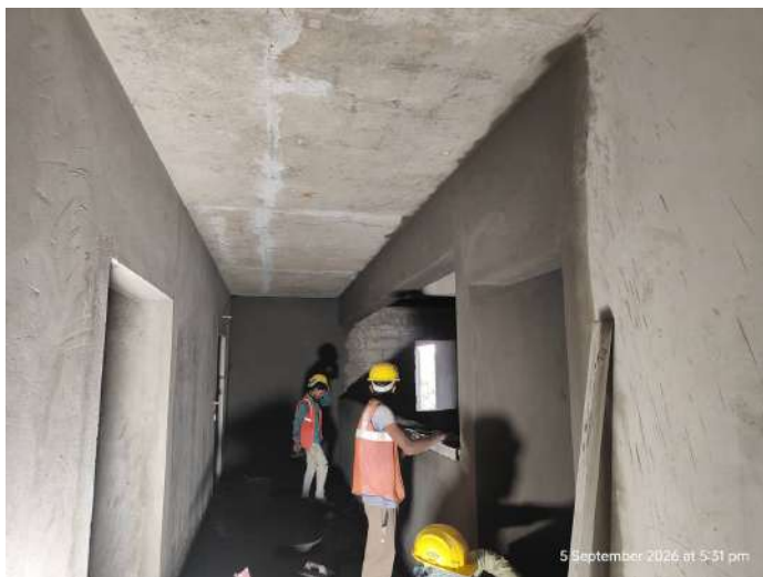
3F - Internal Plastering Corridor Area
