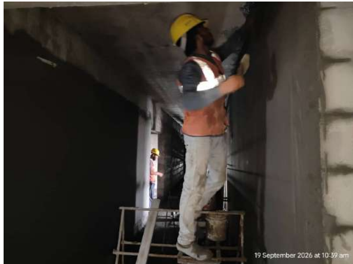
6F - Internal Plastering Corridor Area
