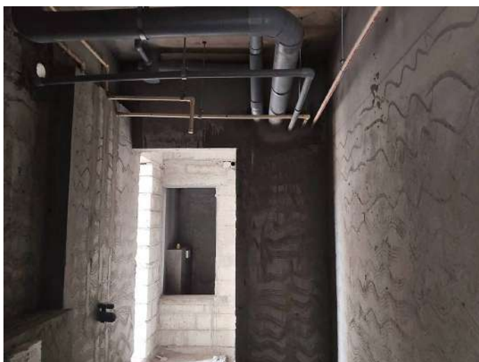
3F - Plumbing Packing & Protection
