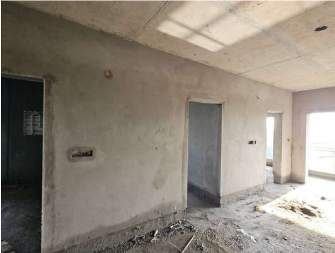
On Completion of Plastering - 6th Floor - 608
