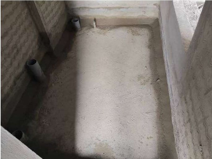
7F - Toilet Waterproofing
