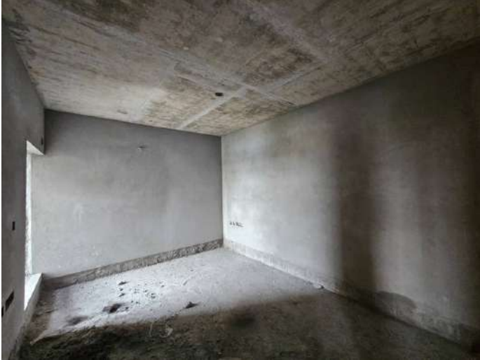
On Completion of Plastering - 6th Floor - 602
