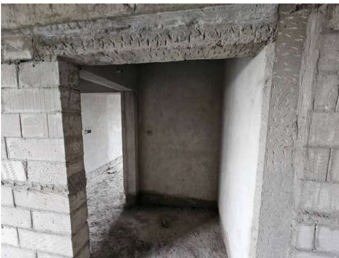
On Completion of Plastering - 6th Floor - 611
