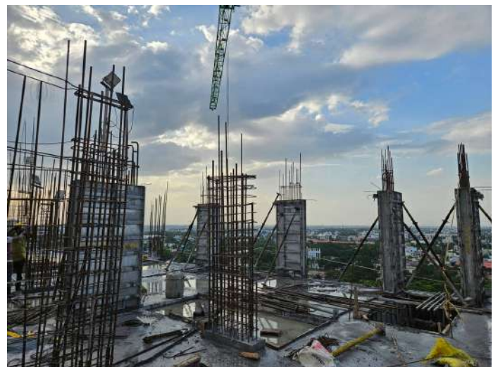
Twelfth Floor P1 - Column Shuttering
