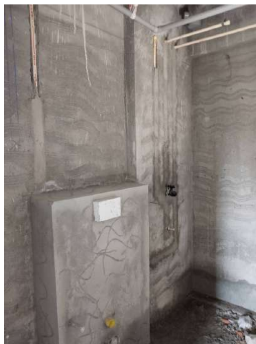
3F - Plumbing Packing & Protection
