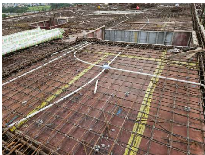
Twelfth Floor P1 - Roof Slab Shuttering
