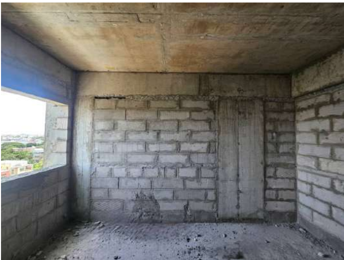
On Completion of Blockwork - 8th Floor - 802
