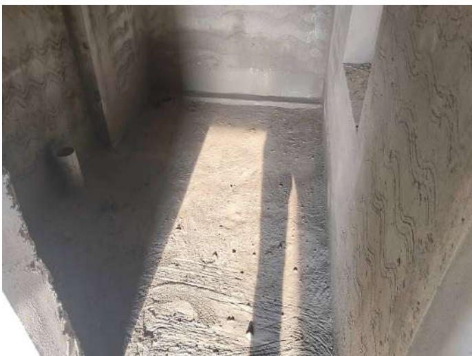
6F - Sunken Pipe Laying
