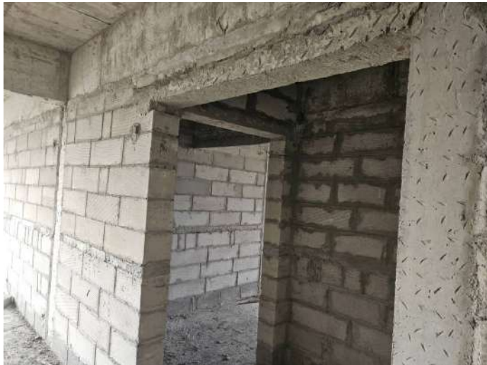
On Completion of Blockwork - 8th Floor - 811
