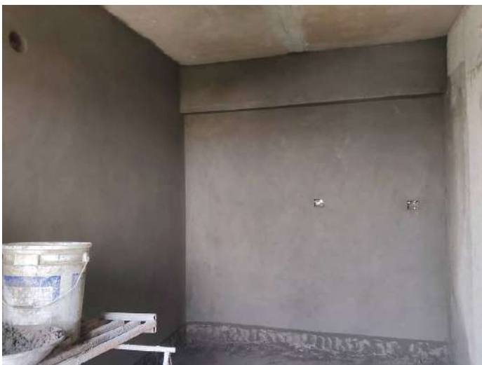
7F - Internal Plastering
