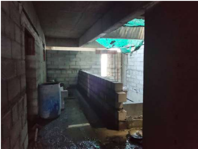
BW Corridor area - Ninth Floor
