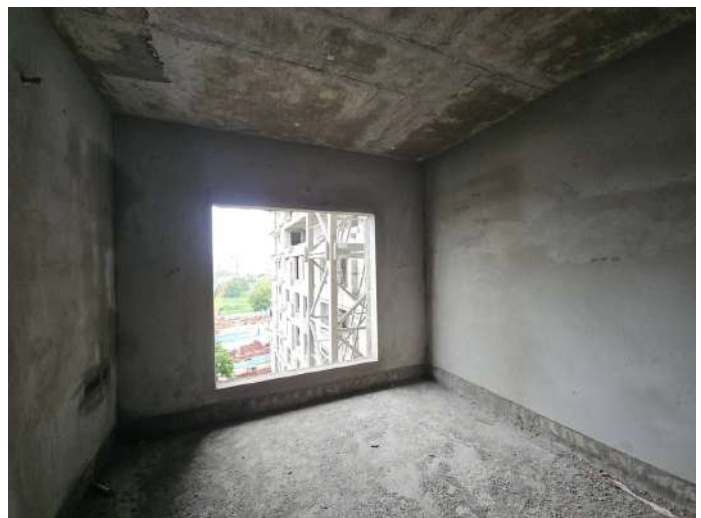
On Completion of Plastering - 6th Floor - 607
