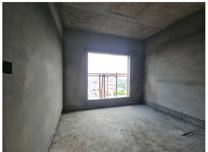
On Completion of Plastering - 6th Floor - 609
