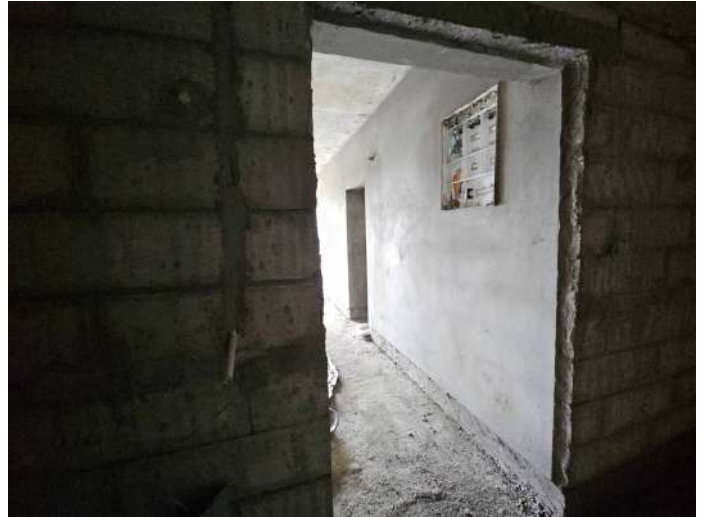
On Completion of Plastering - 6th Floor - 606
