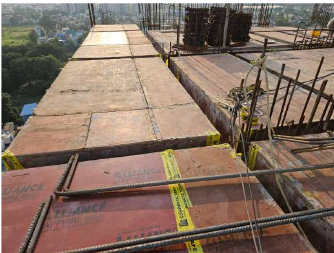
Twelfth Floor P1 - Roof Slab Shuttering
