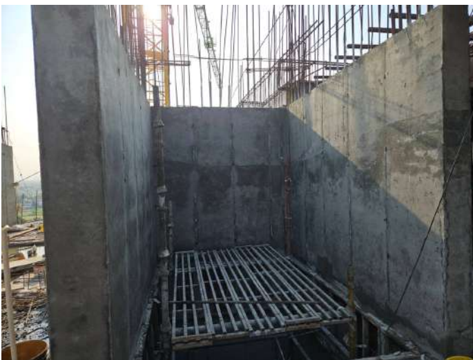
Twelfth Floor P1 - Column Concrete
