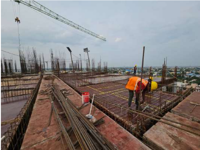
Eleventh Floor P2 - Slab & Beam Reinforcement
