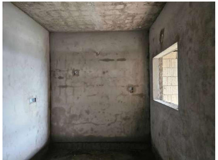
On Completion of Plastering - 6th Floor - 607
