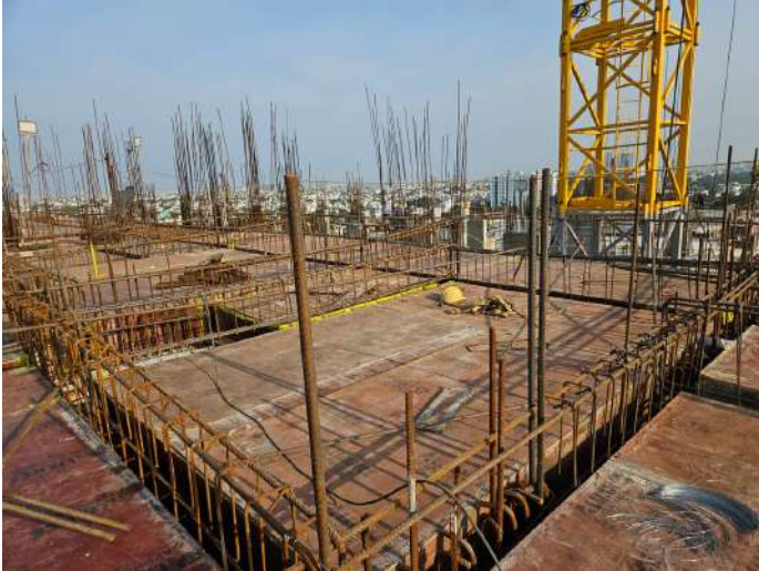
Twelfth Floor P1 - Slab & Beam Reinforcement
