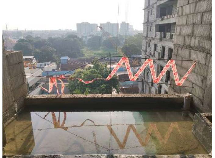
6F - Balcony Water Bond Test
