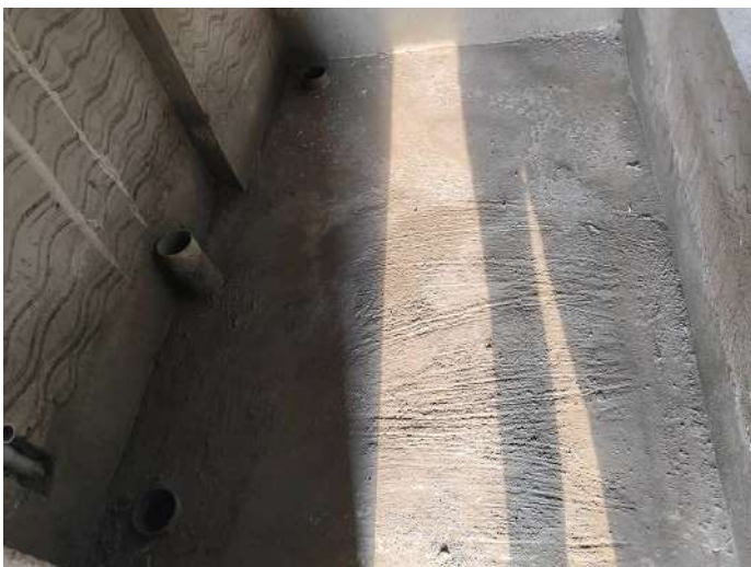
6F - Sunken Pipe Laying
