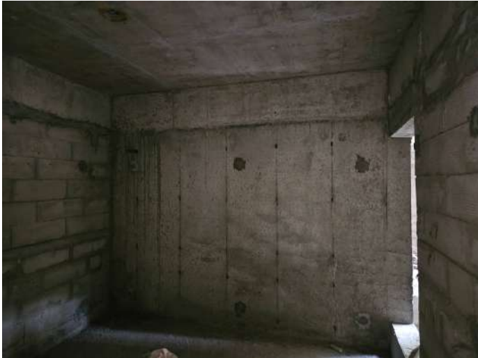
On Completion of Blockwork - 8th Floor - 801
