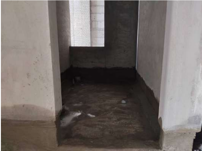
6F - Toilet Waterproofing
