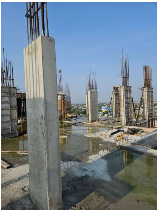
Twelfth Floor P2 - Column Concrete
