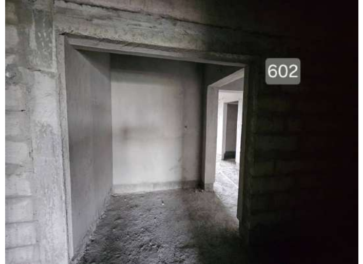
On Completion of Plastering - 6th Floor - 602
