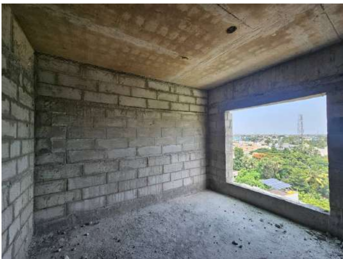
On Completion of Blockwork - 8th Floor - 802
