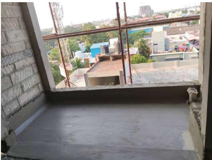
6F - Balcony Waterproofing
