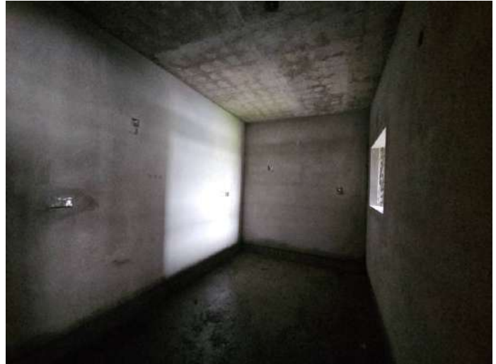
On Completion of Plastering - 6th Floor - 607
