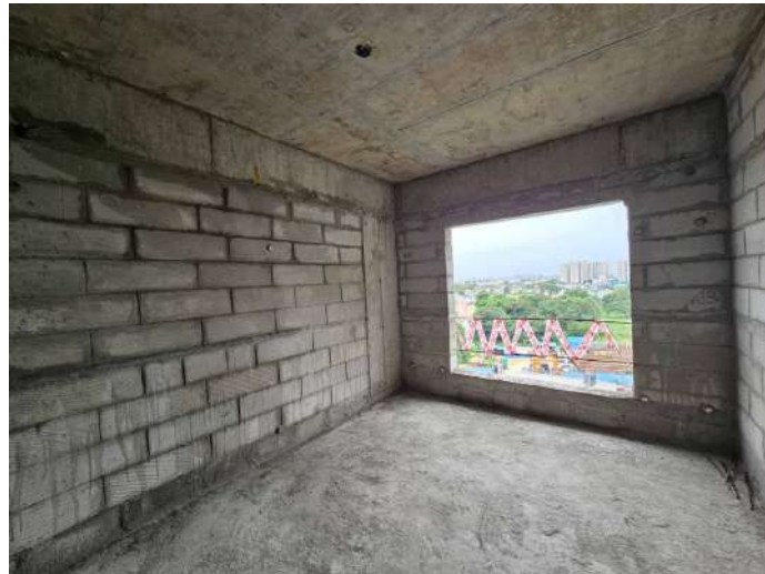
On Completion of Blockwork - 8th Floor - 806
