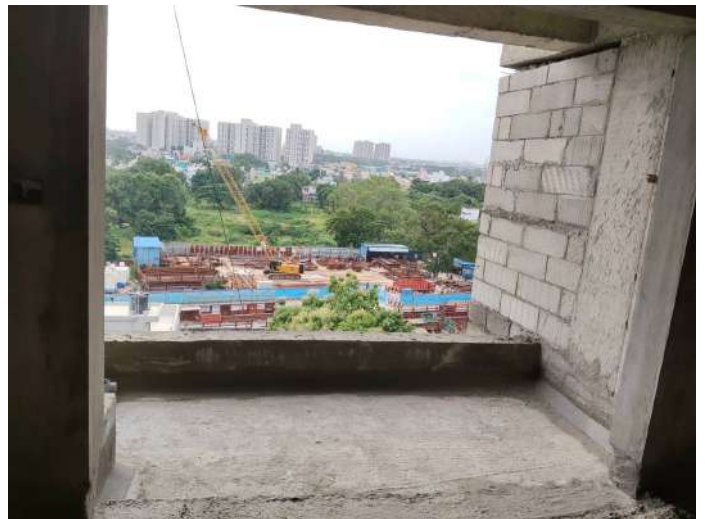
7F - Balcony Waterproofing
