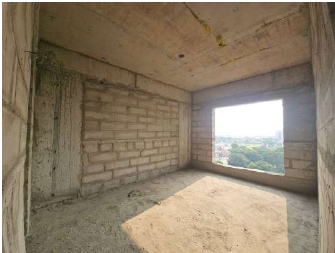
On Completion of Blockwork - 9th Floor - 906
