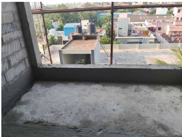
6F - Balcony Waterproofing
