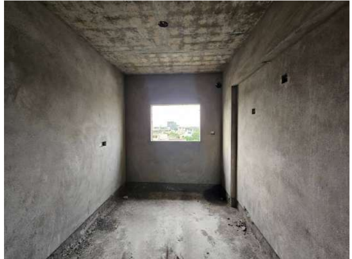
On Completion of Plastering - 6th Floor - 613
