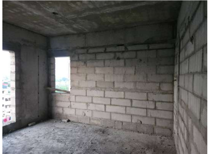
On Completion of Blockwork - 8th Floor - 808
