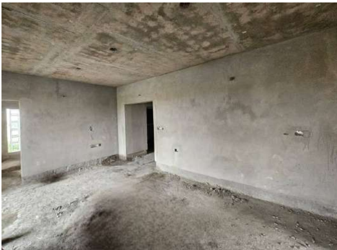
On Completion of Plastering - 6th Floor - 613
