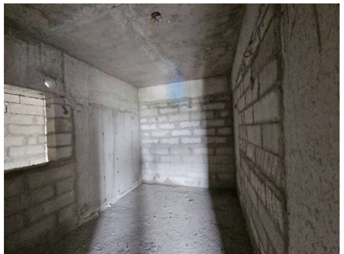
On Completion of Blockwork - 8th Floor - 809
