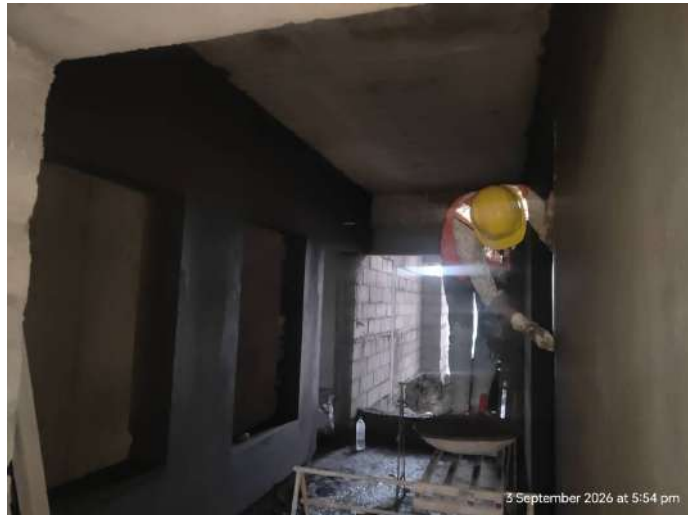
5F - Internal Plastering Corridor Area
