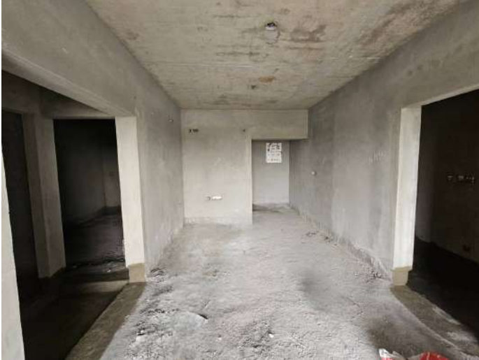
On Completion of Plastering - 6th Floor - 611
