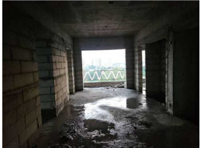
On Completion of Blockwork - 8th Floor - 808
