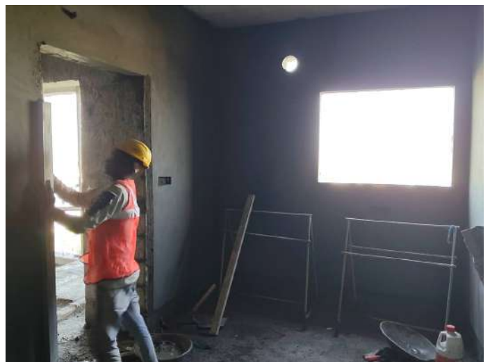
7F - Internal Plastering
