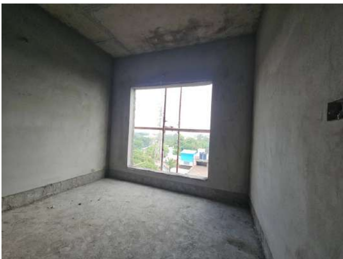
On Completion of Plastering - 6th Floor - 609
