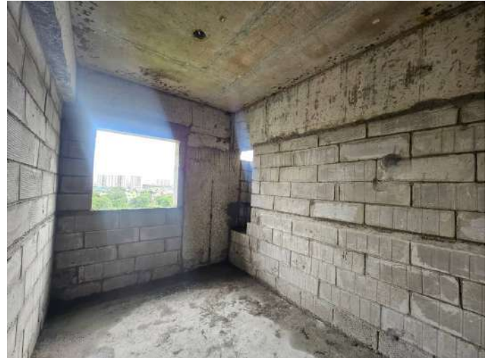
On Completion of Blockwork - 8th Floor - 804
