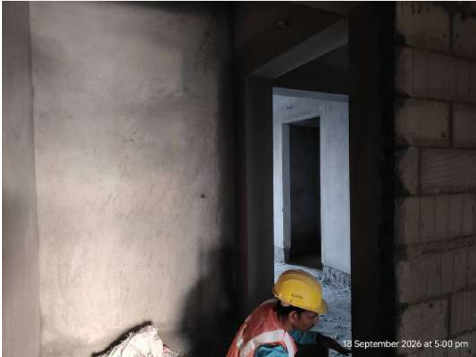
7F - Internal Plastering
