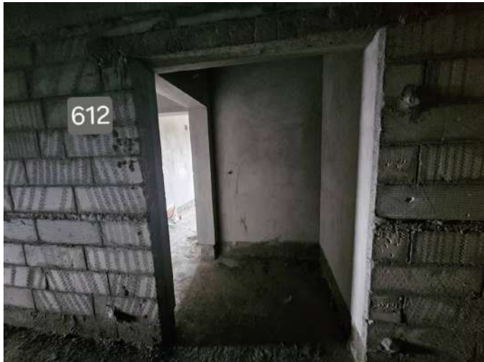
On Completion of Plastering - 6th Floor - 612
