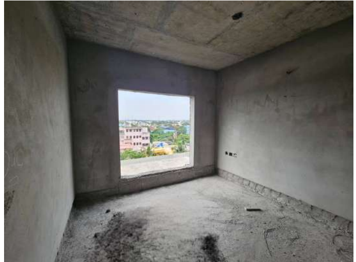
On Completion of Plastering - 6th Floor - 610
