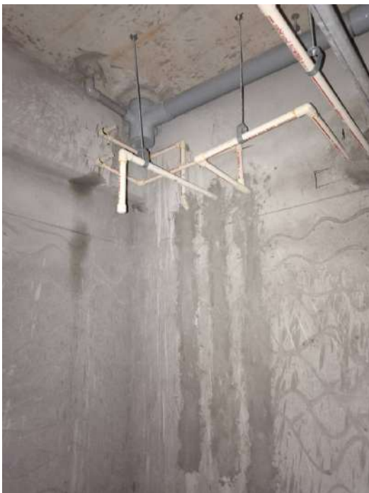
3F - Plumbing Packing & Protection
