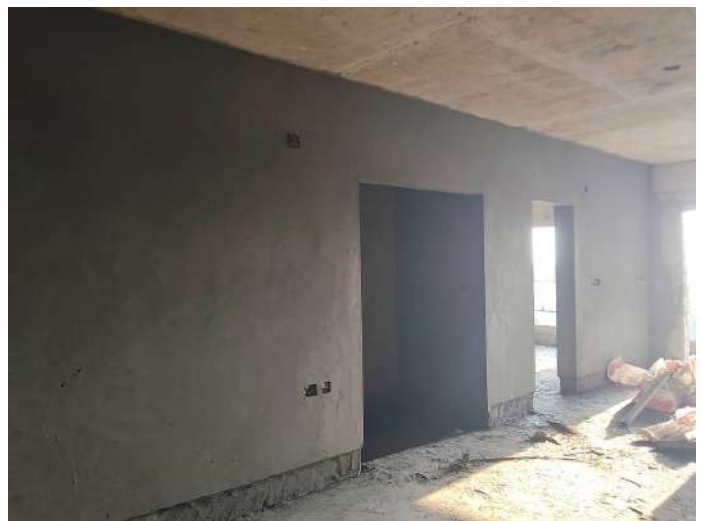
7F - Internal Plastering
