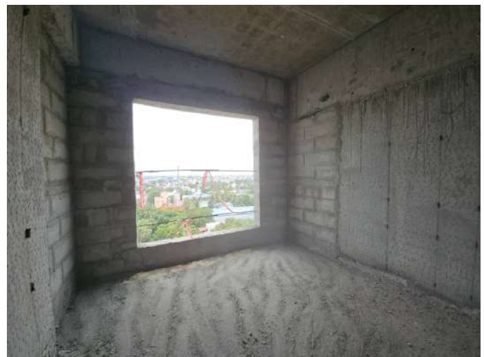
On Completion of Blockwork - 8th Floor - 813
