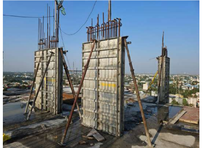
Twelfth Floor P1 - Column Shuttering
