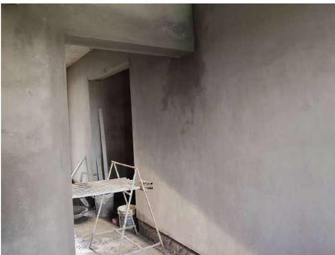
6F - Internal Plastering Corridor Area
