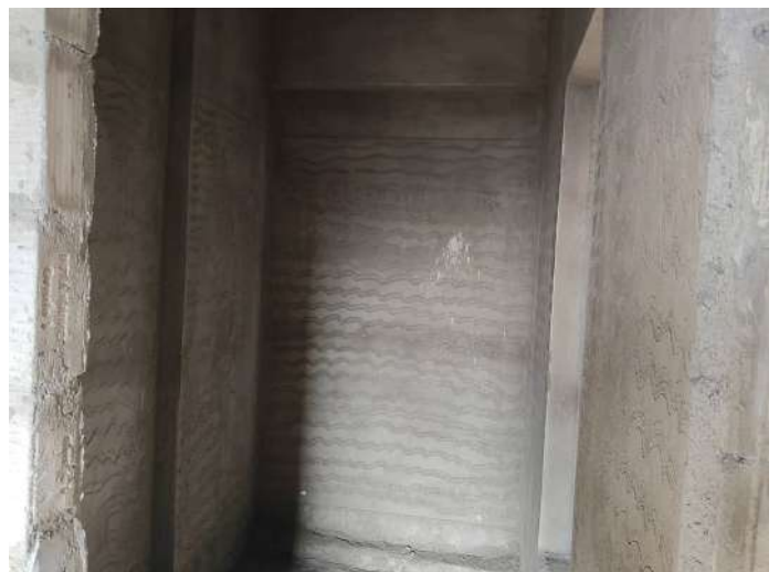
8F - Internal Plastering
