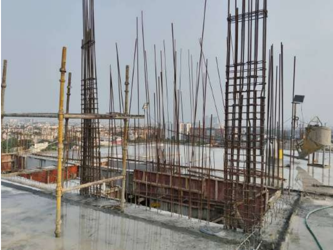
SHR - Col Marking & Reinforcement
