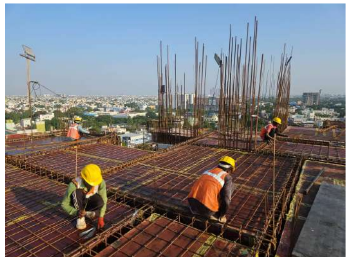
Eleventh Floor P2 - Slab & Beam Reinforcement
