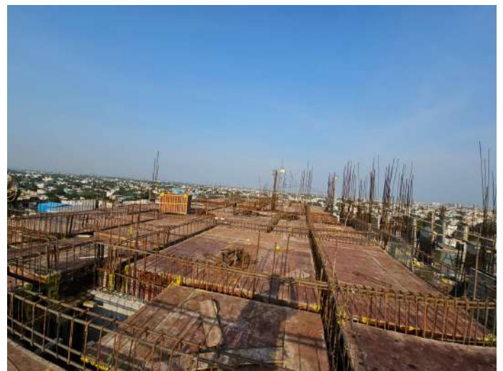
Twelfth Floor P1 - Roof Slab Shuttering
