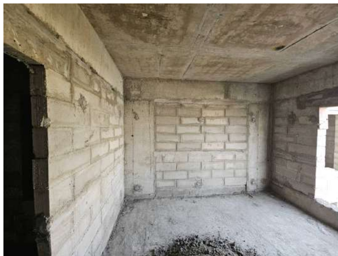
On Completion of Blockwork - 8th Floor - 801
