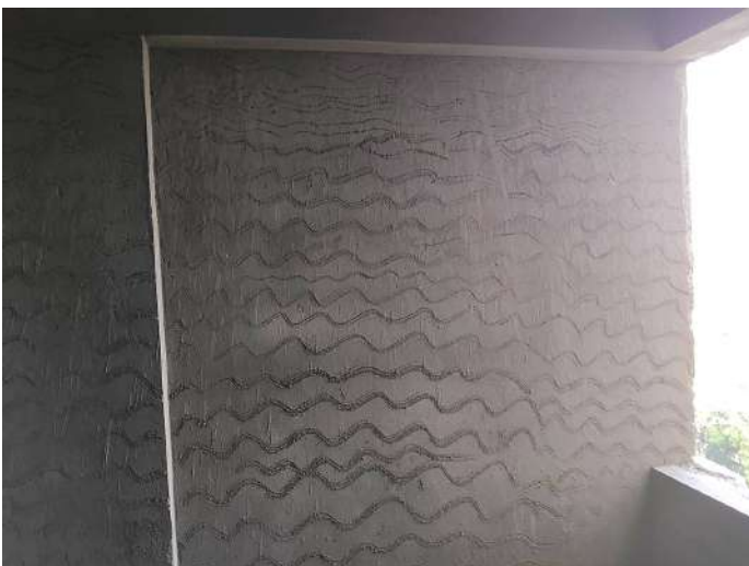
7F - Internal Plastering
