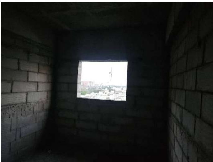
On Completion of Blockwork - 8th Floor - 808
