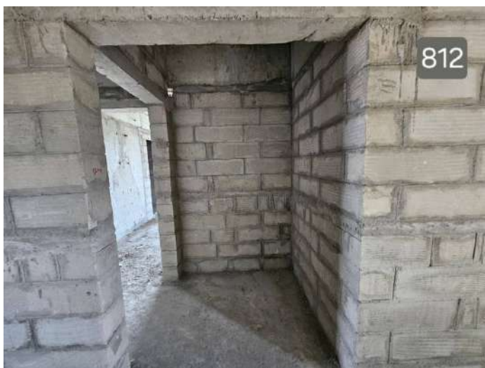
On Completion of Blockwork - 8th Floor - 812
