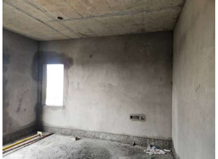
On Completion of Plastering - 6th Floor - 608
