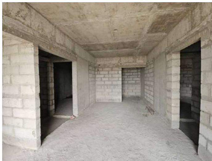
On Completion of Blockwork - 8th Floor - 811
