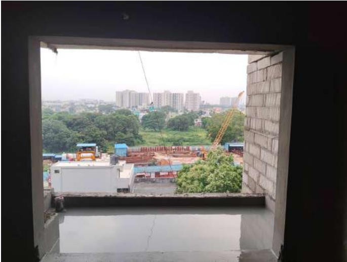
6F - Balcony Water Bond Test
