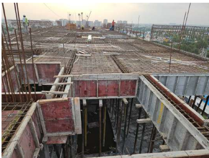
Twelfth Floor P1 - Roof Slab Shuttering
