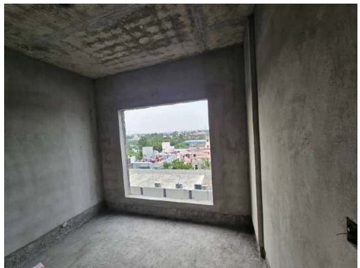
On Completion of Plastering - 6th Floor - 612
