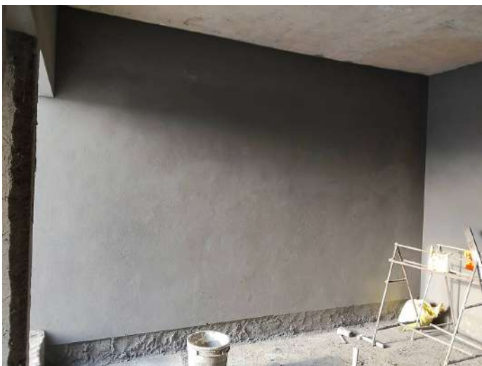
7F - Internal Plastering
