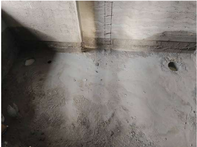
7F - Core& Wall Cutting
