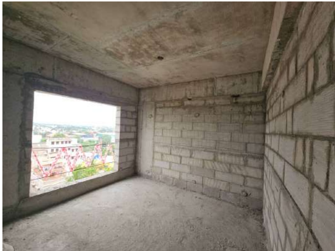
On Completion of Blockwork - 8th Floor - 809
