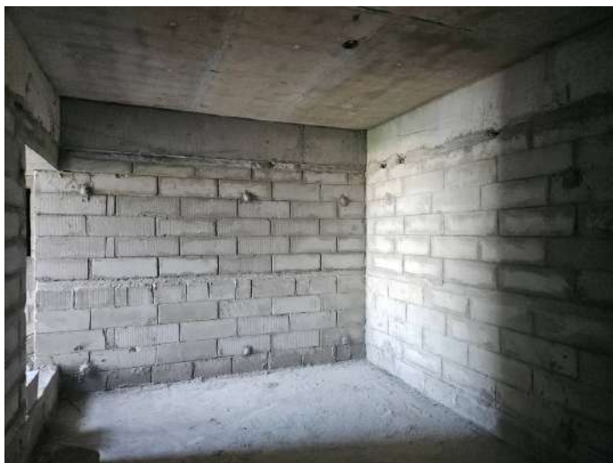
On Completion of Blockwork - 8th Floor - 801
