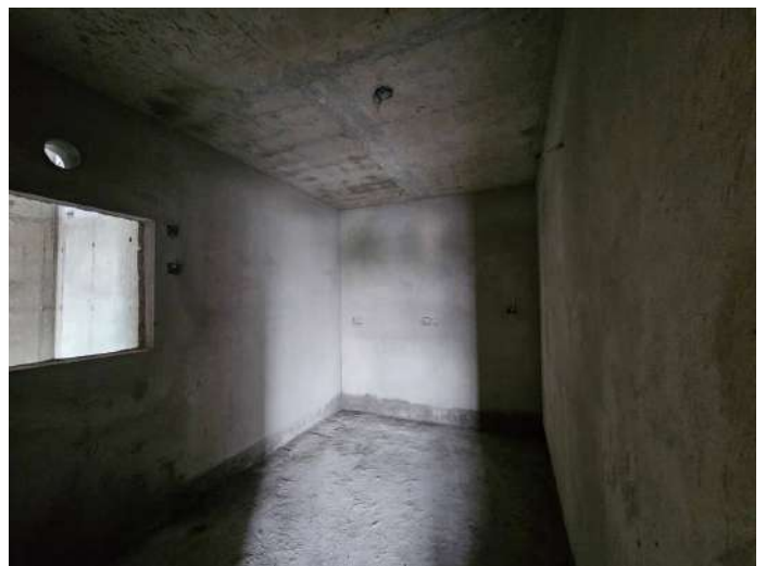
On Completion of Plastering - 6th Floor - 611
