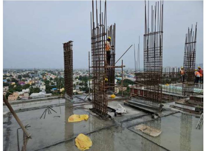
Twelfth Floor P2 - Col Marking & Reinforcement
