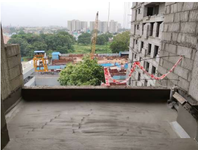
6F - Balcony Waterproofing
