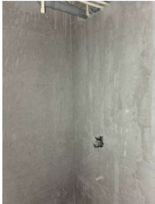
4F - Wall Concealed Pipe laying & Suspended Line
