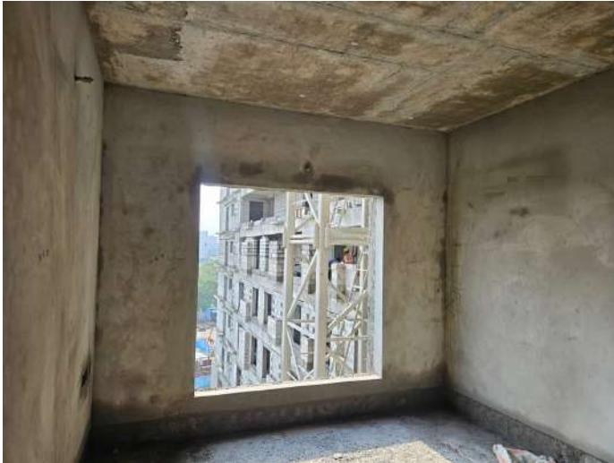
On Completion of Plastering - 6th Floor - 607
