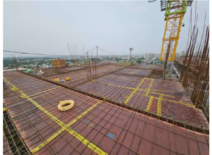
Twelfth Floor P2 - Roof Slab Shuttering
