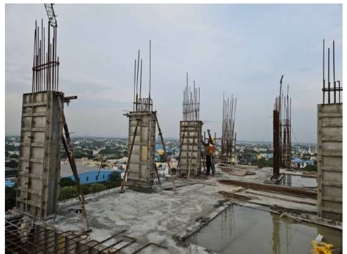
Twelfth Floor P1 - Column Shuttering
