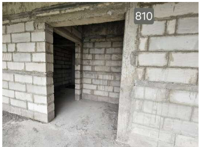
On Completion of Blockwork - 8th Floor - 810
