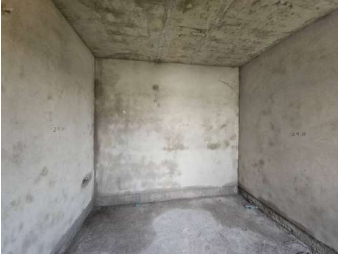
On Completion of Plastering - 6th Floor - 604
