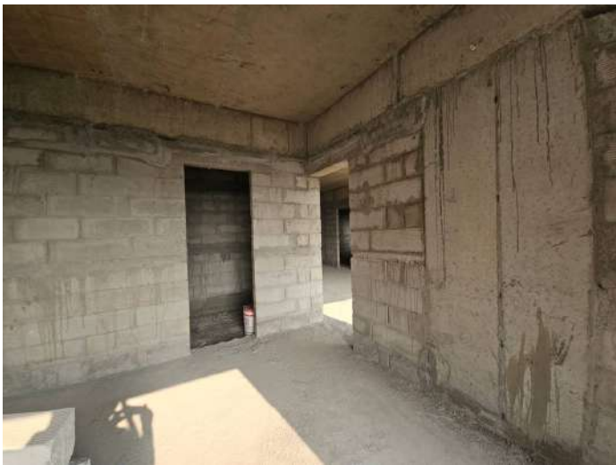
On Completion of Blockwork - 9th Floor - 906
