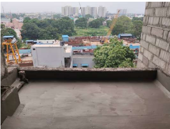
6F - Balcony Waterproofing
