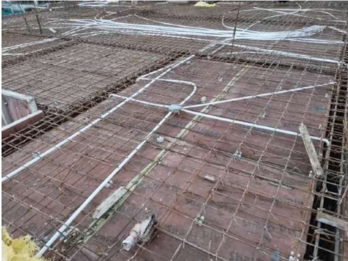
Eleventh Floor P2 - Electrical - Conduit Laying
