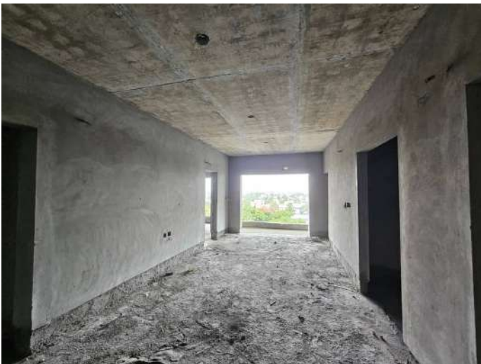
On Completion of Plastering - 6th Floor - 602
