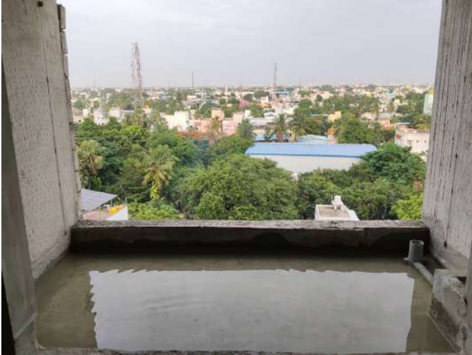
7F - Balcony Water Bond Test
