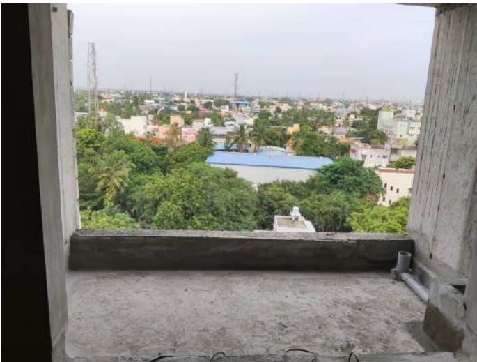
7F - Balcony Surface Cleaning
