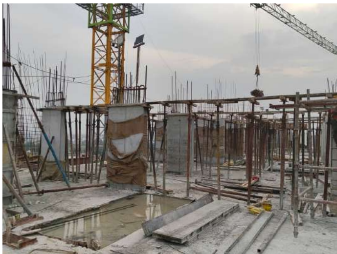
Twelfth Floor P1 - Roof Slab Shuttering
