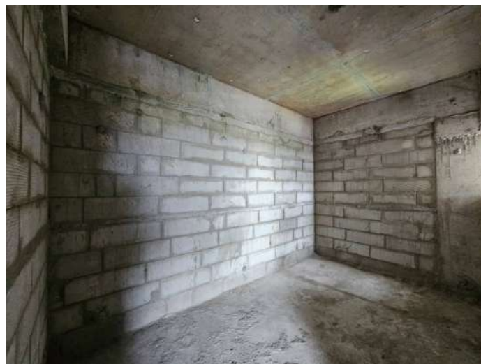
On Completion of Blockwork - 8th Floor - 806
