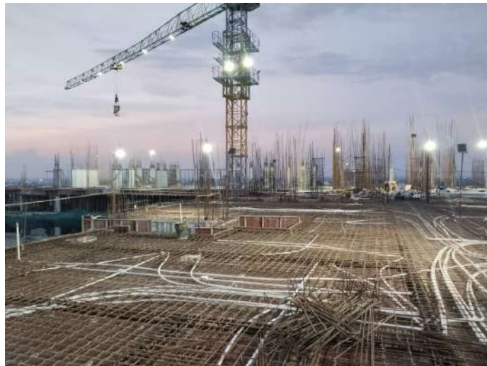
Eleventh Floor P2 - Electrical - Conduit Laying
