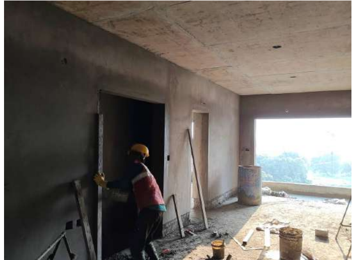
7F - Internal Plastering
