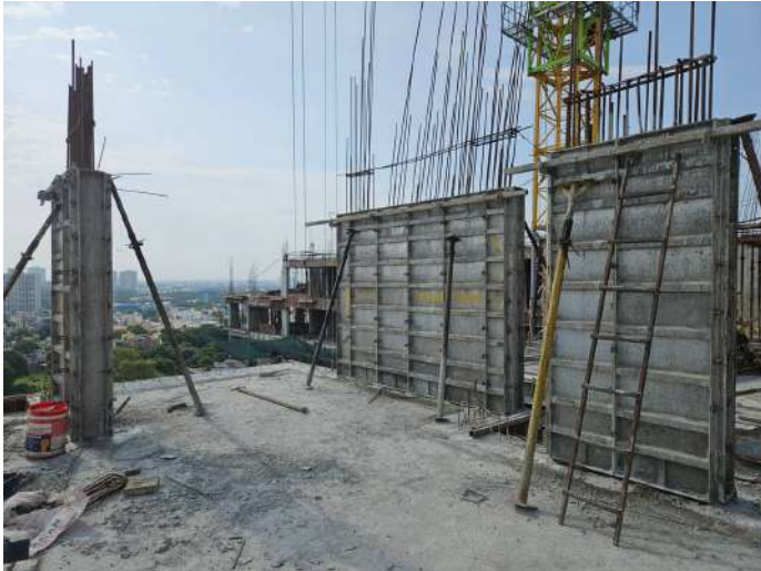
Twelfth Floor P2 - Column Shuttering
