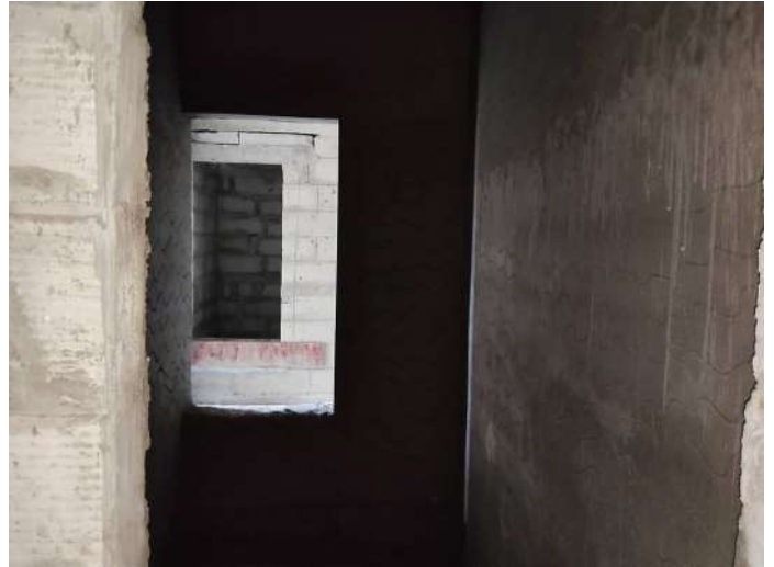
8F - Internal Plastering
