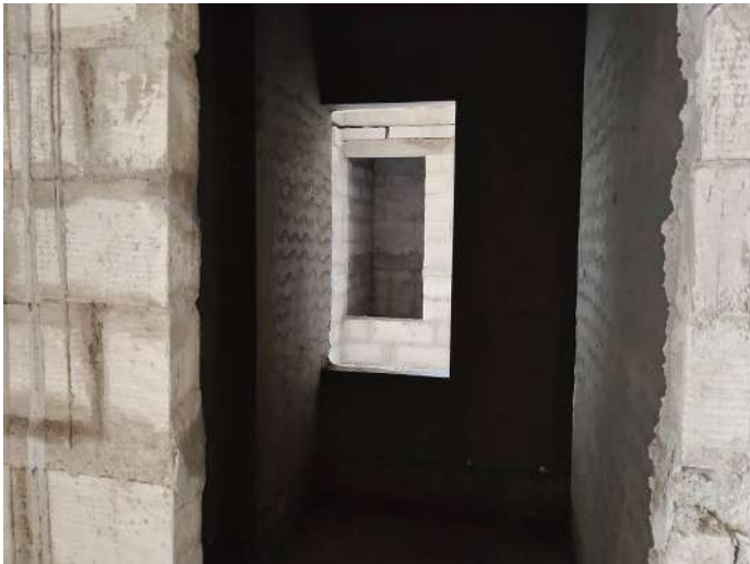
8F - Internal Plastering
