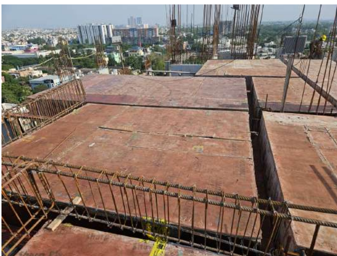
Eleventh Floor P2 - Roof Slab Shuttering
