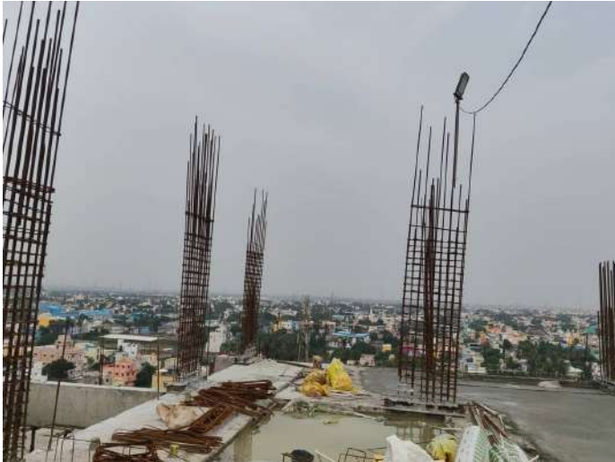
Twelfth Floor P1 - Col Marking & Reinforcement
