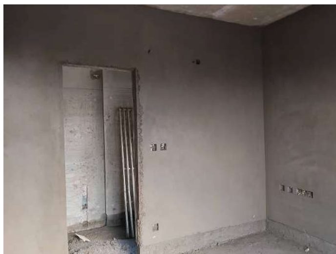
7F - Internal Plastering
