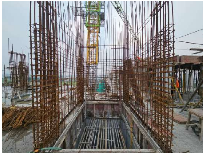
Twelfth Floor P1 - Col Marking & Reinforcement
