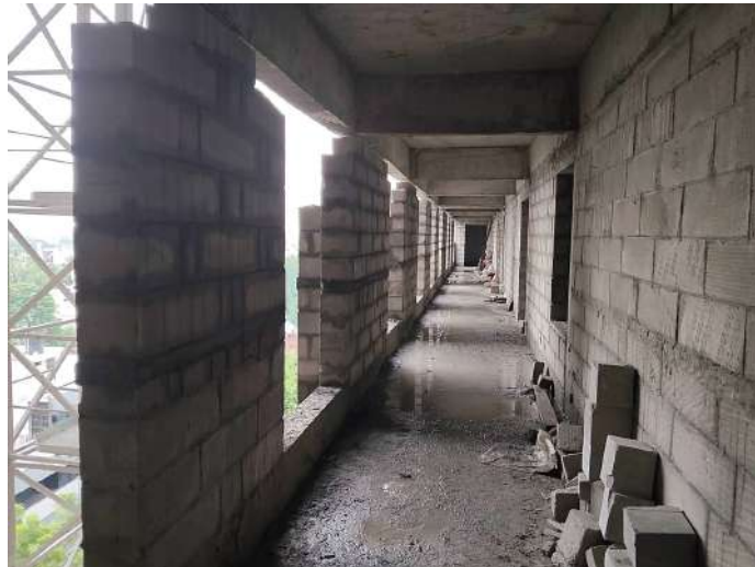
BW Corridor area - Sixth Floor
