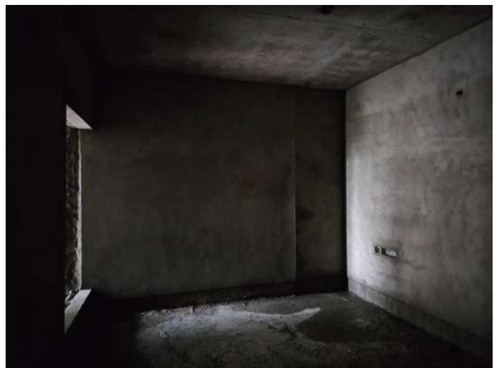
On Completion of Plastering - 6th Floor - 607
