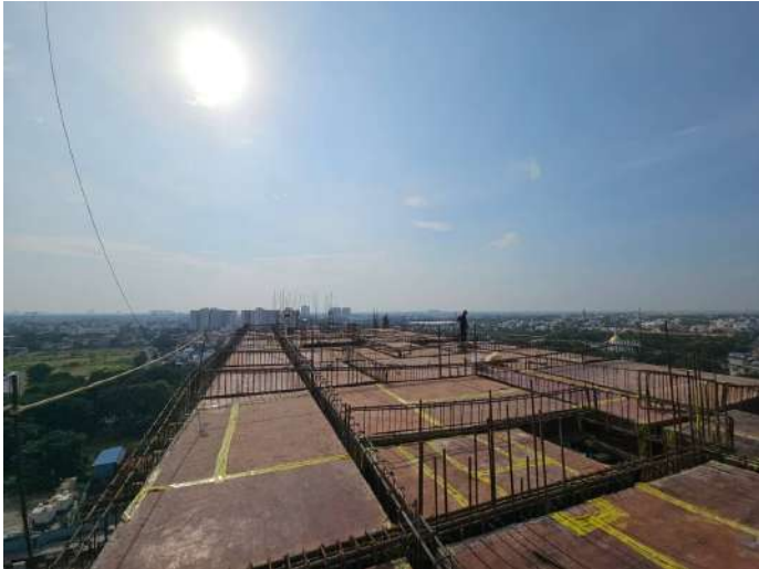
Twelfth Floor P1 - Slab & Beam Reinforcement
