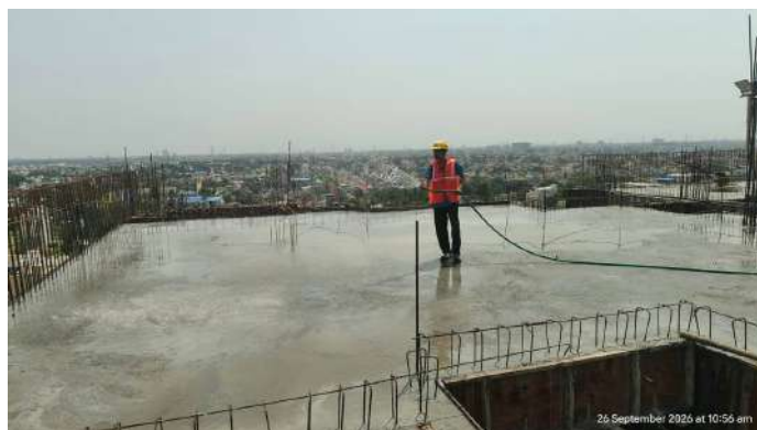
On Completion of Roof Level - 12th Floor
