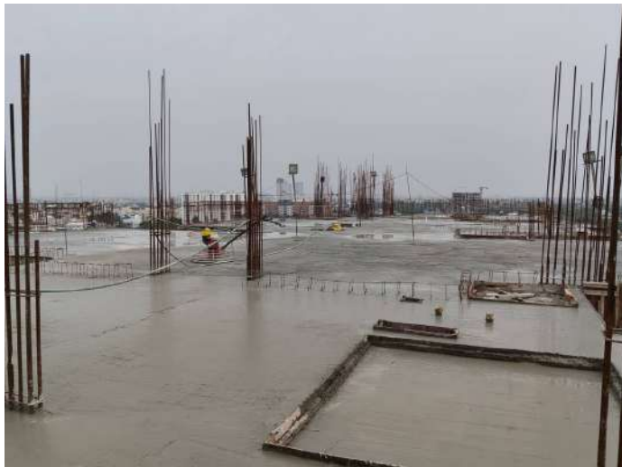
Eleventh Floor P2 - Roof Slab Concreting
