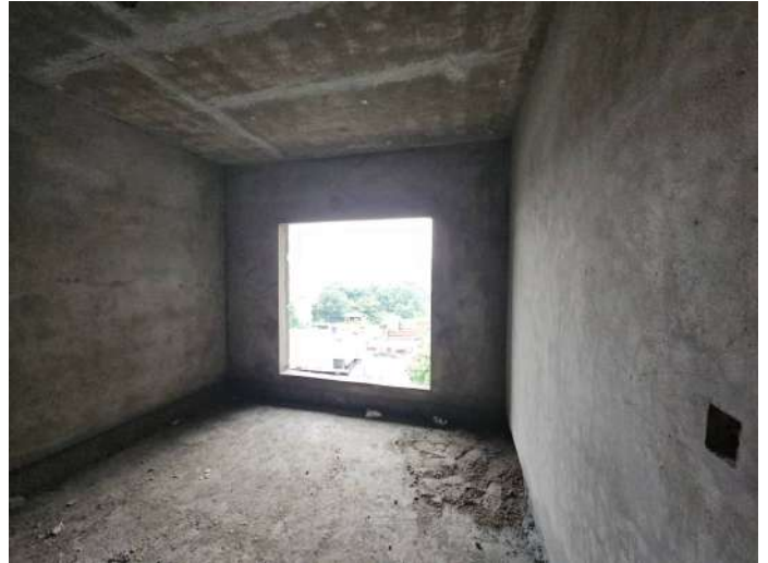
On Completion of Plastering - 6th Floor - 607
