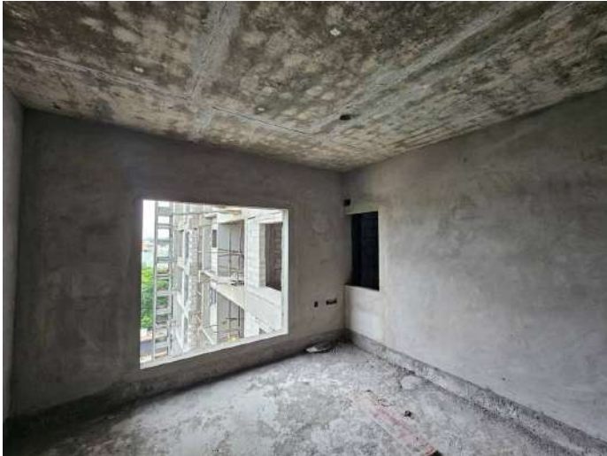
On Completion of Plastering - 6th Floor - 613
