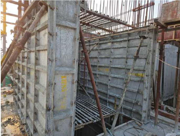
Twelfth Floor P1 - Column Shuttering
