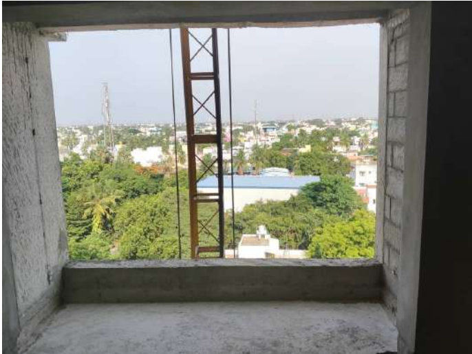
7F - Balcony Surface Cleaning
