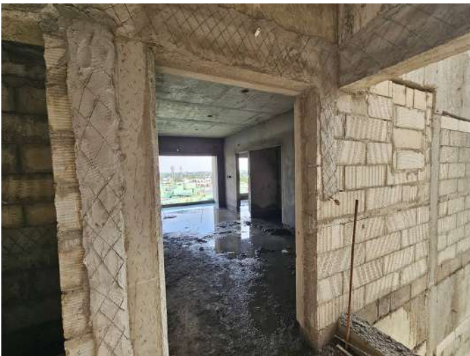
On Completion of Plastering - 6th Floor - 604
