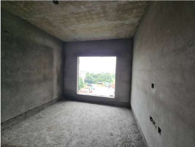
On Completion of Plastering - 6th Floor - 606
