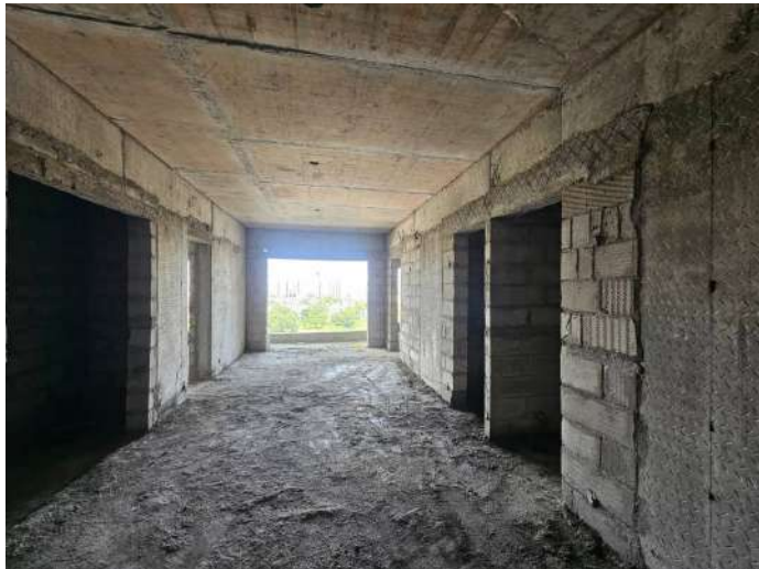
On Completion of Blockwork - 8th Floor - 806
