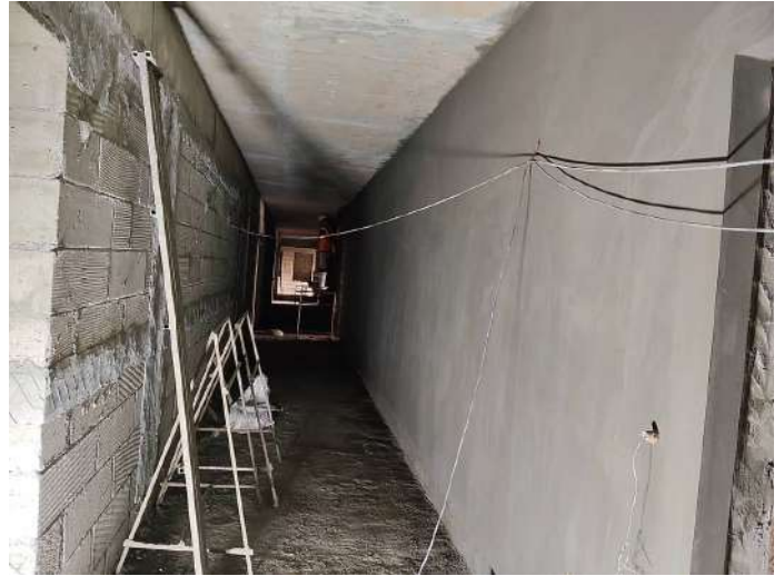
7F - Internal Plastering Corridor Area
