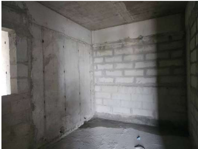
On Completion of Blockwork - 8th Floor - 811
