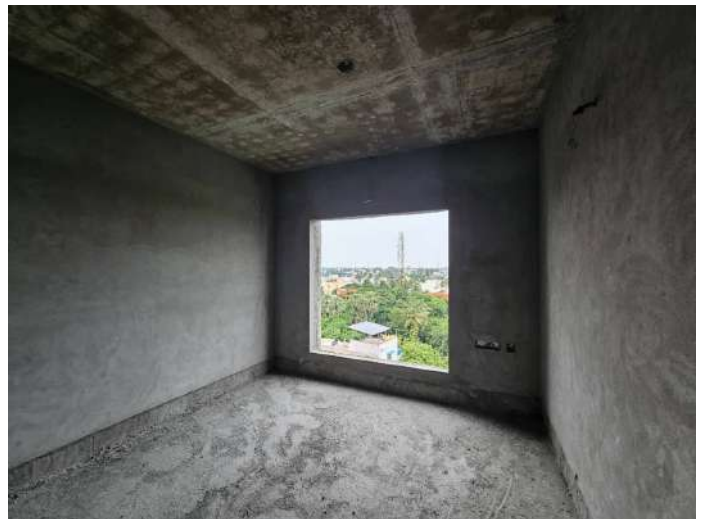
On Completion of Plastering - 6th Floor - 602
