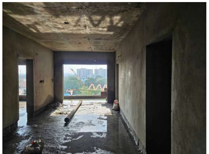
On Completion of Plastering - 6th Floor - 607
