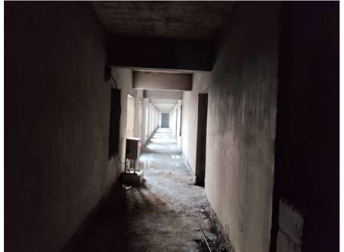
5F - Internal Plastering Corridor Area
