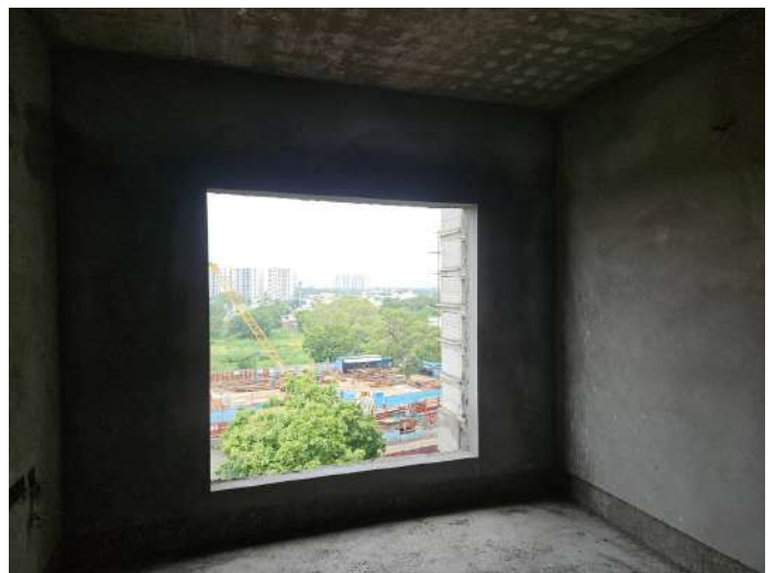
On Completion of Plastering - 6th Floor - 606
