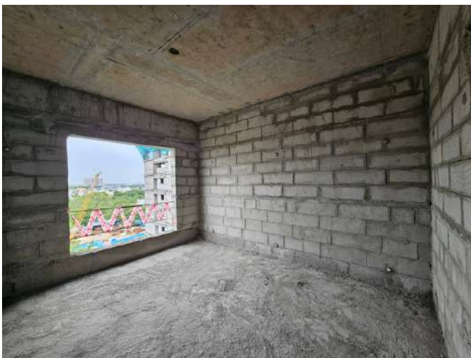
On Completion of Blockwork - 8th Floor - 806
