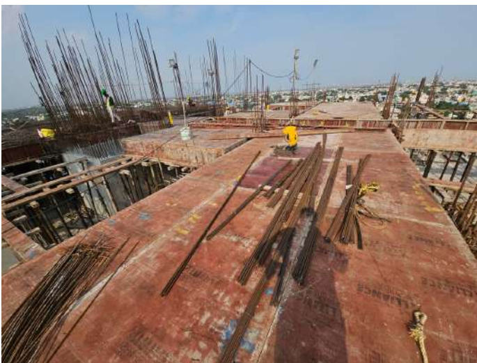
Twelfth Floor P1 - Roof Slab Shuttering
