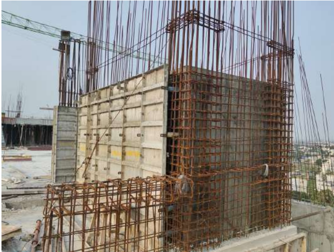
LMR - Reinforcement, Shuttering, Concreting
