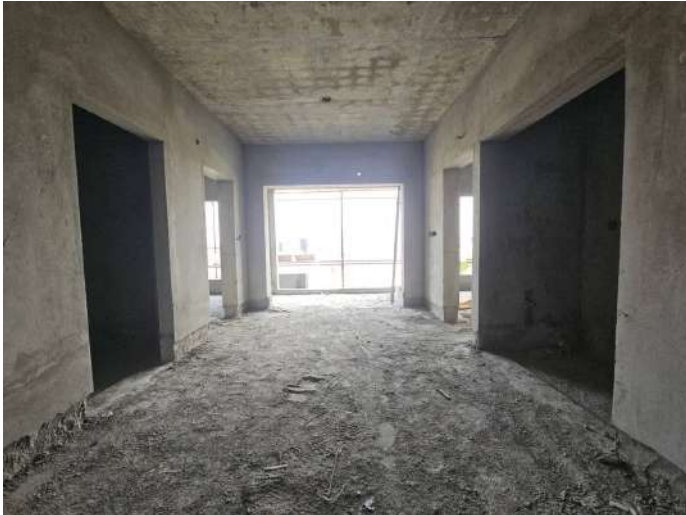
On Completion of Plastering - 6th Floor - 609
