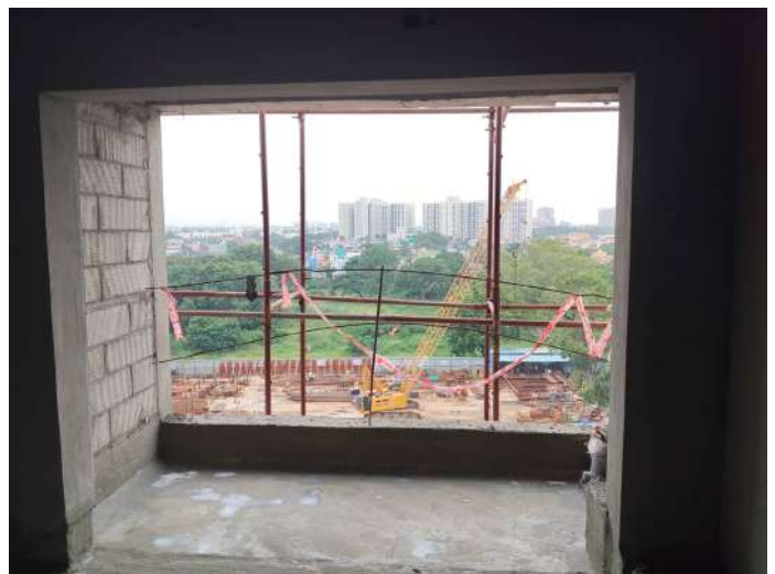
6F - Balcony Waterproofing
