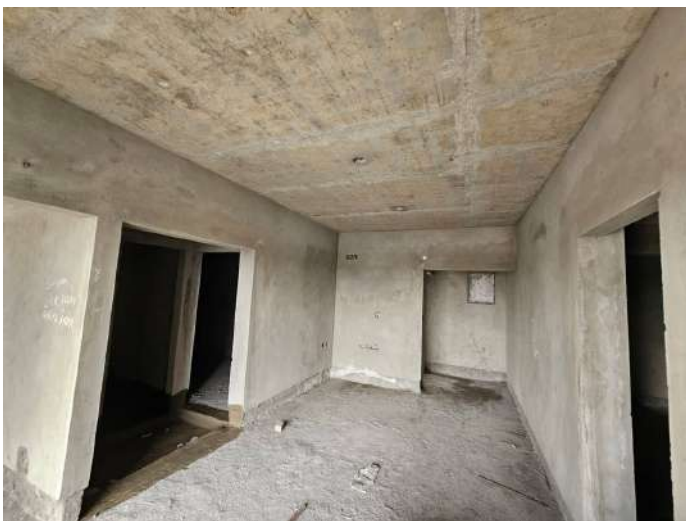
On Completion of Plastering - 6th Floor - 612
