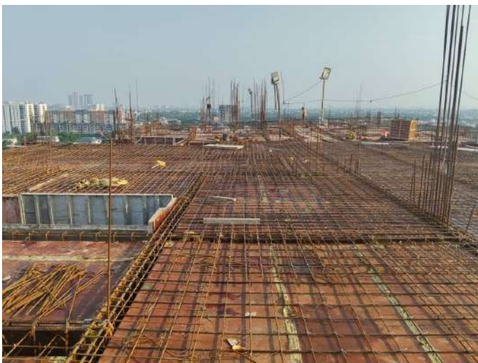
Eleventh Floor P2 - Slab & Beam Reinforcement
