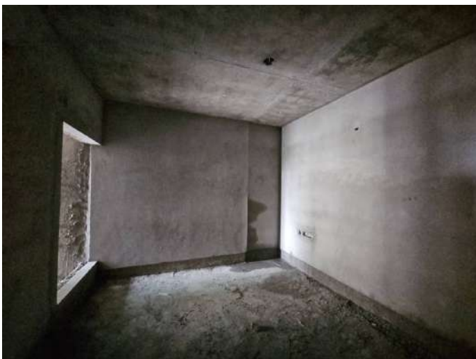
On Completion of Plastering - 6th Floor - 607
