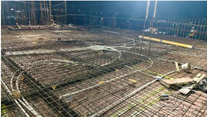
Twelfth Floor P2 - Electrical - Conduit Laying
