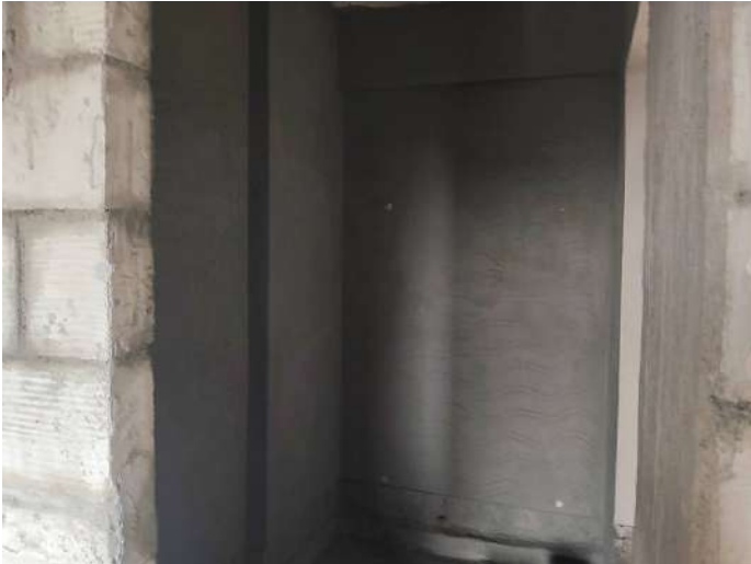
9F - Internal Plastering
