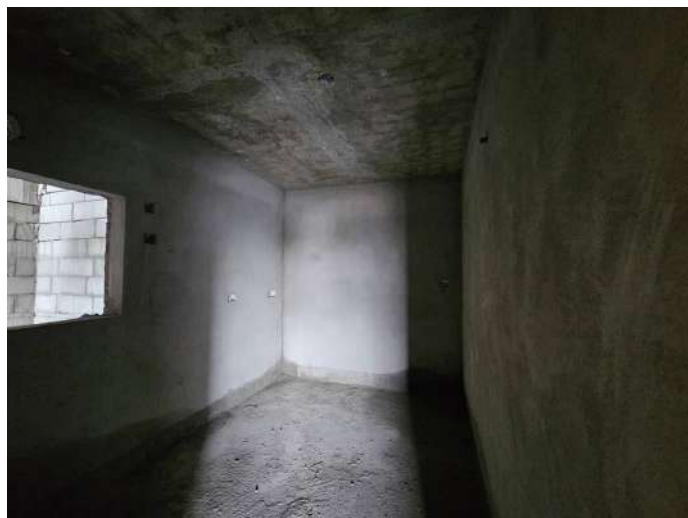
On Completion of Plastering - 6th Floor - 612
