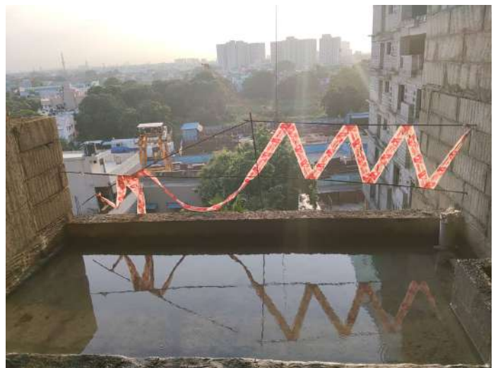
6F - Balcony Water Bond Test
