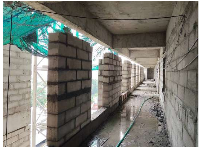
BW Corridor area - Seventh Floor
