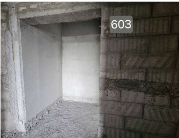
On Completion of Plastering - 6th Floor - 603
