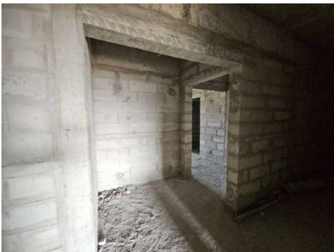
On Completion of Blockwork - 8th Floor - 801
