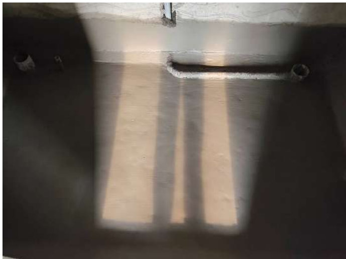
6F - Toilet Waterproofing
