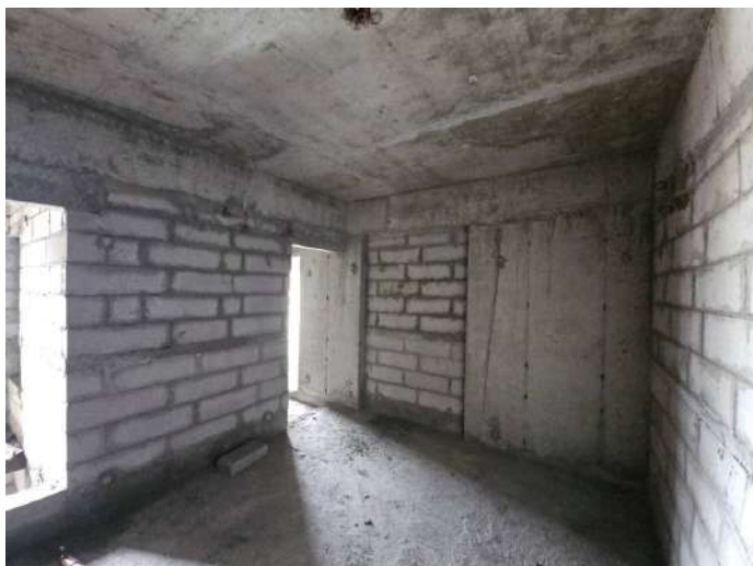
On Completion of Blockwork - 8th Floor - 809
