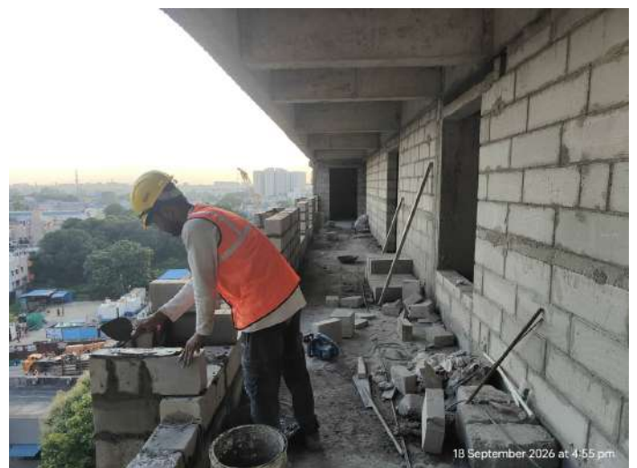
BW Corridor area - Seventh Floor
