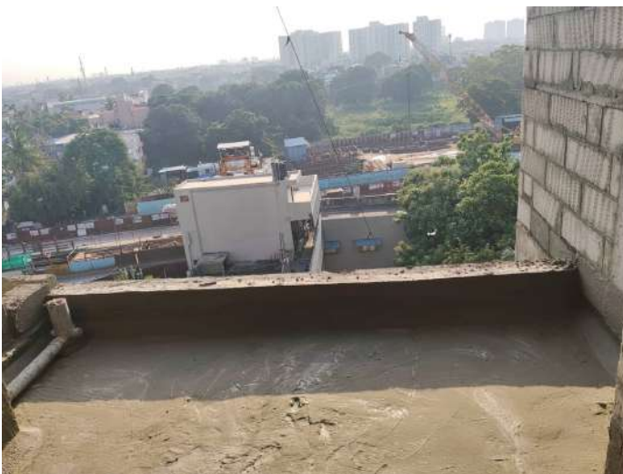
6F - Balcony Waterproofing
