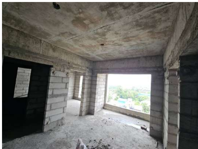
On Completion of Blockwork - 8th Floor - 809
