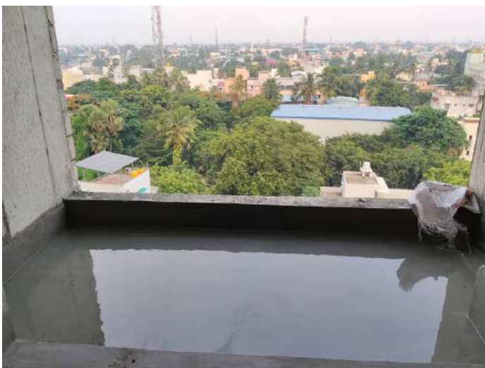
7F - Balcony Water Bond Test
