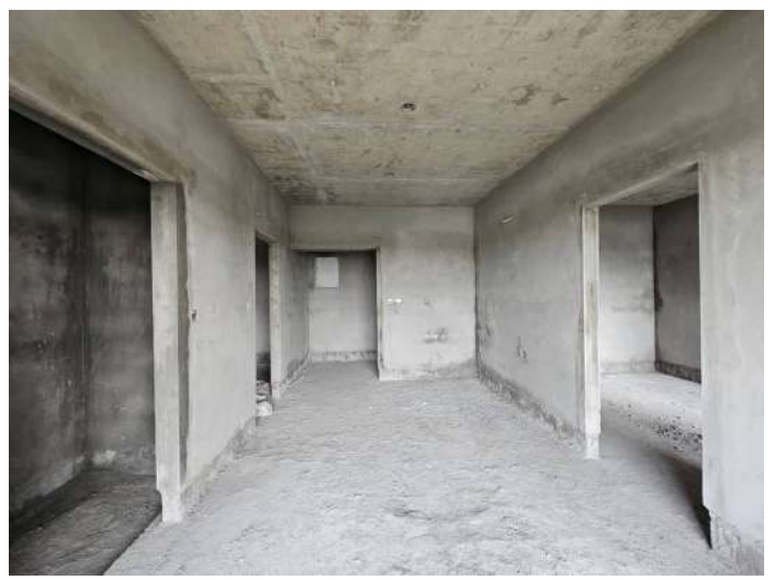
On Completion of Plastering - 6th Floor - 603
