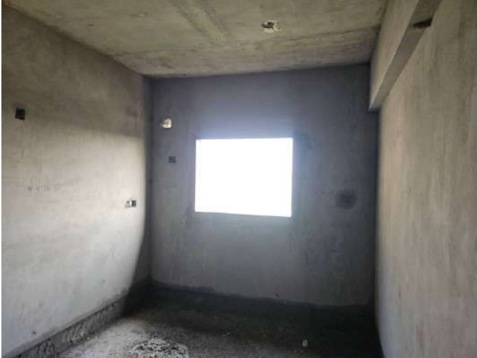
On Completion of Plastering - 6th Floor - 608
