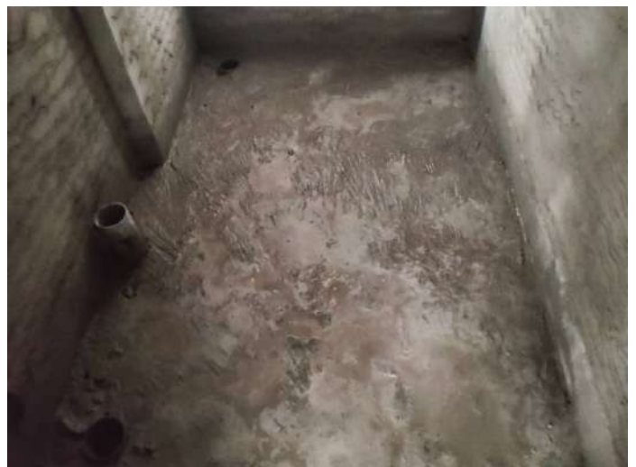
6F - Sunken Pipe Laying
