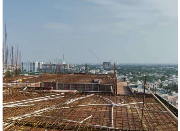
Eleventh Floor P2 - Roof Slab Shuttering
