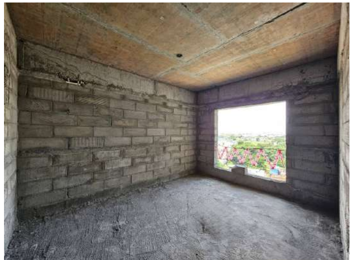
On Completion of Blockwork - 8th Floor - 807
