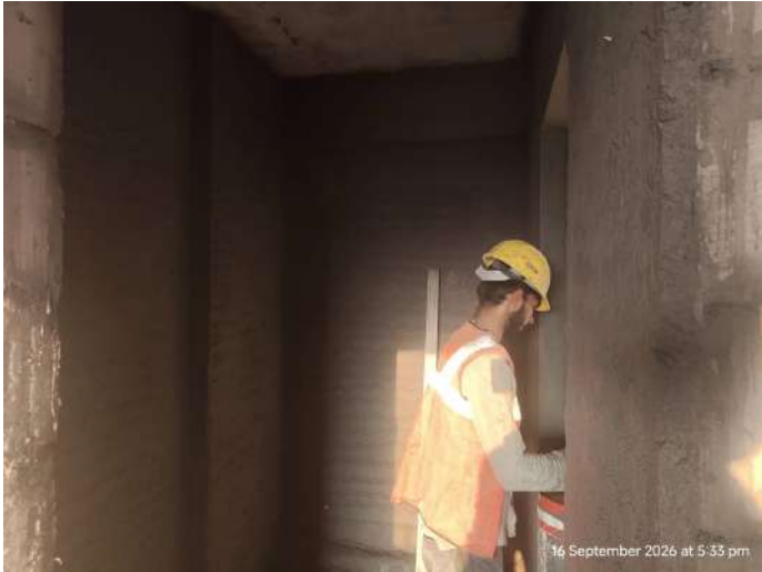
8F - Internal Plastering
