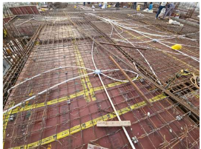
Twelfth Floor P2 - Roof Slab Shuttering
