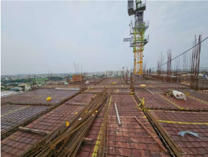
Twelfth Floor P2 - Slab & Beam Reinforcement
