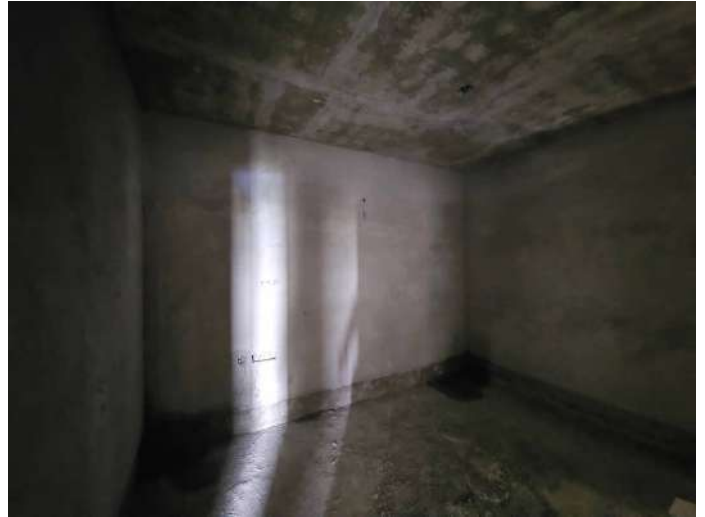
On Completion of Plastering - 6th Floor - 601
