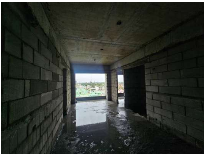
On Completion of Blockwork - 8th Floor - 804
