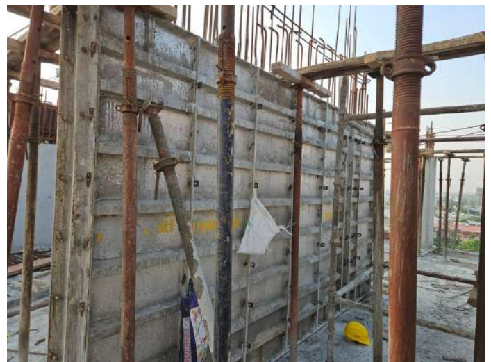
Twelfth Floor P1 - Column Concrete
