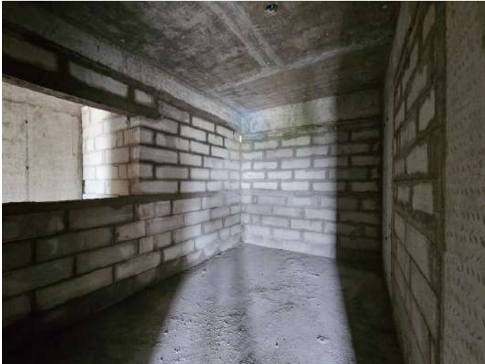
On Completion of Blockwork - 8th Floor - 810
