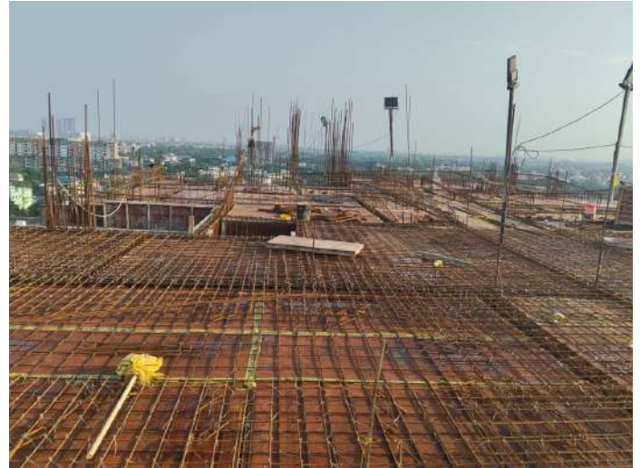
Eleventh Floor P2 - Roof Slab Shuttering
