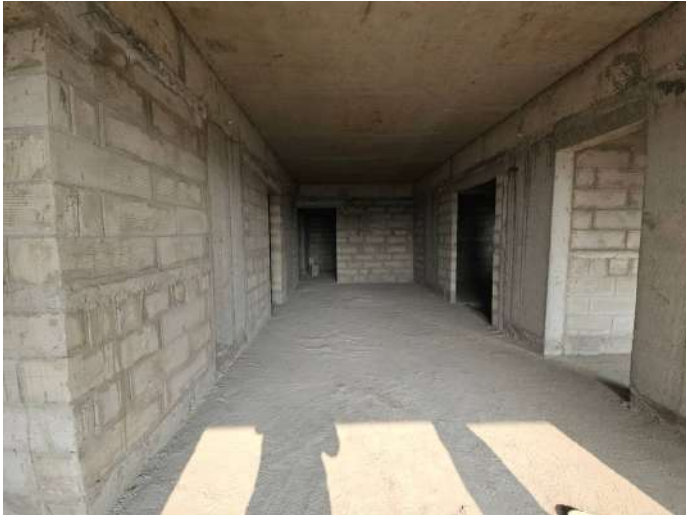
On Completion of Blockwork - 9th Floor - 906
