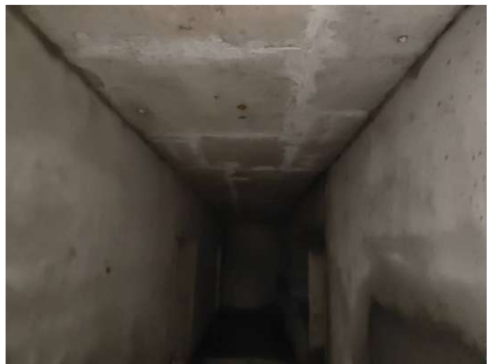
3F - Internal Plastering Corridor Area
