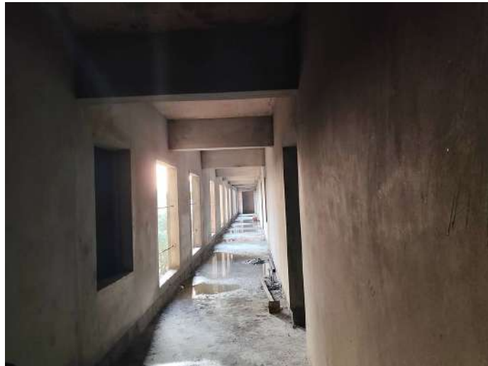
3F - Internal Plastering Corridor Area
