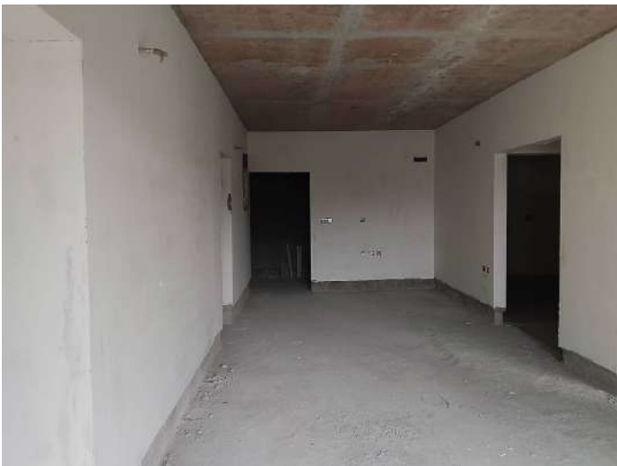
2F - Putty 1st Coat
