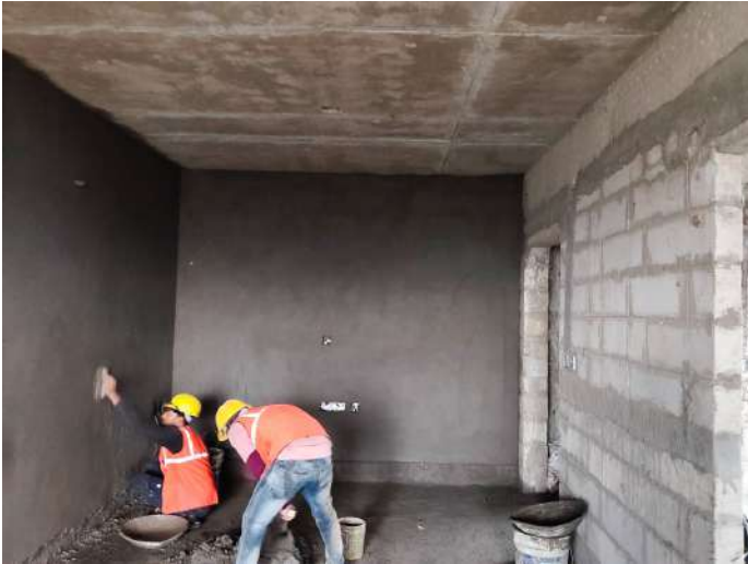
7F - Internal Plastering
