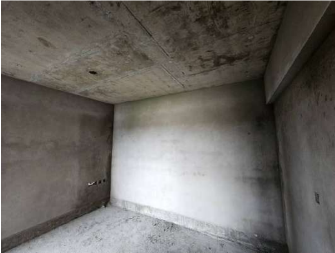
On Completion of Plastering - 6th Floor - 603
