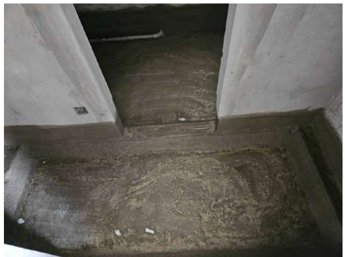
6F - Toilet Waterproofing
