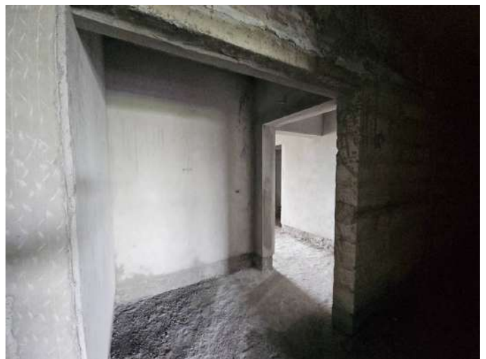
On Completion of Plastering - 6th Floor - 601
