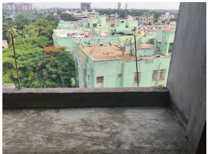
6F - Balcony Surface Cleaning
