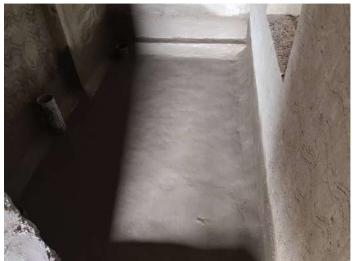
6F - Toilet Waterproofing
