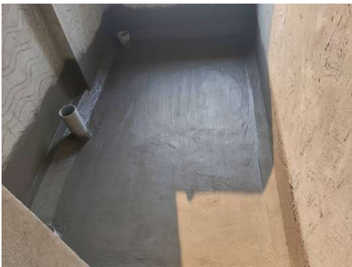
6F - Toilet Waterproofing
