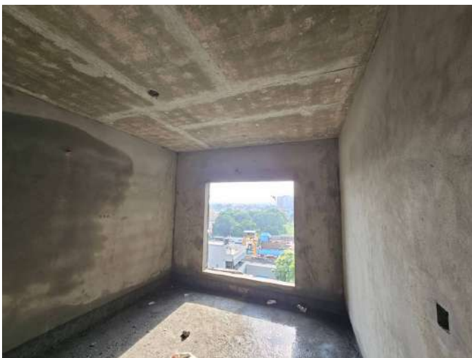
On Completion of Plastering - 6th Floor - 607
