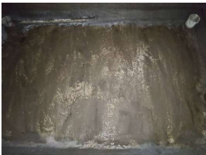
6F - Toilet Waterproofing
