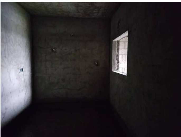
On Completion of Plastering - 6th Floor - 607
