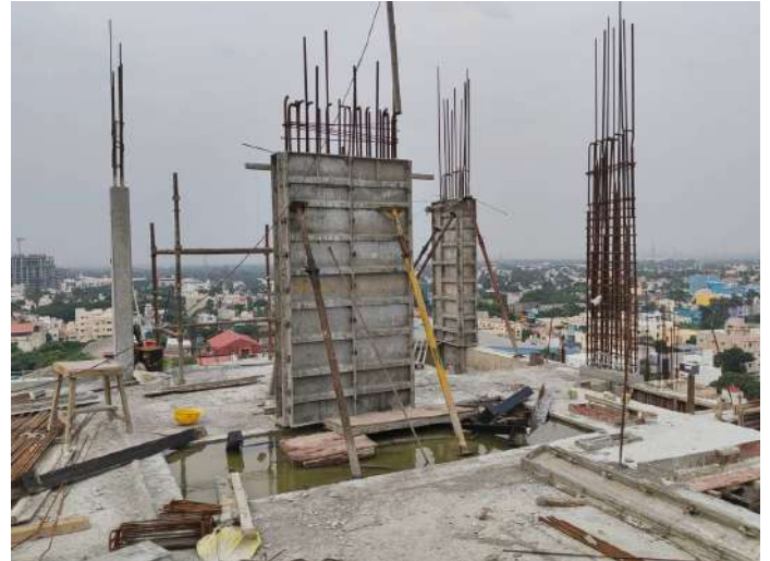
Twelfth Floor P1 - Column Shuttering
