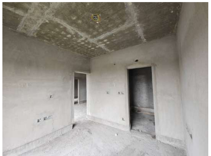
On Completion of Plastering - 6th Floor - 605
