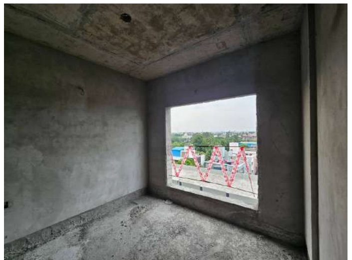
On Completion of Plastering - 6th Floor - 611
