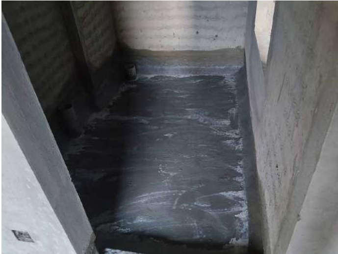
7F - Toilet Waterproofing
