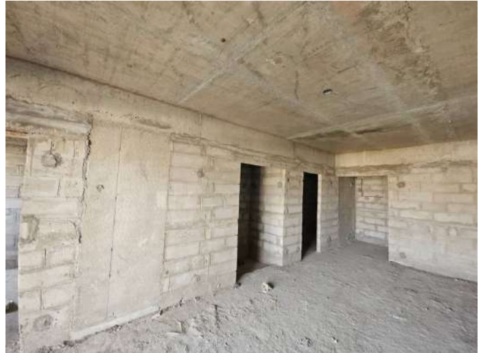
On Completion of Blockwork - 8th Floor - 801
