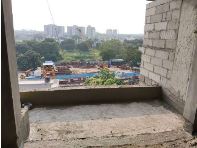
7F - Balcony Waterproofing
