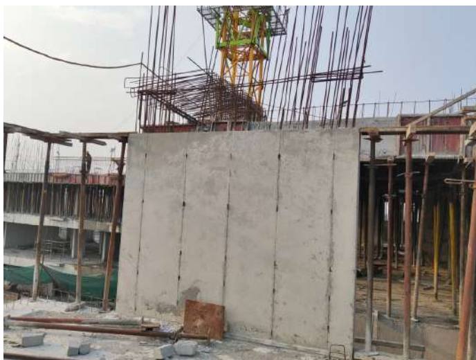
Twelfth Floor P2 - Column Concrete
