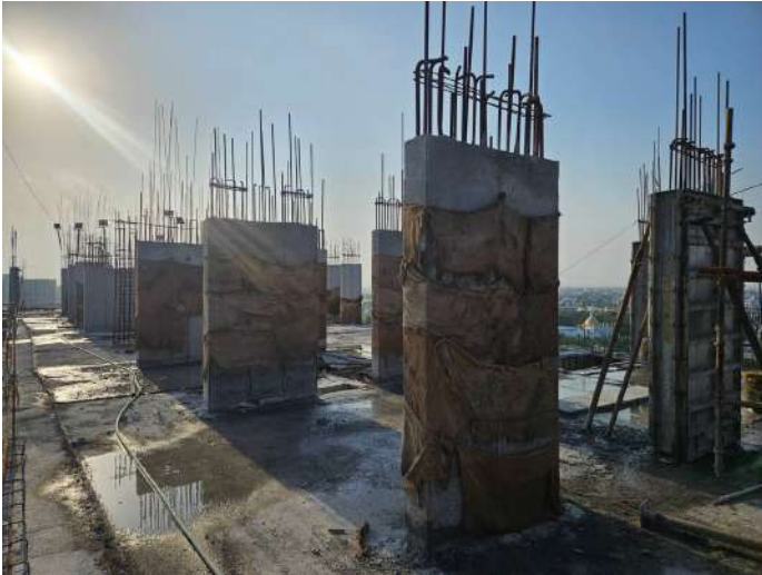
Twelfth Floor P1 - Column Concrete
