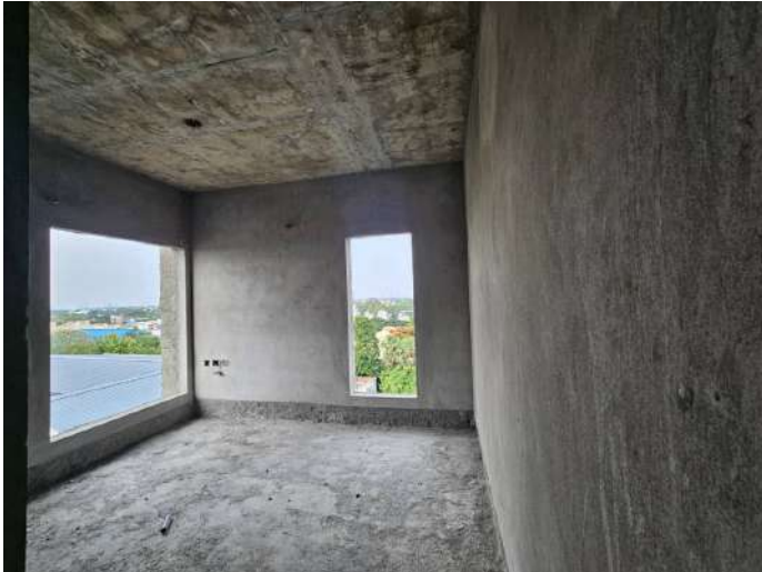
On Completion of Plastering - 6th Floor - 613
