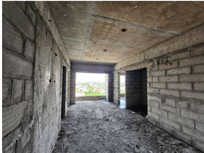
On Completion of Blockwork - 8th Floor - 812
