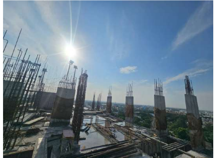
Twelfth Floor P1 - Column Concrete
