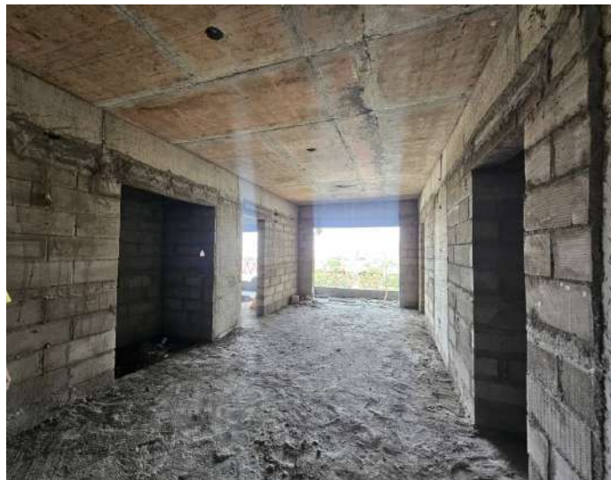
On Completion of Blockwork - 8th Floor - 807
