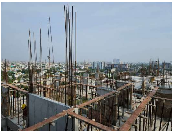
Twelfth Floor P1 - Roof Slab Shuttering
