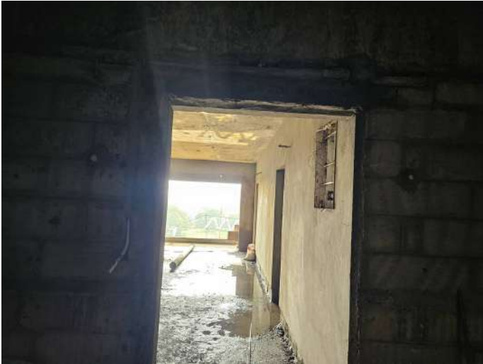
On Completion of Plastering - 6th Floor - 607
