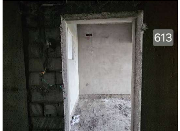
On Completion of Plastering - 6th Floor - 613
