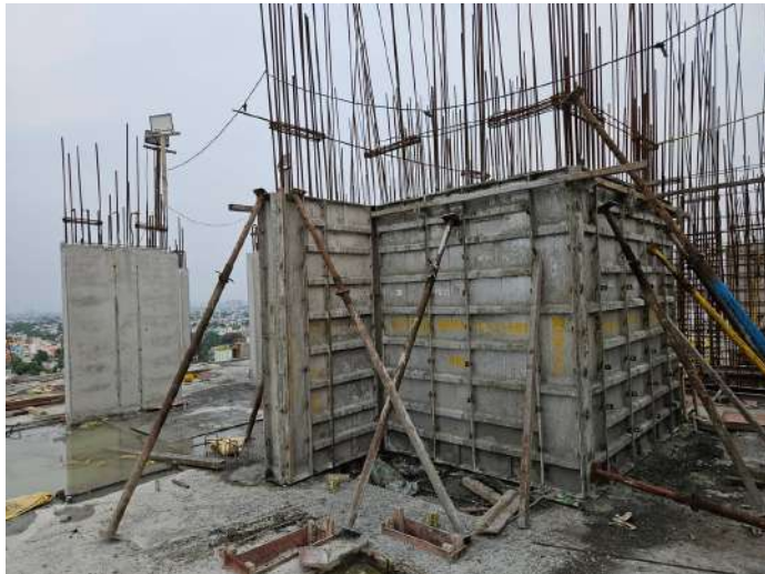
Twelfth Floor P1 - Column Concrete
