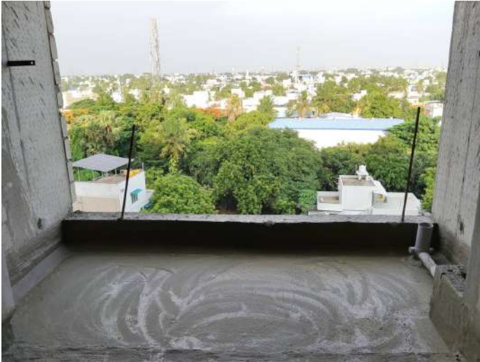
6F - Balcony Waterproofing
