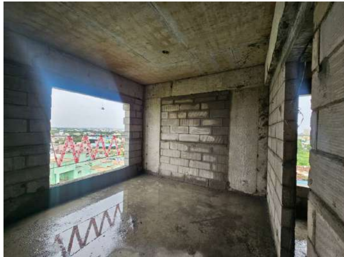
On Completion of Blockwork - 8th Floor - 804
