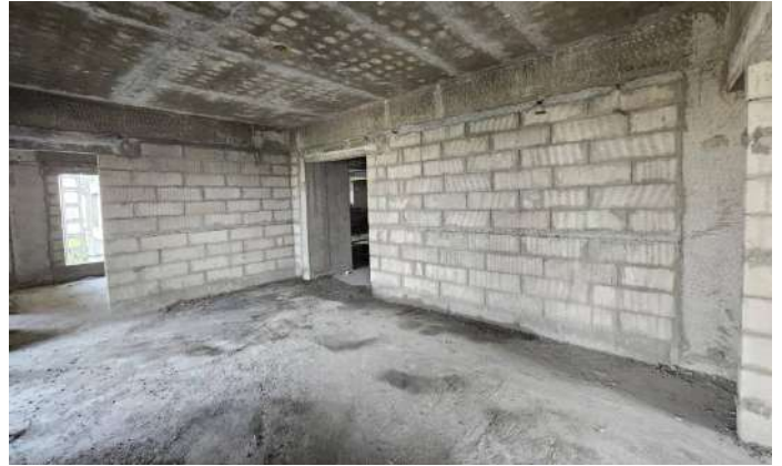
On Completion of Blockwork - 8th Floor - 813
