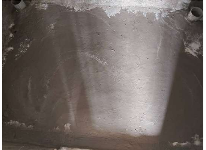
6F - Toilet Waterproofing
