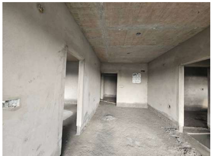
On Completion of Plastering - 7th Floor - 705
