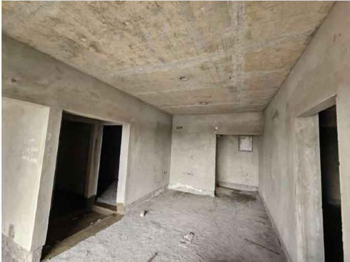
On Completion of Plastering - 6th Floor - 610
