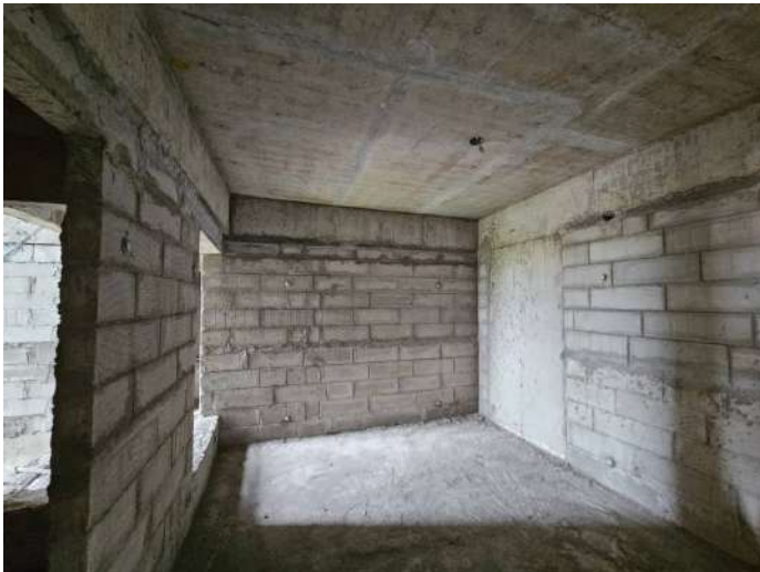
On Completion of Blockwork - 8th Floor - 806
