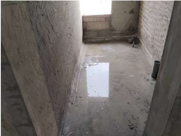
7F - Toilet Waterproofing
