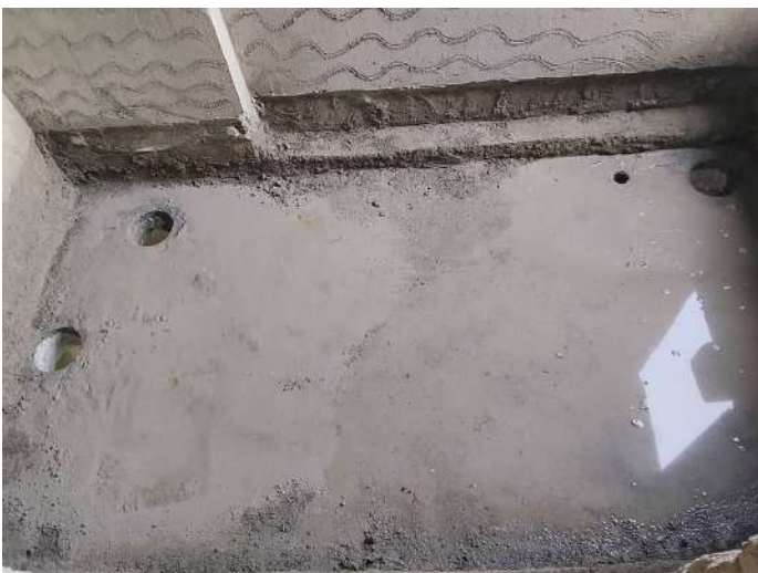
7F - Core& Wall Cutting
