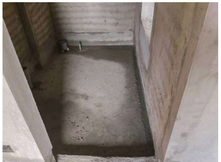
7F - Balcony Waterproofing
