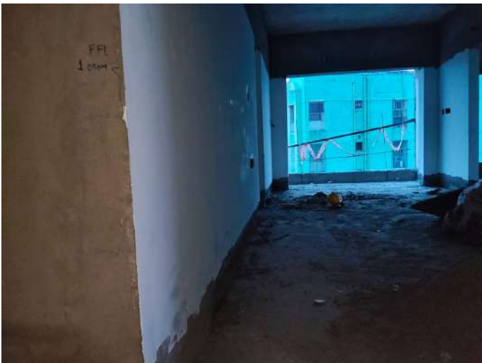
2F - Putty 1st Coat
