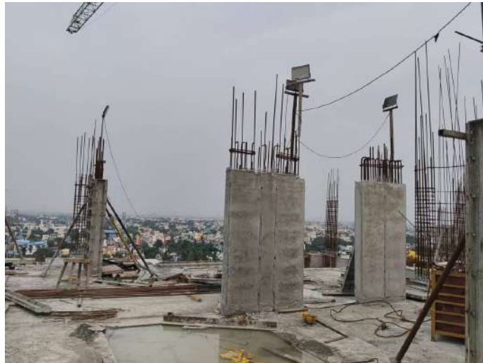
Twelfth Floor P1 - Column Concrete
