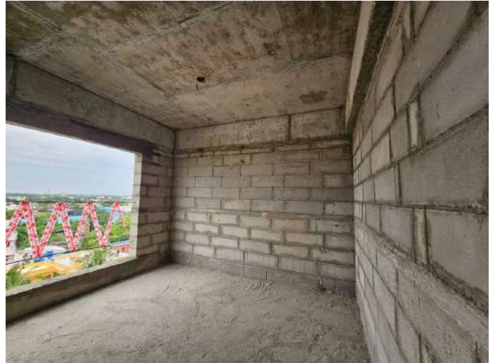
On Completion of Blockwork - 8th Floor - 810
