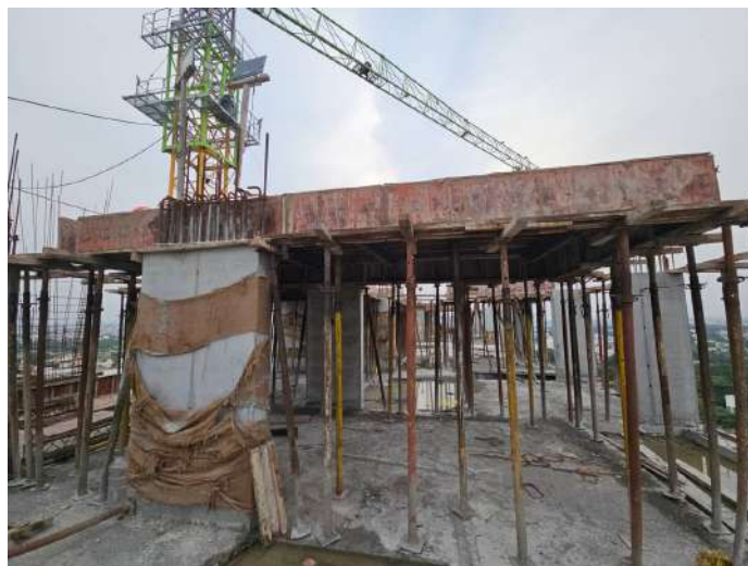
Twelfth Floor P1 - Roof Slab Shuttering
