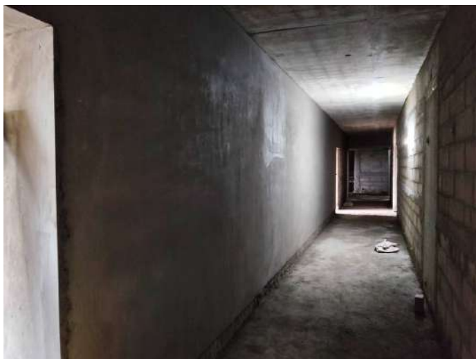
5F - Internal Plastering Corridor Area
