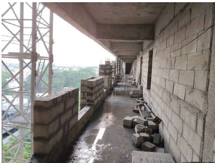
BW Corridor area - Sixth Floor
