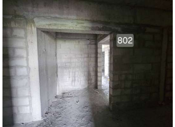
On Completion of Blockwork - 8th Floor - 802
