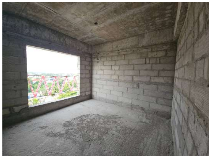
On Completion of Blockwork - 8th Floor - 811
