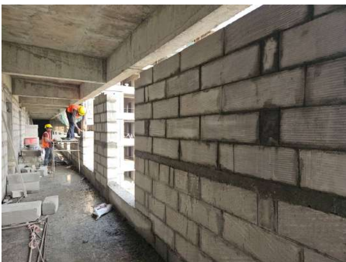
BW Corridor area - Seventh Floor
