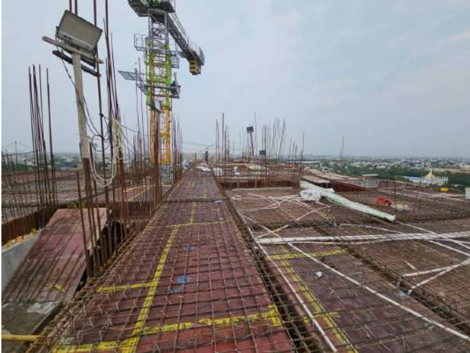
Twelfth Floor P1 - Slab & Beam Reinforcement
