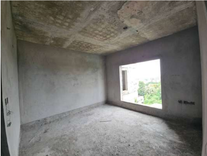
On Completion of Plastering - 6th Floor - 601
