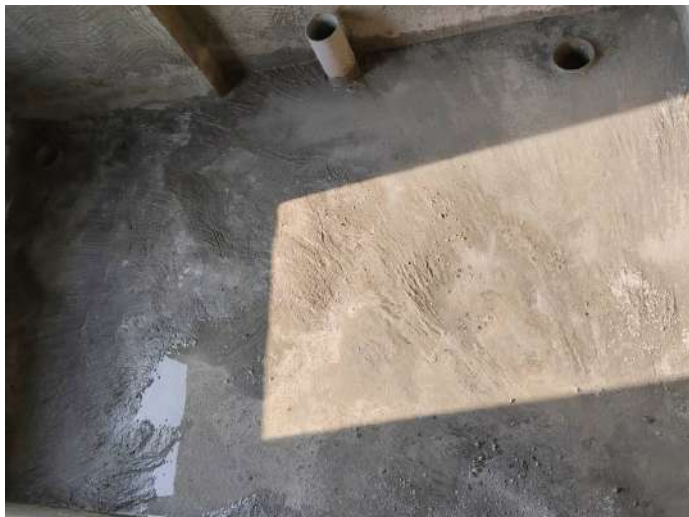
6F - Sunken Pipe Laying
