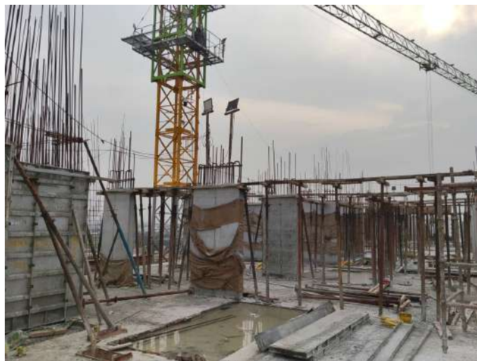
Twelfth Floor P1 - Roof Slab Shuttering
