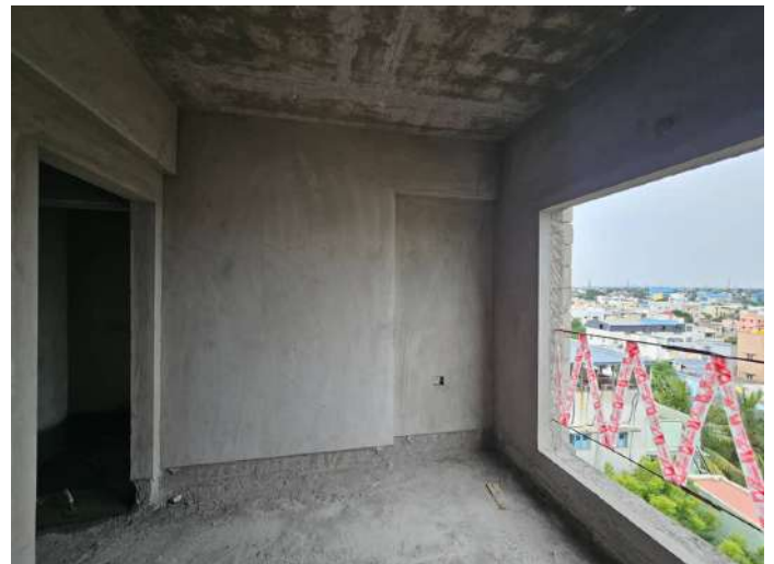
On Completion of Plastering - 6th Floor - 613
