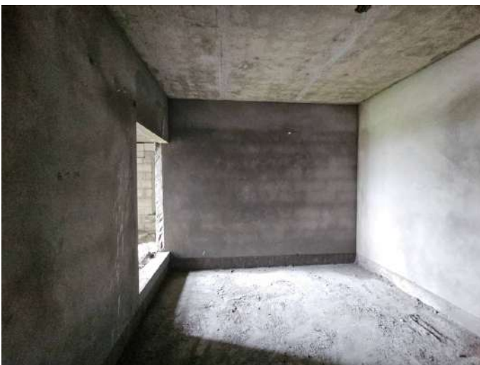
On Completion of Plastering - 6th Floor - 606
