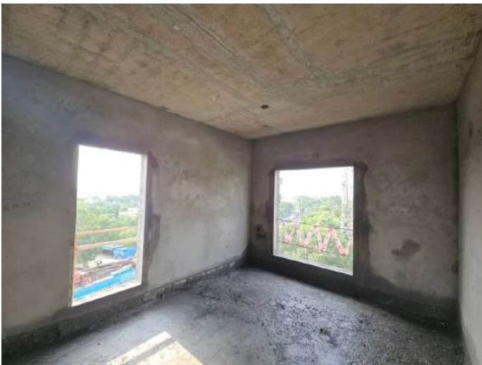
On Completion of Plastering - 6th Floor - 608
