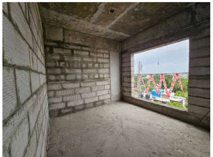
On Completion of Blockwork - 8th Floor - 810
