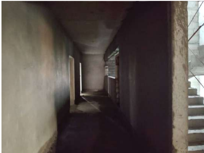
4F - Internal Plastering Corridor Area
