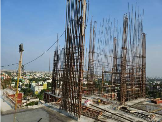
Twelfth Floor P2 - Col Marking & Reinforcement
