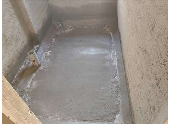
6F - Toilet Waterproofing
