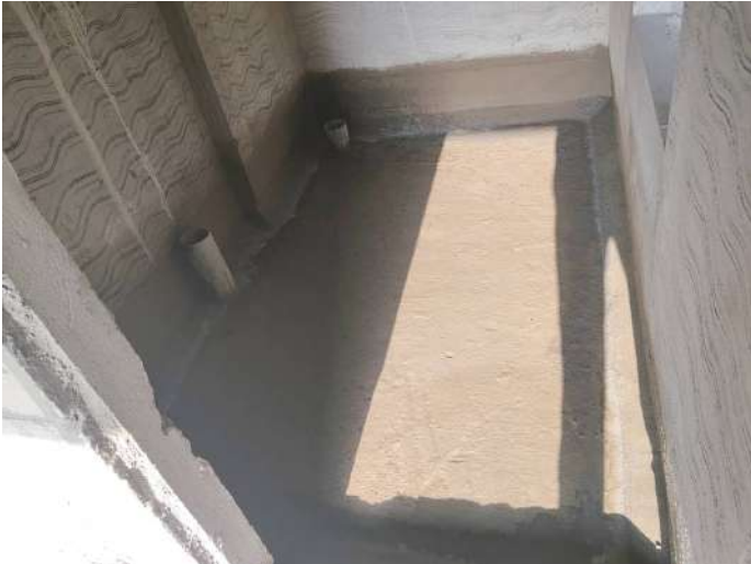
6F - Toilet Waterproofing
