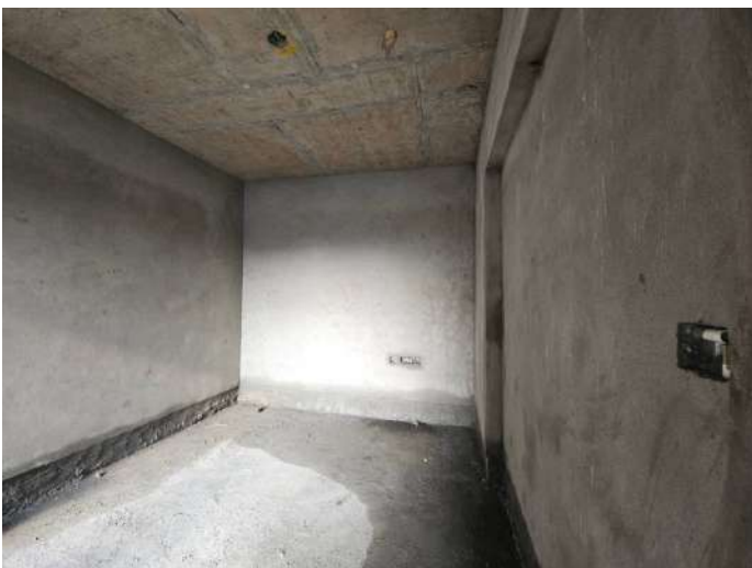
On Completion of Plastering - 7th Floor - 705
