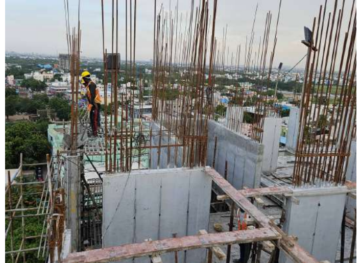
Eleventh Floor P2 - Column Concrete
