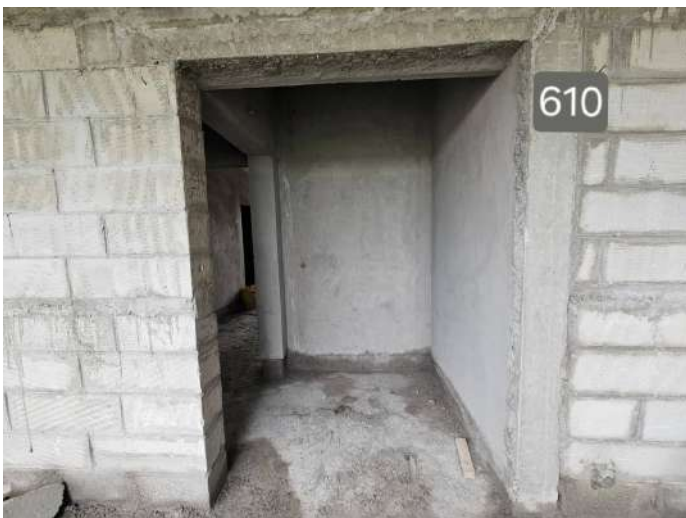
On Completion of Plastering - 6th Floor - 610
