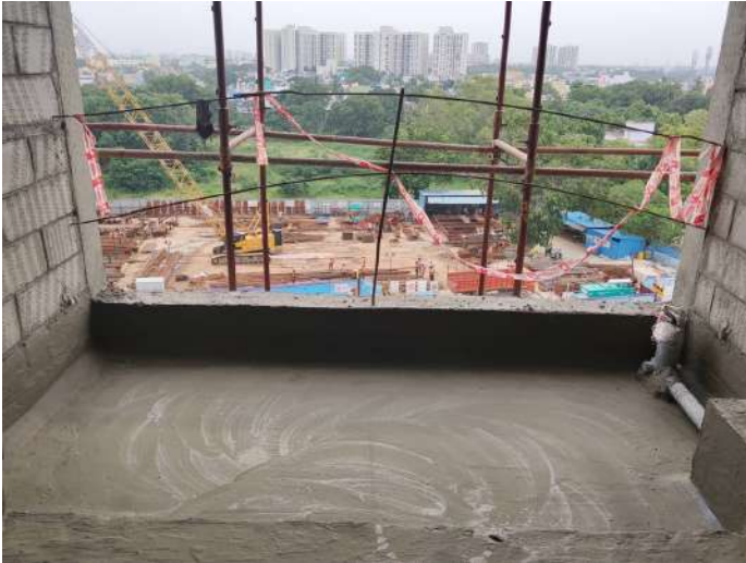
6F - Balcony Waterproofing
