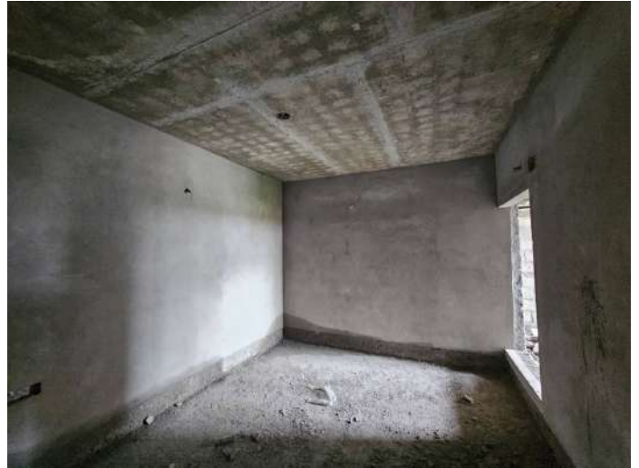
On Completion of Plastering - 6th Floor - 602
