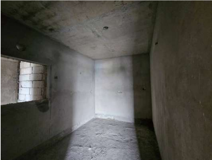
On Completion of Plastering - 6th Floor - 610
