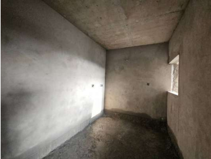
On Completion of Plastering - 7th Floor - 705
