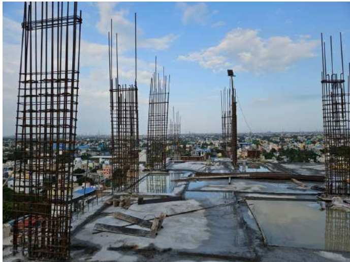
Twelfth Floor P1 - Col Marking & Reinforcement
