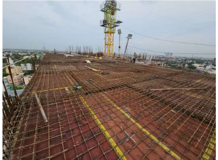
Twelfth Floor P1 - Slab & Beam Reinforcement
