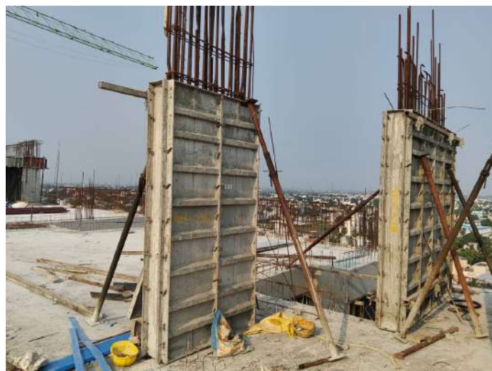
Twelfth Floor P2 - Column Shuttering
