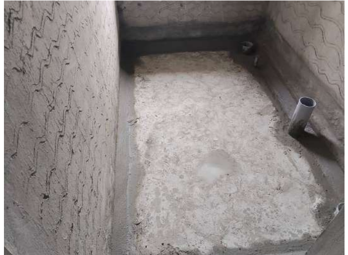
7F - Toilet Waterproofing
