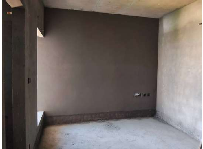
7F - Internal Plastering
