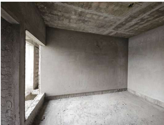
On Completion of Plastering - 6th Floor - 605
