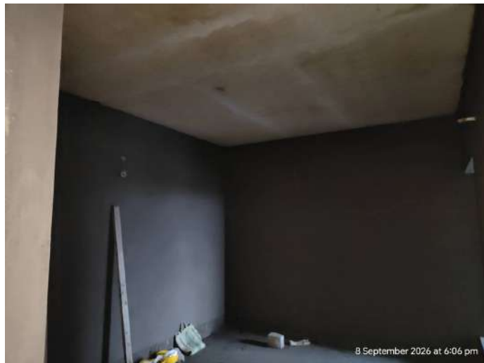
7F - Internal Plastering
