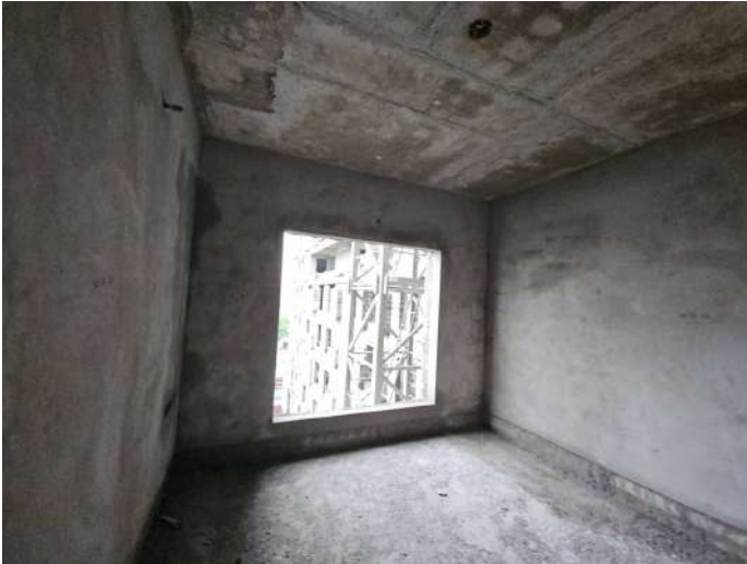
On Completion of Plastering - 6th Floor - 607
