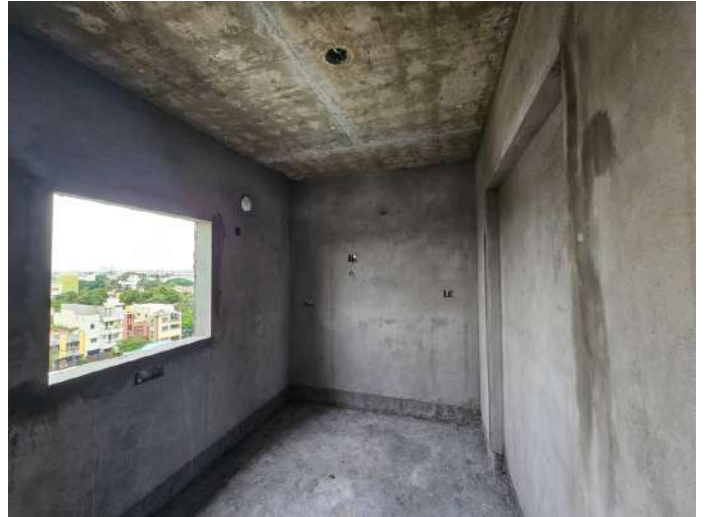
On Completion of Plastering - 6th Floor - 603
