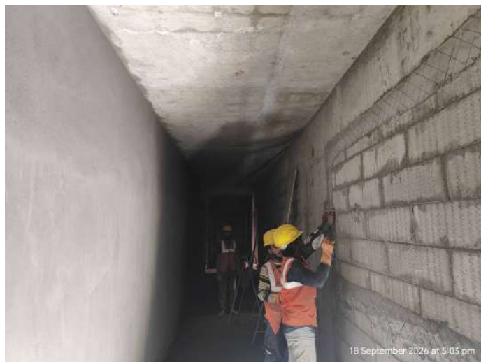
6F - Internal Plastering Corridor Area
