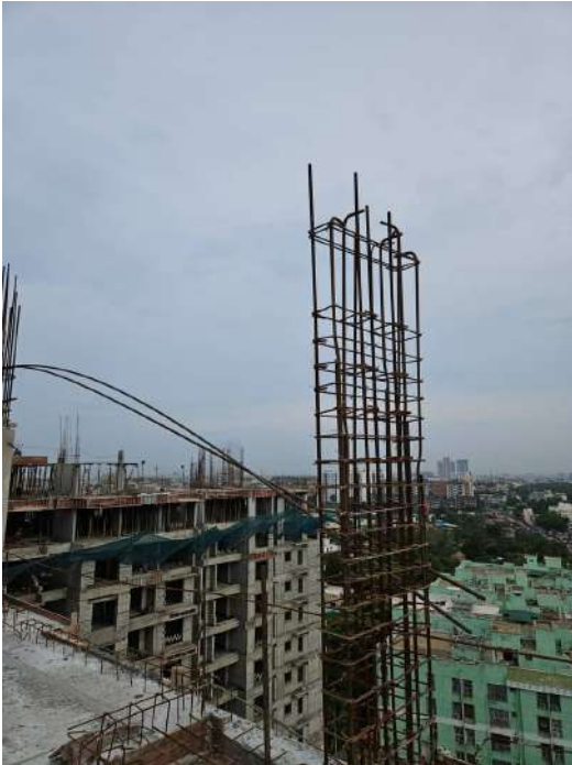
Twelfth Floor P1 - Col Marking & Reinforcement
