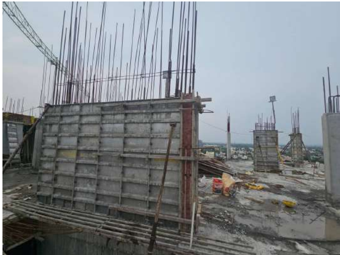
Twelfth Floor P1 - Column Shuttering
