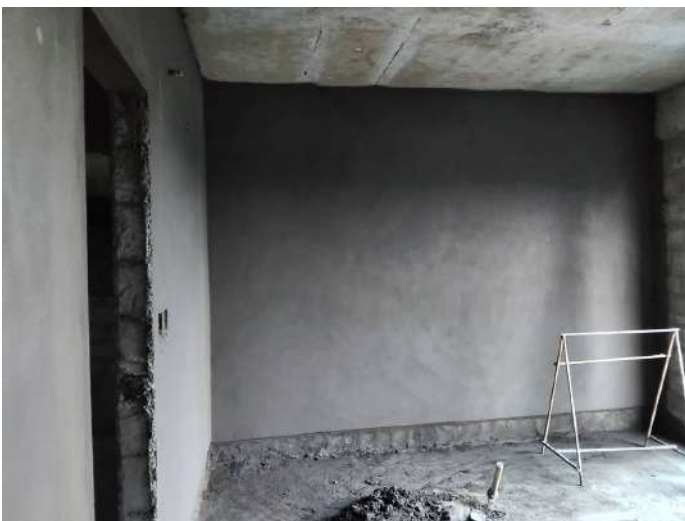
7F - Internal Plastering
