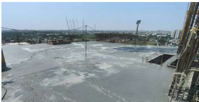
On Completion of Roof Level - 12th Floor
