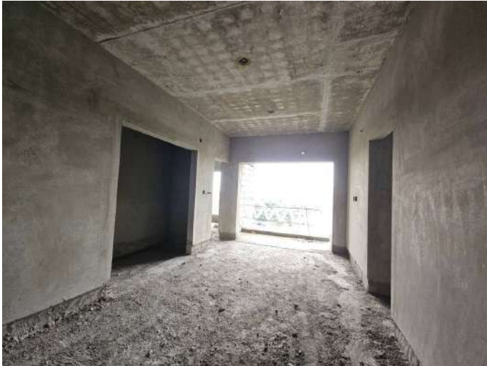
On Completion of Plastering - 6th Floor - 605
