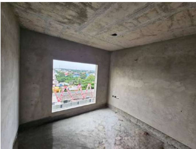
On Completion of Plastering - 6th Floor - 611
