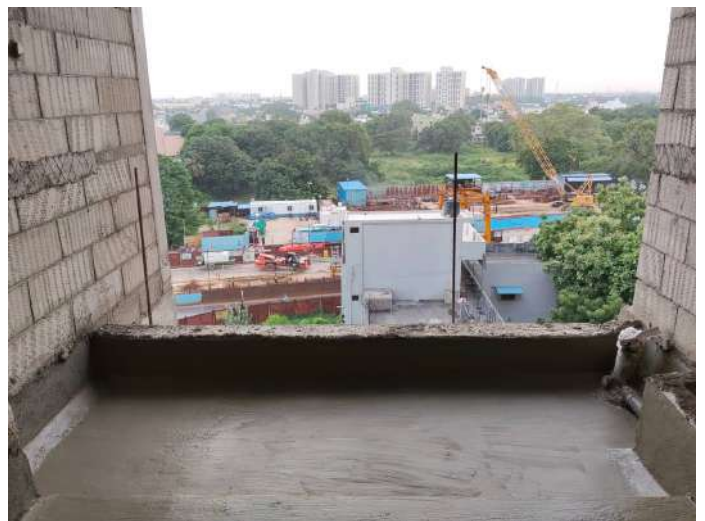
6F - Balcony Waterproofing
