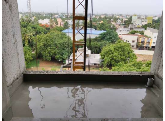
6F - Balcony Water Bond Test
