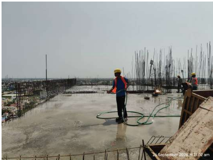
Twelfth Floor P1 - Roof Slab Concreting
