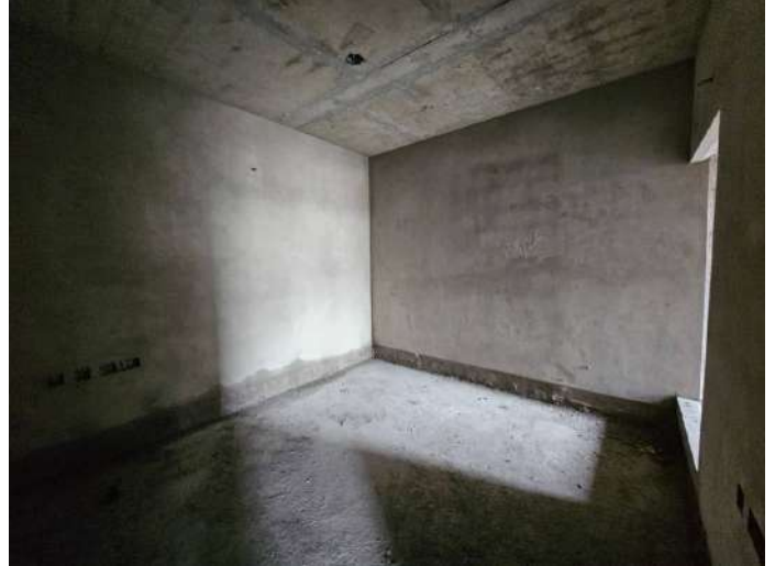
On Completion of Plastering - 6th Floor - 611
