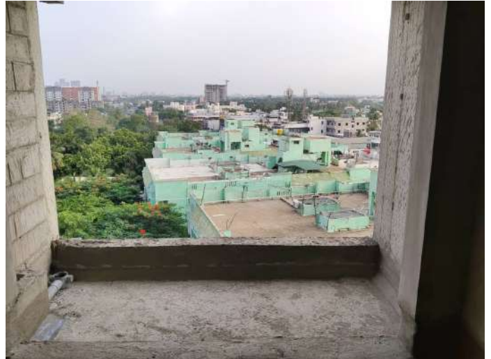
7F - Balcony Waterproofing
