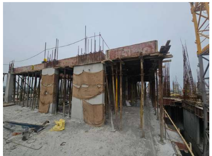
Twelfth Floor P1 - Roof Slab Shuttering
