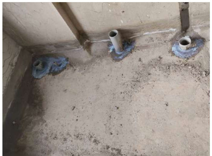
7F - Toilet Waterproofing
