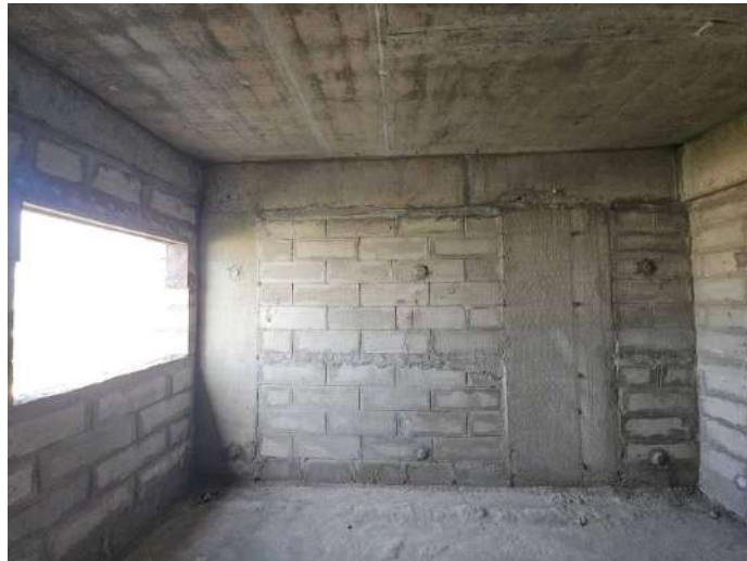
On Completion of Blockwork - 8th Floor - 801
