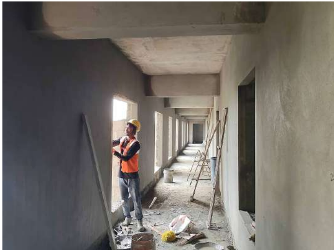
6F - Internal Plastering Corridor Area
