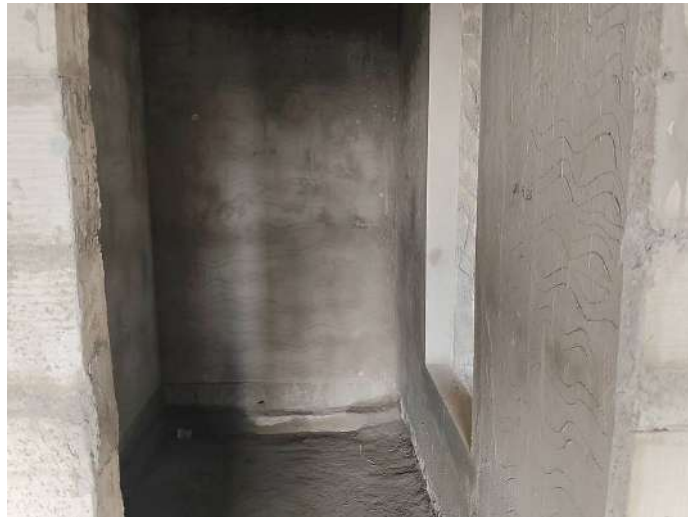
9F - Internal Plastering
