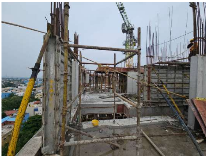
Twelfth Floor P1 - Column Shuttering
