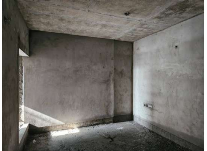
On Completion of Plastering - 6th Floor - 607
