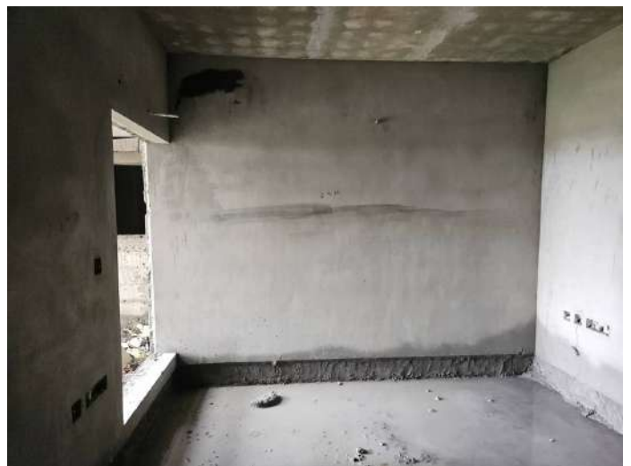
On Completion of Plastering - 6th Floor - 601
