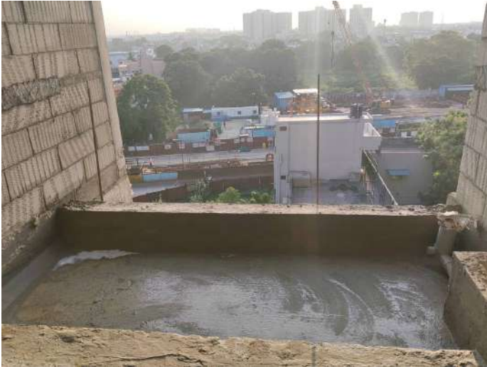
6F - Balcony Waterproofing
