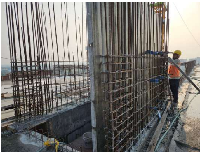
LMR - Reinforcement, Shuttering, Concreting
