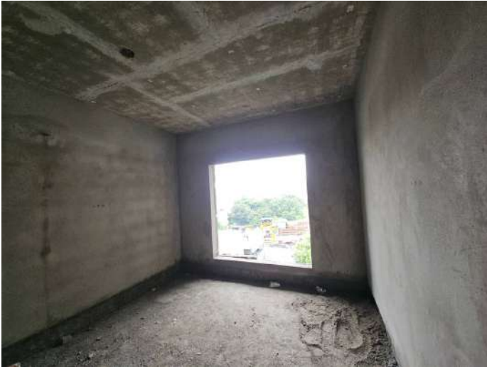
On Completion of Plastering - 6th Floor - 607
