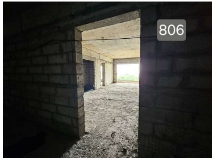
On Completion of Blockwork - 8th Floor - 806
