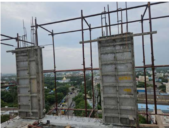
Twelfth Floor P1 - Column Shuttering
