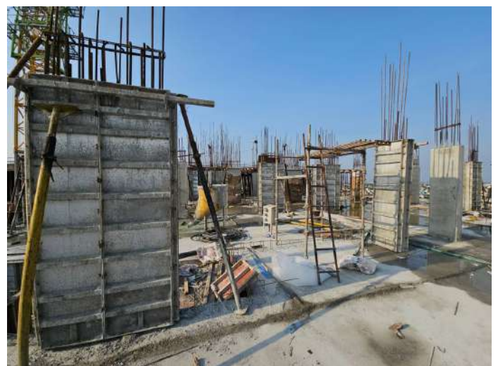
Twelfth Floor P2 - Column Shuttering
