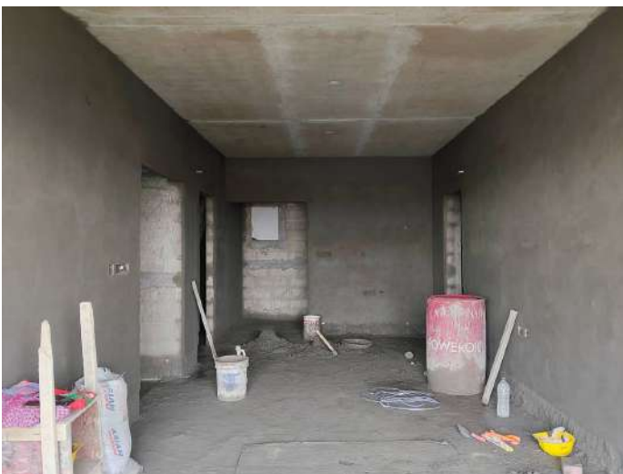
7F - Internal Plastering
