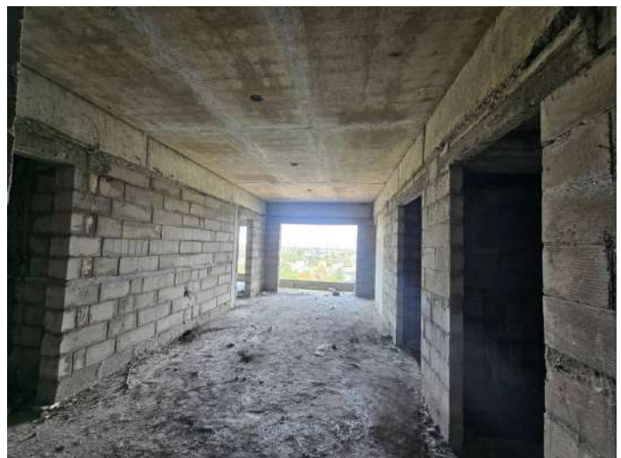
On Completion of Blockwork - 8th Floor - 802
