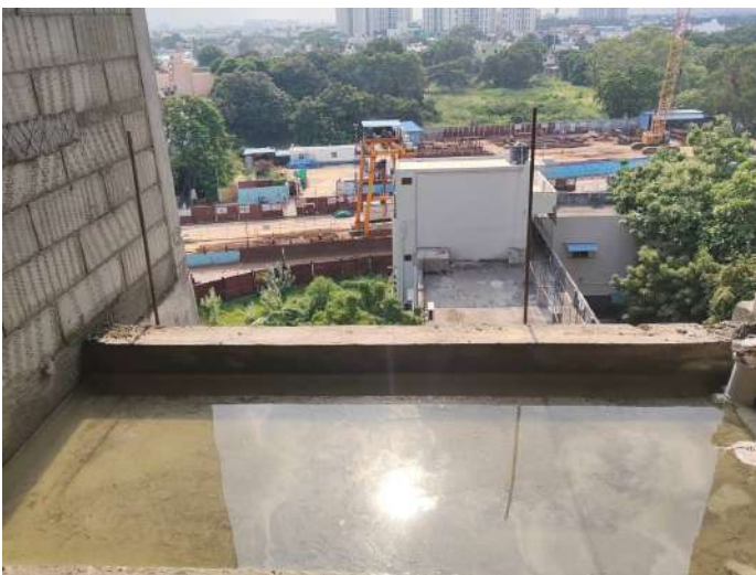
6F - Balcony Water Bond Test
