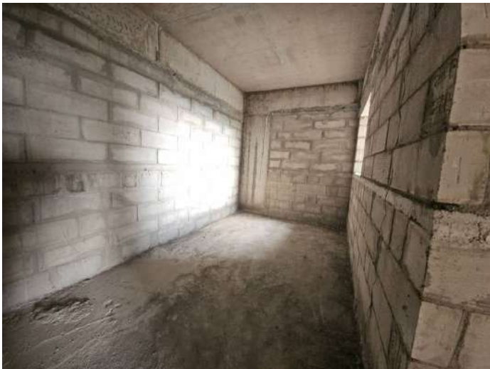
On Completion of Blockwork - 9th Floor - 906
