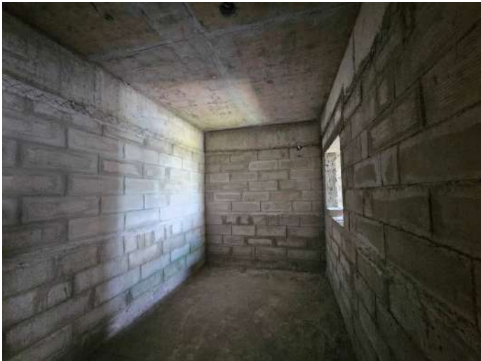
On Completion of Blockwork - 8th Floor - 807
