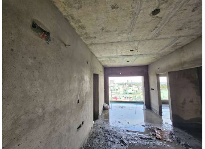
On Completion of Plastering - 6th Floor - 604
