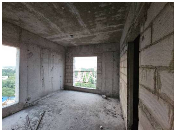
On Completion of Blockwork - 8th Floor - 808
