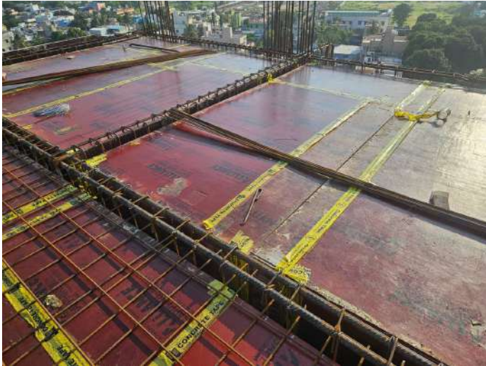
Eleventh Floor P2 - Roof Slab Shuttering
