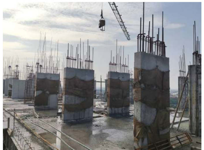
Twelfth Floor P1 - Column Concrete
