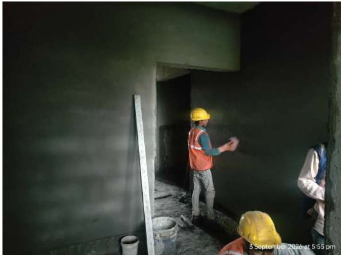
3F - Internal Plastering Corridor Area
