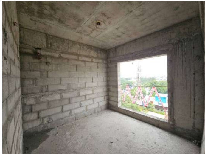
On Completion of Blockwork - 8th Floor - 809
