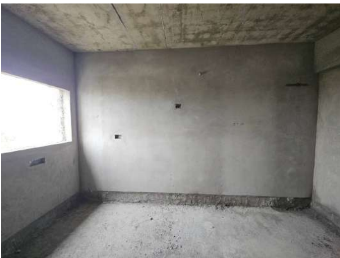
On Completion of Plastering - 6th Floor - 601
