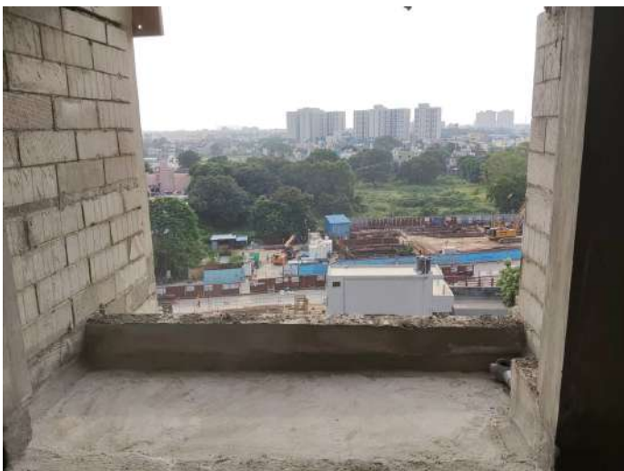
7F - Balcony Surface Cleaning
