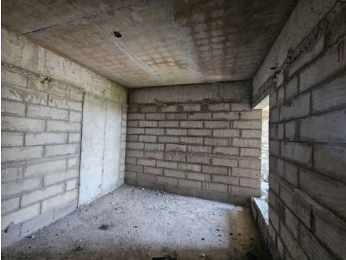
On Completion of Blockwork - 8th Floor - 802
