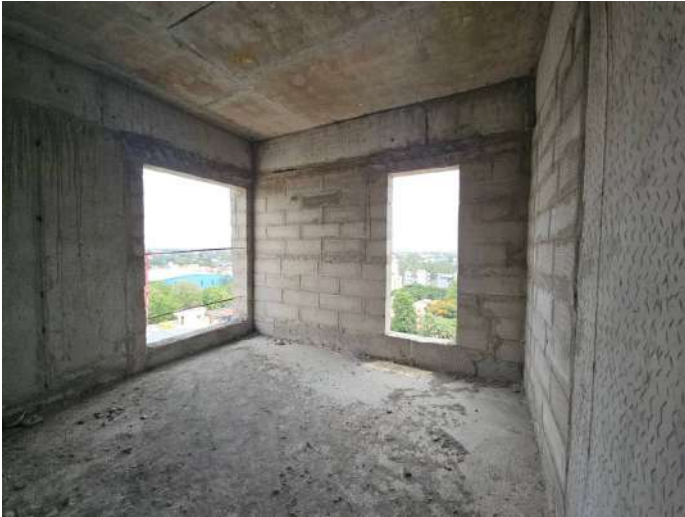
On Completion of Blockwork - 8th Floor - 813
