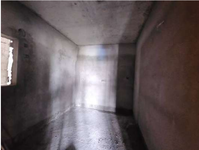
On Completion of Plastering - 6th Floor - 609
