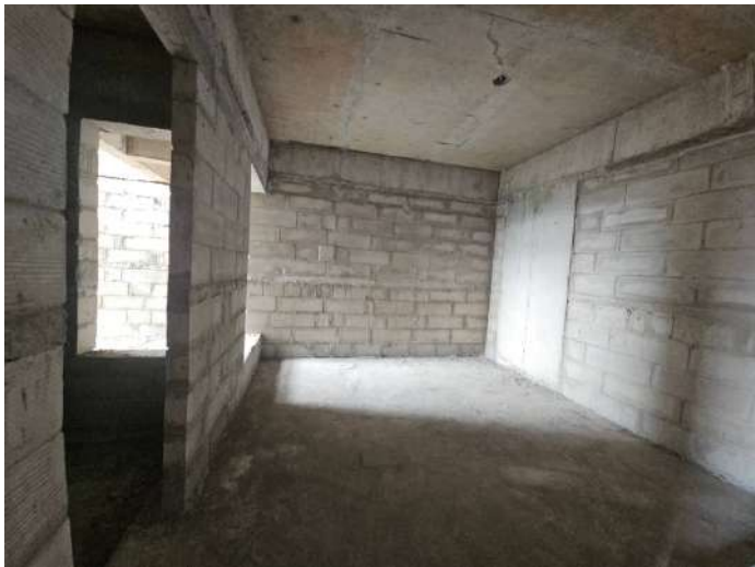
On Completion of Blockwork - 9th Floor - 906
