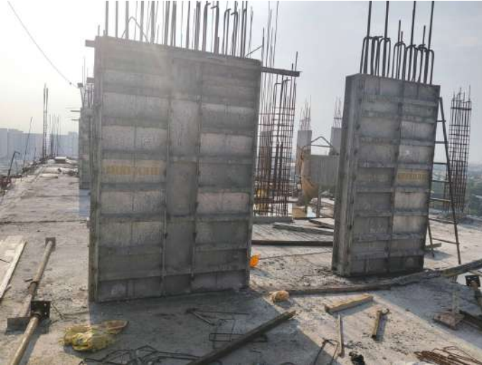
Twelfth Floor P1 - Column Shuttering
