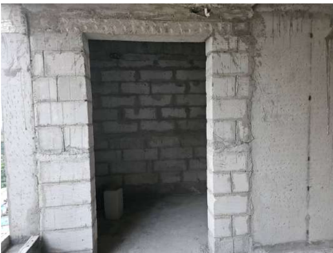
On Completion of Blockwork - 8th Floor - 808
