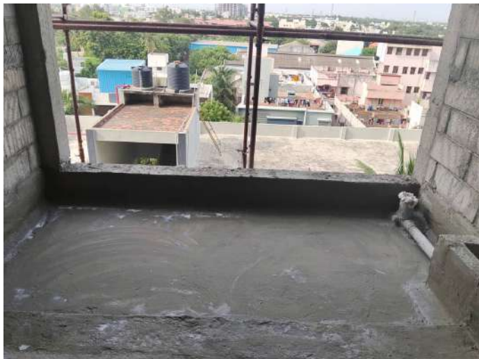
6F - Balcony Waterproofing
