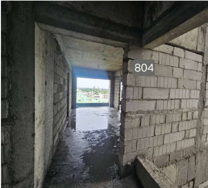
On Completion of Blockwork - 8th Floor - 804
