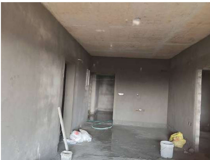
7F - Internal Plastering
