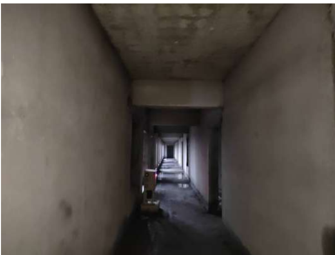
5F - Internal Plastering Corridor Area
