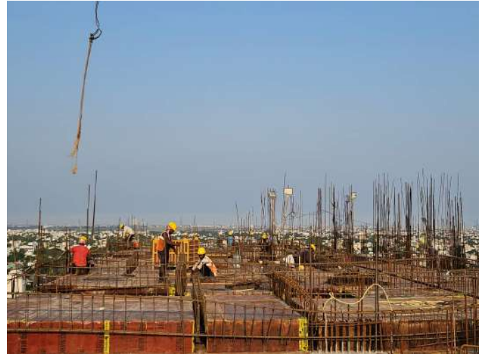
Twelfth Floor P1 - Slab & Beam Reinforcement
