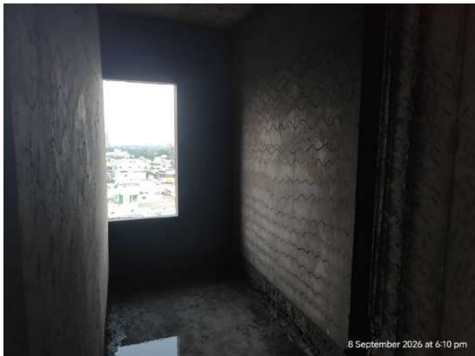
8F - Internal Plastering
