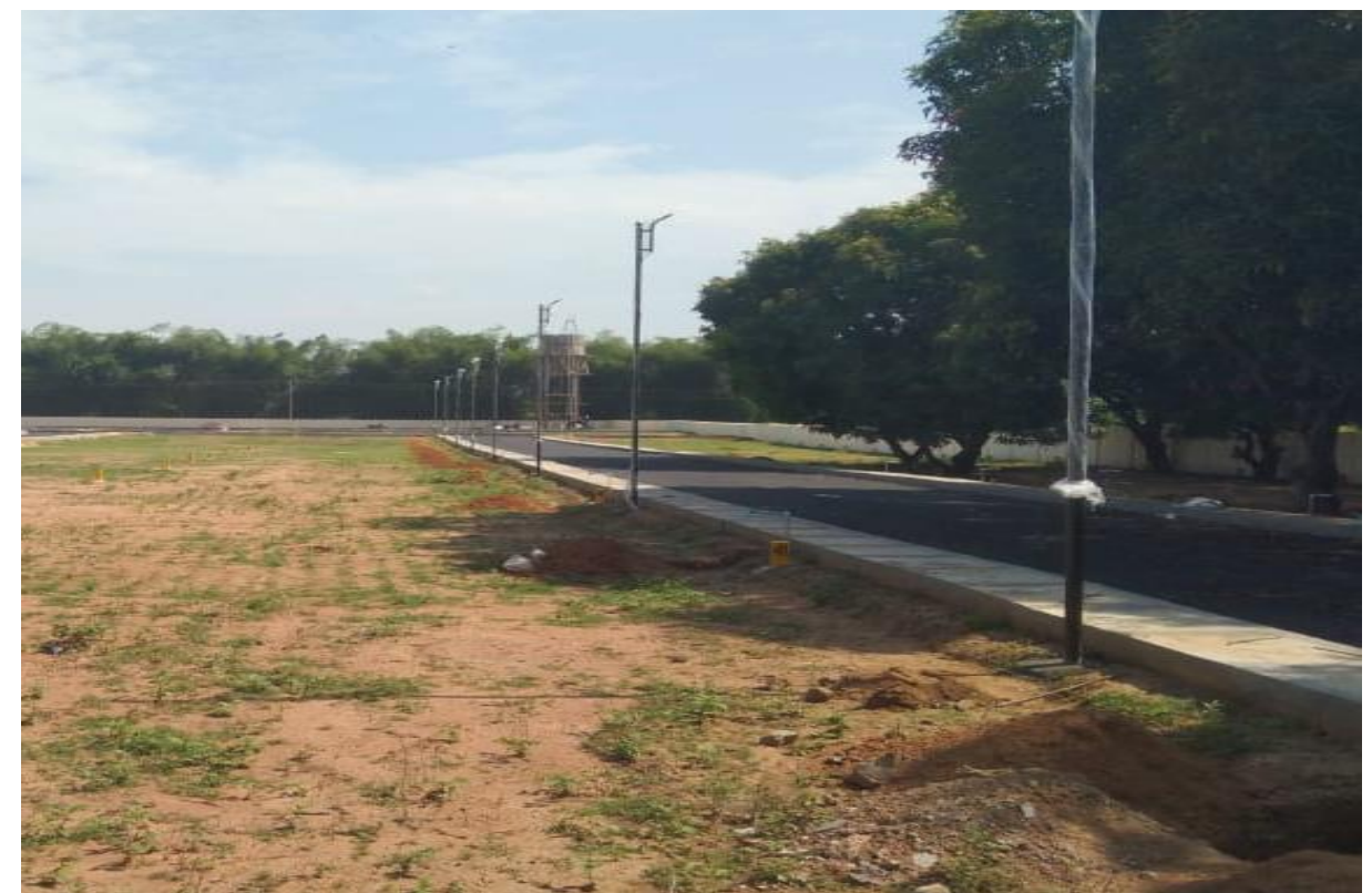
STREET LAMP POST FIXING WORK IN PROGRESS
