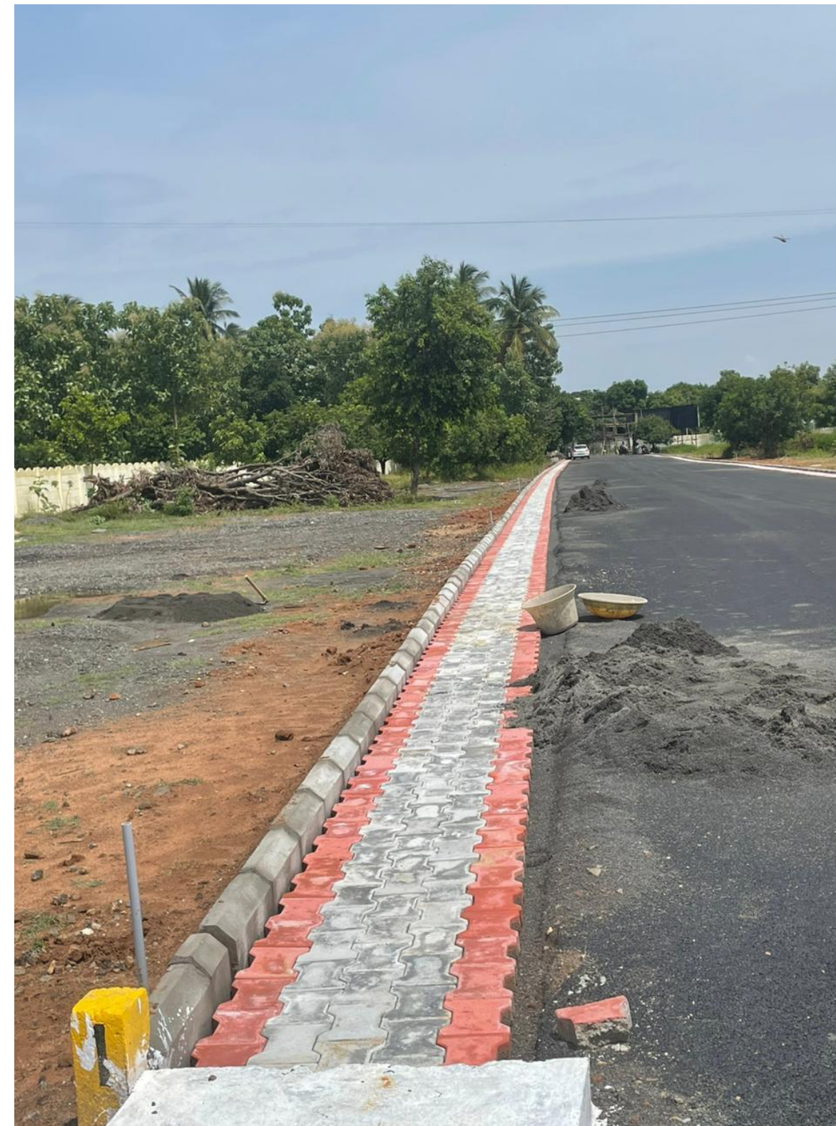
ROAD SIDE PATHWAY PAVER LAYING WORK
