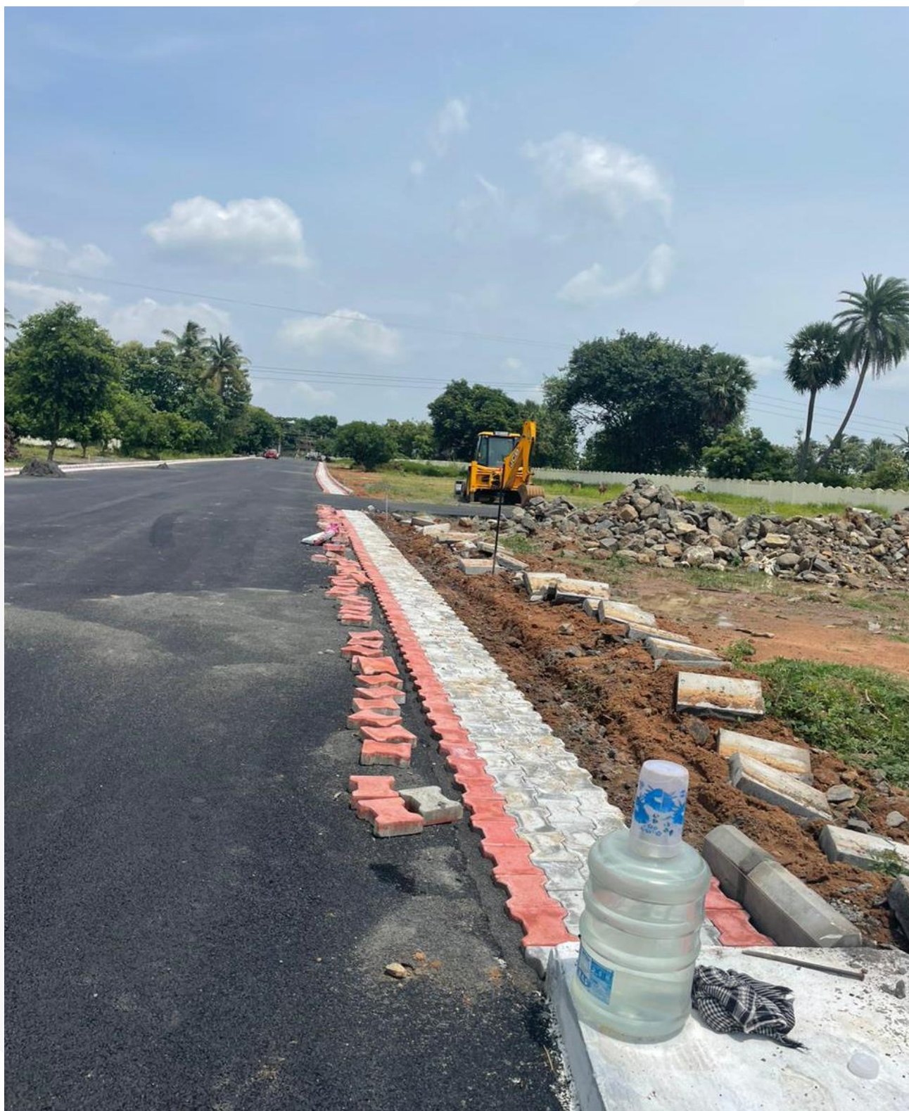
ROAD SIDE PATHWAY PAVER LAYING WORK
