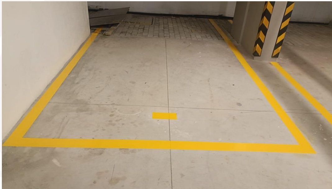
Car Park Demarcation Work Completed
