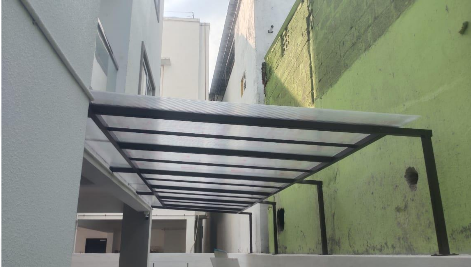
Car Park Covering Work Completed
