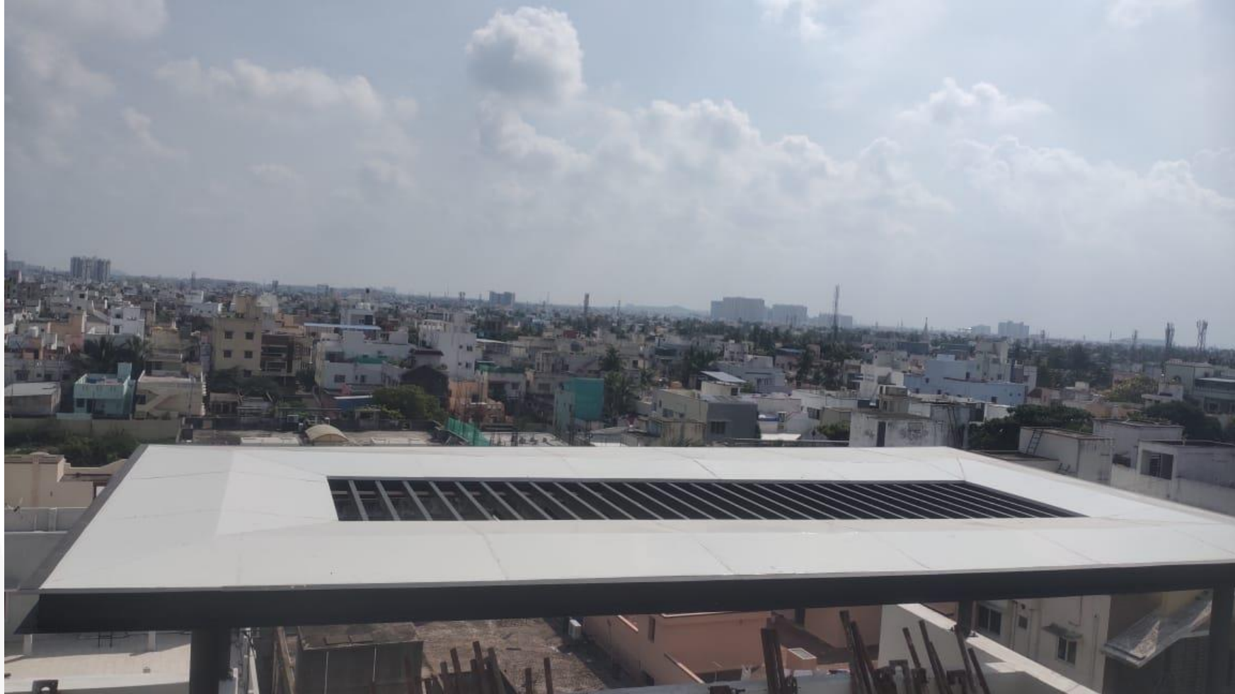
Terrace Pergola Works Completed
