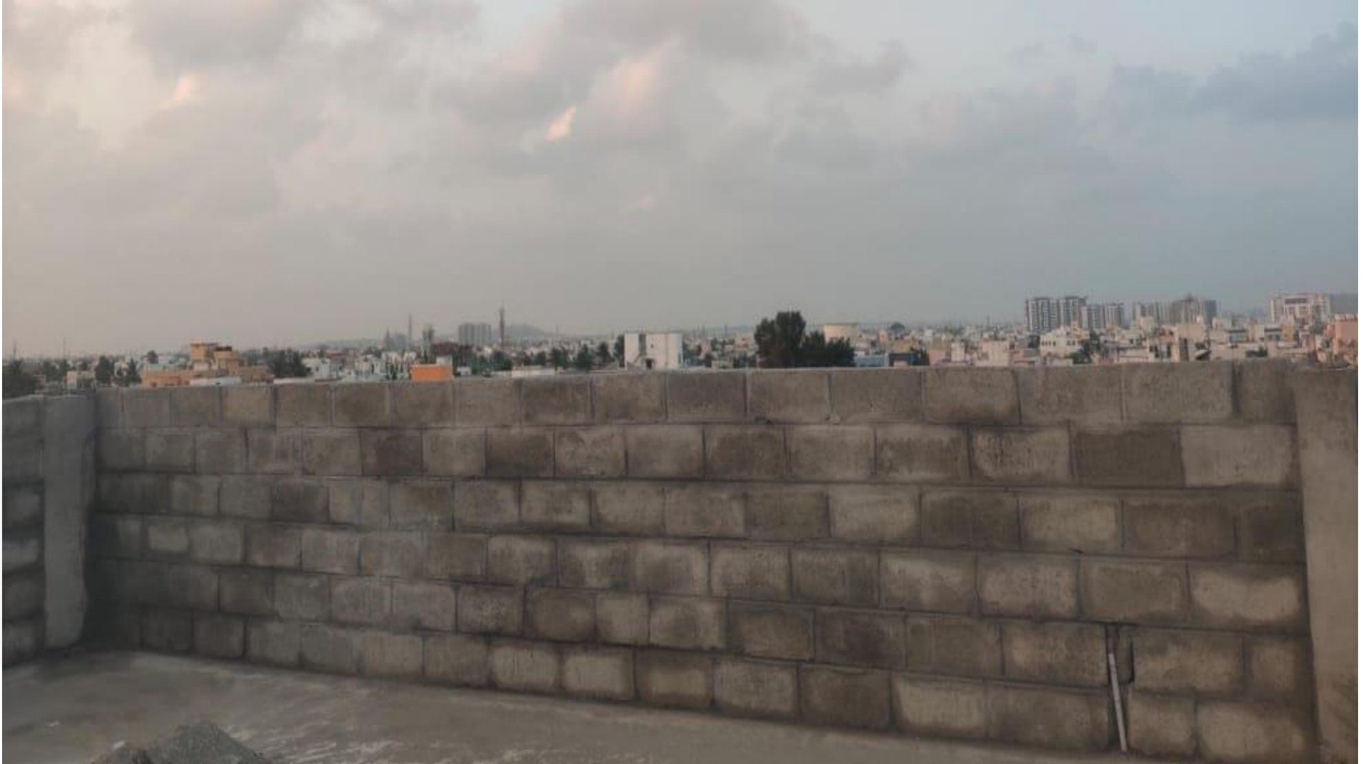
Terrace Floor Parapet Wall Masonry Work Completed
