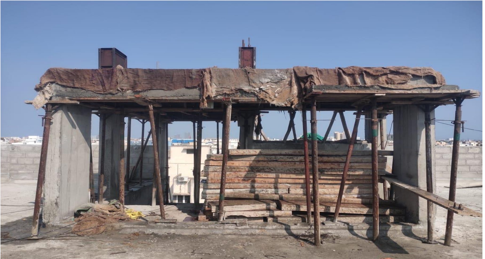
Terrace SHR Roof Work Completed
