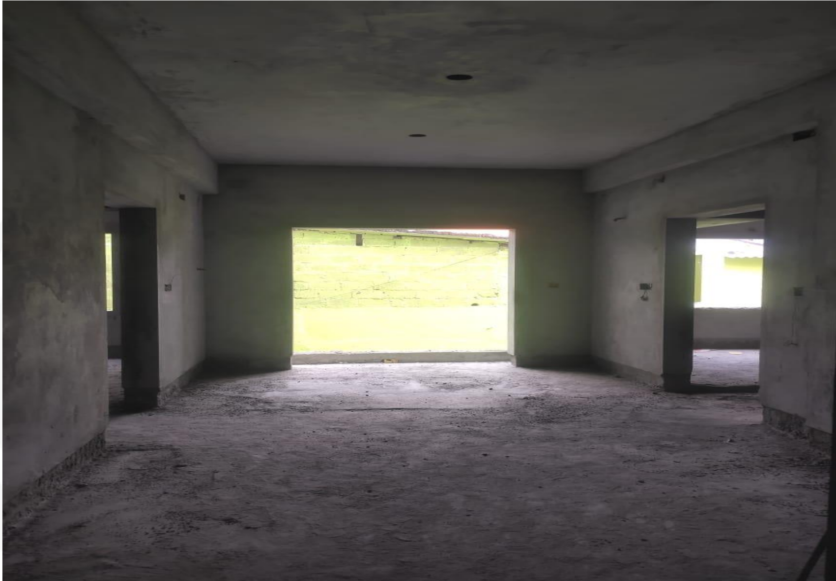
Third Floor Plastering Work Completed
