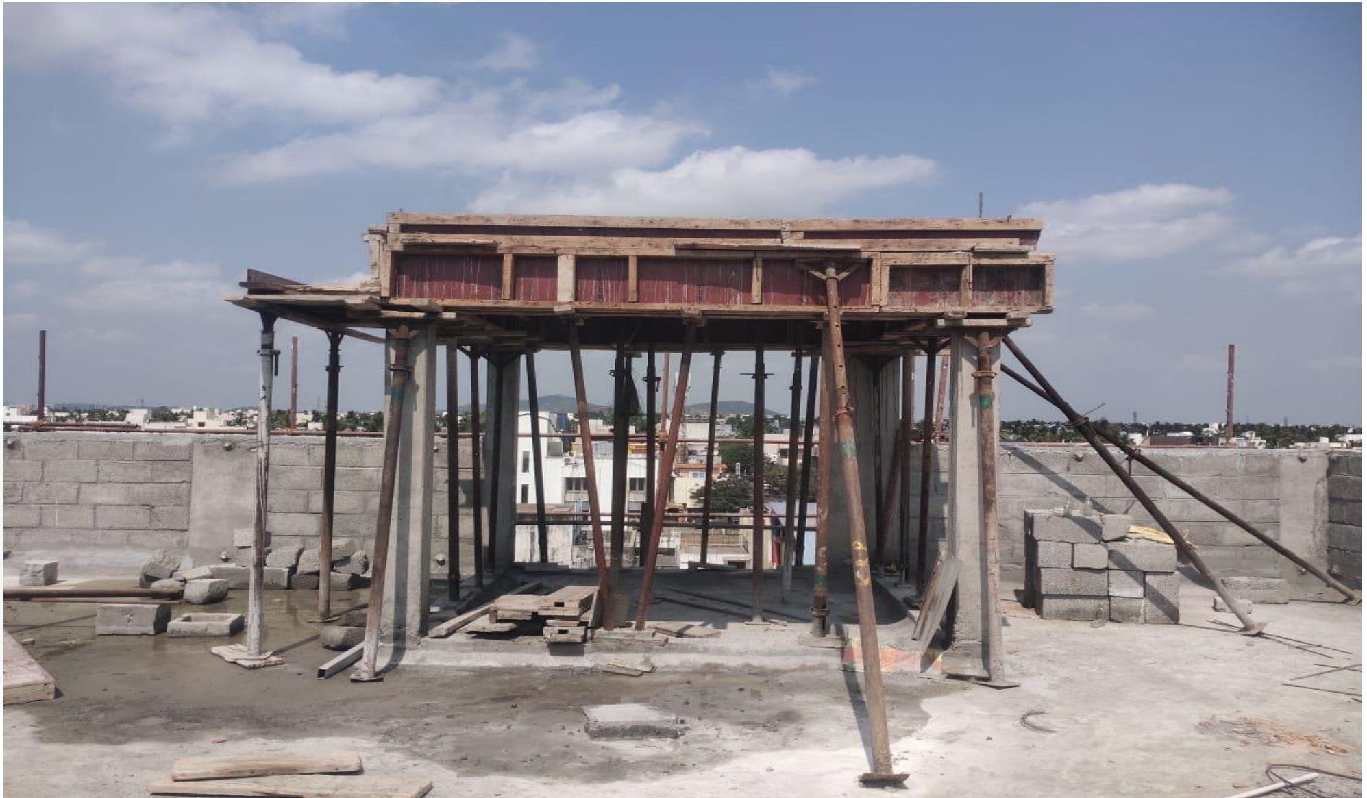
Terrace Toilet Slab Work Completed
