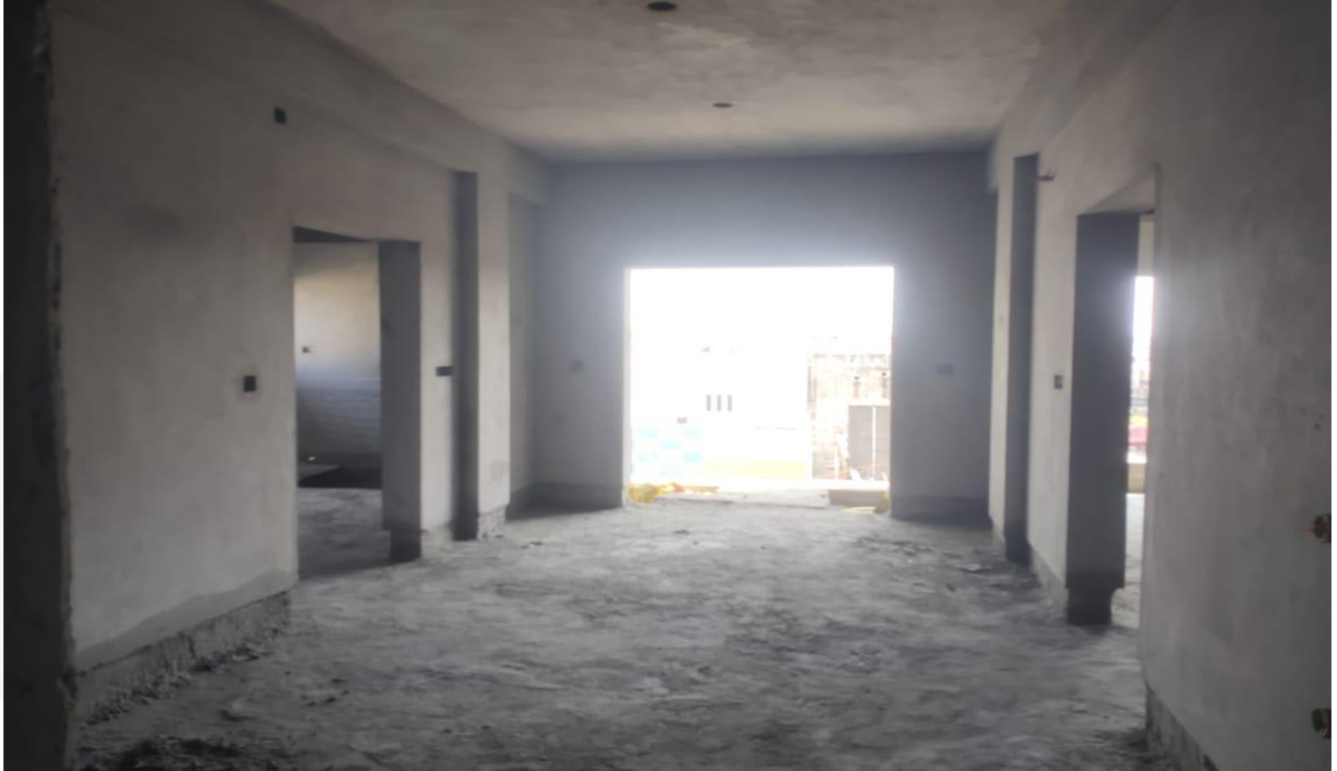
Fourth Floor Plastering Work Completed
