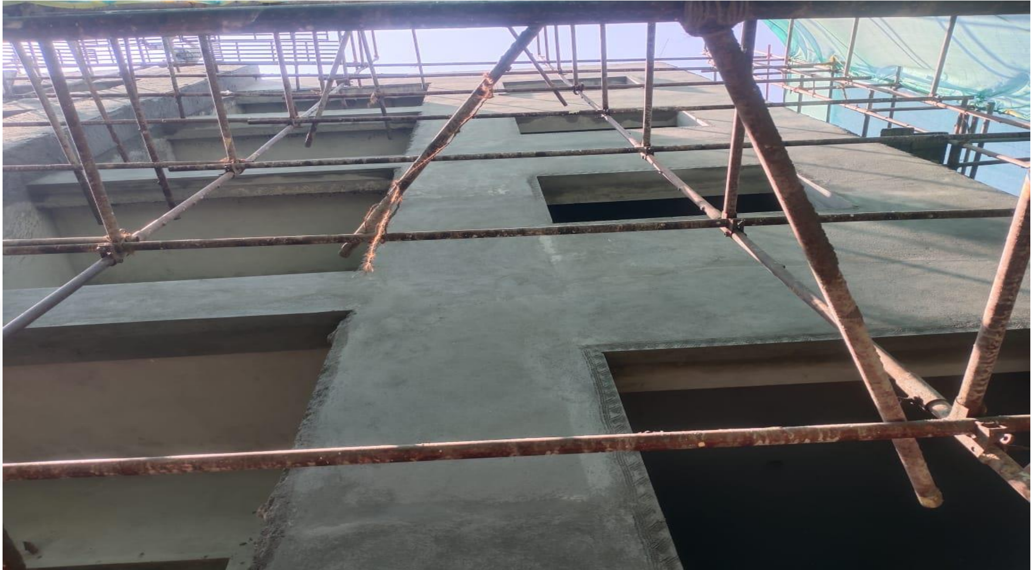
External Plastering Work In progress -Northside
