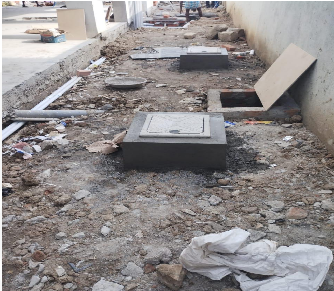
External stilt floor Electrical earth pit chamber work in progress
