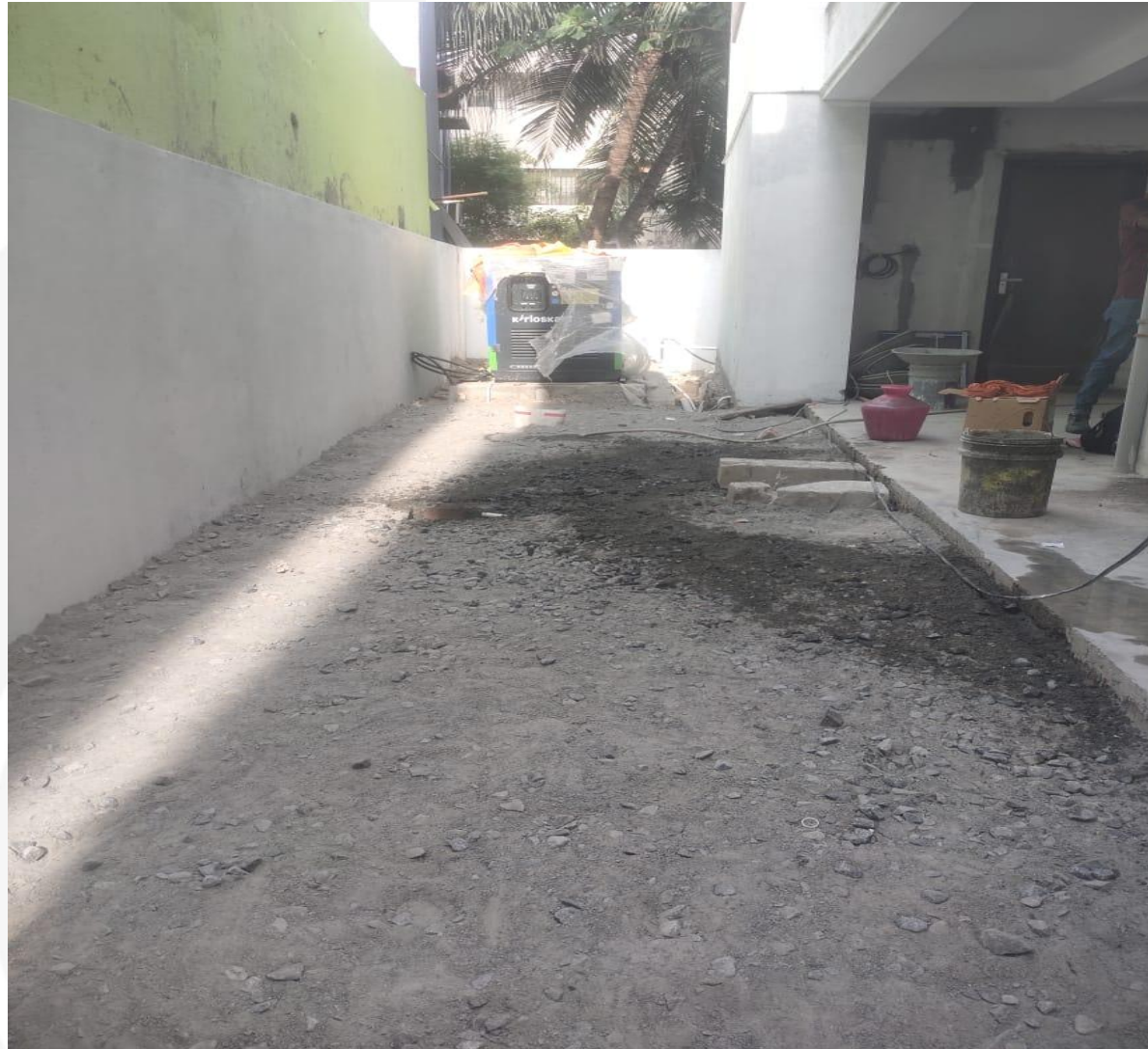
Stilt floor paver area WMM filling work in progress
