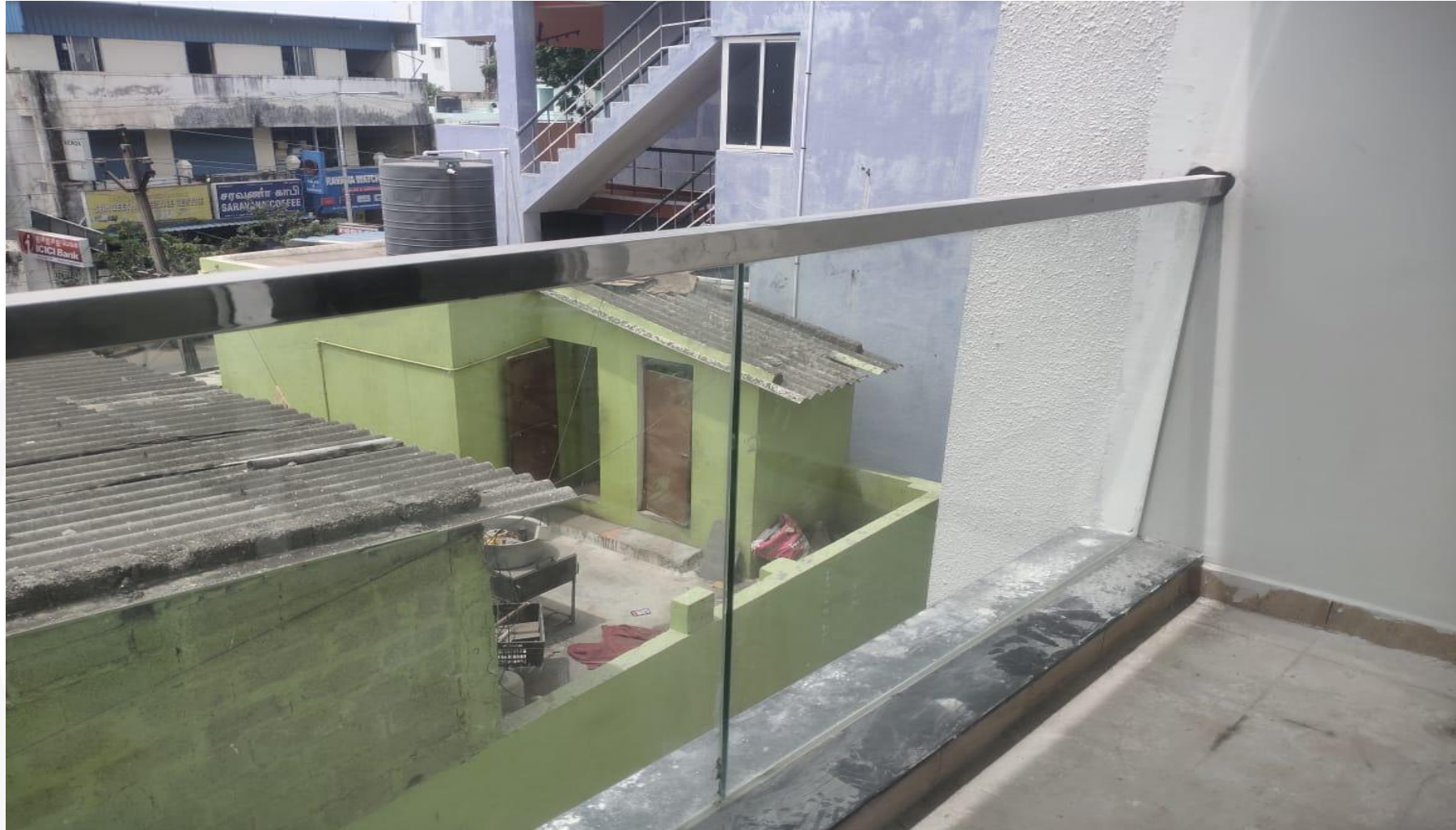
Balcony Hand rail work completed
