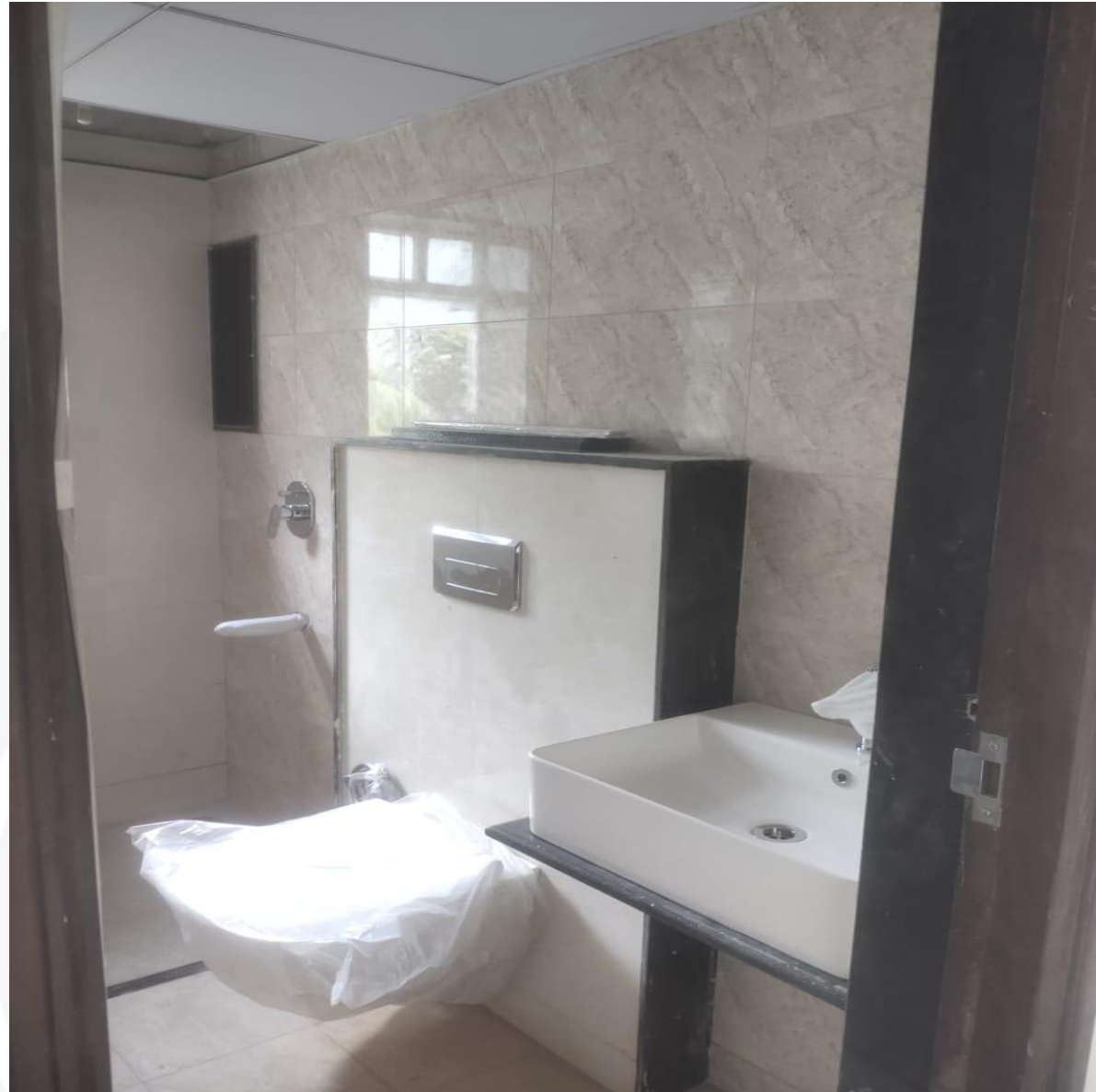
Toilet CP fittings fixing Work in progress
