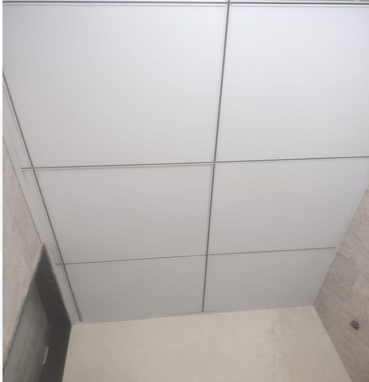
Toilet inner false ceiling Work in progress
