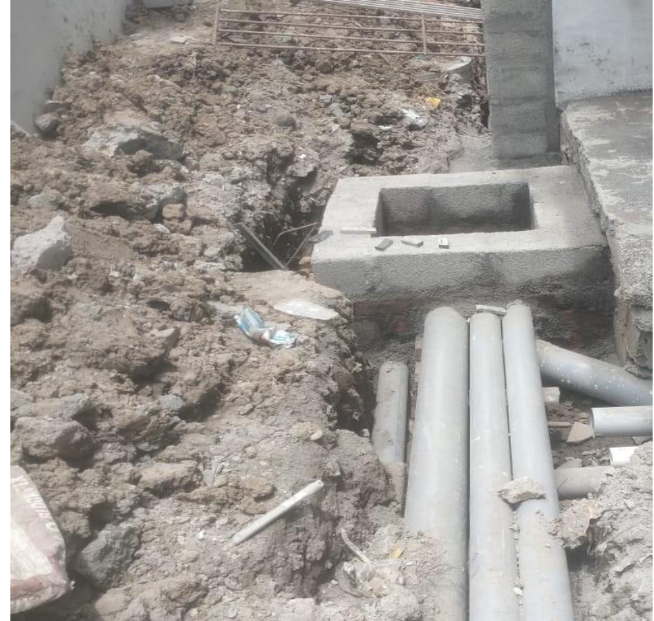
East side External plumbing Shaft plumbing pipe line work & chamber work in progress
