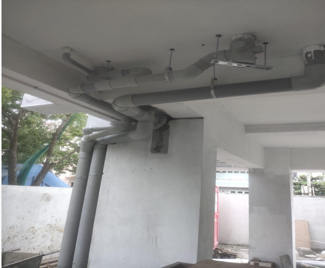
East side External plumbing Shaft plumbing pipe line work & chamber work in progress
