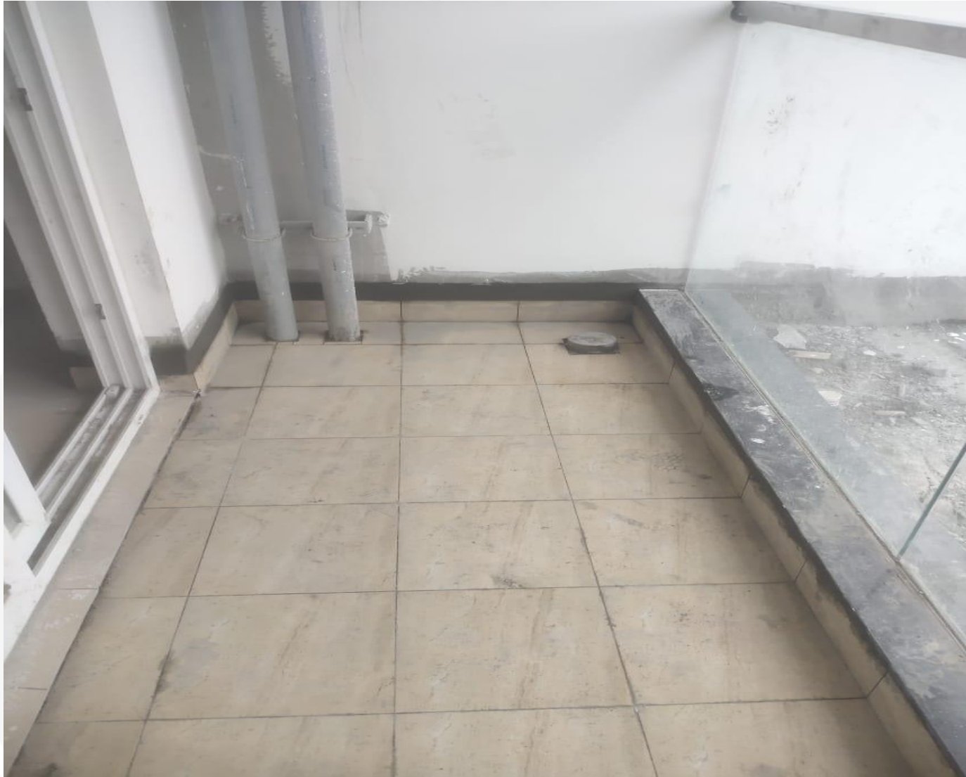
Balcony flooring Tiling Work Completed
