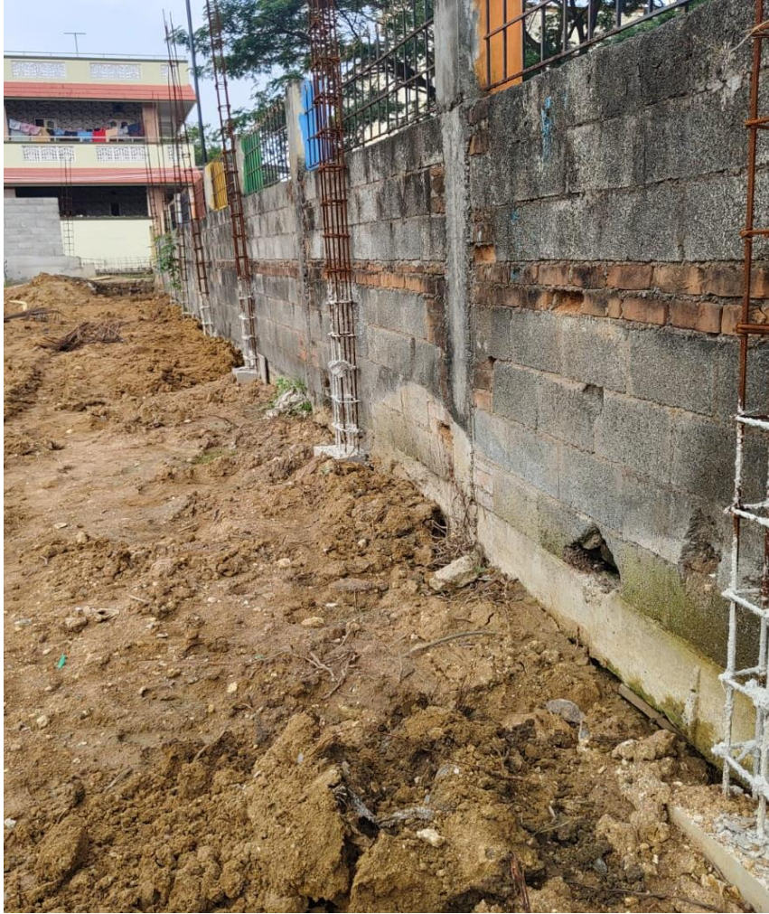
East Side Compound Wall Footing & Column Concrete Work in Progress
