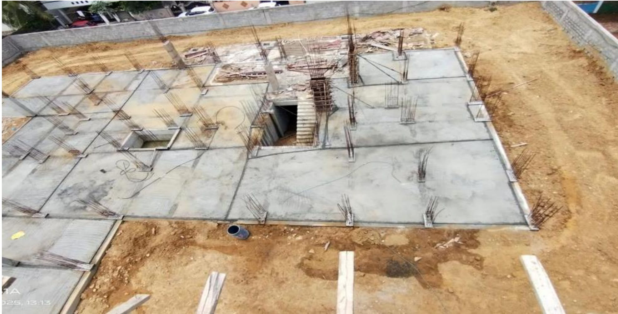
Block-2- Pour 1 - Stilt Floor Pcc Work Completed
