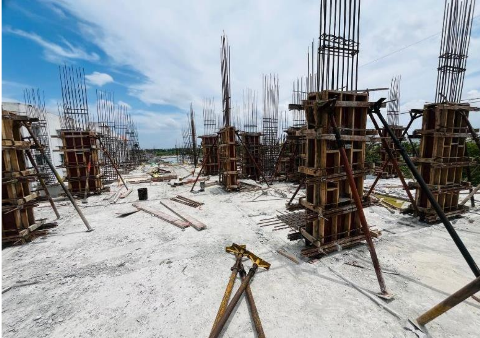
Block-4- Third Floor Column Shuttering & Concrete Work in Progress
