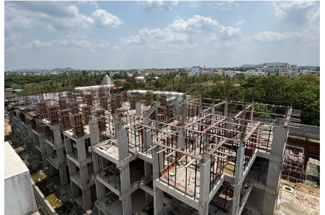
Block-4- Pour 1- Fourth Floor Slab Shuttering Work in Progress
