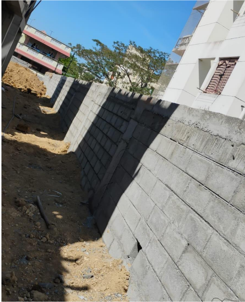
East Side Compound Wall Block Work Completed & Coping Beam concrete Work in Progress
