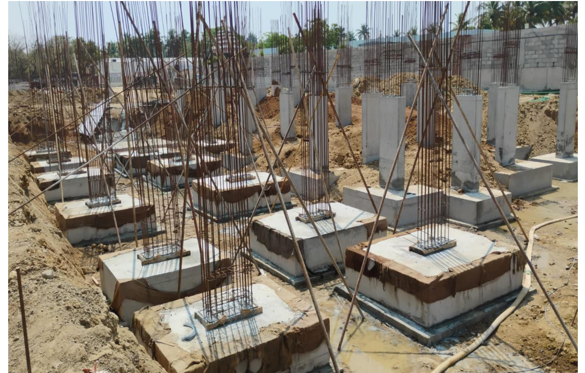
Block-1-Pour 2 Sub Structure Column Concrete Work in Progress
