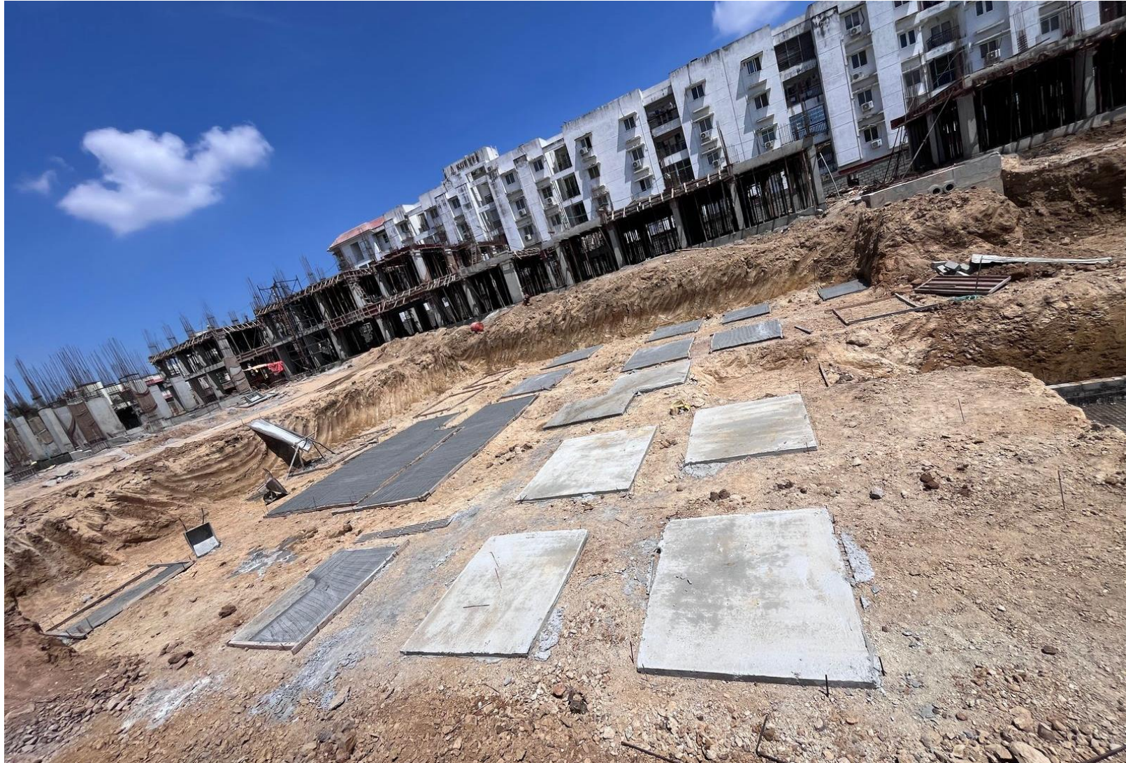
Block-2-Pour 3-Footing PCC work in progress
