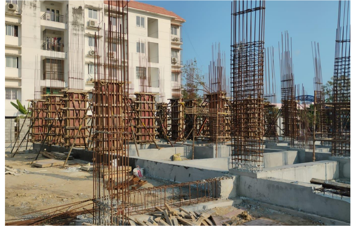
Block-1-Pour 1 Stilt Floor Column shuttering & concrete Work in Progress
