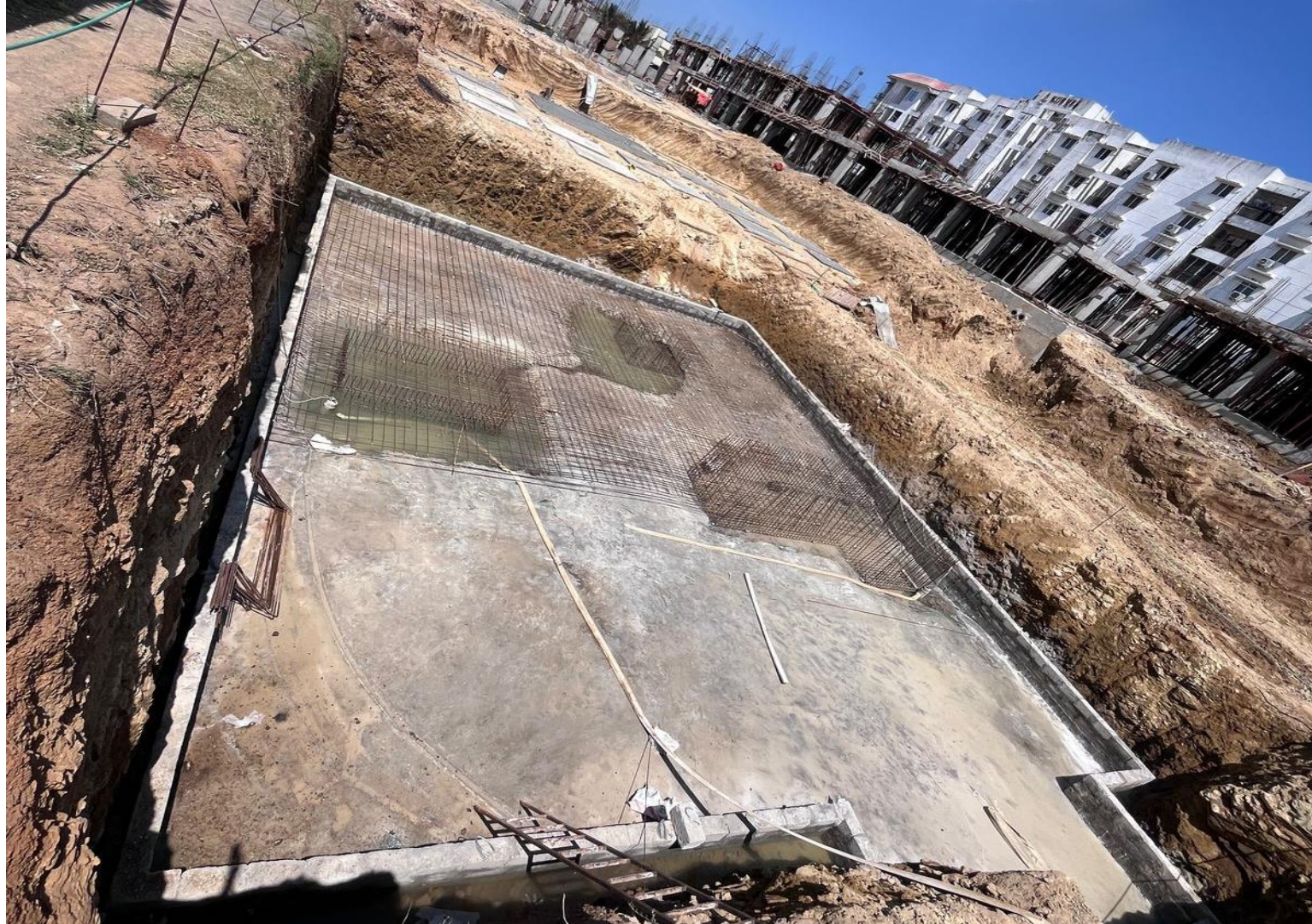
Block-1-STP Raft Reinforcement Work in Progress
