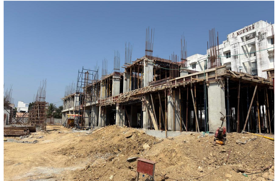
Block-3-Pour 1-Second Floor Slab Shuttering & Reinforcement Work in Progress
