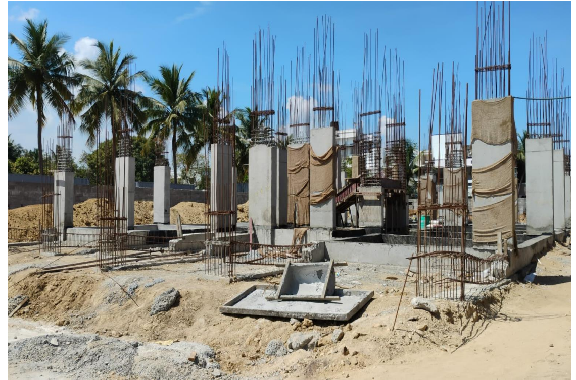
Block-2-Pour 1&2-Stilt Floor Column Concrete work in progress
