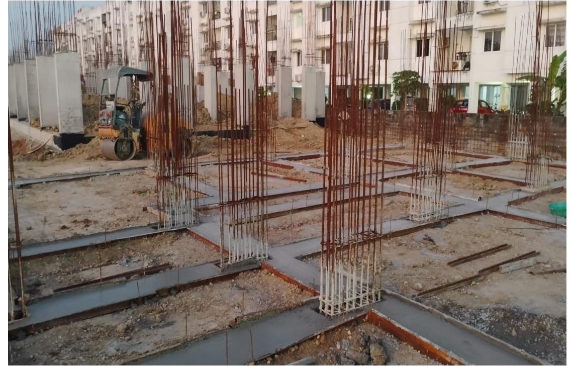
Block-1-Pour 1 Plinth beam Pcc Work in Progress
