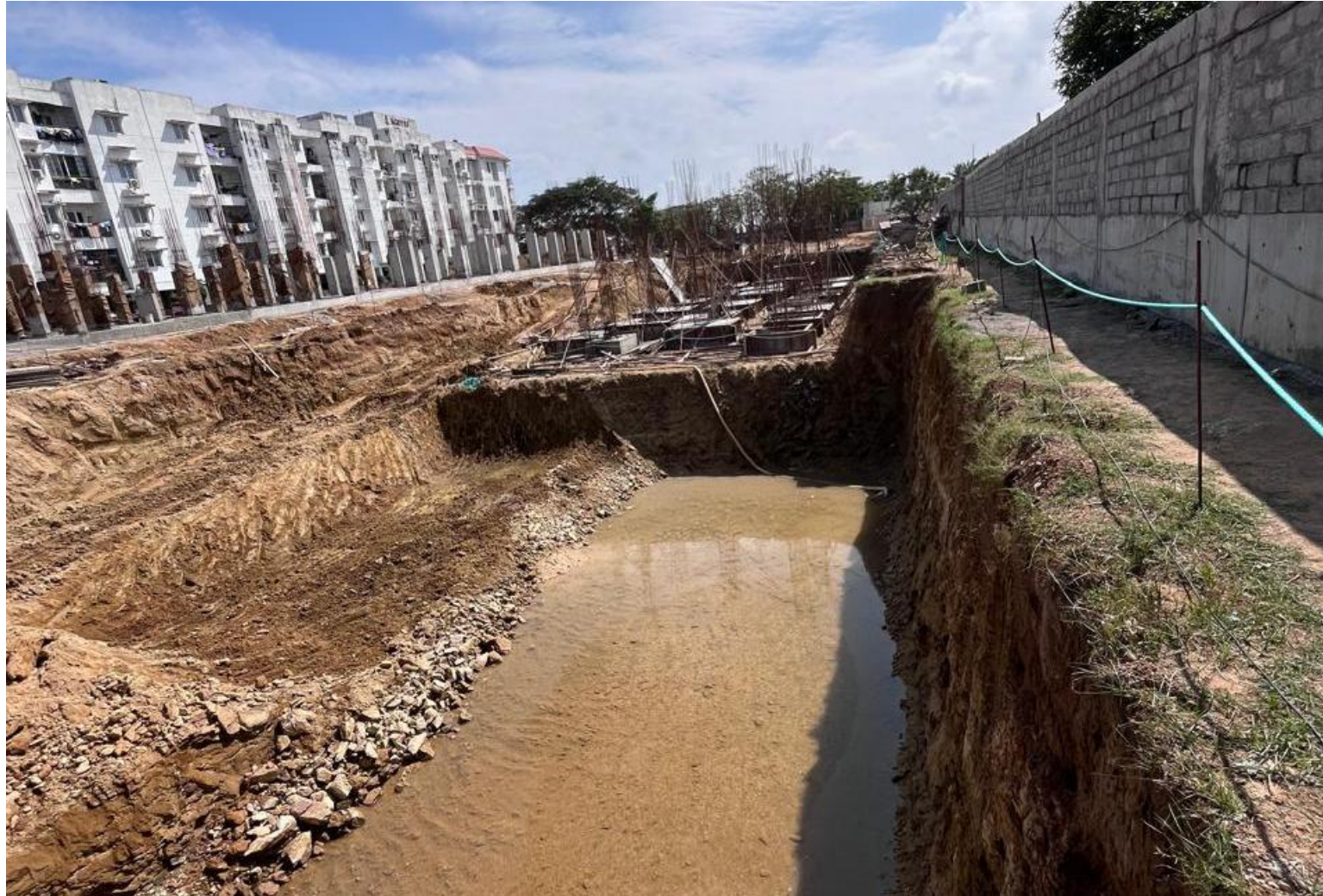
Block-1-STP Excavation Work in Progress
