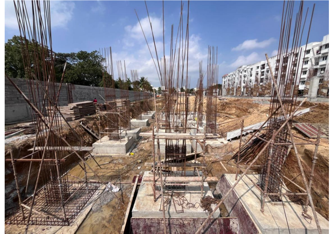
Block-1-Pour 2 Footing Concrete Work in Progress
