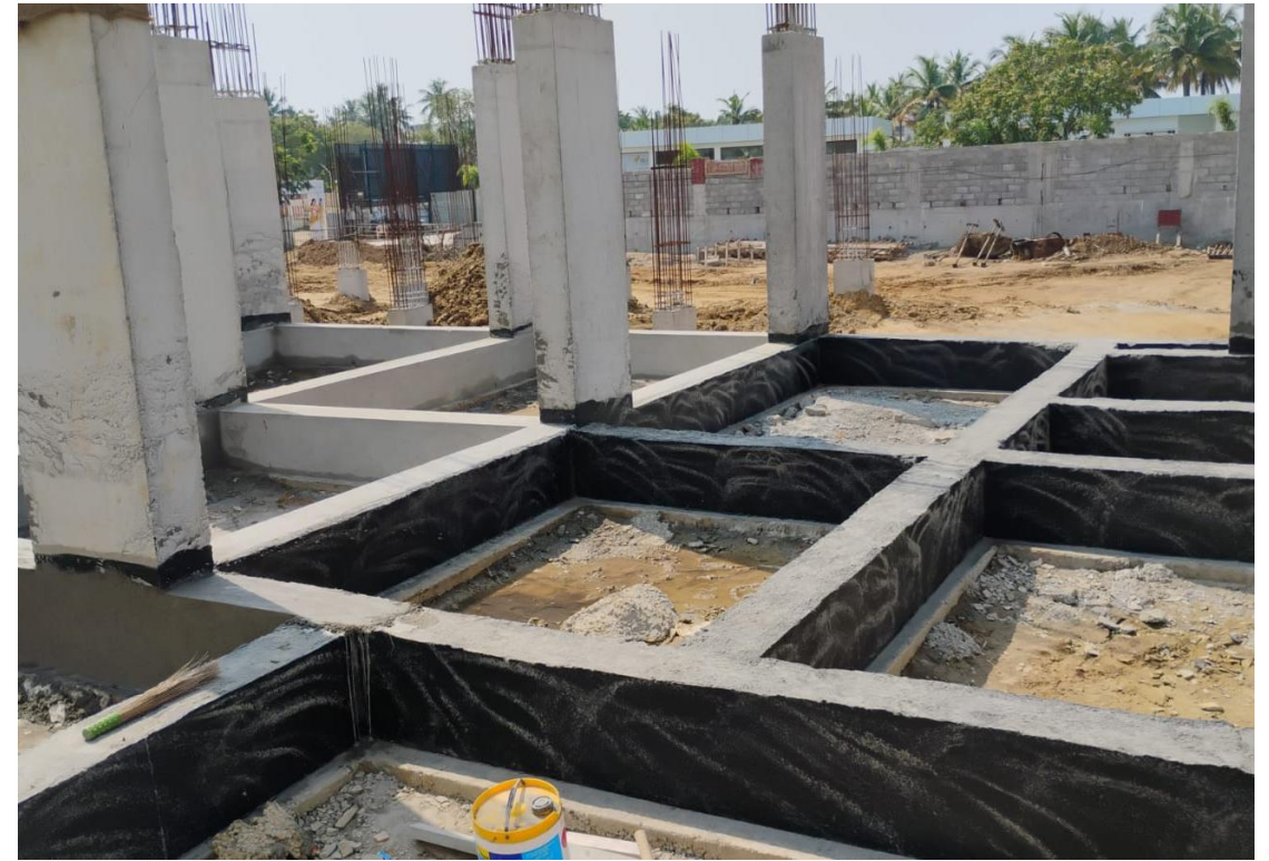
Block-4- Stilt floor column concrete Work completed & DPC work in Progress
