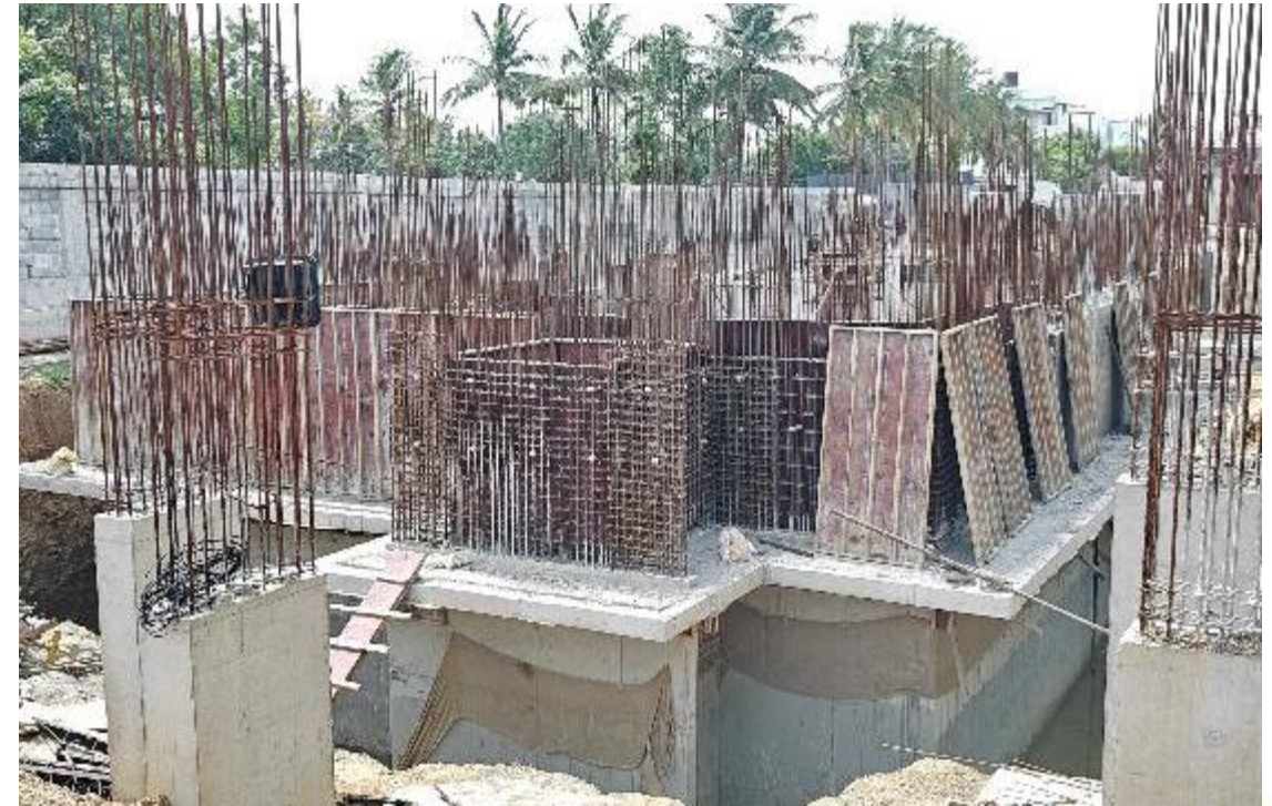
Block-1-STP Third Lift Wall Concrete Work in progress
