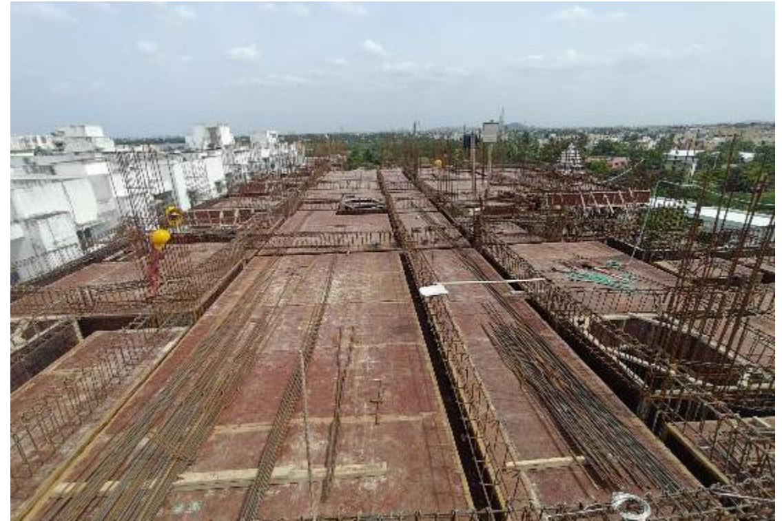
Block-4- Pour 1- Fifth Floor Beam Reinforcement Work in Progress
