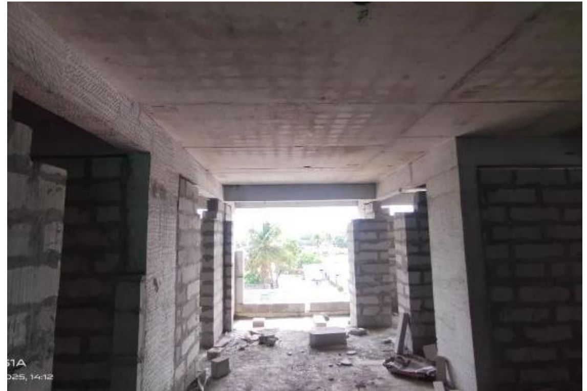
Block-3- First Floor Block work in Progress
