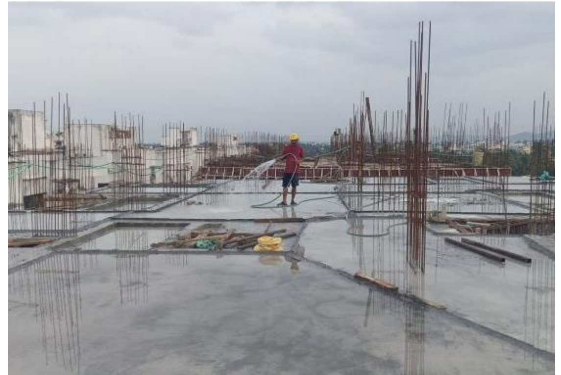
Block-3-Pour 2- Fifth Floor Slab Concrete Completed
