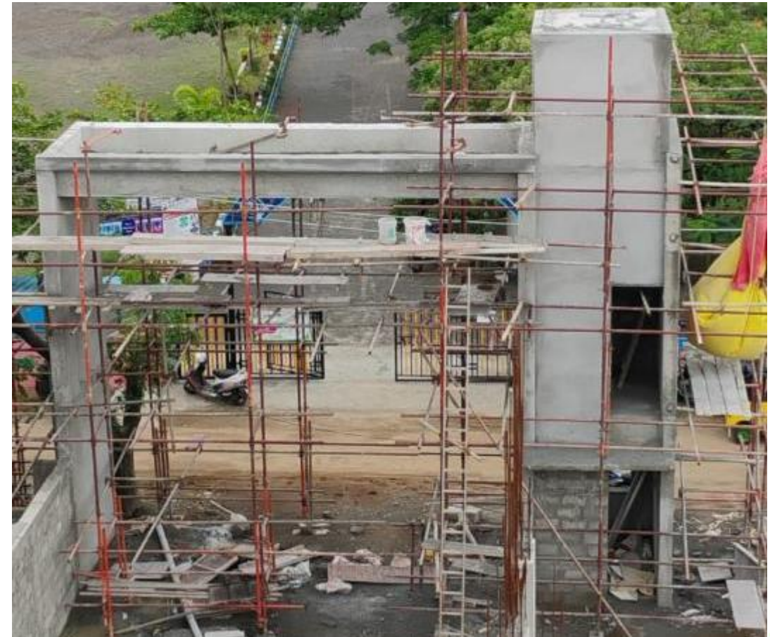
Exit Arch Outer Plastering work in Progress
