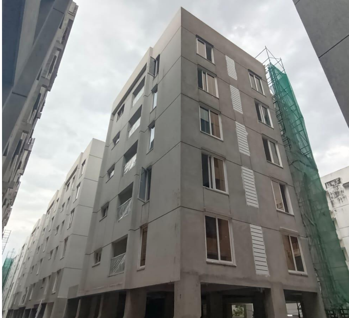
Block-04 – Elevation View
