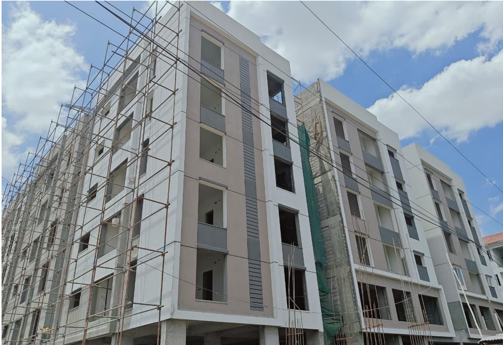
Block-01 – Elevation View
