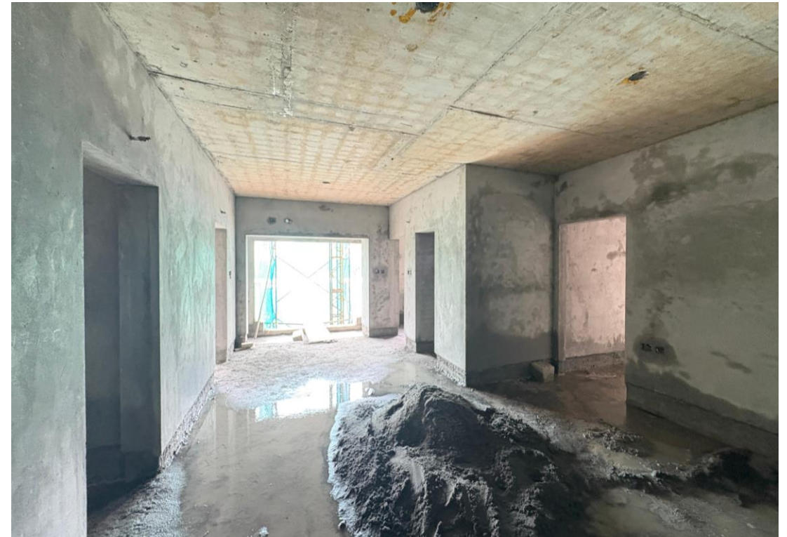
Block-3- First Floor Wall Plastering work in Progress
