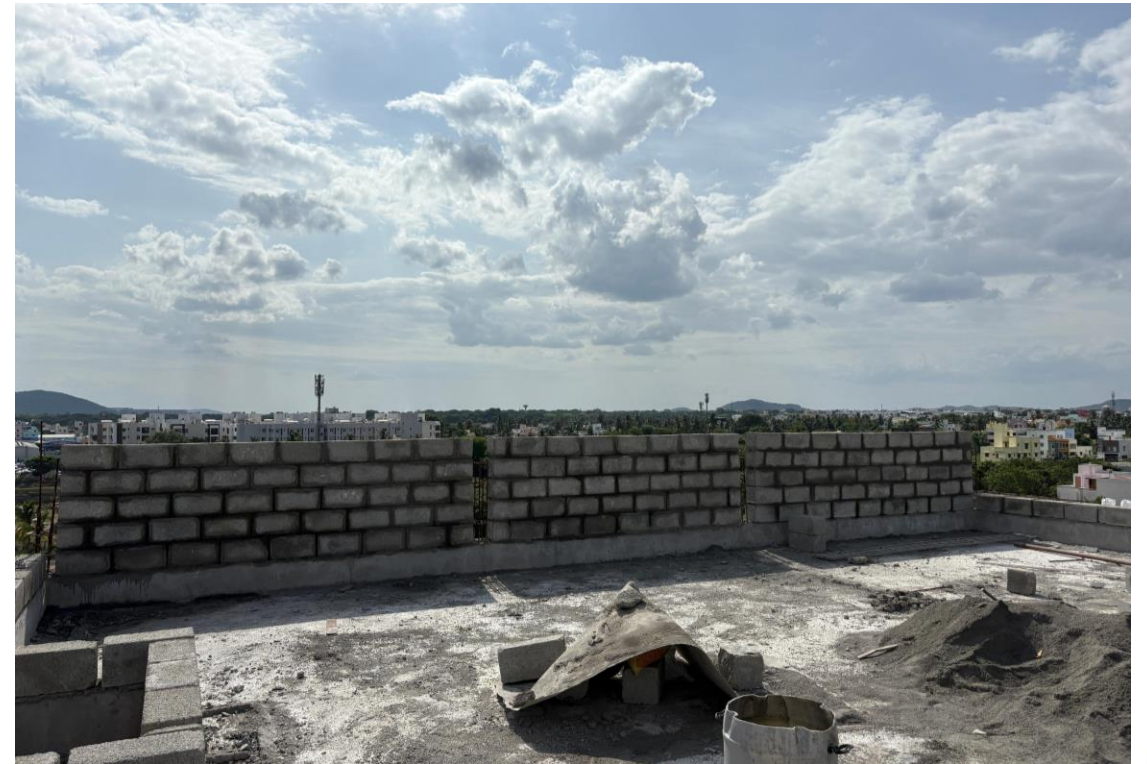
Block-3 Terrace Floor Parapet Blockwork in Progress
