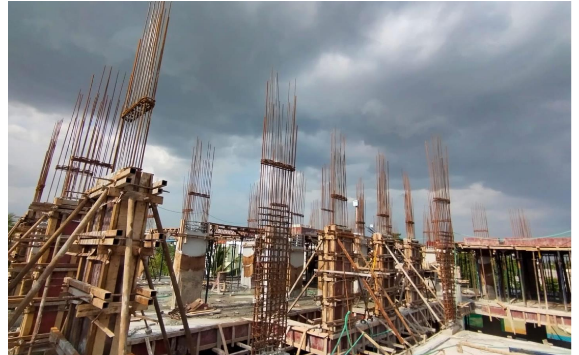
Block-2- Pour 1 – Third Floor Slab Shuttering Work in Progress
