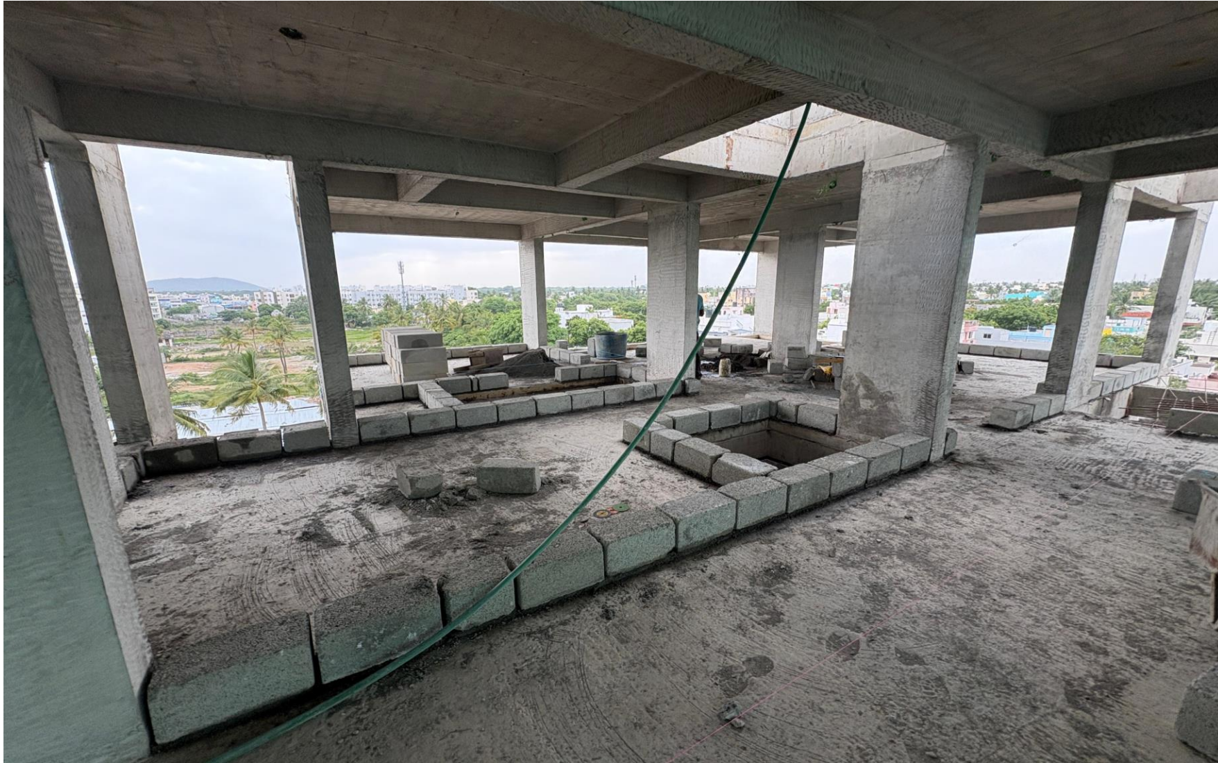
Block-3 Fifth Floor Blockwork Layout Commenced
