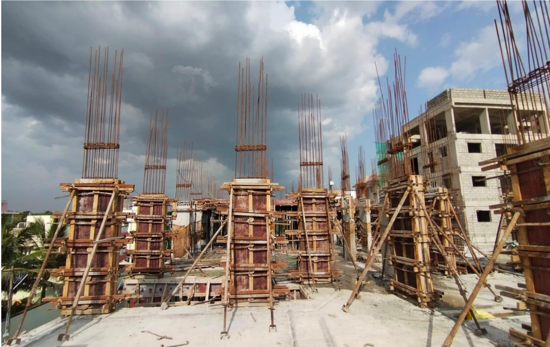
Block-2- Pour 1 – Second Floor Column Concrete Work in Progress
