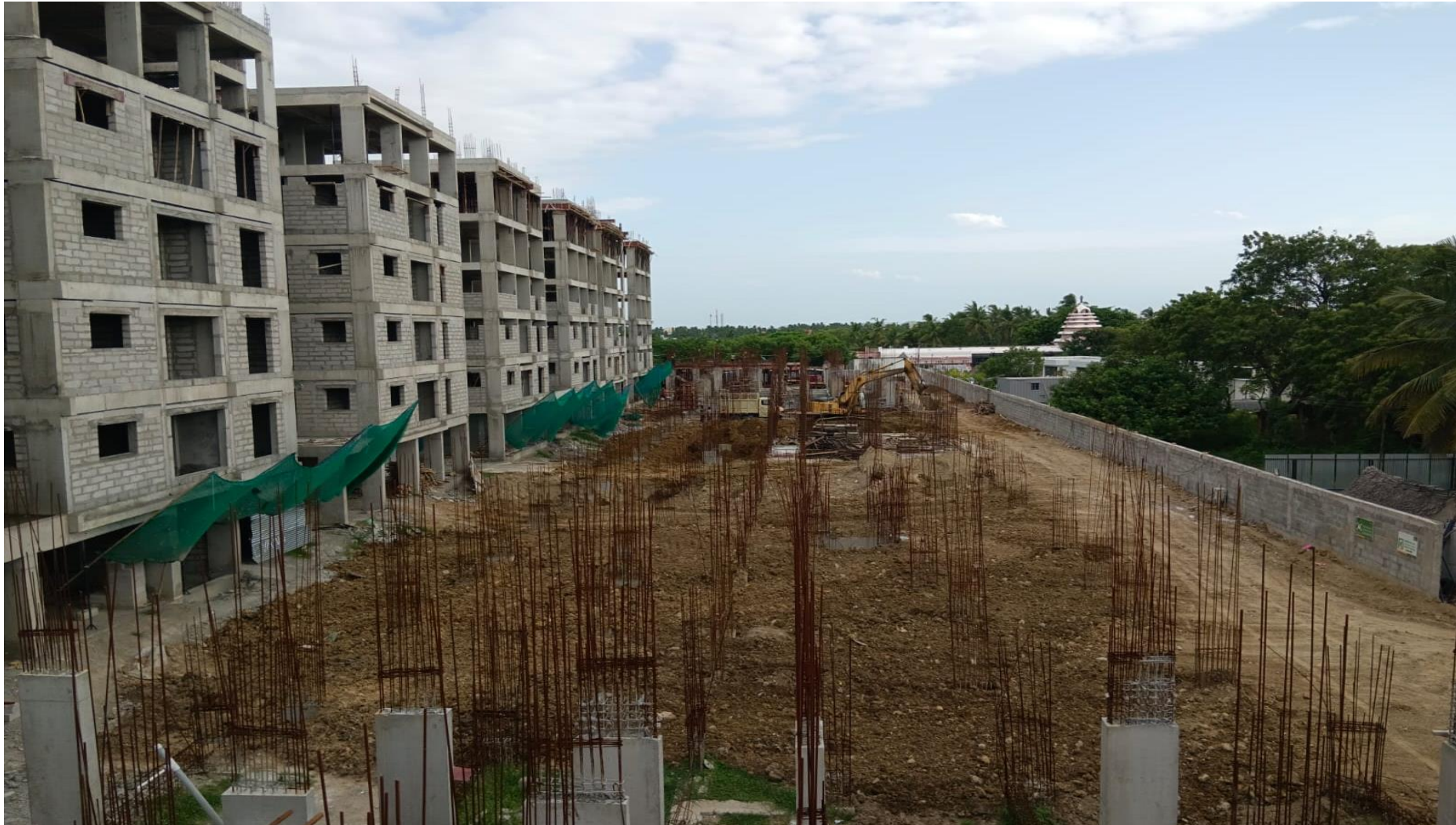
Block-2-Pour 2- Soil Filling Work in progress
