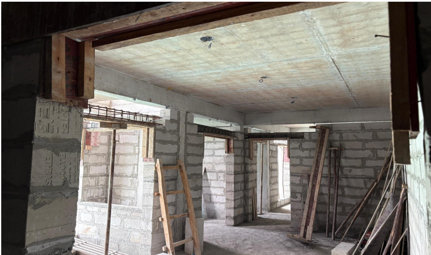
Block-3 Fourth Floor Block Work in Progress
