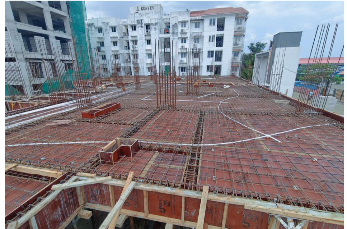
Block-1- Pour-1- First Floor Slab Reinforcement Completed
