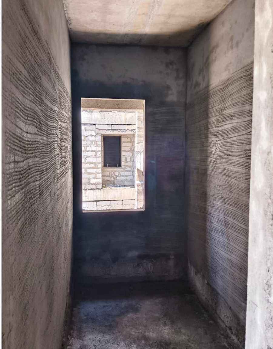
Block-02 – Pour-2 – Third Floor Toilet Plastering work in progress
