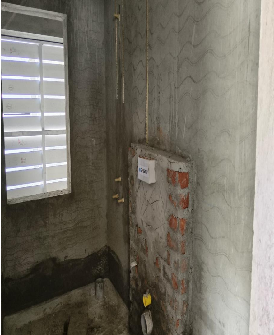
Block-02 – Pour-1 – First Floor Concealed Tank & Ledge Wall Brick Work in Progress.
