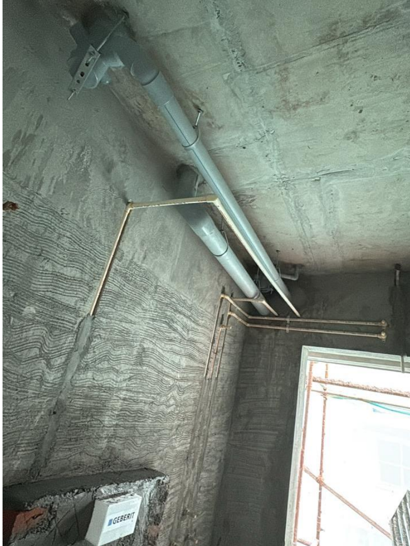
Block-03 – Toilet Plumbing Concealed & Suspended Pipeline Work Completed Up to 5 th Floor
