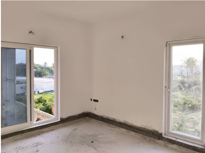
Block 2 - UPVC Works Second Floor
