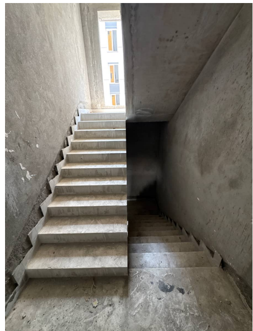
Block 2 - Staircase Flooring - Granite / Terracota
