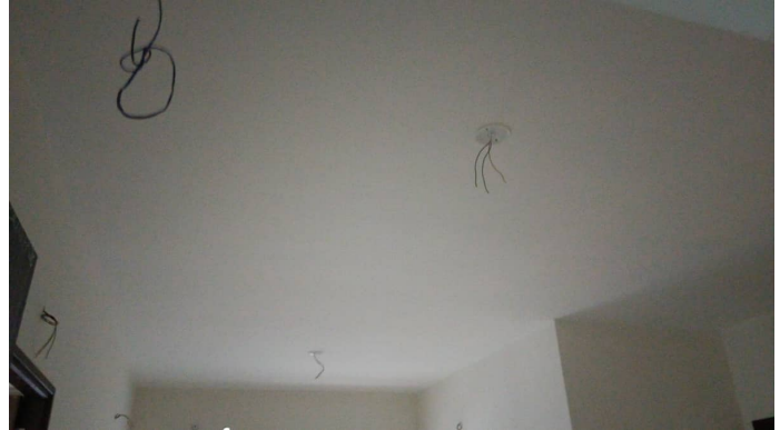
Block 4 - Final Coat Painting First Floor
