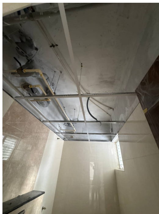
Block 3 - False Ceiling First Floor
