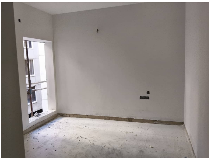
Block 2 - Putty works Second Floor
