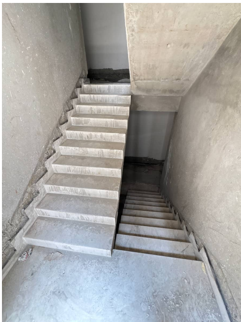
Block 2 - Staircase Flooring - Granite / Terracota
