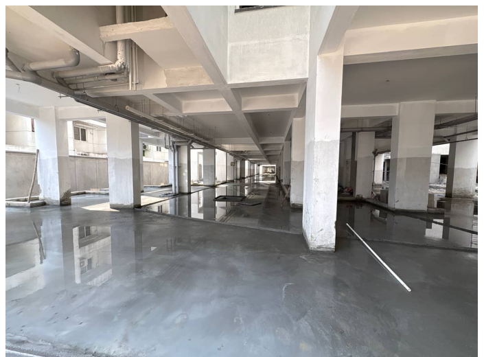
Block 3 - Masonry /RCC works in stilt floor Common Area
