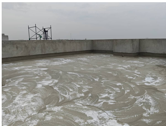
Block 1 - External Terrace Water proofing works
