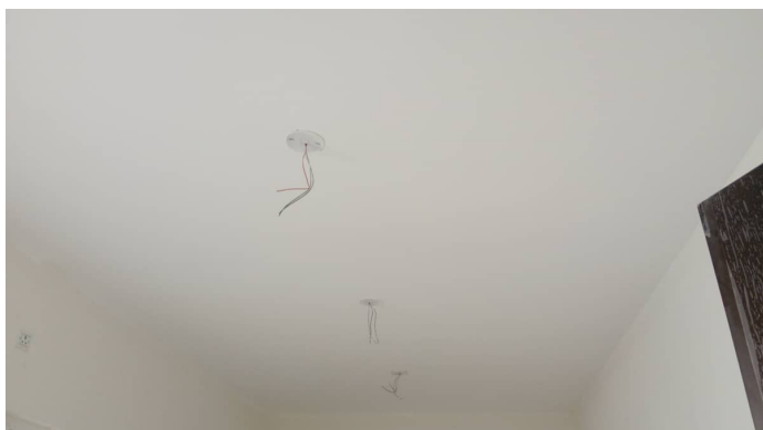
Block 4 - Final Coat Painting Third Floor
