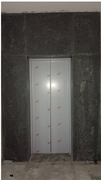
Block 4 - Elevator Erection
