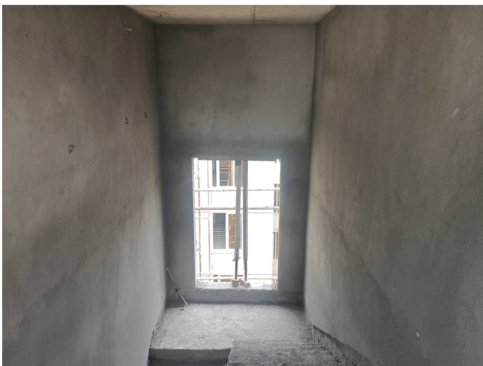
Block 1 - Internal Plastering Above Terrace
