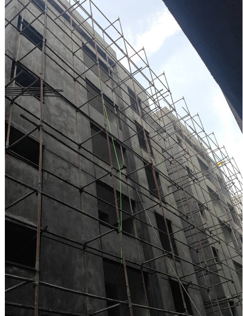
Block 1 - External Plastering
