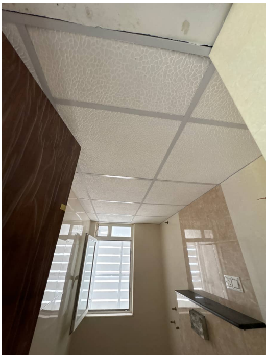
Block 3 - False Ceiling First Floor
