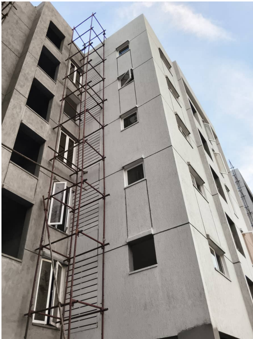
Block 2 - External Elevation Works
