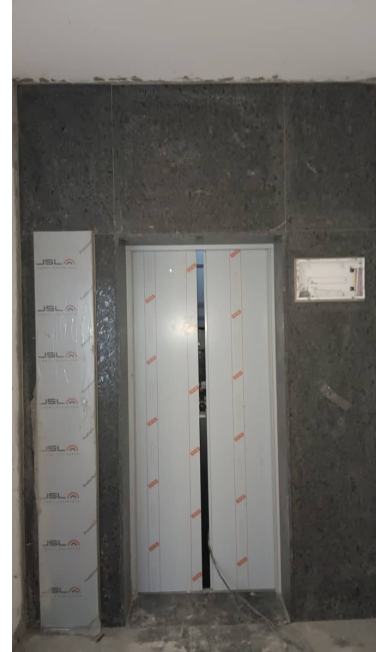
Block 4 - Elevator Erection
