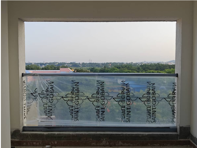
Block 1 - Balcony & Staircase Handrail Second Floor
