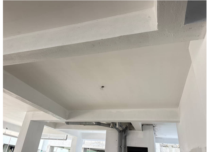
Block 3 - Primer & 1st Coat Paint Common Area
