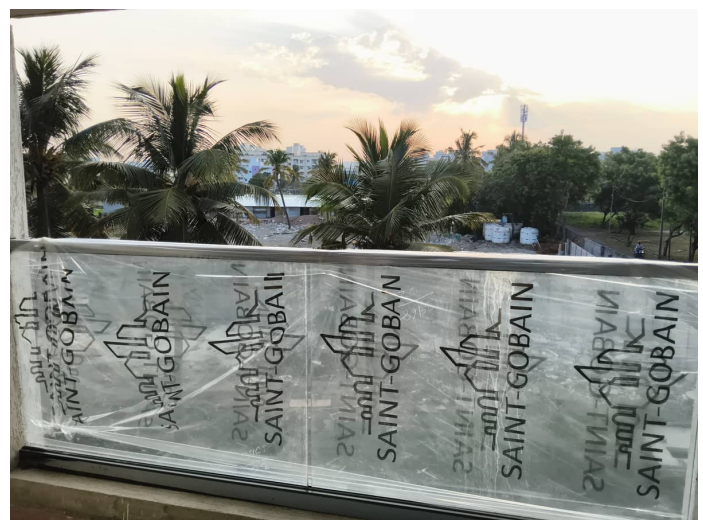
Block 2 - Balcony & Staircase Handrail Second Floor
