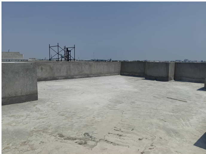
Block 1 - External Terrace Water proofing works
