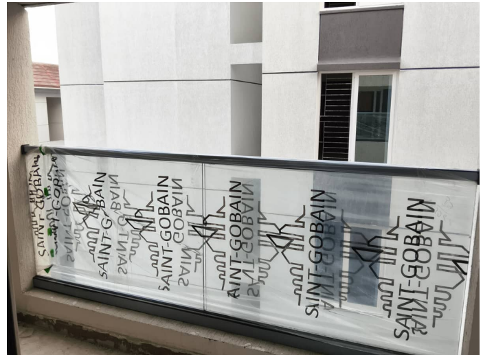
Block 2 - Balcony & Staircase Handrail Fourth Floor
