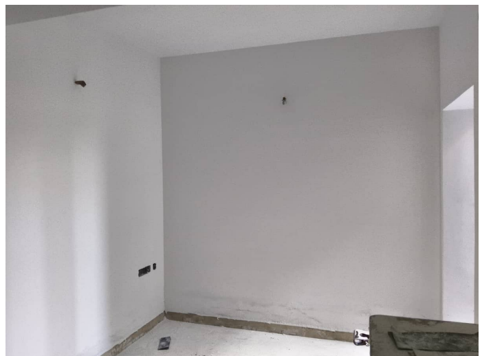
Block 2 - Putty works Second Floor
