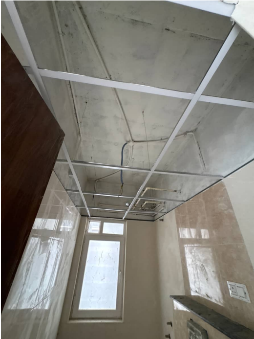
Block 3 - False Ceiling Fifth Floor
