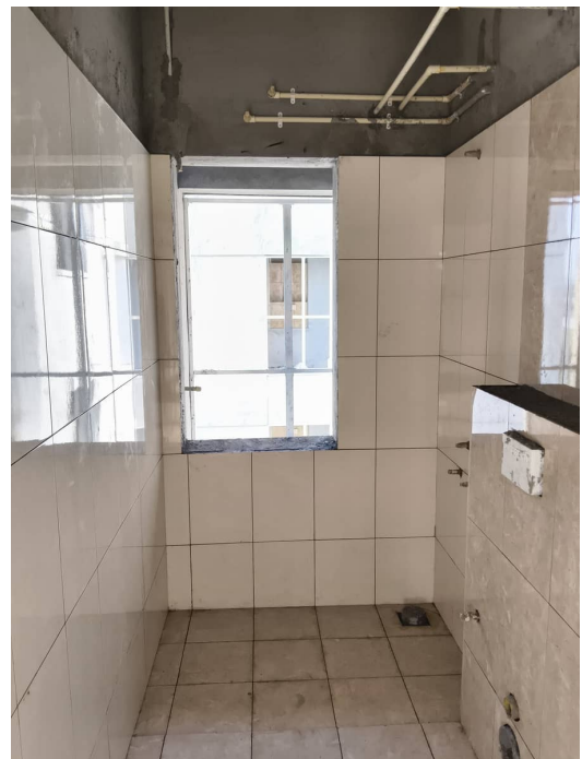
Block 2 - Wall Tile Fifth Floor
