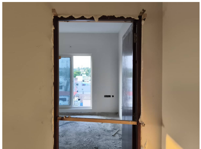
Block 2 - Joinery Fourth Floor
