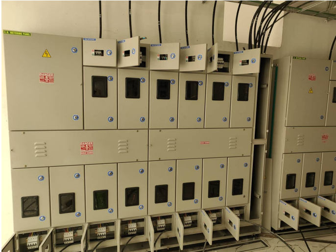
Block 3 - Electrical Panel board installation
