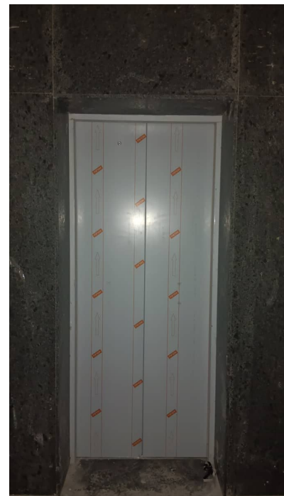
Block 4 - Elevator Erection
