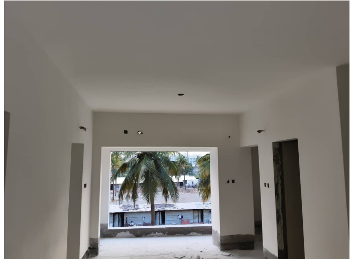
Block 2 - Putty works Second Floor
