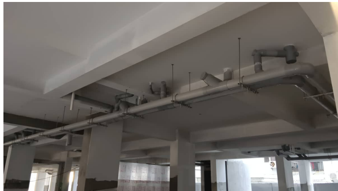
Block 4 - Internal Plumbing Works Stilt Floor
