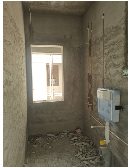
Block 1 - Internal Plumbing Works Fifth Floor
