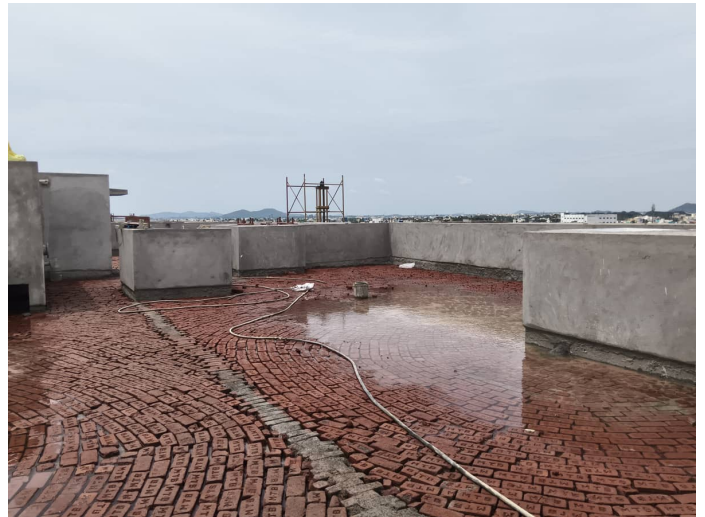
Block 2 - External Terrace Water proofing works
