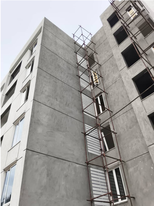
Block 2 - External Elevation Works
