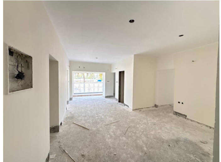
Block 2 - Primer & 1st Coat Paint First Floor
