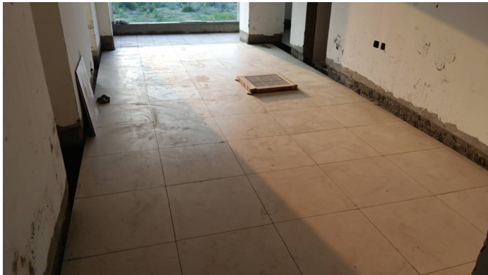
Block 1 - Floor Tiles Second Floor
