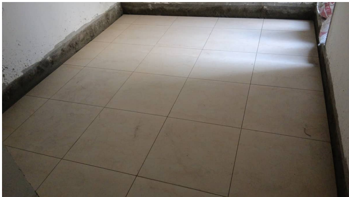
Block 1 - Floor Tiles Second Floor
