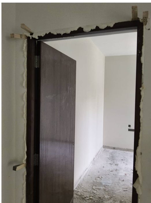
Block 2 - Joinery First Floor
