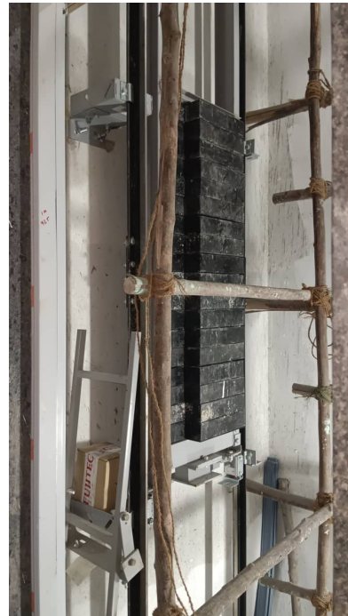
Block 4 - Elevator Erection
