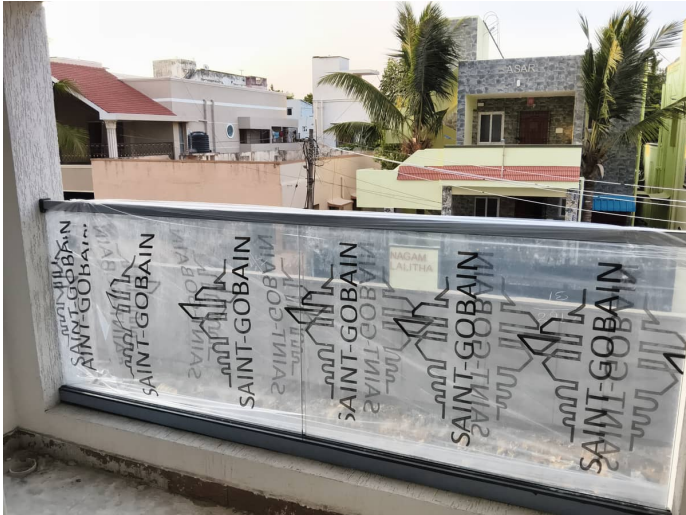
Block 2 - Balcony & Staircase Handrail First Floor
