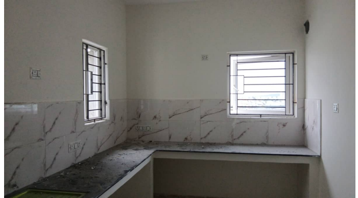
Block 4 - Switches & Socket Fifth Floor
