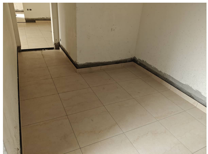
Block 1 - Floor Tiles First Floor
