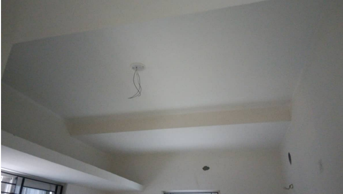
Block 4 - Final Coat Painting First Floor
