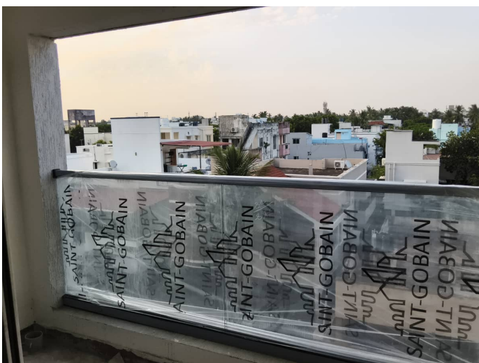
Block 2 - Balcony & Staircase Handrail Third Floor
