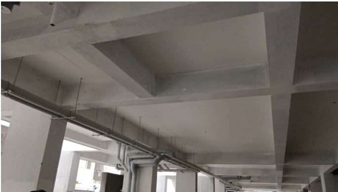
Block 4 - Primer & 1st Coat Paint Common Area
