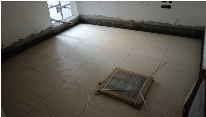
Block 1 - Floor Tiles Second Floor
