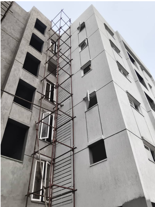
Block 2 - External Elevation Works
