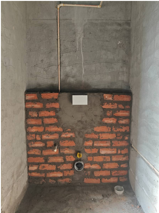
Block 1 - Internal Plumbing Works Fourth Floor
