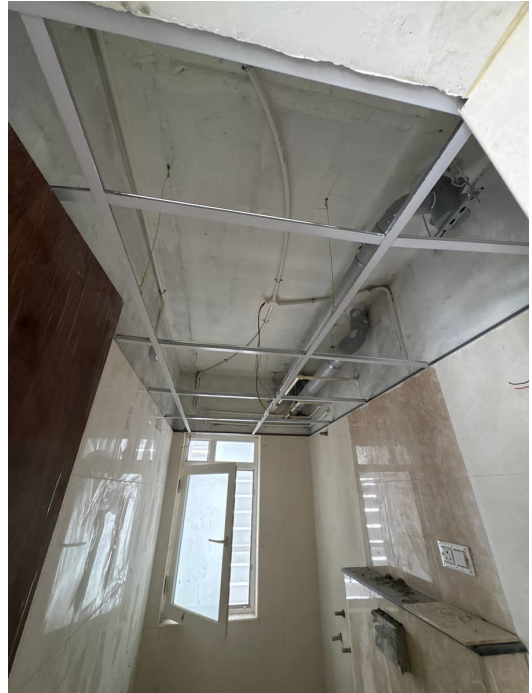
Block 3 - False Ceiling Fourth Floor
