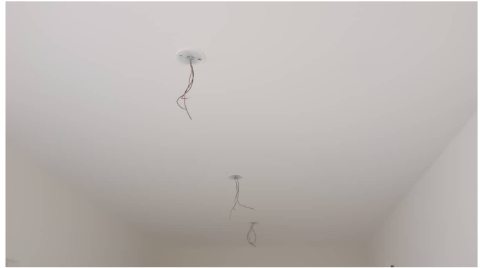
Block 4 - Final Coat Painting Fourth Floor
