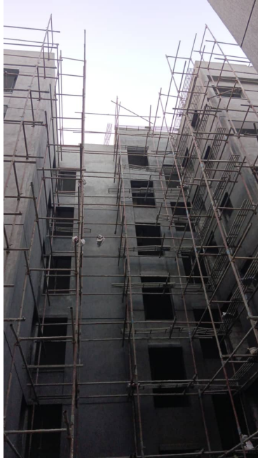
Block 1 - External Plastering
