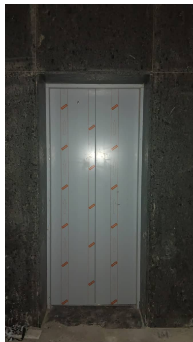
Block 4 - Elevator Erection
