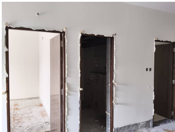
Block 2 - Joinery First Floor
