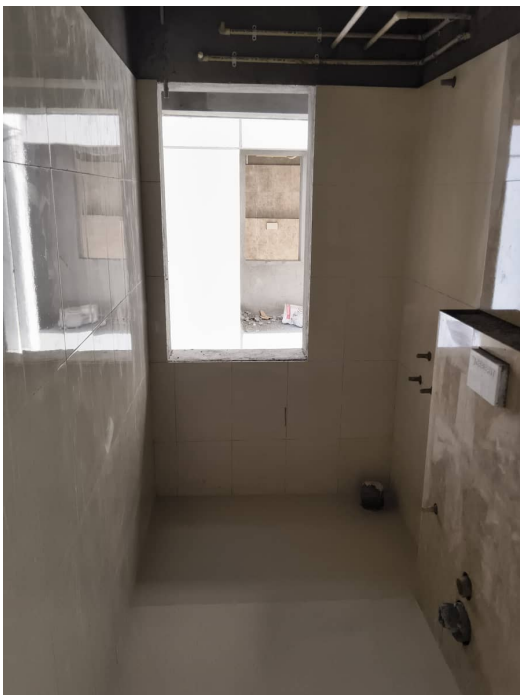
Block 2 - Wall Tile Fourth Floor
