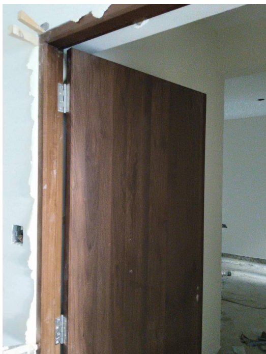
Block 2 - Joinery Second Floor
