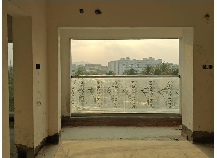
Block 1 - Balcony & Staircase Handrail Third Floor
