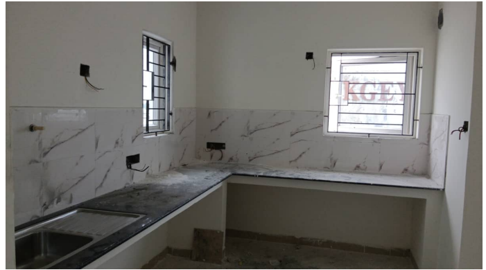
Block 4 - Wiring Fifth Floor
