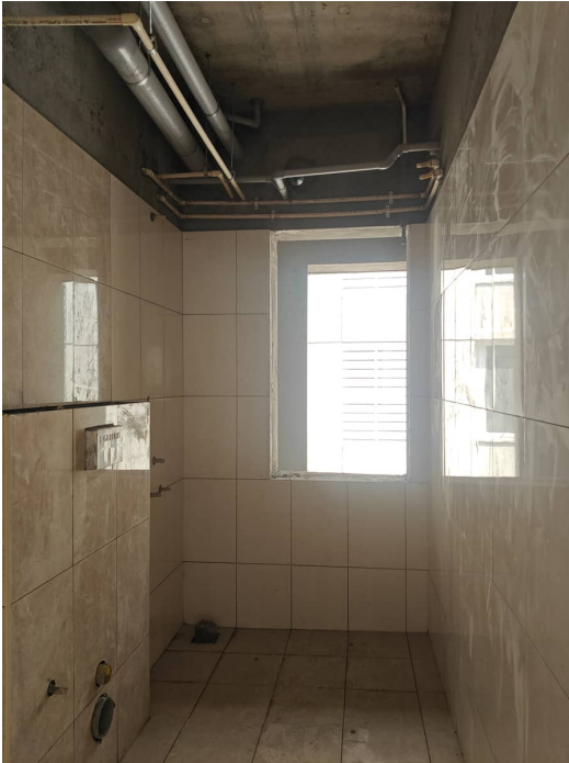
Block 1 - Wall Tiles Fourth Floor
