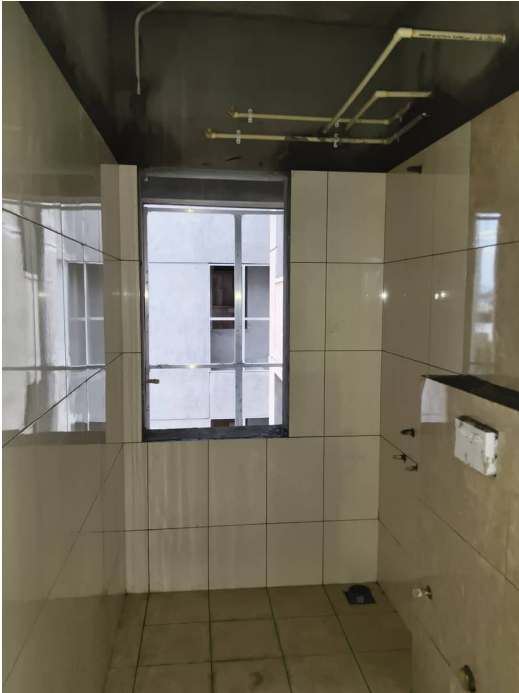
Block 2 - Wall Tile Fifth Floor
