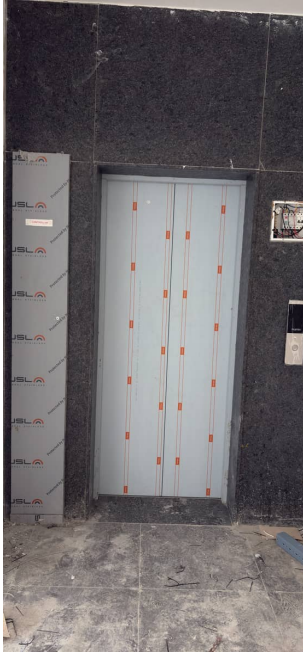
Block 3 - Elevator Testing
