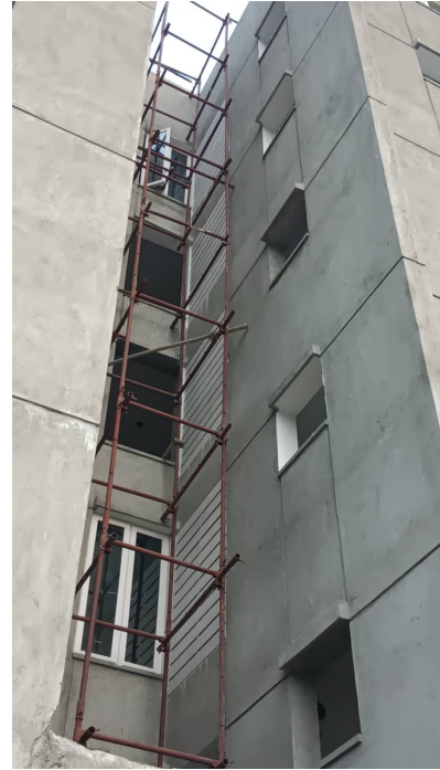
Block 1 - External Elevation Works
