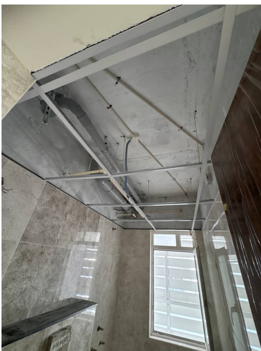
Block 3 - False Ceiling First Floor
