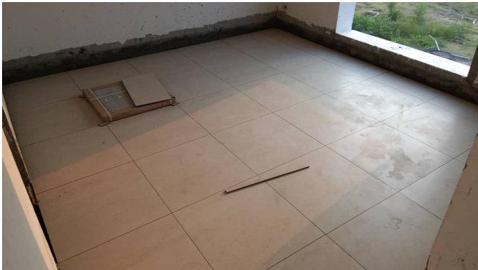
Block 1 - Floor Tiles Second Floor
