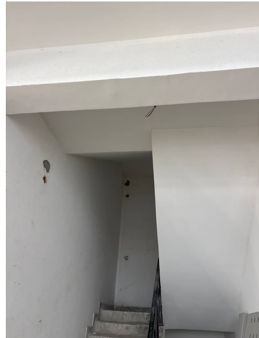
Block 3 - 1st Putty Coat Common Area
