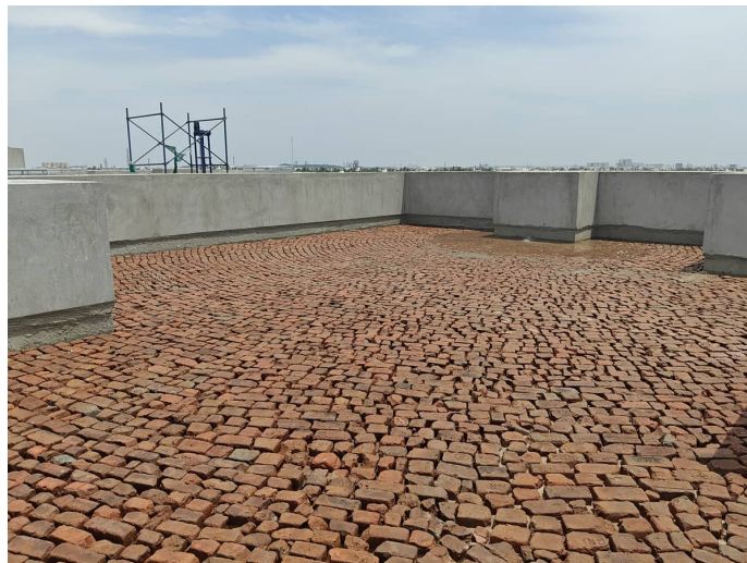
Block 1 - External Terrace Water proofing works
