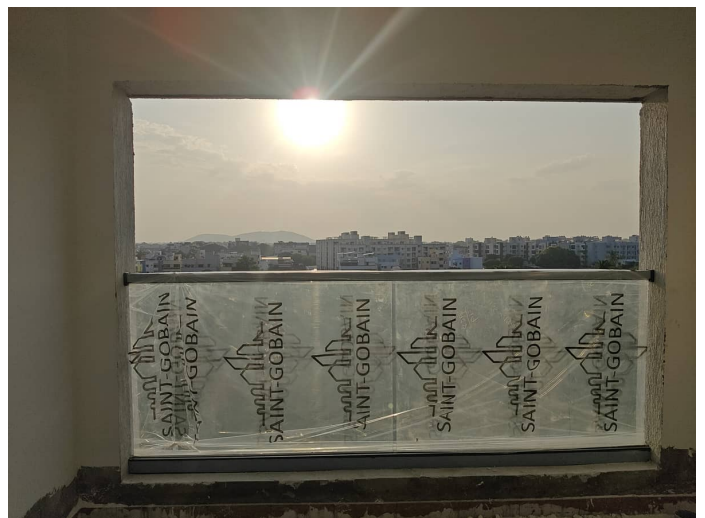
Block 1 - Balcony & Staircase Handrail Fifth Floor
