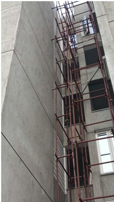
Block 1 - External Elevation Works
