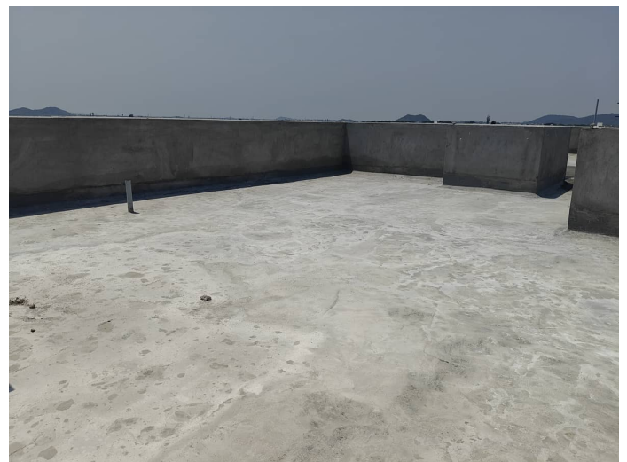
Block 1 - External Terrace Water proofing works
