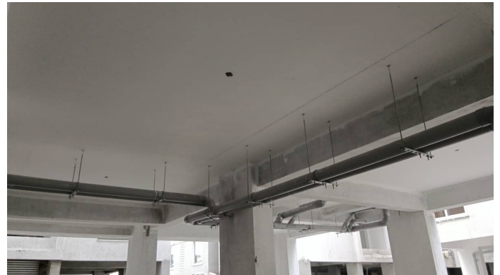
Block 4 - Primer & 1st Coat Paint Common Area
