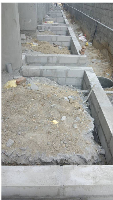
Block 4 - Masonry /RCC works in stilt floor Common Area
