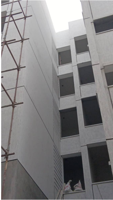
Block 1 - External Elevation Works
