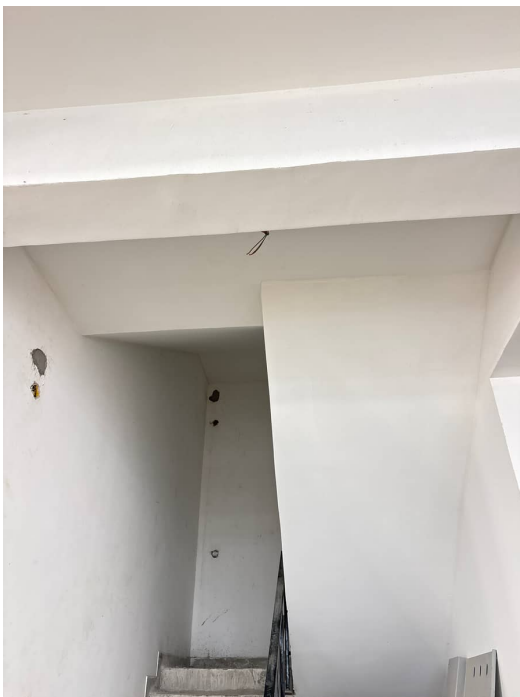
Block 3 - Putty 2nd Coat Common Area
