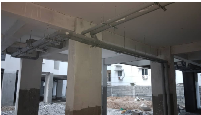
Block 4 - Internal Plumbing Works Stilt Floor
