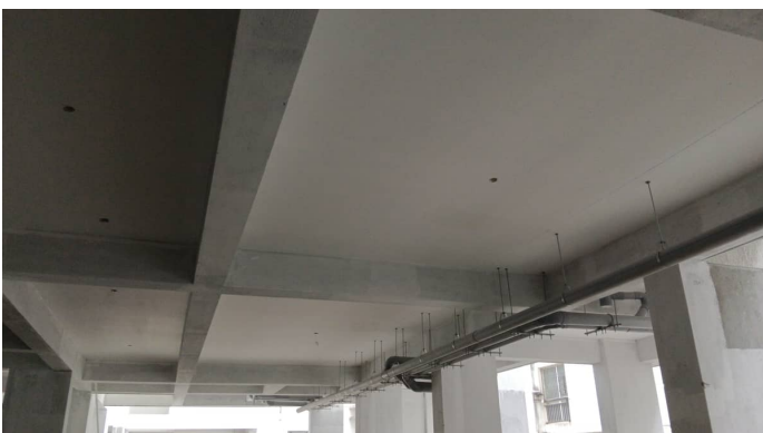
Block 4 - Primer & 1st Coat Paint Common Area
