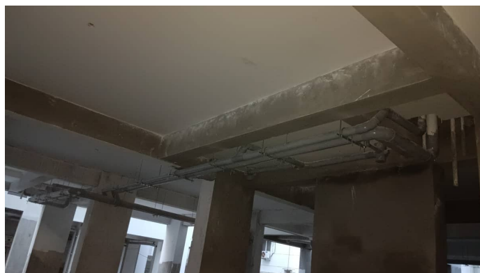
Block 4 - Internal Plumbing Works Stilt Floor
