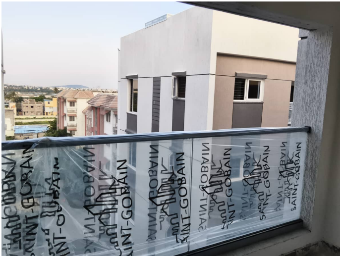
Block 2 - Balcony & Staircase Handrail Fifth Floor
