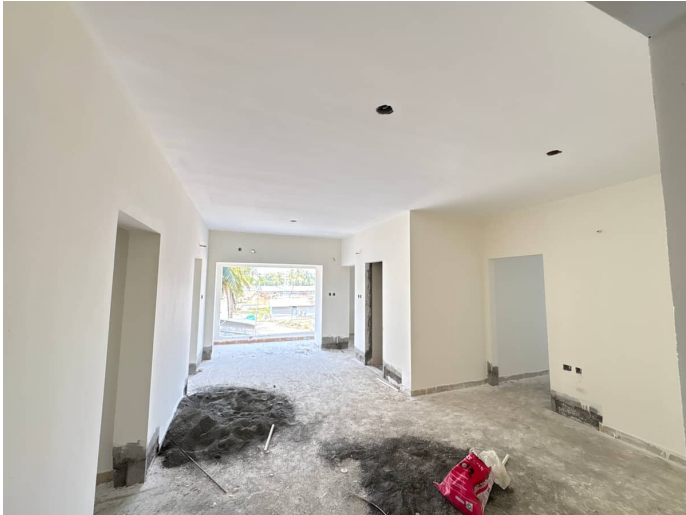
Block 2 - Primer & 1st Coat Paint First Floor
