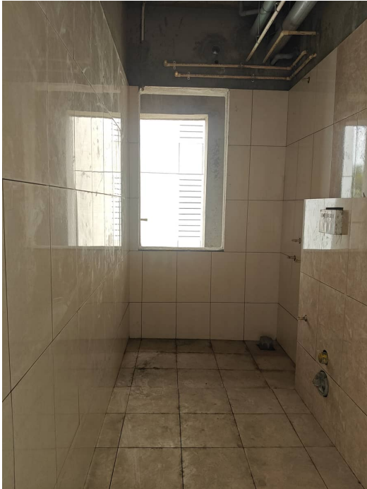
Block 1 - Wall Tiles First Floor
