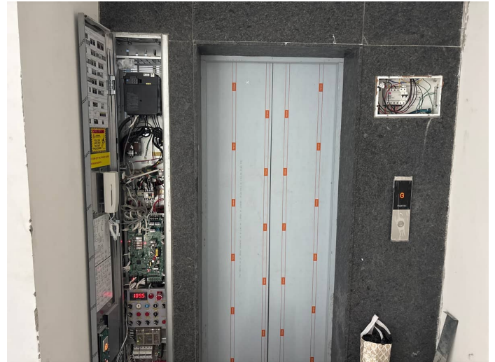
Block 3 - Elevator Testing
