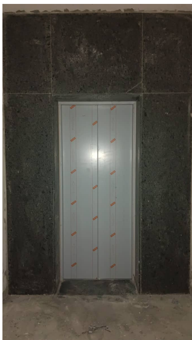
Block 4 - Elevator Erection
