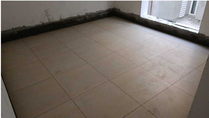
Block 1 - Floor Tiles Second Floor
