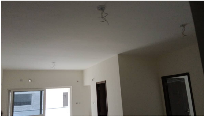
Block 4 - Wiring Fourth Floor
