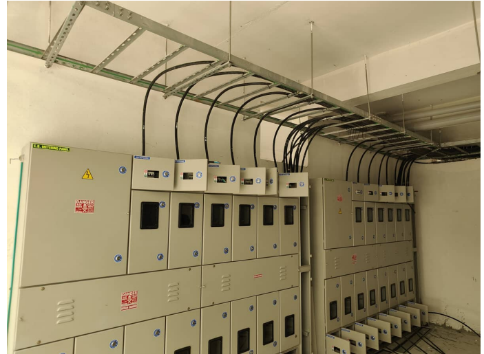
Block 3 - Electrical Panel board installation
