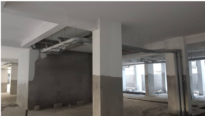
Block 4 - Internal Plumbing Works Stilt Floor
