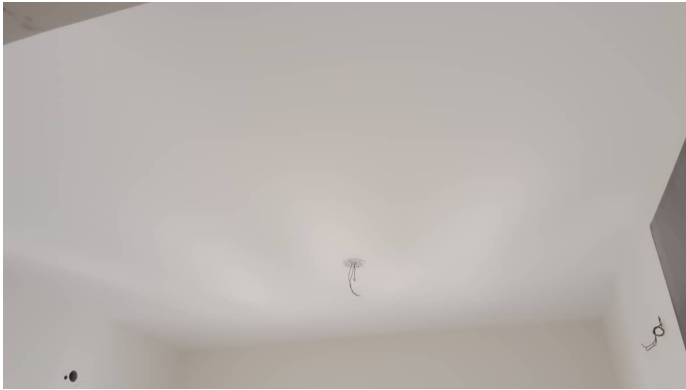
Block 4 - Final Coat Painting Fourth Floor
