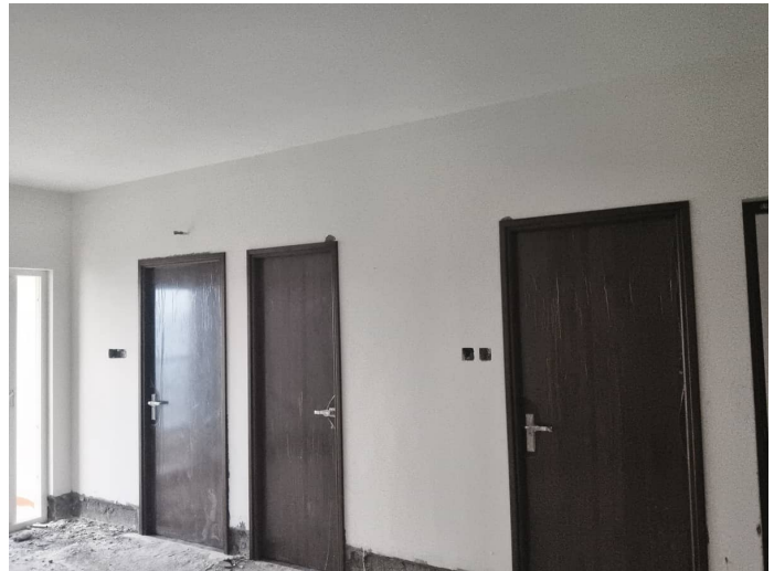
Block 2 - Joinery Third Floor
