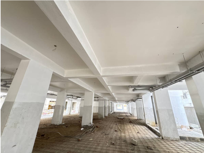
Block 3 - Primer & 1st Coat Paint Common Area
