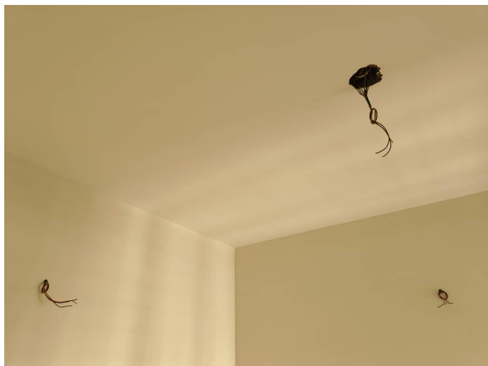
Block 4 - Wiring Second Floor
