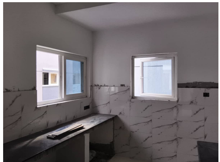
Block 2 - UPVC Works Second Floor
