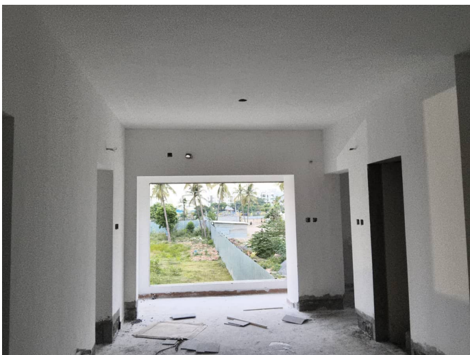
Block 2 - Primer & 1st Coat Paint First Floor
