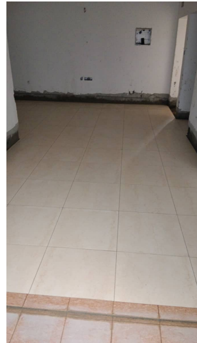
Block 1 - Floor Tiles Second Floor
