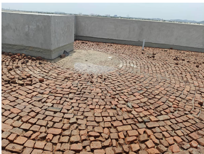
Block 1 - External Terrace Water proofing works
