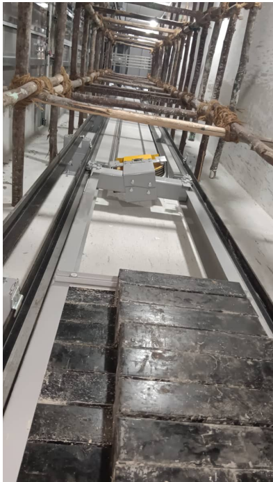
Block 4 - Elevator Erection
