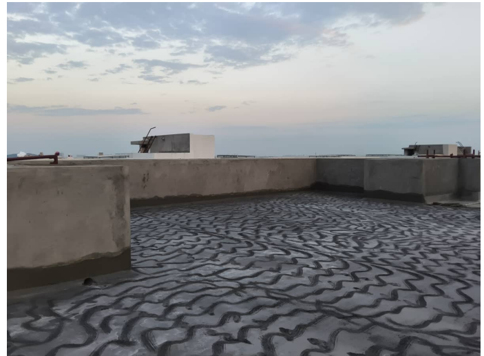
Block 2 - External Terrace Water proofing works
