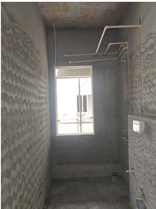
Block 1 - Internal Plumbing Works Fifth Floor
