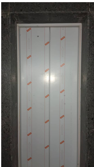
Block 4 - Elevator Erection
