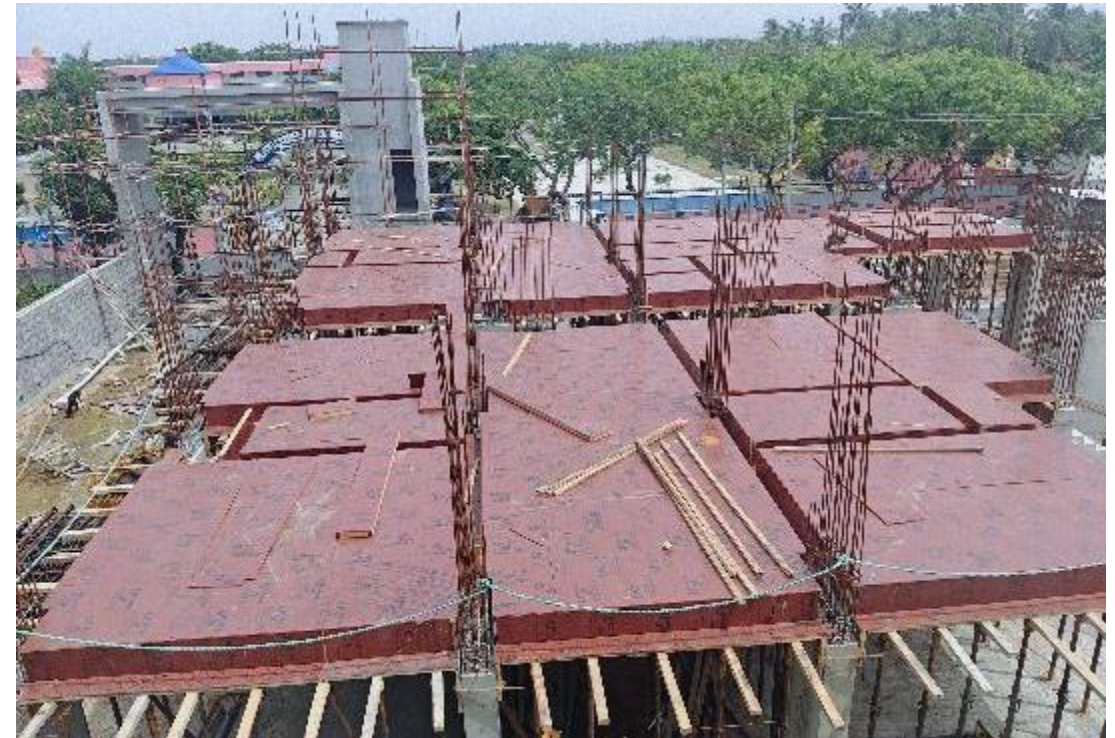
Block-1- Pour-1-Stilt Floor Shuttering work in Progress
