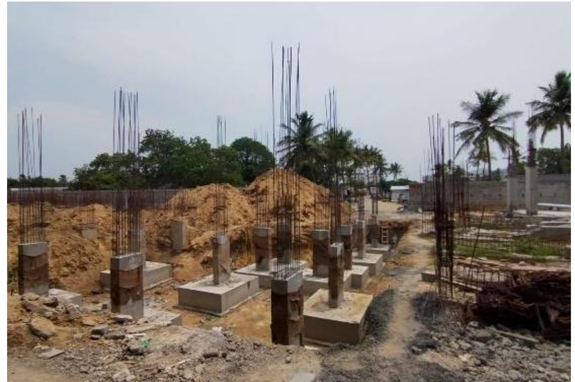
Block-2-Pour 3- Sub Structure Column Concrete Work Completed
