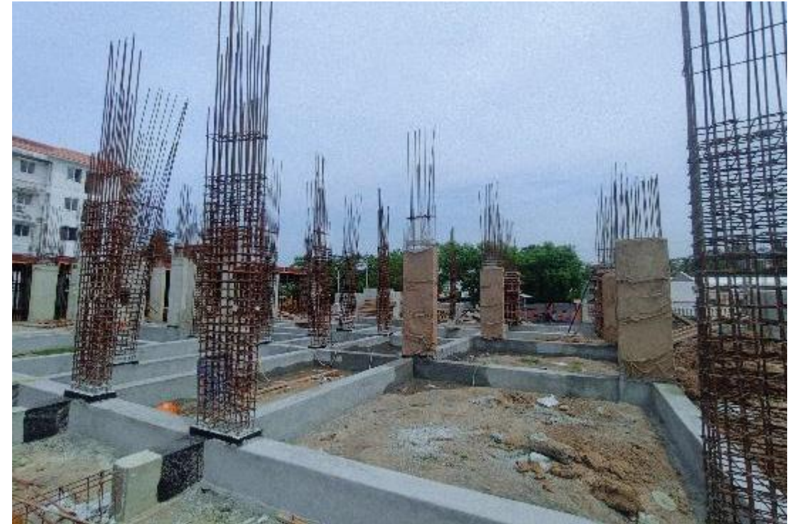
Block-1- Pour-1-Plinth Beam DPC work Completed
