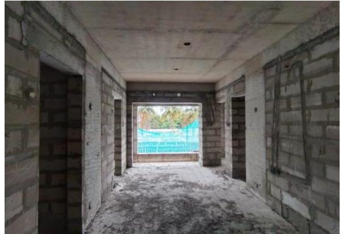
Block-3- First Floor Wall Chasing work in Progress
