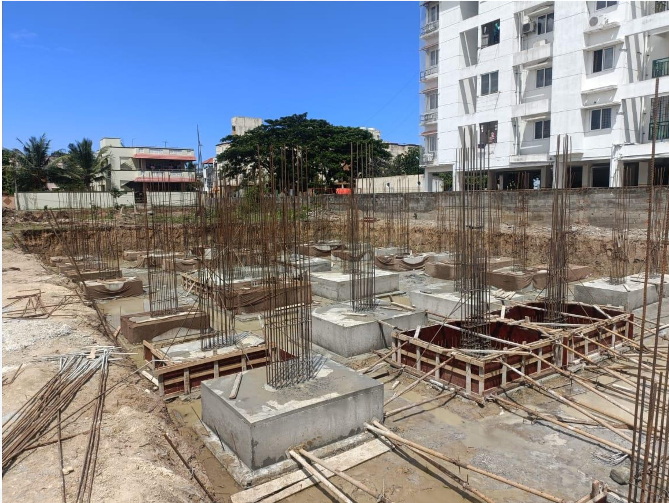
BLOCK-3 FOOTING CONCRETE WORK IN PROGRESS
