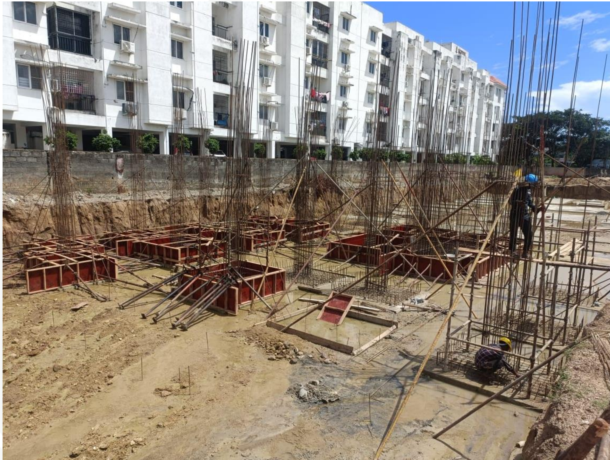
BLOCK-4 FOOTING CONCRETE WORK IN PROGRESS
