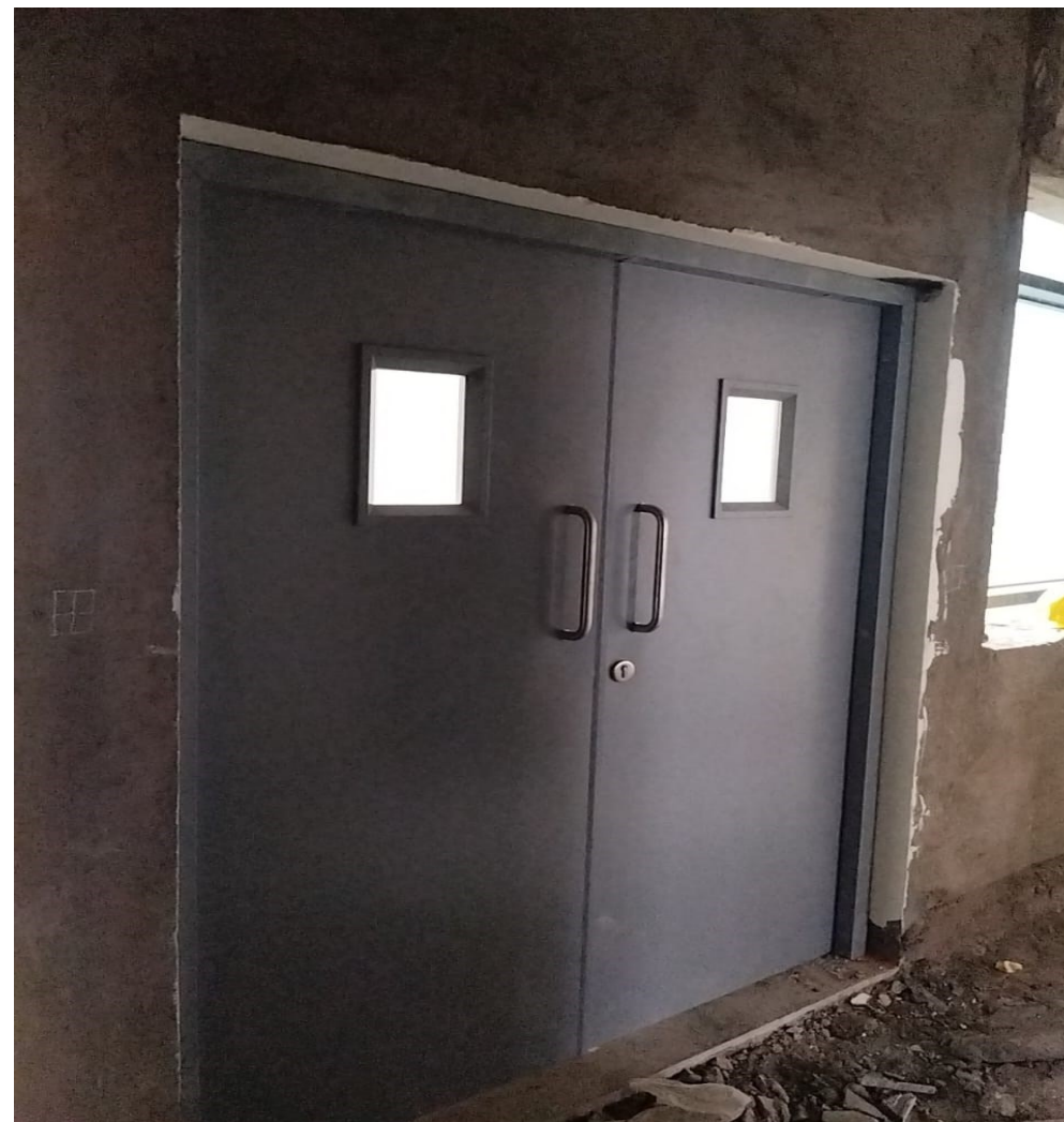
Staircase No.1 8 th to Head Room Fire Door Installation Work Completed
