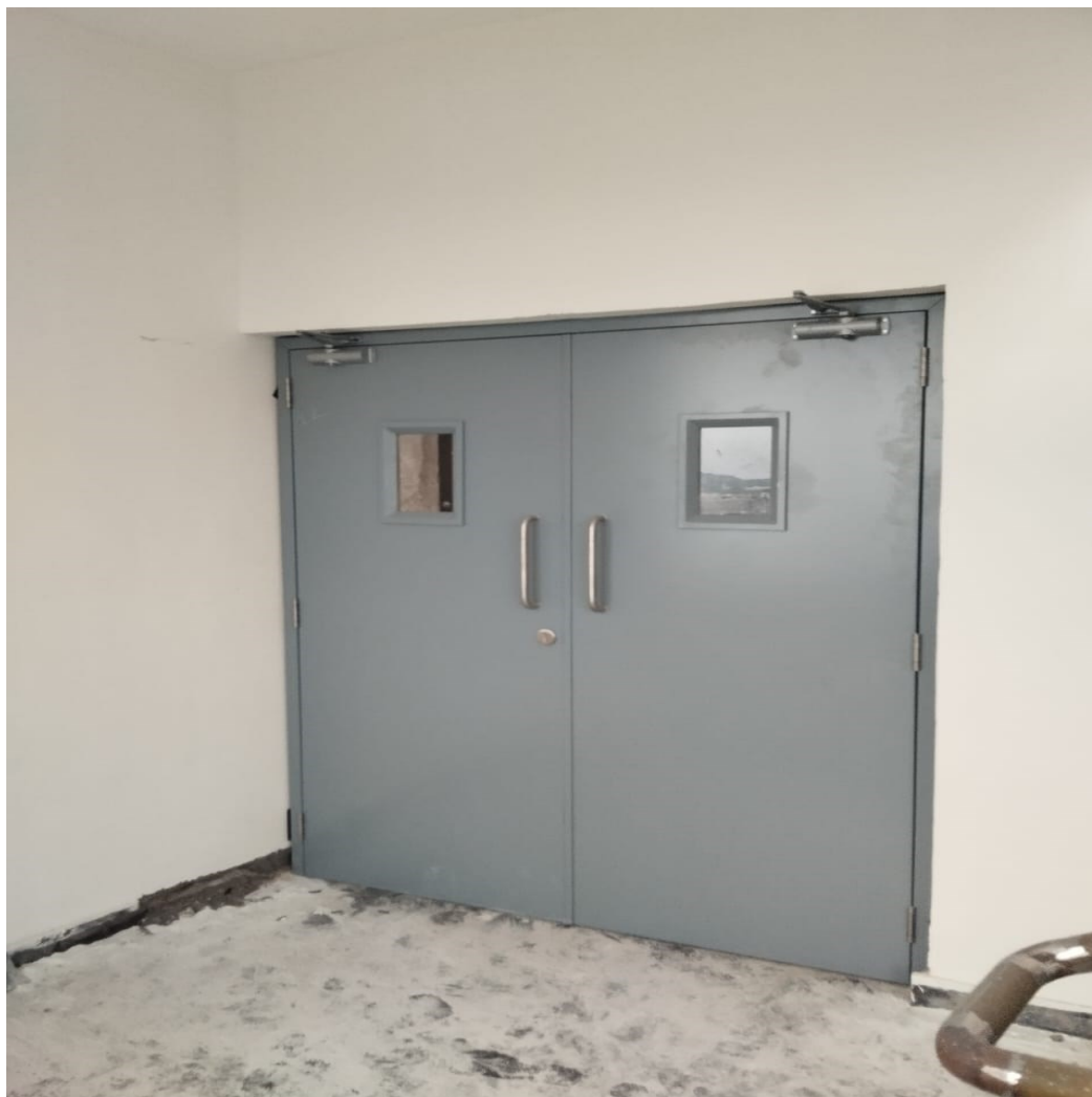
Staircase No.1 8 th to Head Room Fire Door Installation Work Completed
