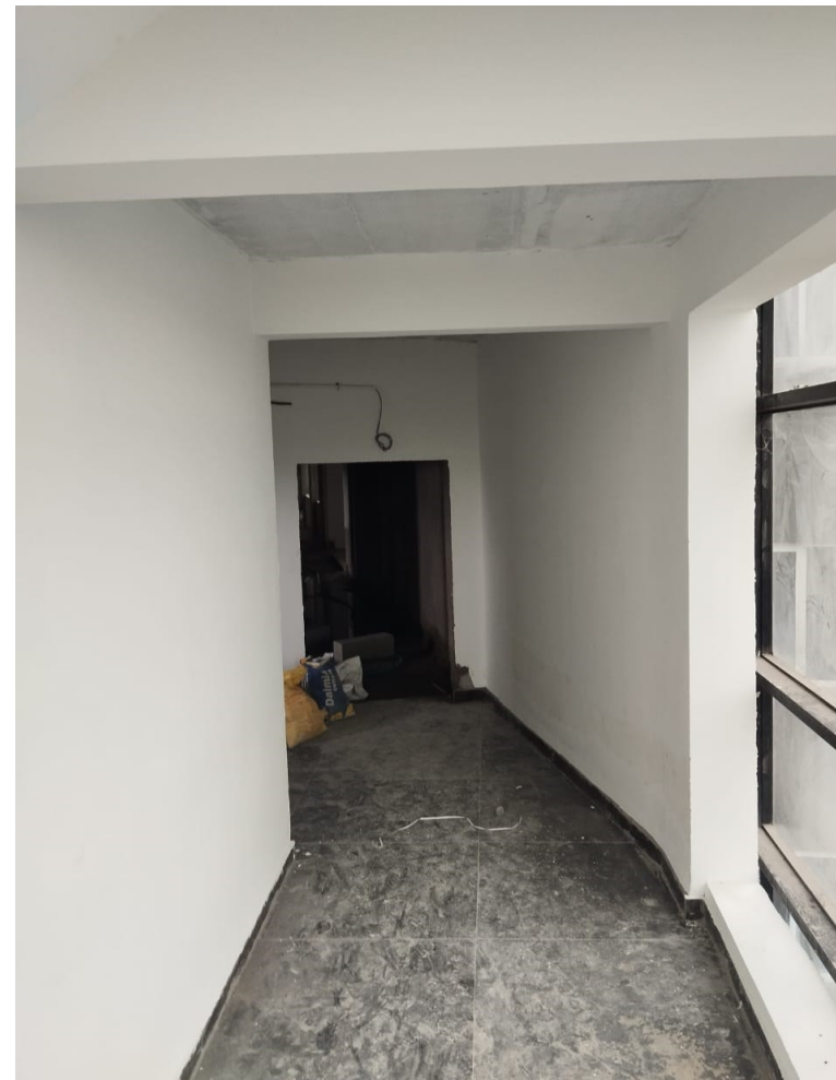
Staircase no.3 Wall 1 st Floor to 12 th Floor Primer Completed 1 st Coat Painting work in Progress
