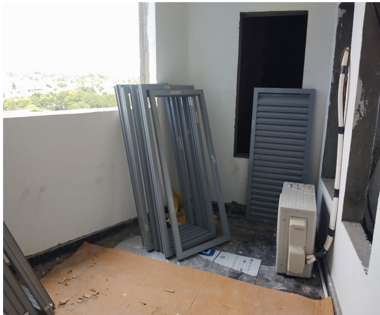
8 th to 12 th Floor Plumbing Shaft Aluminium Louvers Fixing work in Progress
