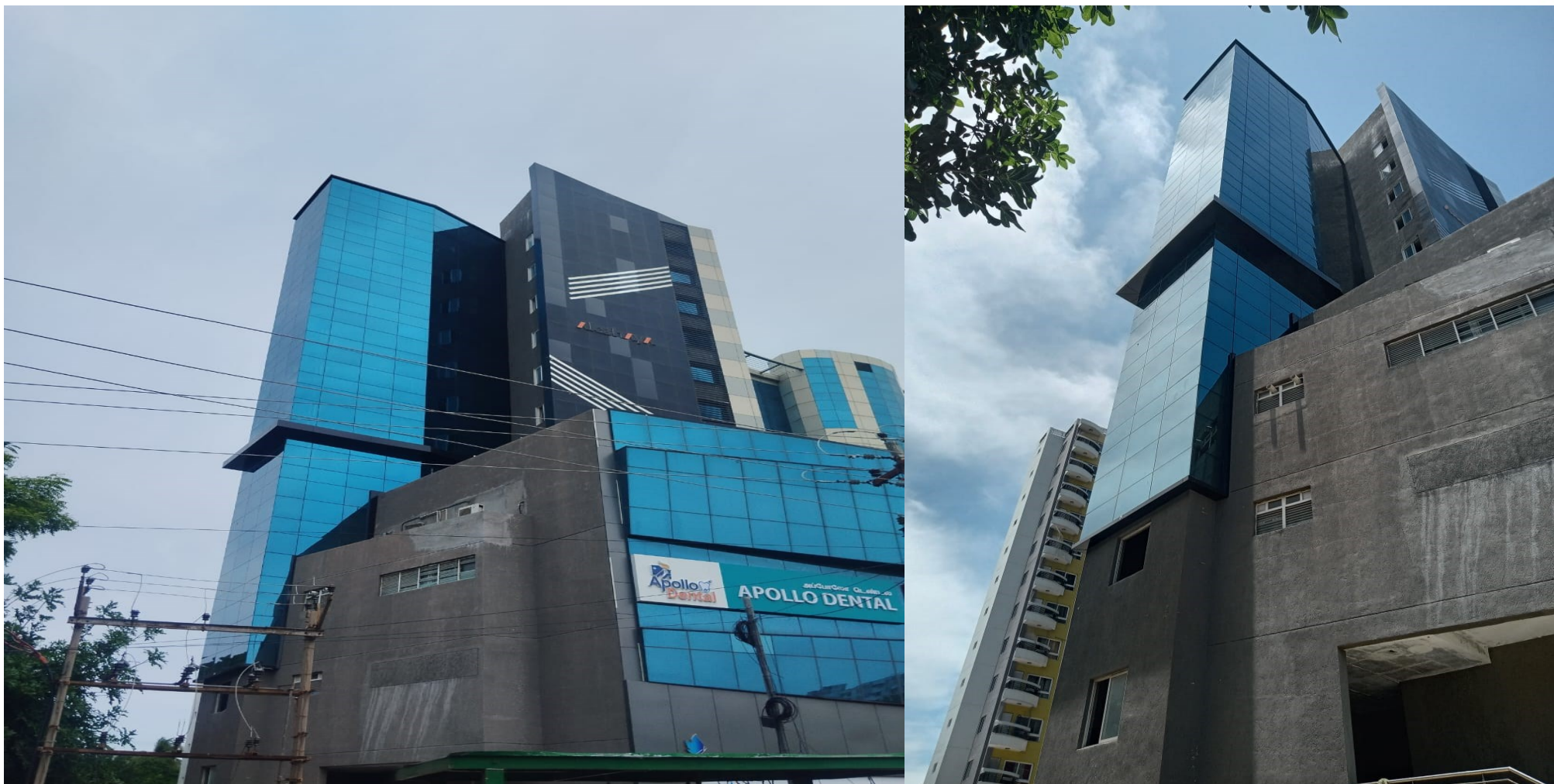
Truliv Cove Project Weekly Progress Photos – AUGUST 2025 – 4th Week
