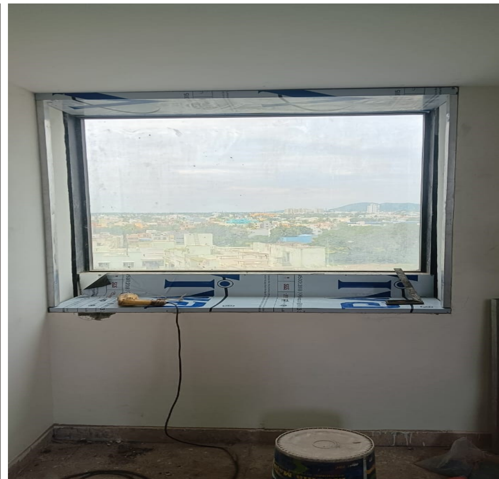
Staircase no.2 Lobby 8 th to 12 th Floor Façade Glass Window ACP Covering work Completed
