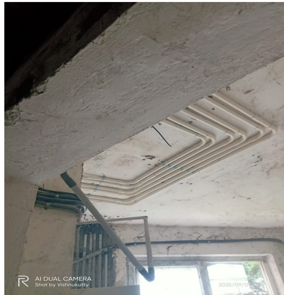
Stilt Floor Ceiling – Electrical Line Wire Pulling work Completed
