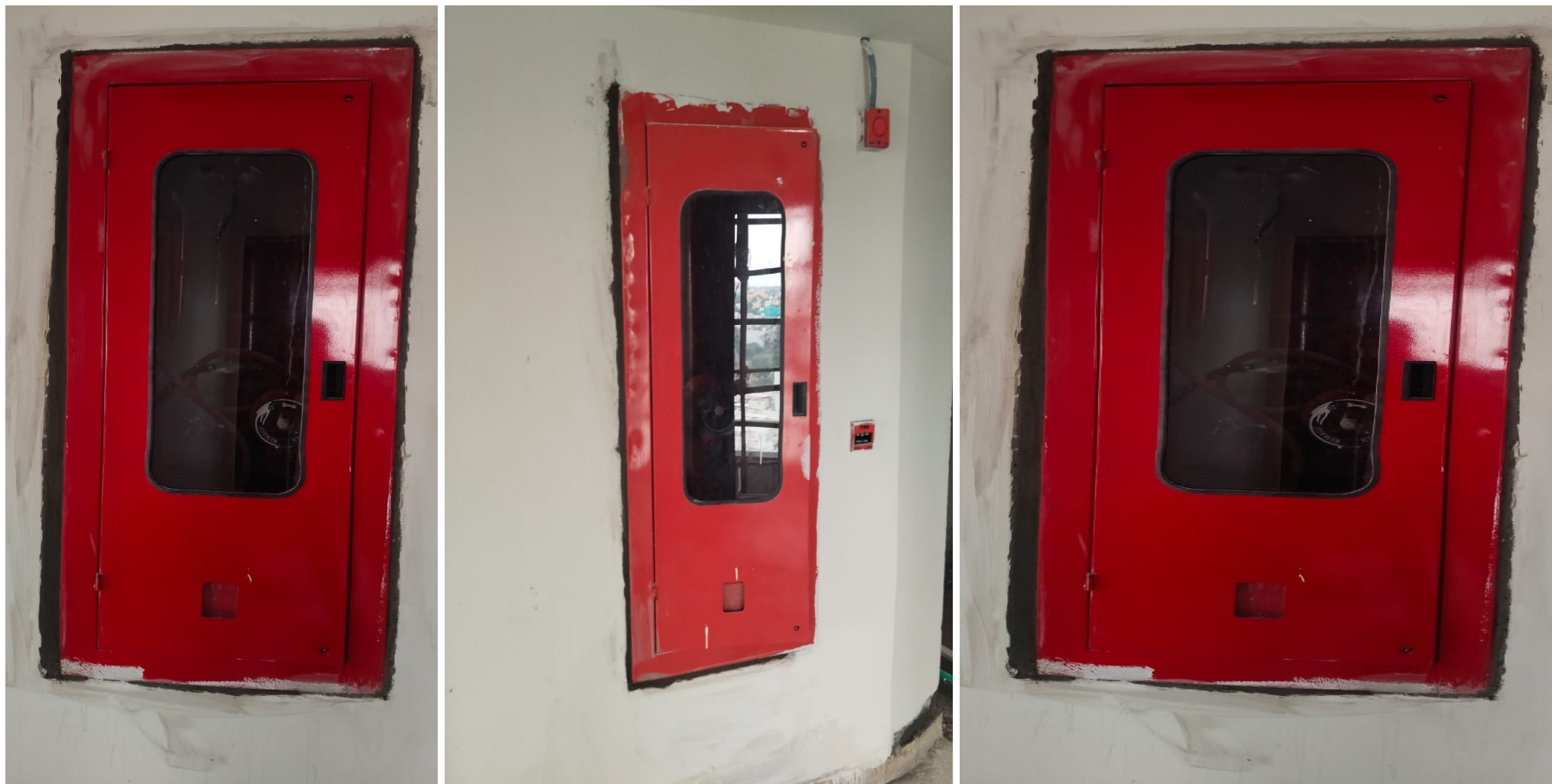
Staircase No.2 – Fire Shaft Door Fixing work Completed
