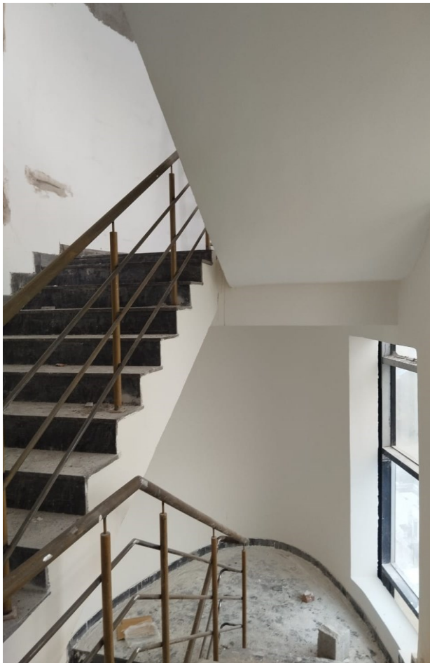
Staircase no.1 Steps Wall 1 st /Floor to 12 th Floor 1 st Coat Painting work Completed
