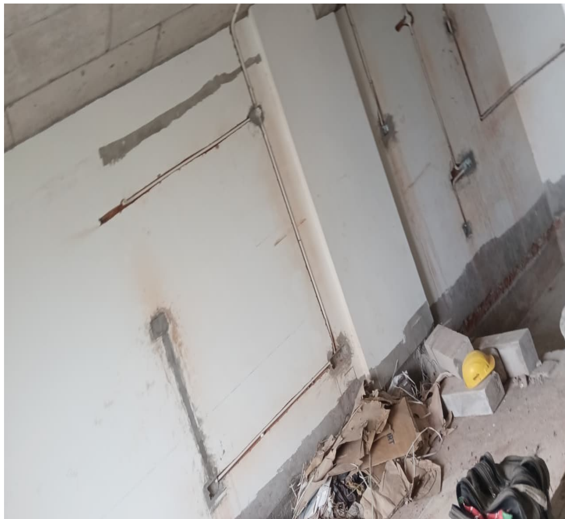
8 th Floor Room No.2 – Model Flat Electrical Wall Chasing work Completed
