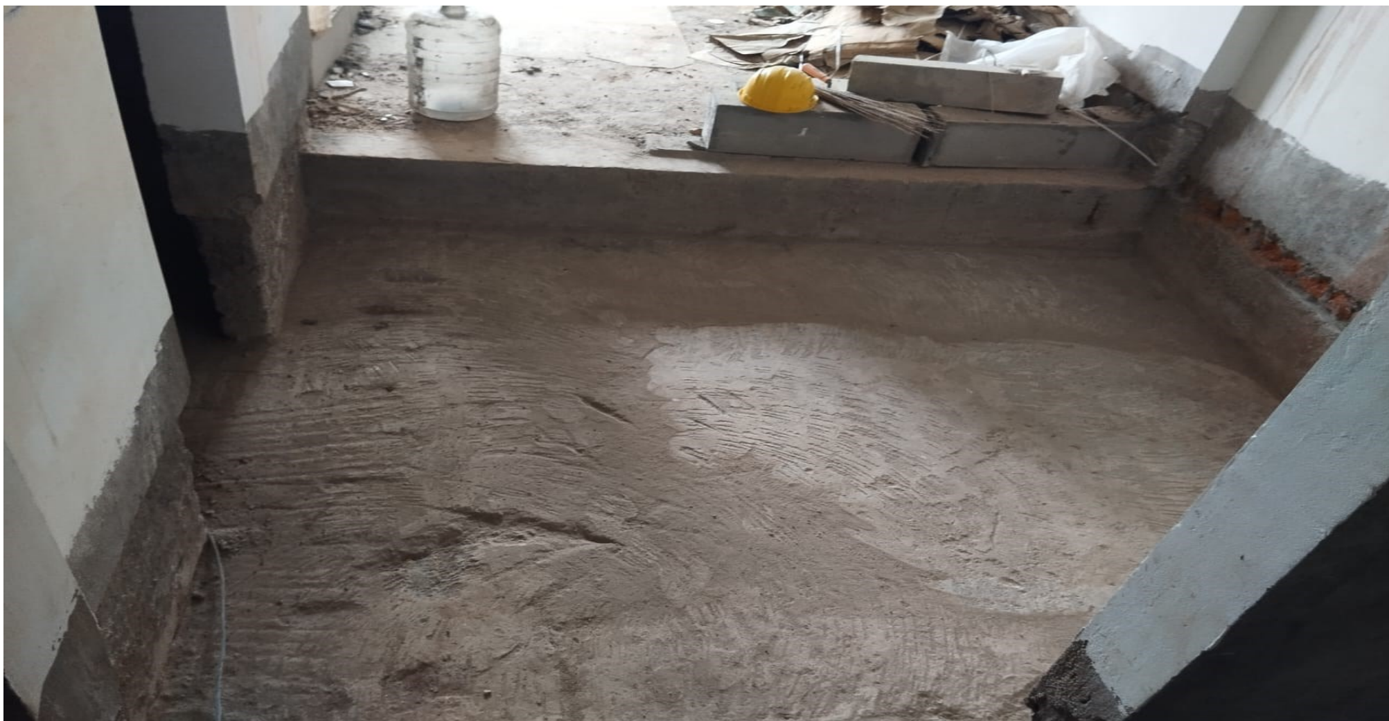
8 th Floor Room No.2 – Model Flat Toilet Sunkan Waterproofing work in Progress
