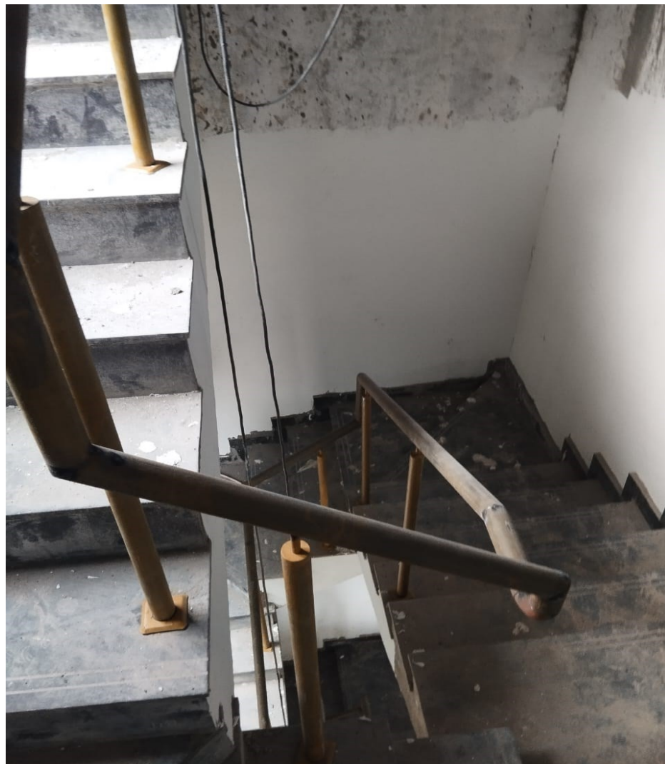
Staircase No.3 MS Handrail Fixing work in Progress
