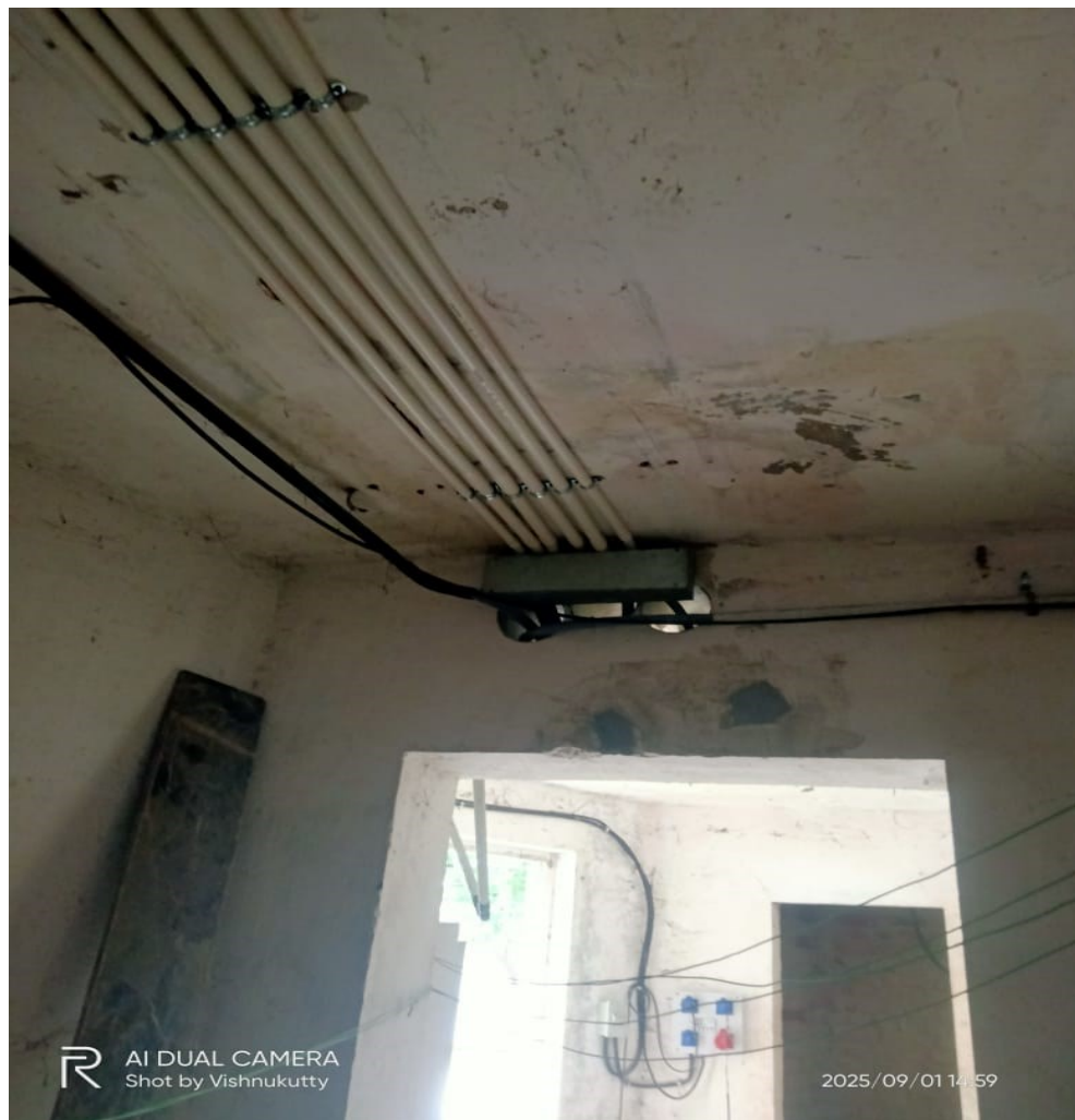
Stilt Floor Ceiling – Electrical Line Wire Pulling work Completed
