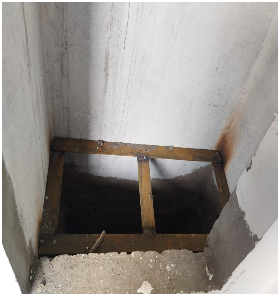
Communication Shaft Chequered Plate Fixing work in Progress
