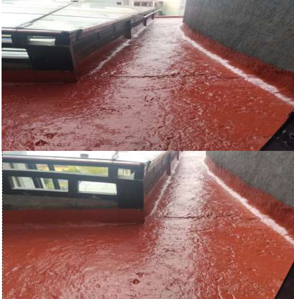
4th floor private terrace Waterproofing Coating work in progress
