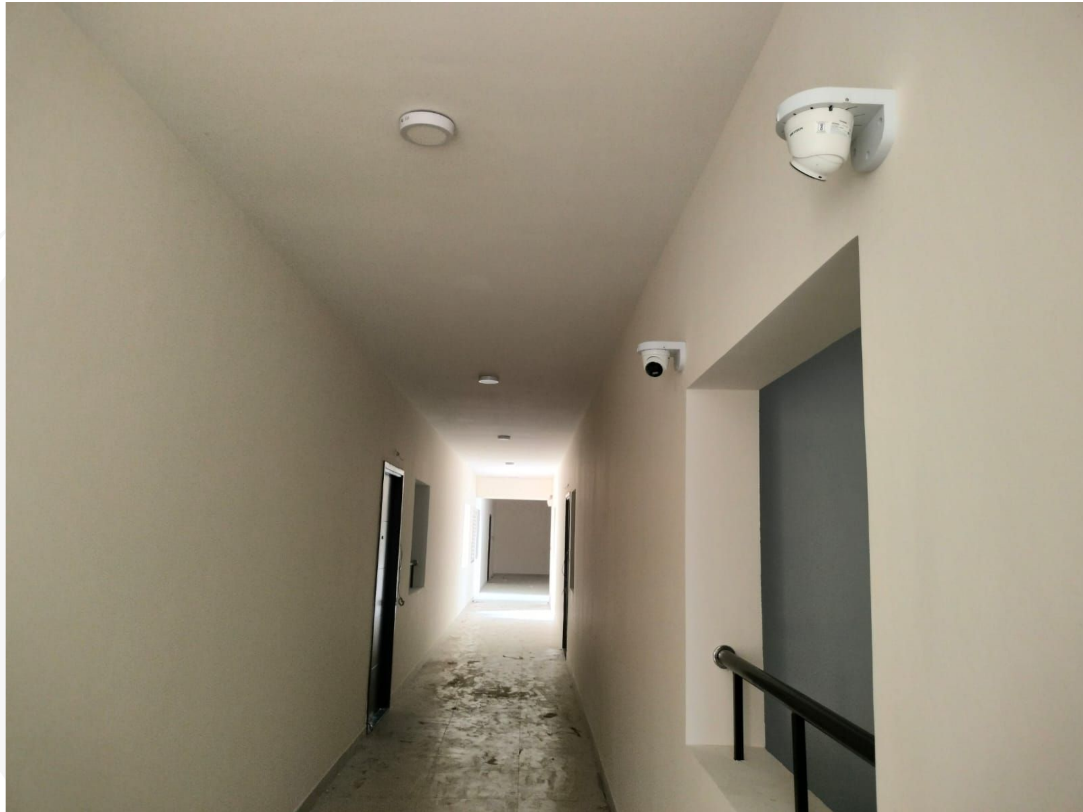
Common Area CCTV Camera Fixing Work In Progress
