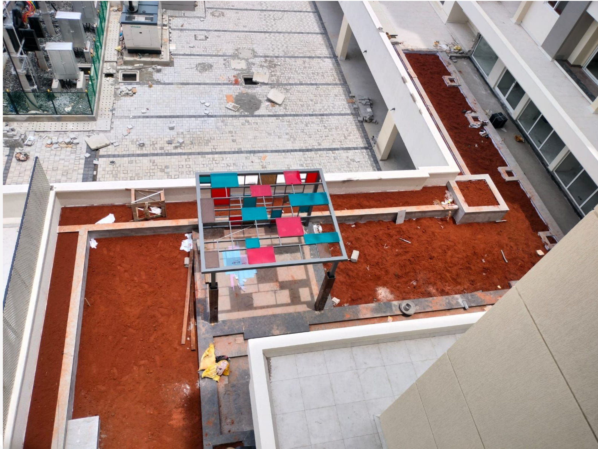
1 st Floor Amenities Hardscape Work in progress
