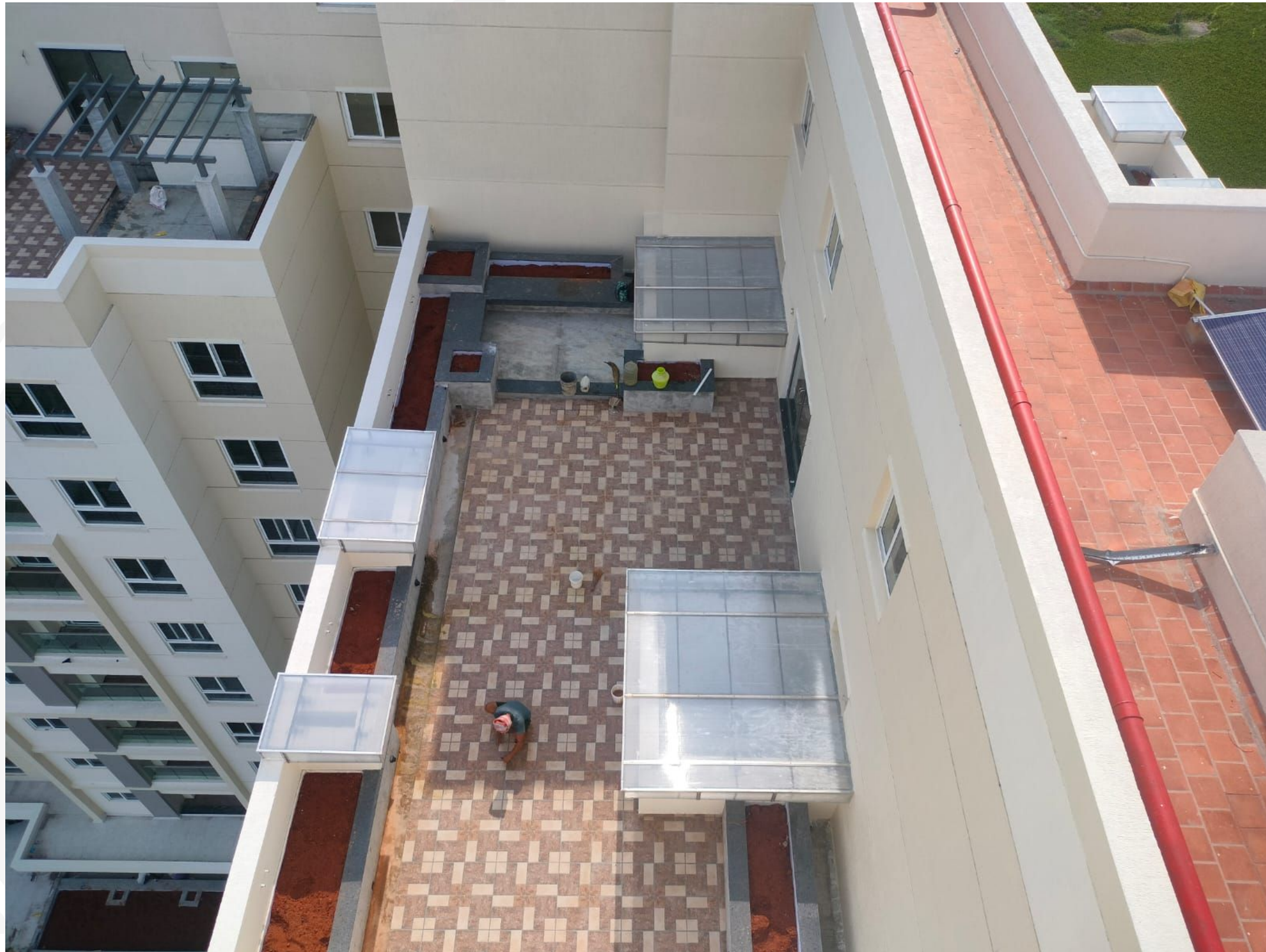
10 th Floor Low Terrace OTS Covering Work completed
