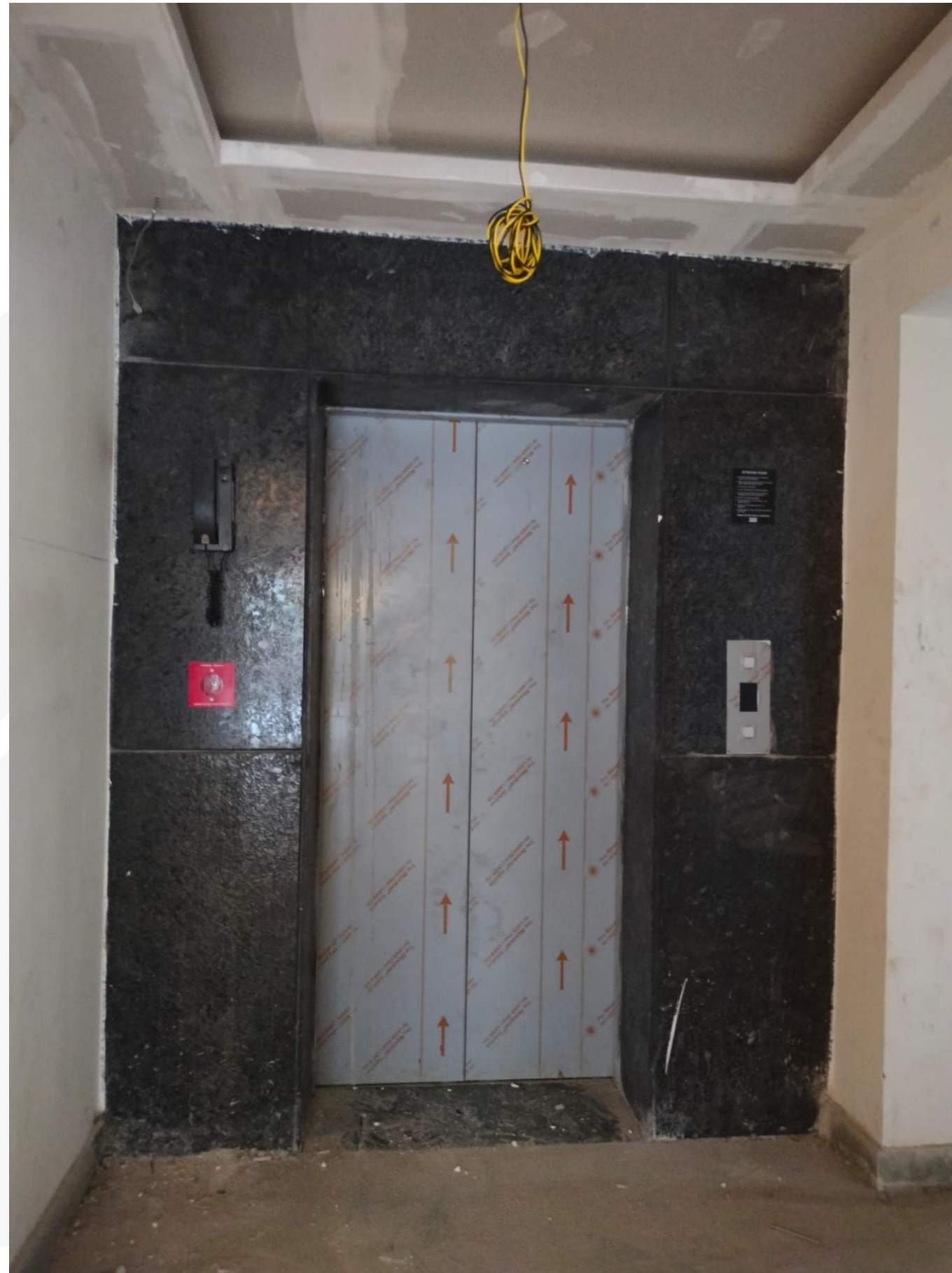
Lift -2 & 3 Erection Work In Progress ,
