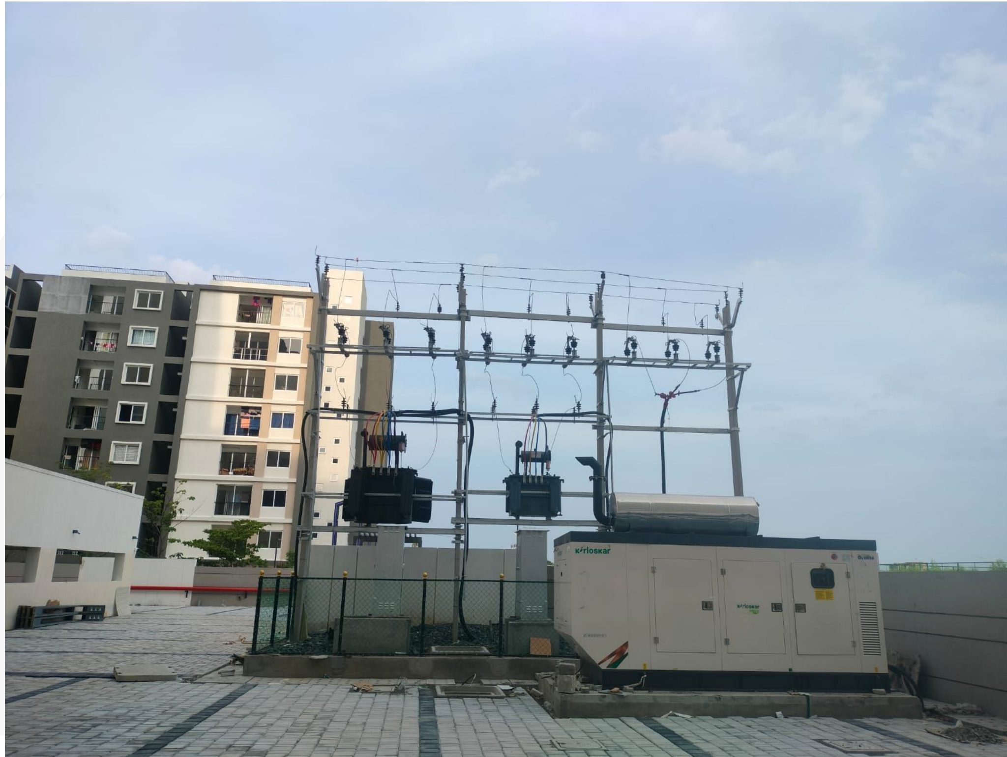
Transformer Erection Work Completed
