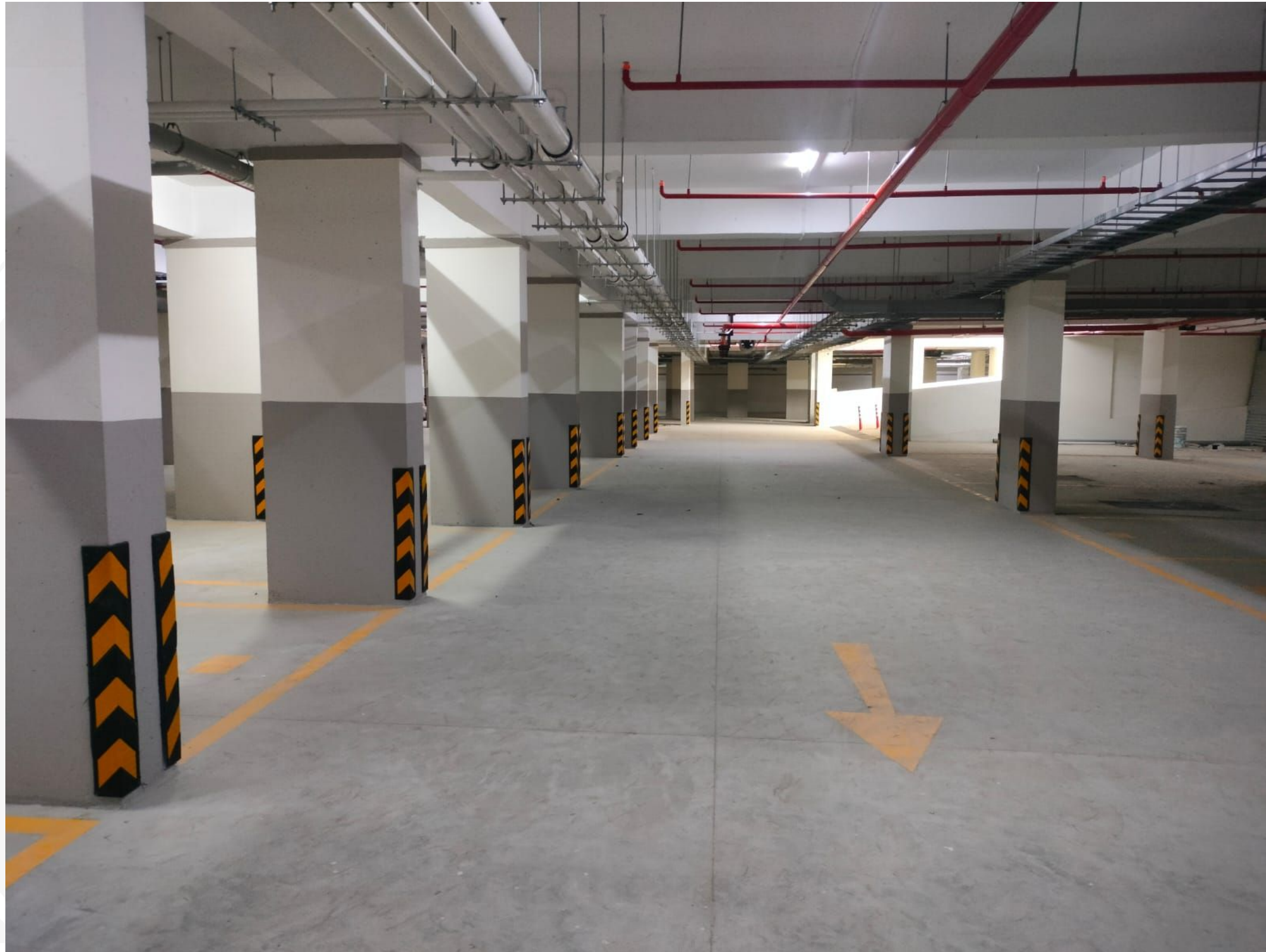
Basement 2 nd Coat painting Work Completed
