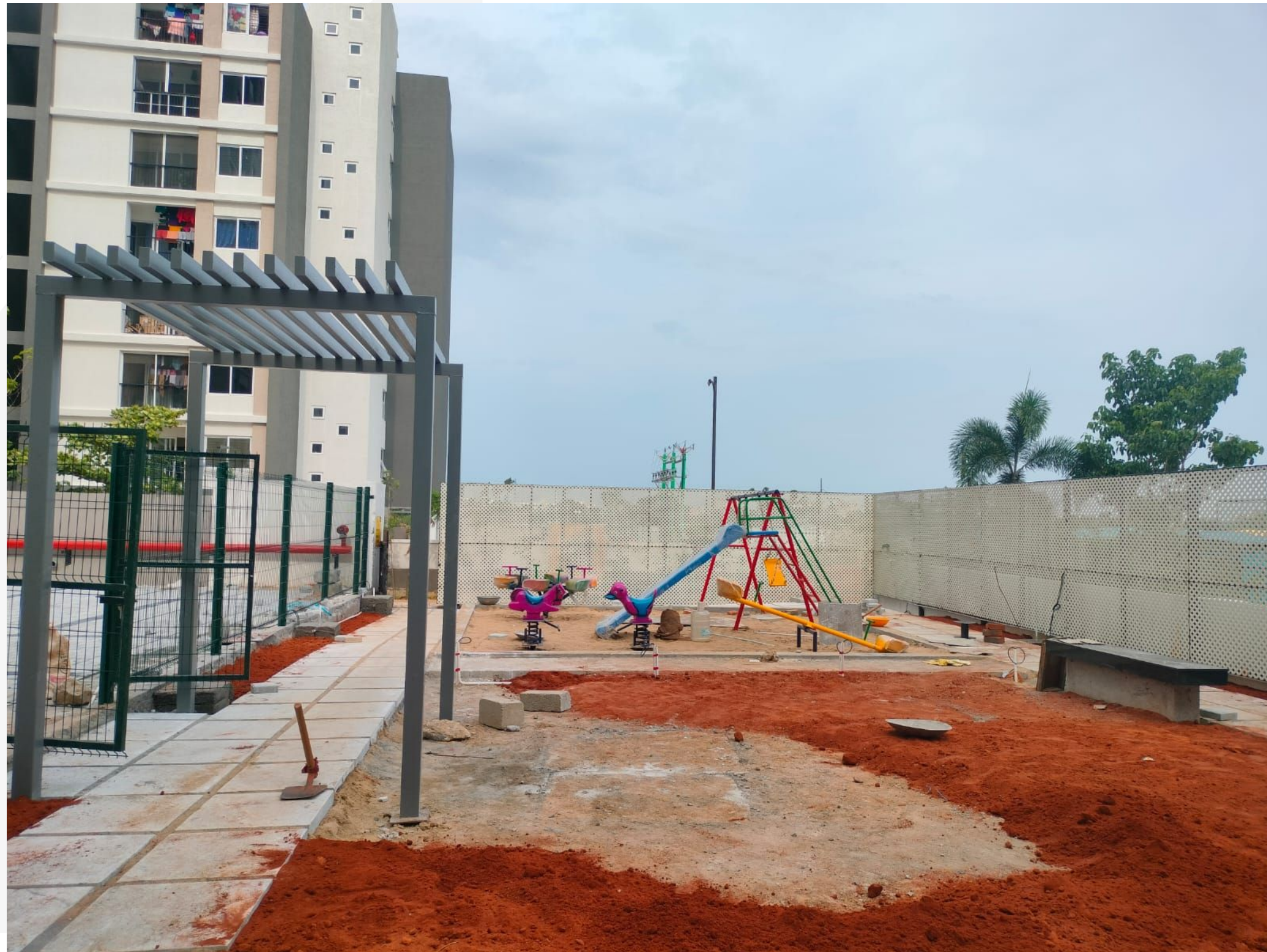
OSR Landscape Work In Progress
