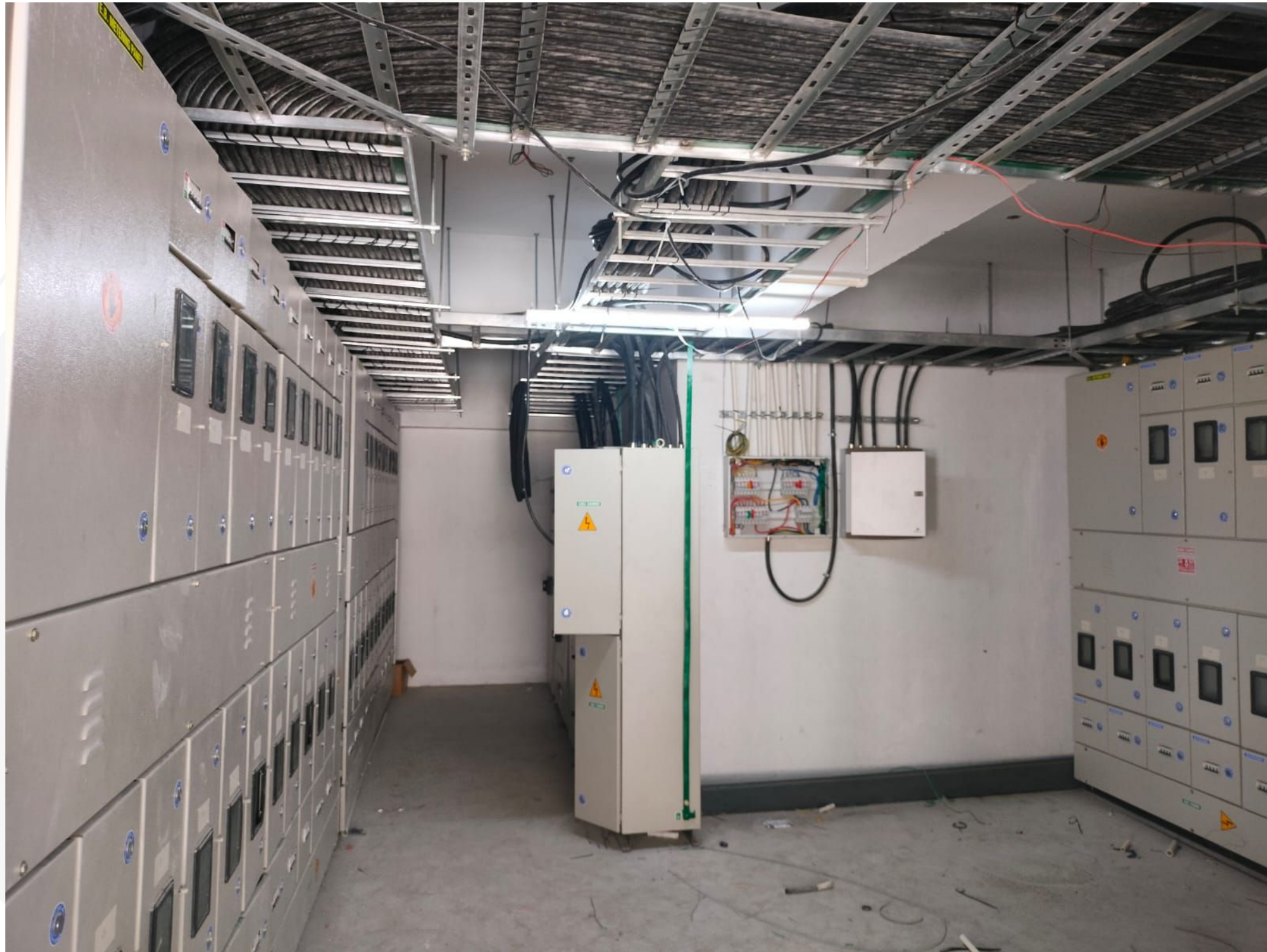
Electrical Room-1&2 Termination Work In Progress ,
