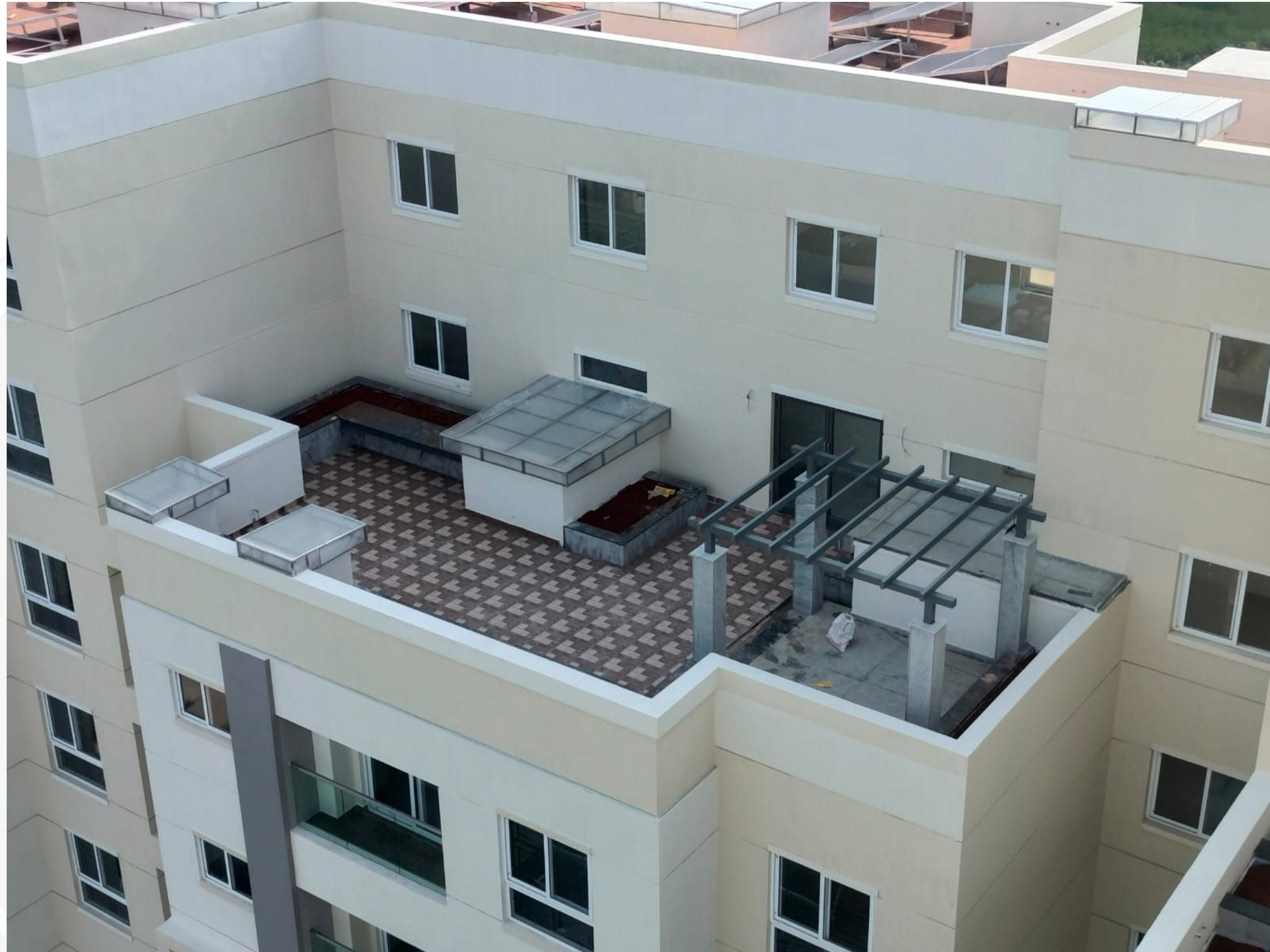
10 th Floor Levell Low Terrace Hardscape Work In Progress
