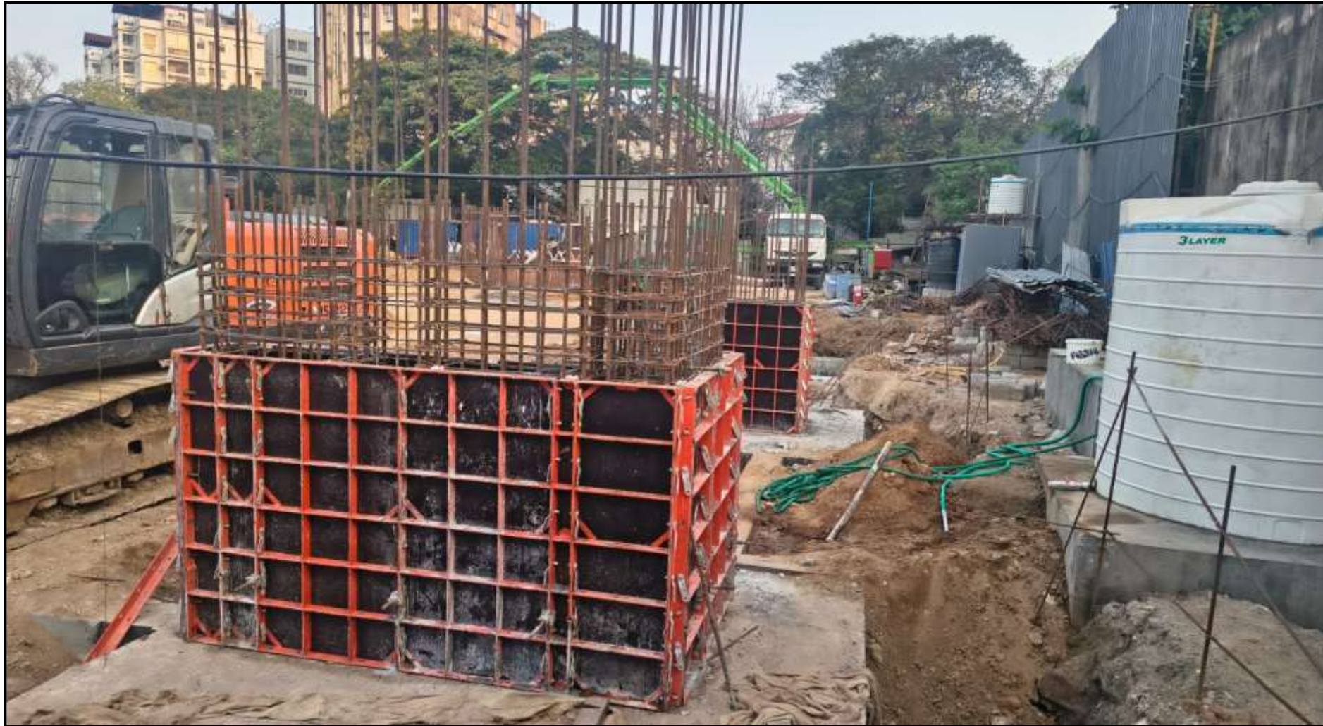
Column foundation level shuttering work in progress (15/24) – 62.5% completed
