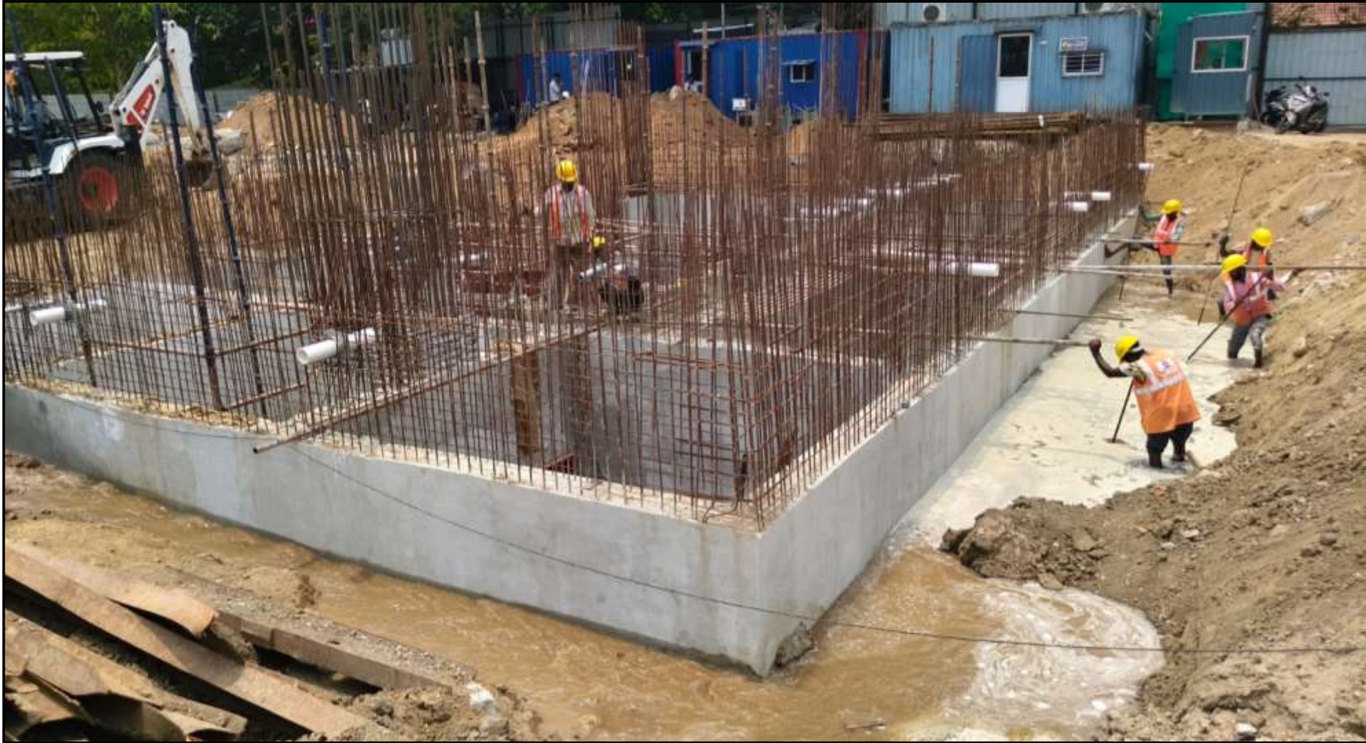
UG Sump backfilling soil consolidation work in progress
