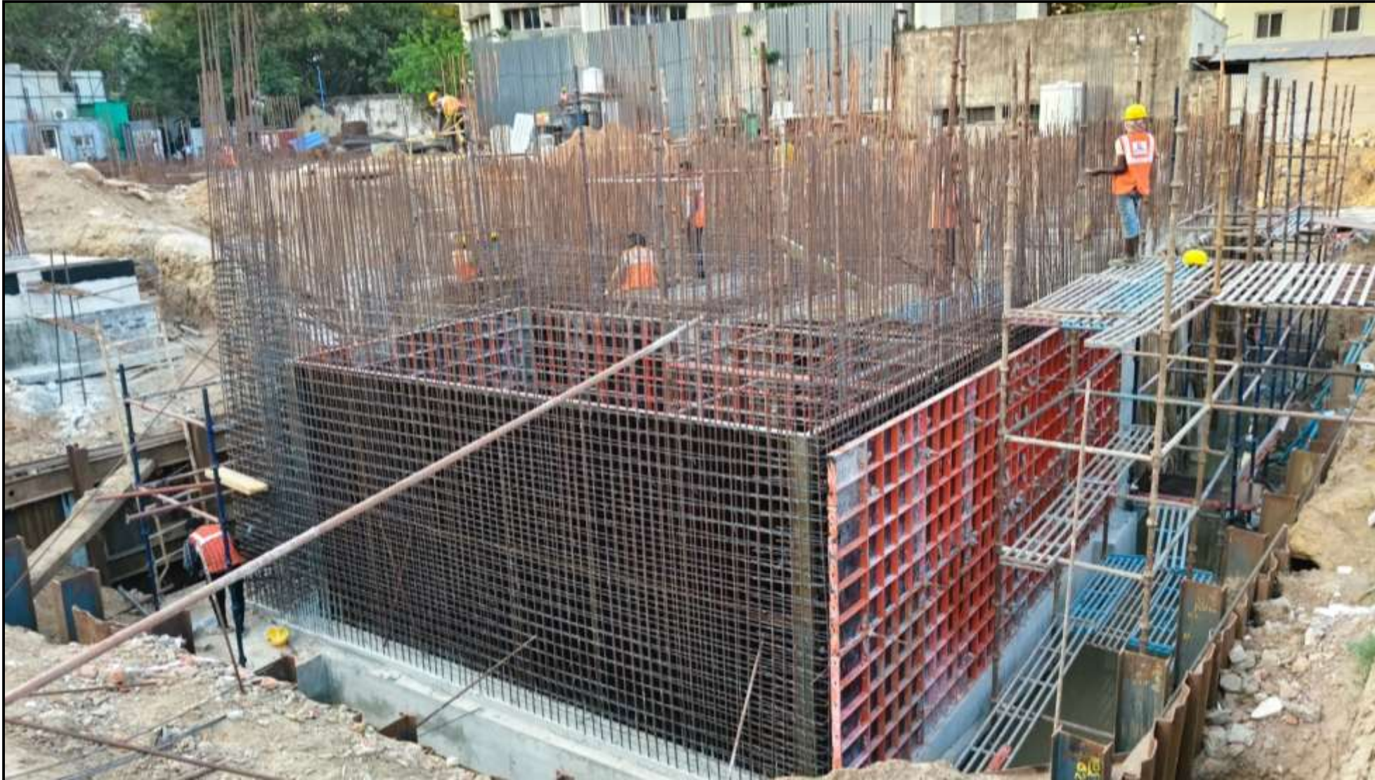
STP – RC wall reinforcement work completed
