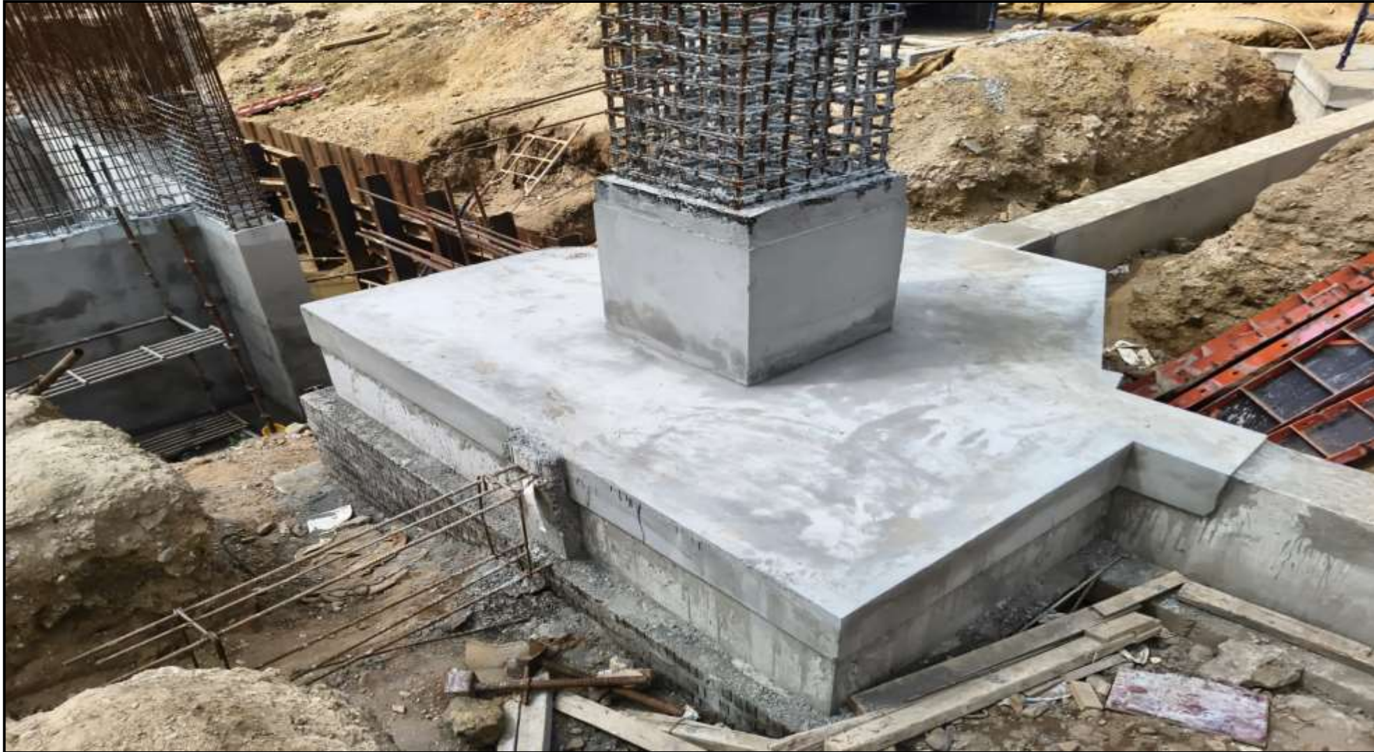
Pile cap & column DPC coating & protective plastering work in progress (8/24nos)
