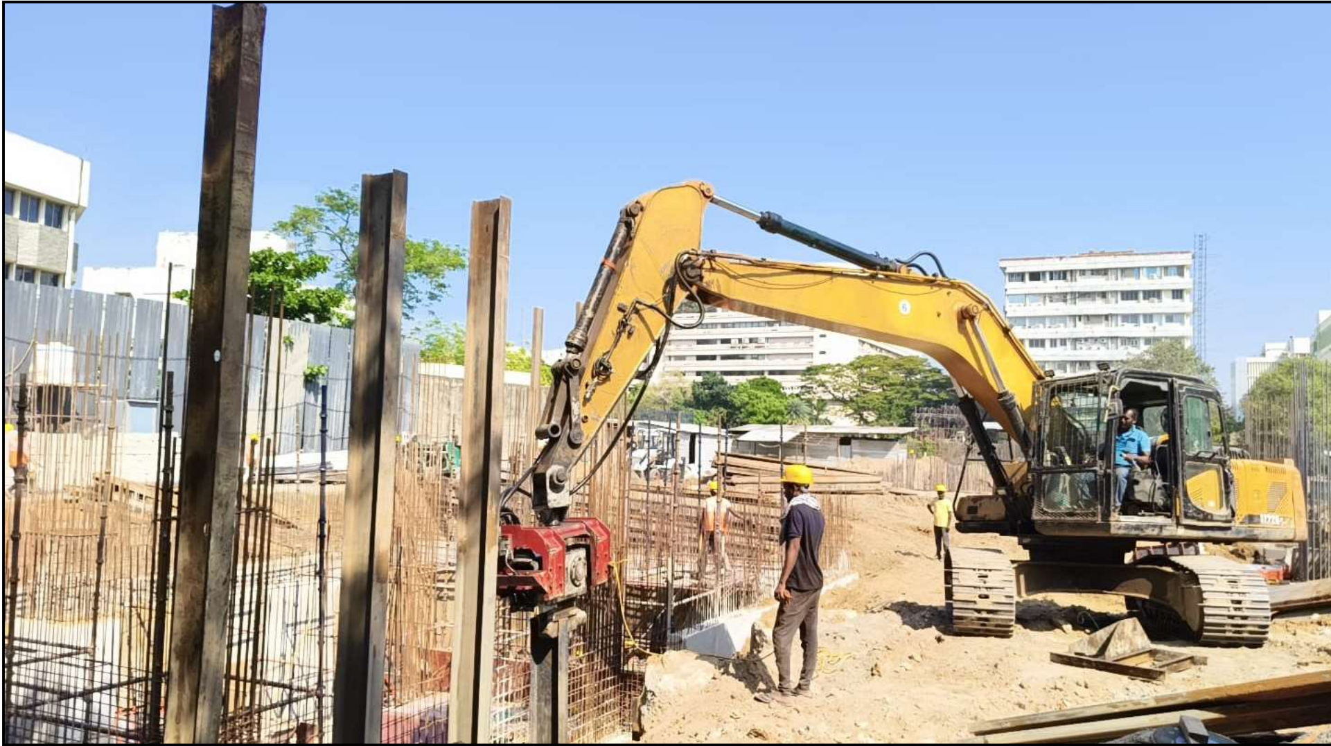
UG Sump sheet shoring removing work completed
