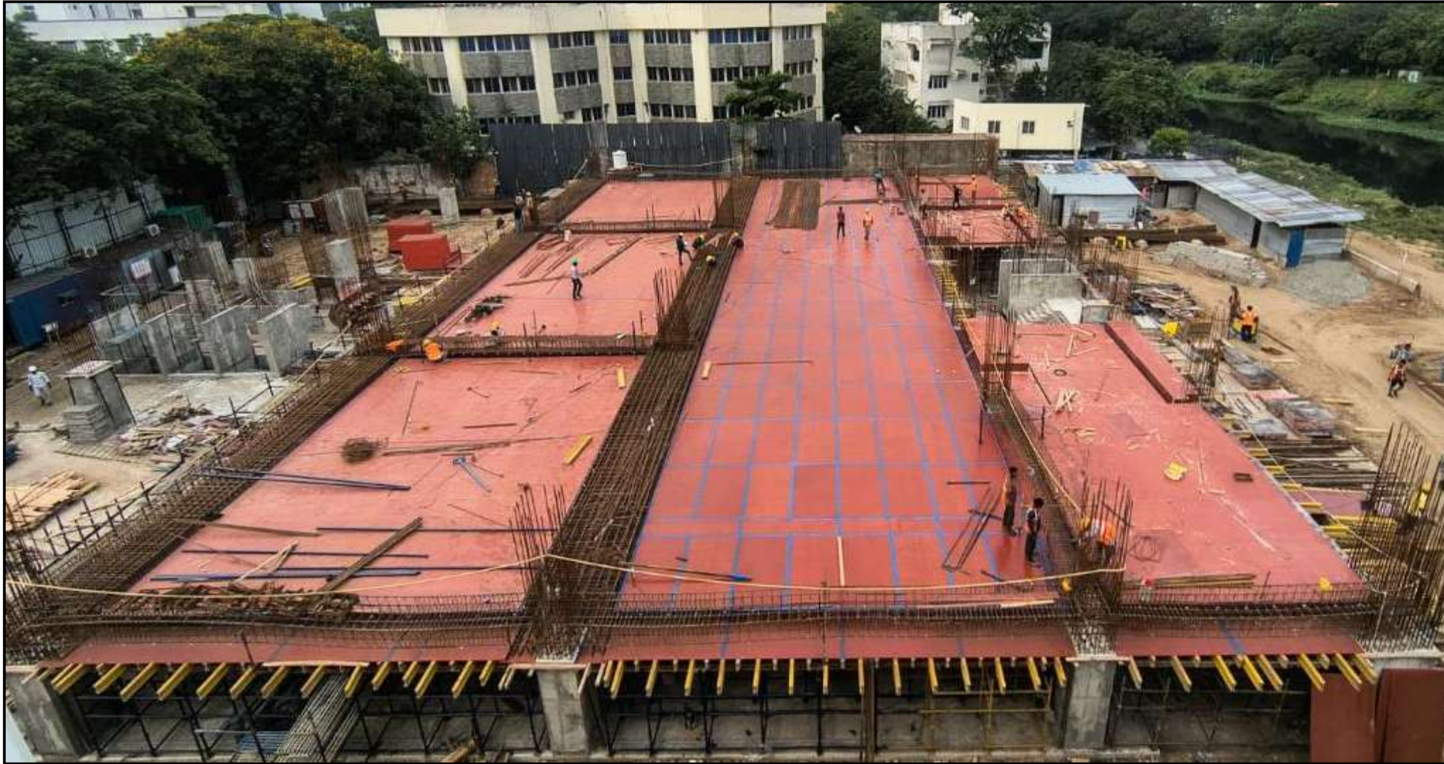
Stilt floor Pour 1 roof slab shuttering work in progress
