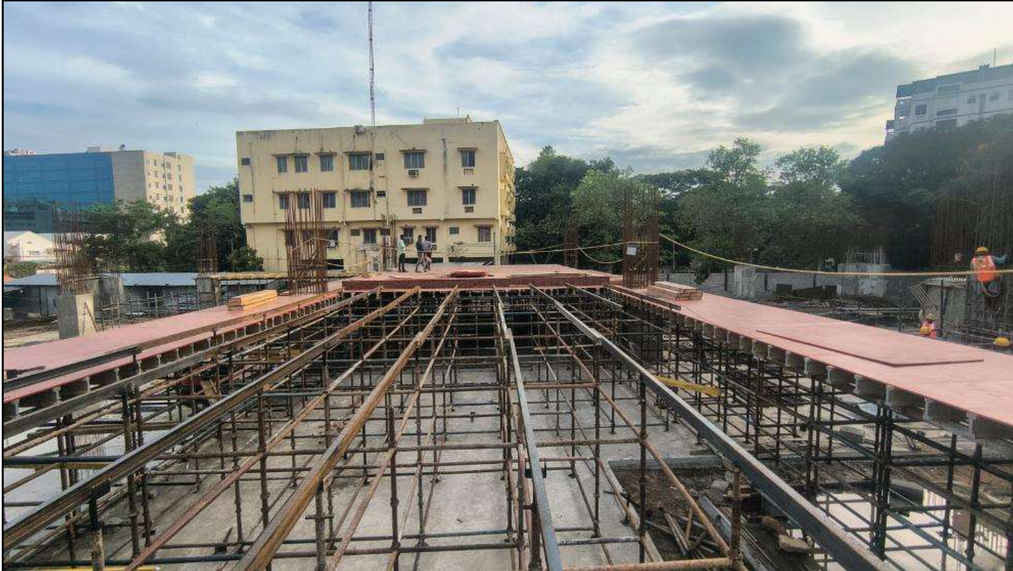
Stilt Floor Roof – Pour:1 Staging Work in Progress
