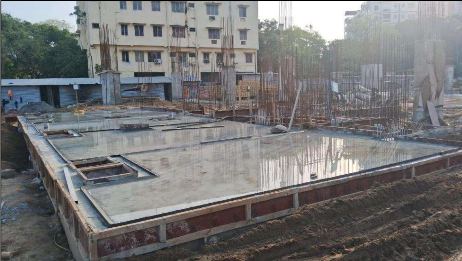
STP Cover Slab Concrete Work completed
