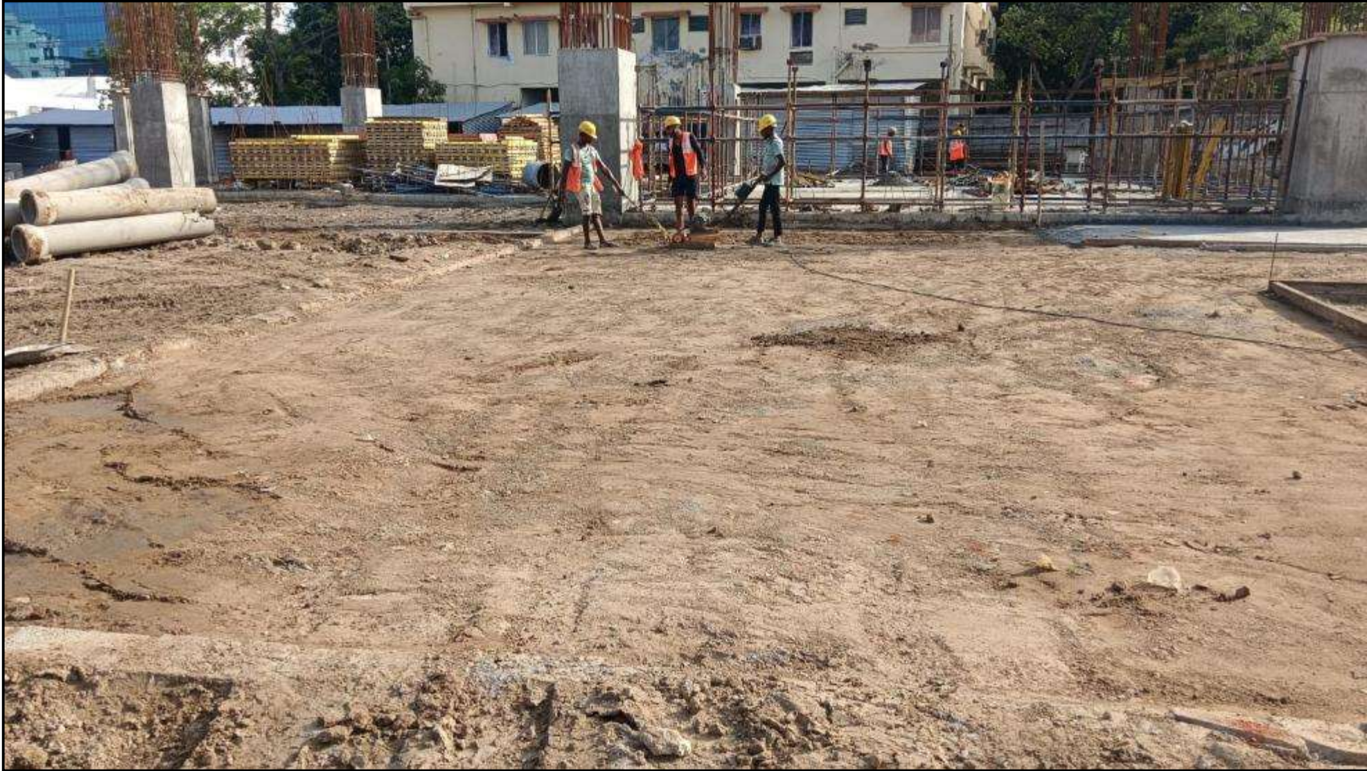
Basement Level – Soil compaction work in Progress for Grade slab work
