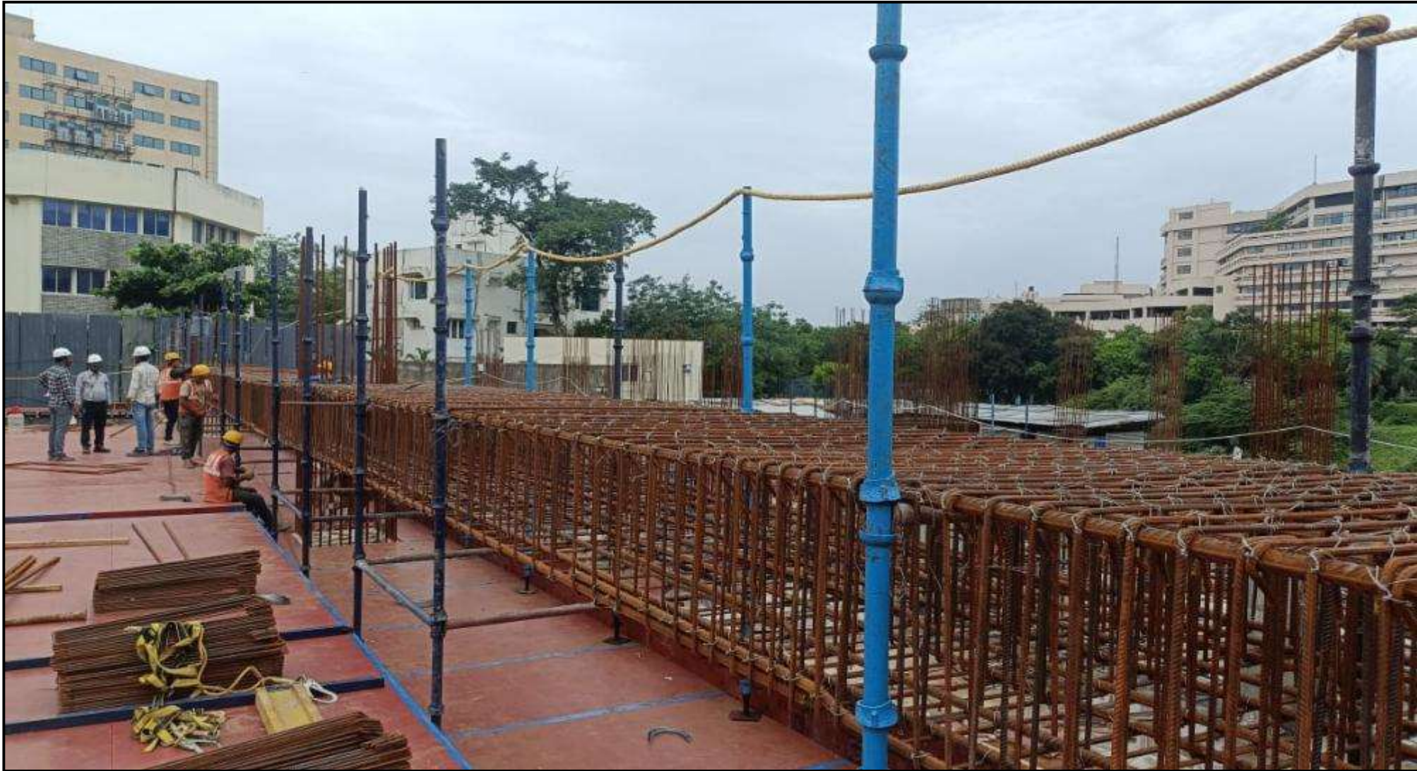
Stilt Floor – Pour 1 Roof Beam Reinforcement Work in Progress
