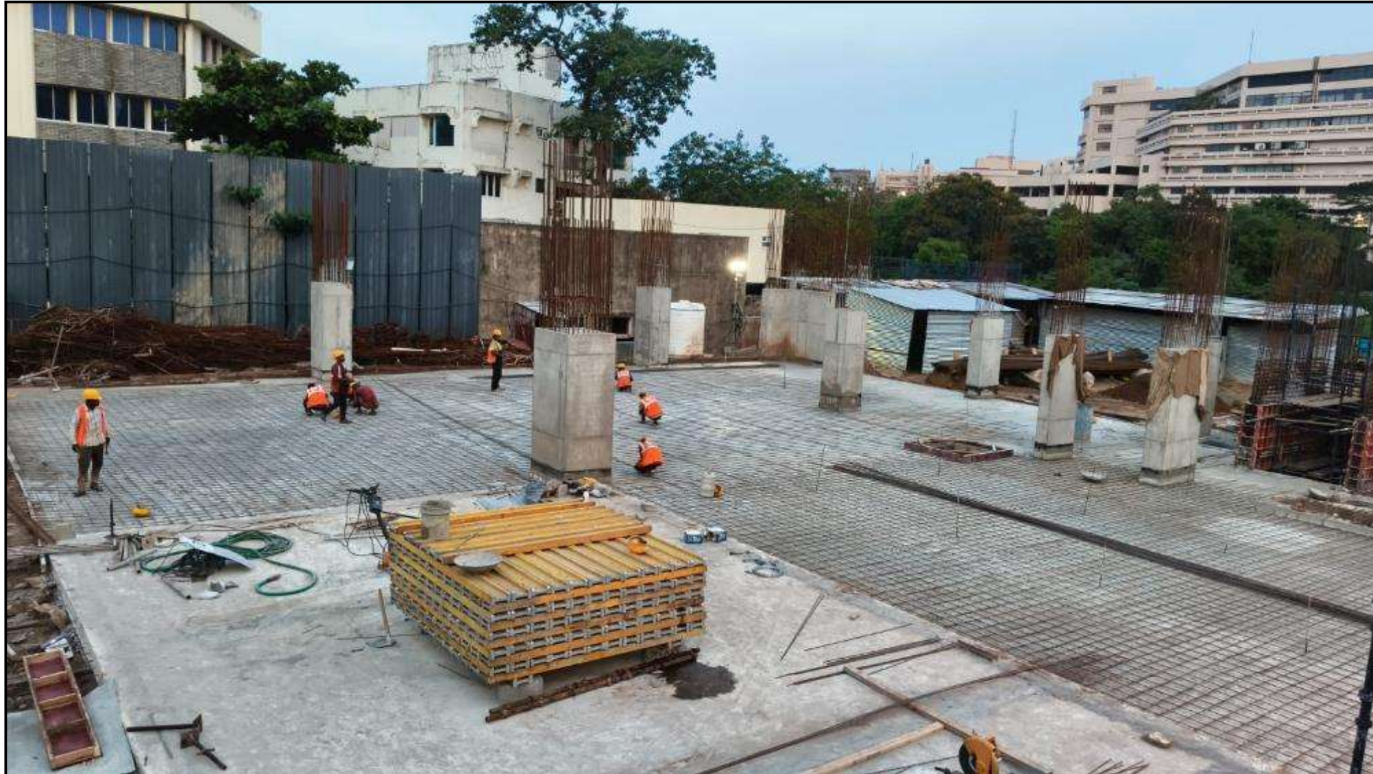
Grade Slab Reinforcement work in progress
