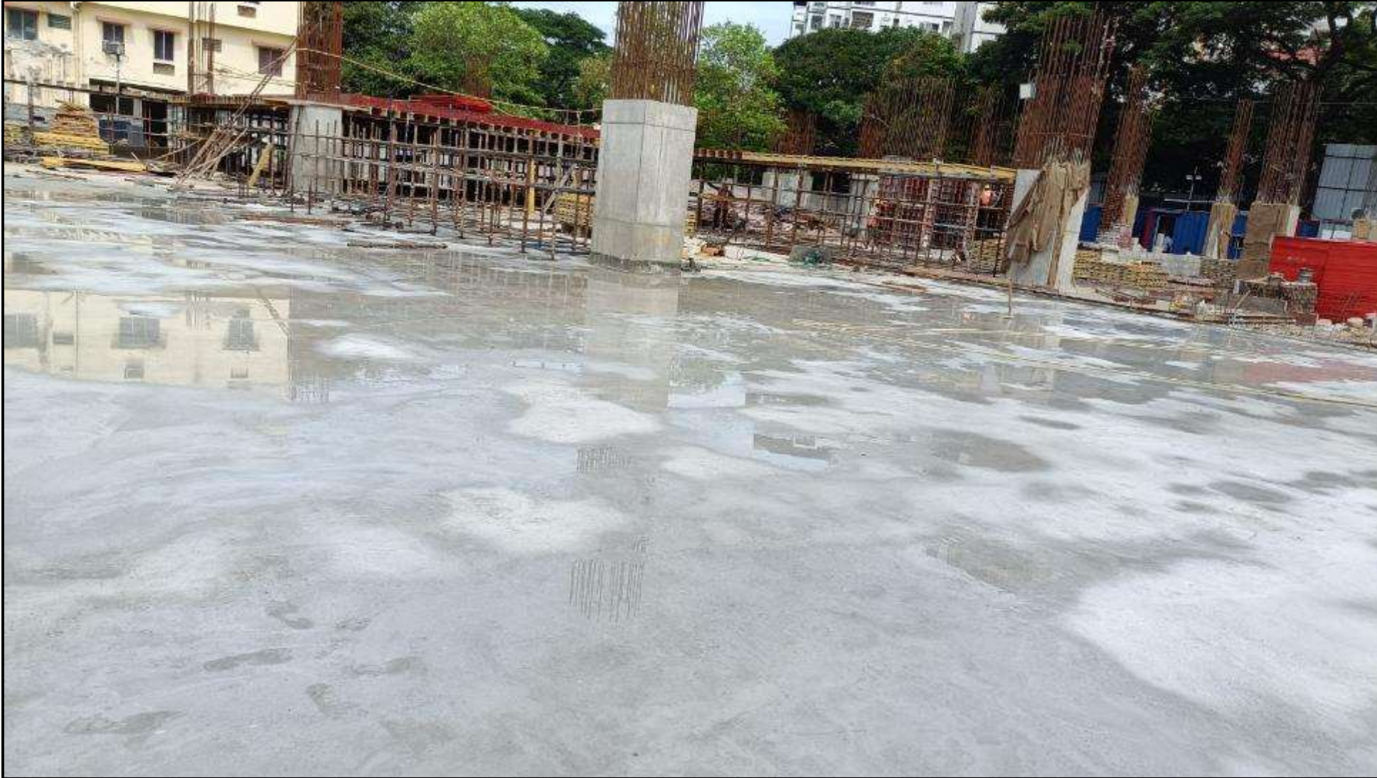
Grade Slab – Concrete laying Completed
