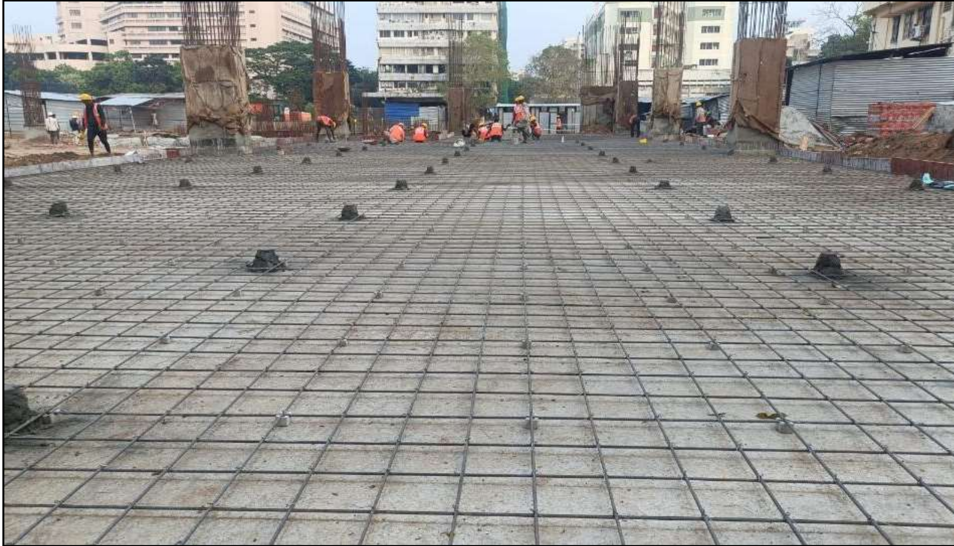
Grade slab reinforcement work in Progress – 25% Completed
