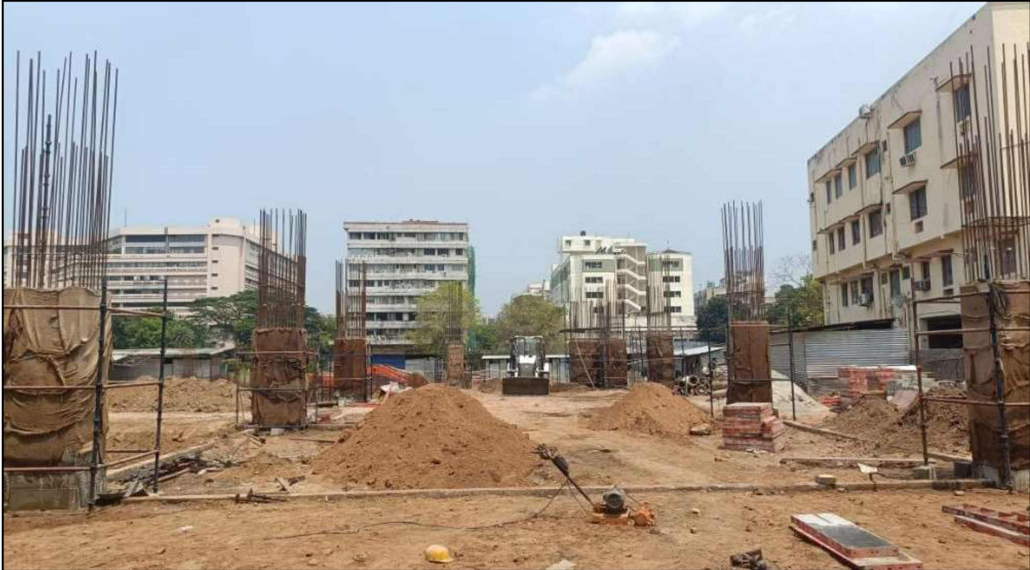
Stilt roof level column concrete work in progress (22/42nos) – 52.3% completed
