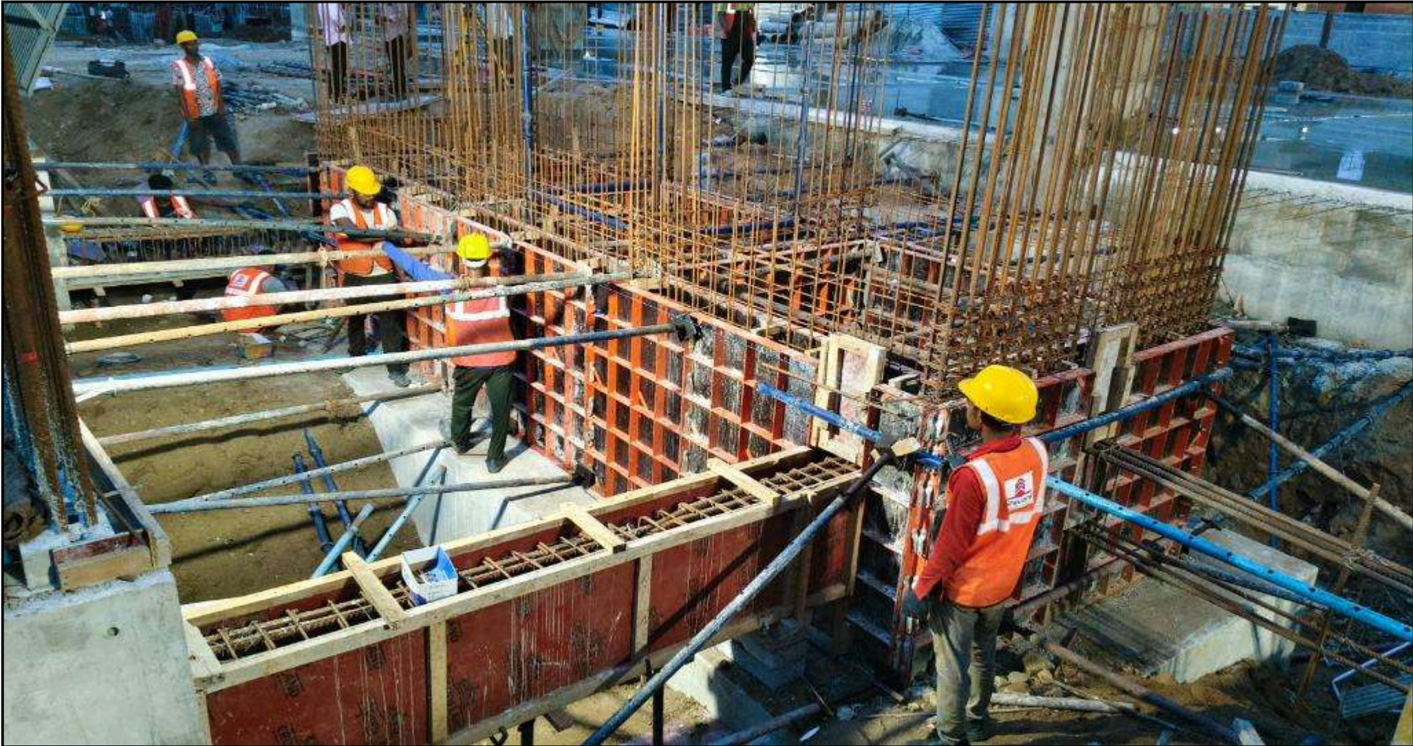
Lift wall reinforcement & shuttering work completed
