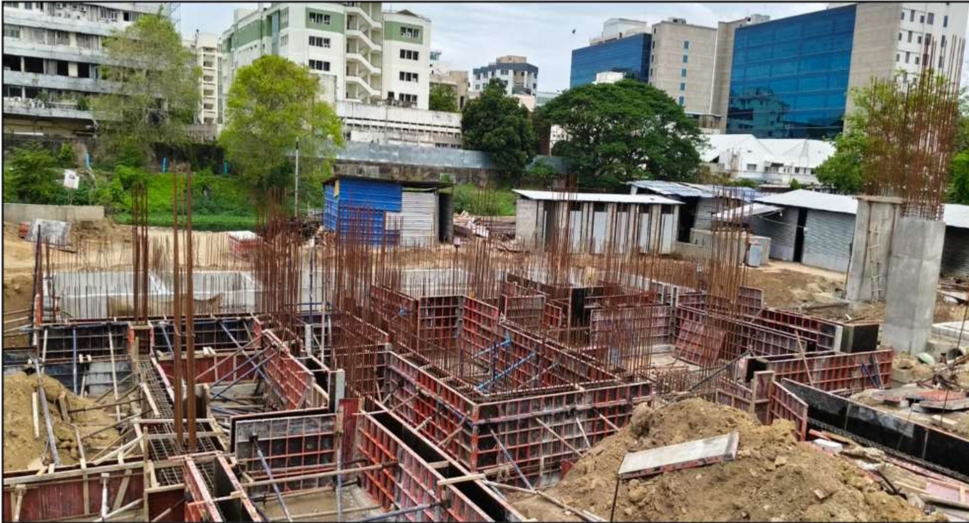
STP 2 nd lift RC wall shuttering work completed
