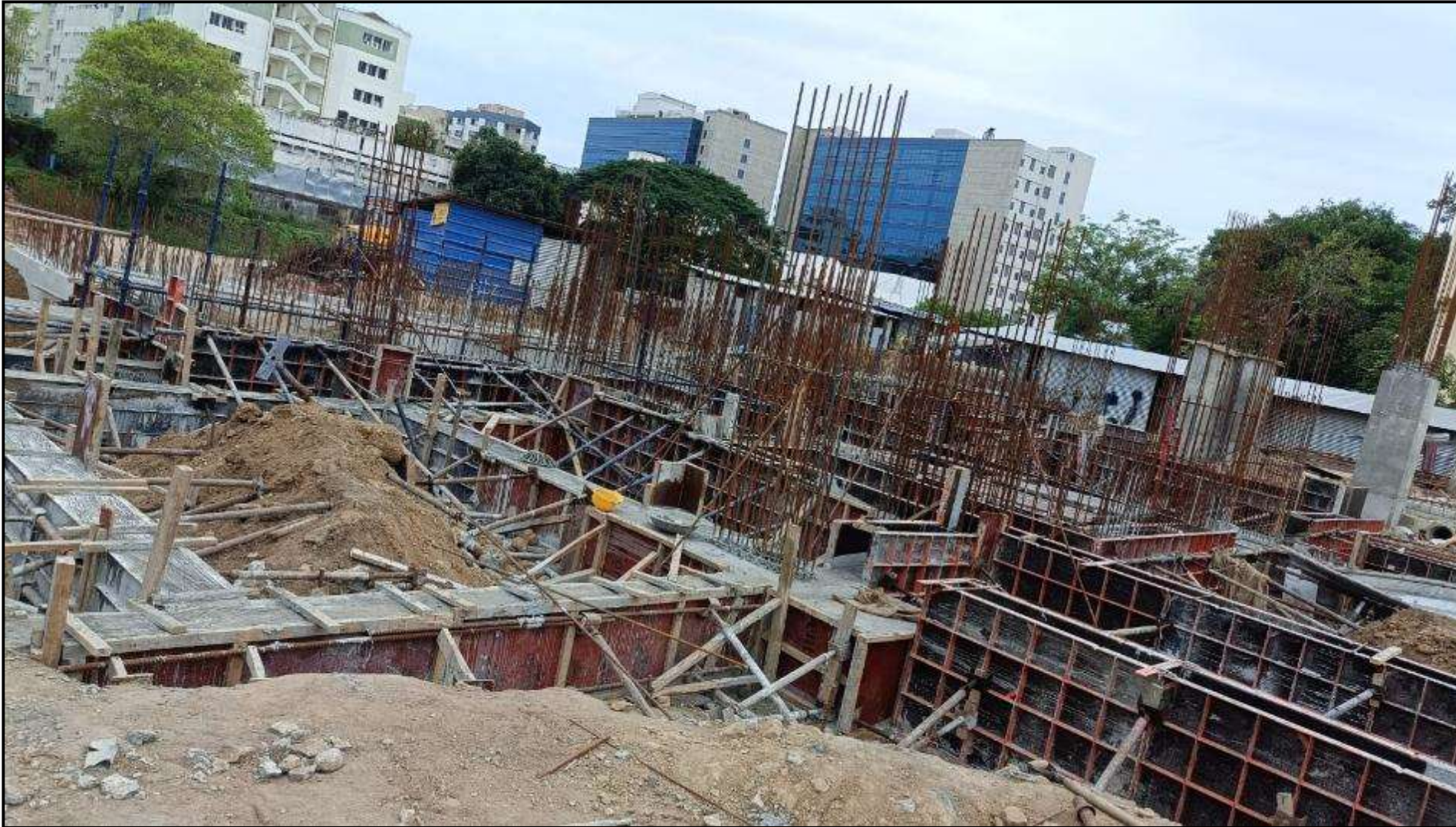
STP 2 nd lift RC wall concrete work completed
