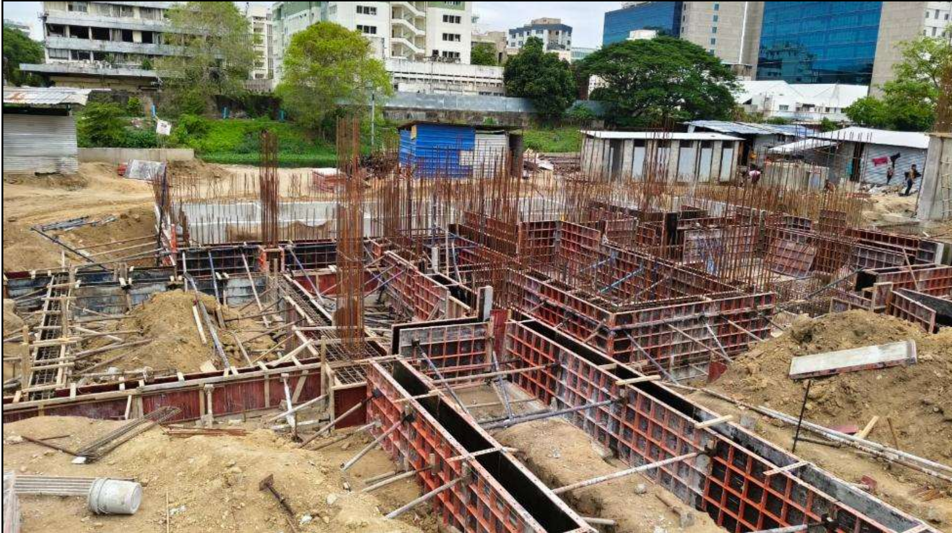
Plinth beam shuttering work in progress (280/370Sqm) – 75.7% completed
