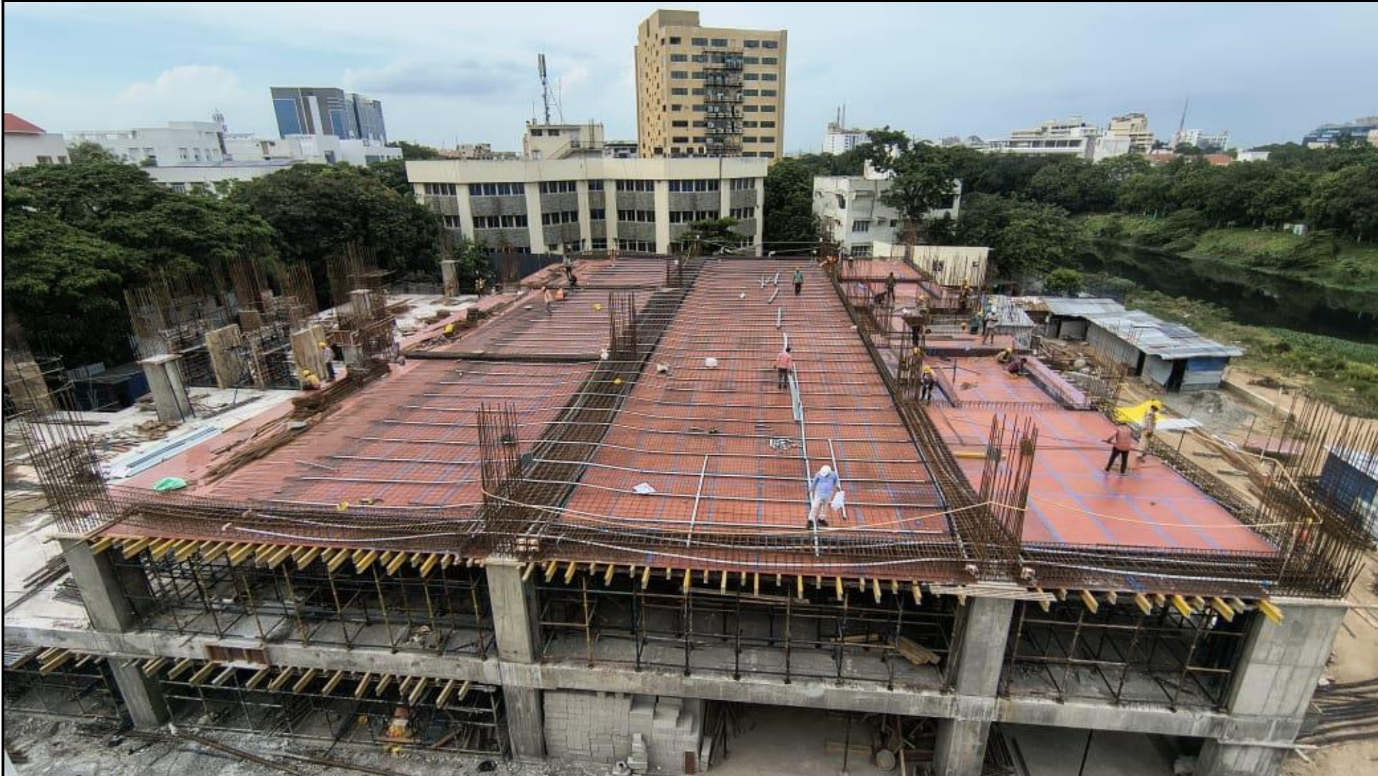
First Floor – Pour 1 Roof Slab Shuttering work is completed ( 1598/1598 Sqm)
