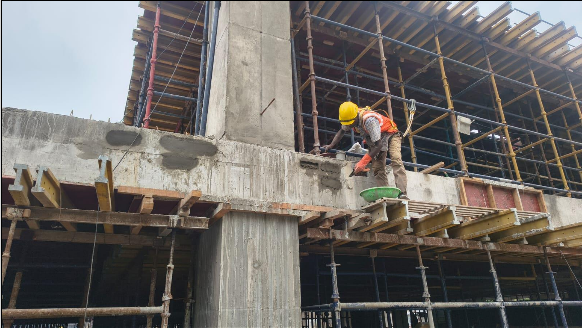
Stilt floor – Pour 2 Roof slab PT Strands Stressed ends packing work is Completed
