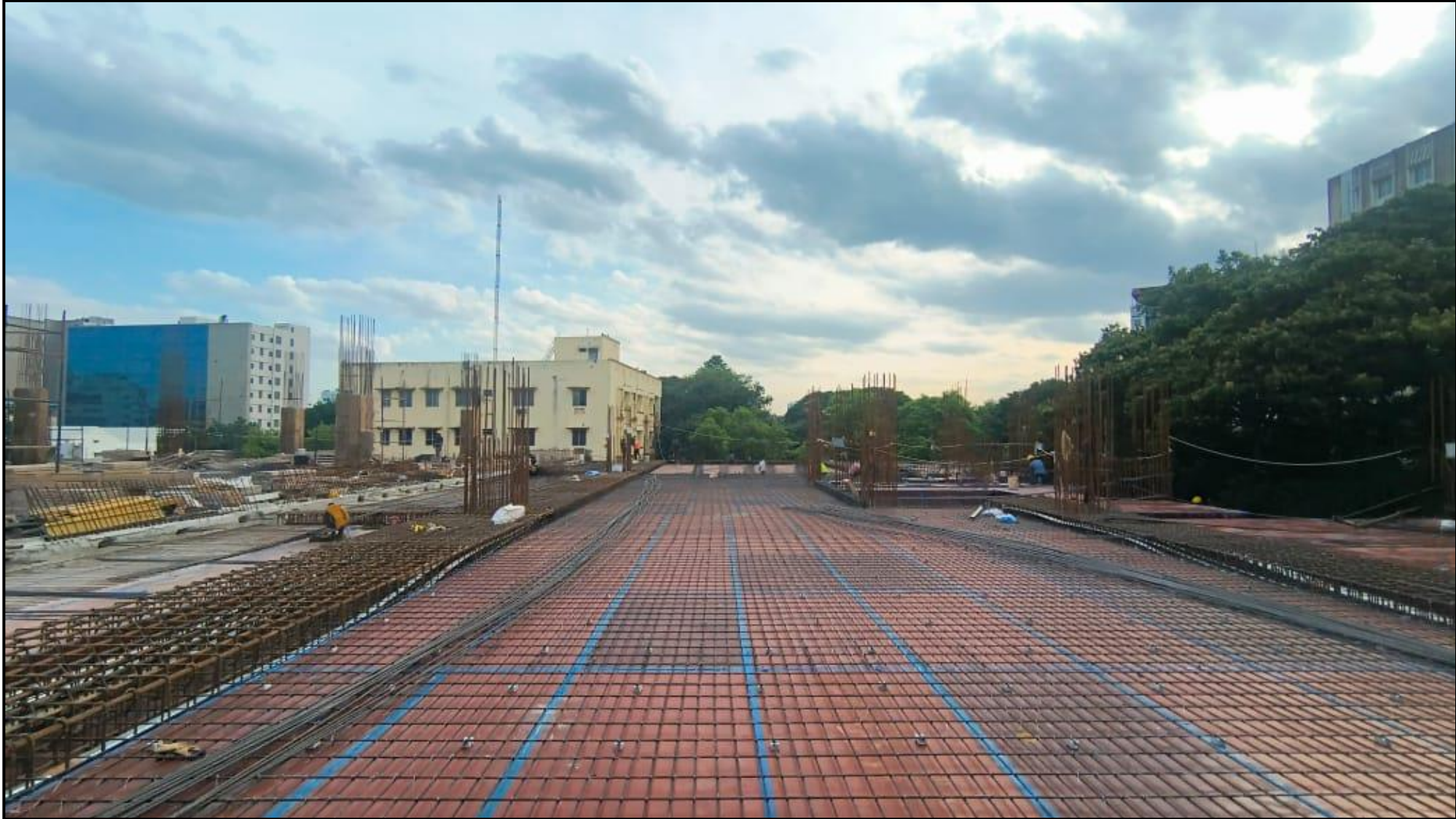
First floor pour-02 roof slab reinforcement work in progress (28/42MT) – 66.6% Completed
