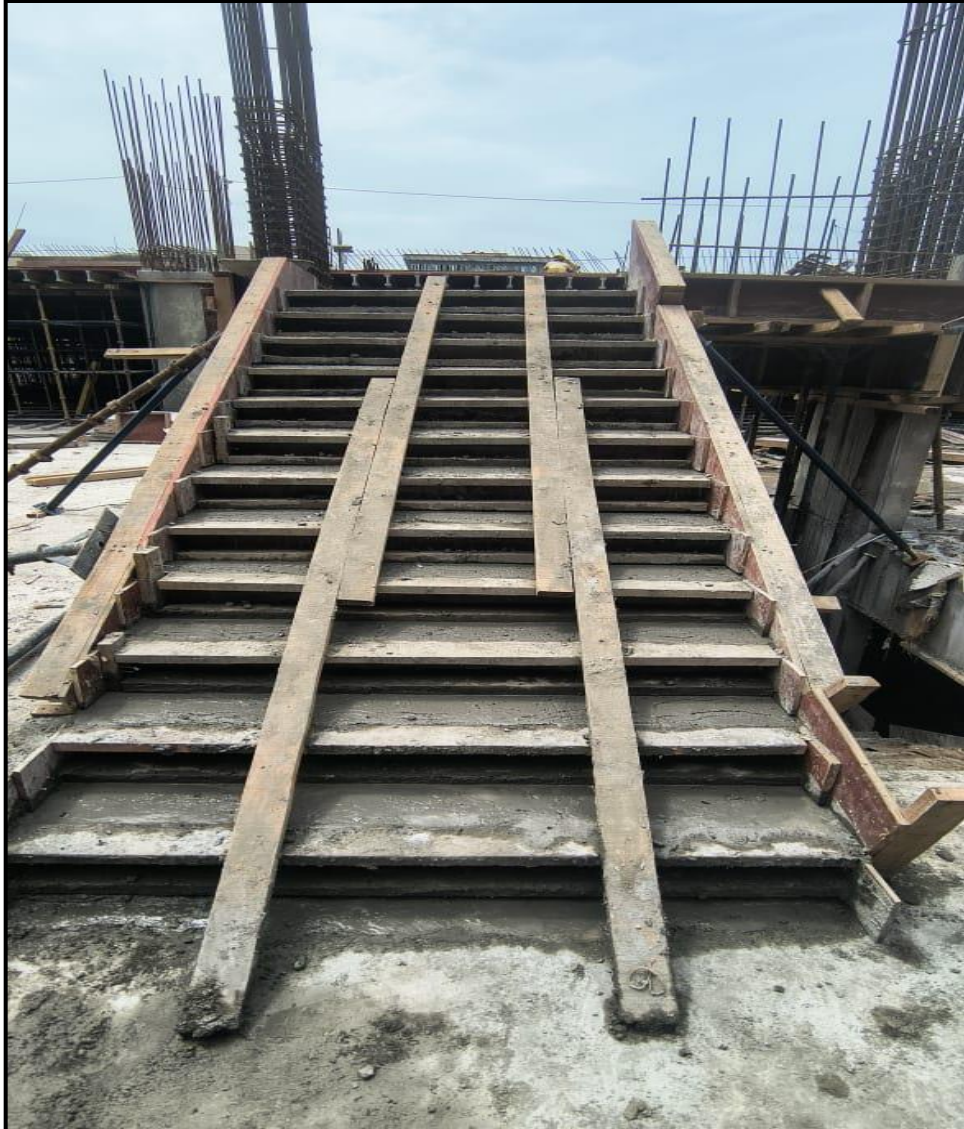
First floor pour-02 staircase 1st flight slab concrete work completed
