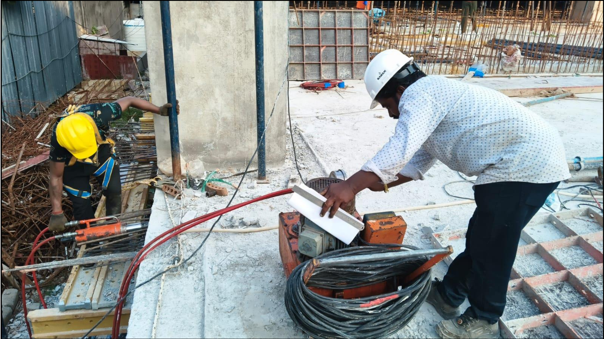
Stilt floor – Pour 2 Roof slab PT Strands Stressing work is Completed
