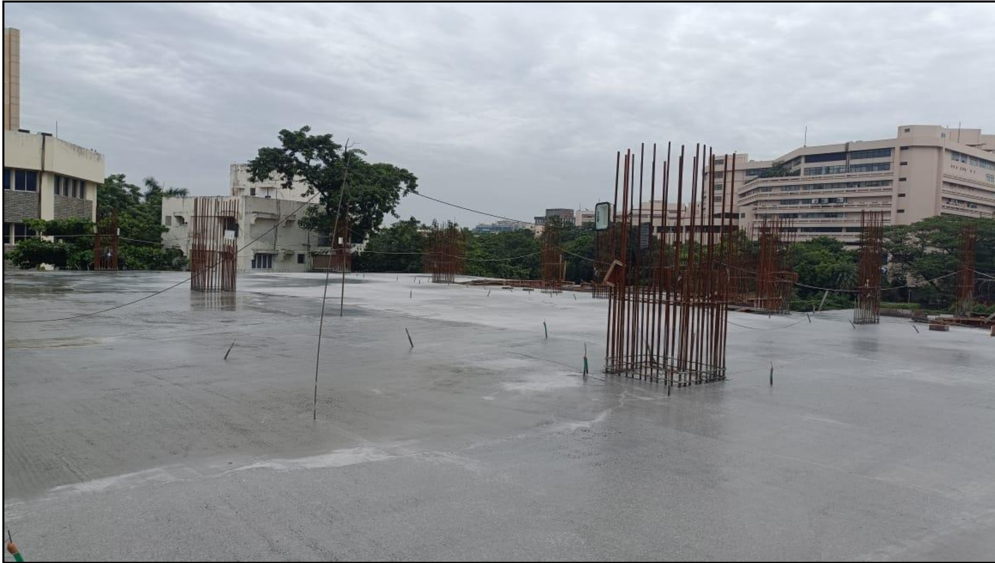
First floor pour-01 roof slab concrete work completed (370/370Cum) – 100%completed
