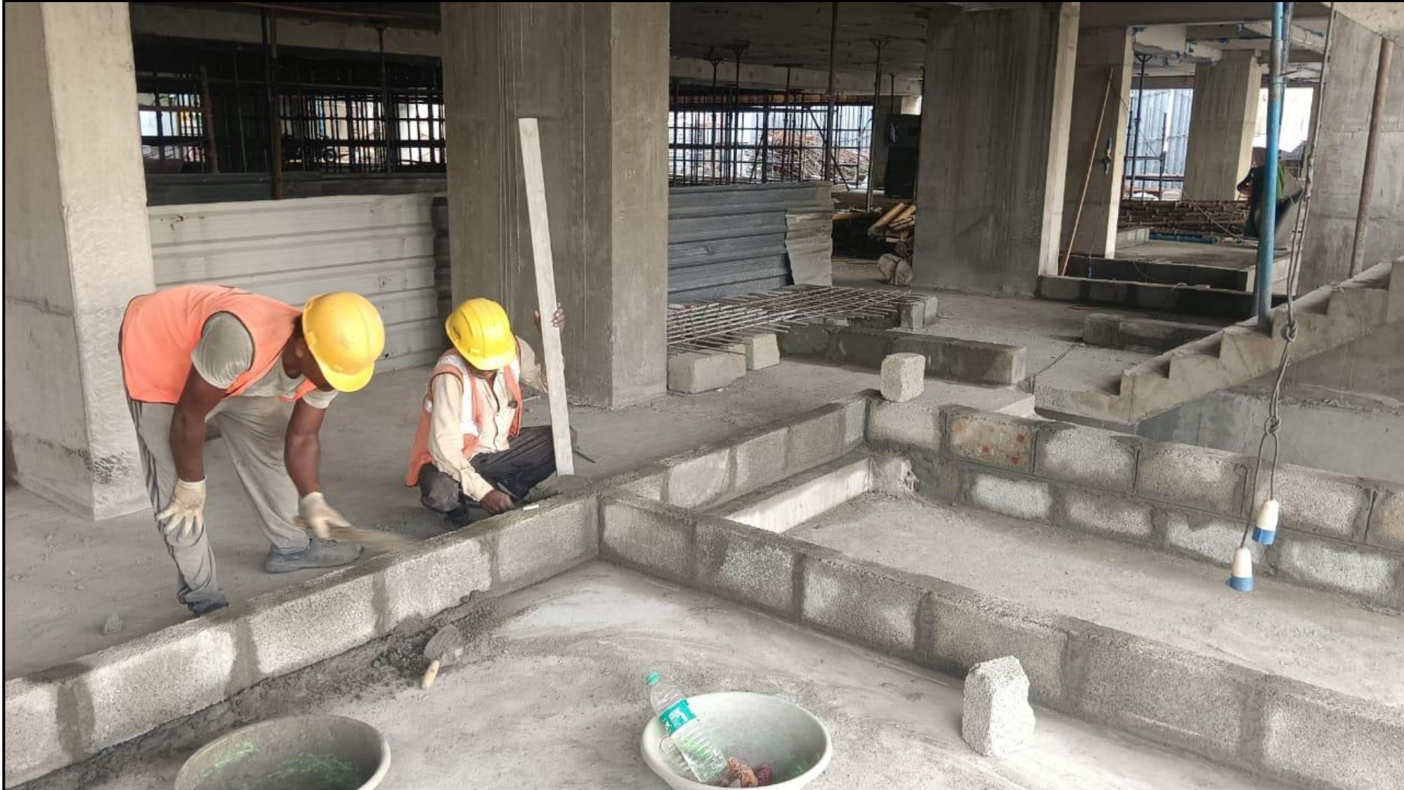
Stilt floor Single line blockwork marking work completed
