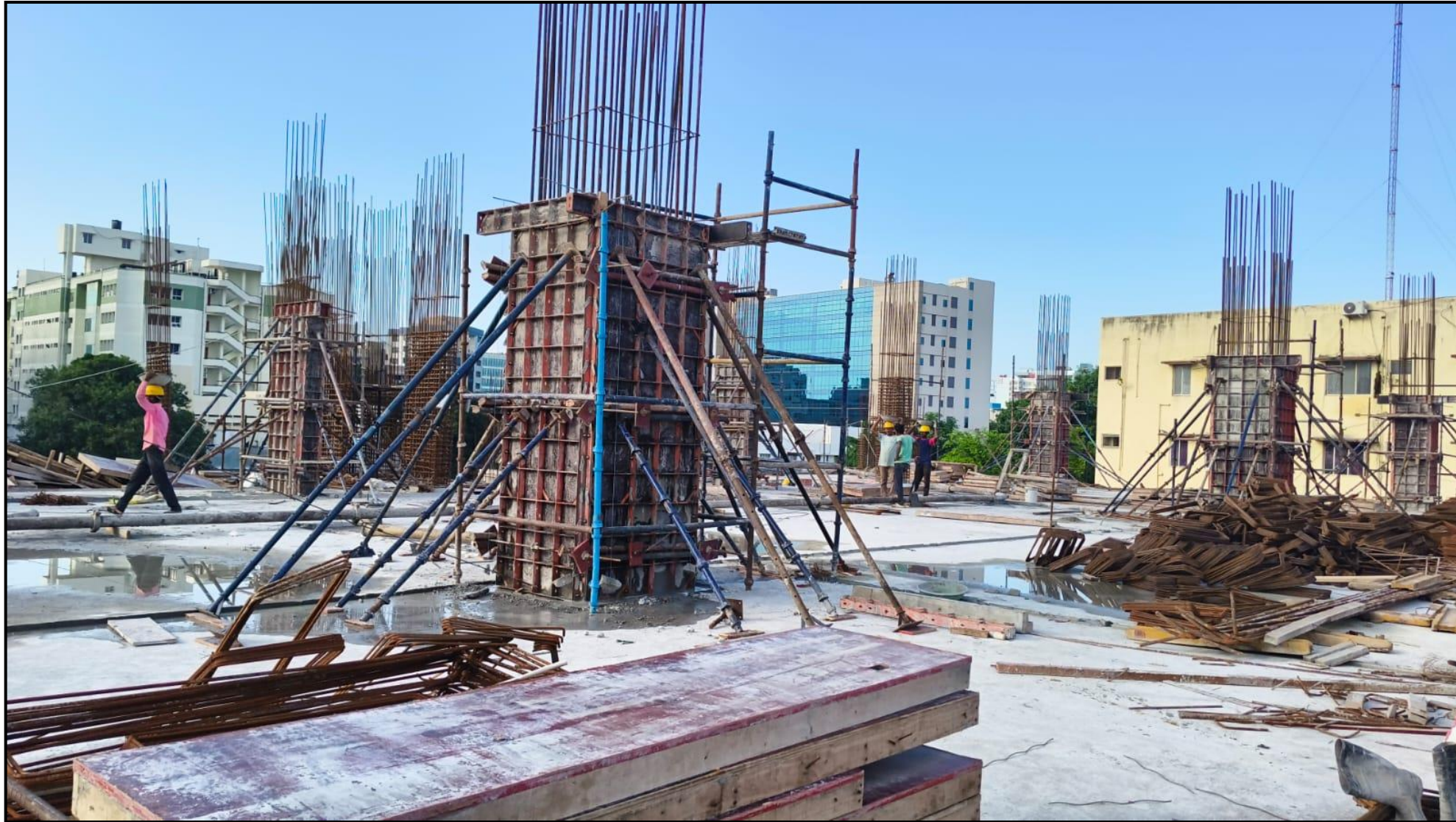
Second floor pour 1 column concrete work in progress (8/22nos) – 36% Completed
