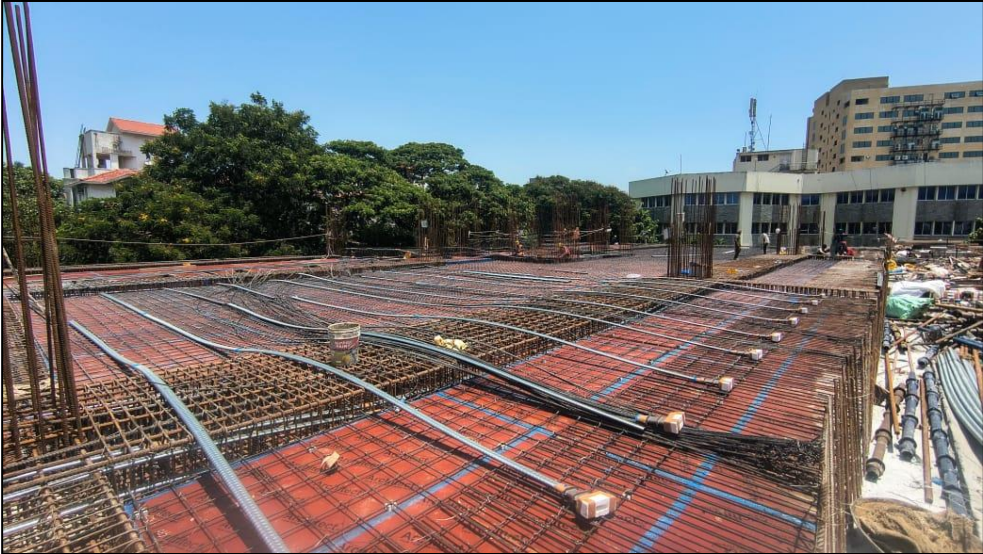
First Floor – Pour 2 Roof Slab PT Strands laying in Progress ( 2/6 MT) – 33.3% Completed
