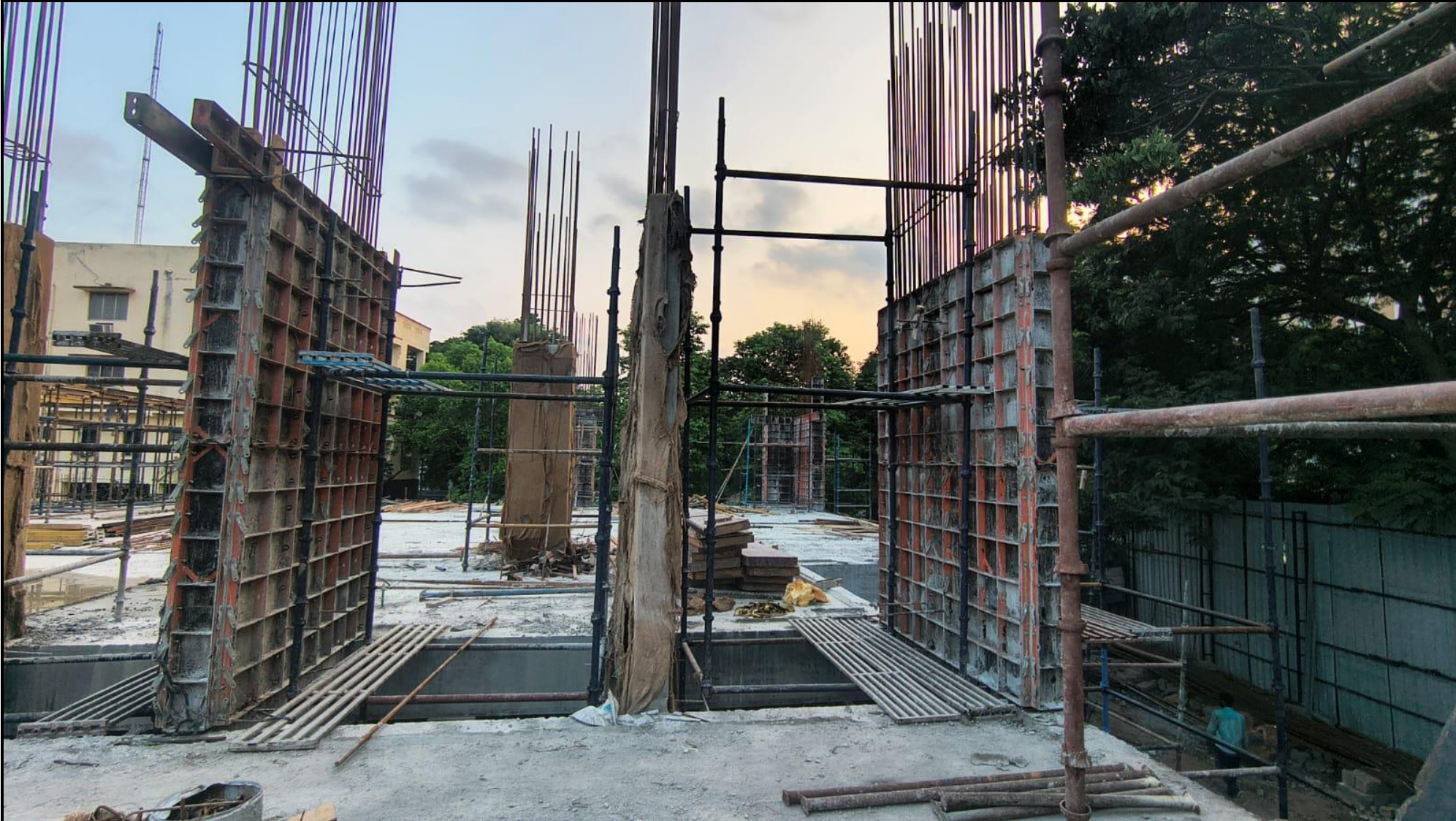
First Floor – Pour 2 – Column shuttering work in progress (20/20 Nos Completed)
