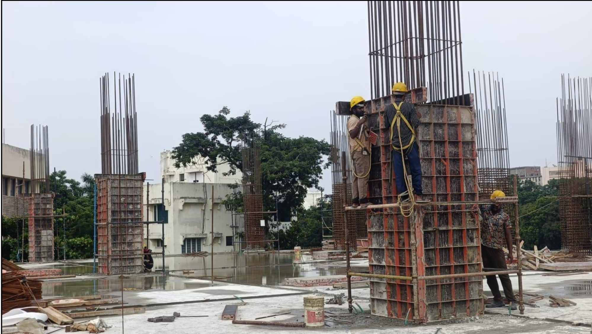
Second floor pour 1 column shuttering work in progress (12/22nos) – 55% Completed
