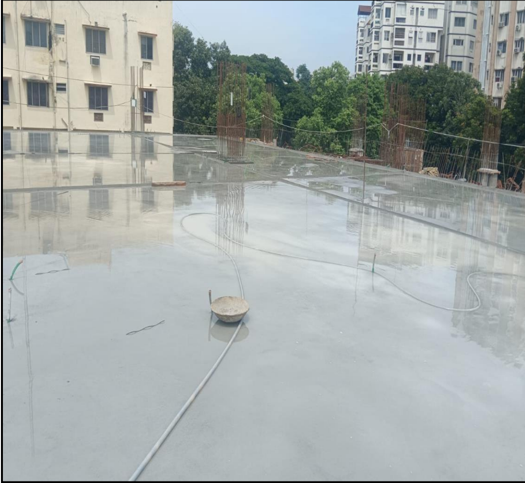
First floor pour-01 roof slab curing work
