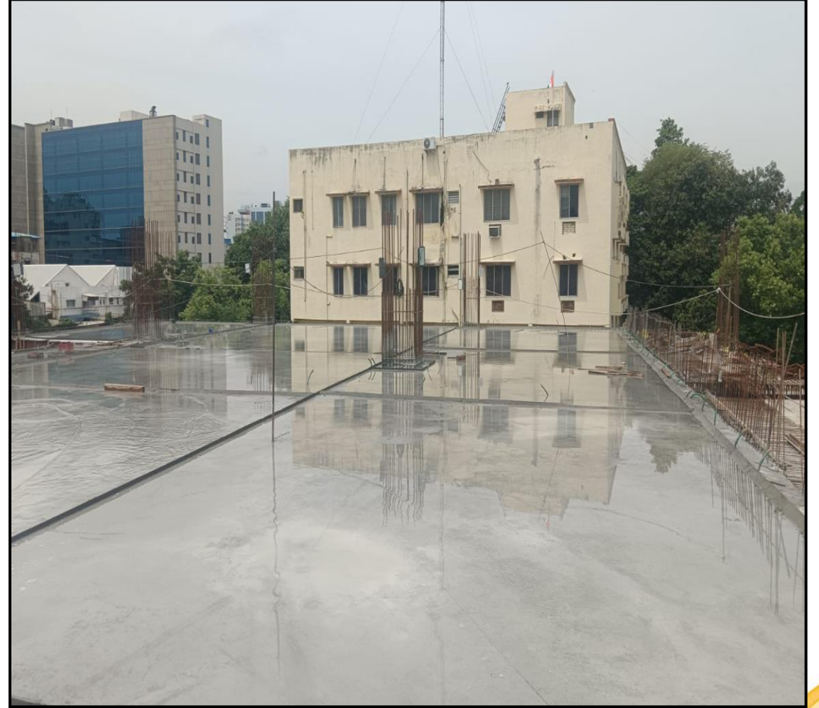
First floor pour-01 roof slab curing work
