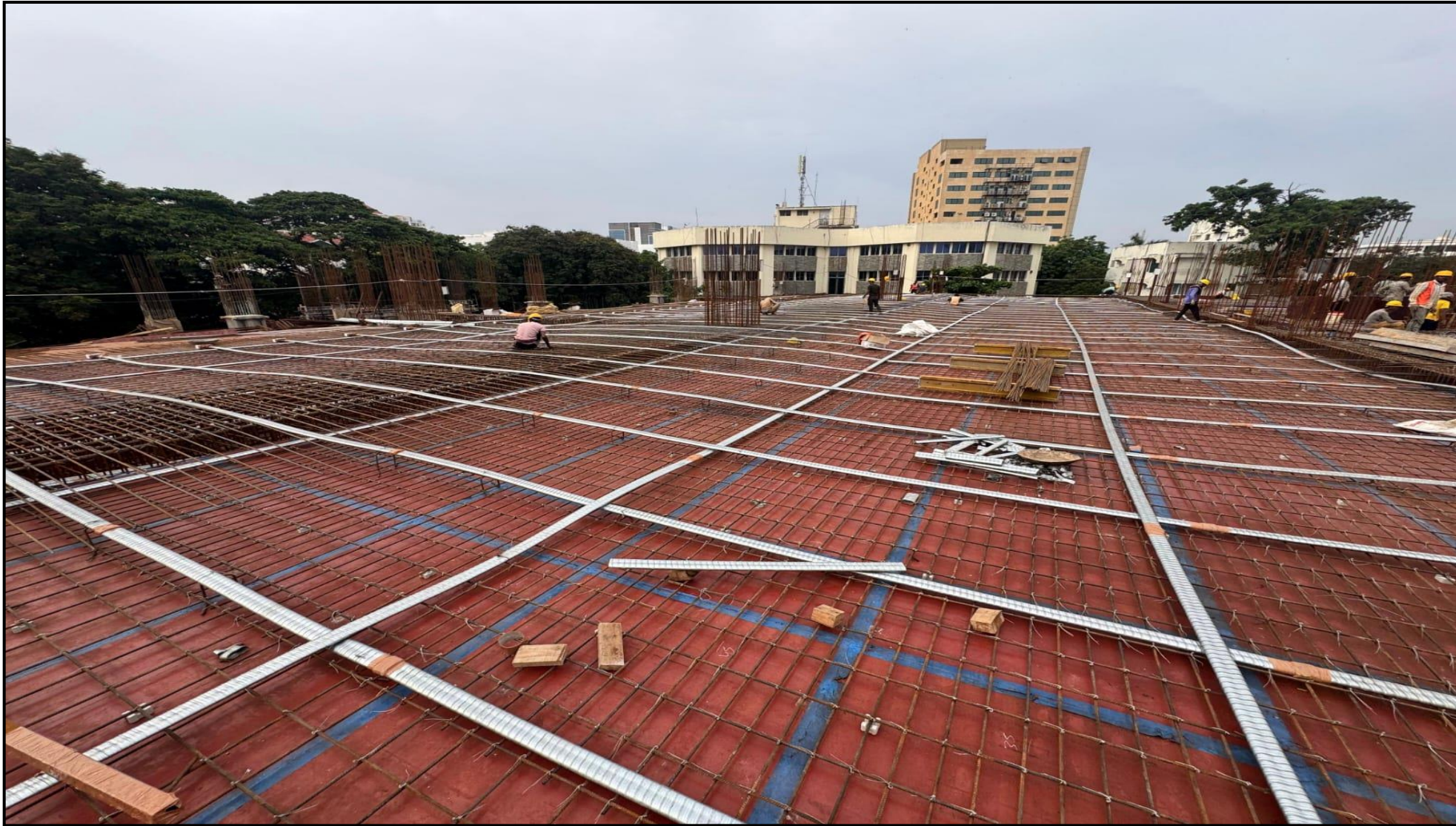
First floor pour-01 roof slab PT work completed (6.5/6.5MT) – 100%completed
