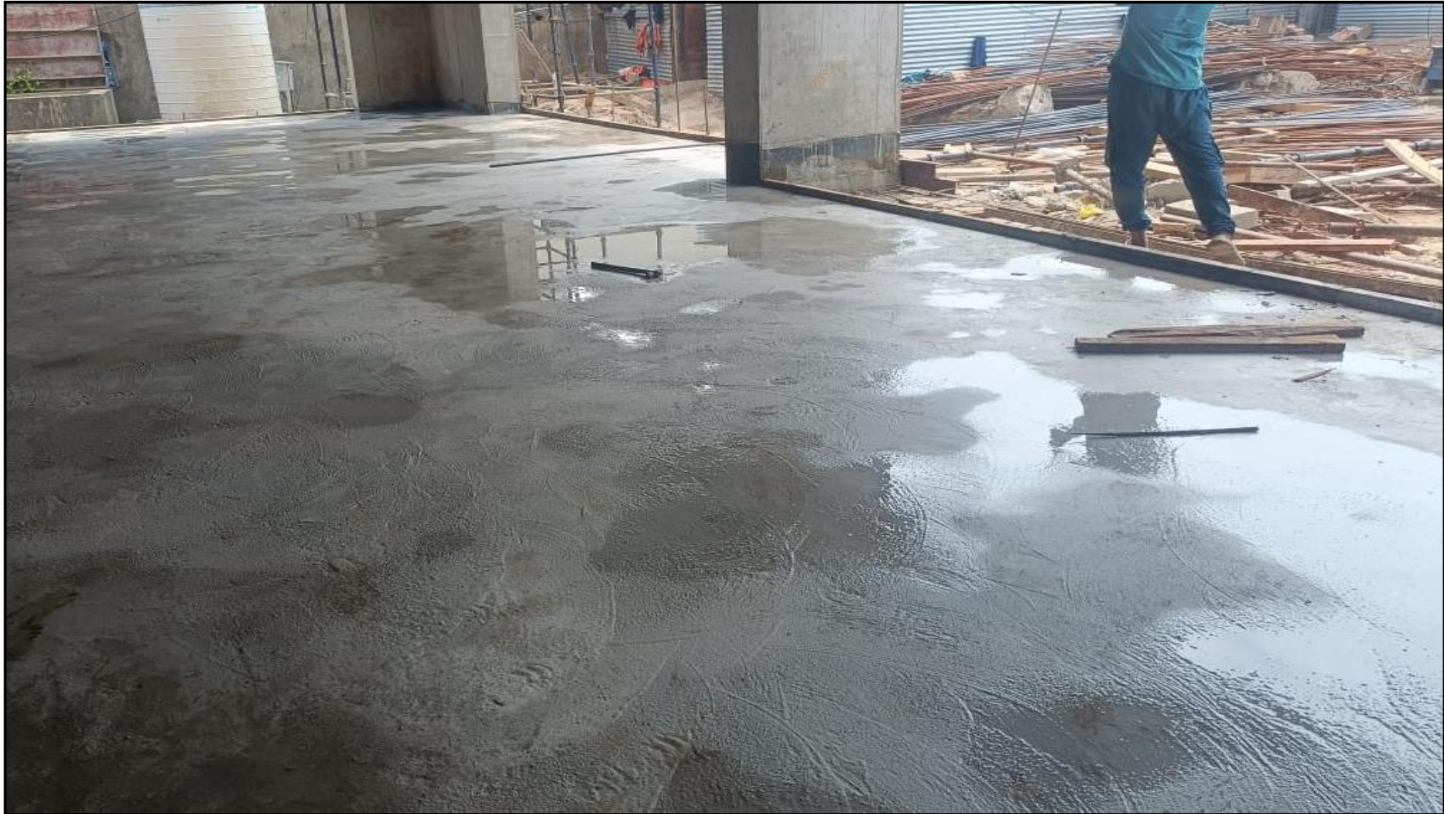
Stilt floor – Grade slab concrete work Completed
