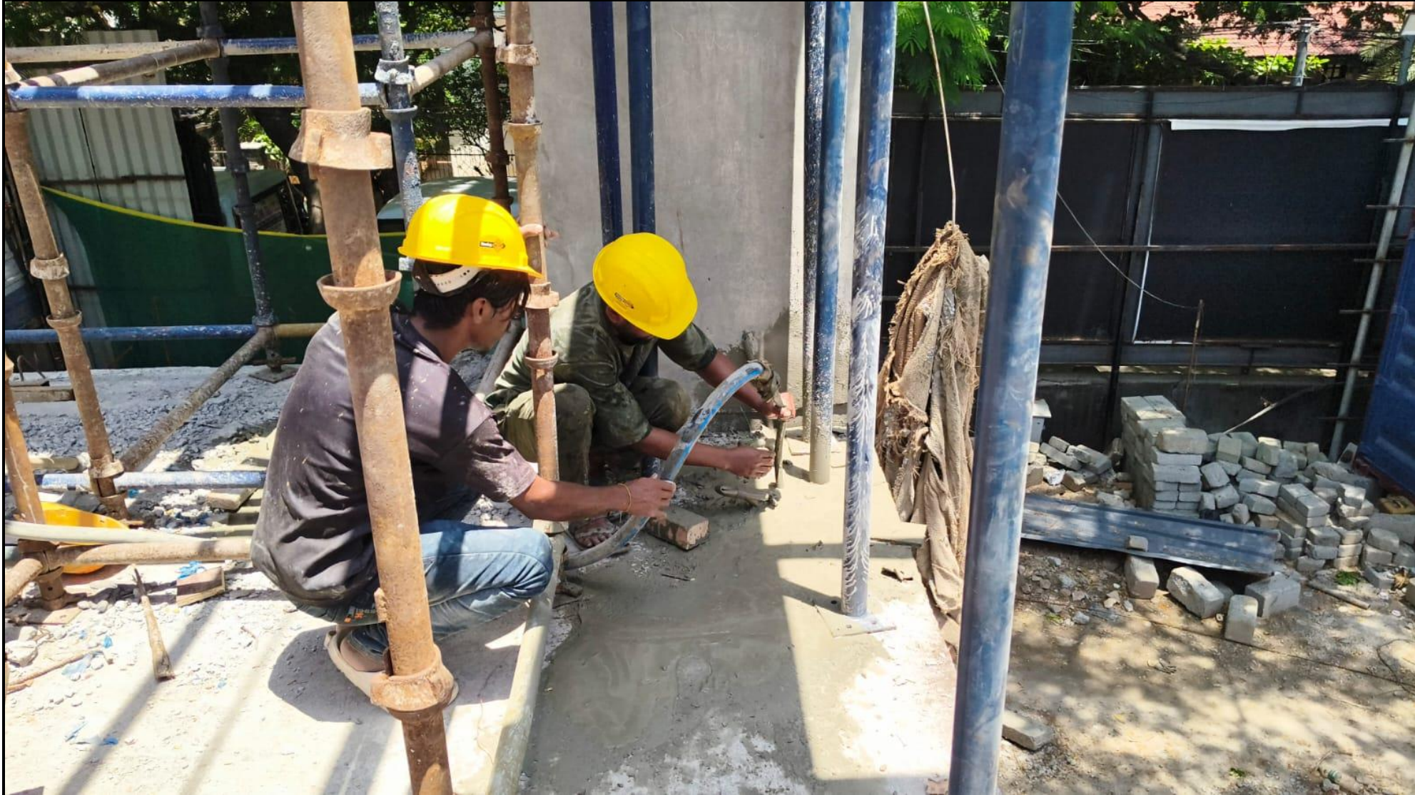
Stilt floor roof slab pour-02 PT grouting work completed (74/74nos) – 100% Completed
