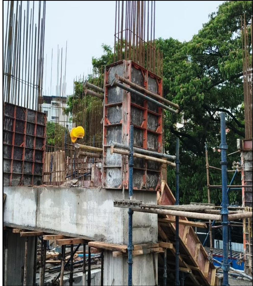
First floor pour-02 staircase 1st flight slab concrete work completed
