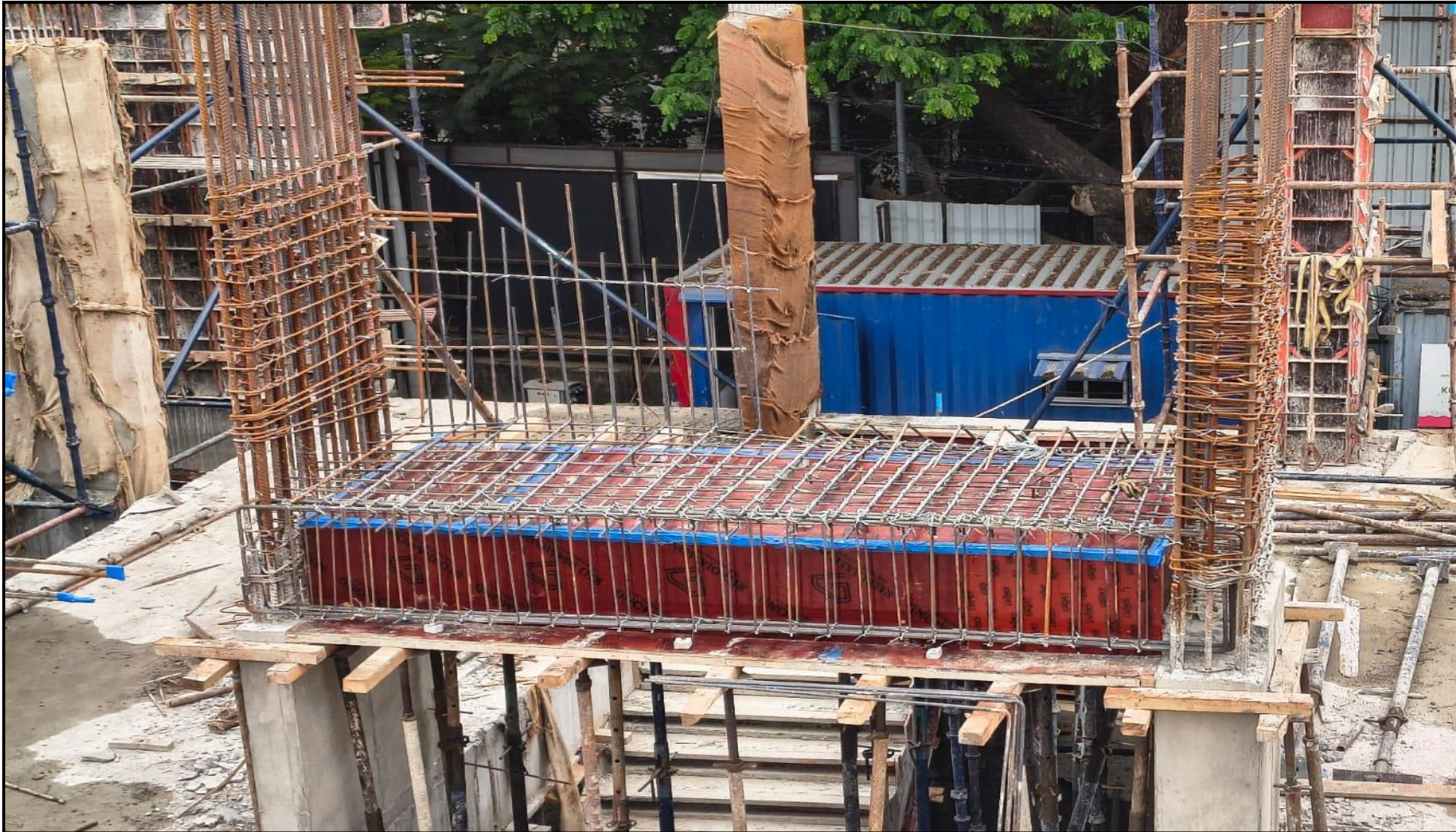
First Floor – Pour 2 Staircase 1 st Flight – Shuttering & Reinforcement works Completed
