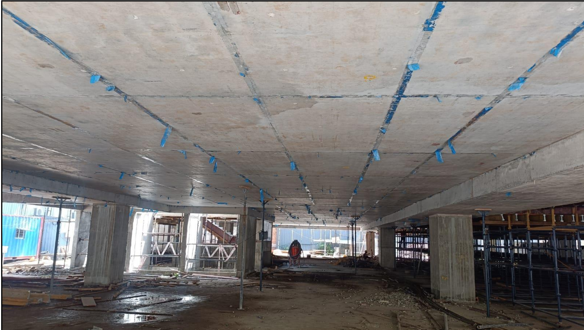
Stilt floor pour-02 slab de-shuttering work in progress (2040/2478Sqm) – 82.32%completed
