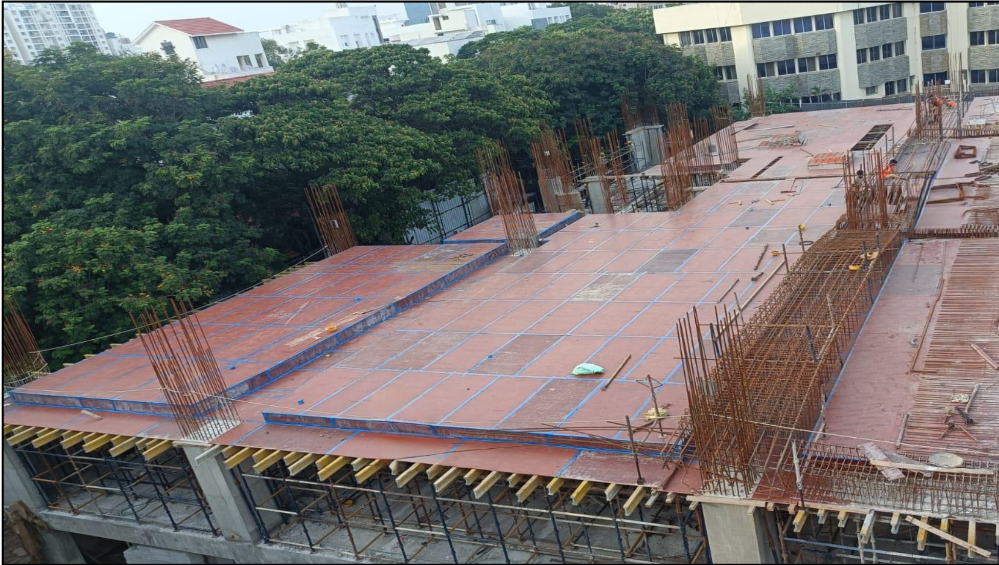
First floor pour-02 roof slab shuttering work in progress (920/998Sqm) – 95%completed
