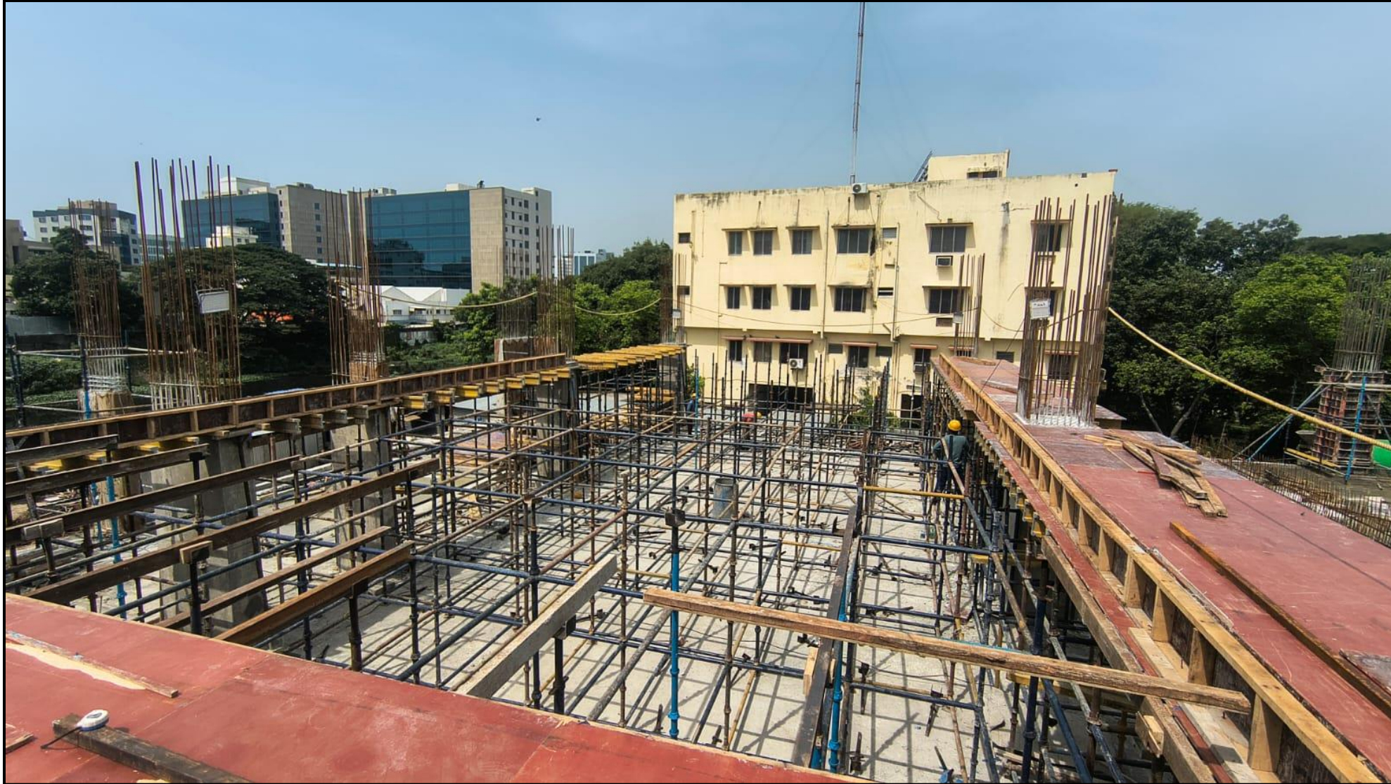
First Floor Roof Slab Pour-1 Roof Slab – Staging Work Completed
