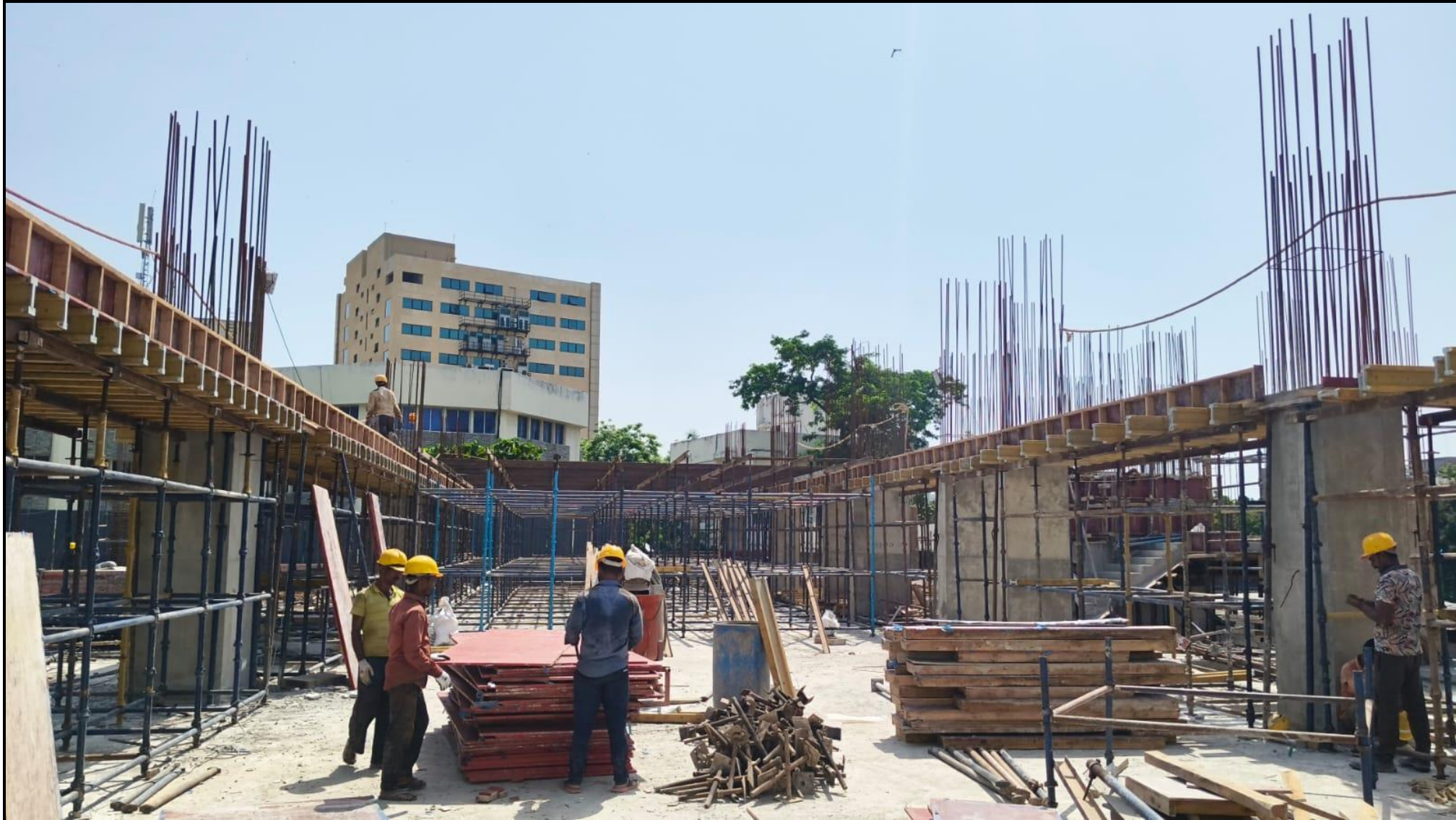
First floor pour:01 – roof slab shuttering work in progress (300/1475Sqm) – 20% completed
