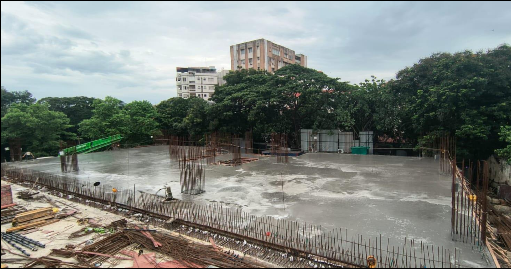
Stilt floor pour:02 - Roof slab concrete work completed(329/329Cum) - 100%completed
