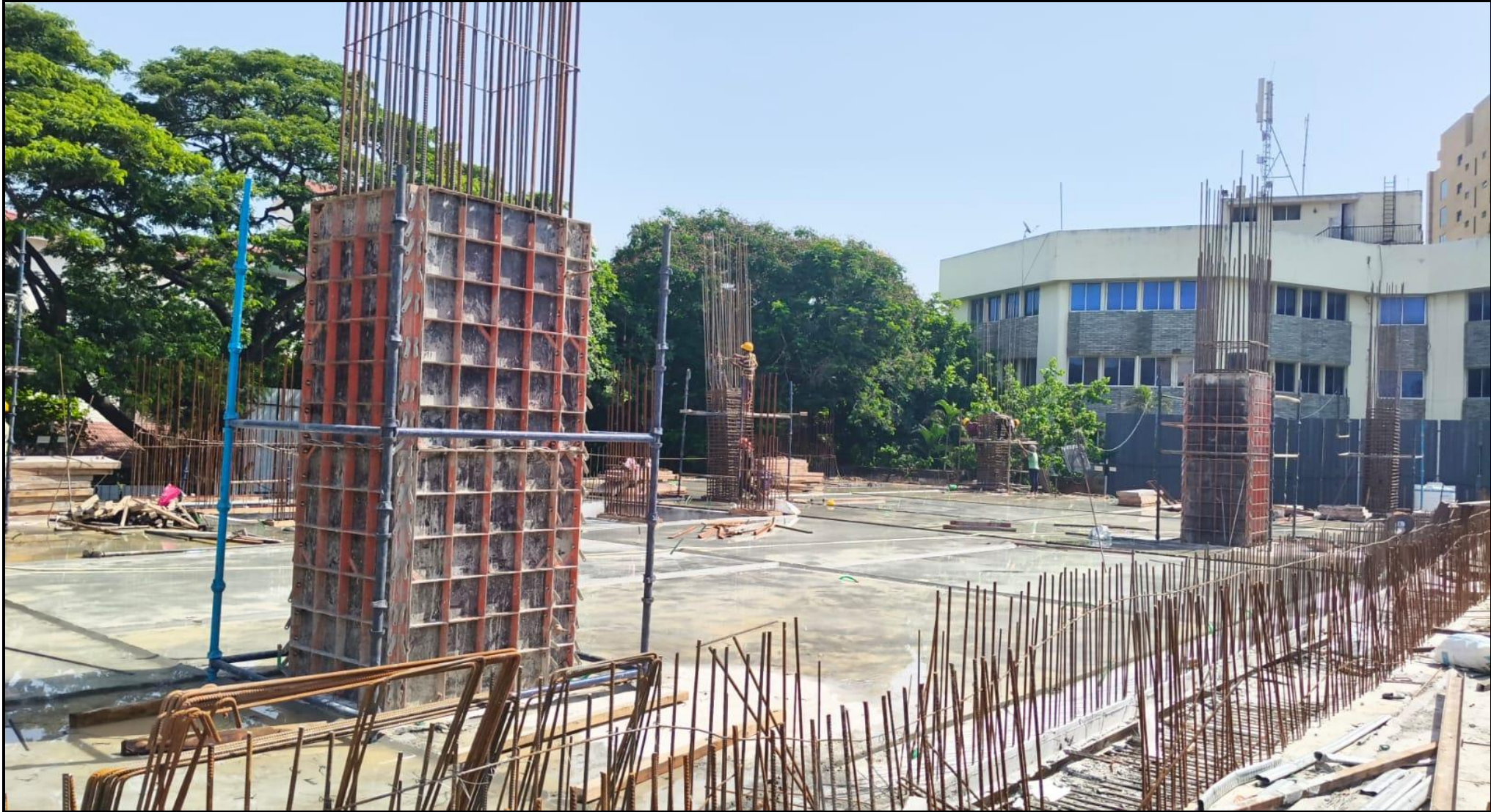
First floor pour:01– columns shuttering work in progress (6/20 Nos)
