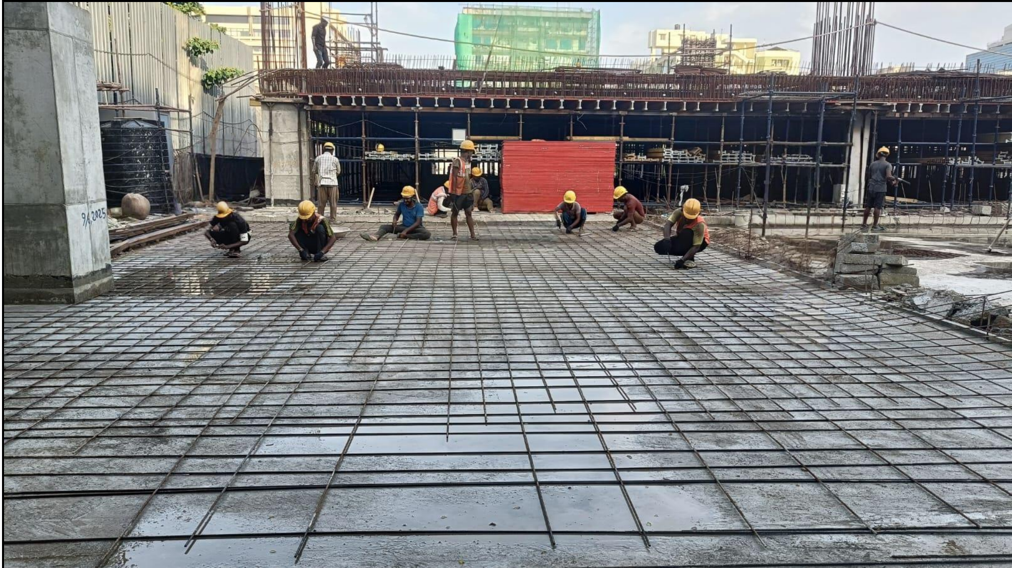
Stilt floor pour-02: Grade slab reinforcement work completed (17/17MT)
