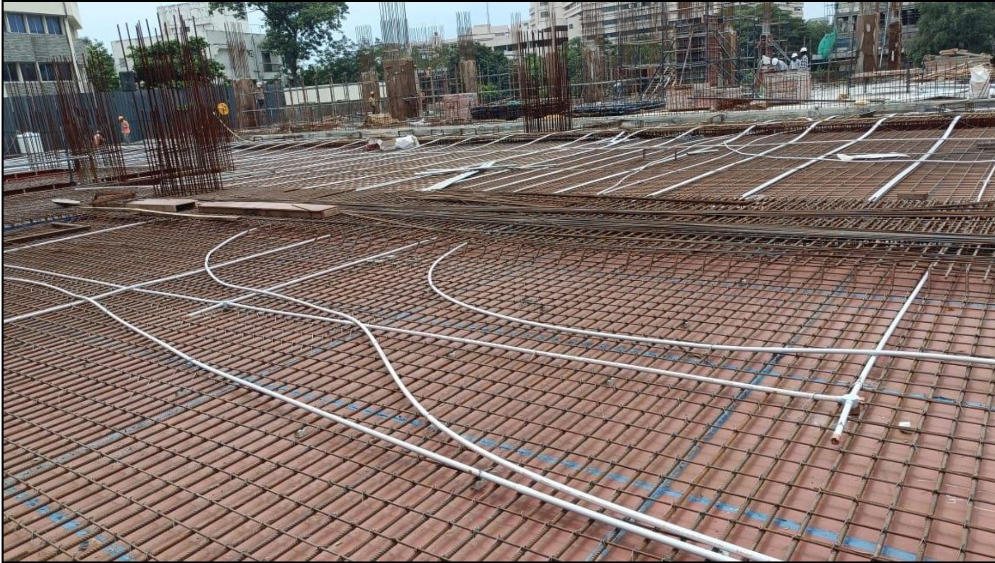
Stilt floor pour:02 - Roof slab electrical conduit laying work completed (462/462Rmt)
