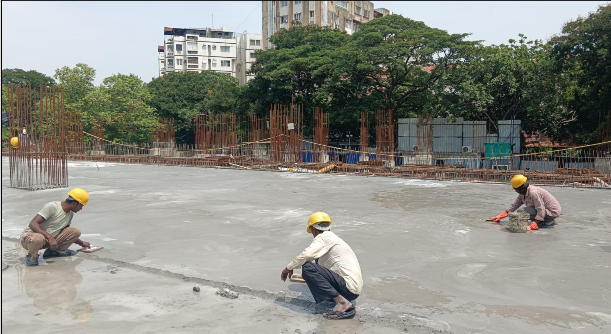
Stilt floor roof slab Pour 1: Concrete – Float Finish work – 100% Completed
