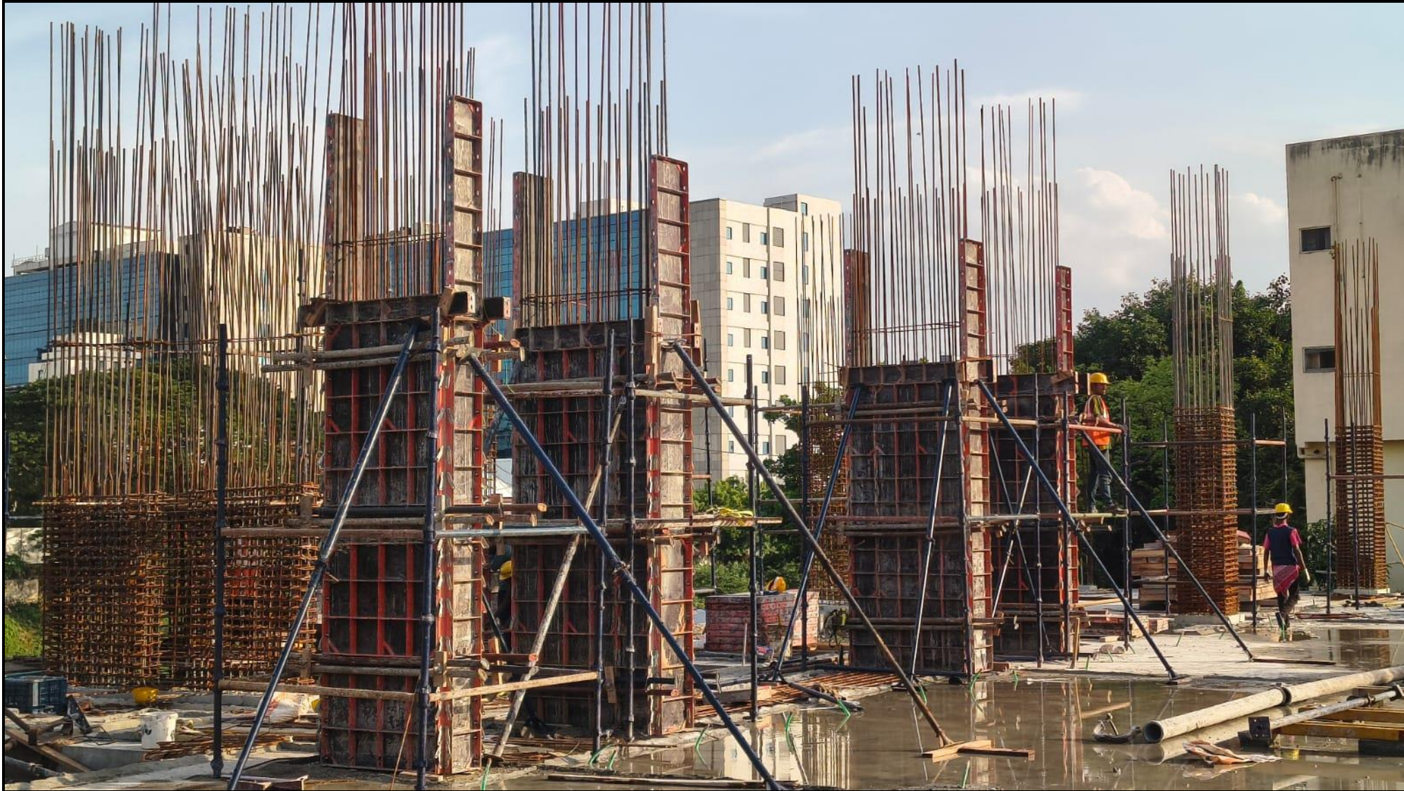
First floor pour:01 - Column shuttering work completed (22/22 Nos) - 100%completed
