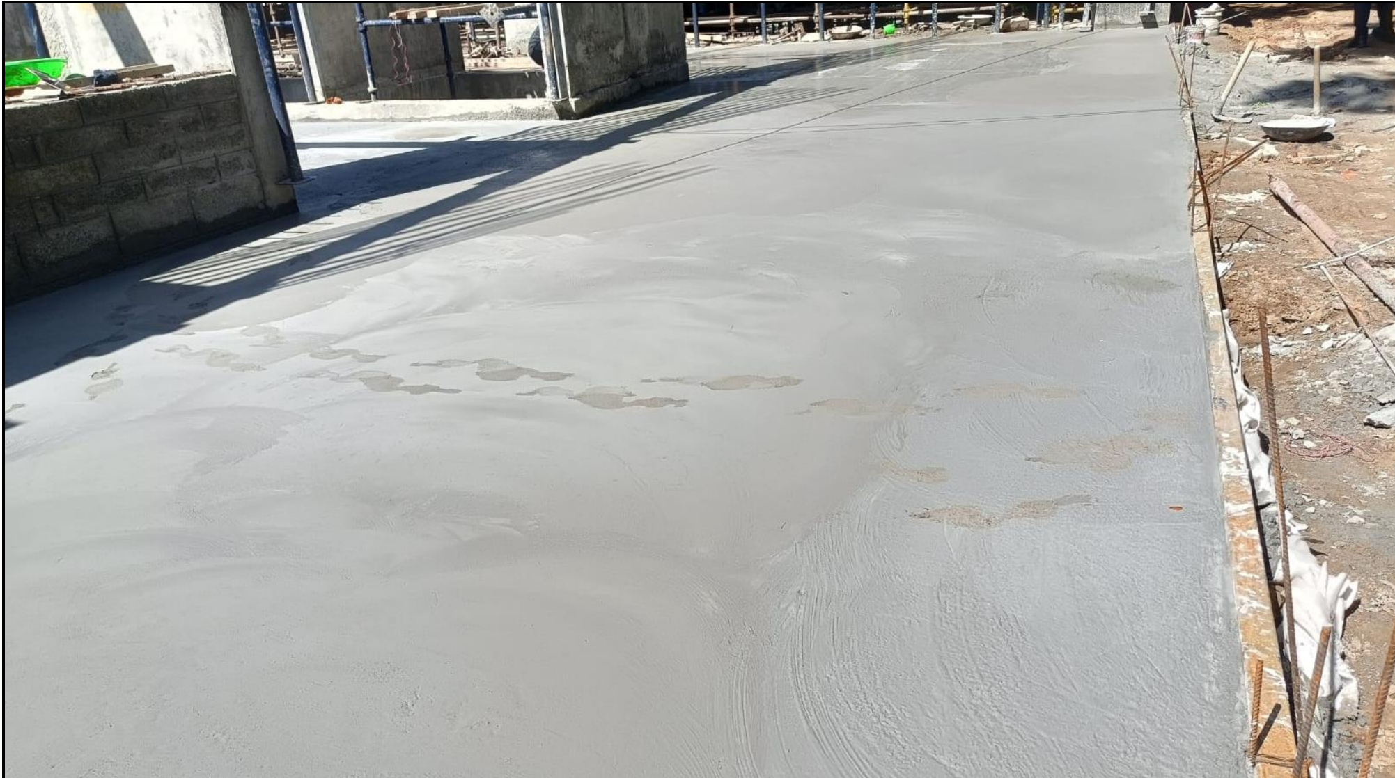
Stilt floor pour-02: Grade slab concrete work in progress (68/68 Cum) – 100%completed
