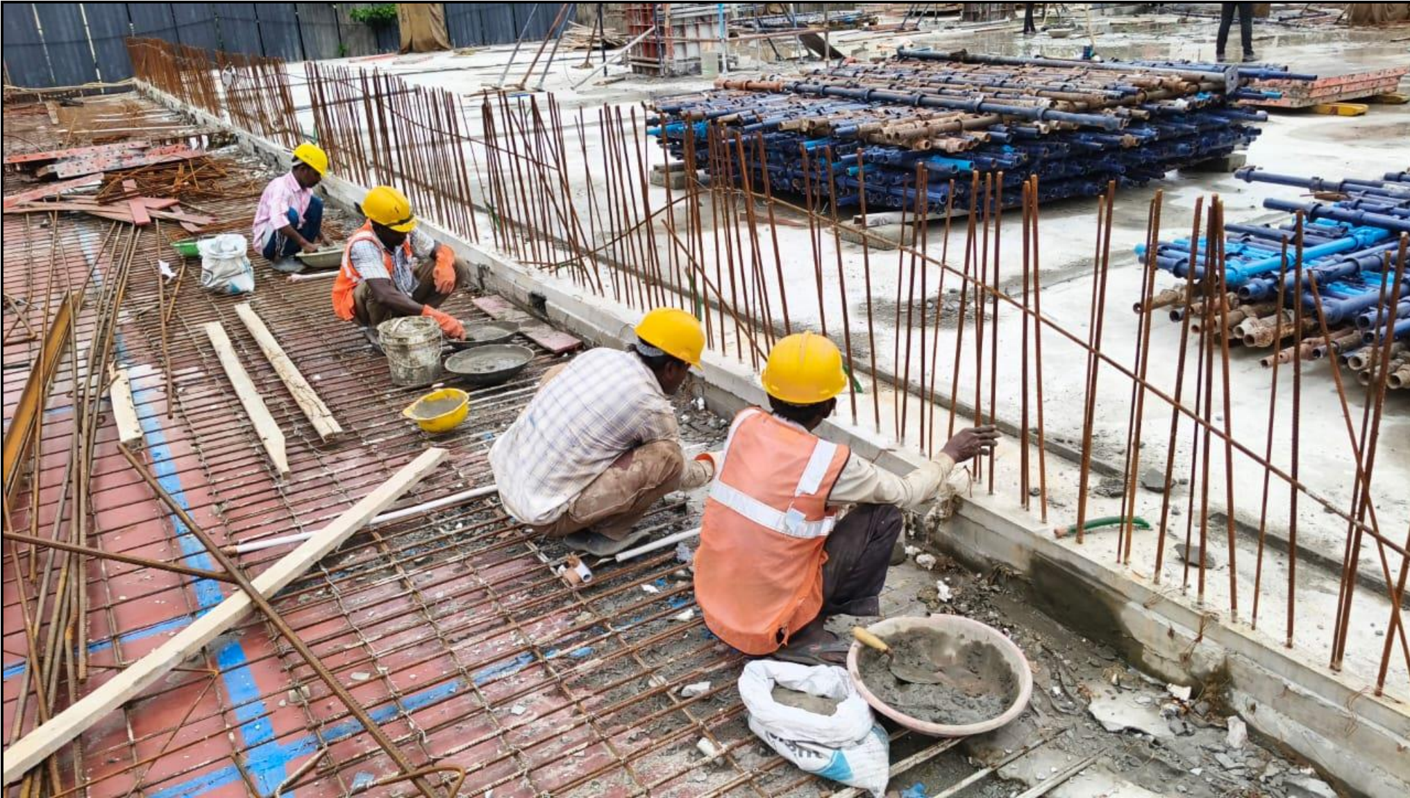
Stilt floor pour:01 - Roof PT slab & beam stressing end packing work completed (64/64 Nos)
