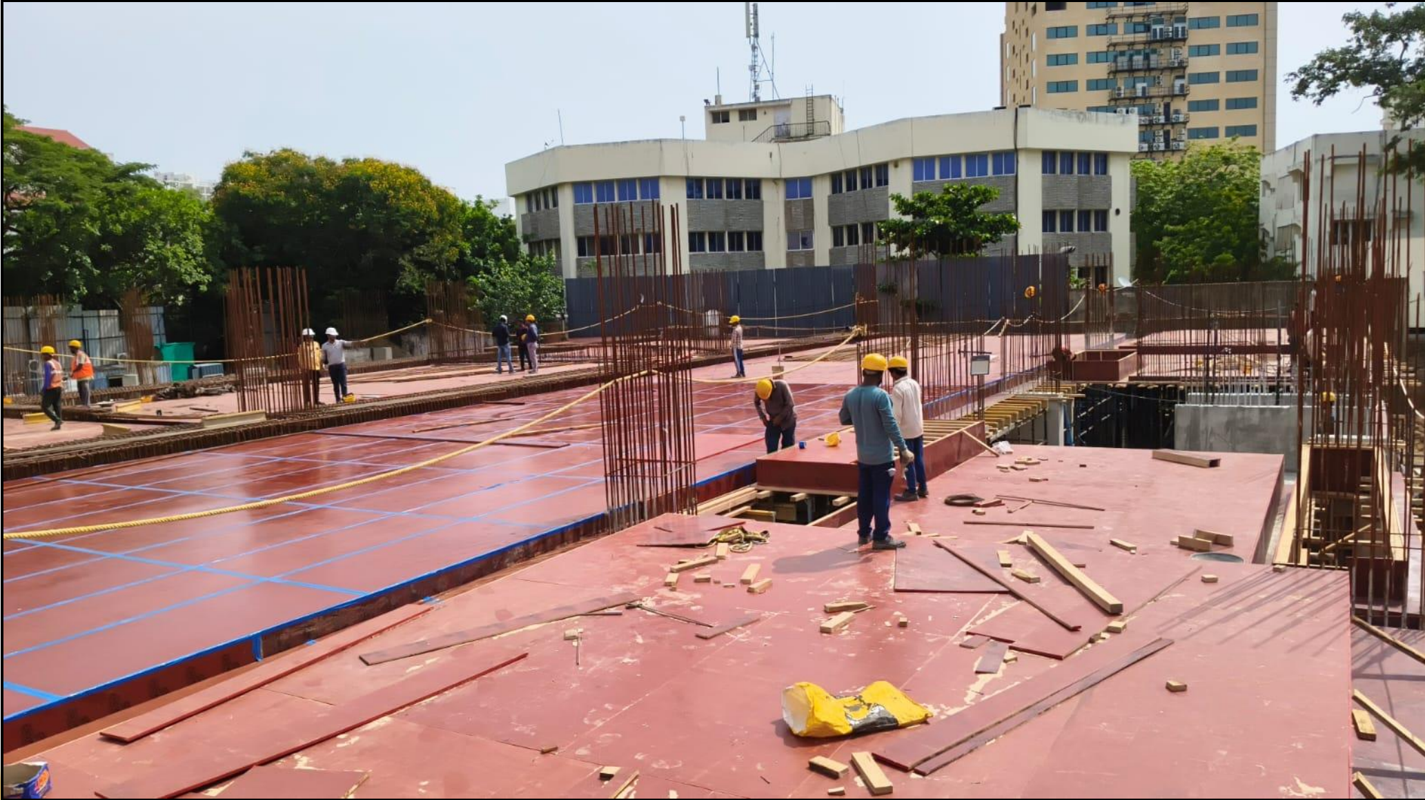
Stilt floor Pour 1 roof slab shuttering work completed (1475/1475 Sqm) – 100% completed
