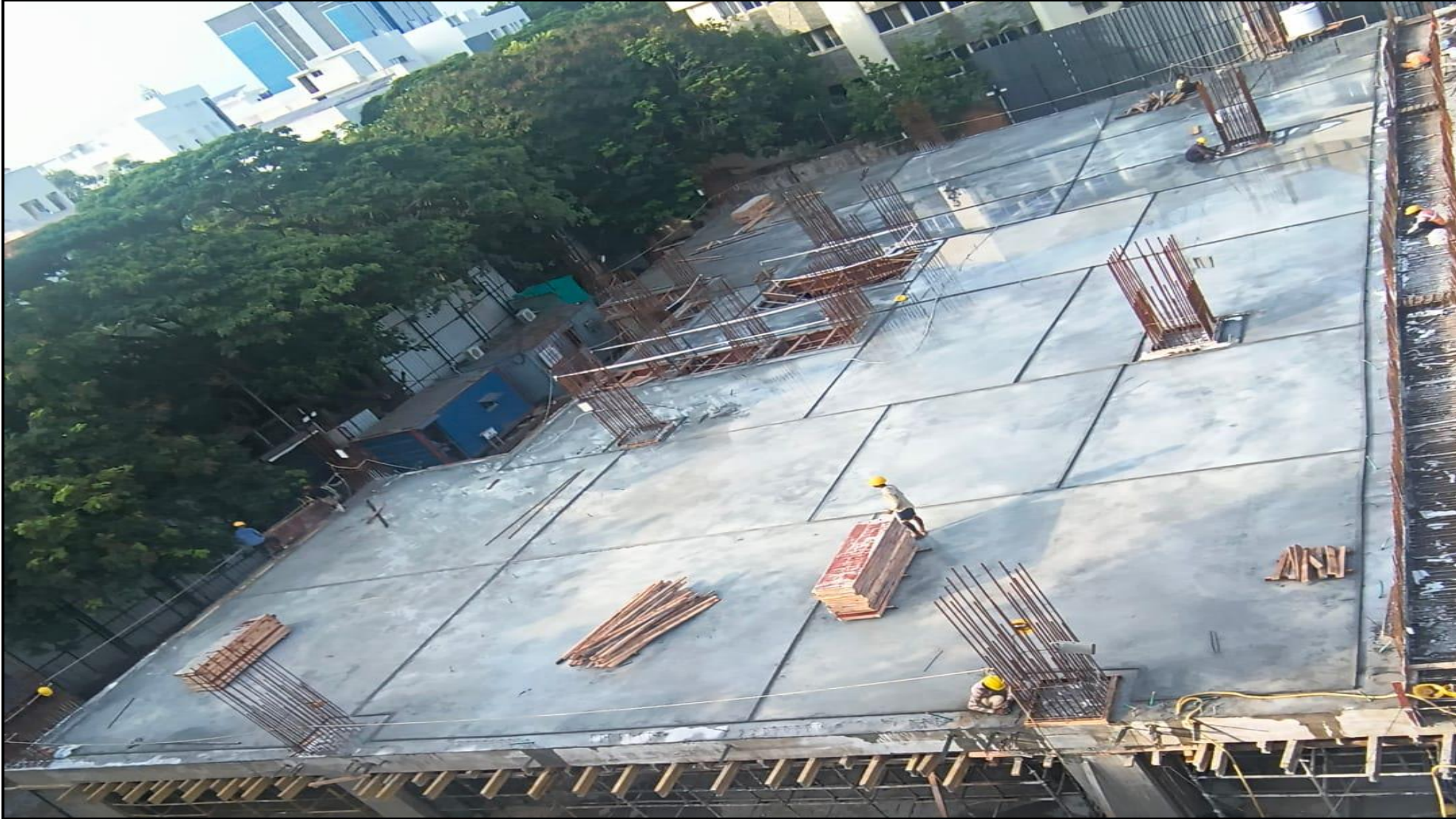
Stilt floor pour:02 - Roof slab curing and bonding work in progress
