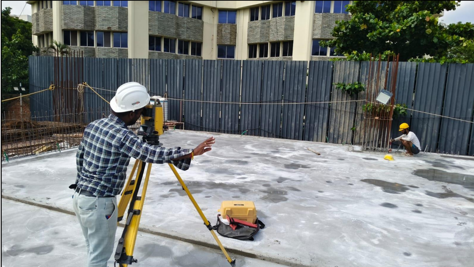
First floor Pour 1 Columns marking work. – 100% completed
