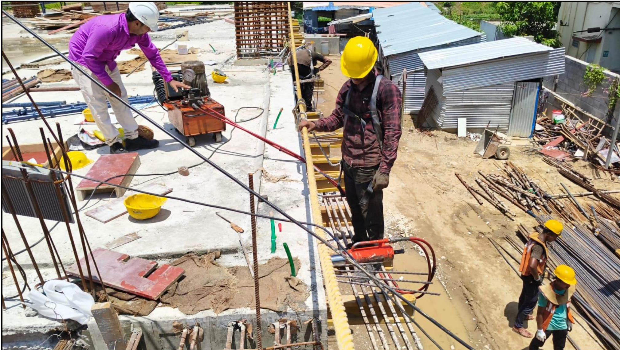
Stilt floor roof slab pour:01 - PT slab & beam strand stressing work completed (64/64 Nos)
