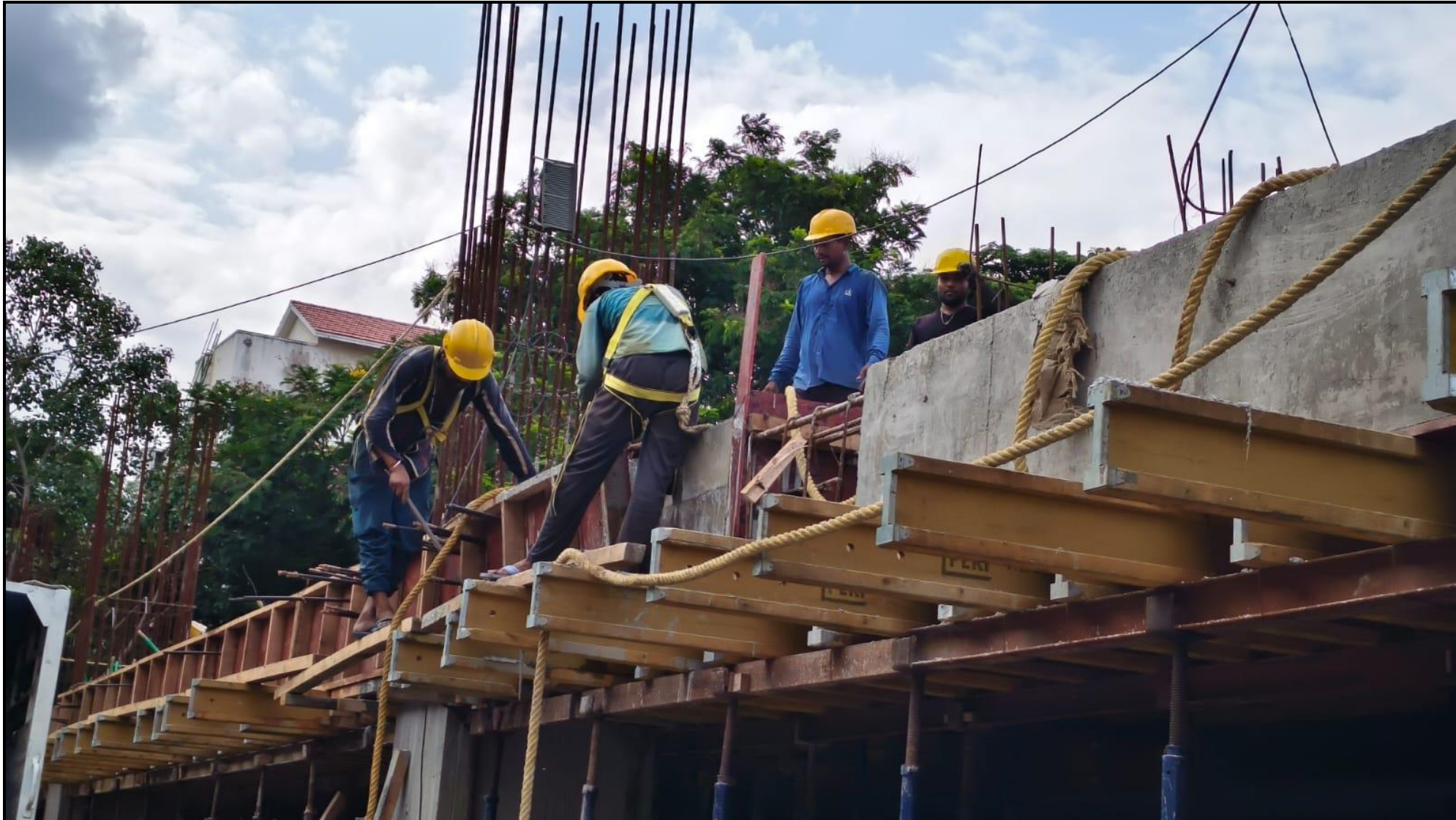
Stilt floor pour:02 - Roof slab outer beam de-shuttering work Completed – 100%completed
