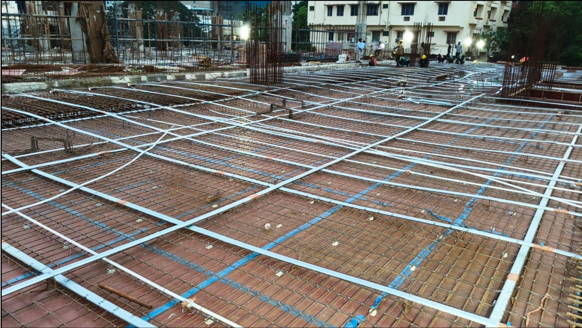
Stilt floor pour:02 - Roof slab PT work completed (4.5/4.5MT) - 100%completed
