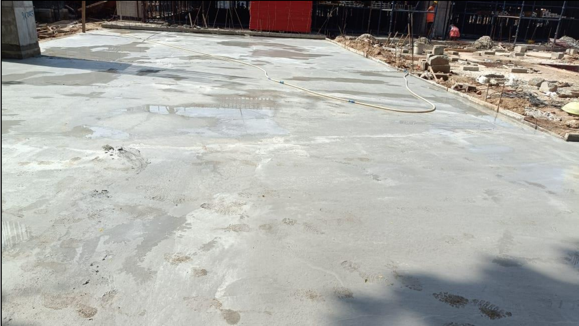
Stilt floor pour-02 : Grade slab PCC work is completed (132/132 Cum)
