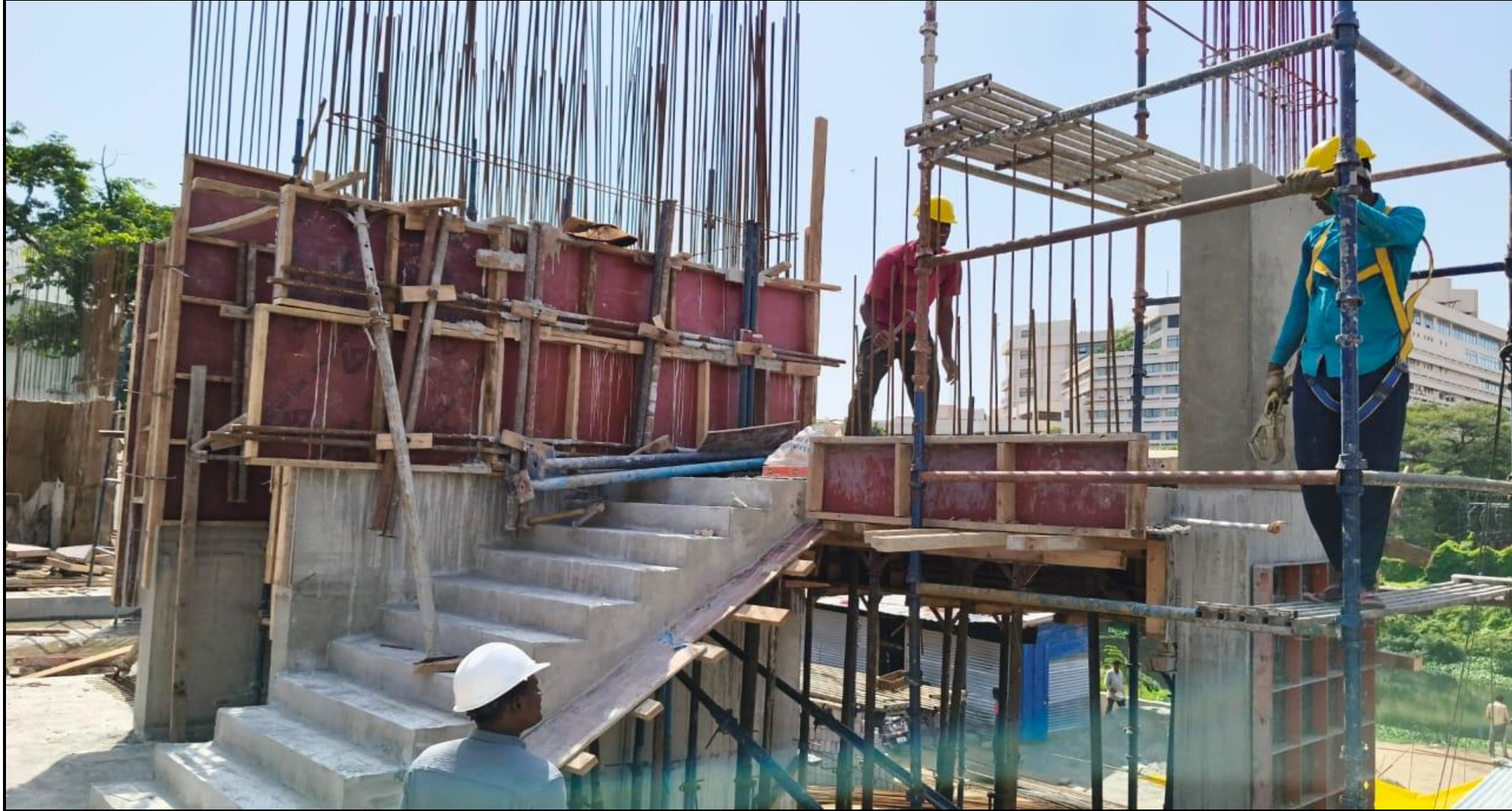
First floor pour:01 – Staircase first flight & column concrete work completed
