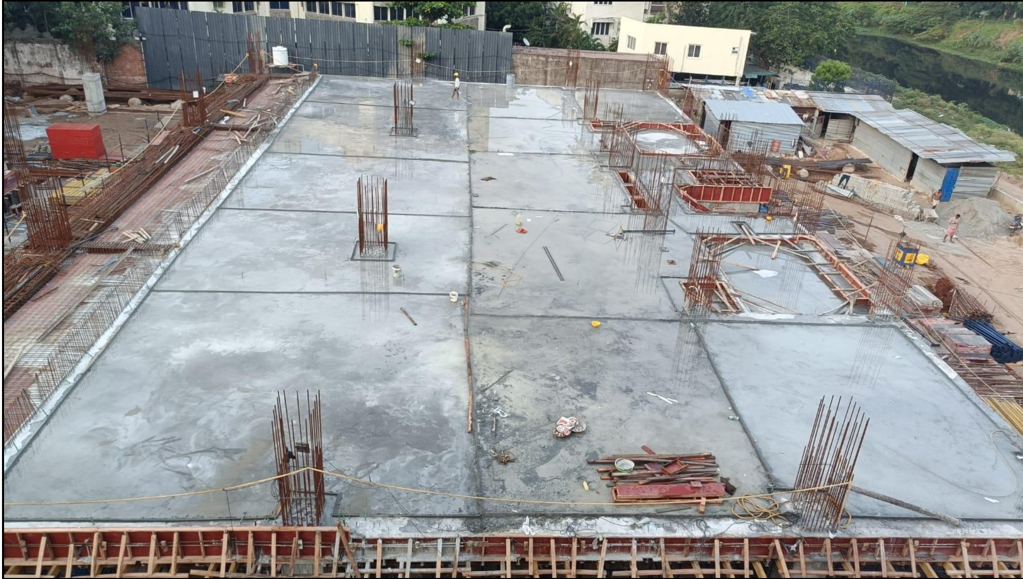
Stilt floor roof slab Pour 1: Concrete work completed ( 365.3/365.3 Cum) – 100% completed
