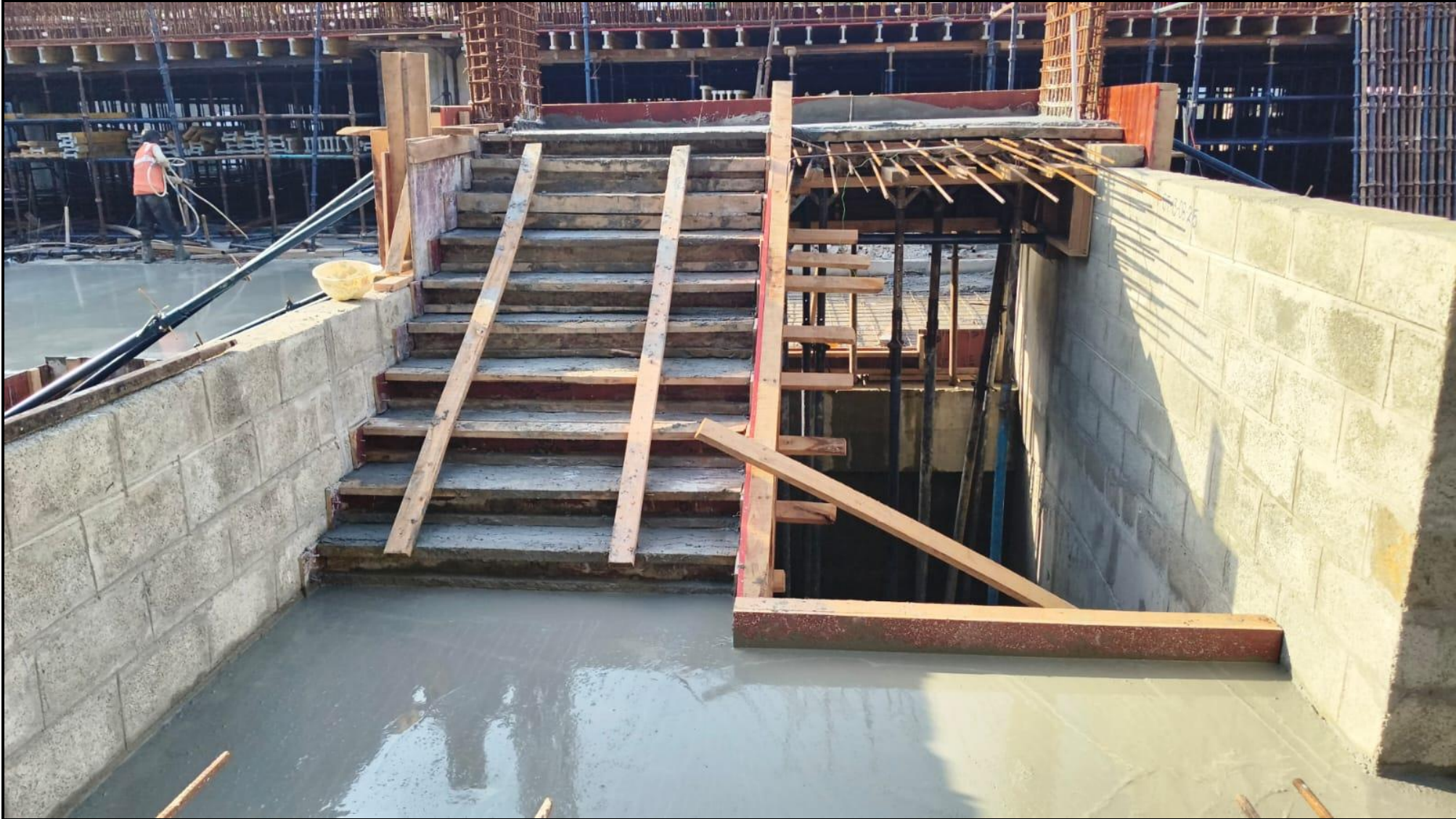
Stilt floor Pour-2: Staircase concrete work completed
