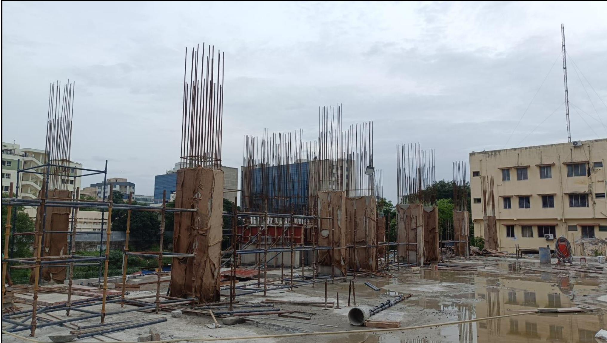
First floor pour-01: Column concrete work completed (22/22 Nos) - 100% completed
