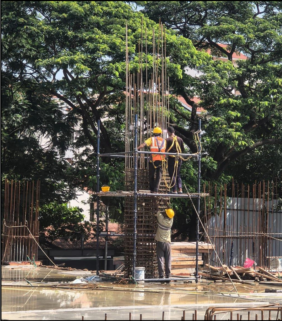
First floor pour:02– column reinforcement work in Progress (8/20nos)
