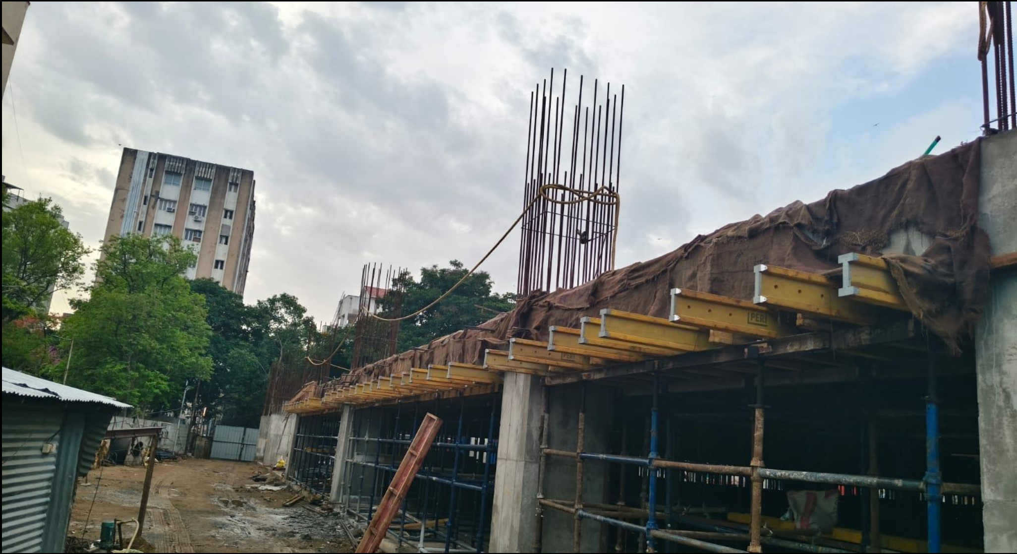
Stilt floor Pour 1 roof beam external side deshuttering work completed (86.25/86.25 Sqm)
