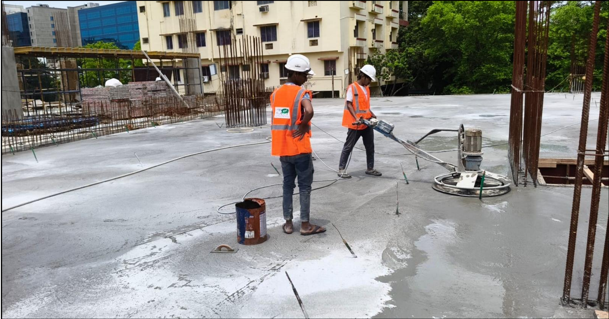
Stilt floor pour:02 - Roof slab concrete float finishing work completed
