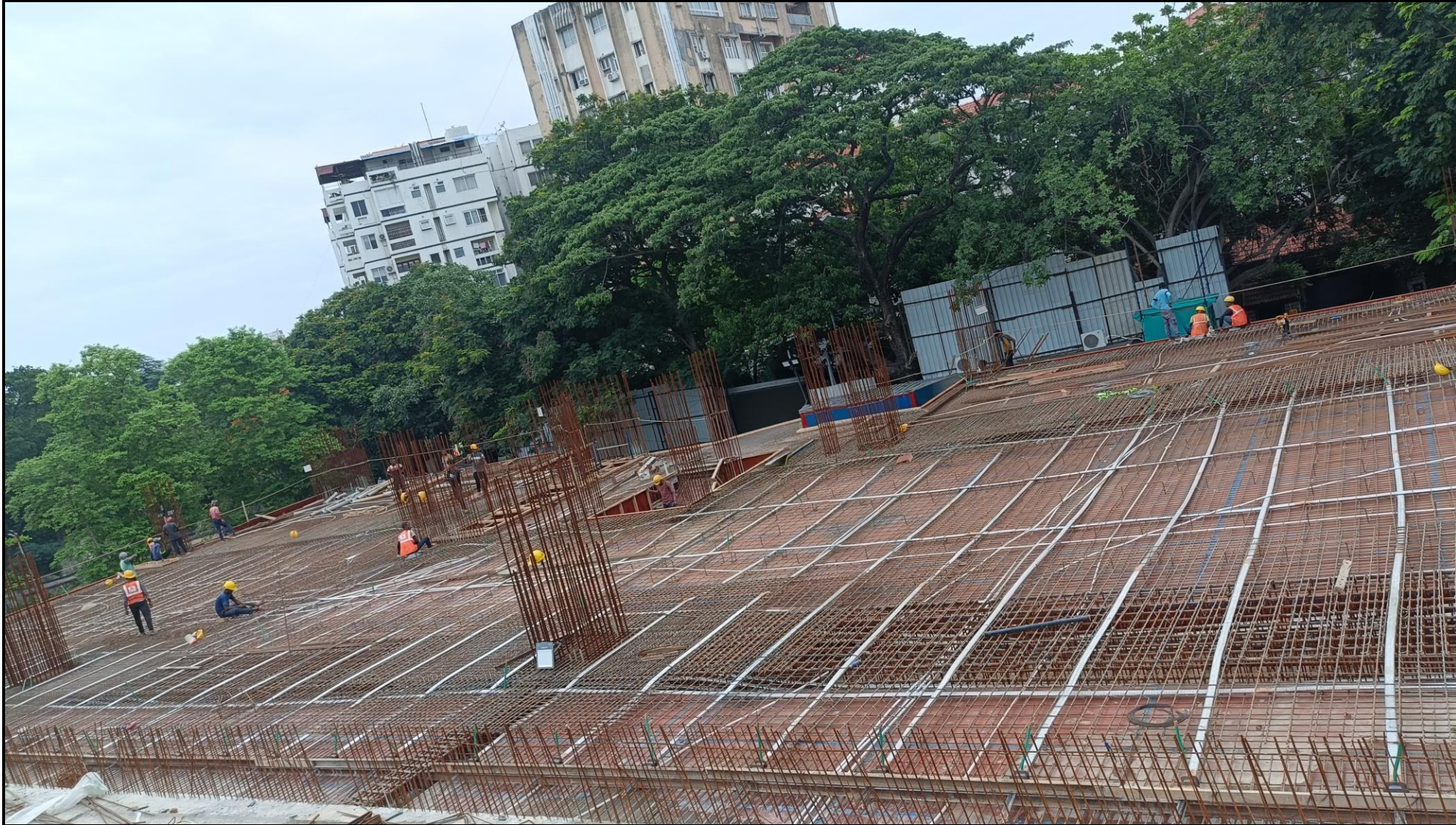
Stilt floor pour:02 - Roof slab reinforcement work completed (38/38MT) – 100%completed
