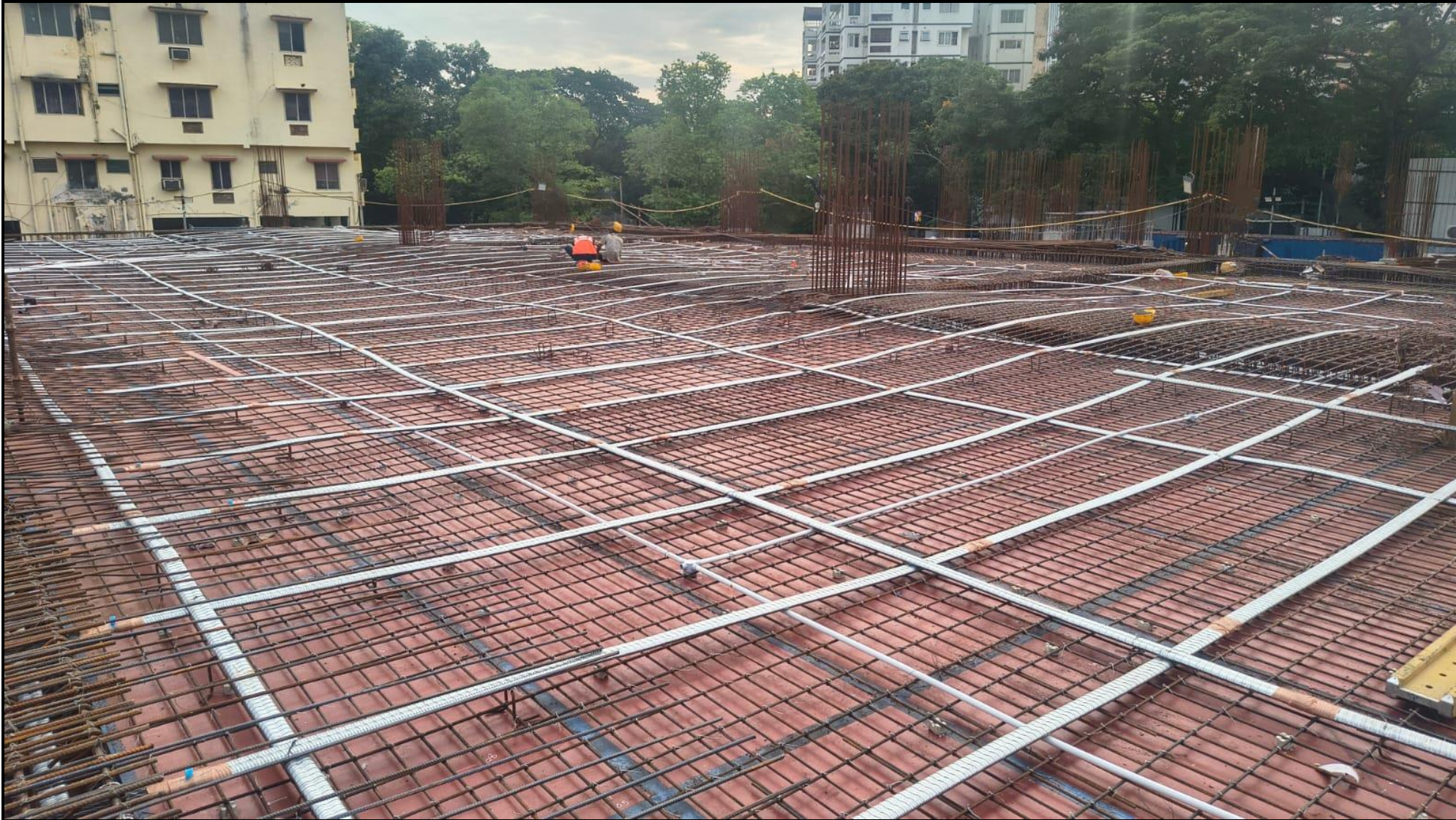
Stilt floor Pour 1 PT Strand placing work completed (05/05 MT) – 100% completed
