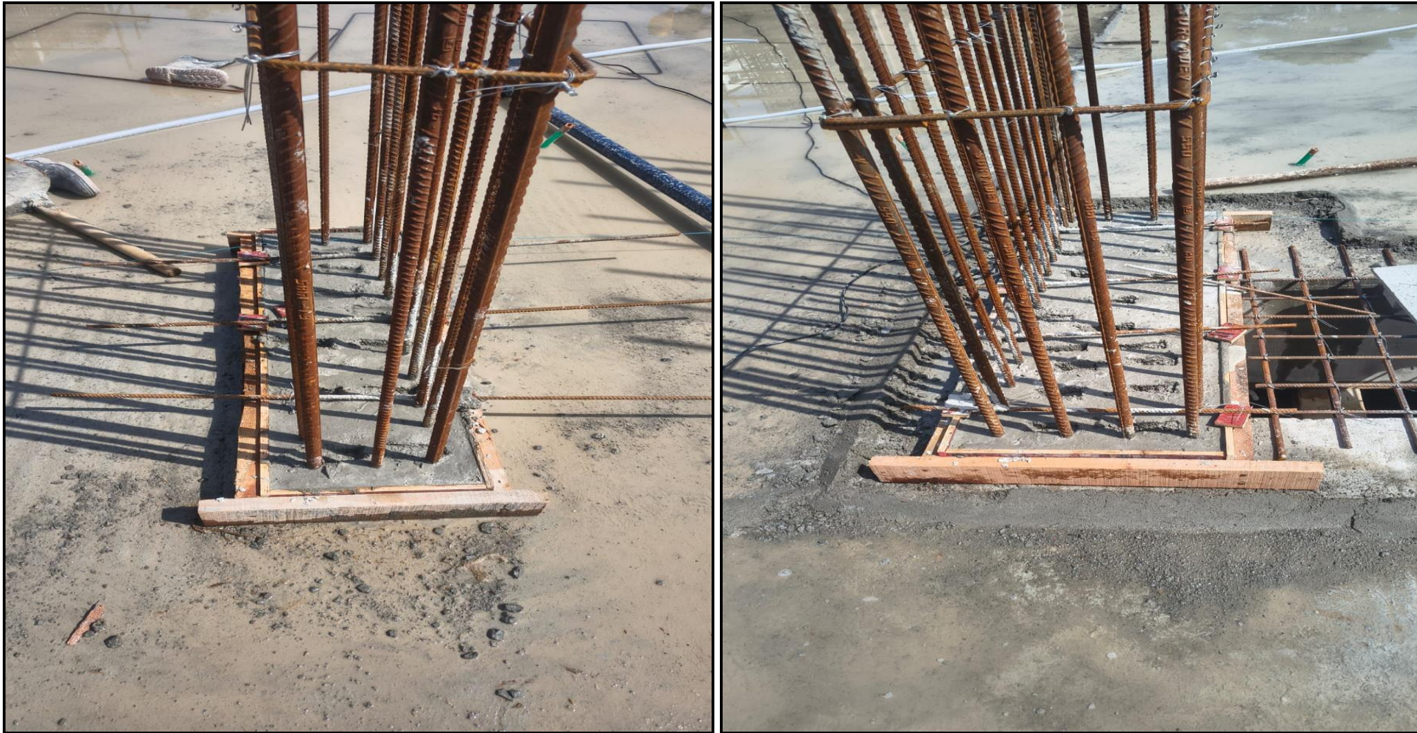
First floor pour-01: Columns starter marking & concrete work completed (22/22 Nos)
