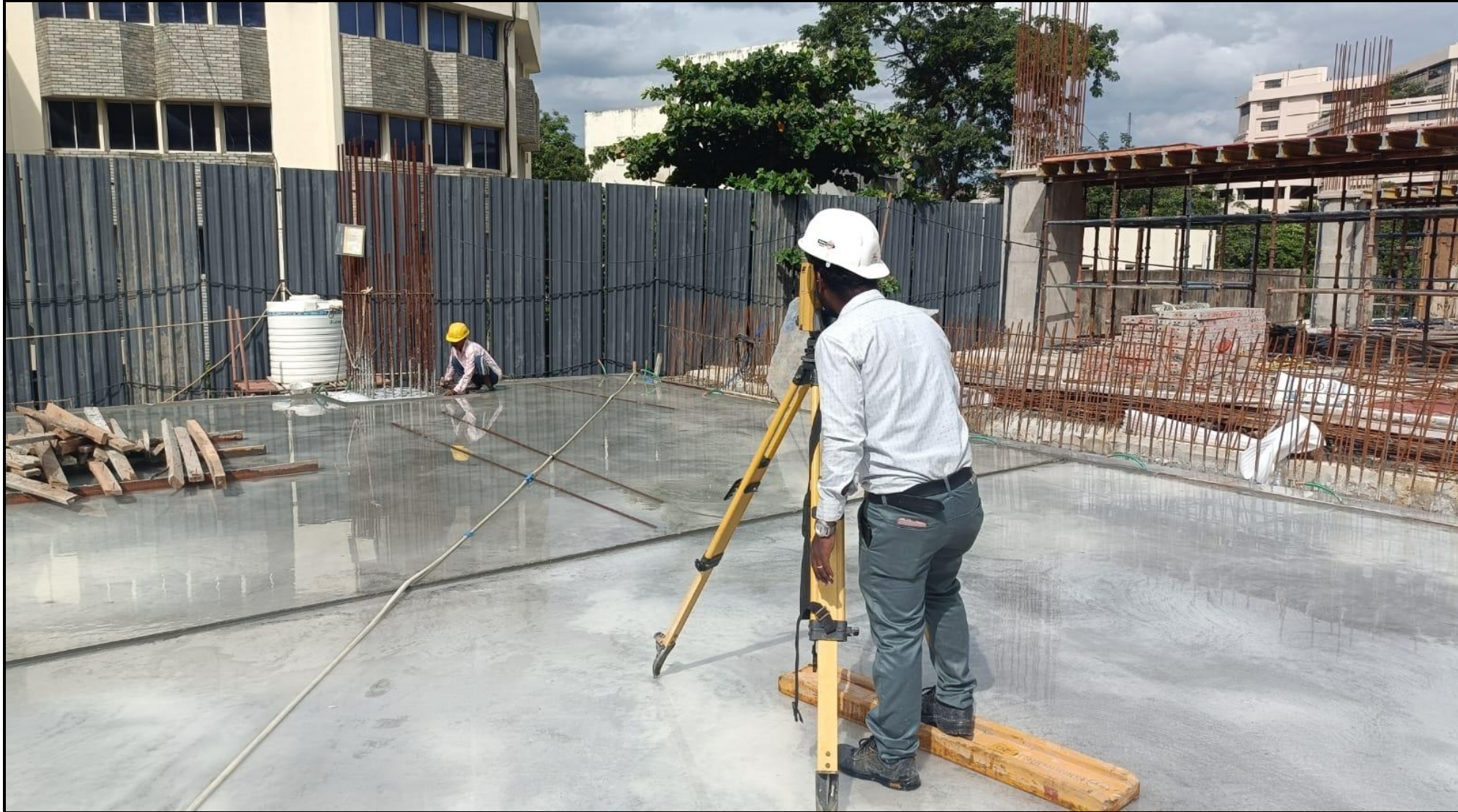
First floor pour:02– column marking work completed (20/20nos)
