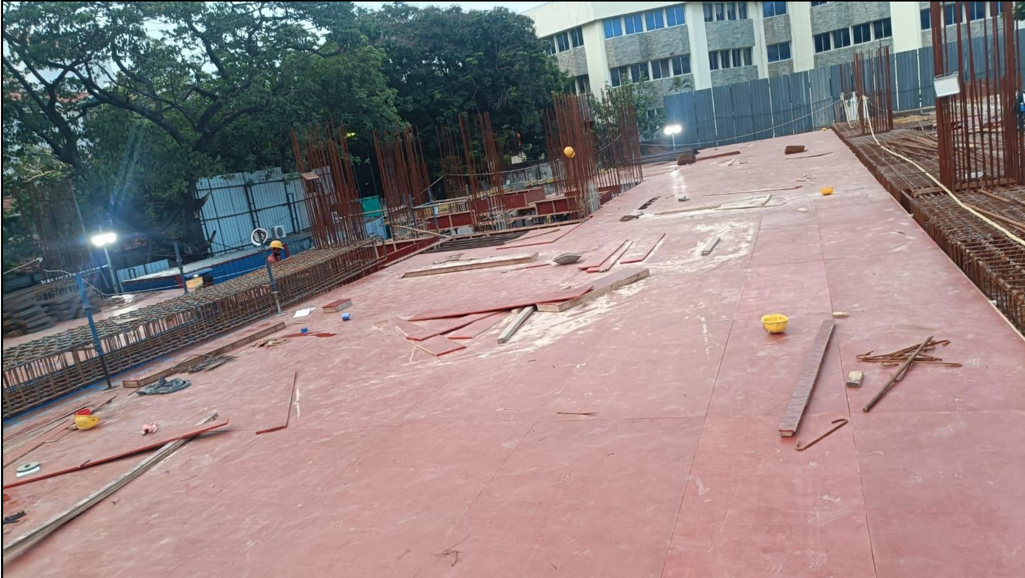
Stilt floor pour:02 - Roof slab shuttering work in progress (990/990 Sqm) - 100%completed
