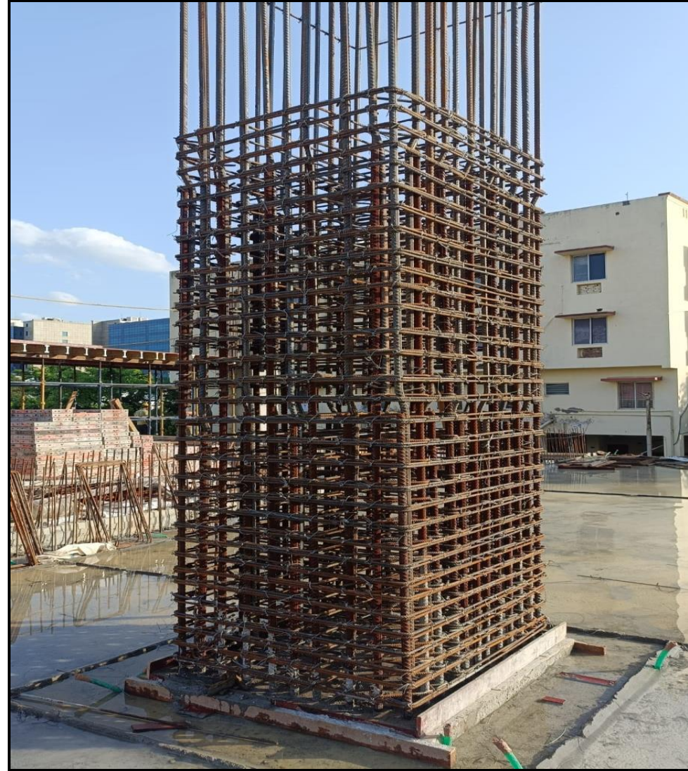
First floor pour:02– column reinforcement work in Progress (8/20nos)
