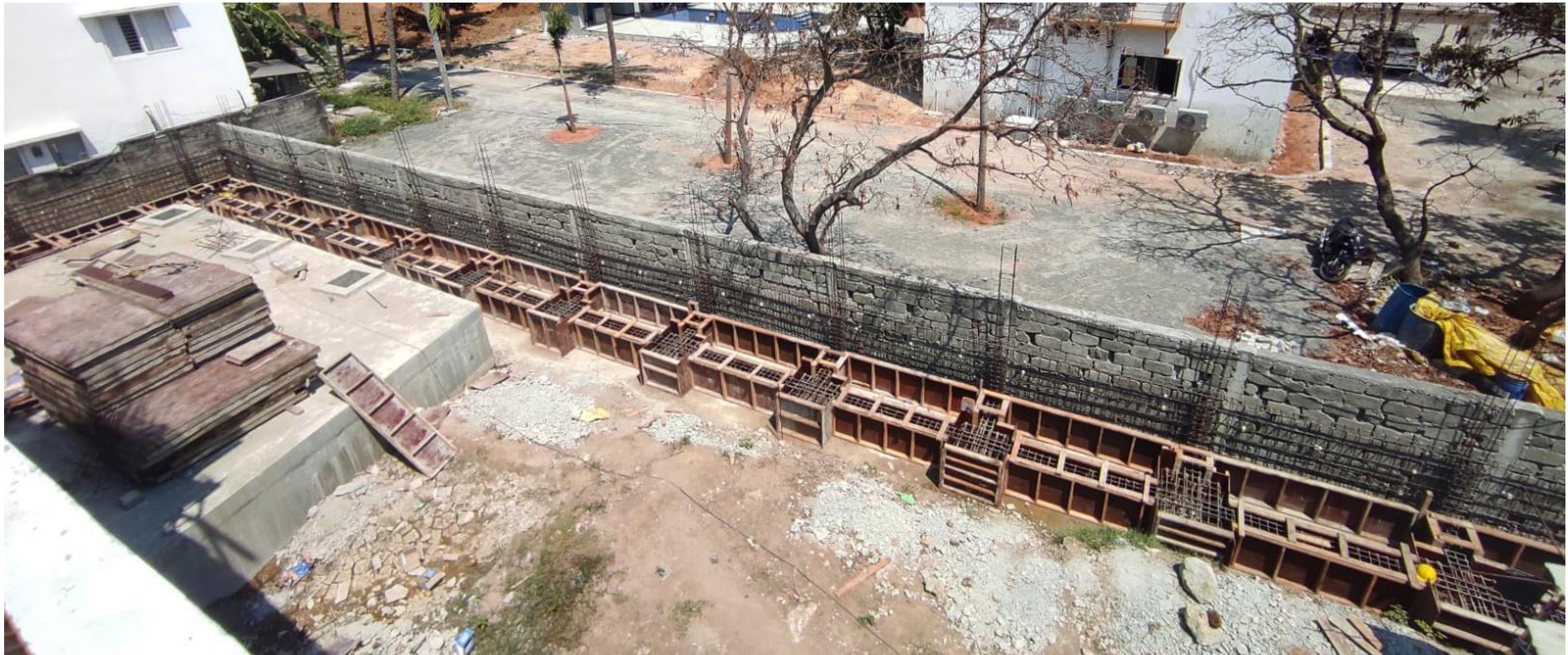
Eastside Compound Wall Shuttering Work In Progress
