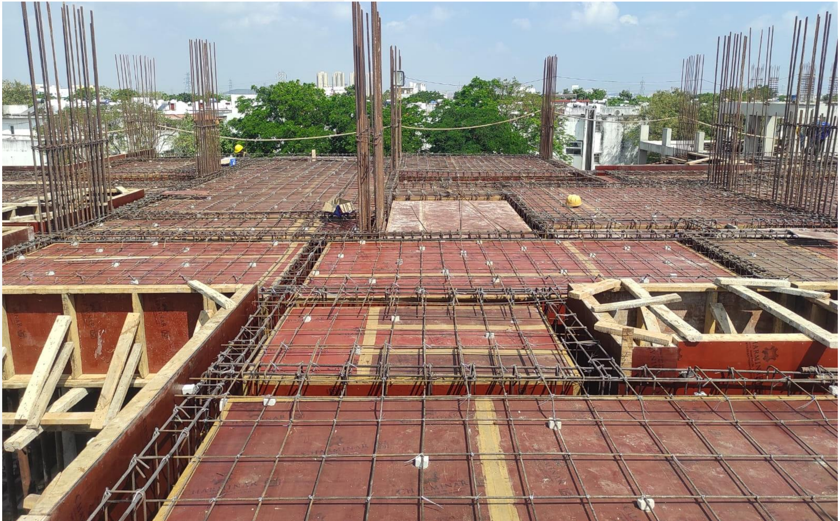
Main Building – Second Floor Slab Reinforcement Work in Progress
