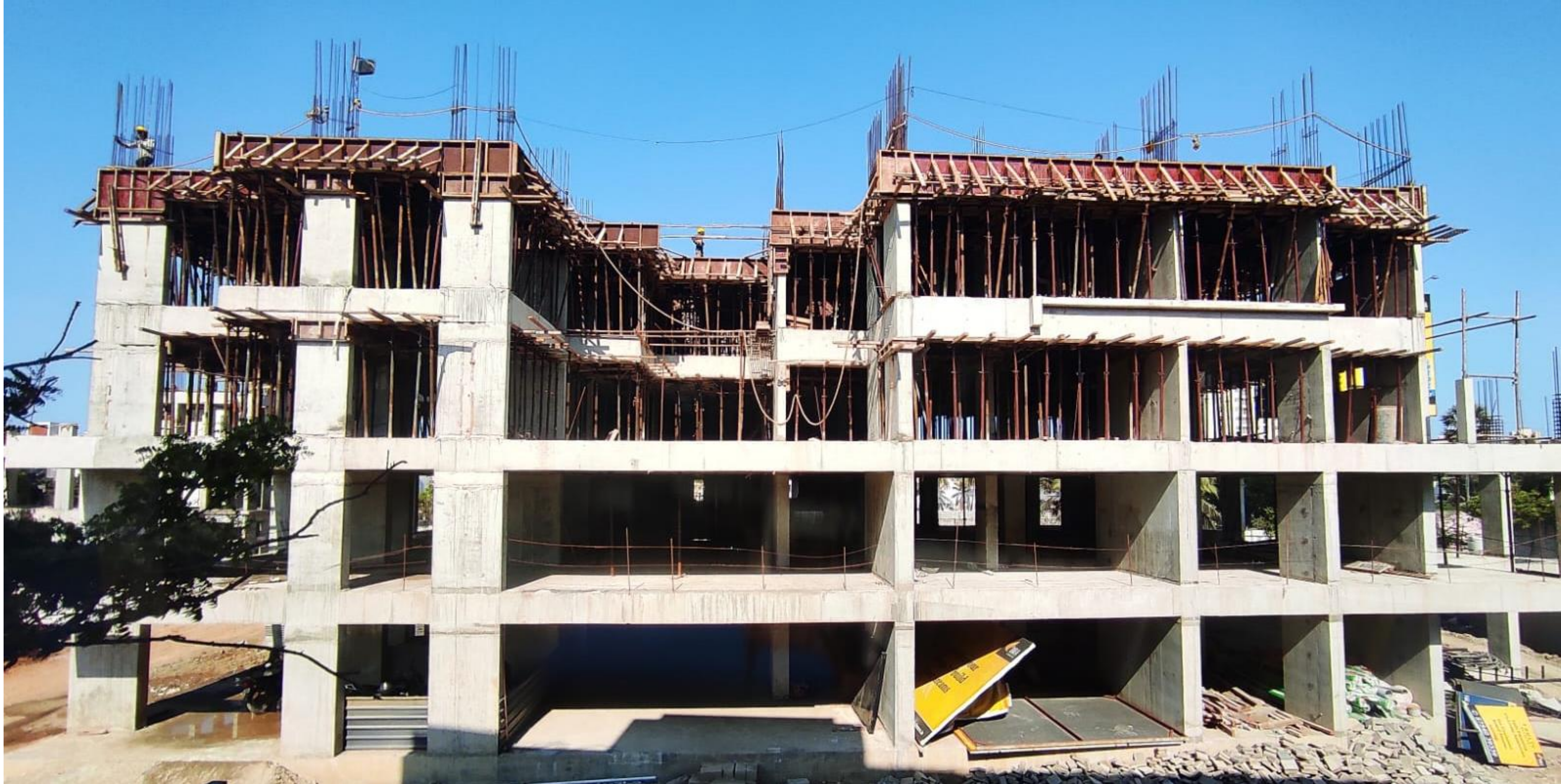
Main Building - West Side View
