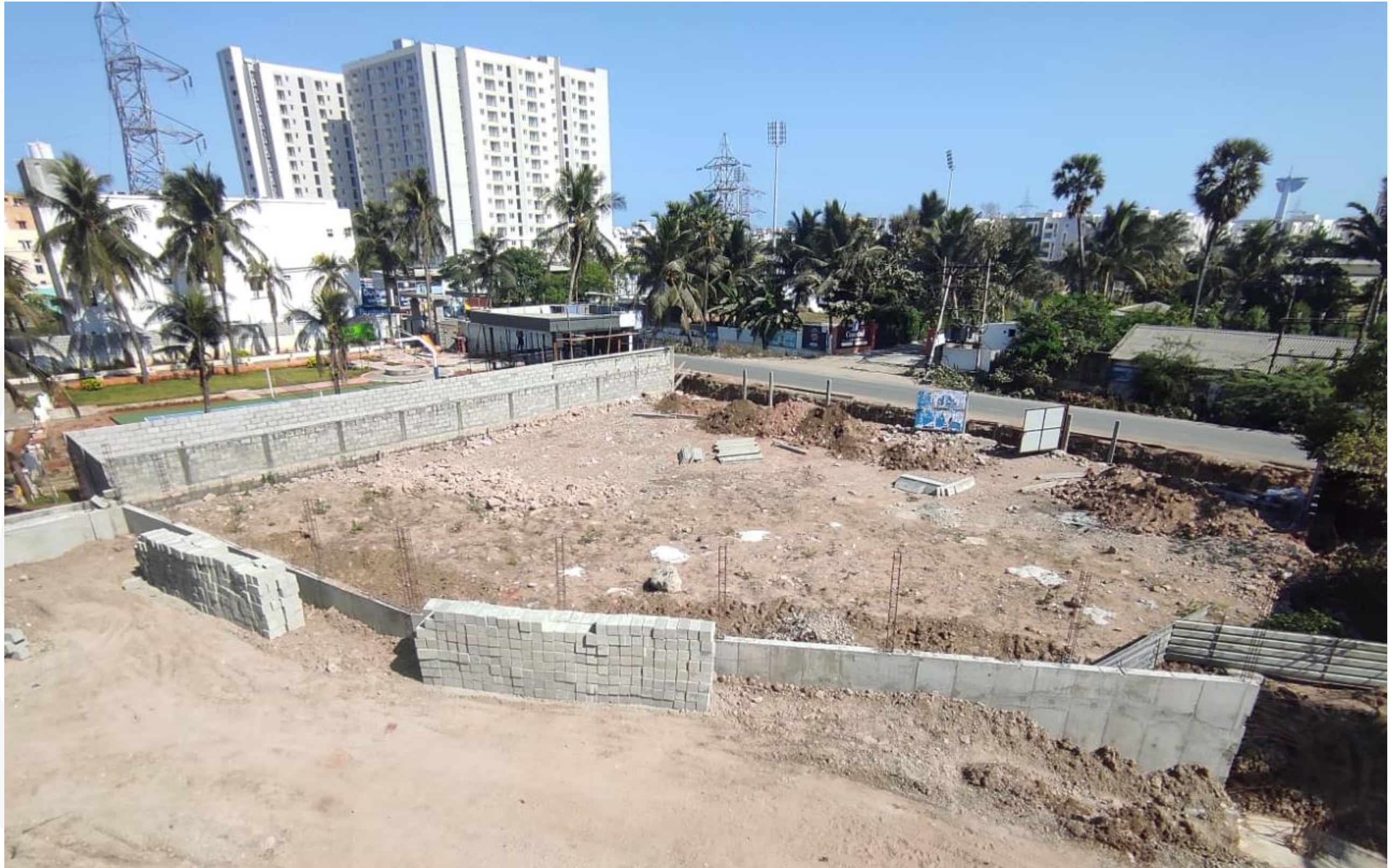
Compound Wall - South Side View
