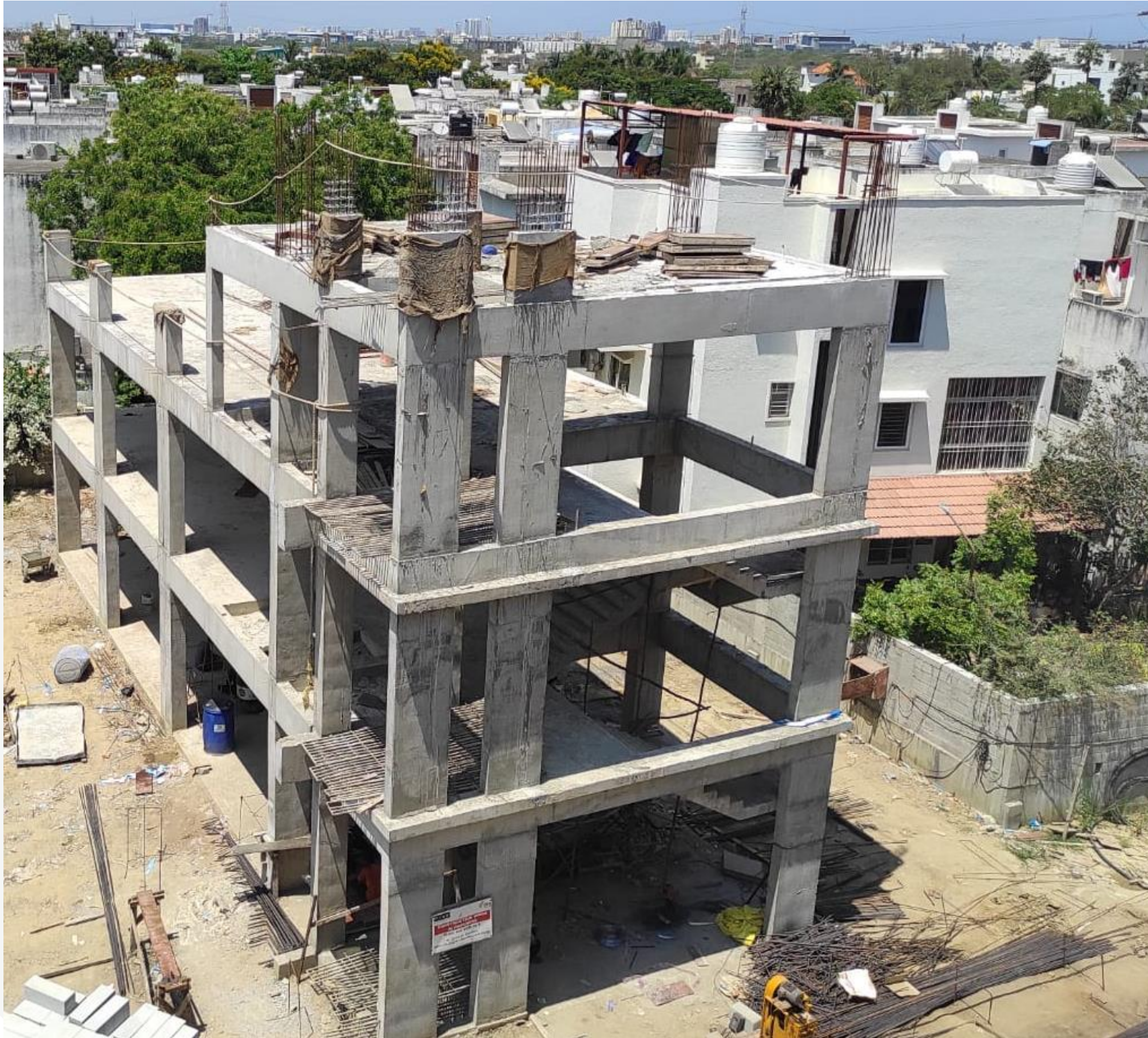
Amenity Block - LMR Column Work Completed
