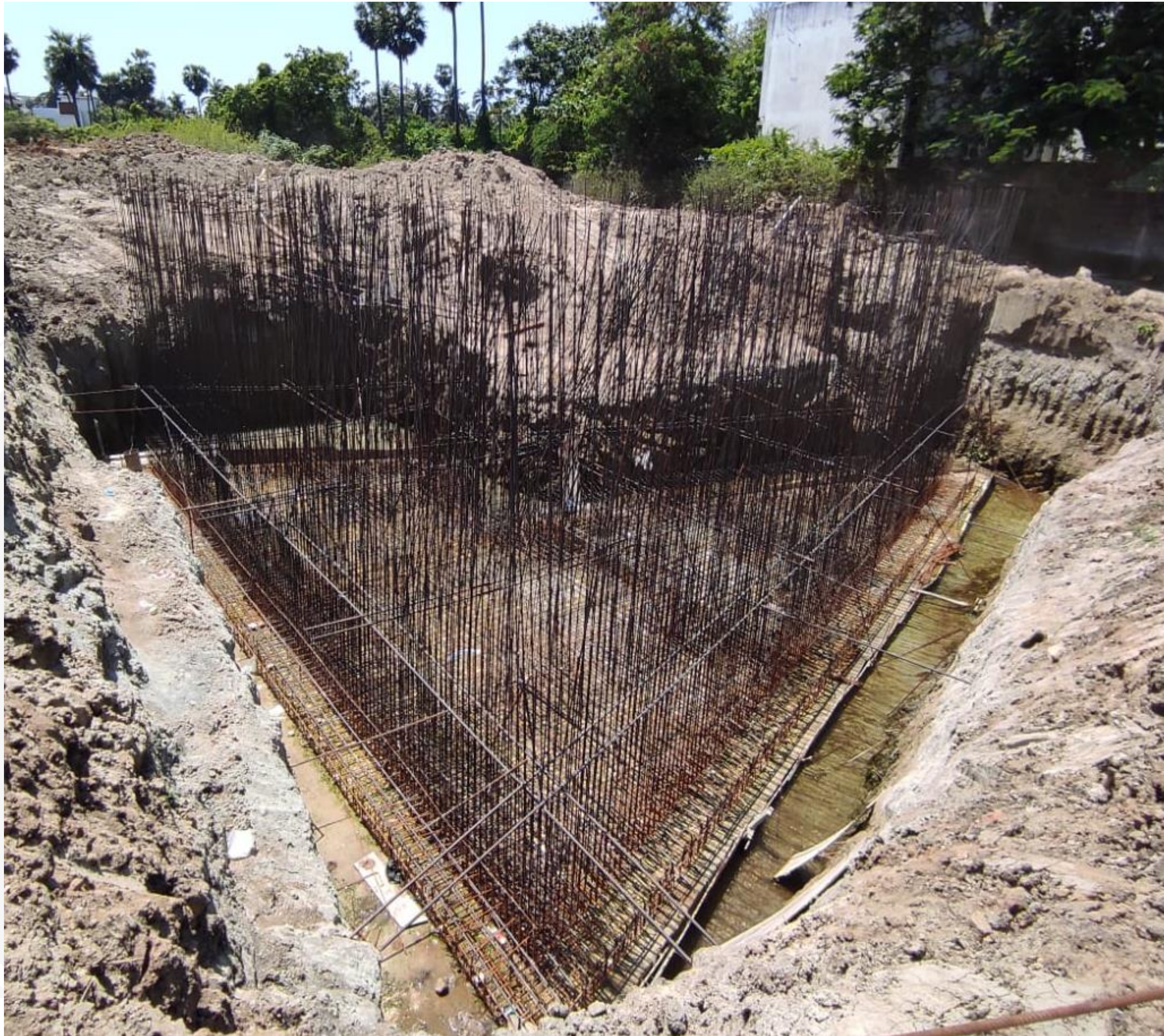
STP - Raft Reinforcement Work In Progress
