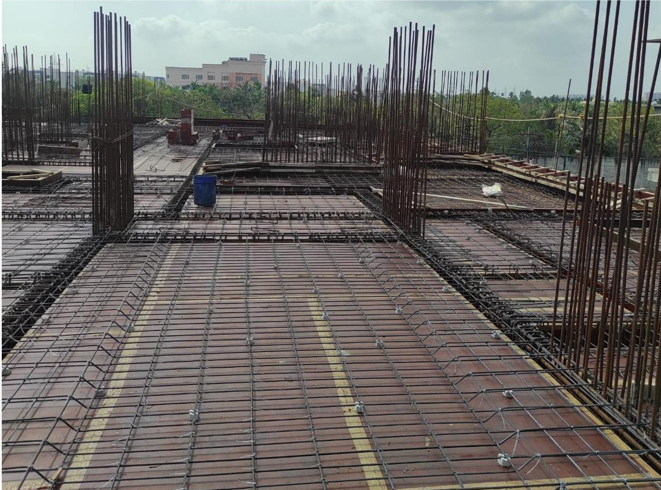
Main Building - Third Floor Roof Slab Reinforcement Work In Progress
