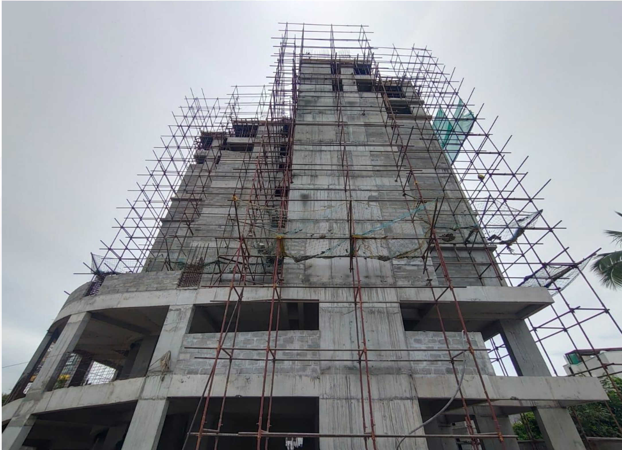
Main Building –East Side View.
