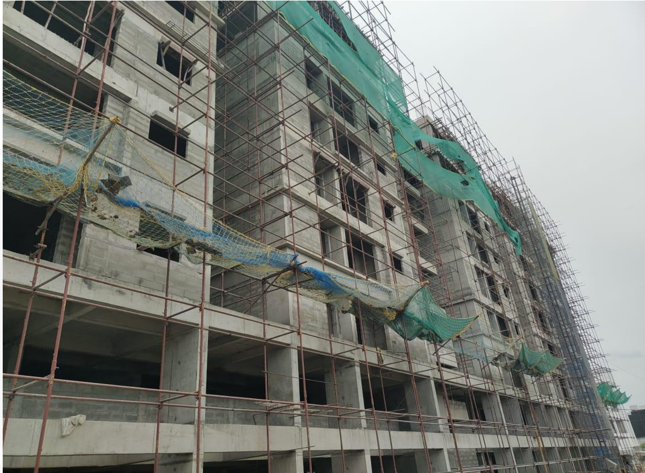
Main Building - North Side View
