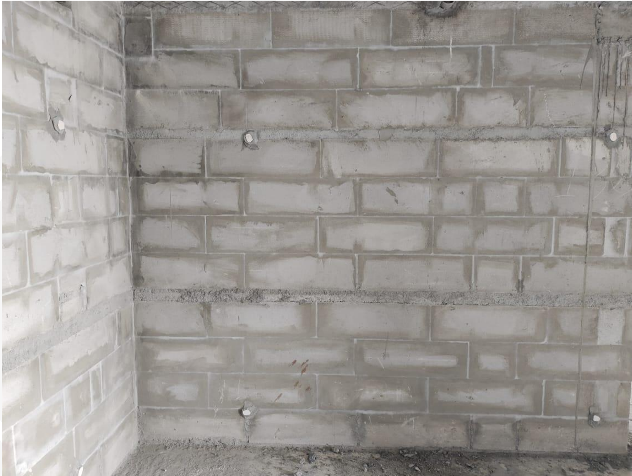
Main Building – Fourth Floor Button Marking Work In Progress.
