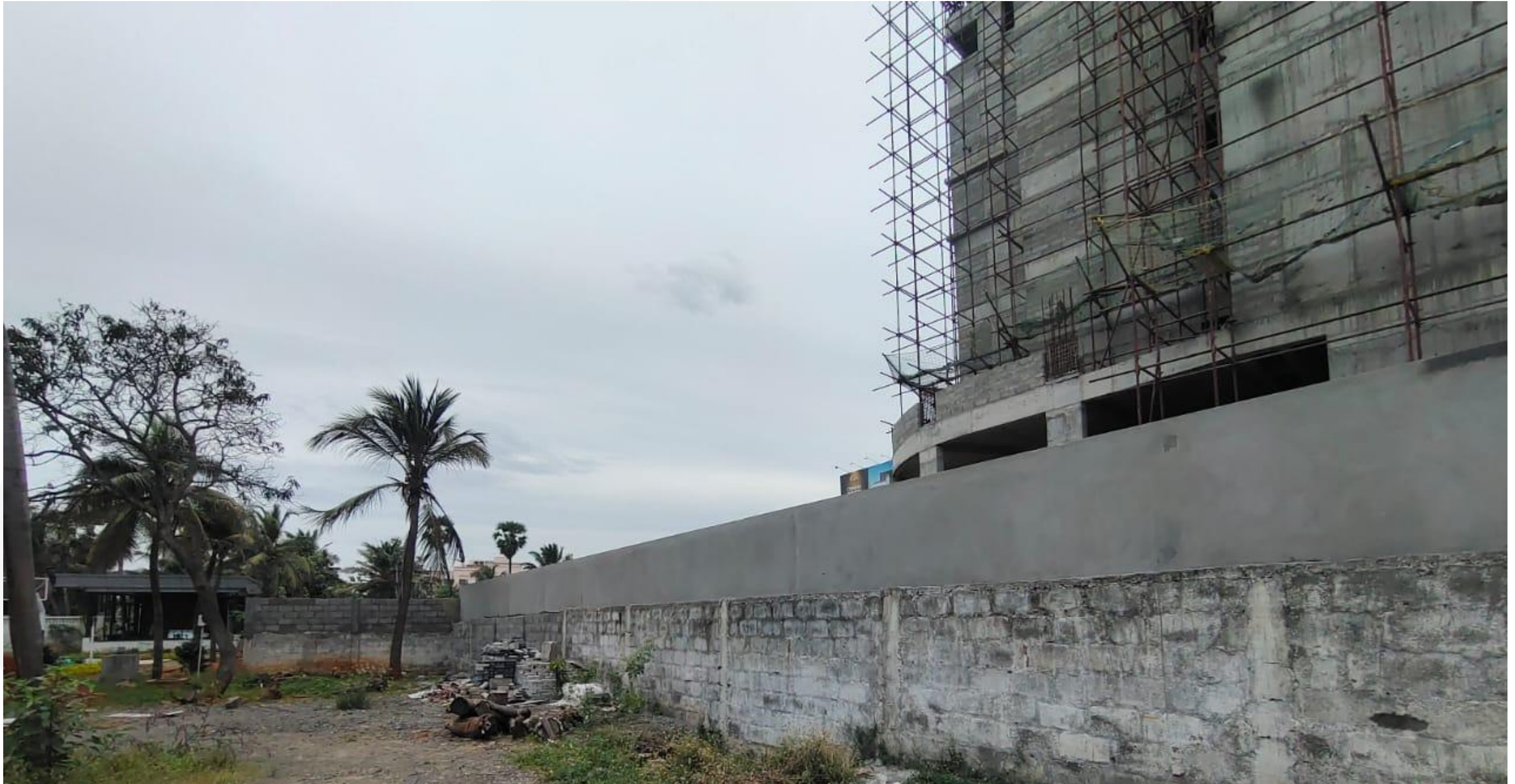
External Compound Wall Plastering – East side Plastering Work In Progress.
