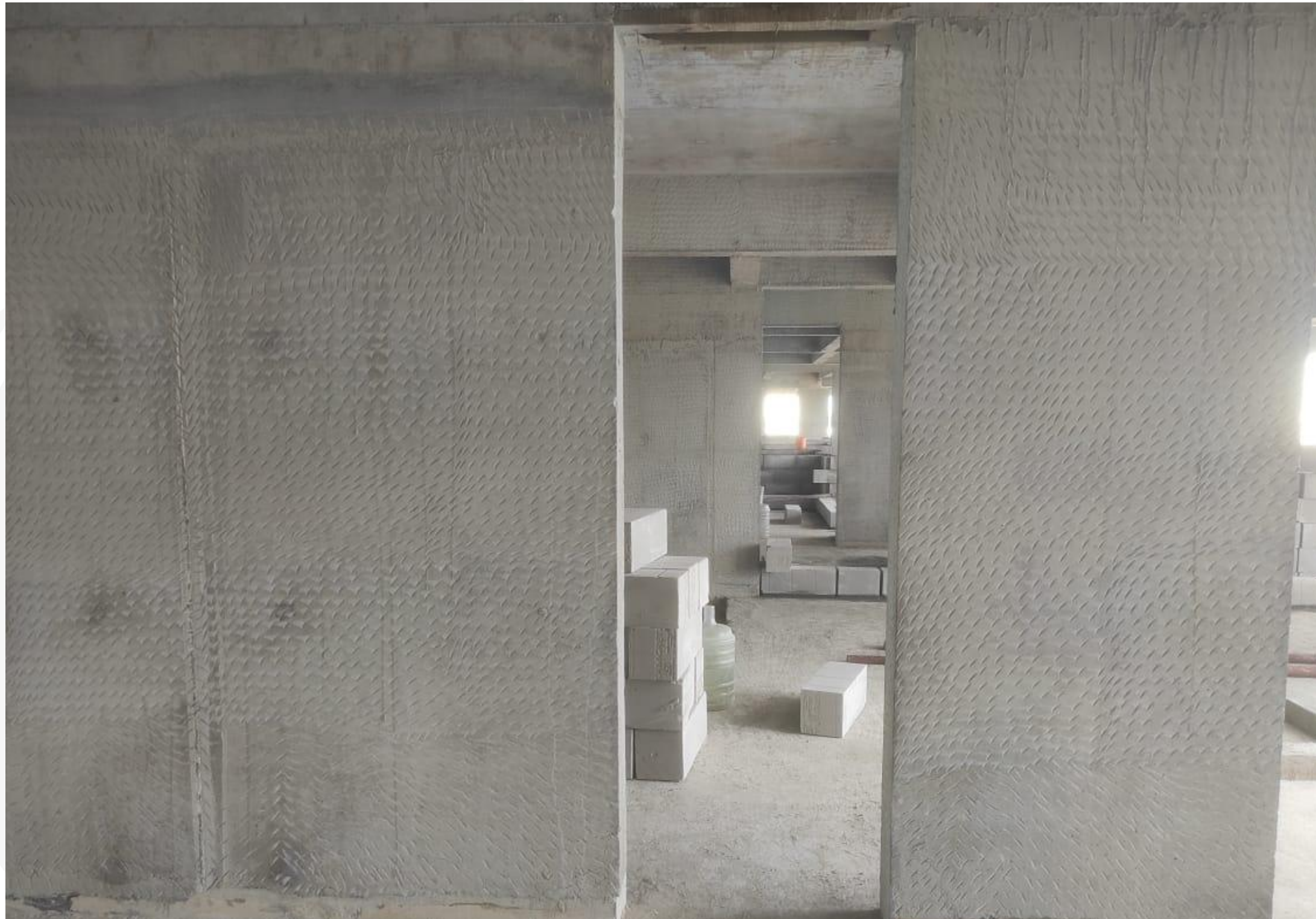
Main Building – Sixth Floor Hacking & Surface Grinding Work In Progress.
