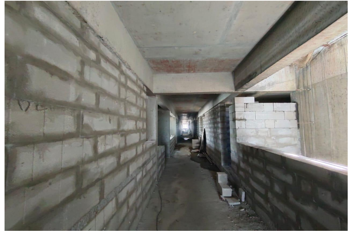
Main Building –Fifth Floor Block Work In progress.
