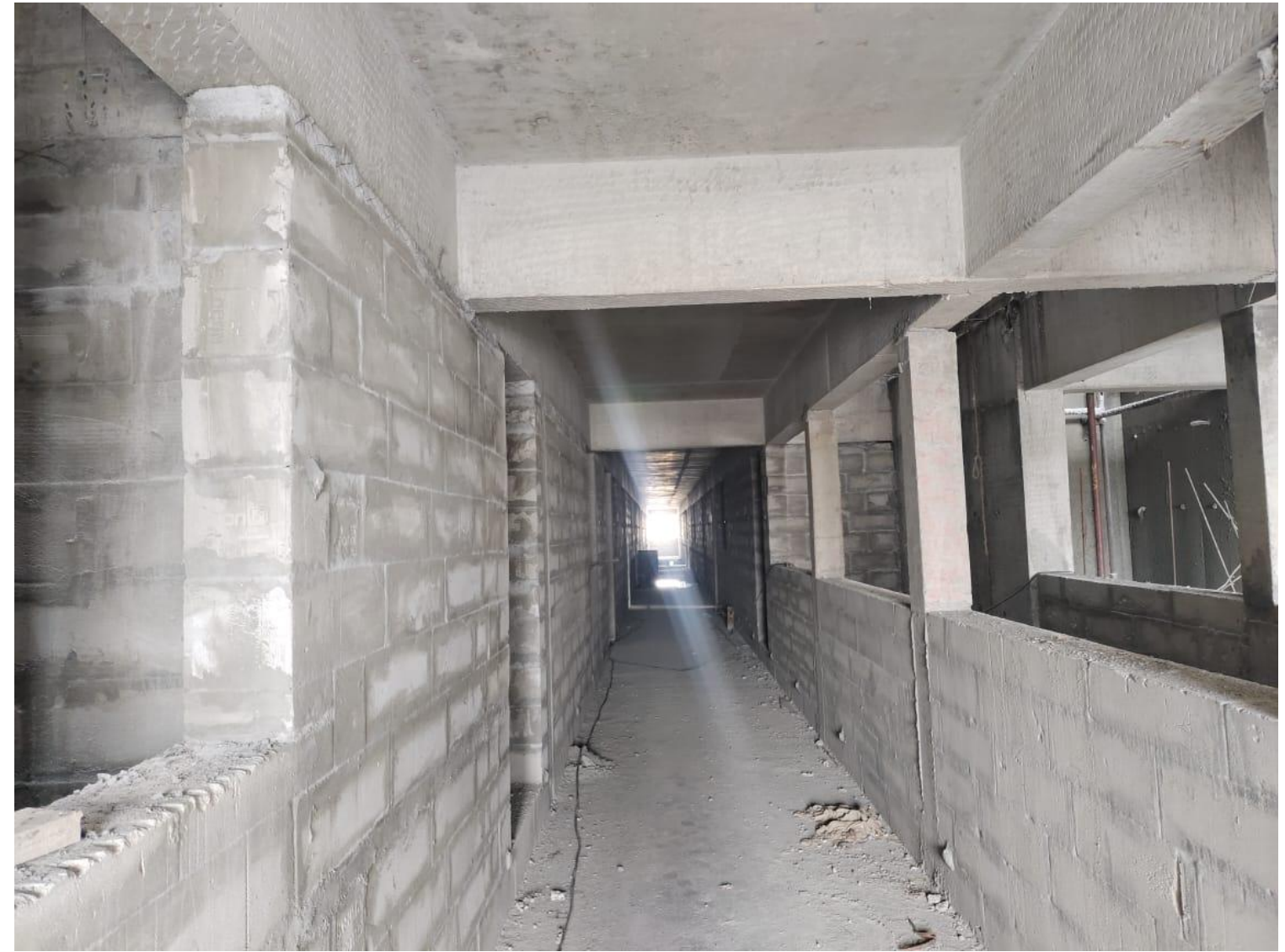
Main Building – Fourth Floor Block Work Completed.
