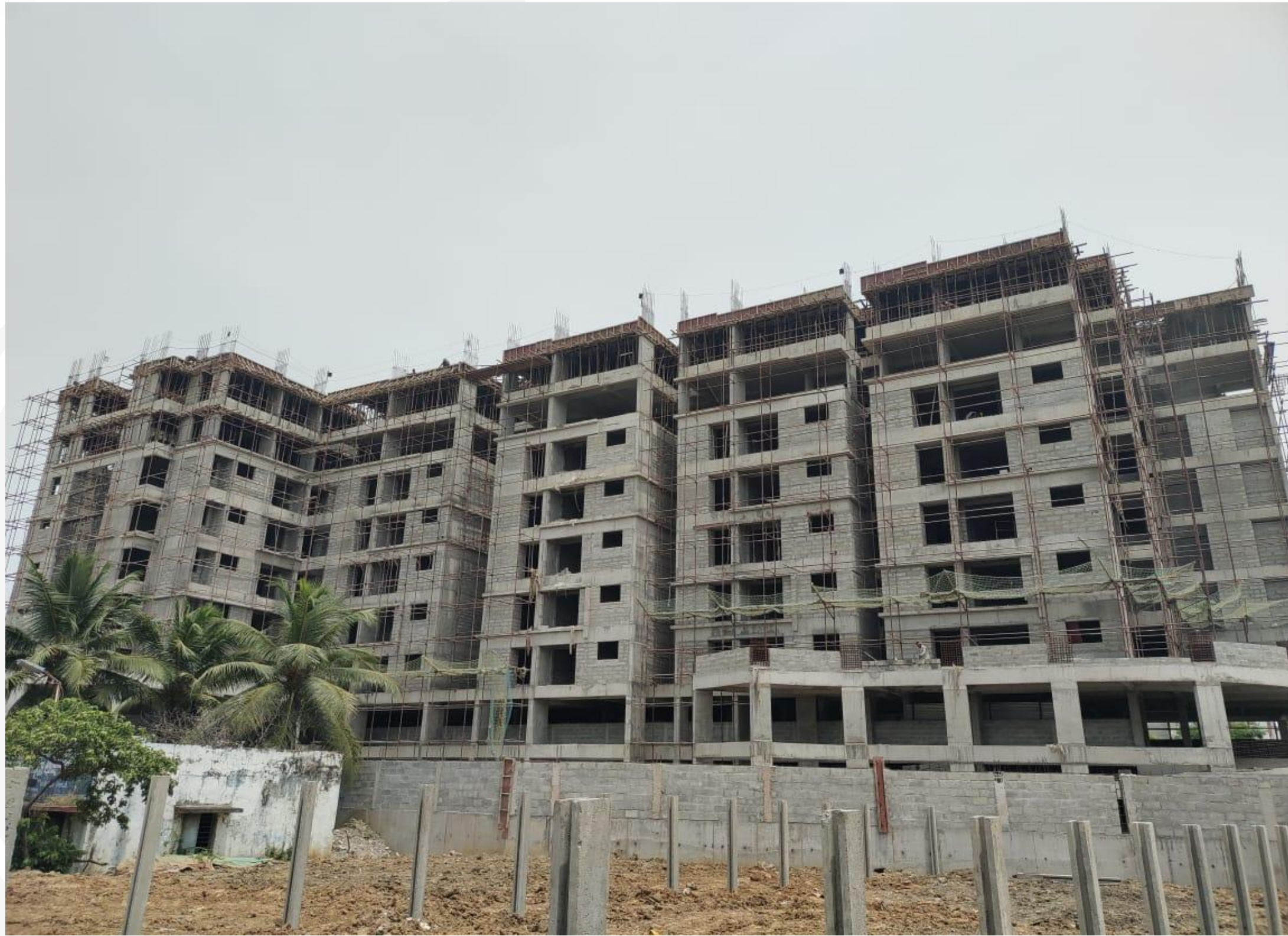
Main Building - South Side View.
