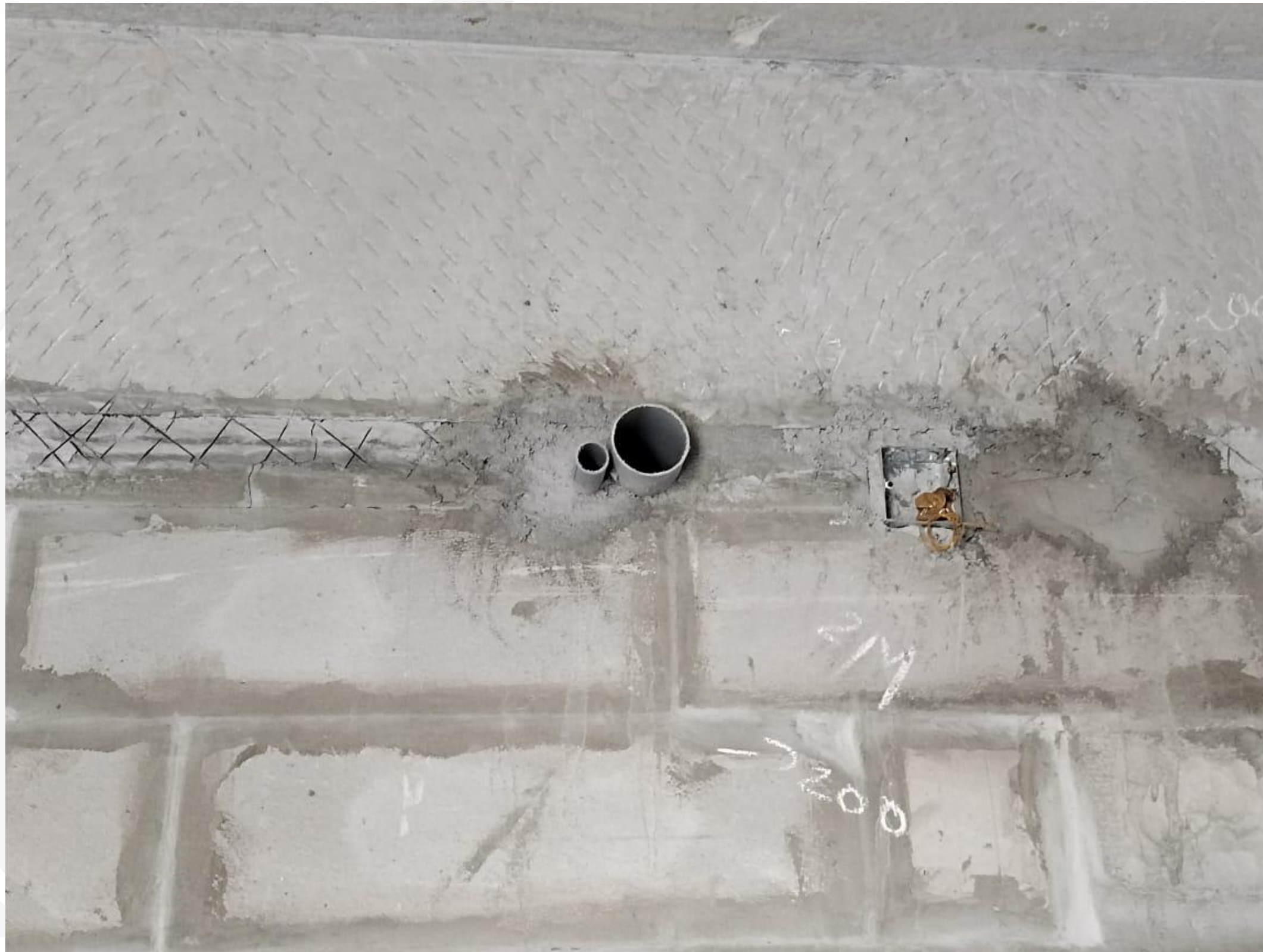
Main Building Plumbing – Third Floor AC Sleeve Fixing Work In Progress.
