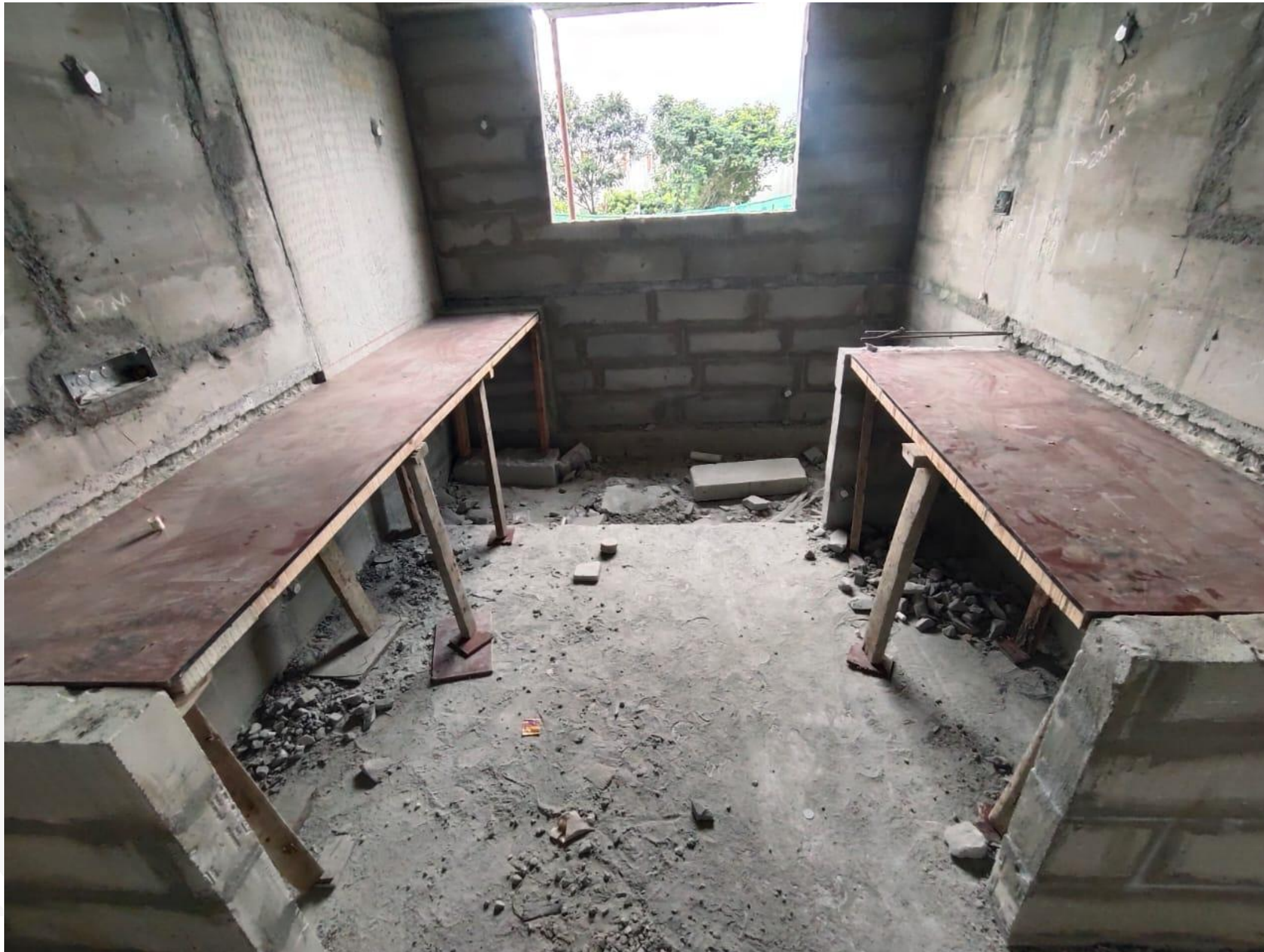
Main Building – First Floor Kitchen Counter Slab Work In Progress.
