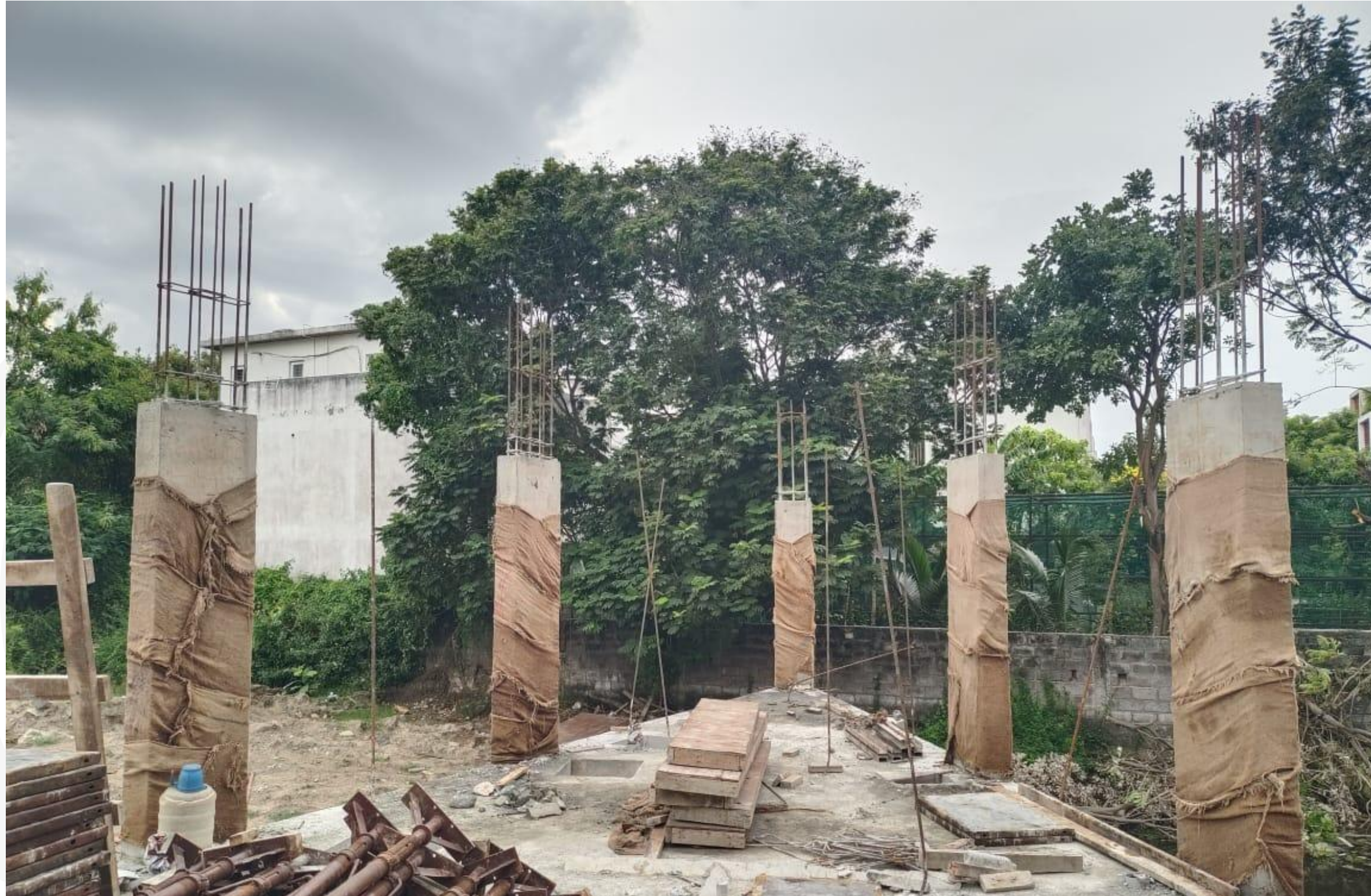
STP – Head Room Column Concrete Work Completed.
