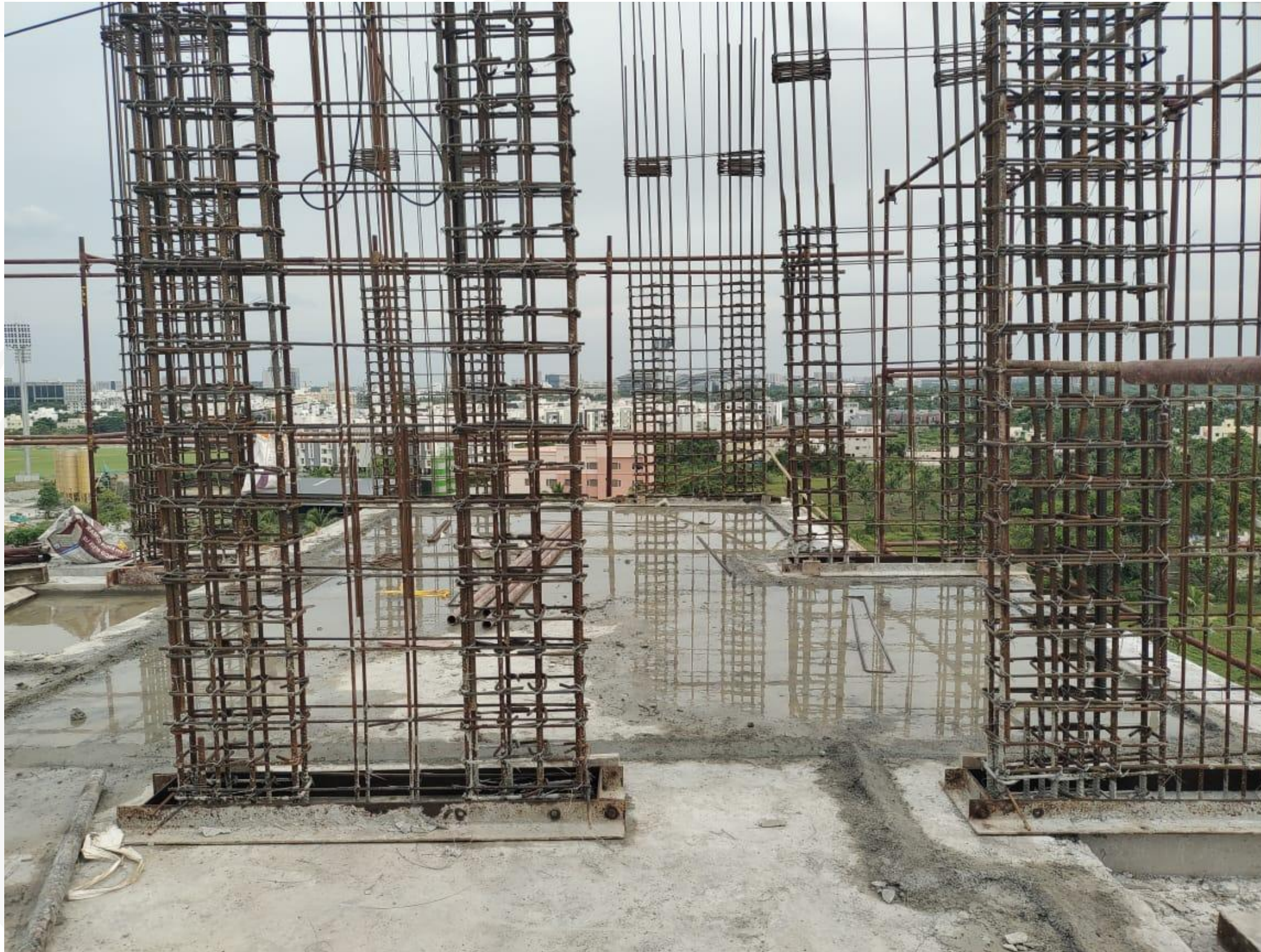
Main Building – Eighth Floor Column Starter & Reinforcement Work In Progress.
