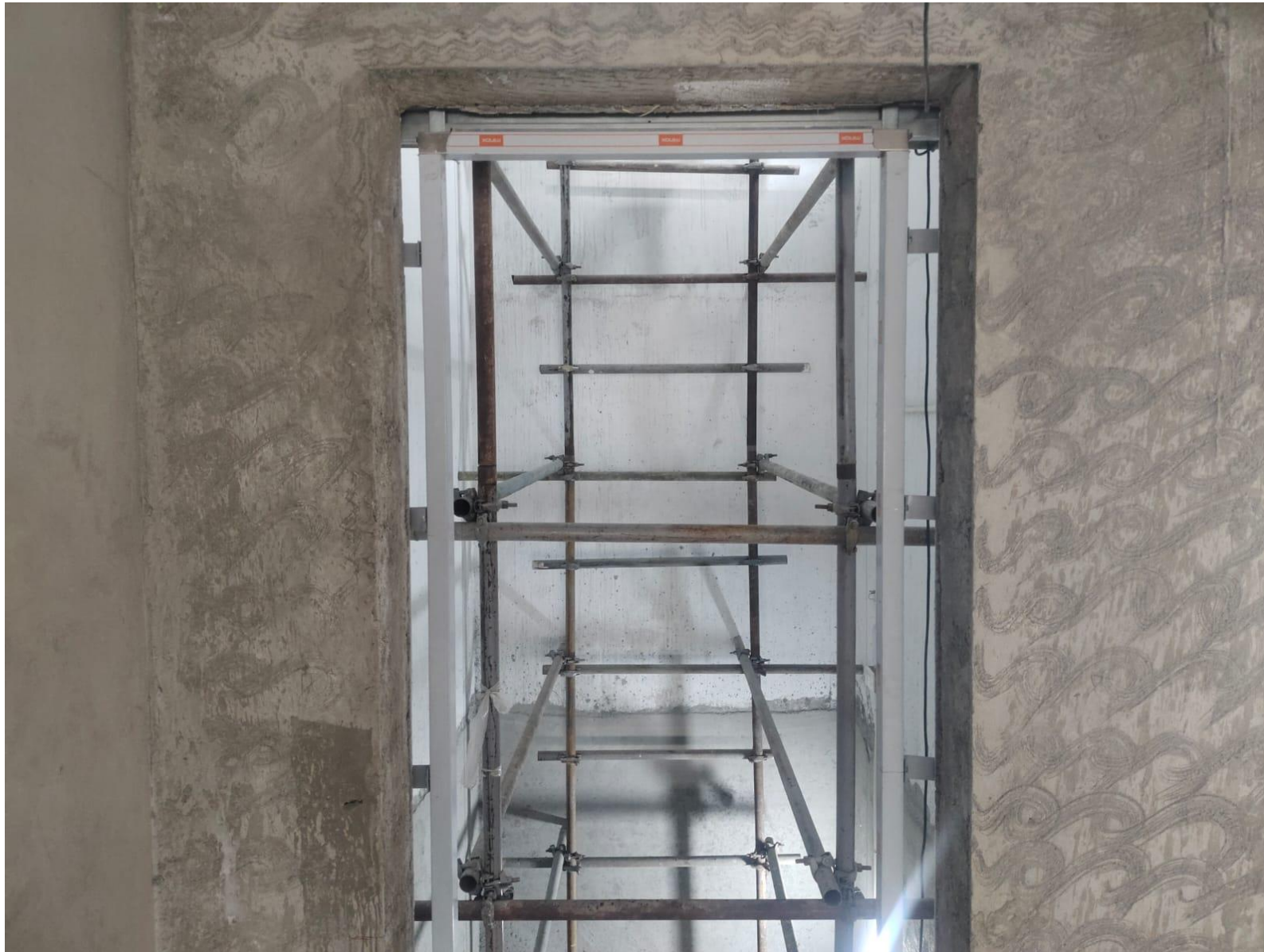
Lift – Frame Fixing Work In Progress
