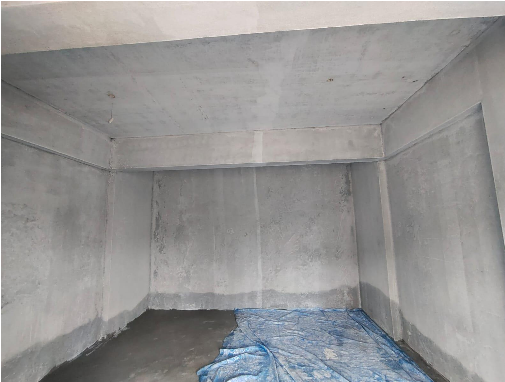
EB Panel room – Primer Work In Progress
