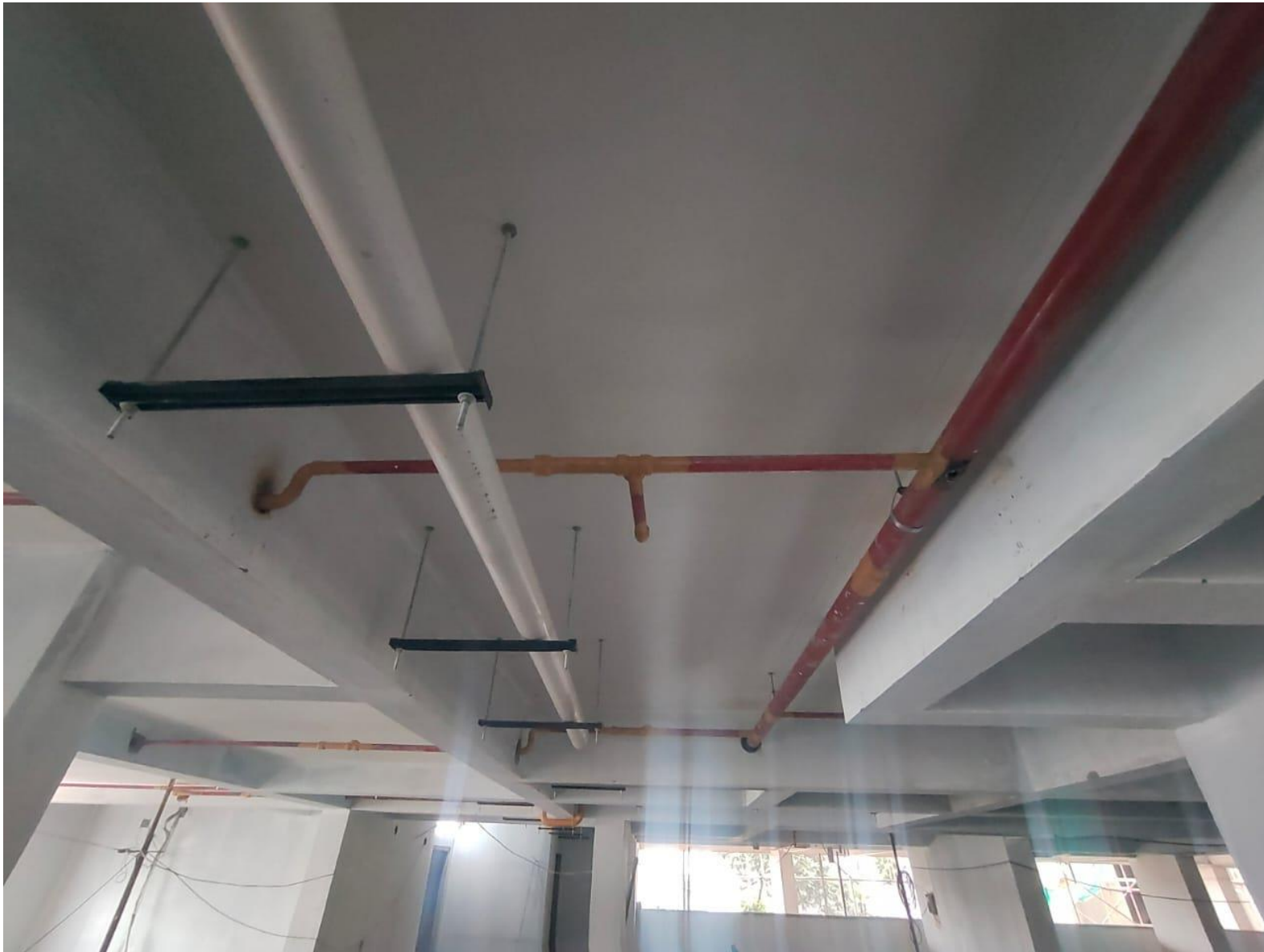
Upper Stilt – Fire Fighting Work In Progress
