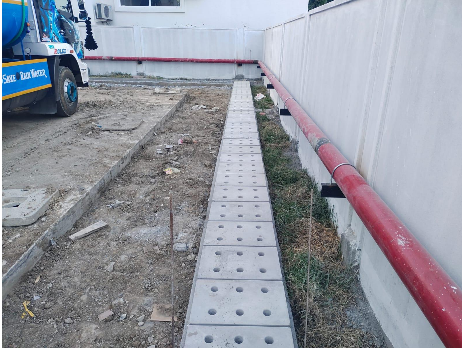
Trench – Precast Slab Laying Work In Progress
