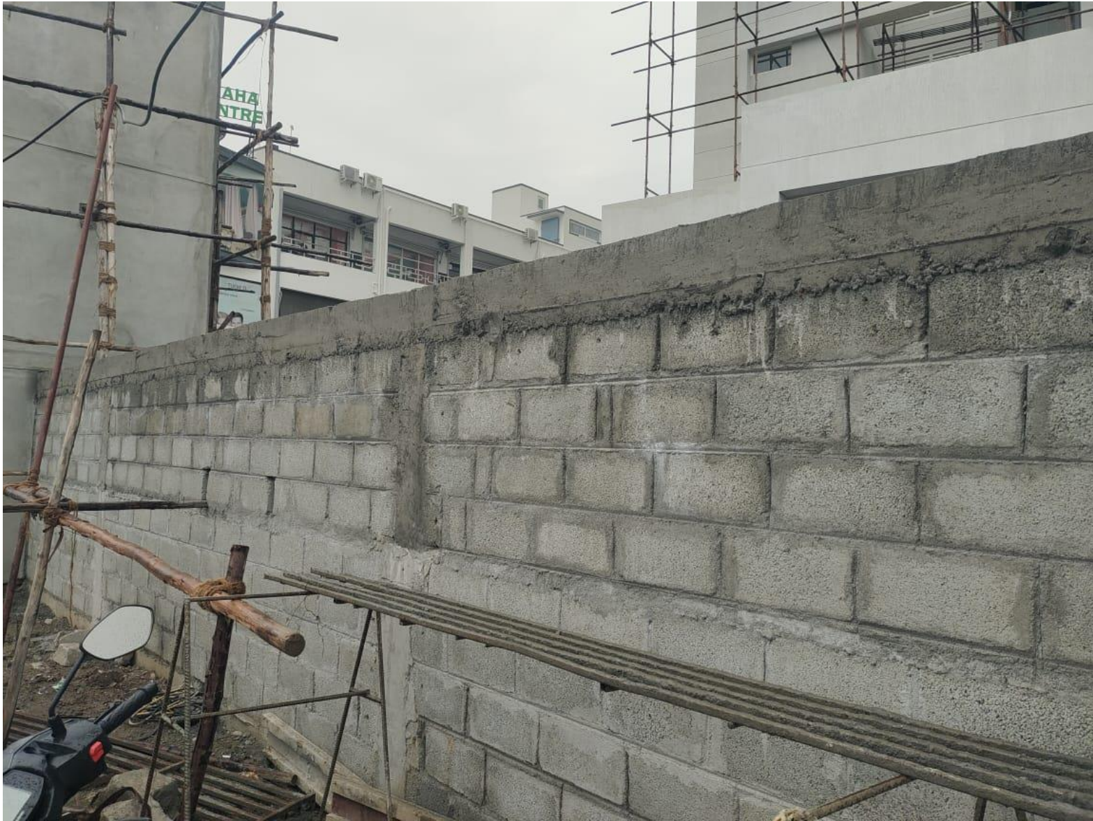
Entrance- Landscape Wall Block Work Completed
