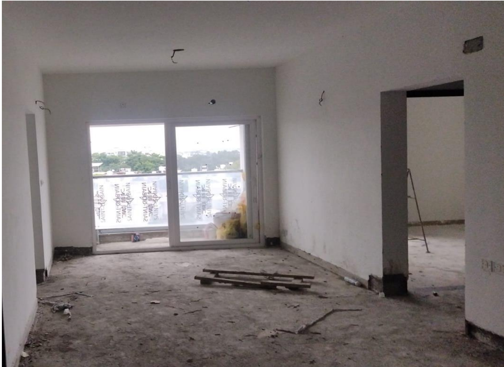
Tenth Floor – Primer Work In Progress
