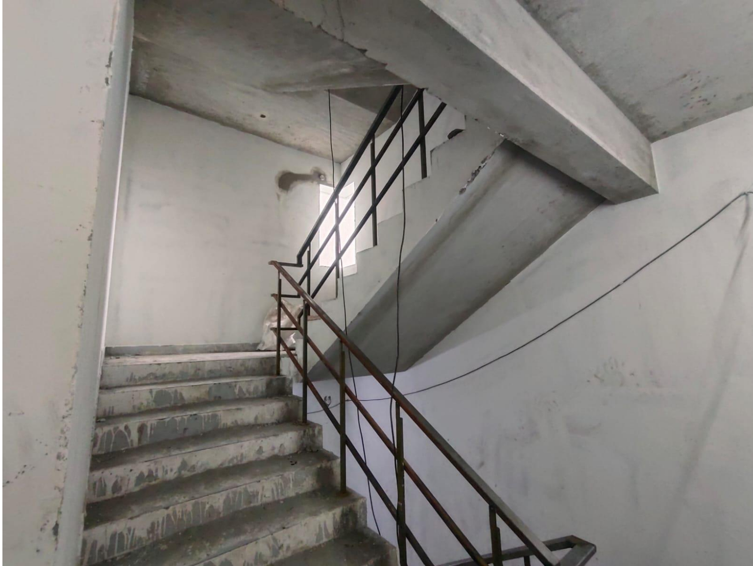
Staircase Handrail – West Side Fixing Work In Progress
