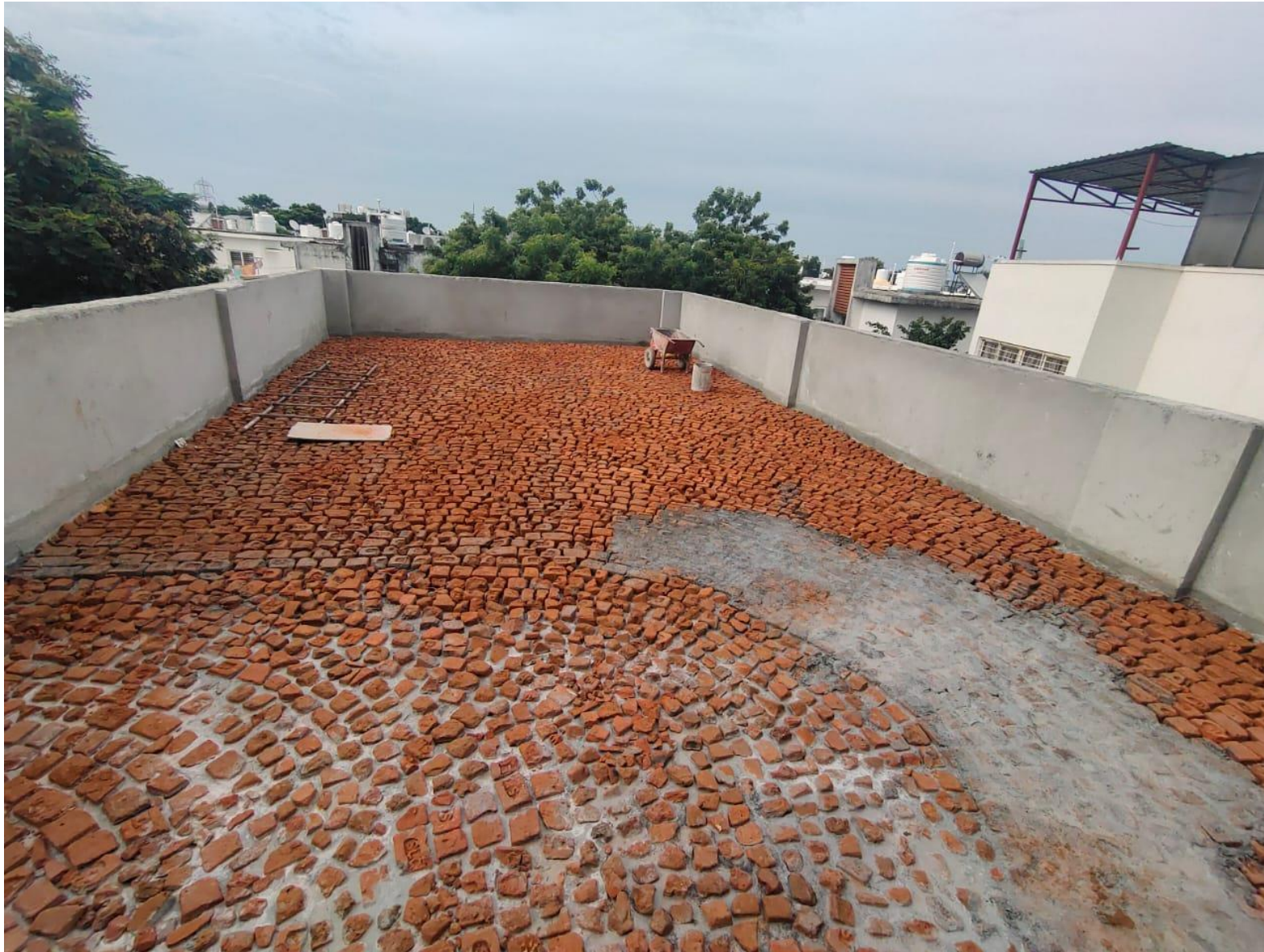
Amenity Block – Brickbat Work Completed
