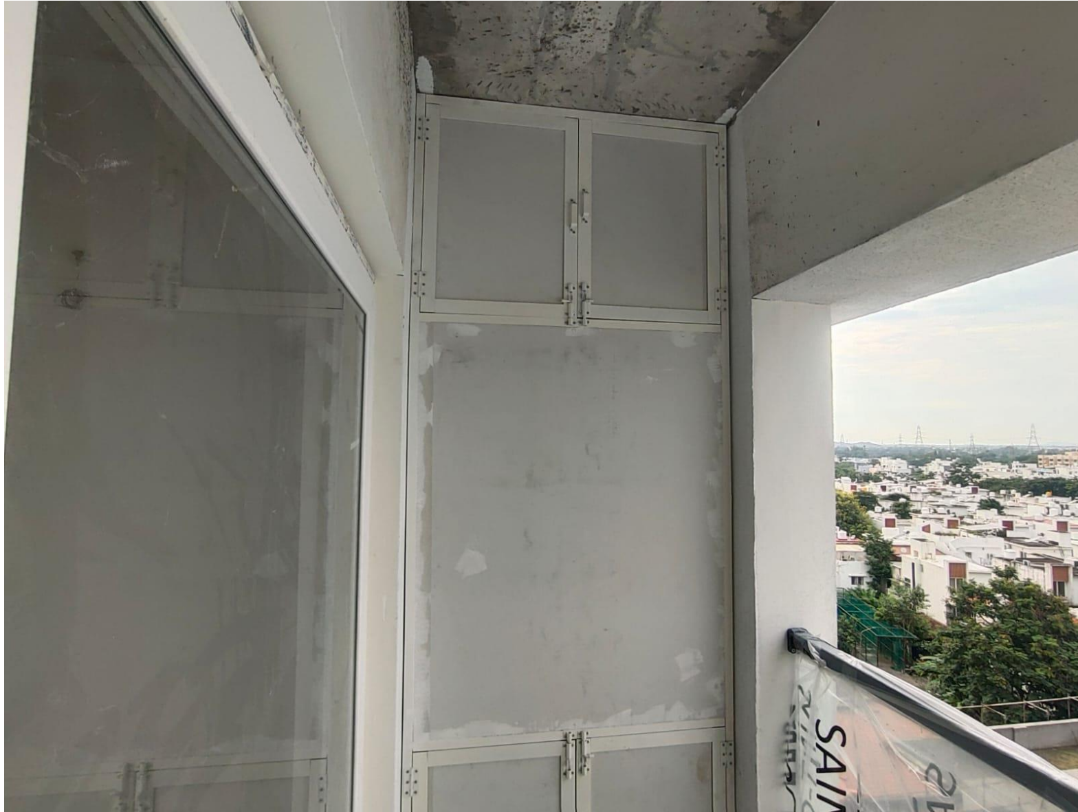
Balcony Trap Door – Fixing Work In Progress
