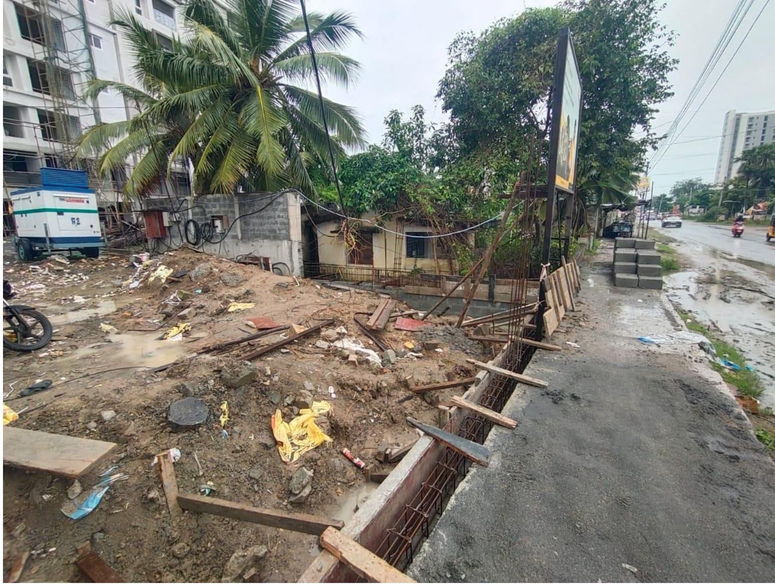
Entrance Compound wall – Plinth Beam Work In Progress
