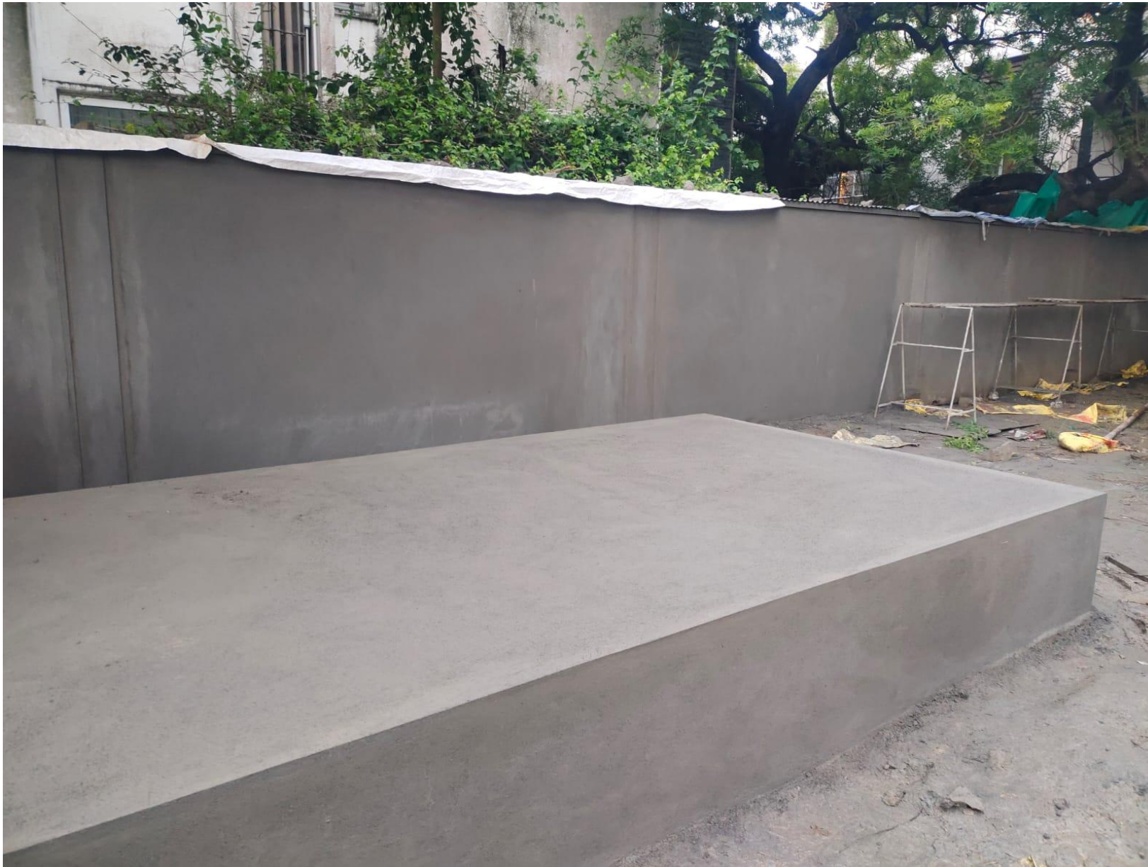
DG Bed Work Completed
