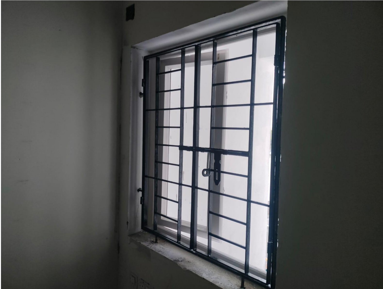
Window Grill – Fixing Work In Progress
