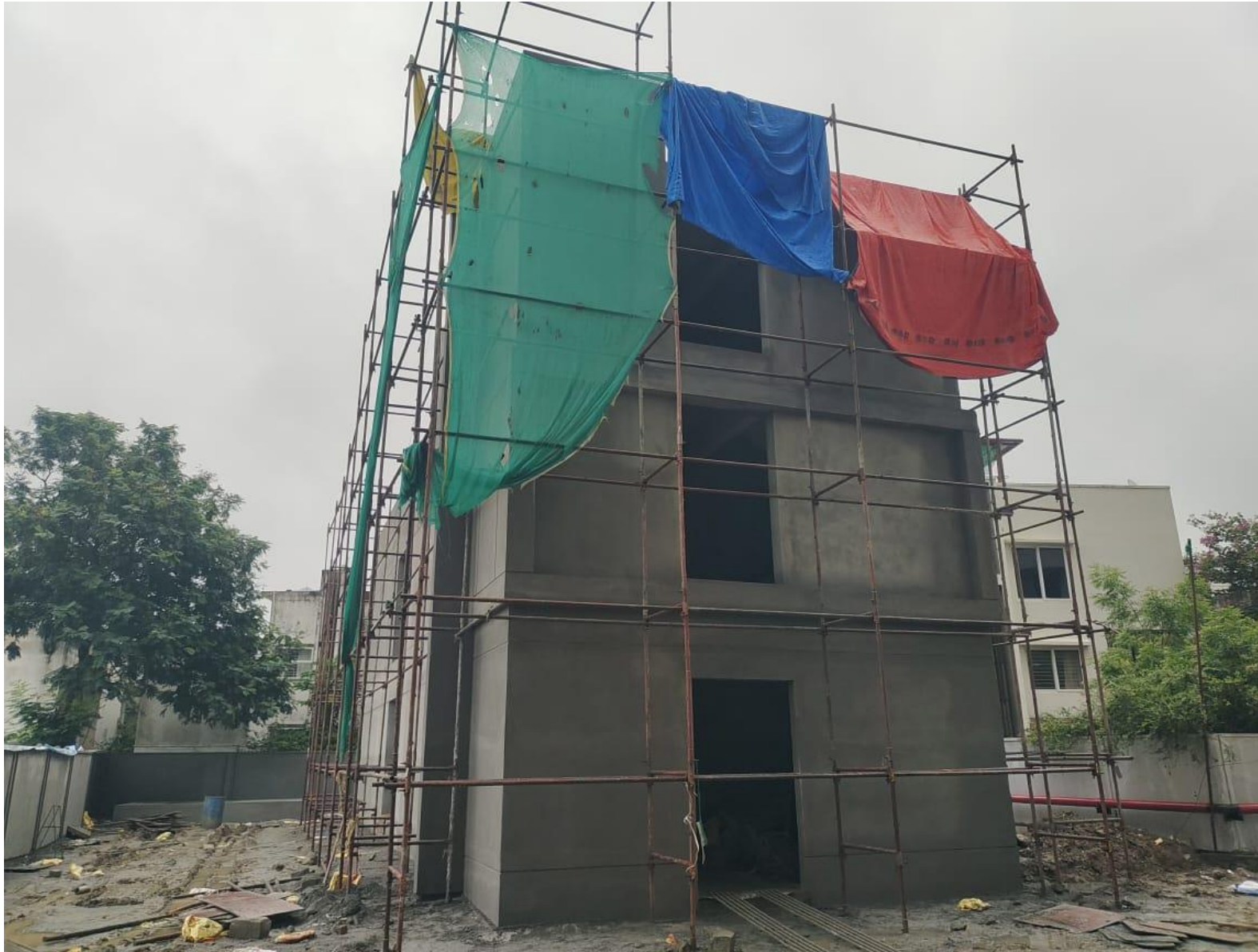
Amenity Block External Plastering – South Side Work In Progress
