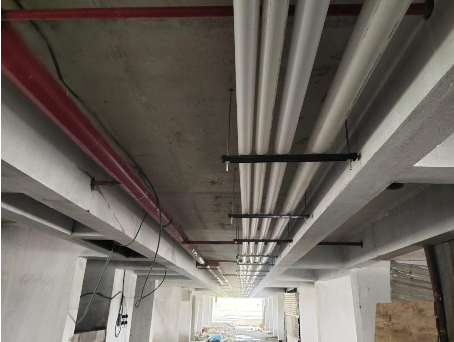
Plumbing – Upper Stilt Ring Main Line Work In Progress
