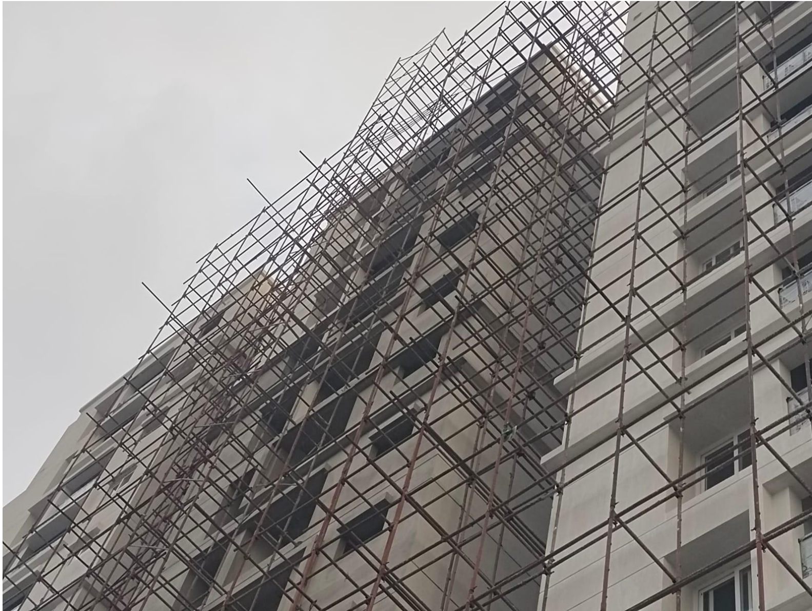
External Texture – North Side Work In Progress
