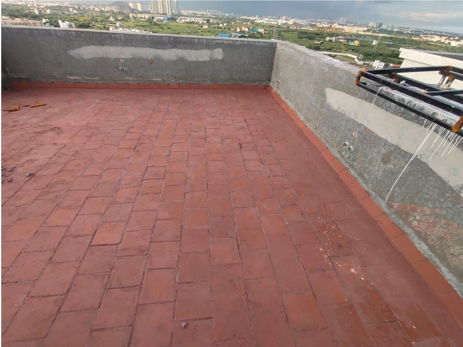
Terrace – Press Tiles Laying Grouting Work Completed
