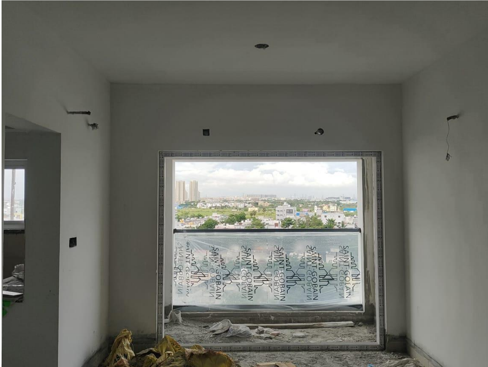
Balcony Glass Handrail – Fixing Work In Progress
