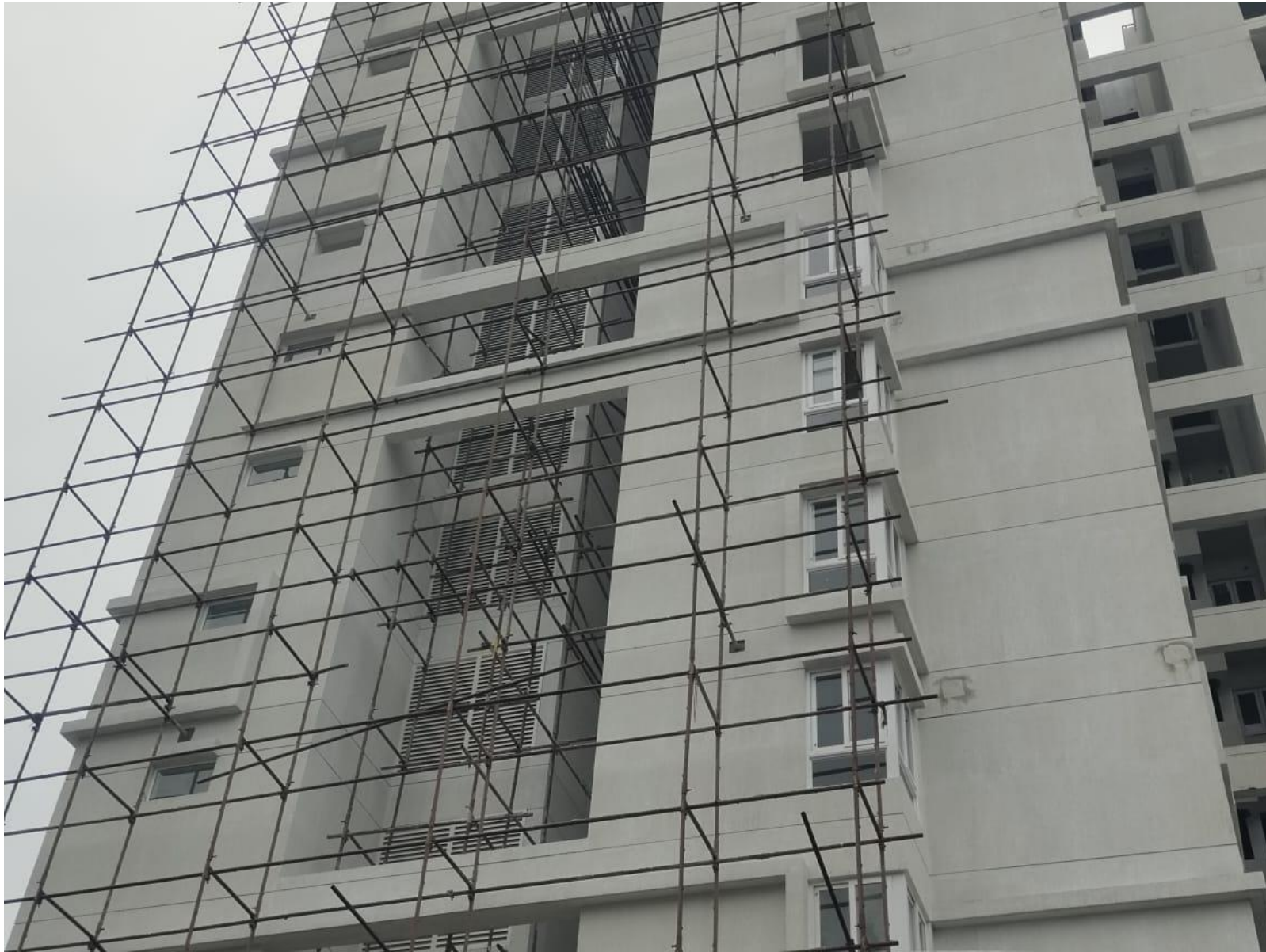
Aluminum Louver – Elevation Fixing Work In Progress
