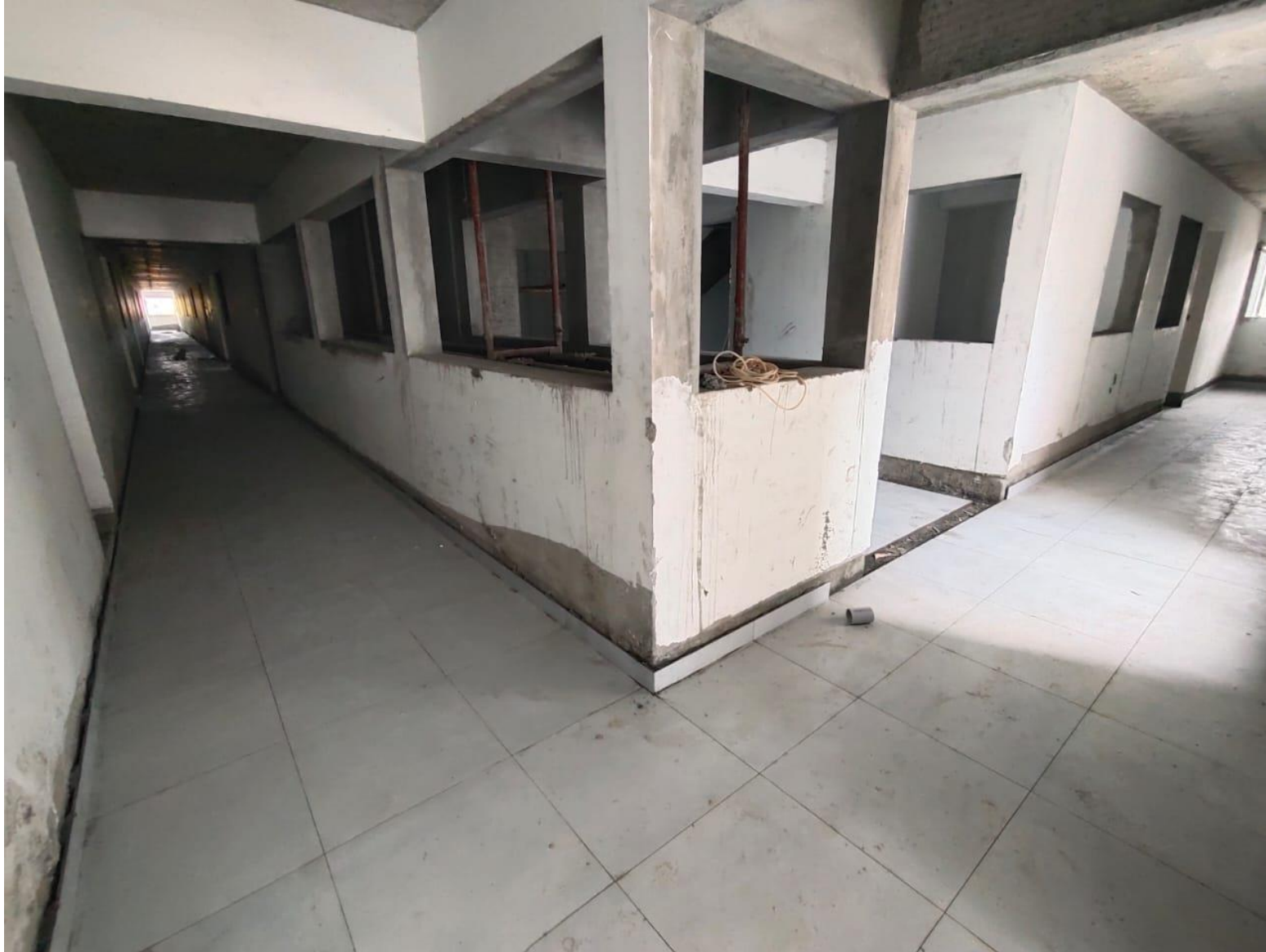
Corridor Tiles – Up to 13 th Floor Completed
