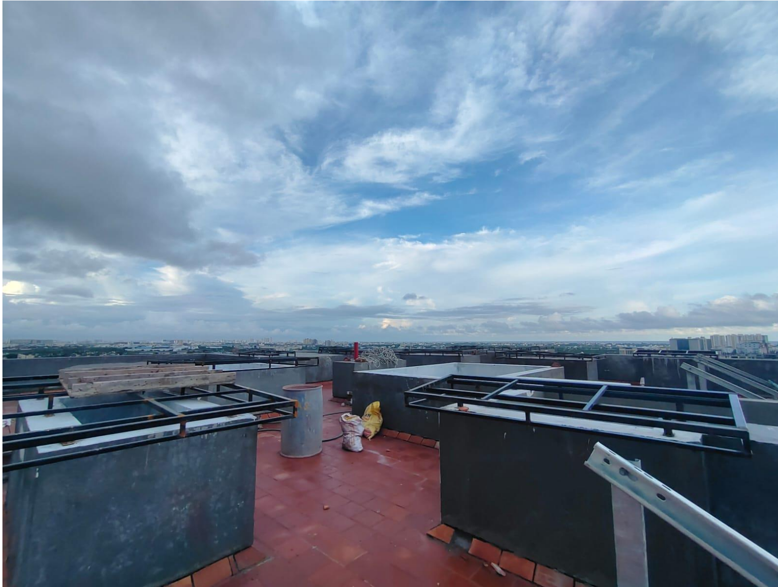
OTS Covering – Fabrication Work In Progress
