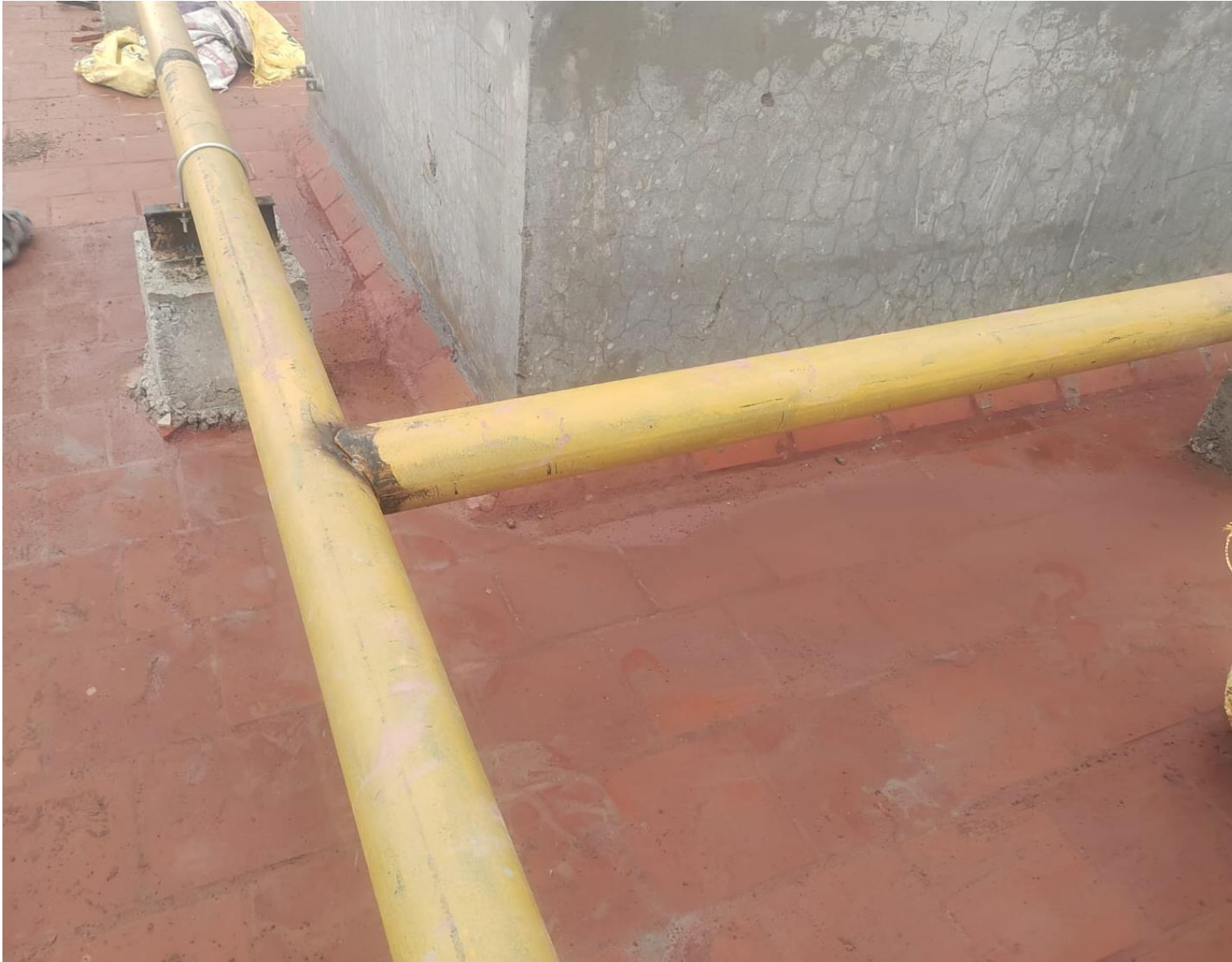
Terrace – Hydrant Line Work In Progress
