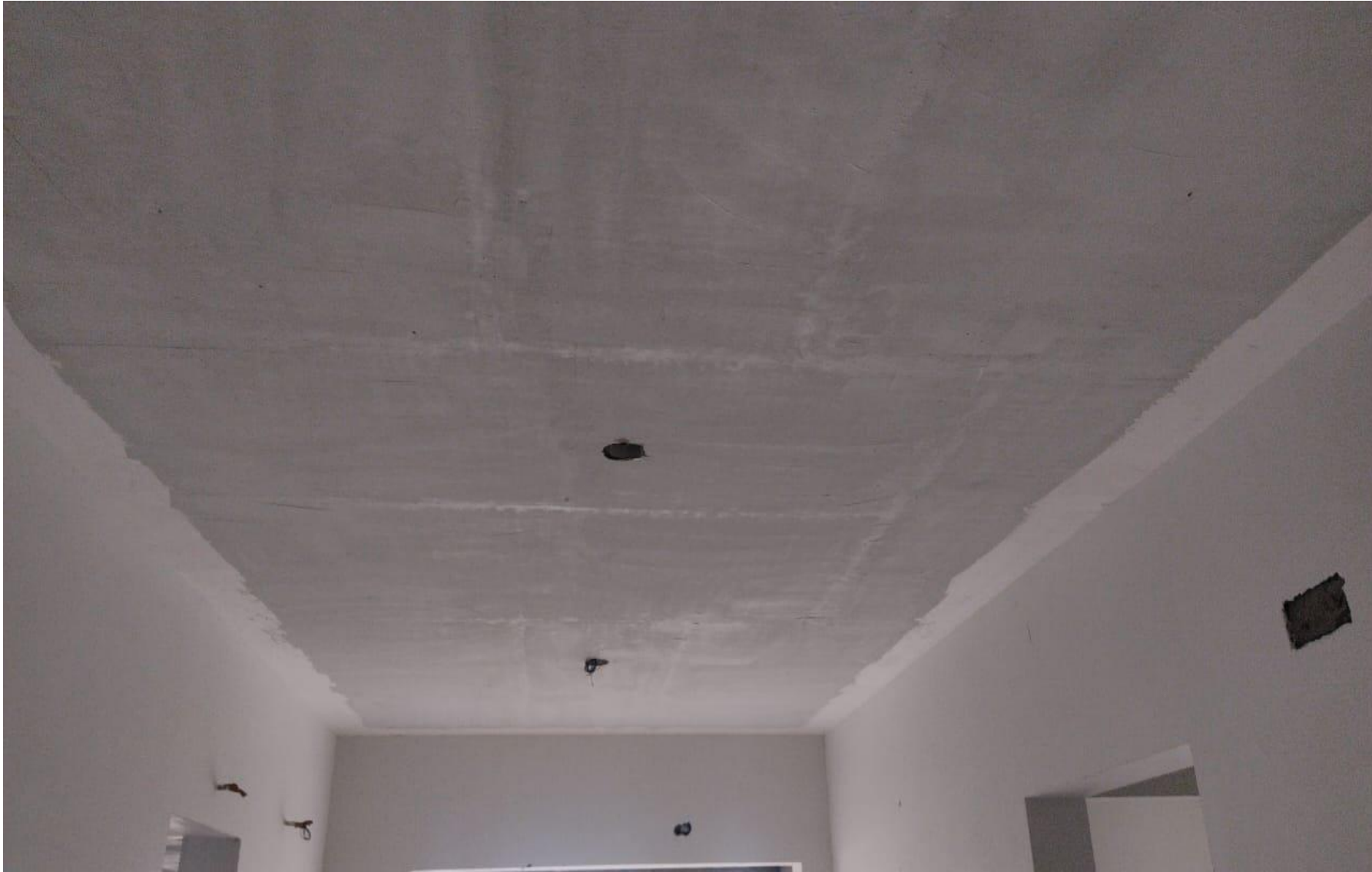
Putty Work – 11 th Floor Work In Progress
