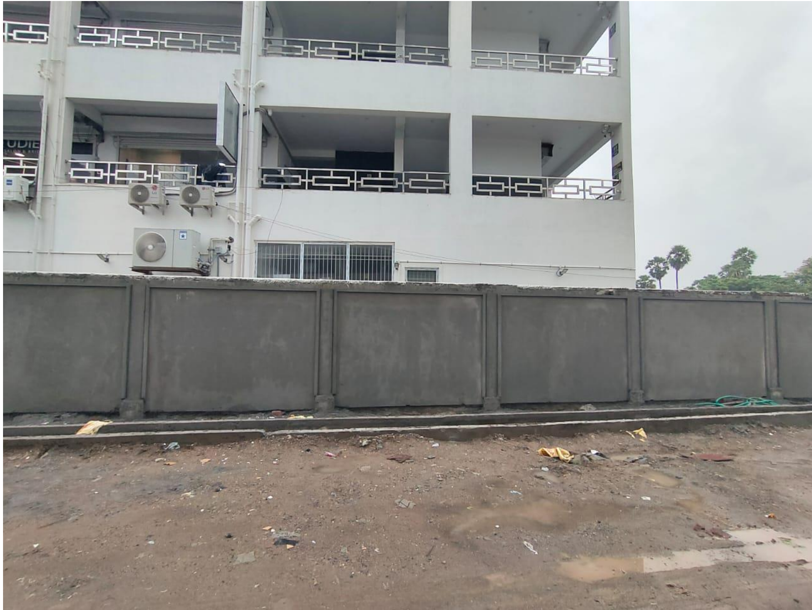
Compound Wall Plastering – West Side Work In Progress
