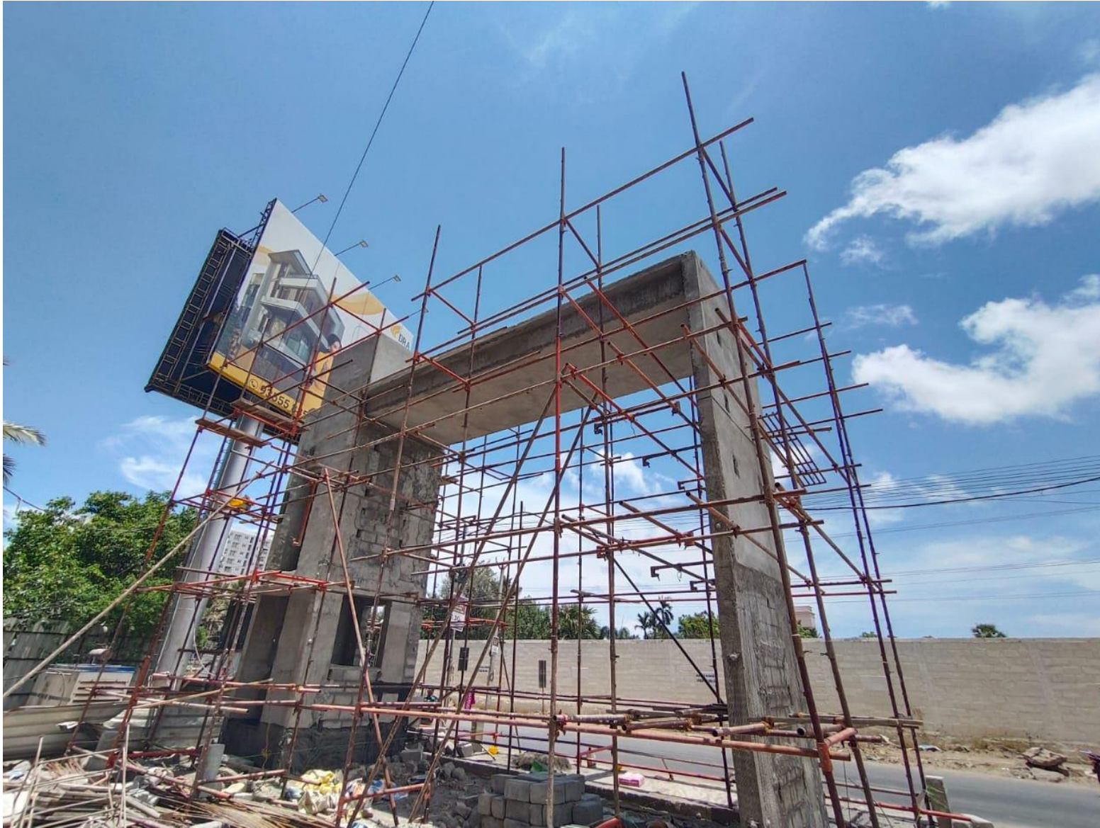
Entrance Plaza– Entry Arch Plastering Work In Progress
