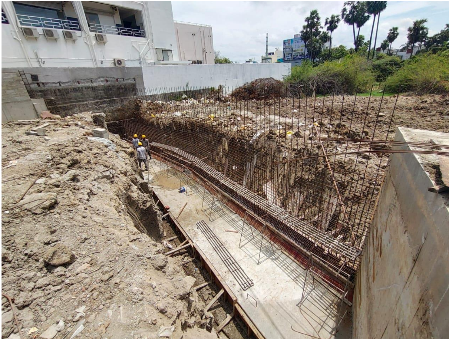
Compound Wall – Type-6 Raft Concrete Completed & Wall Work In Progress
