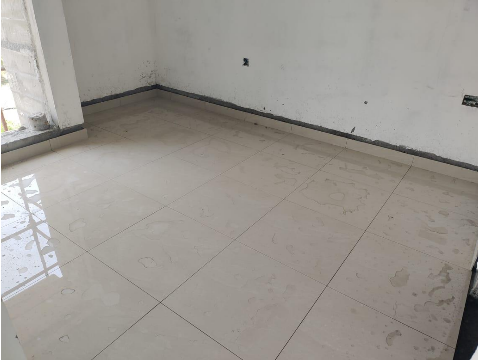
Floor Tile - Sixth Floor Tile Laying Work In Progress
