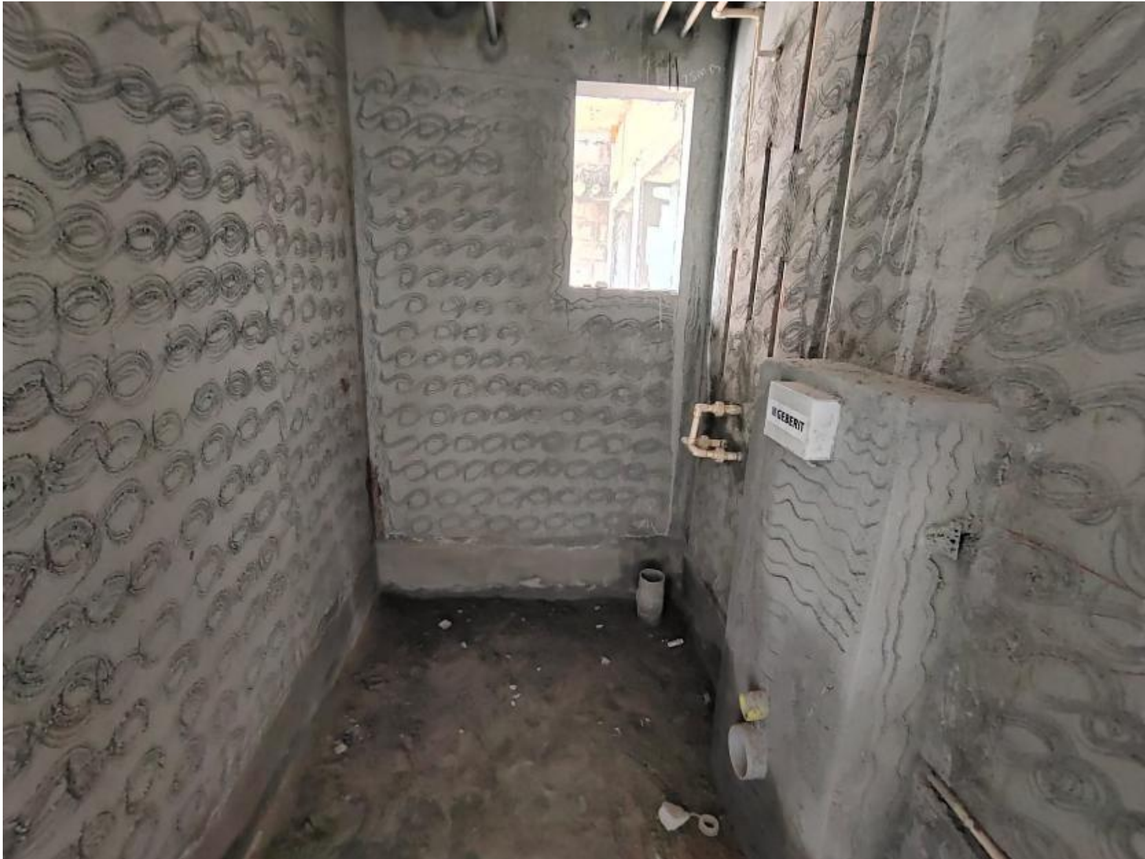
Plumbing – Tenth Floor Ledge Wall Work Completed
