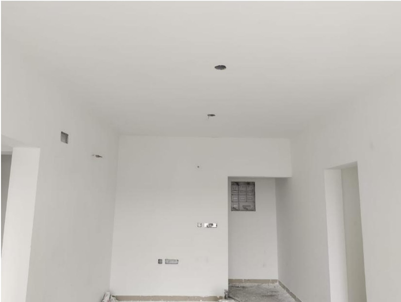
Third Floor – 2 nd Coat Wall Putty Work Completed
