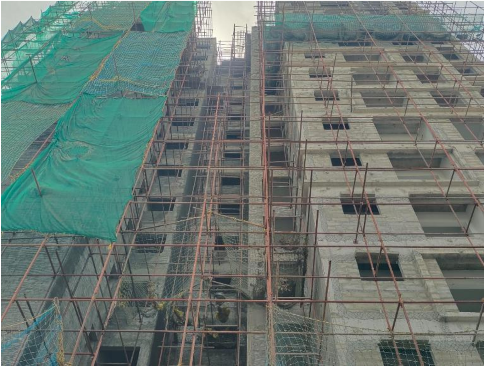
External Plastering – West Side Rough & Final Coat Work In Progress
