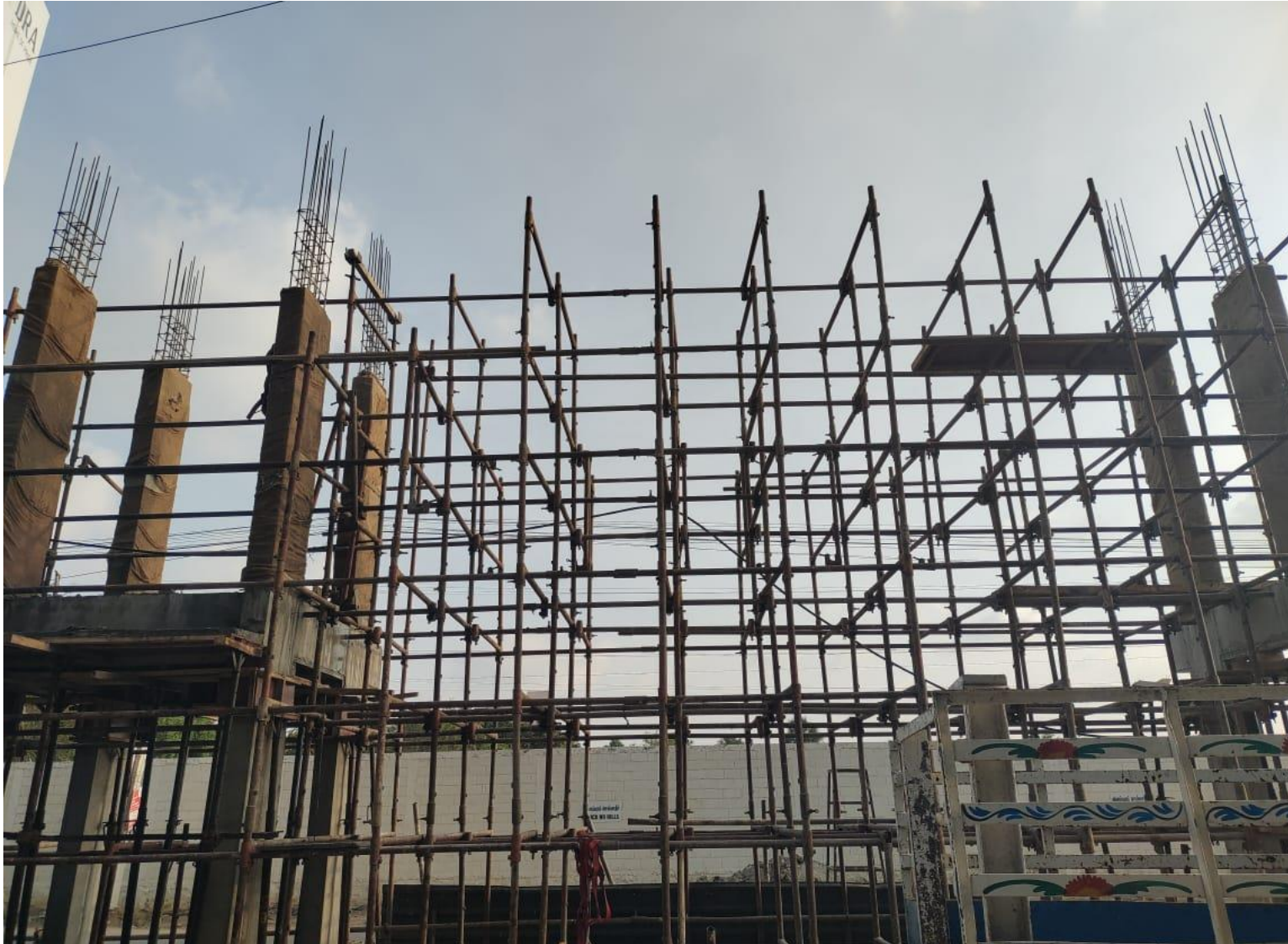
Entrance Structure – Column Concrete Work Completed & Roof Slab Work In Progress
