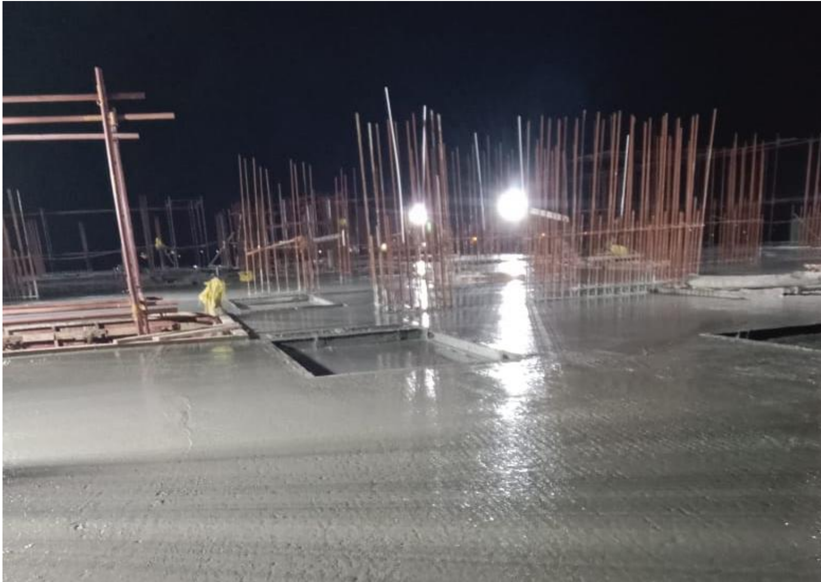
Twelfth Floor Roof Slab Concrete Work Completed
