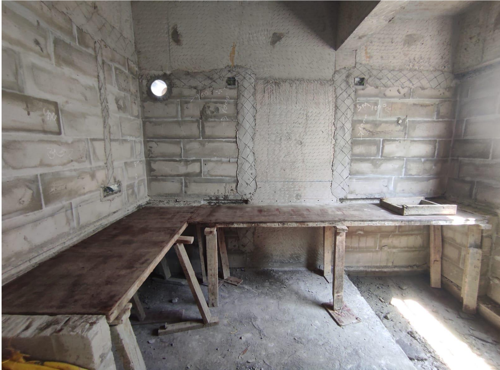
Tenth Floor Kitchen Counter Slab Work In Progress
