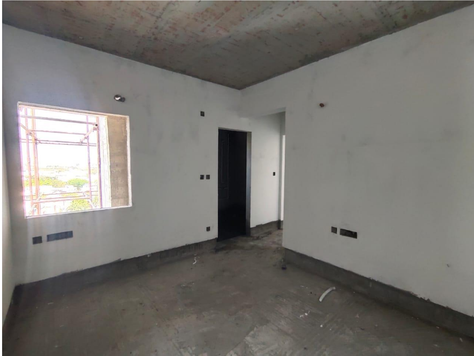
Seventh Floor 1 st Coat Wall Putty Work In Progress
