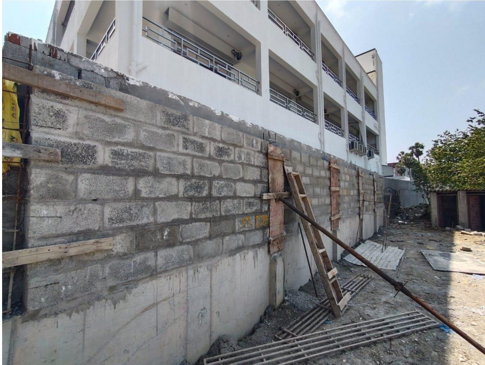
External – Type-1 Compound wall Block Work In Progress
