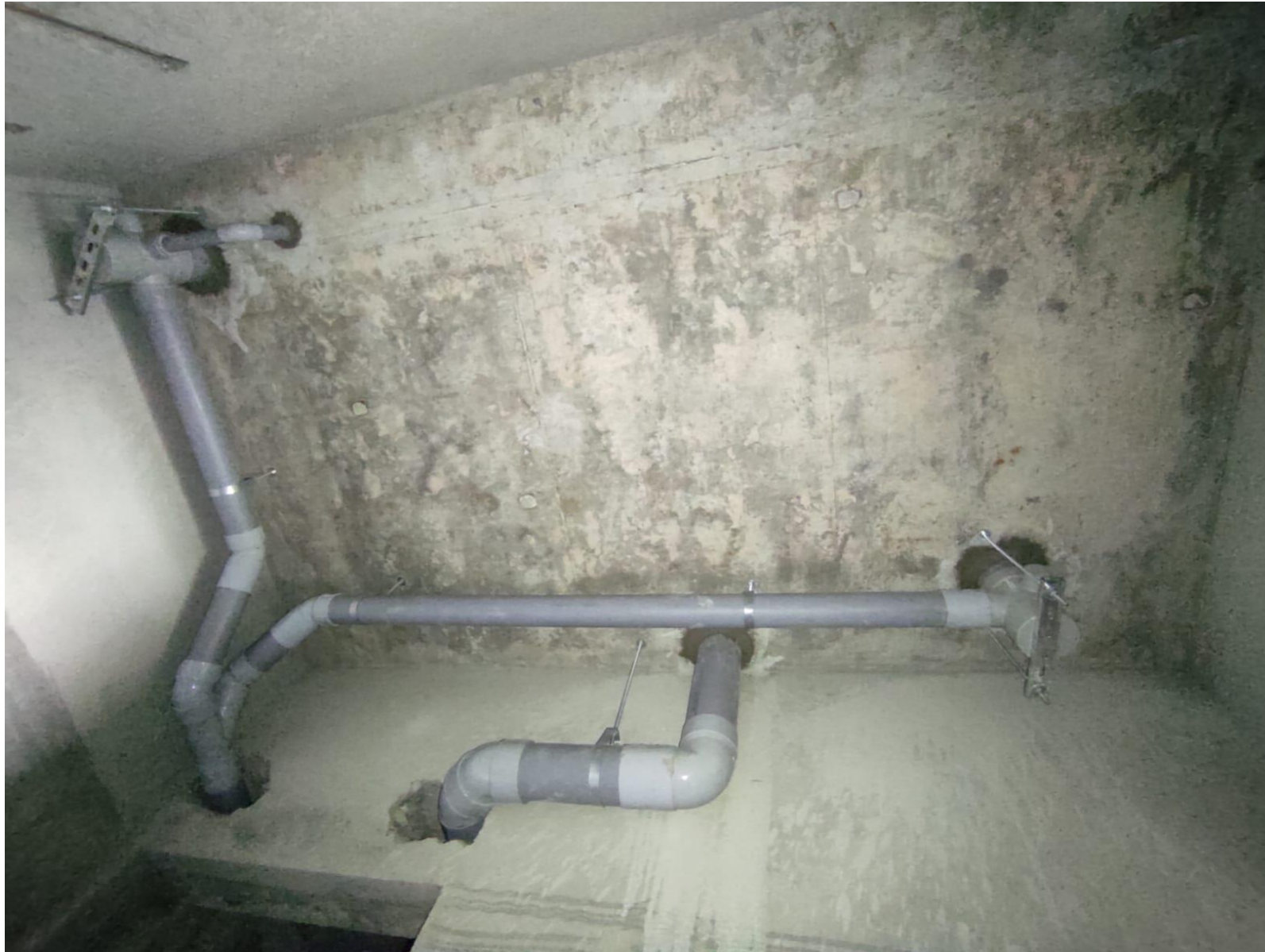
Plumbing – Seventh Floor Suspended Line Work In Progress
