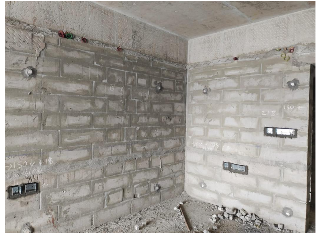
Electrical –Thirteenth Floor Electrical Wall Chasing Work In Progress
