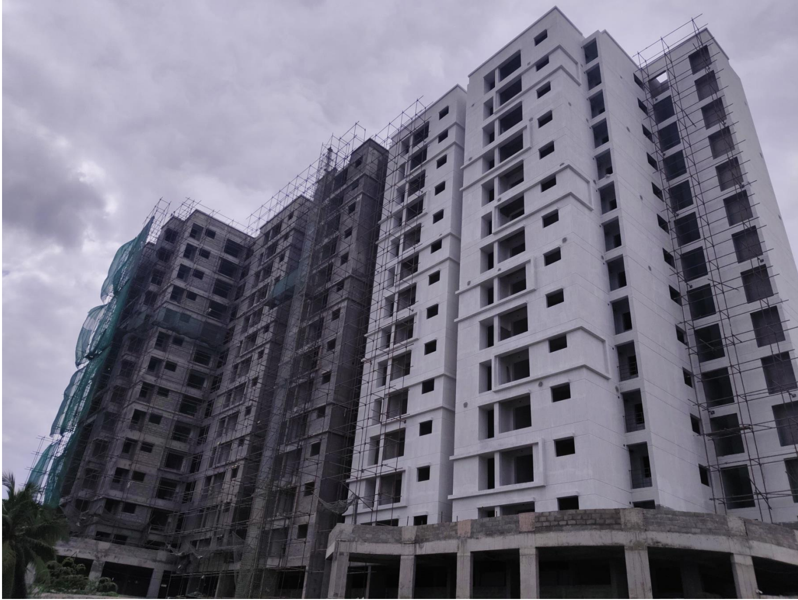
External Texture – South Side Primer Work In Progress
