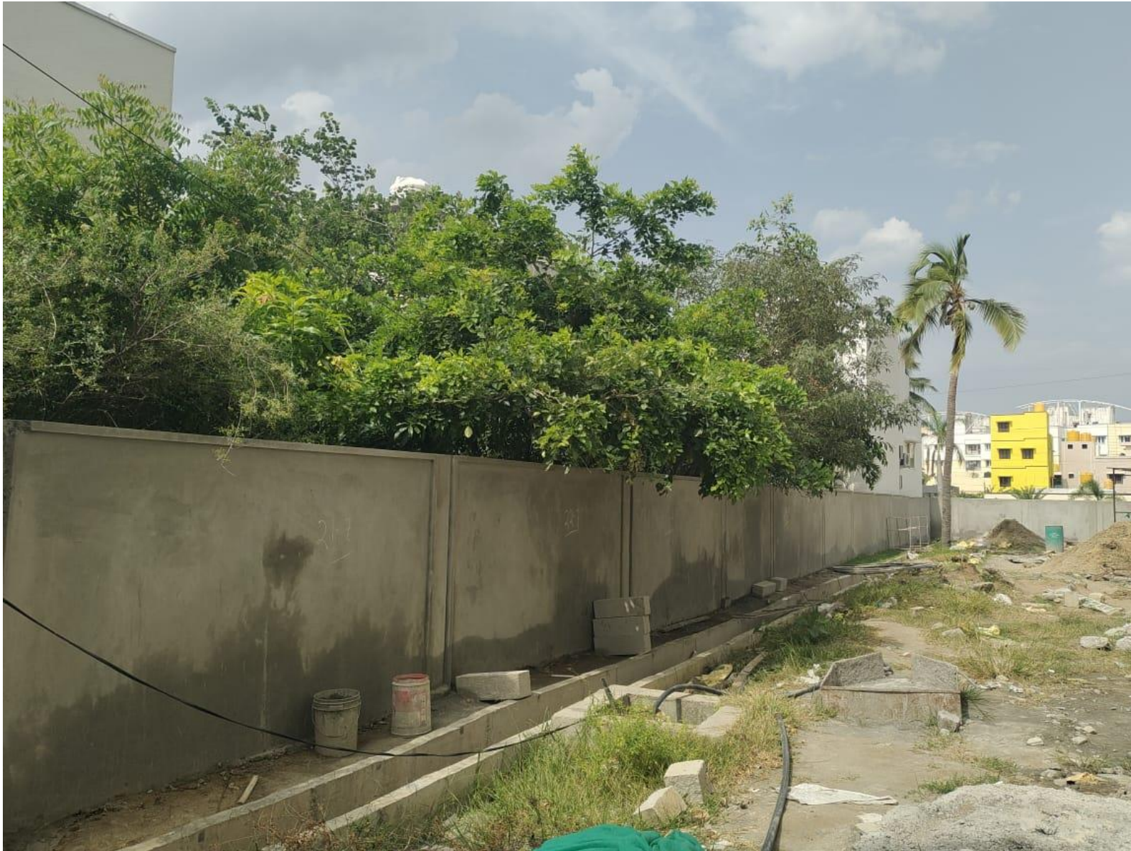
Compound wall Plastering – North & East Side Work In Progress
