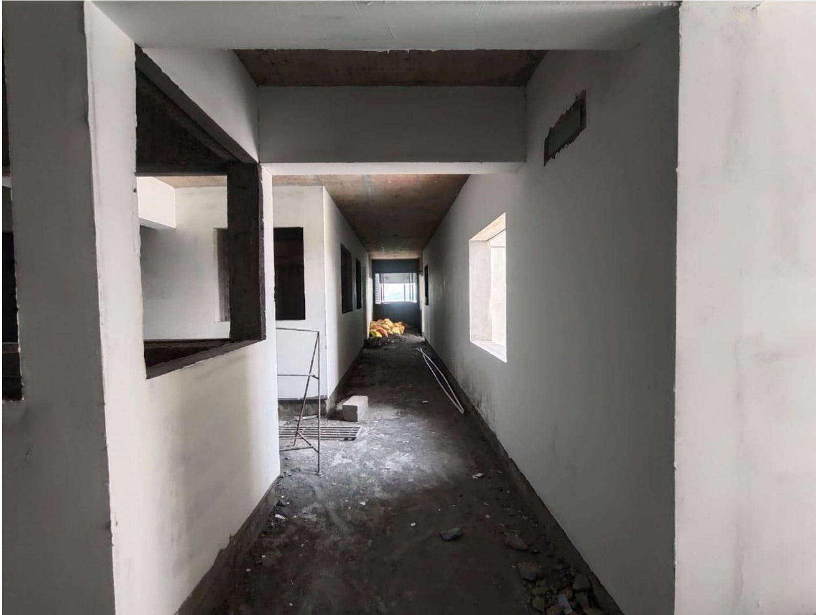
Corridor – 1 st Coat Putty Work In Progress
