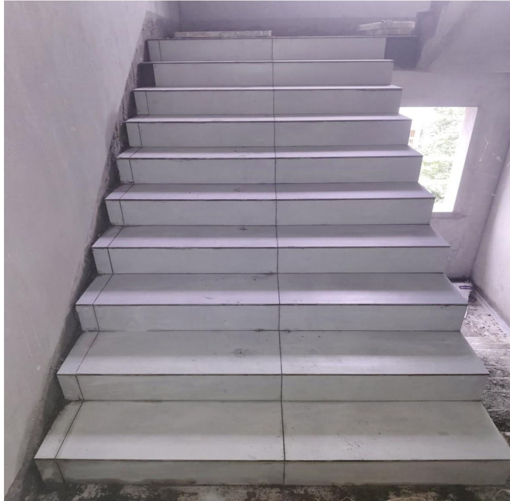
Staircase Tiles Work In Progress
