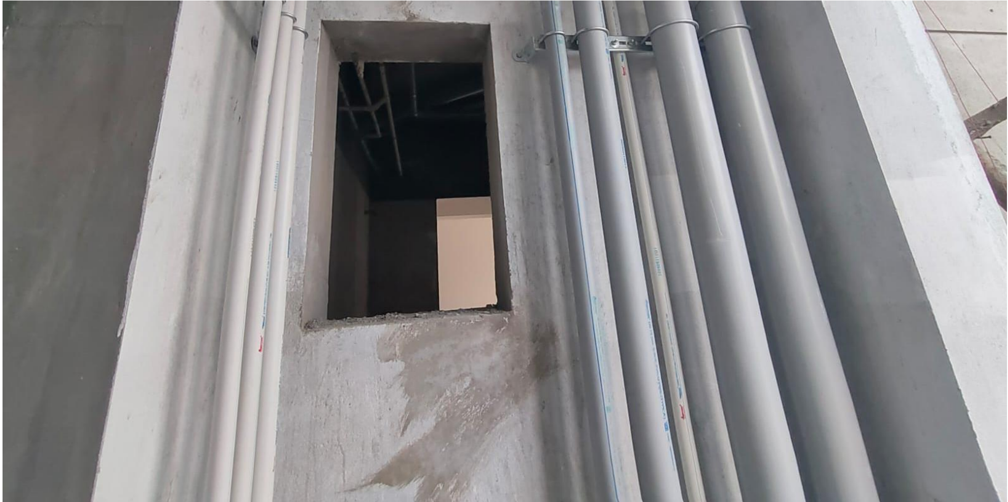
Plumbing – External Vertical Shaft clamp Fixing Work In Progress
