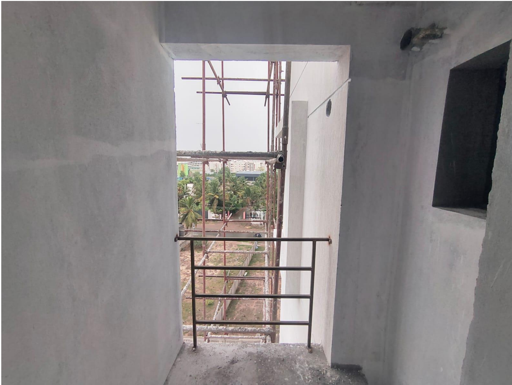
Plumbing Shaft – Primer Work In Progress
