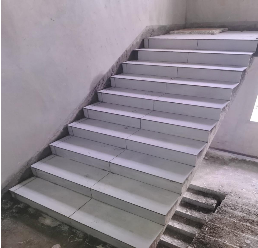
Staircase Tiles Work In Progress
