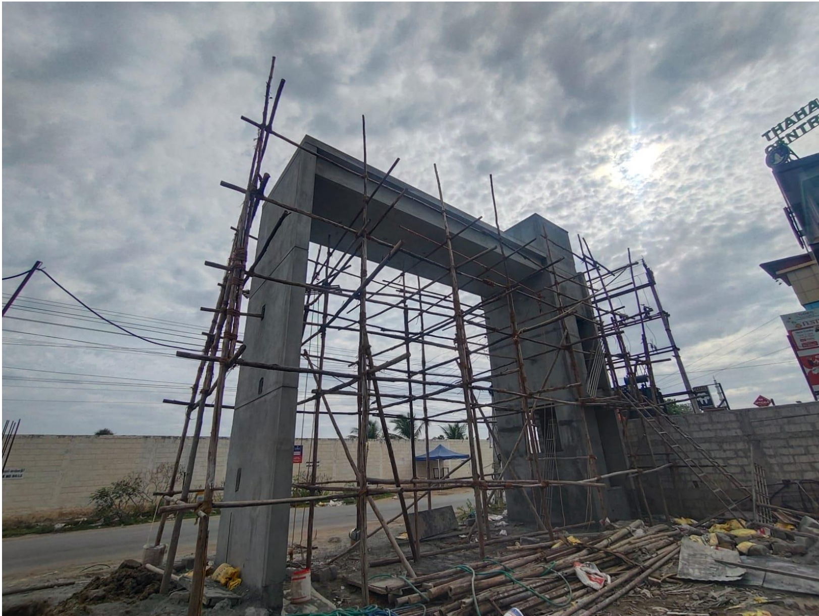
Entry Entrance Arch- Plastering Work In Progress
