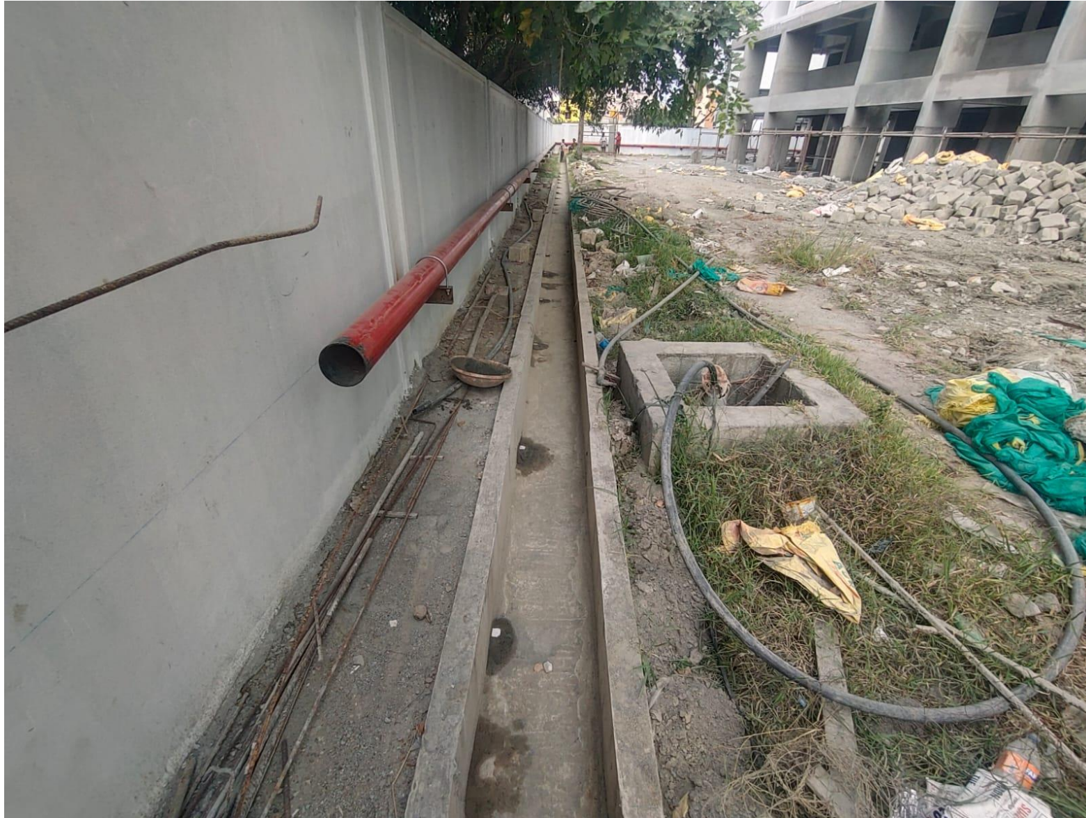
External Fire Fighting – Hydrant Line Fixing Work In Progress
