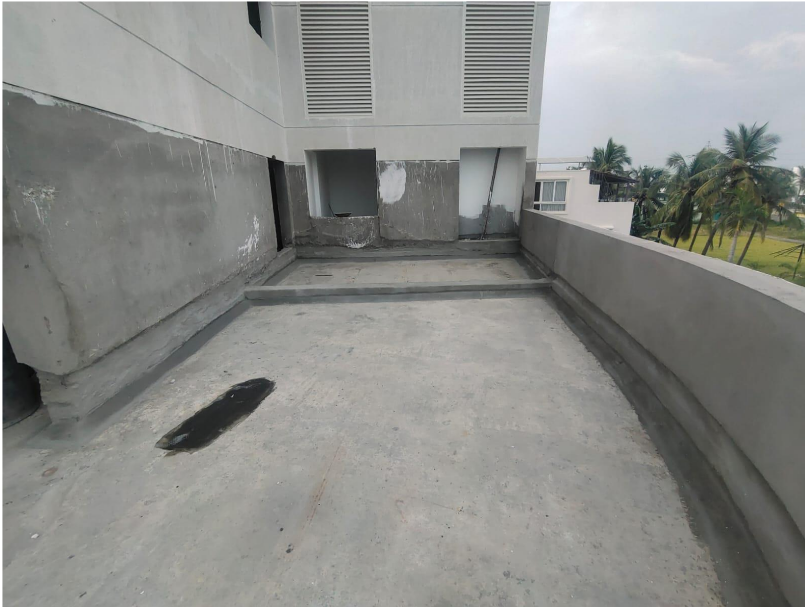
Private Terrace – Waterproofing Work In Progress
