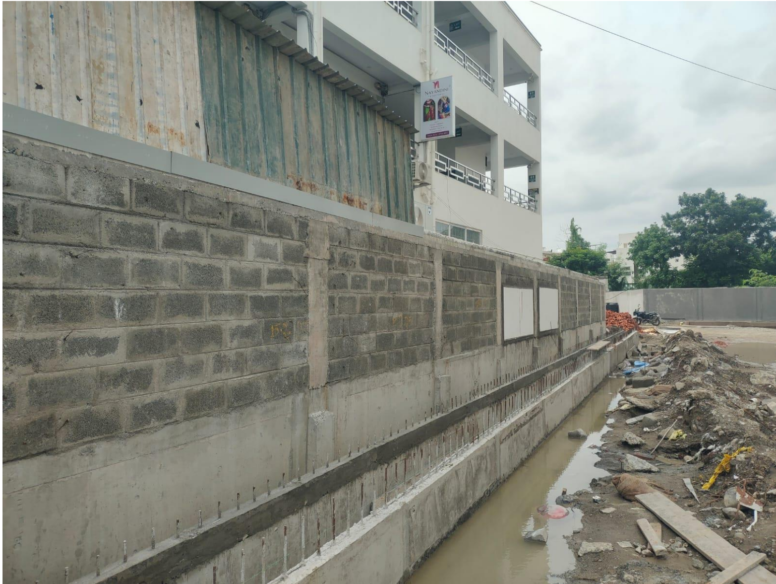
Storm Water Trench – West Side Wall Completed
