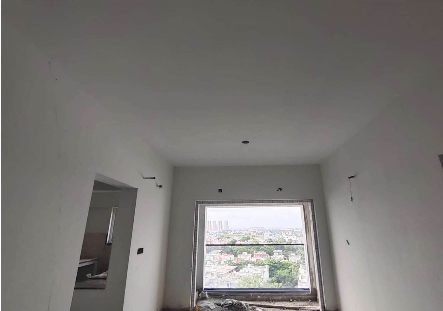
Seventh Floor – Primer Work In Progress
