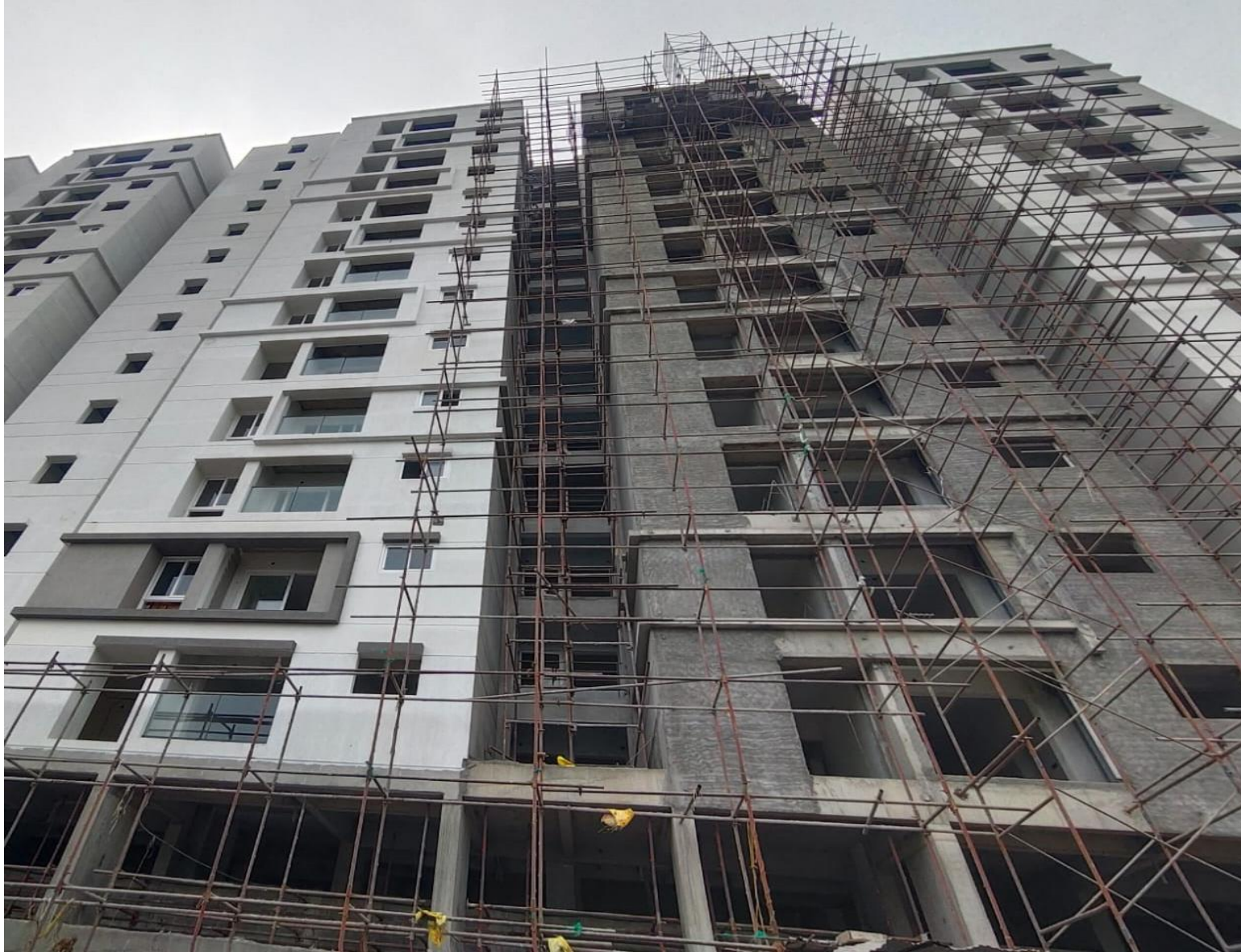
External Plastering – North Side Work In Progress
