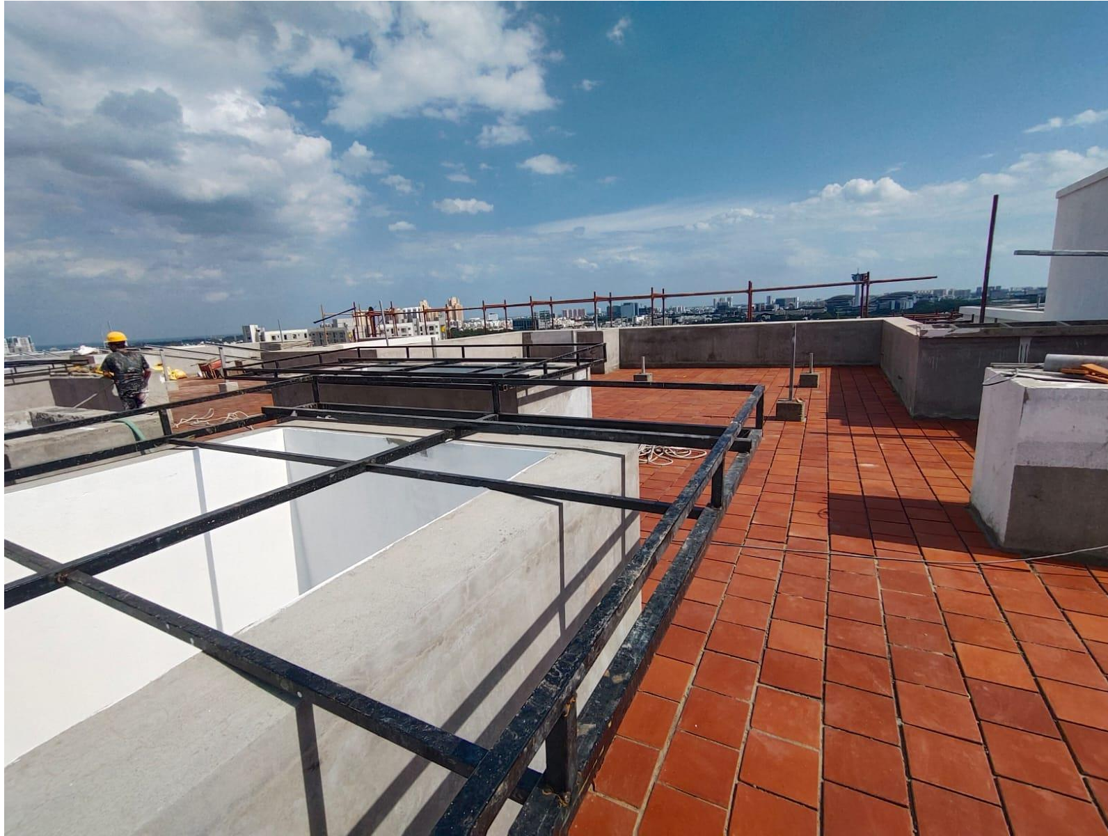
OTS Covering – Fabrication Work In Progress
