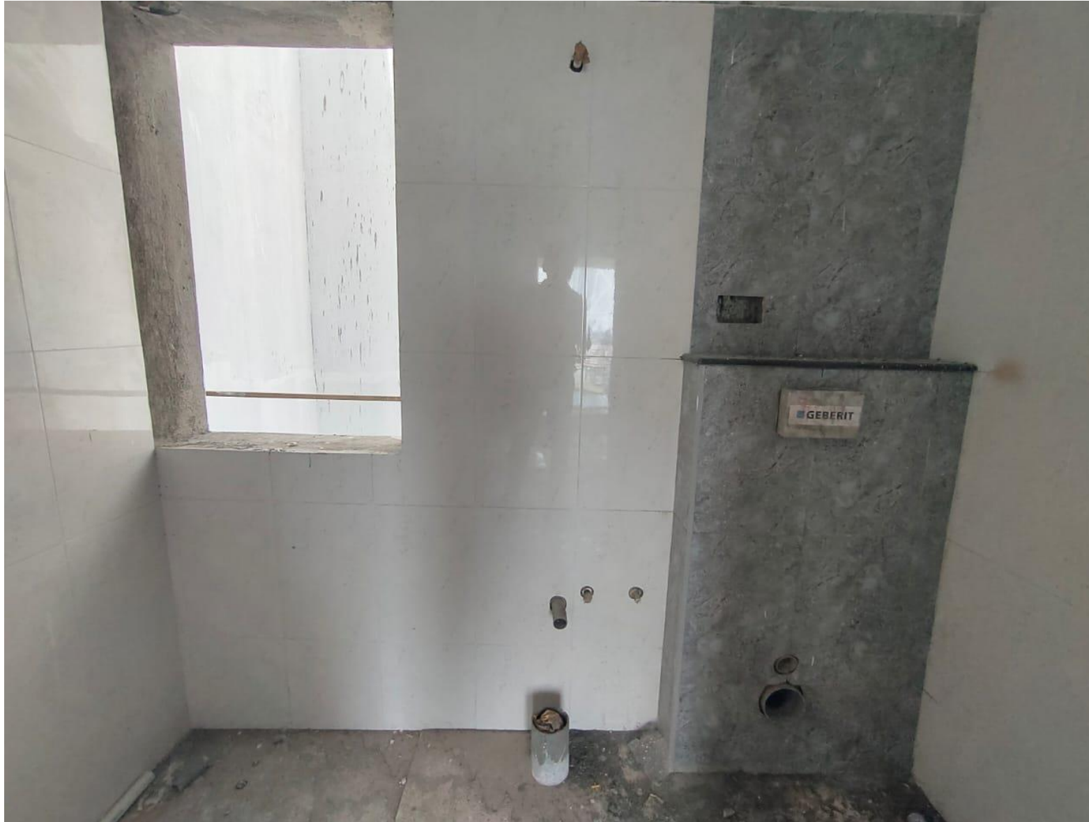
Wall Tiles – Thirteenth Floor Work Completed
