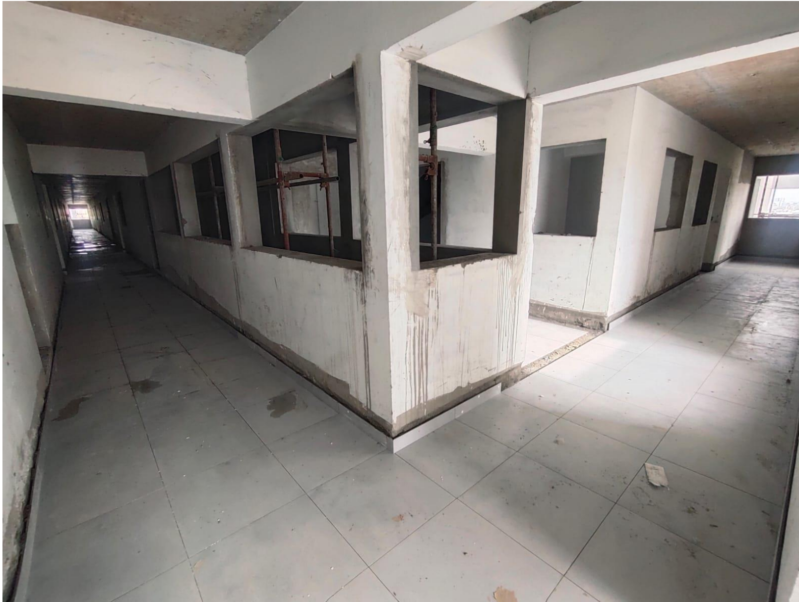
Corridor Tiles – Seventh Floor Work In Progress
