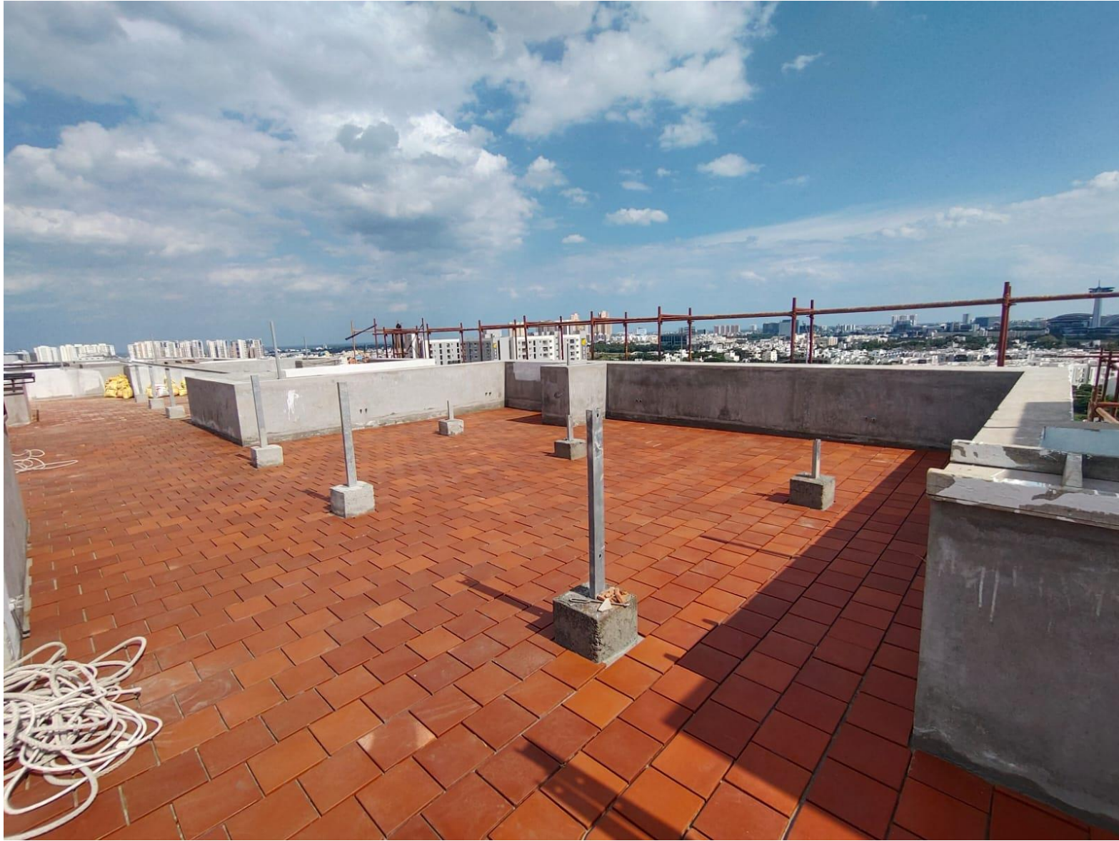
Terrace – Press Tiles Laying Work In Progress
