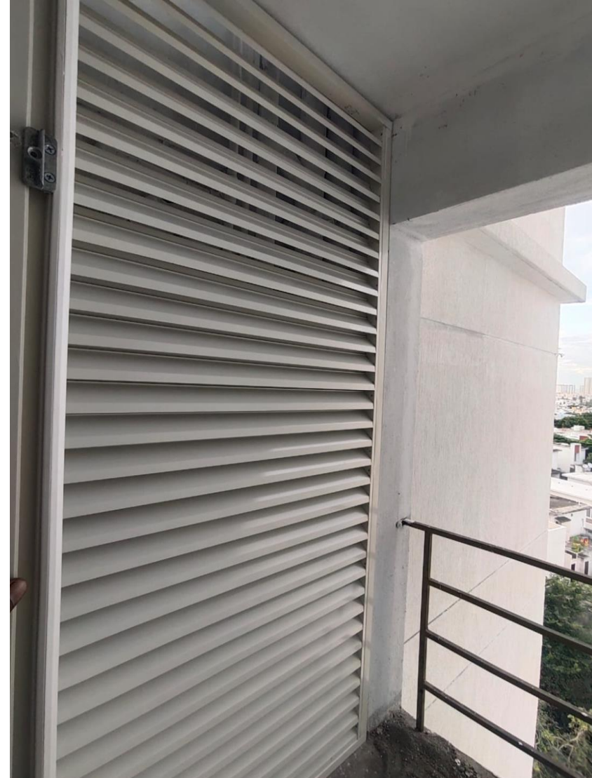
Shaft Louver – Fixing Work In Progress
