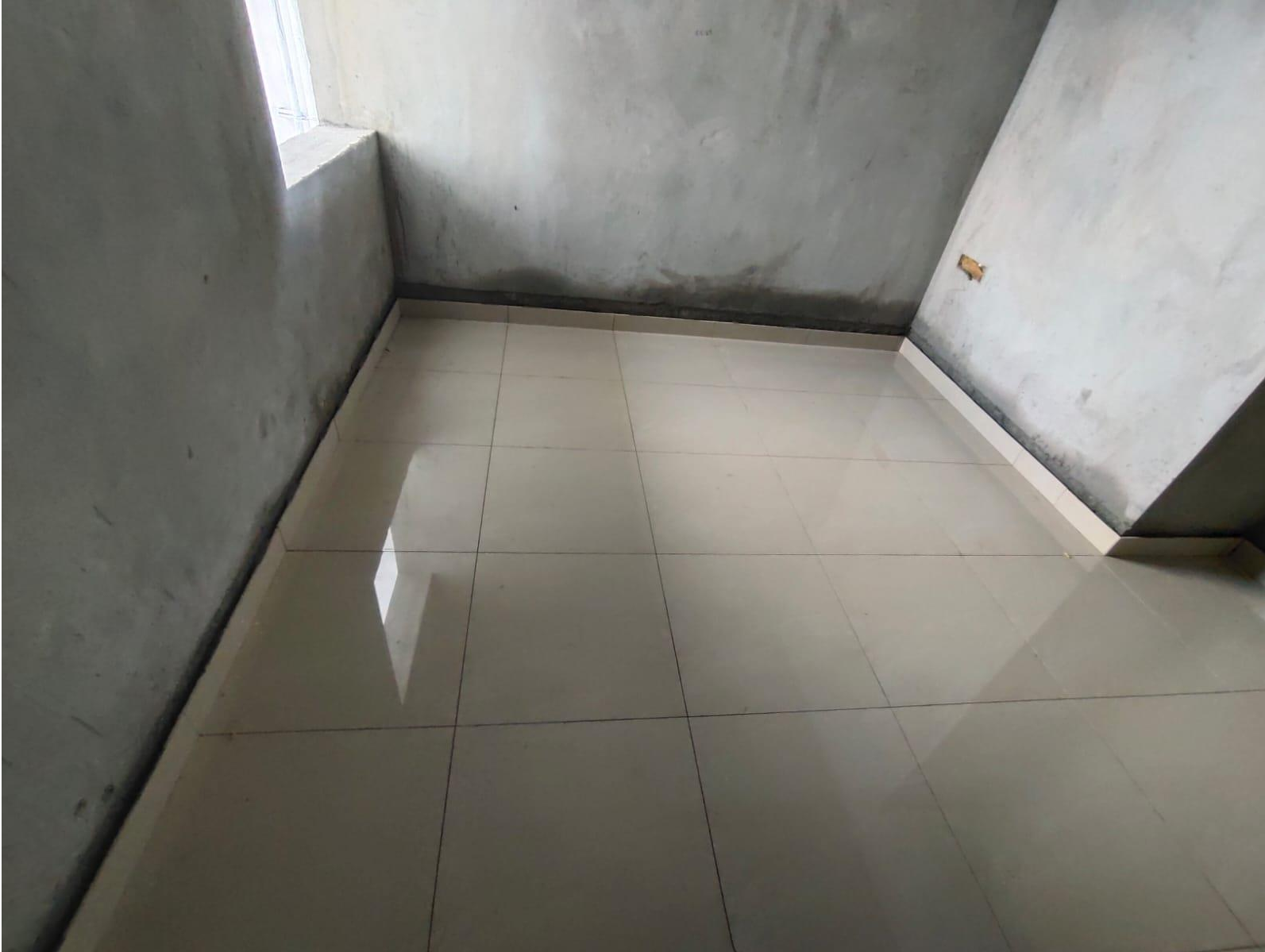
Flooring Tiles – Thirteenth Floor Work Completed
