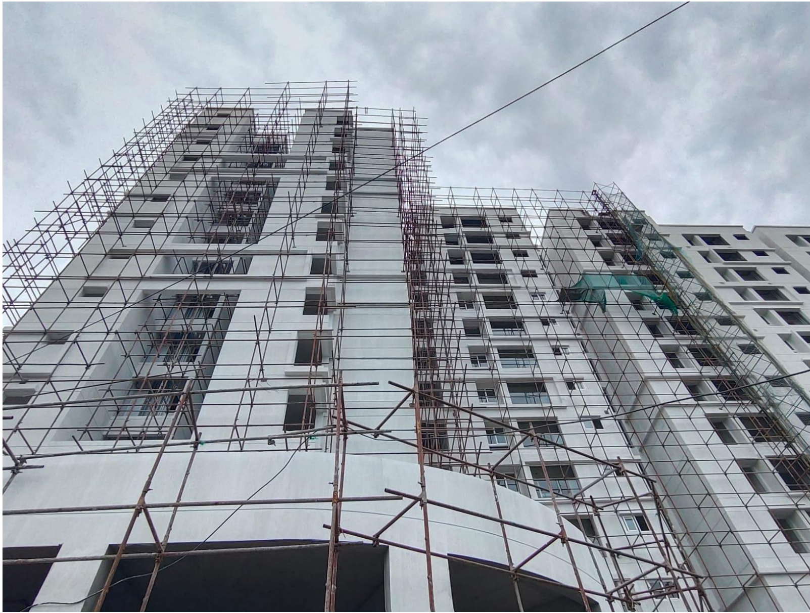
External Texture – South Side Work Completed
