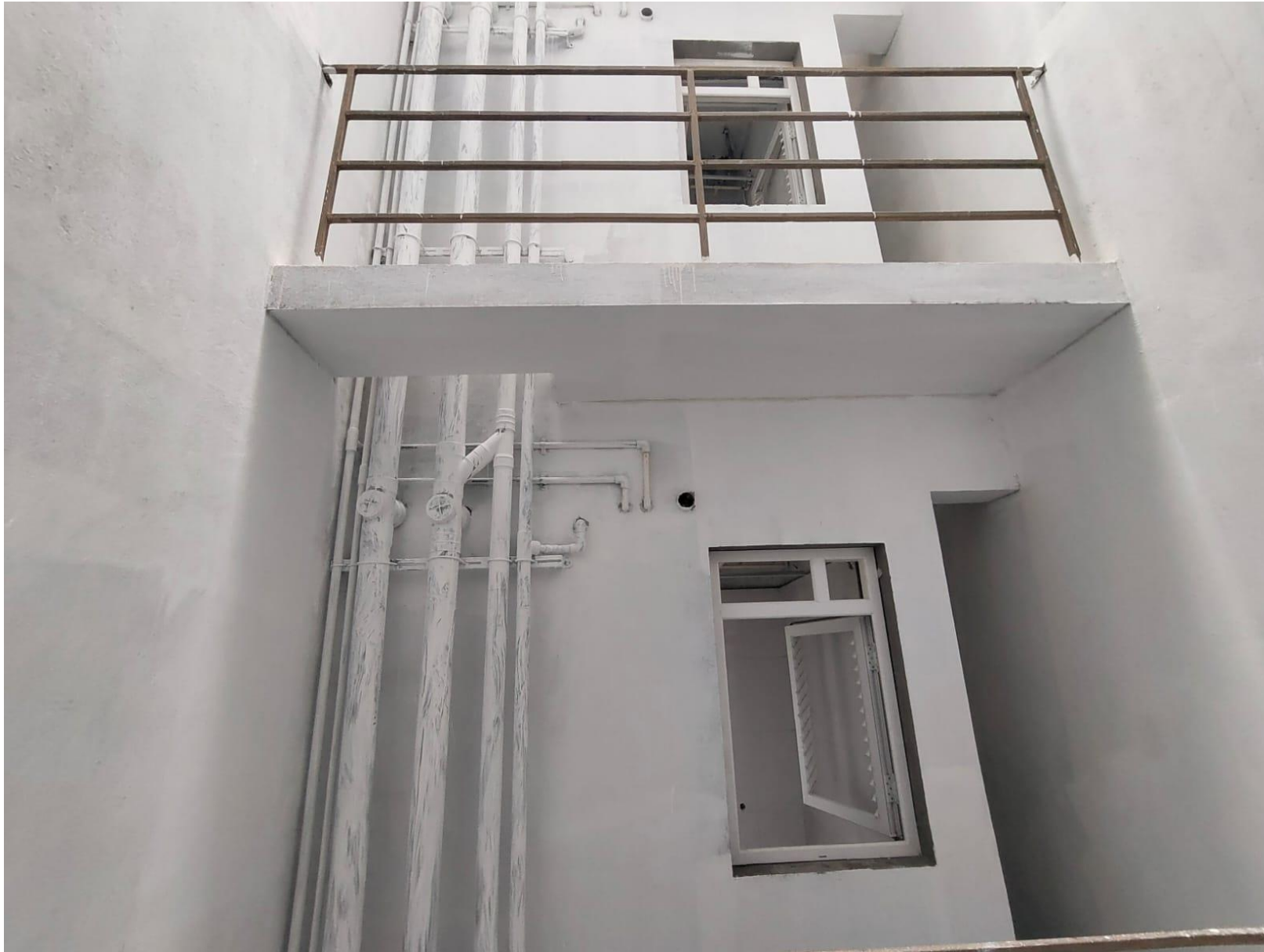
OTS & Shaft - Painting Work In Progress
