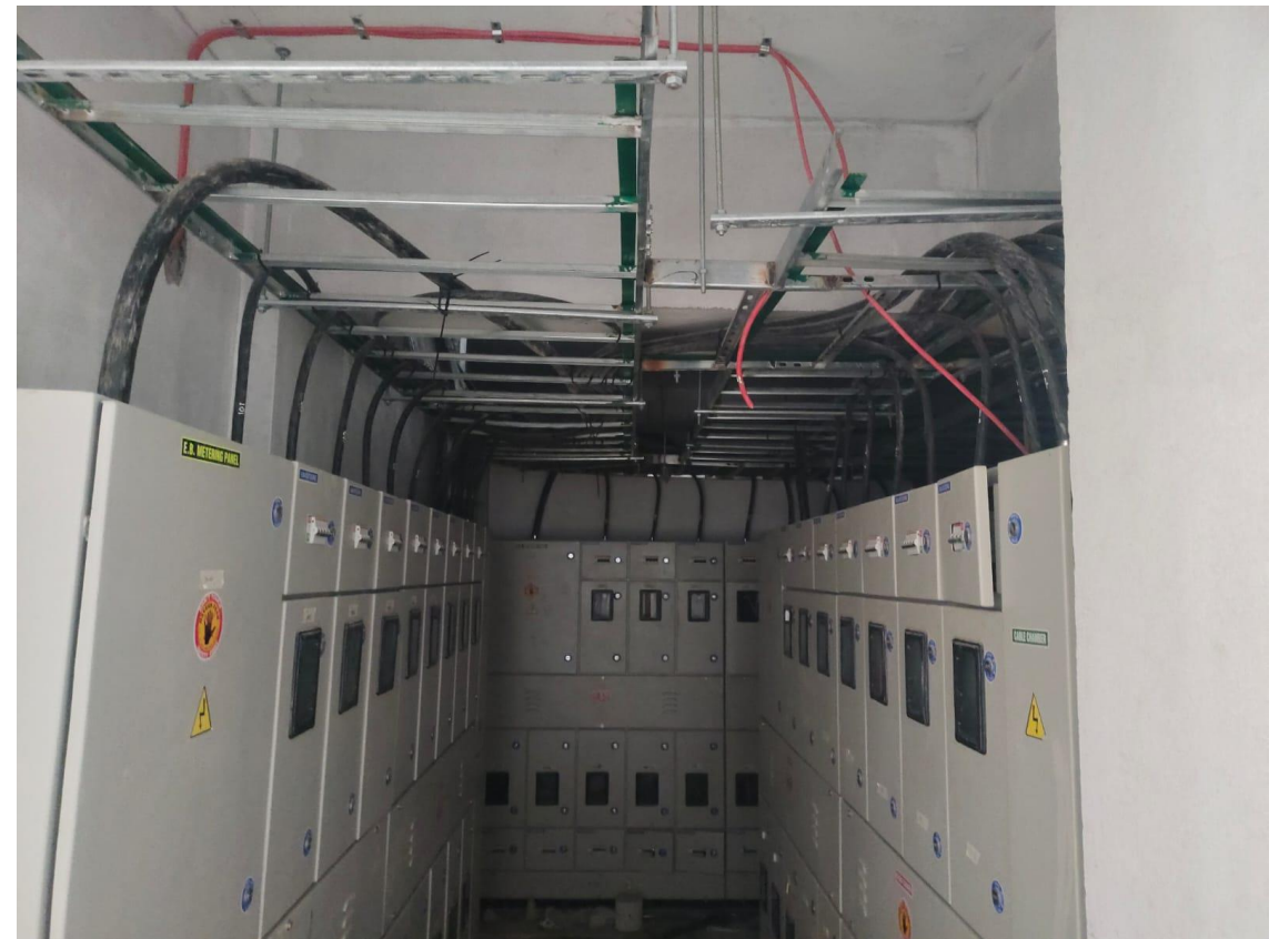
ELECTRICAL – PANEL ROOM1 & 2 CABLE GLAND WORK IN PROGRESS
