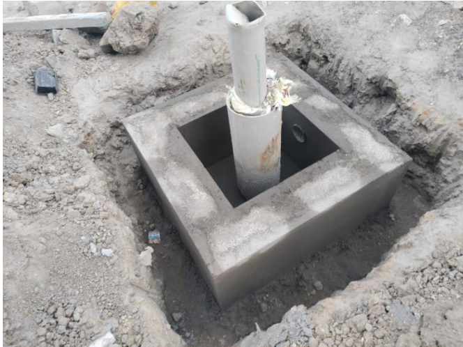
EXTERNAL - BOREWELL CHAMBER WORK IN PROGRESS
