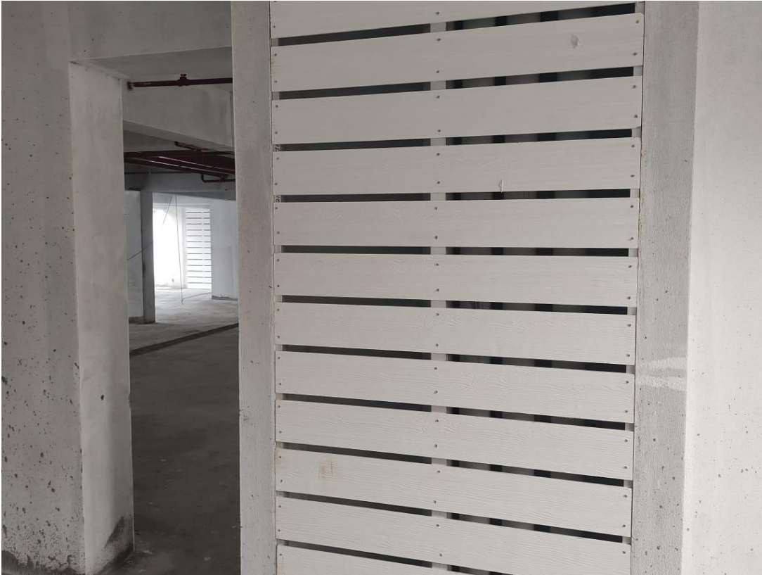
STILT FLOOR SHERA PLANK FIXING WORK IN PROGRESS
