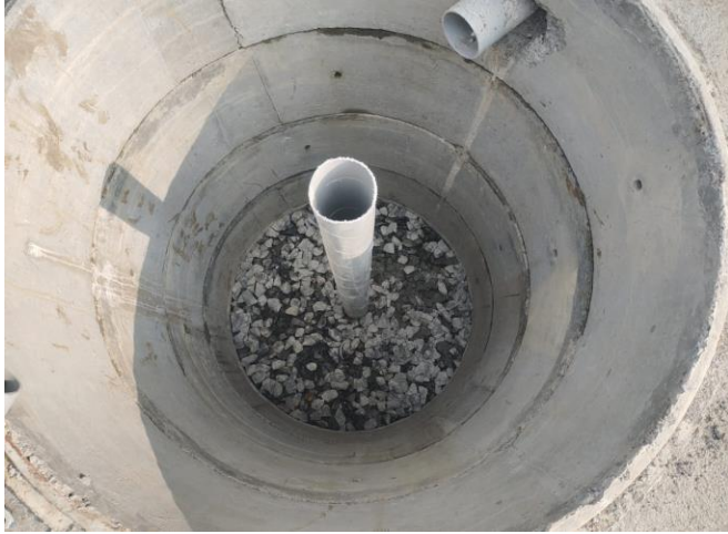
EXTERNAL – RAINWATER CHAMBER COVER FIXING WORK IN PROGRESS
