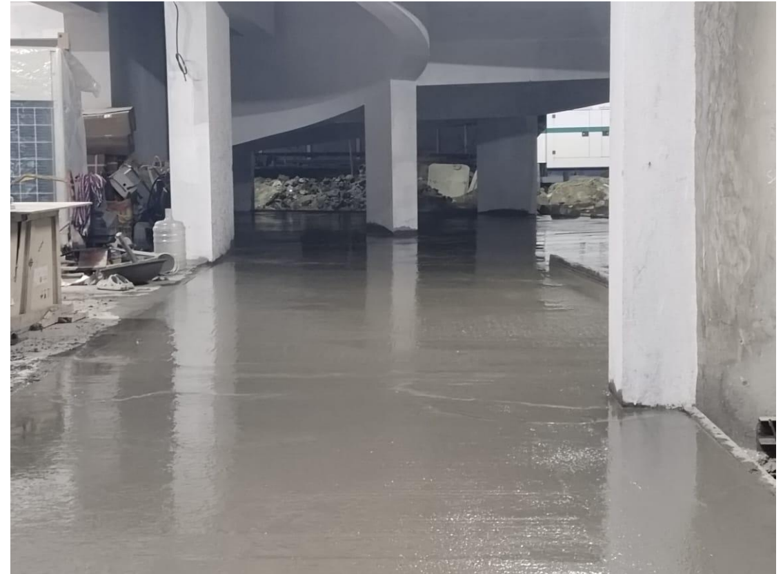
STILT FLOOR SCREED CONCRETE WORK COMPLETED
